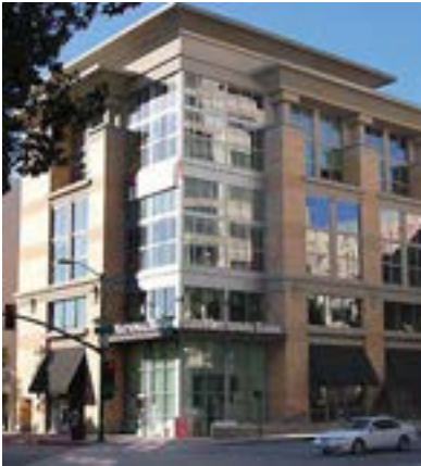
Durable masonry used at the ground level, accent at the main entry and corner, and a continuous architectural accent at the roof line (5D).
