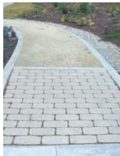
Example of a permeable walkway constructed of pavers and decomposed granite.
