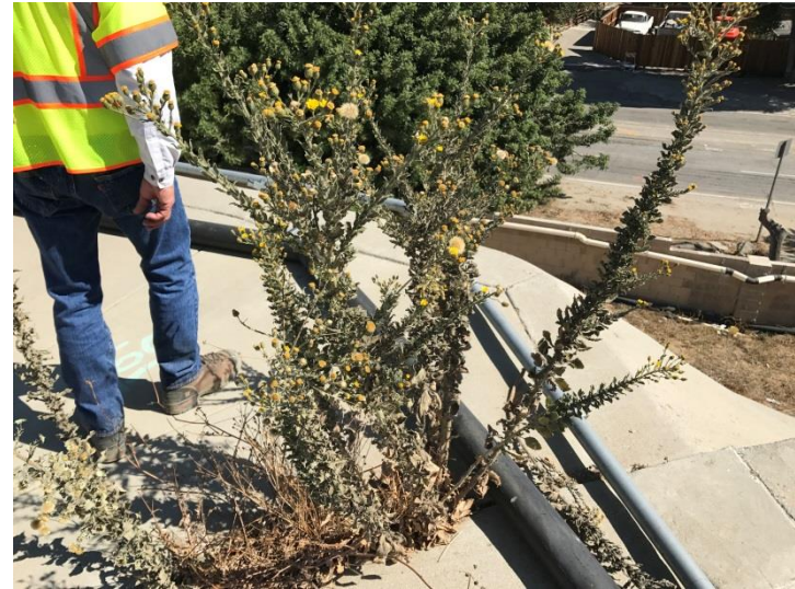
Photo 210: Vegetation Growing Out of Terminal Basin Concrete: September 27, 2016
