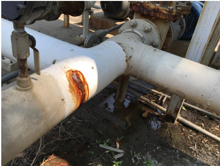
Photo 217: Potable Water Piping Leaks: August 24, 2016
