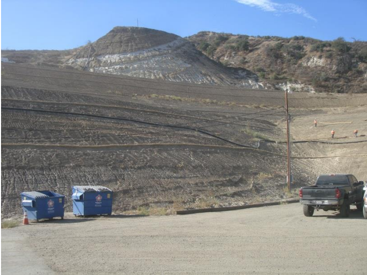
Photo 343: Graded and Storm Protected Slopes Old City South: September 27, 2016
