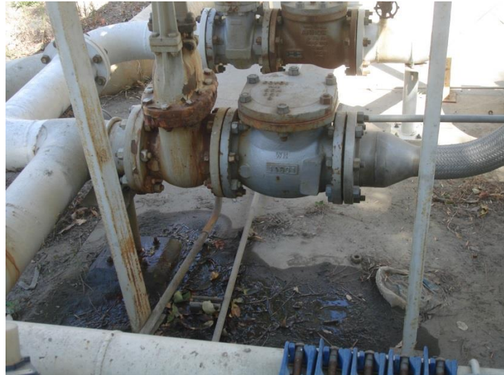
Photo 220: Potable Water Supply Piping Leak: September 27, 2016
