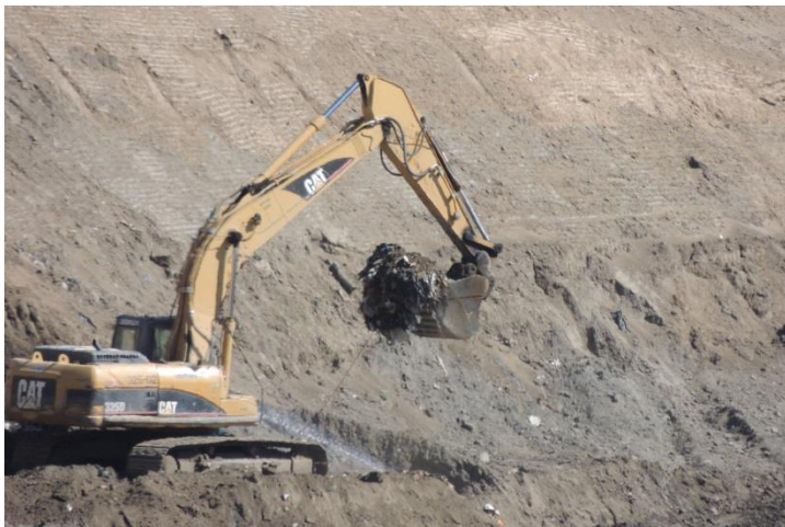
Photo 263: Uncovering Edge of Liner for Cell CC4A: September 14, 2016
