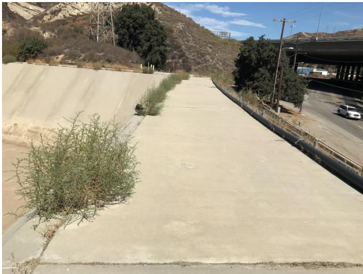
Photo 211: Vegetation Growing Out of Terminal Basin Concrete: September 27, 2016
