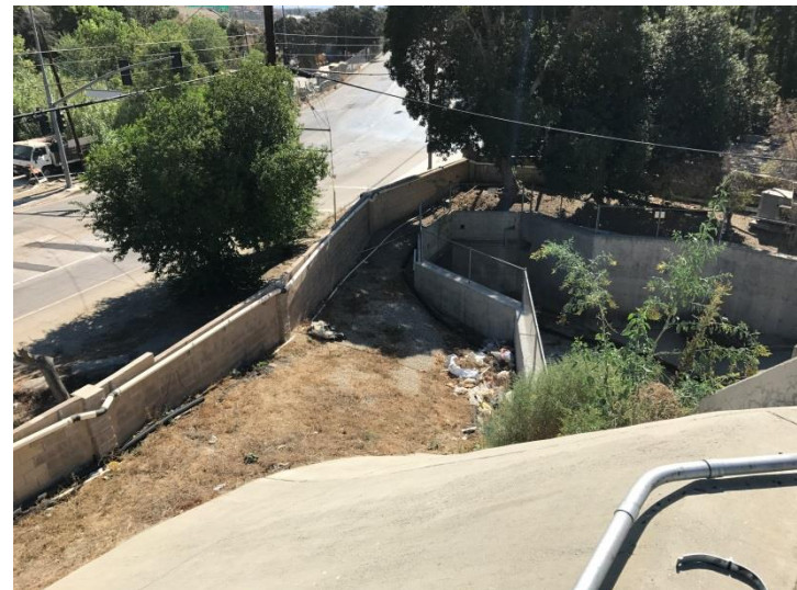
Photo 212: Vegetation Growing Out of Terminal Basin Concrete: September 27, 2016
