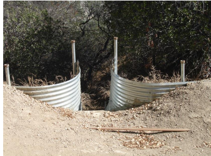
Photo 68: Edison Unprotected Drainage Hazard at pole 38: September 14, 2016
