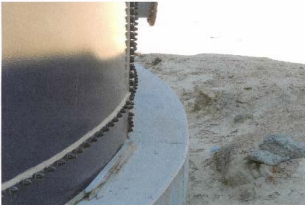
Photo 4: Ring foundation of water tank
