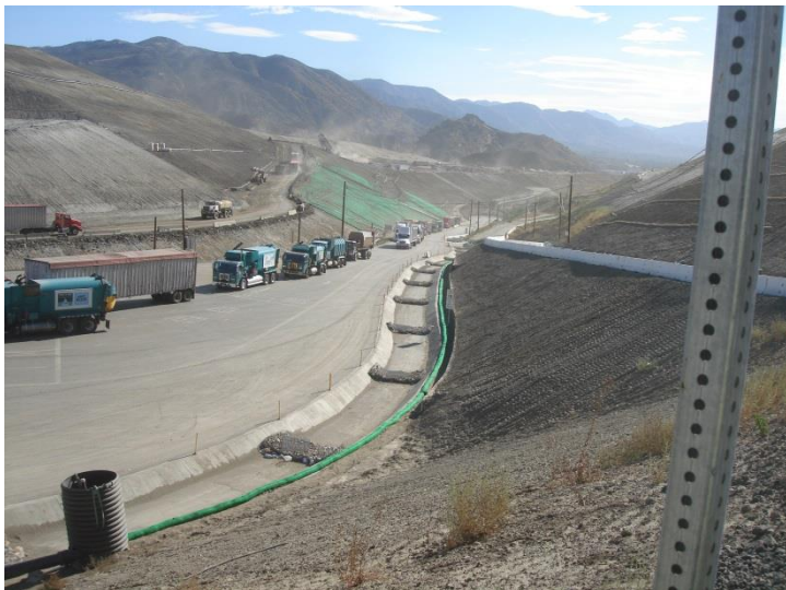
Photo 339: Graded and Storm Protected Slopes Old City South: September 27, 2016
