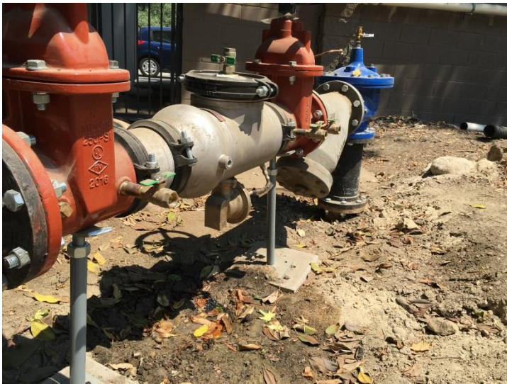
Photo 219: Potable Water Piping Leaks: August 24, 2016
