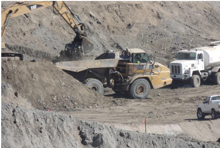
Photo 265: Uncovering Edge of Liner for Cell CC4A: September 14, 2016
