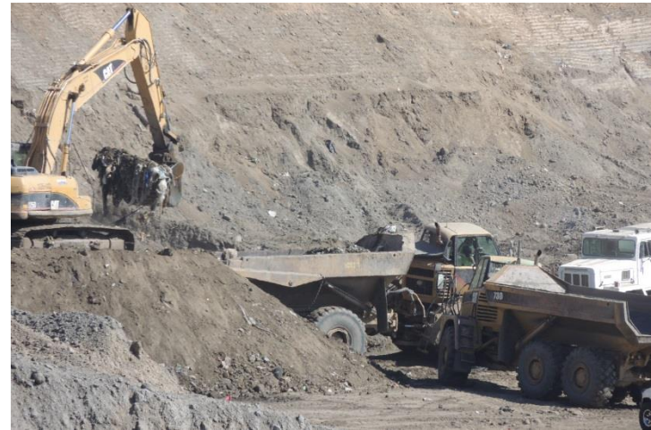
Photo 266: Uncovering Edge of Liner for Cell CC4A: September 14, 2016
