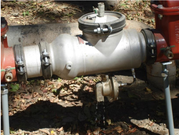
Photo 221: Potable Water Supply Piping Leak: September 27, 2016
