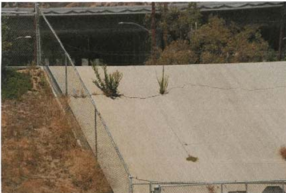
Photo 6: Vegetation in cracks on outside wall of the Terminal Basin
