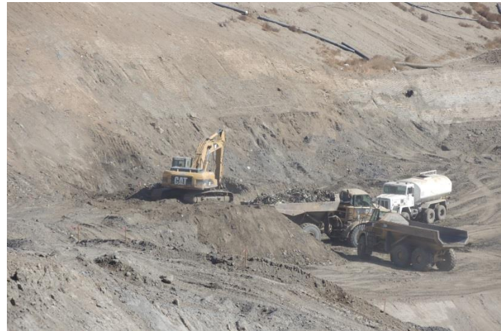
Photo 268: Uncovering Edge of Liner for Cell CC4A: September 14, 2016
