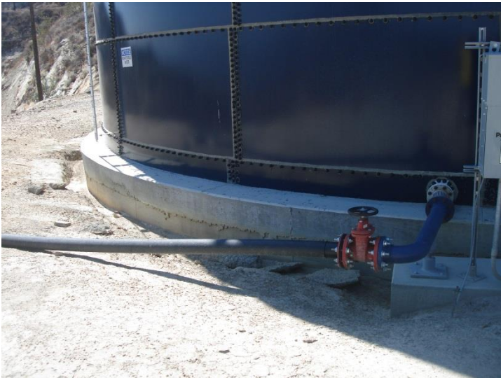
Photo 227: Deck A Water Tank Foundation Not Backfilled: September 14, 2016
