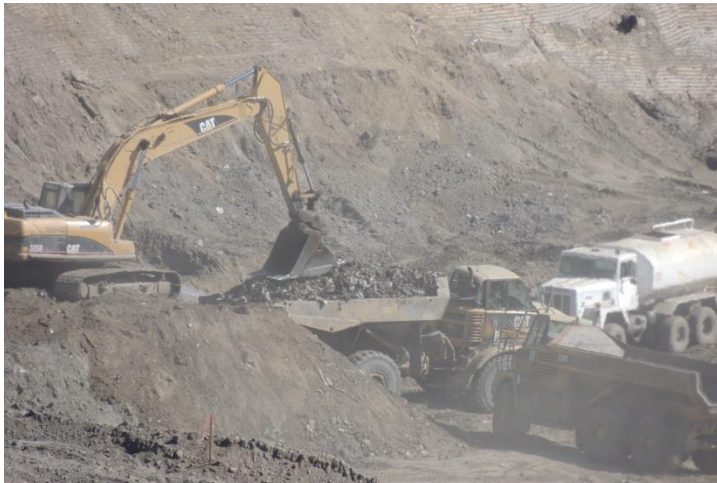
Photo 269: Uncovering Edge of Liner for Cell CC4A: September 14, 2016
