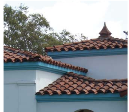
When planning a re-roof attention should be paid to how tiles are stacked, how ridges are adorned and to any other decorative features that exist.
