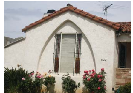
This window has been replaced with an ill-fitted window that diminishes the historic integrity of the house.
