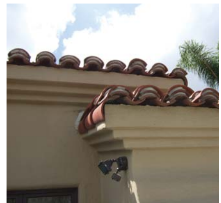
A close-up of a clay tile roof edge is shown. Birdstops are not used, nor is extensive metal flashing.
