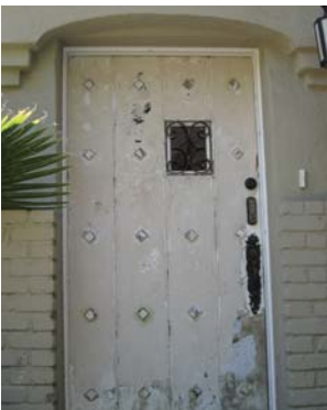
This door with its original hardware and decorative features should be repaired and refinished before replacement is considered.
