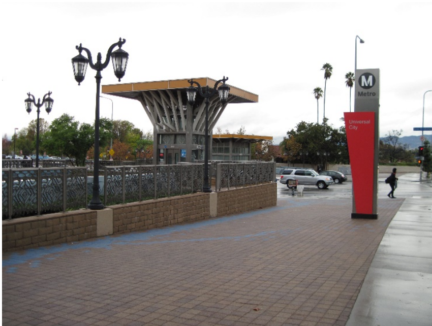
Figure 9 - Universal City/Studio City Metro Red Line Station Image Source: Wikimedia Commons - GTD Aquitaine
