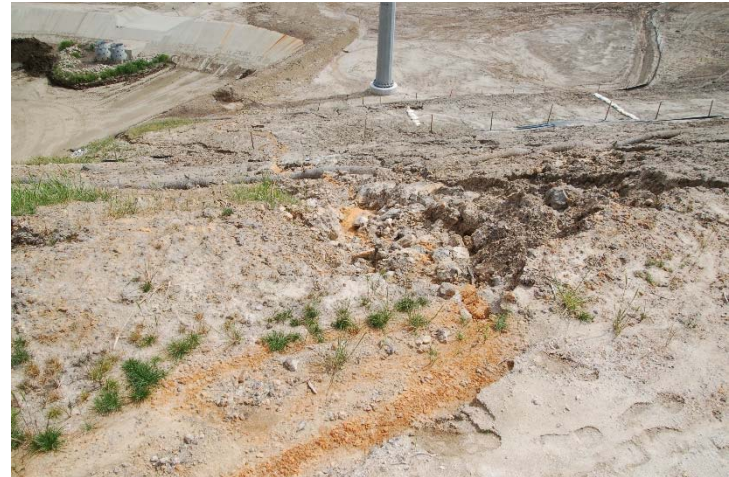
Photo 8: Slope Erosion near Basin A: April 18, 2017
