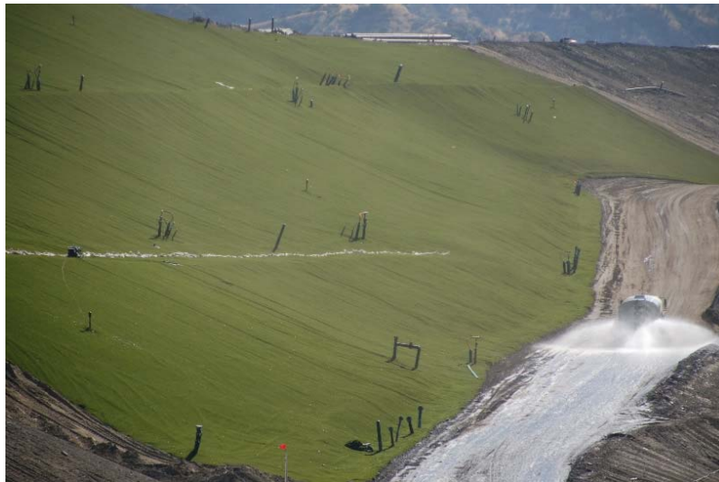
Photo 439: Closure Turf: June 20, 2017
