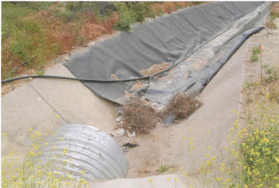
Photo 15: Geomembrane detached from headwall at drainage channel between Basin D and access road to Flare 9 and 10
