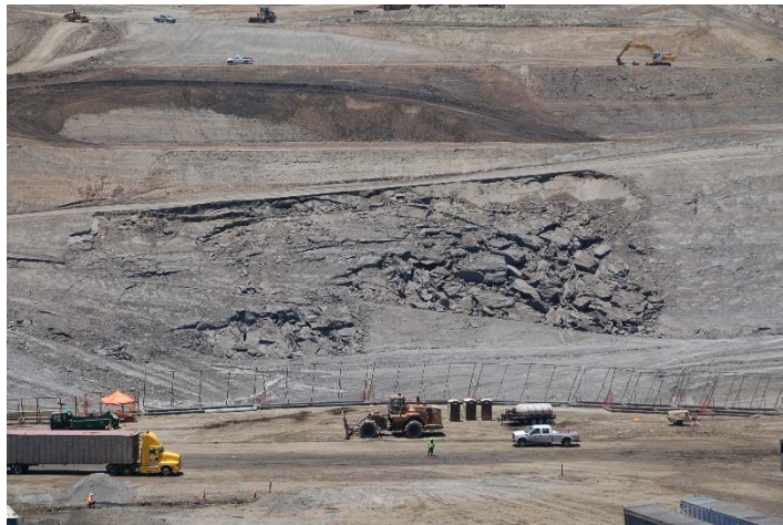
Photo 331: CC4A Part 2 Excavation Area Slide: June 20, 2017
