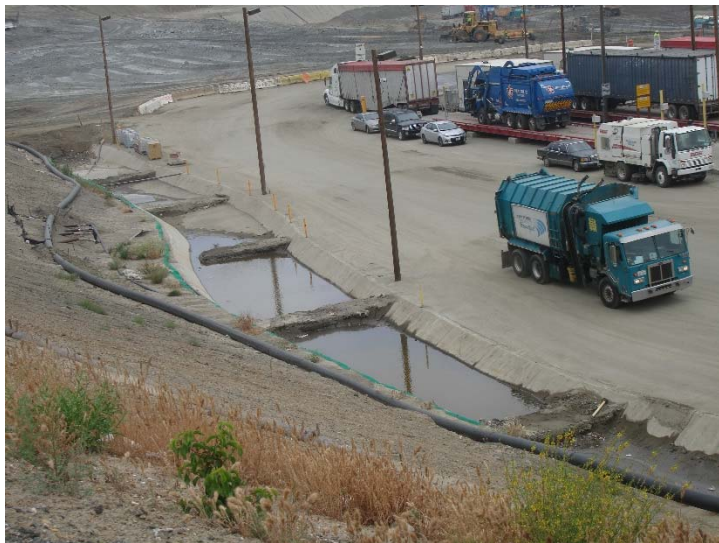
Photo 55: Westside Drainage Channel Gabions: May 9, 2017
