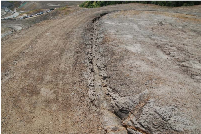
Photo 79: Flare 3 Access Road Erosion Ruts: April 18, 2017
