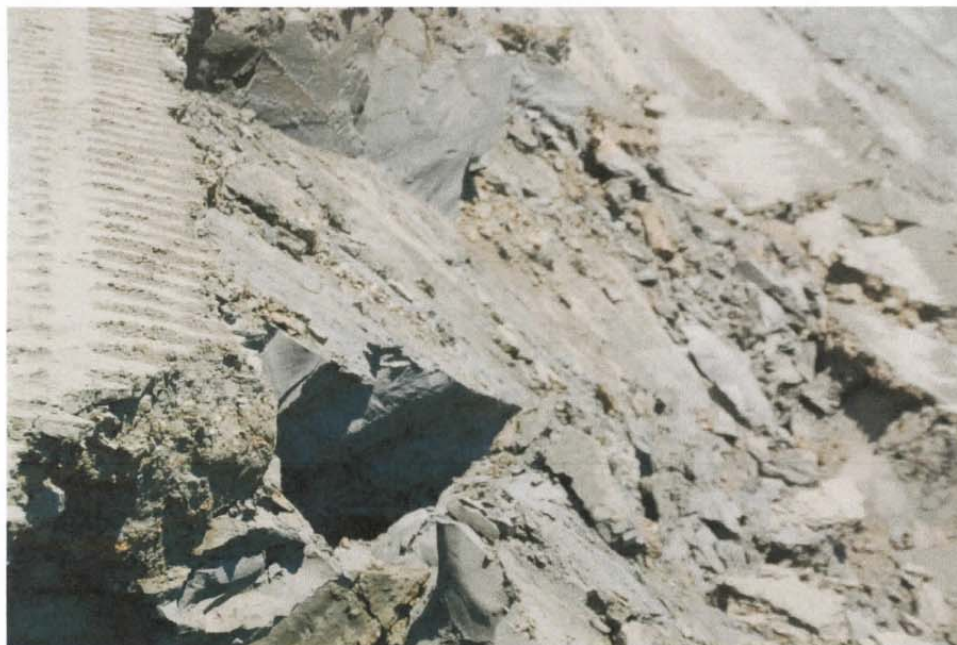
Photo 6: Plane of slickenslide in debris of excavation of Cell CC4
