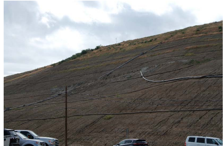
Photo 362: Stockpile Soils Slumps on Old City Area: April 18, 2017
