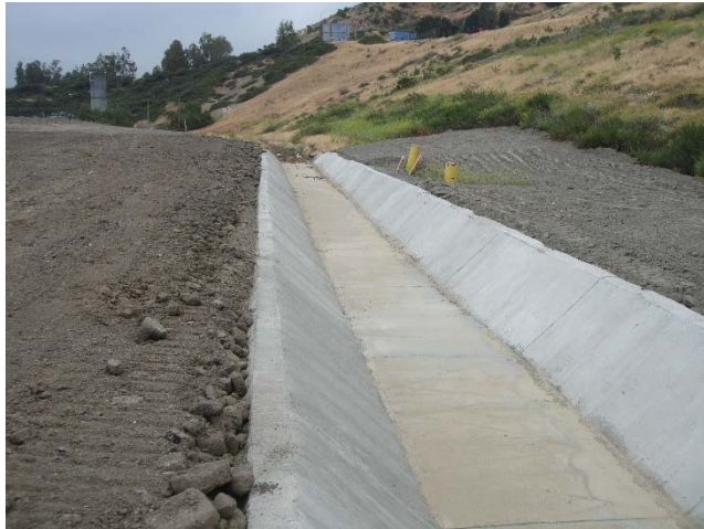
Photo 405: Deck B Drainage Channel Repair: May 9, 2017
