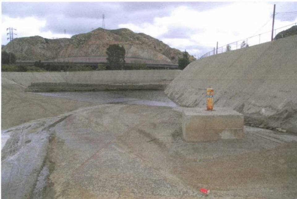
Photo 6: Sediments removed from front half of Terminal Basin
