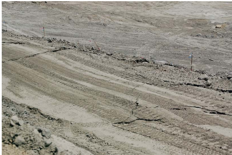
Photo 351: CC4A Part 2 Excavation Area Slide: June 20, 2017
