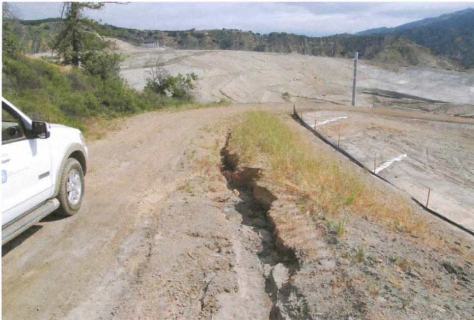
Photo 17: Excessive gullies along access road to Flare 3
