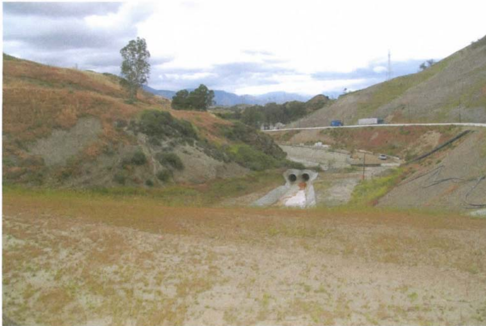
Photo 3: Graw growing on downstream face of temporary basin
