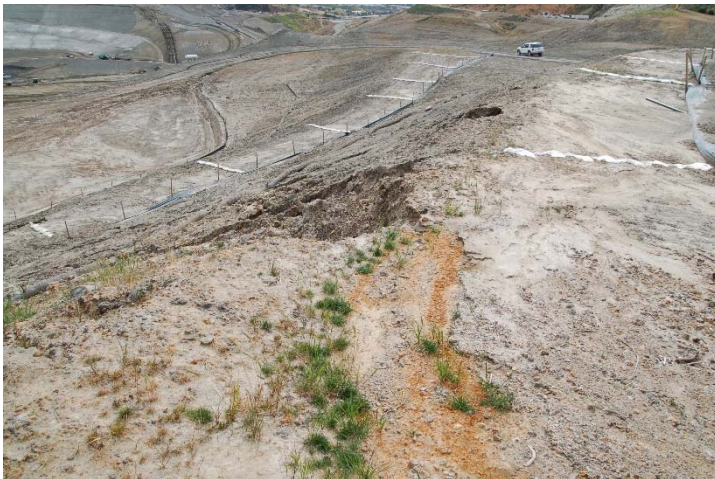
Photo 7: Slope Erosion near Basin A: April 18, 2017
