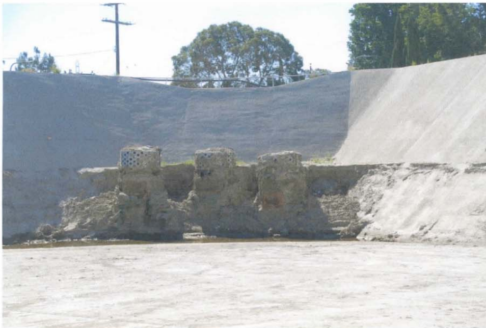
Photo 2: Sediments behind decant towers at Terminal Basin
