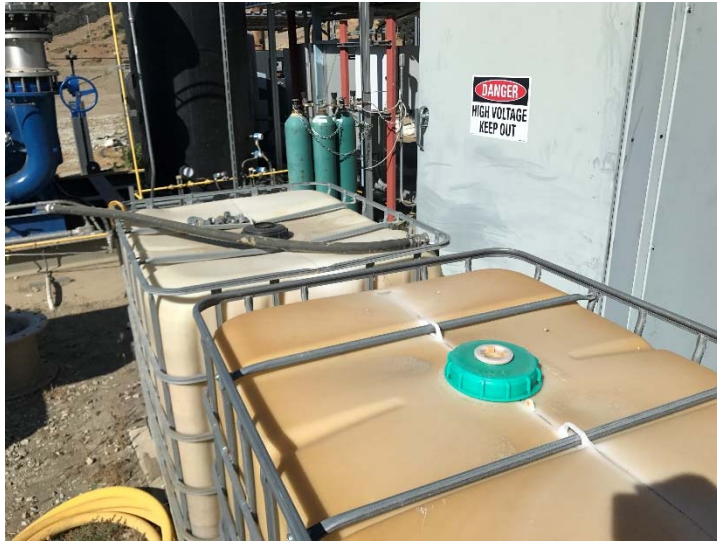
Photo 145: Flare 9 & 10 Blower Knockout Liquids: May 23, 2017
