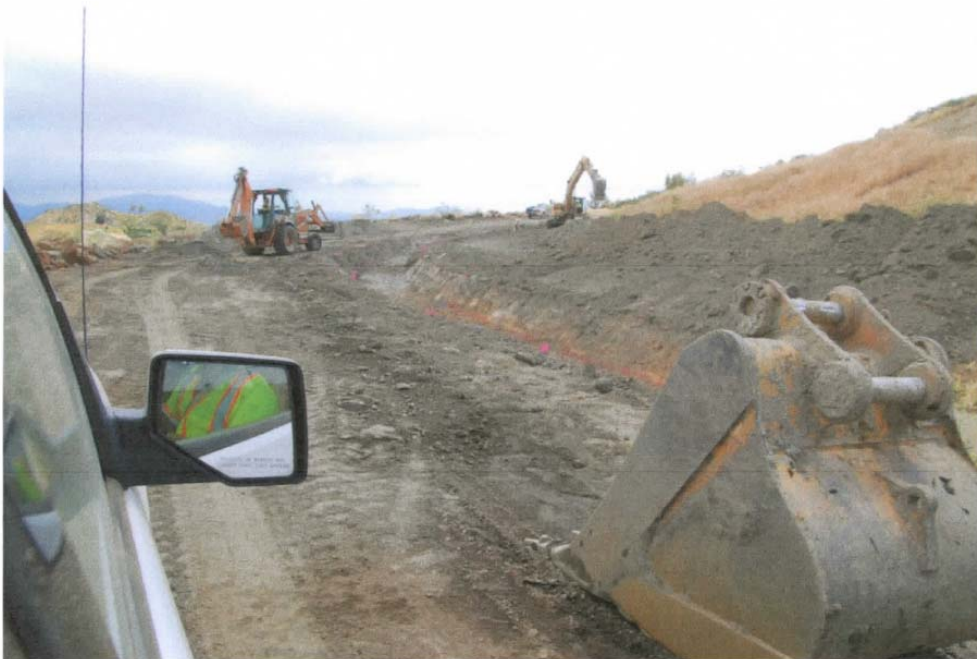
Photo 14: Repair of Channel on old city landfill deck
