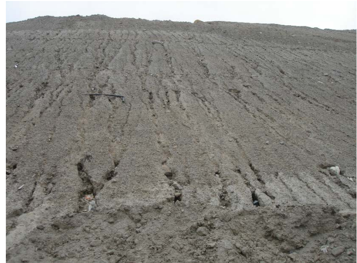
Photo 286: CC3A Soil Stockpile Erosion: May 9, 2017
