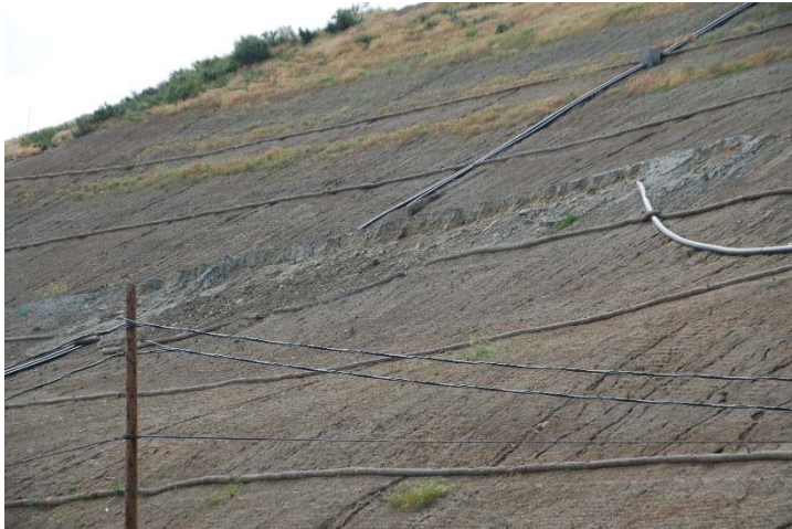
Photo 361: Stockpile Soils Slumps on Old City Area: April 18, 2017
