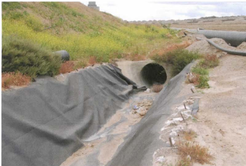
Photo 16: Geomembrane detached from headwall at drainage channel between Basin D and access road to Flare 9 and 10
