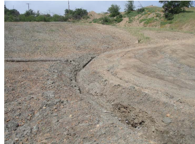
Photo 80: Flare 3 Access Road Erosion Ruts: April 18, 2017
