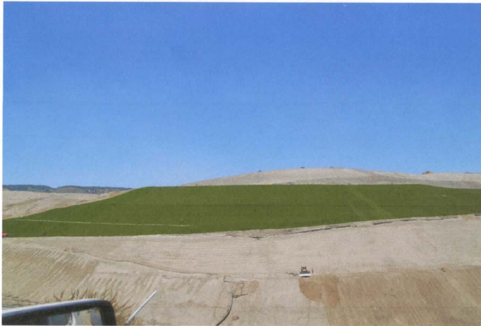
Photo 7: Overview of Closure Turf on Cell CC3 slope
