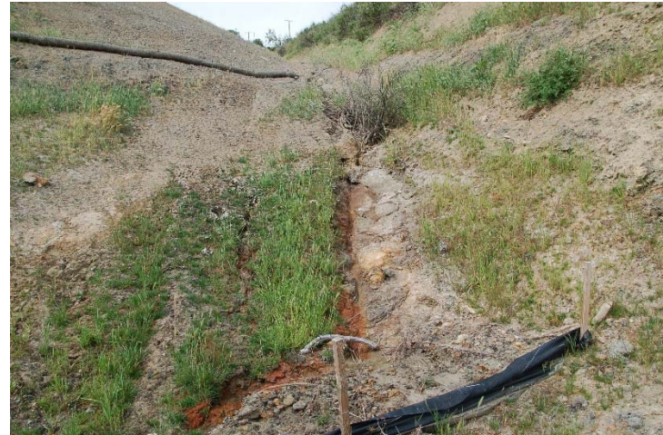
Photo 6: Slope Erosion near Basin A: April 18, 2017
