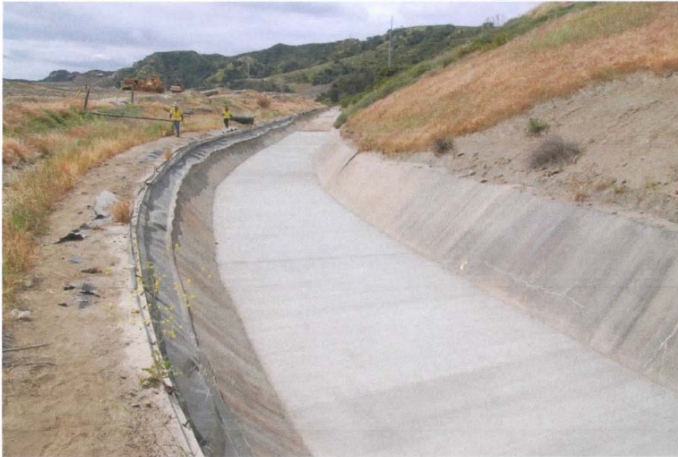
Photo 13: Repaired floor of west drainage channel
