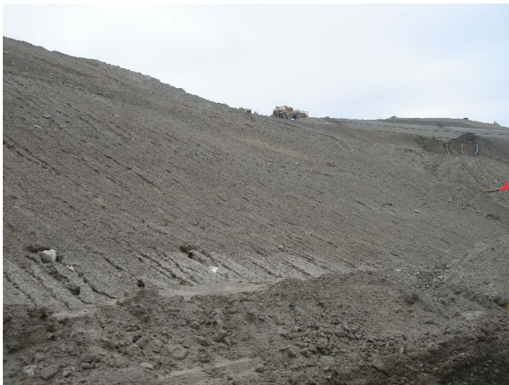
Photo 287: CC3A Soil Stockpile Erosion: May 9, 2017
