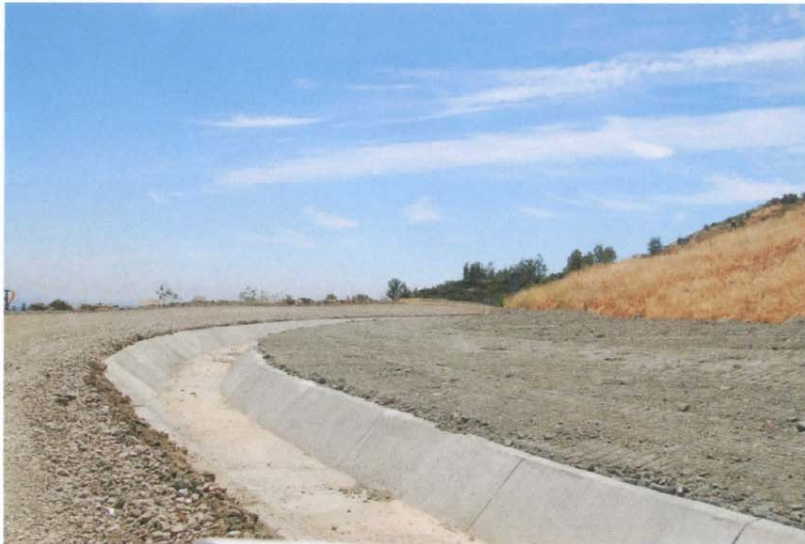
Photo 9: Repaired channel on old City Landfill Deck
