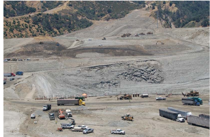
Photo 330: CC4A Part 2 Excavation Area Slide: June 20, 2017
