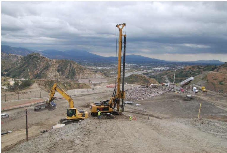
Photo 243: Well Drilling on Deck Cell CC3B: April 18, 2017
