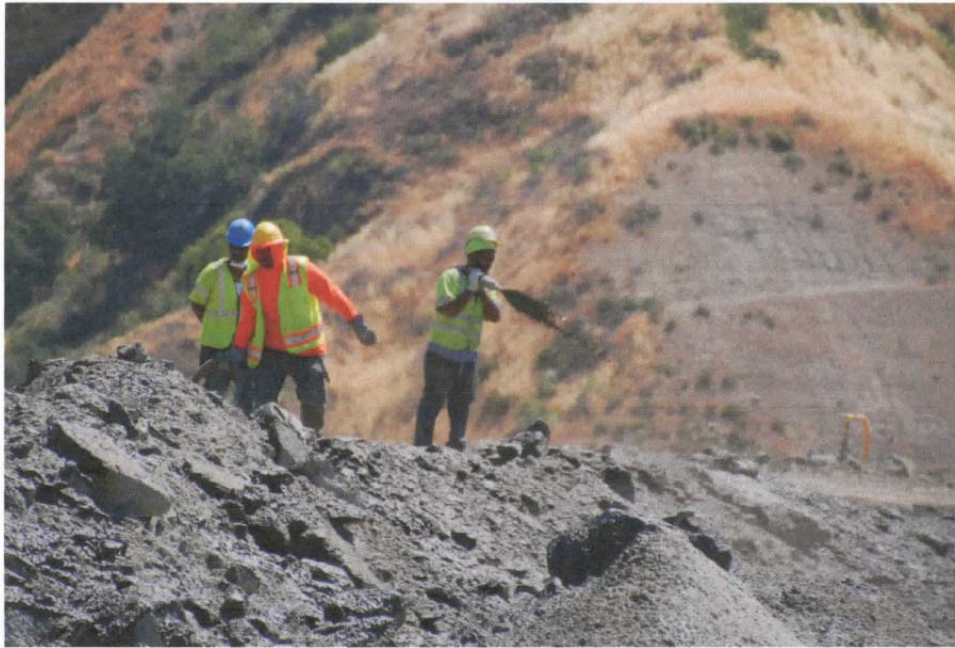
Photo 5: Spraying of Posi shell
