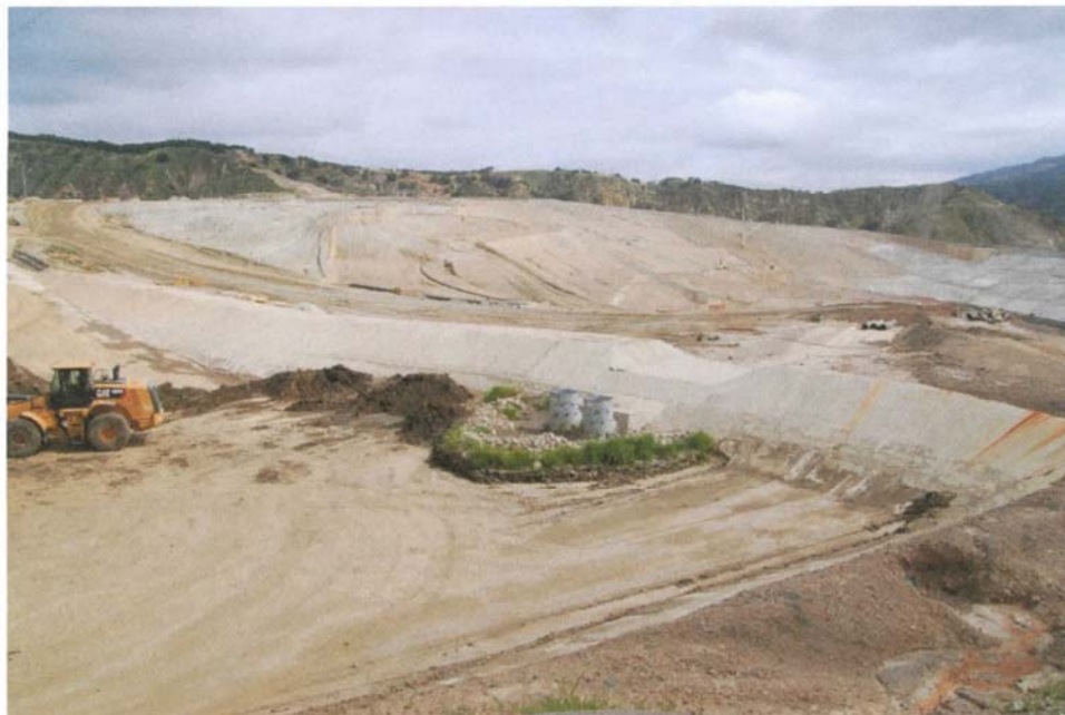
Photo 8: Removal of sediments from Basin A
