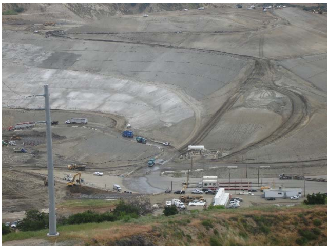
Photo 267: CC3A Slope Posi-Shell: April 18, 2017
