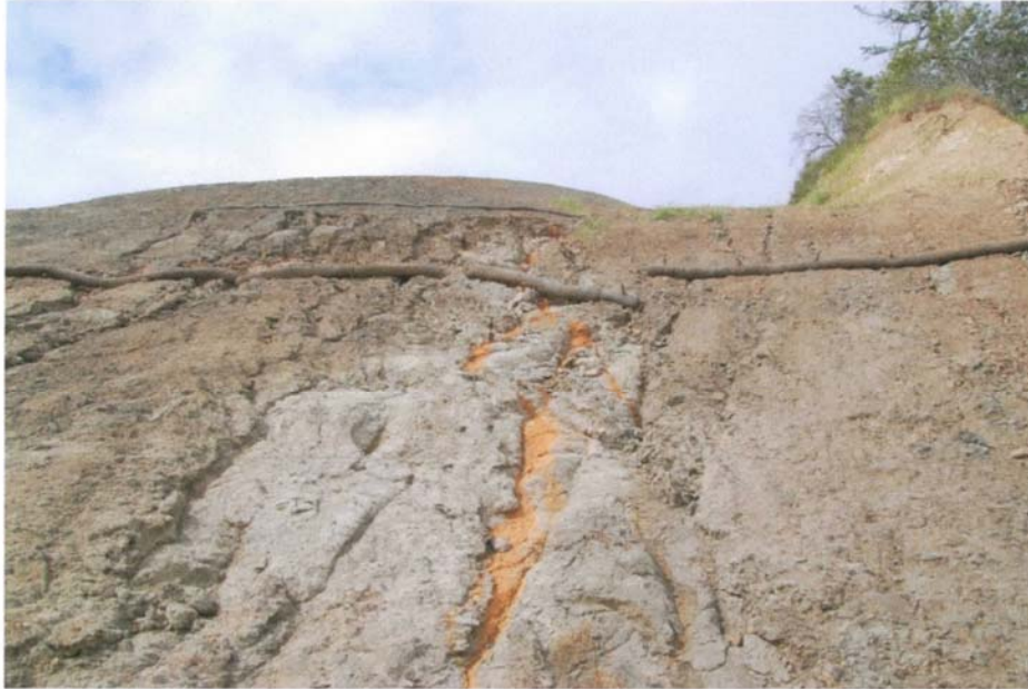
Photo 9: Erosion gullies on fill next to Basin A supporting access road to Flare 3
