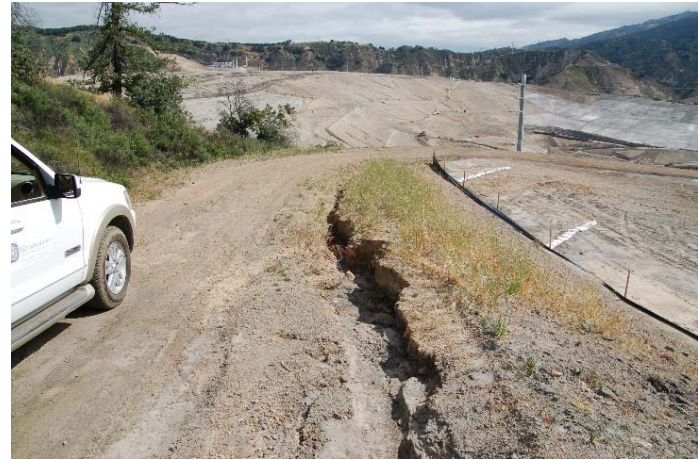
Photo 78: Flare 3 Access Road Erosion Ruts: April 18, 2017
