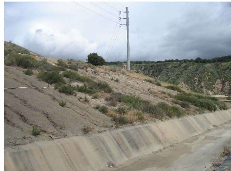
Photo 432: County Sage Mitigation Area Slope Erosion: April 18, 2017
