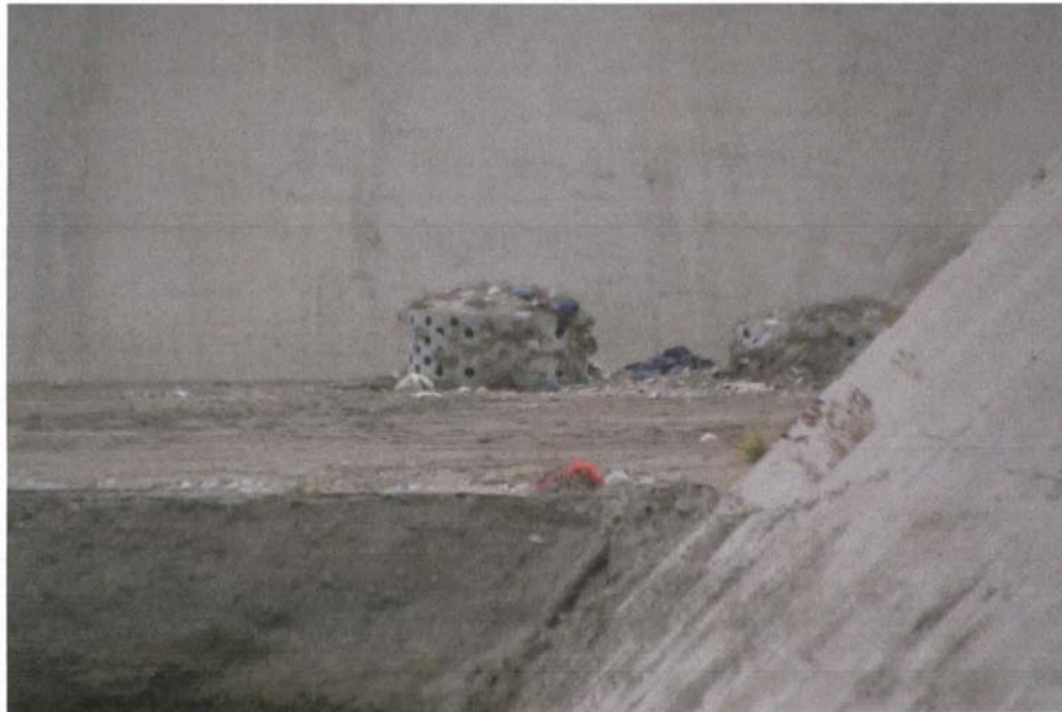
Photo 7: Sediments in back half of Terminal Basin partially obstructing the decant towers
