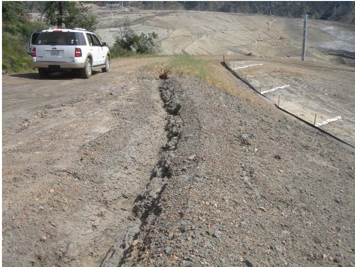
Photo 81: Flare 3 Access Road Erosion Ruts: April 18, 2017
