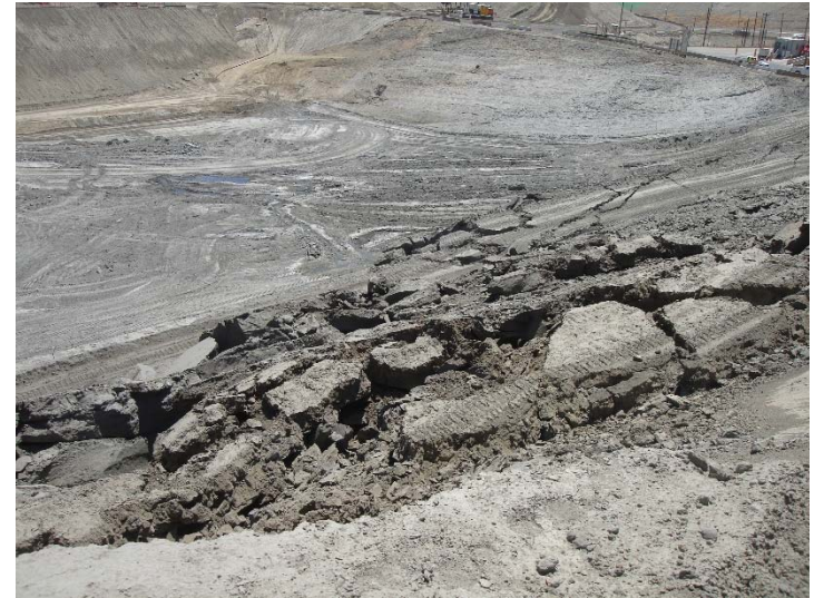
Photo 336: CC4A Part 2 Excavation Area Slide: June 20, 2017
