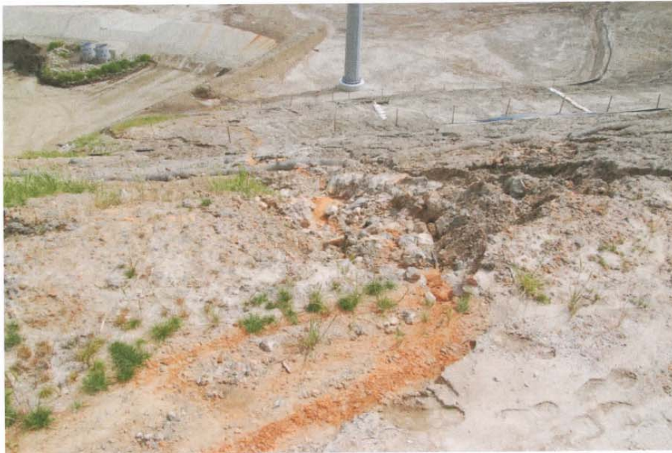
Photo 11: Detail of Erosion gullies toward Basin A from water running down slope
