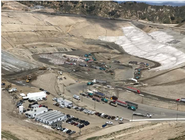
Photo 265: CC3A Slope Posi-Shell: April 18, 2017
