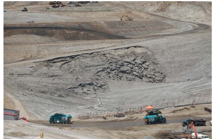
Photo 332: CC4A Part 2 Excavation Area Slide: June 20, 2017
