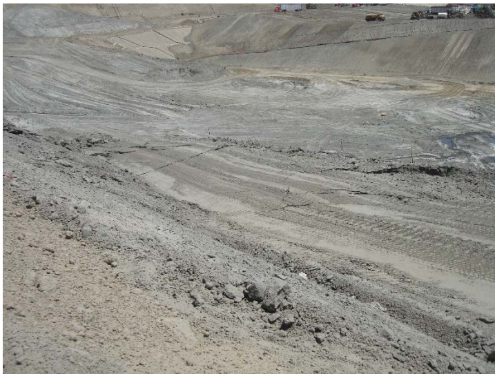
Photo 355: CC4A Part 2 Excavation Area Slide: June 20, 2017
