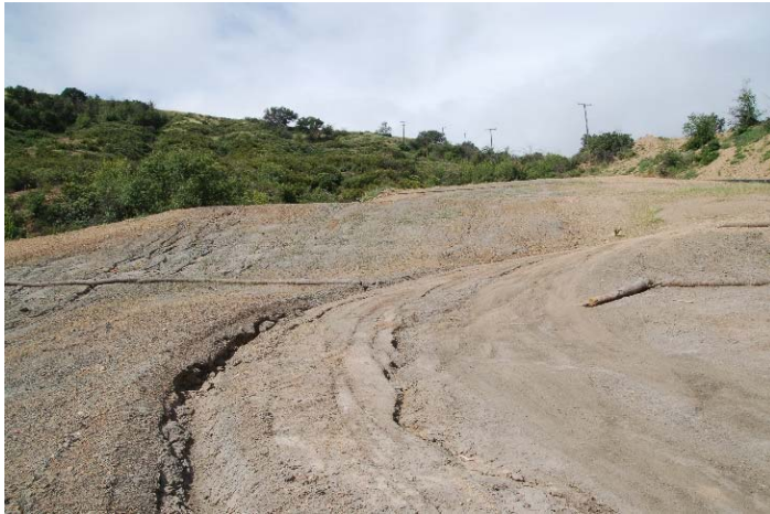
Photo 77: Flare 3 Access Road Erosion Ruts: April 18, 2017
