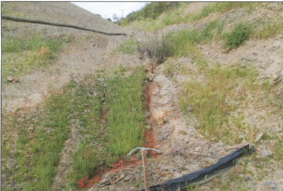
Photo 10: View of water gullies between native and fill supporting access road to Flare 3
