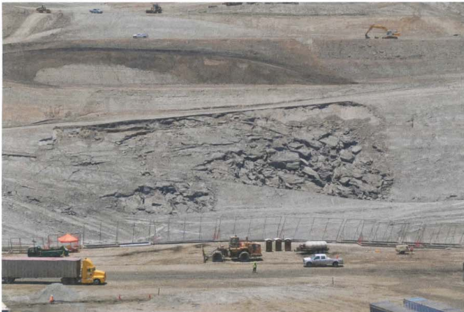
Photo 4: Landslide on west side of excavation for Cell CC4 Phase 2
