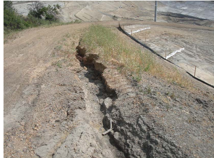
Photo 82: Flare 3 Access Road Erosion Ruts: April 18, 2017
