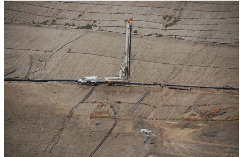
Photo 242: Well Drilling on Slope Cell CC3B: April 18, 2017
