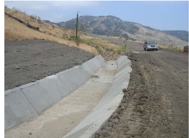
Photo 408: Deck B Drainage Channel Repair: May 9, 2017
