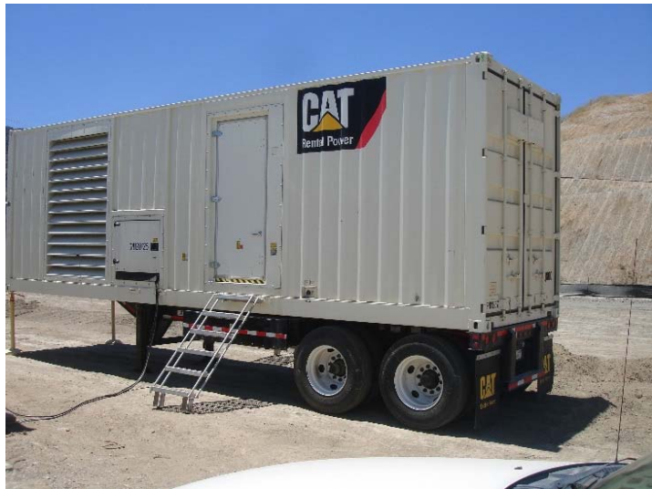
Photo 151: Flare 9 & 10 Standby Power Supply: June 20, 2017
