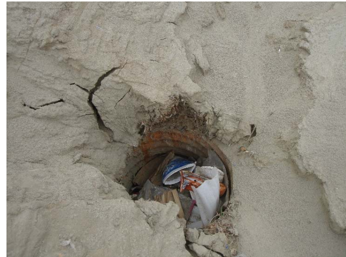
Photo 252: CC3B Temporary Basin Plugged Low-Flow Outlet to Terminal Basin: May 9, 2017
