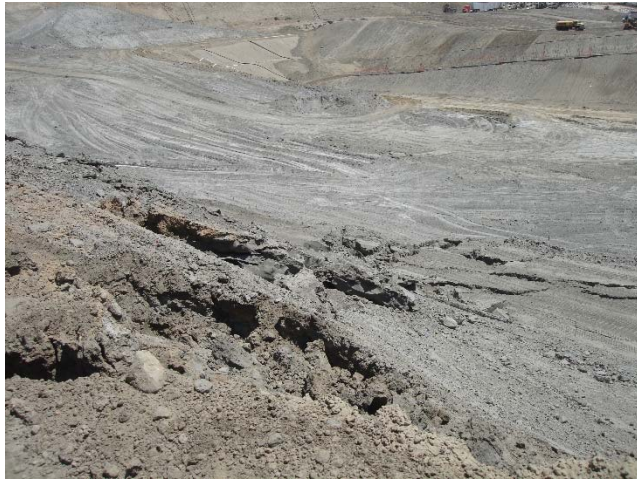
Photo 341: CC4A Part 2 Excavation Area Slide: June 20, 2017
