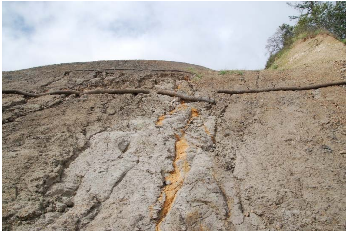
Photo 5: Slope Erosion near Basin A: April 18, 2017
