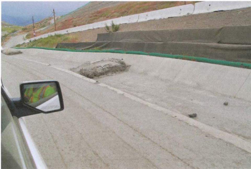
Photo 5: Fines removed from in front Gabions in Channel
