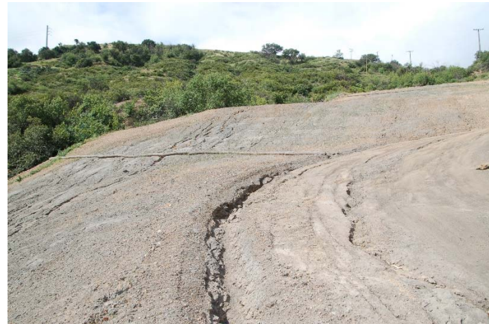
Photo 76: Flare 3 Access Road Erosion Ruts: April 18, 2017
