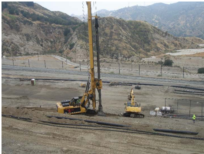
Photo 255: CC3B Top Deck Well Drilling
