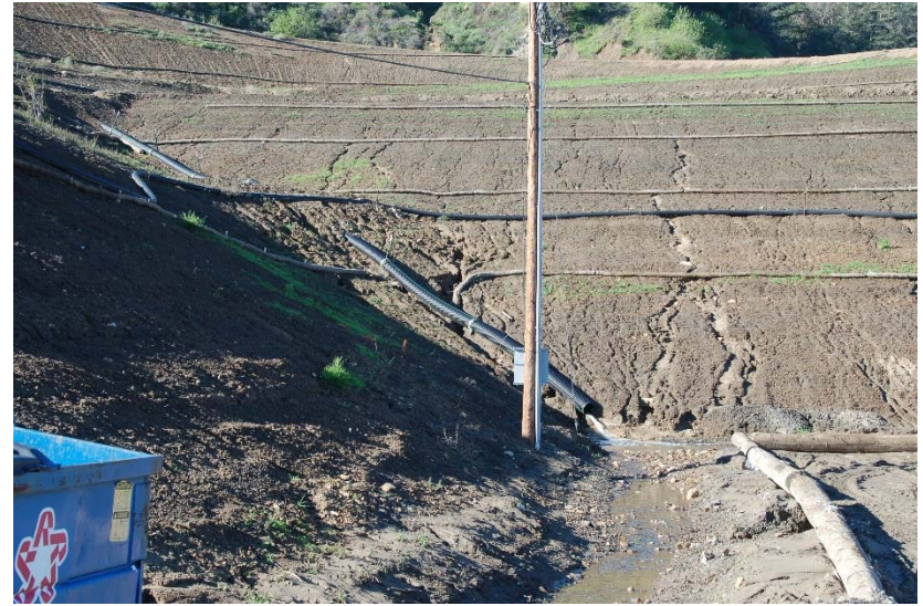
Photo 126: Slope Erosion near CC4 Liner Area: February 23, 2017
