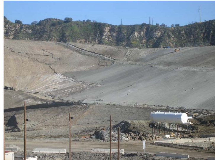
Photo 158: Posi-Shell on Slopes above CC4 Liner Area: March 9, 2017
