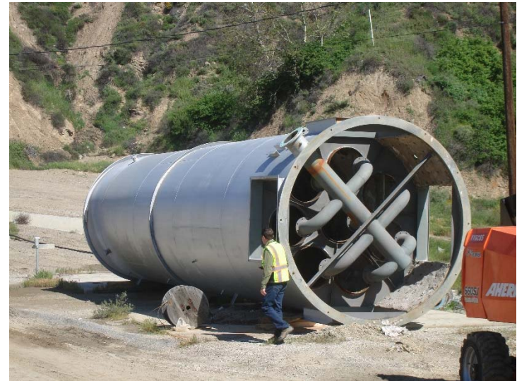
Photo 308: Temporary Flare Stack Dismantle: March 23, 2017
