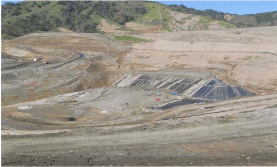
Photo 1: Base of Cell CC4. – Erosion gullies in operation layer
