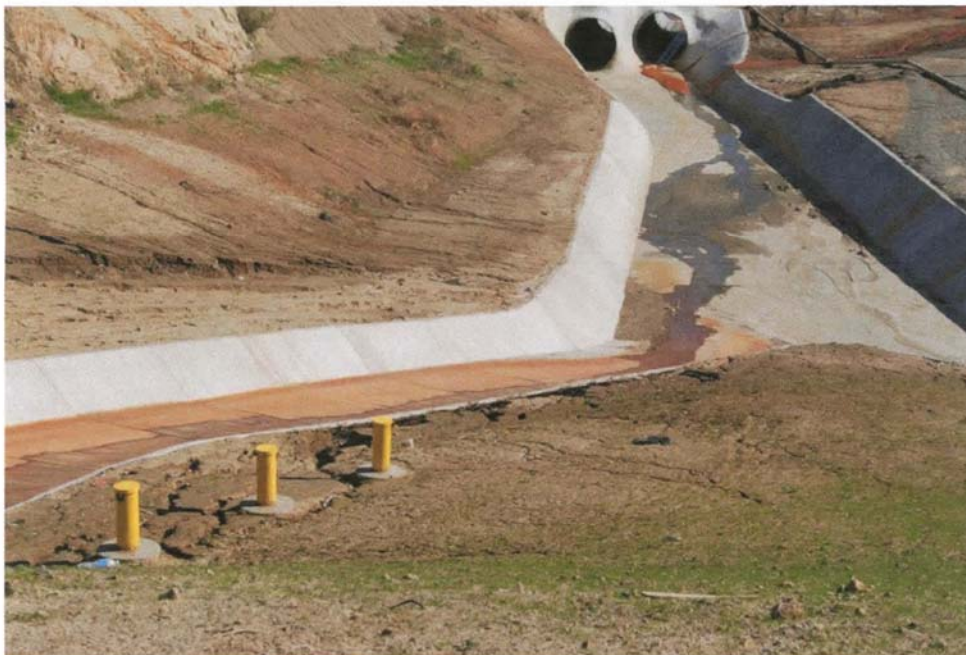
Photo 6: Erosion on slope of new temporary unlined earthen basin at toe of landfill
