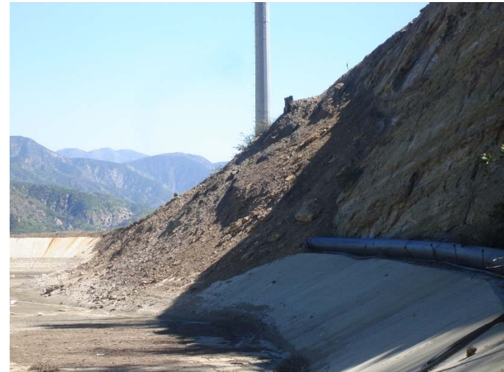
Photo 56: Erosion in Adjacent Hillside to Basin A: March 9, 2017
