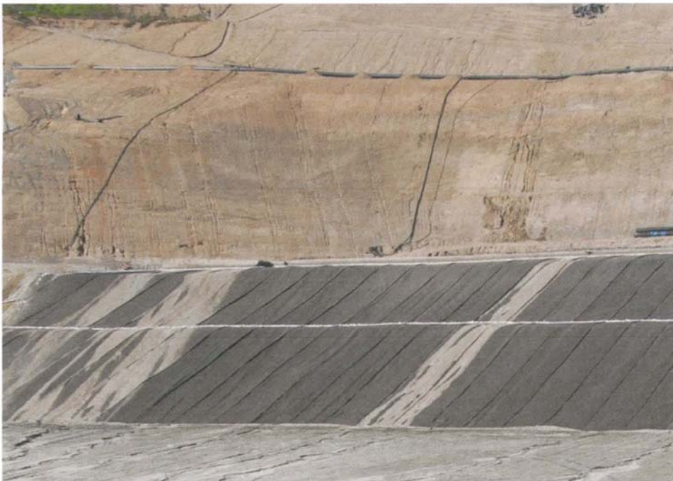
Photo 2: Geosynthetics on slope of CC4 – no damage visible
