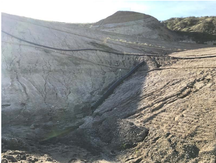
Photo 105: CC3A Slopes Erosion: January 31, 2017
