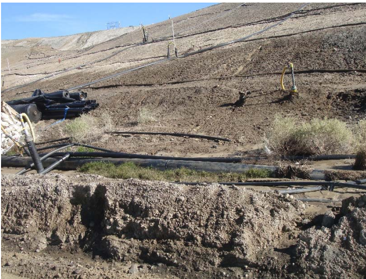
Photo 111: CC3A Slopes Erosion: January 31, 2017
