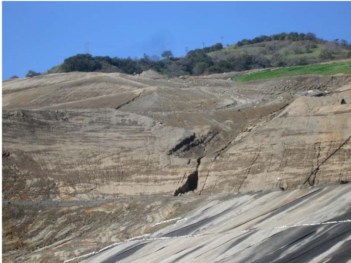
Photo 127: Slope Erosion near CC4 Liner Area: February 23, 2017
