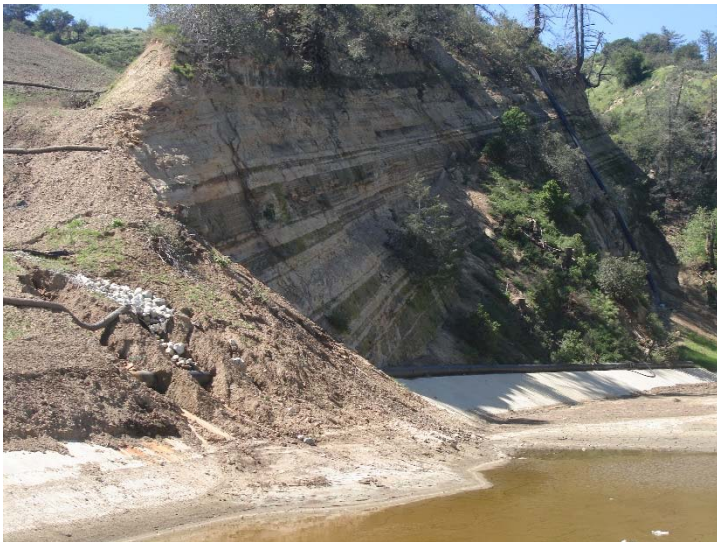
Photo 63: Erosion in Adjacent Hillside to Basin A: March 23, 2017
