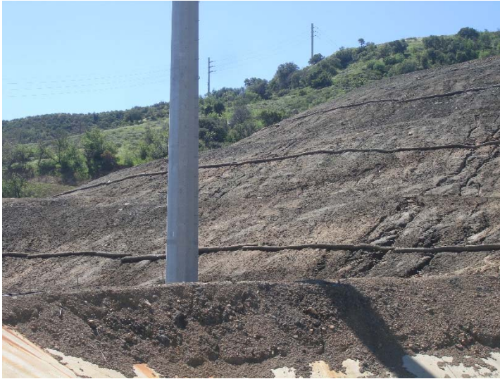
Photo 65: Erosion in Adjacent Hillside to Basin A: March 23, 2017
