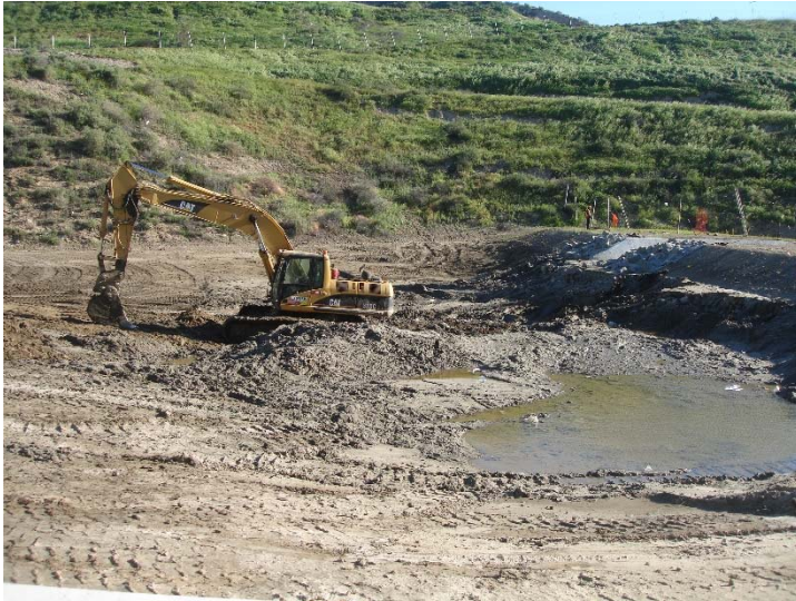
Photo 409: CC3B Temporary Solids Removal: March 23, 2017
