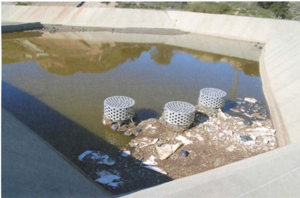
Photo 12: Water level against decant towers
