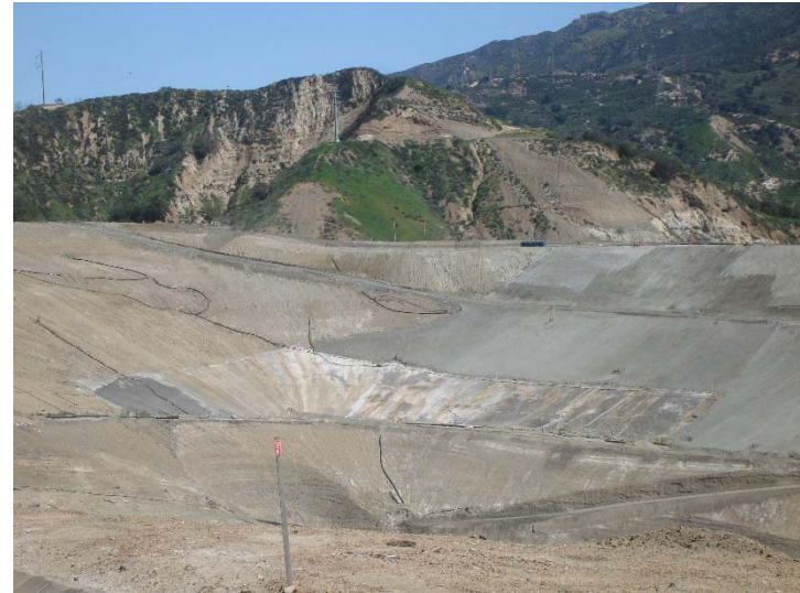
Photo 162: Posi-Shell on Slopes above CC4 Liner Area: March 9, 2017
