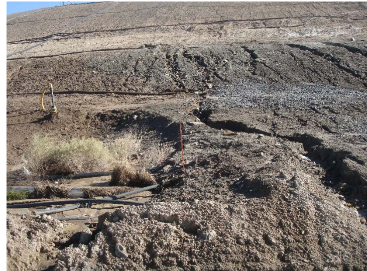
Photo 112: CC3A Slopes Erosion: January 31, 2017
