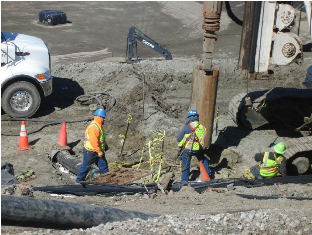
Photo 181: Well Drilling on CC3A Bench: March 23, 2017
