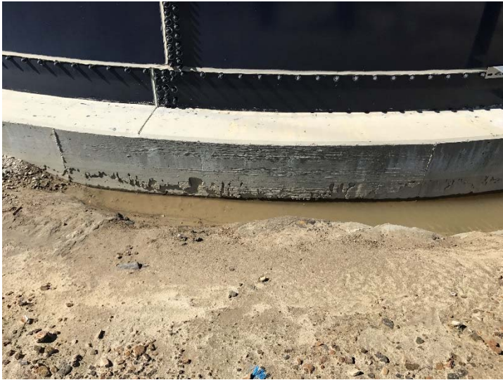
Photo 481: Deck A Water Tank Foundation Partially Backfilled: February 23, 2017
