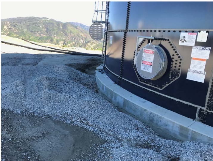
Photo 483: Deck A Water Tank Foundation Partially Backfilled: February 23, 2017
