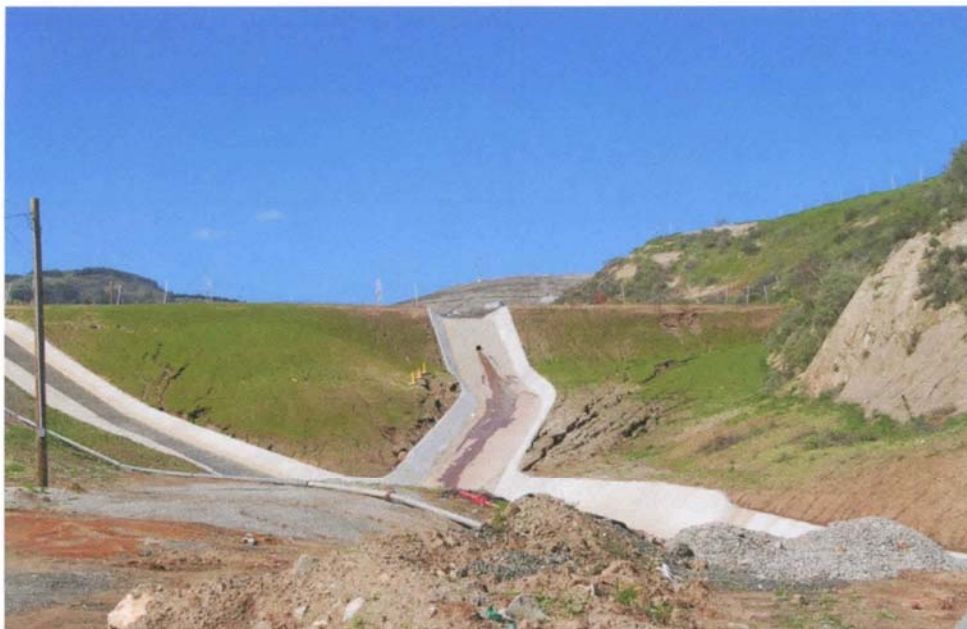
Photo 4: Erosion gullies along spillway of interim basin
