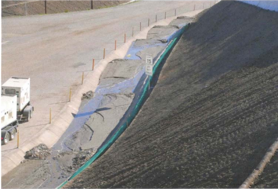
Photo 7: Sediment trapped in South drainage channel reducing area of channel
