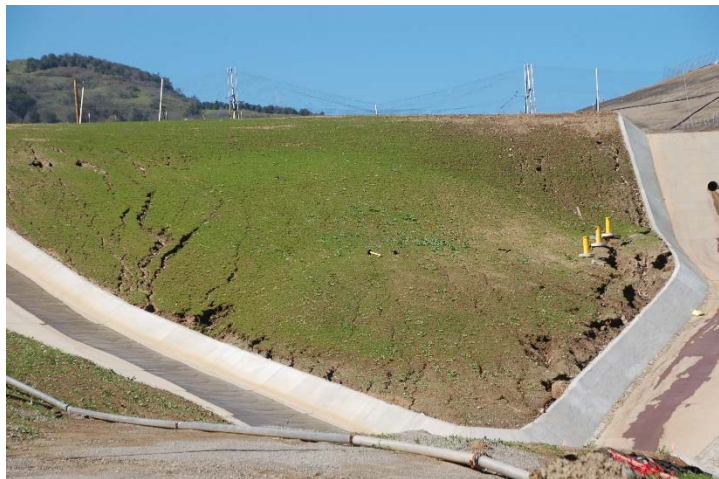
Photo 131: Site Erosion: February 23, 2017
