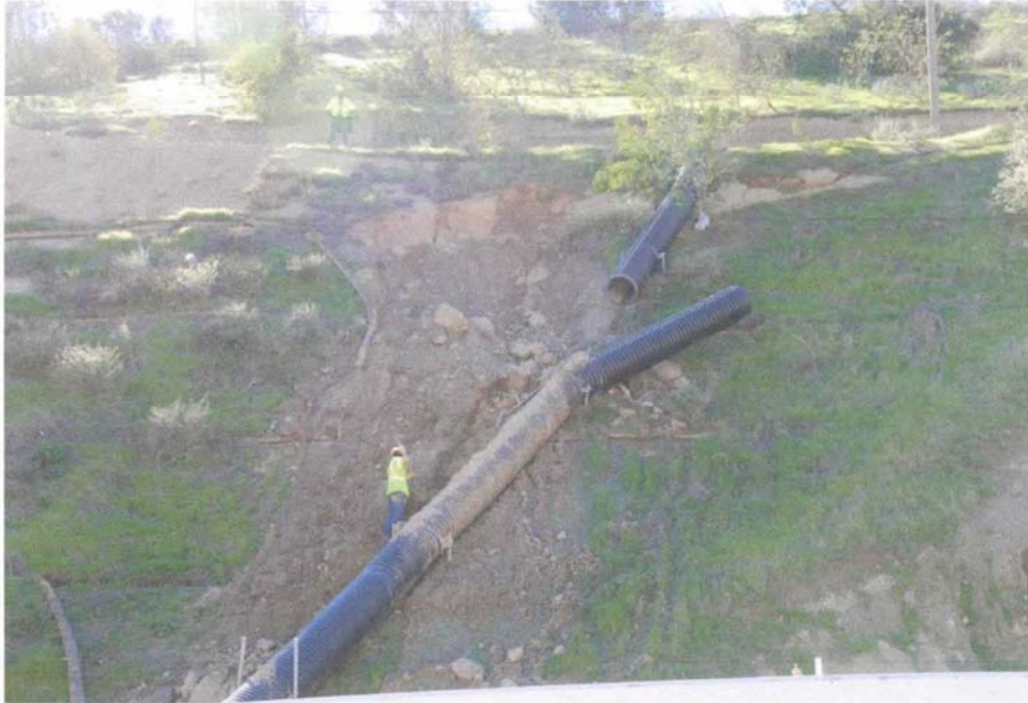
Photo 9: Ruptured downchute undergoing repair
