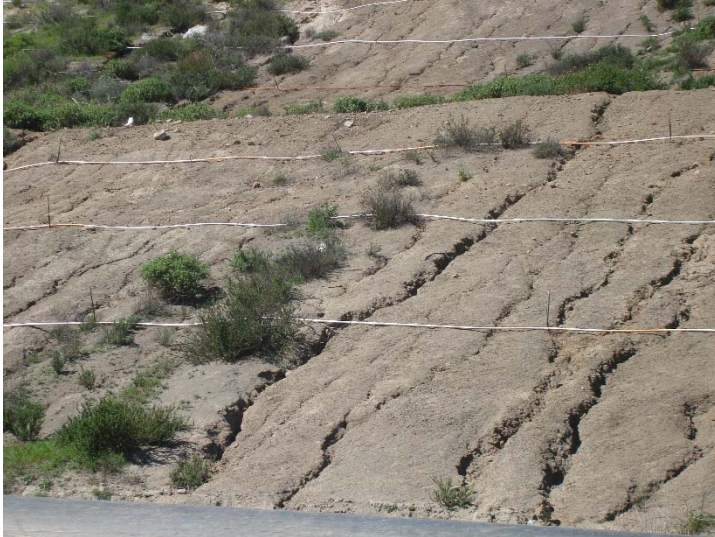
Photo 511: County Sage Mitigation Area Slope Erosion: March 9, 2017
