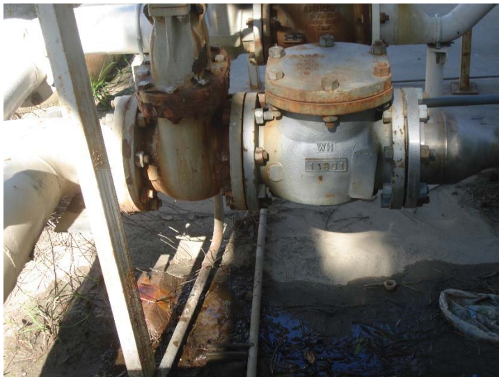
Photo 371: Potable Water Supply Leak: January 31, 2017
