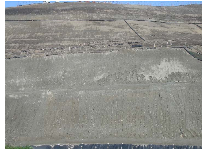
Photo 132: Slope Erosion near CC4 Liner Area: February 23, 2017
