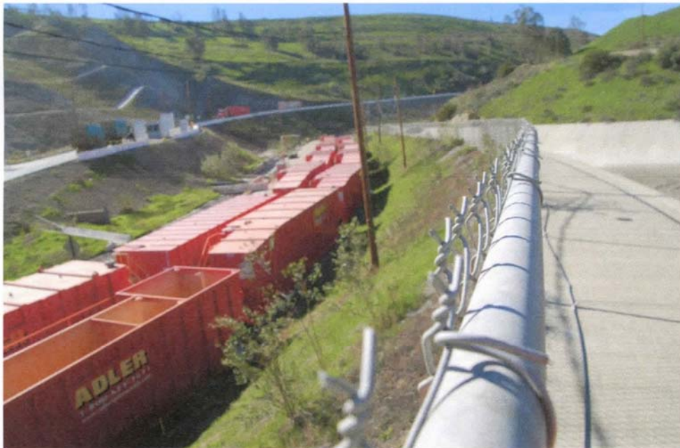
Photo 8: Storage tanks to store stormwater from new temporary unlined earthen basin
