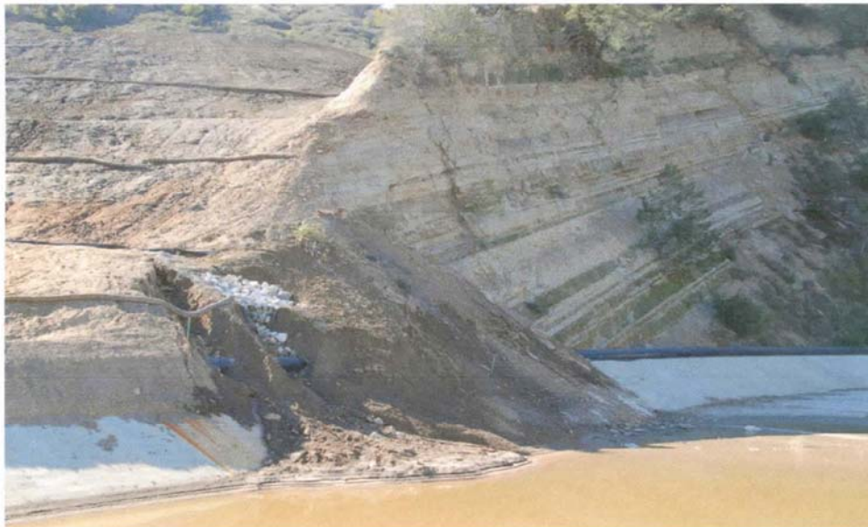
Figure 14: Sloughed soil at Basin A
