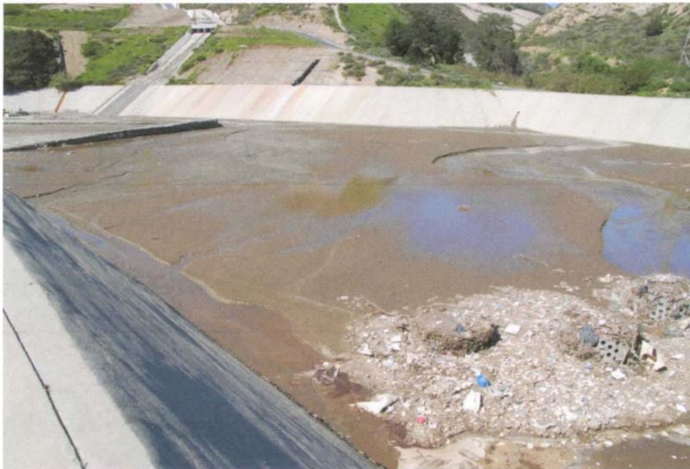
Photo 8: Sediment in Terminal Basin
