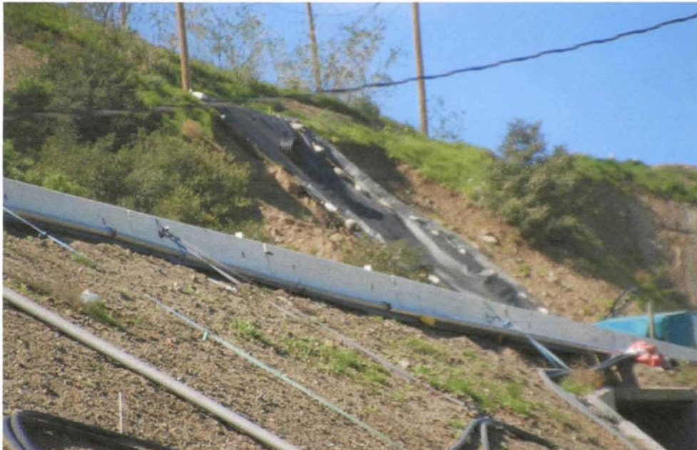
Photo 6: Slip liner installed as repair of downchute on slope along main access road
