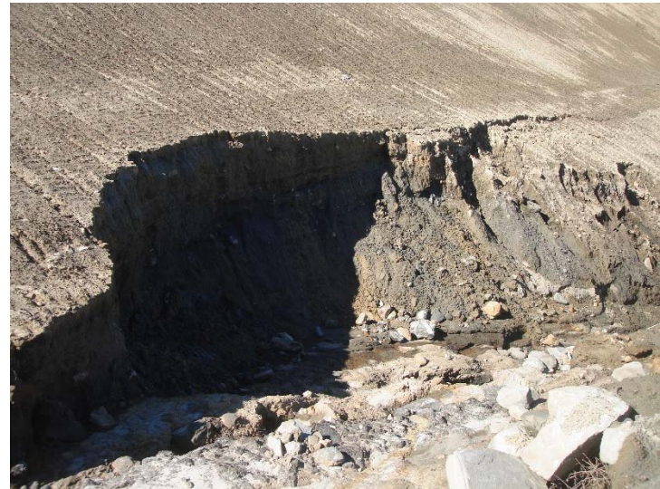
Photo 124: Slope Erosion near CC4 Liner Area: February 23, 2017
