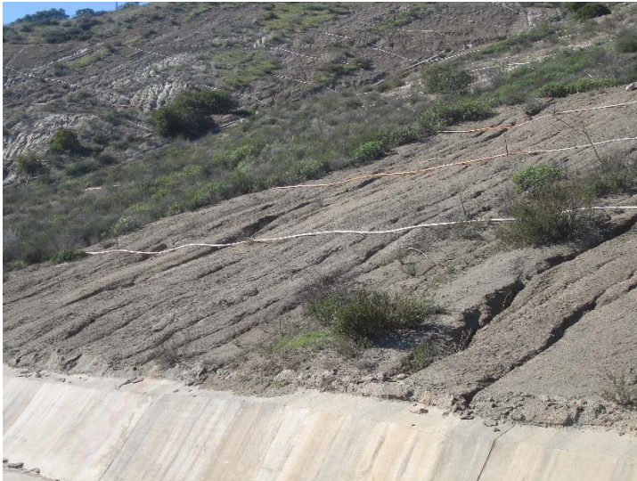
Photo 505: County Sage Mitigation Area Slope Erosion: January 31, 2017
