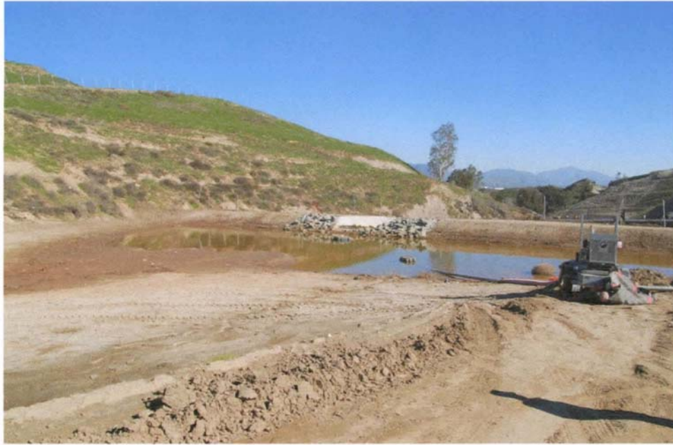
Photo 7: New temporary unlined earthen basin at toe of landfill filled up with sediment
