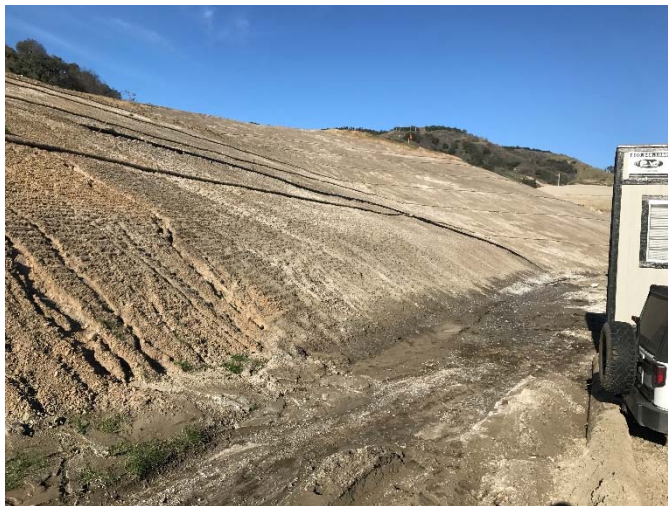
Photo 107: CC3A Slopes Erosion: January 31, 2017
