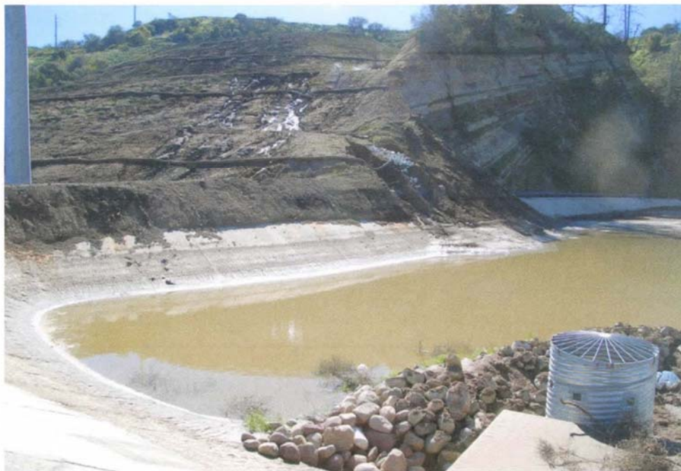
Photo 12: Sloughed soil in Basin A and seep on graded cut slope
