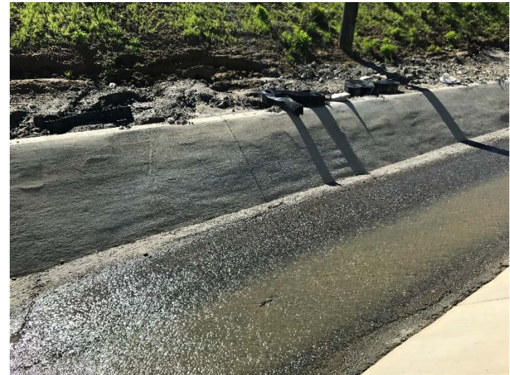
Photo 412: City South Slope Slump: February 23, 2017
