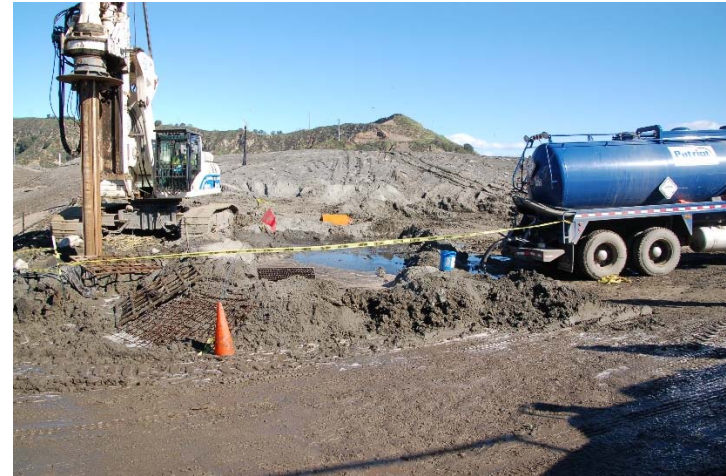
Photo 142: Well Drilling on CC3A Top Deck: February 23, 2017
