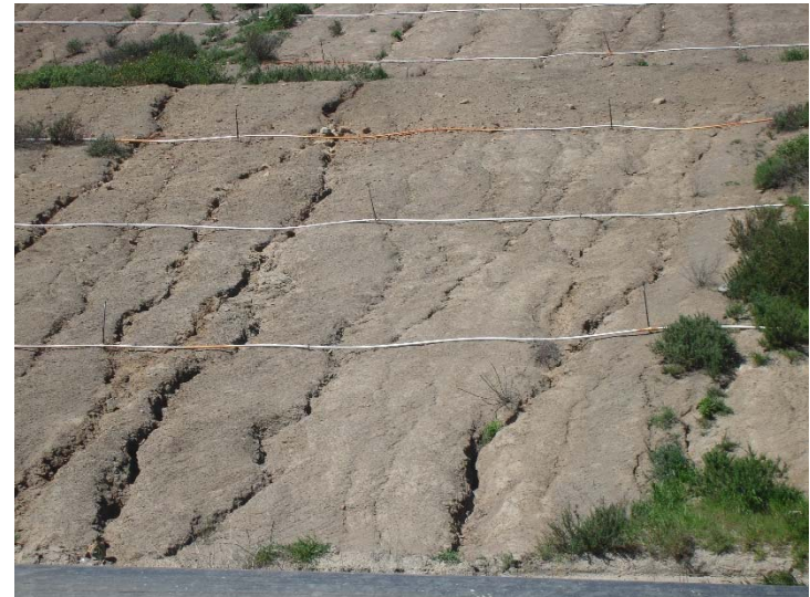
Photo 512: County Sage Mitigation Area Slope Erosion: March 9, 2017
