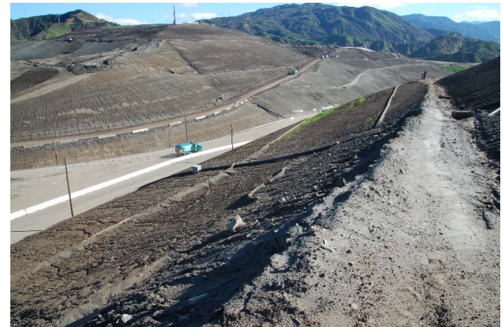
Photo 416: City South Slope Slump: February 23, 2017
