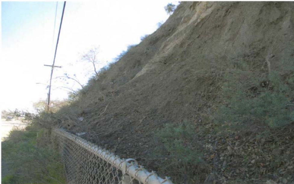
Figure 16: Soil against fence on retaining wall on San Fernando Road
