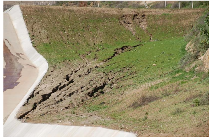
Photo 130: Site Erosion: February 23, 2017
