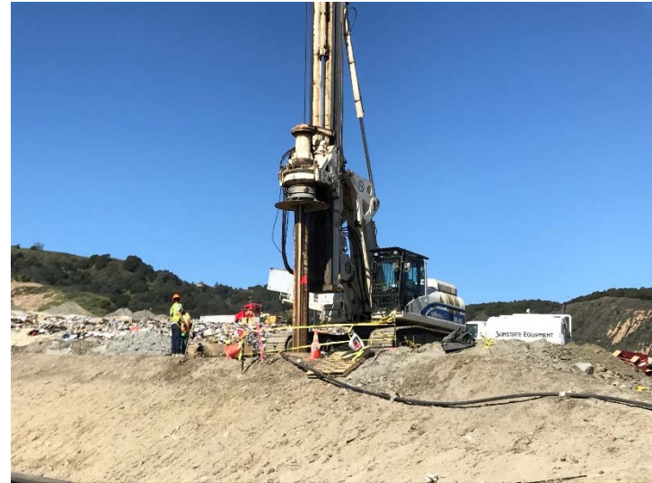
Photo 242: Well Drilling County Top Deck: March 9, 2017
