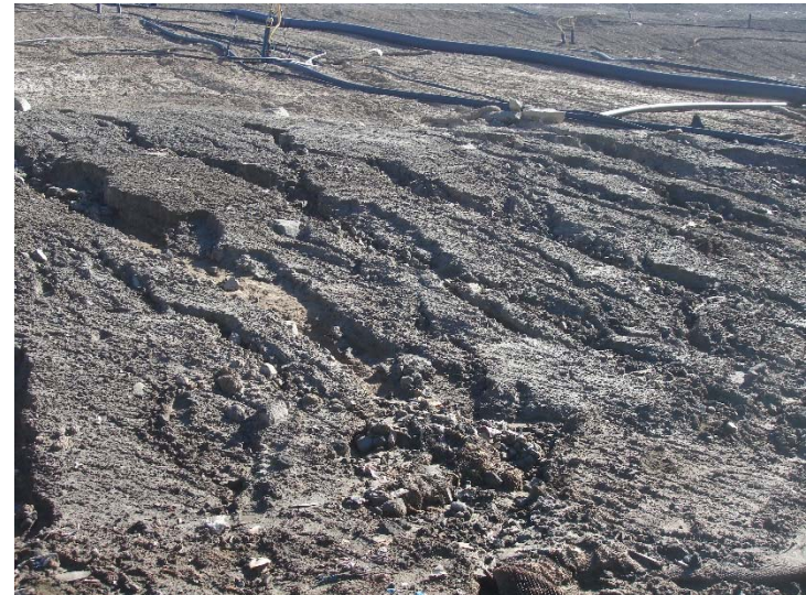
Photo 116: CC3A Slopes Erosion: January 31, 2017
