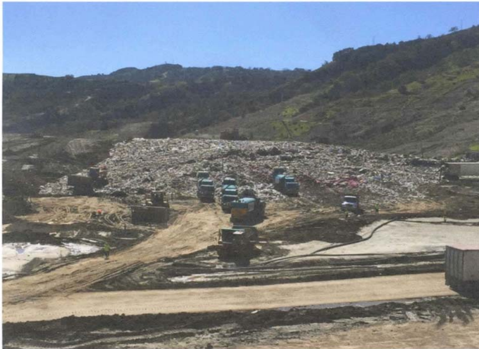
Photo 3: Waste Placement on old County landfill deck Phase IV
