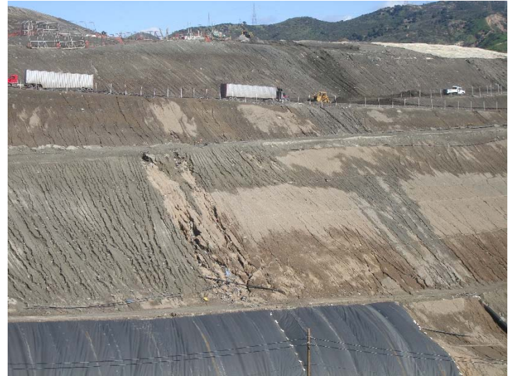
Photo 134: Slope Erosion near CC4 Liner Area: February 23, 2017
