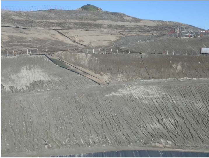
Photo 133: Slope Erosion near CC4 Liner Area: February 23, 2017
