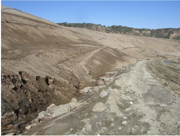
Photo 125: Slope Erosion near CC4 Liner Area: February 23, 2017
