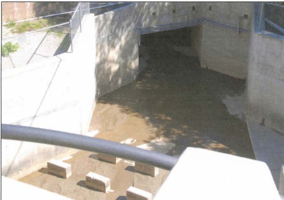
Photo 10: Sediment flowing outside Terminal Basin
