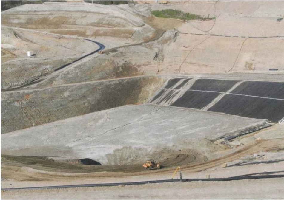
Photo 1: Base of Cell CC4 Protect by operation layer – Some erosion gullies
