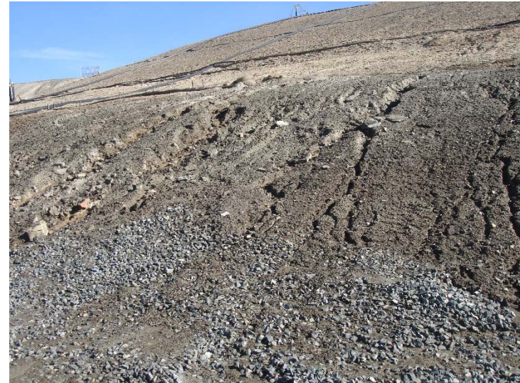
Photo 114: CC3A Slopes Erosion: January 31, 2017
