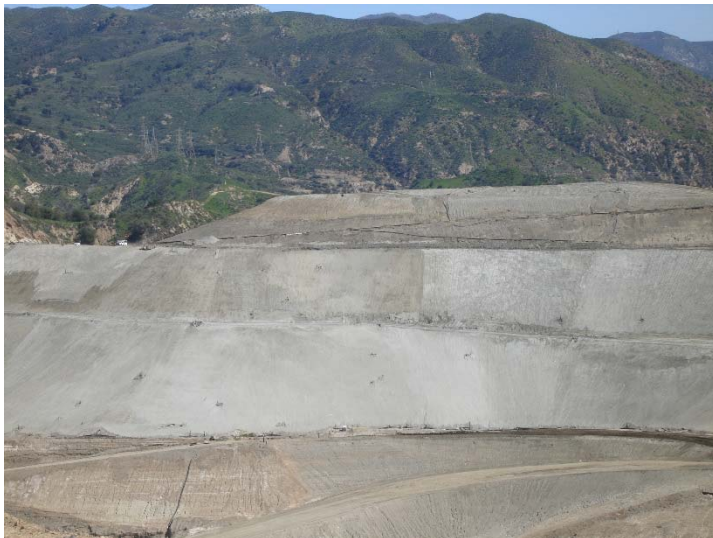
Photo 163: Posi-Shell on Slopes above CC4 Liner Area: March 9, 2017
