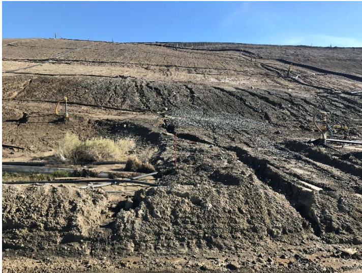
Photo 109: CC3A Slopes Erosion: January 31, 2017
