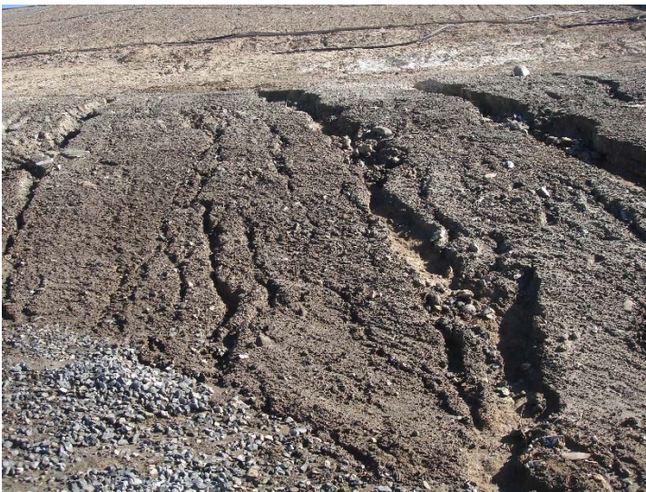
Photo 115: CC3A Slopes Erosion: January 31, 2017
