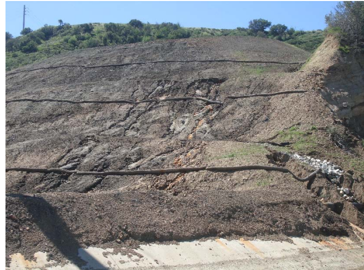
Photo 64: Erosion in Adjacent Hillside to Basin A: March 23, 2017
