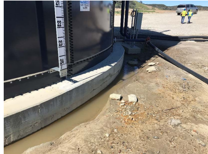
Photo 482: Deck A Water Tank Foundation Partially Backfilled: February 23, 2017
