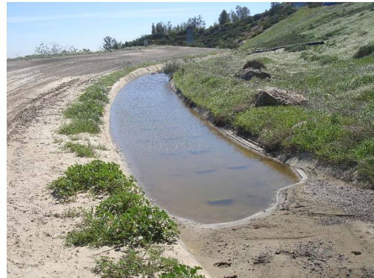
Photo 428: City South Drainage Channel Ponding Water: March 9, 2017
