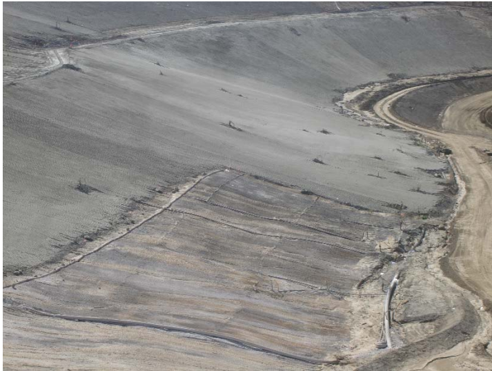
Photo 161: Posi-Shell on Slopes above CC4 Liner Area: March 9, 2017
