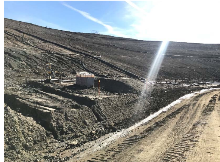
Photo 110: CC3A Slopes Erosion: January 31, 2017
