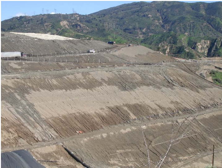
Photo 135: Slope Erosion near CC4 Liner Area: February 23, 2017
