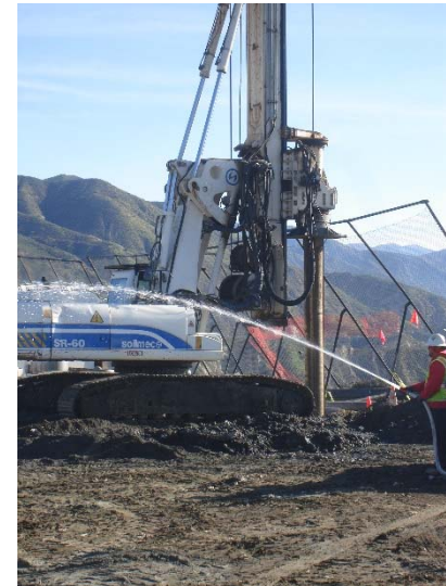
Photo 120: Well Drilling on CC3A Top Deck: January 31, 2017
