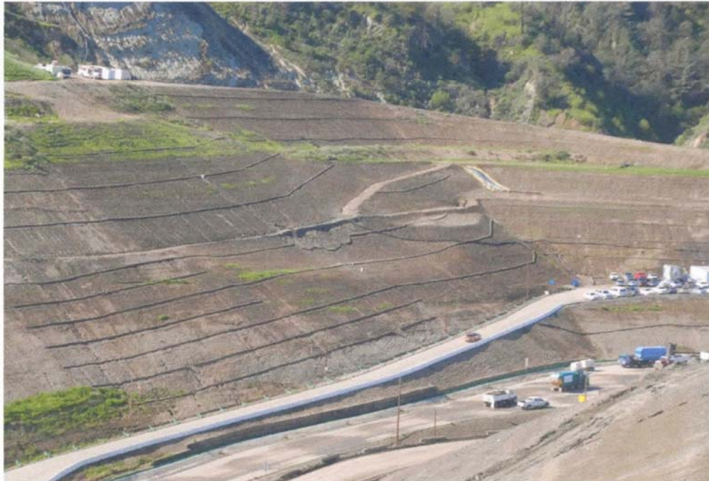
Figure 15: Area exhibiting soil movement above access road to Administration Pad
