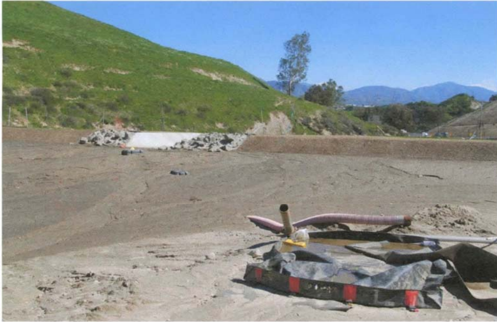
Photo 5: Interim Basin completely full of sediment
