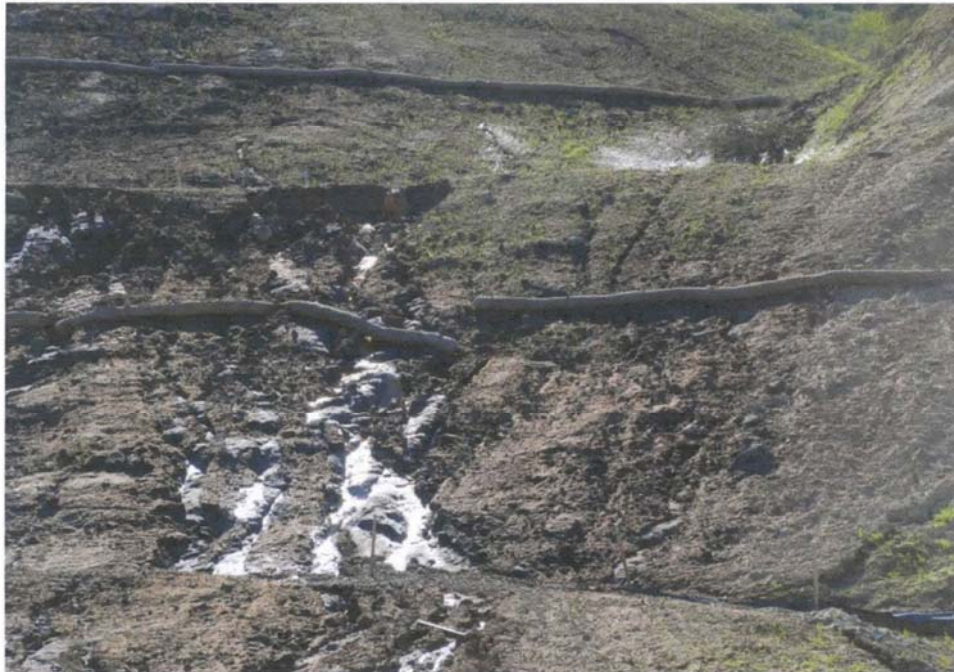
Figure 13: Seep , erosion and sloughed soil on graded cut slope at Basin A
