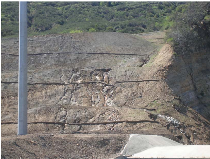
Photo 55: Erosion in Adjacent Hillside to Basin A: March 9, 2017
