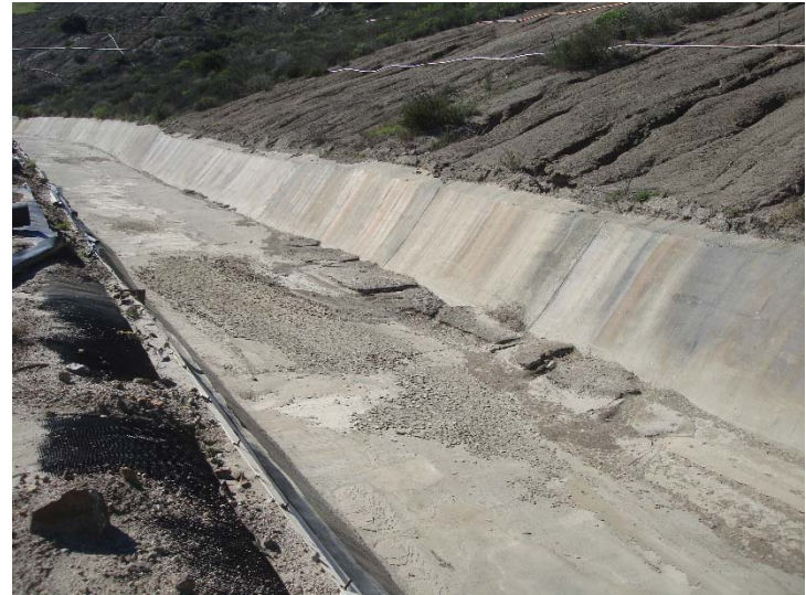
Photo 502: County Sage Mitigation Area Slope Erosion: January 31, 2017
