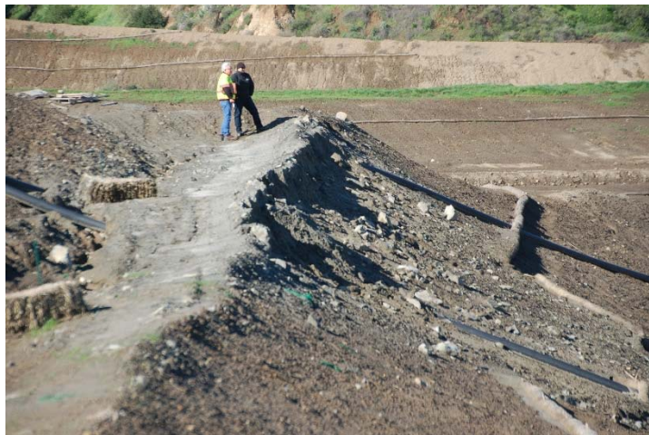
Photo 423: City South Slope Slump: February 23, 2017
