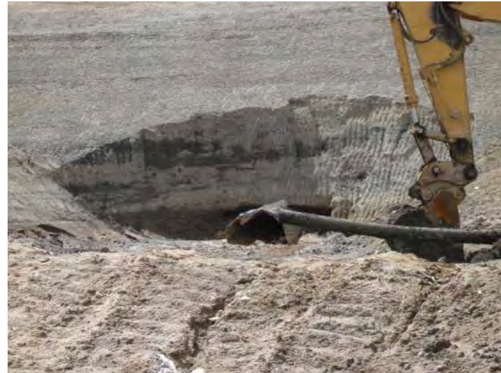
Photo 386: City Stockpile Buried Drainage Pipe: April 2, 2014
