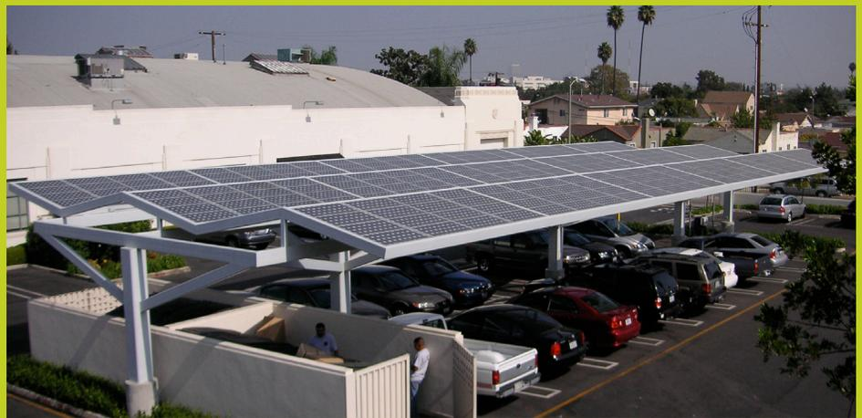
▲ Built in 2003, the parking lot attached to the historic Helms Bakery Building incorporates power generating solar panels. It provides shade for all cars and power for electric cars with charging stations and dedicated spaces for said cars. The project was completed in partnership with the Los Angeles Department of Water and Power.
