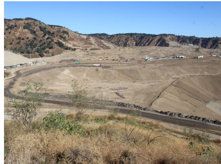
Photo 106: Working Area, CC-4 Part 4/5: August 19, 2024
