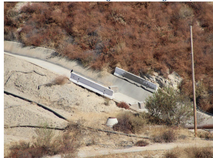
Photo 208: Eastside Drainage Channel: August 19, 2024
