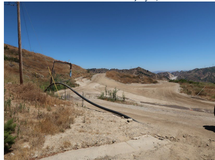
Photo 344: General Site: July 3, 2024
