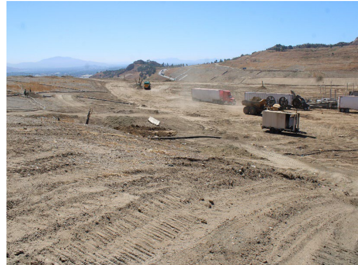
Photo 26: Working Area, CC4 Part 1/2: August 19, 2024
