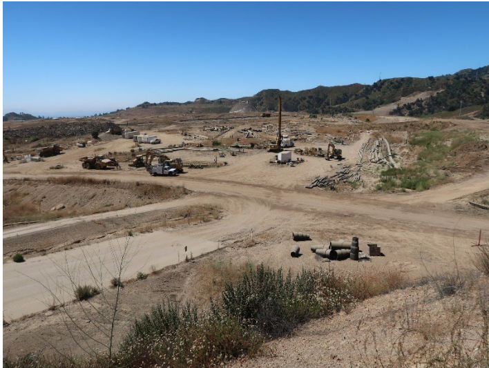
Photo 337: General Site: July 3, 2024
