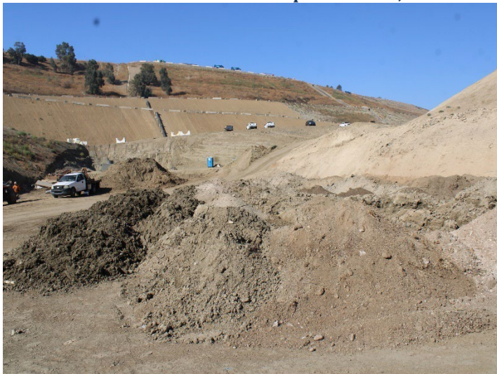
Photo 455: General Site: September 24, 2024
