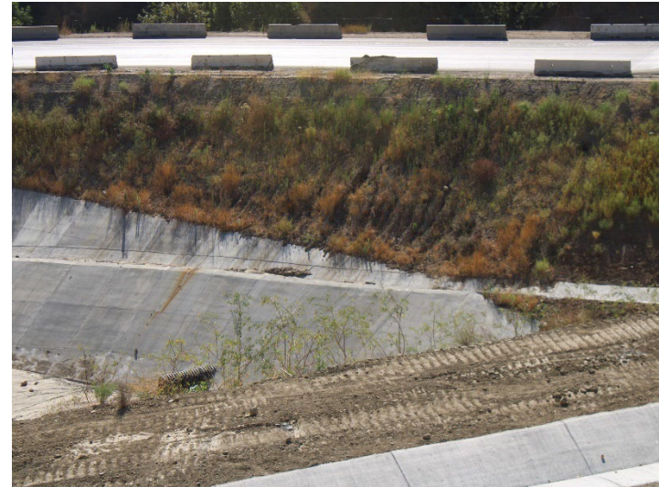
Photo 358: General Site: August 19, 2024
