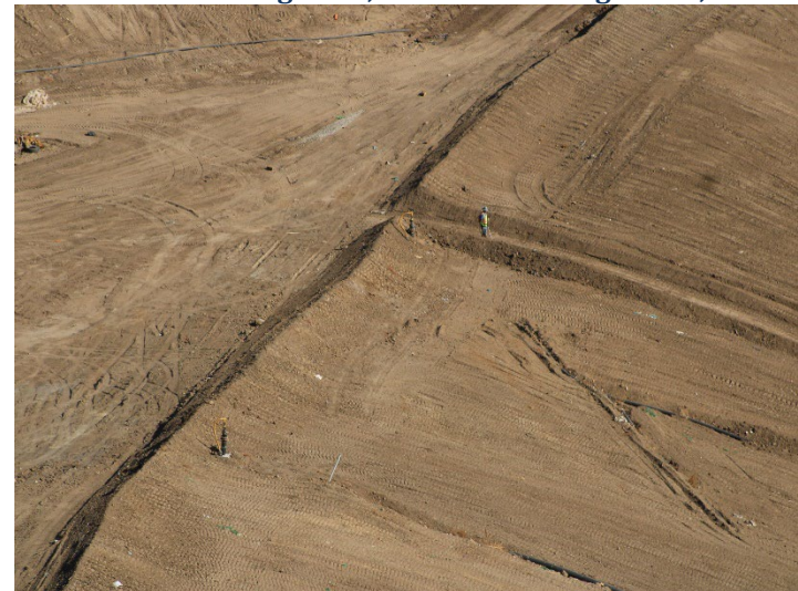
Photo 72: Working Area, CC-4 Part 3: August 19, 2024
