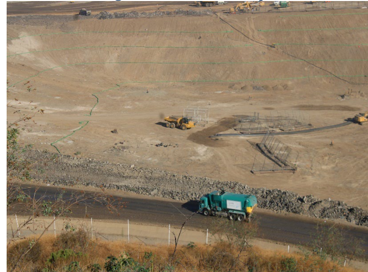
Photo 84: Working Area, CC-4 Part 3: September 24, 2024
