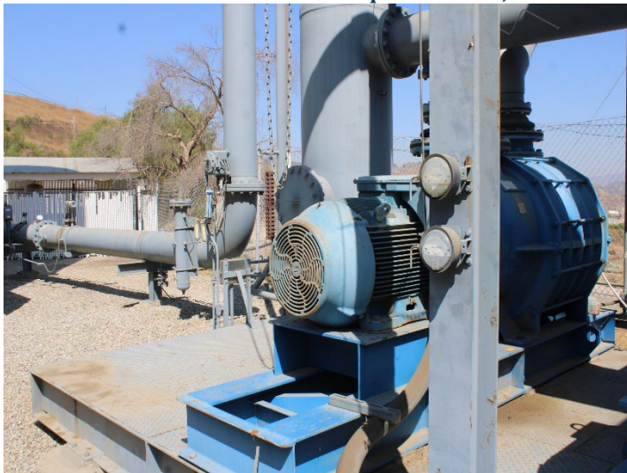
Photo 491: General Site: September 24, 2024
