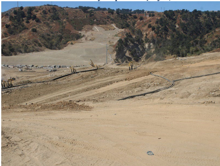
Photo 179: County Top Deck: August 19, 2024
