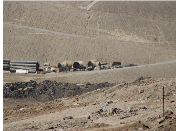
Photo 46: Working Area, CC4 Part 1/2: August 19, 2024
