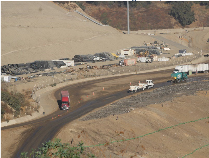
Photo 447: General Site: September 24, 2024
