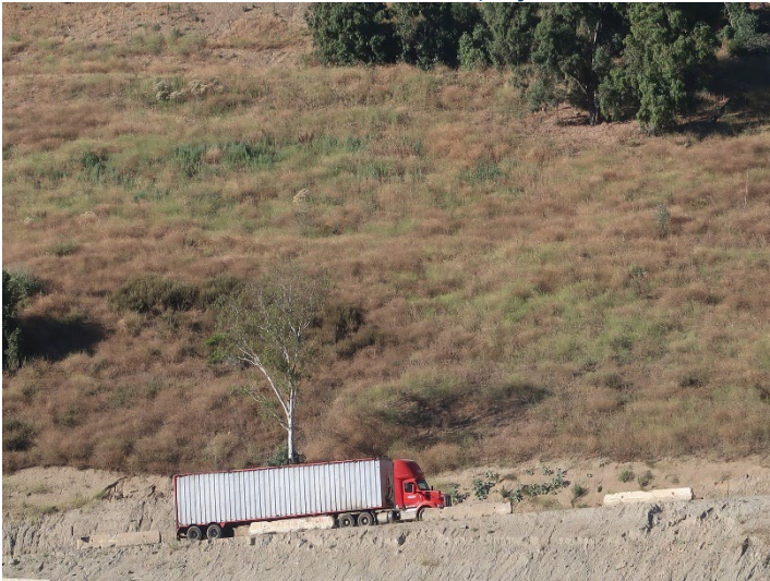
Photo 311: General Site: July 3, 2024
