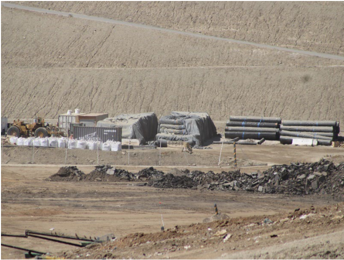
Photo 45: Working Area, CC4 Part 1/2: August 19, 2024
