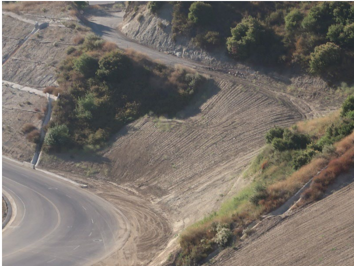
Photo 305: General Site: July 3, 2024
