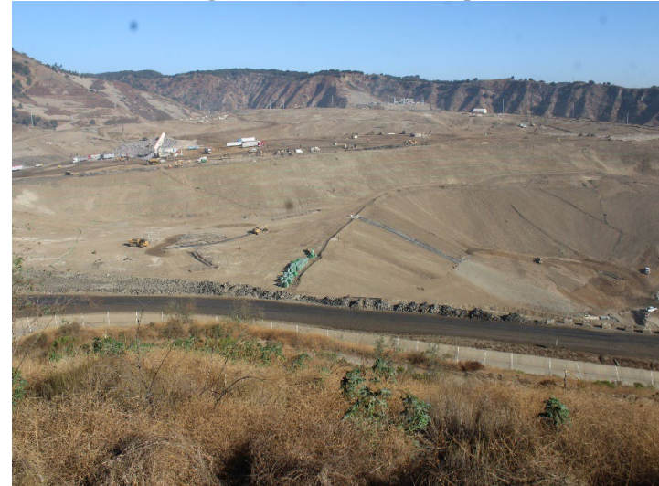
Photo 80: Working Area, CC-4 Part 3: September 24, 2024
