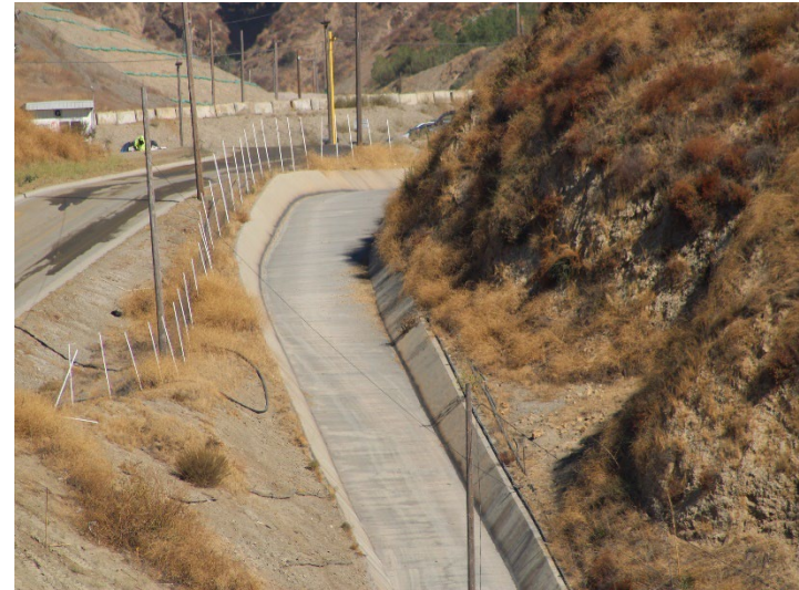
Photo 206: Eastside Drainage Channel: August 19, 2024
