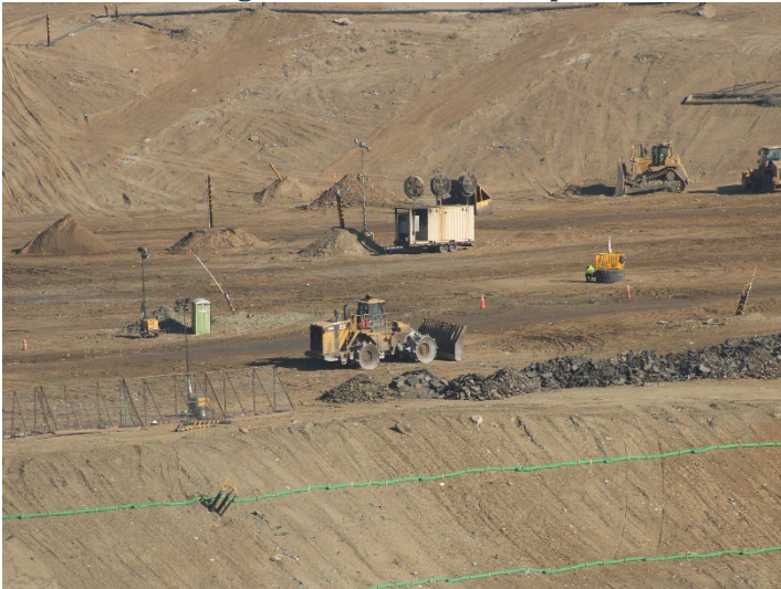
Photo 95: Working Area, CC-4 Part 3: September 24, 2024
