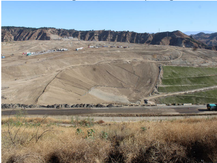
Photo 107: Working Area, CC-4 Part 4/5: August 19, 2024
