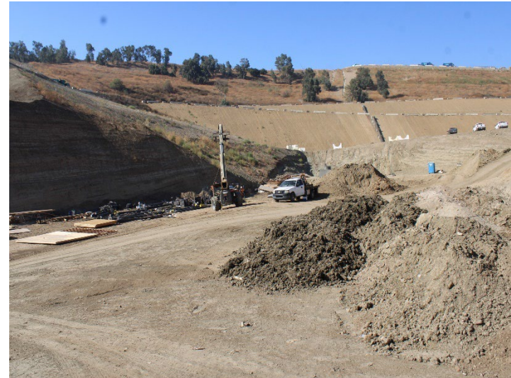
Photo 454: General Site: September 24, 2024
