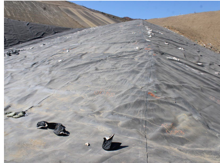
Photo 458: General Site: September 24, 2024
