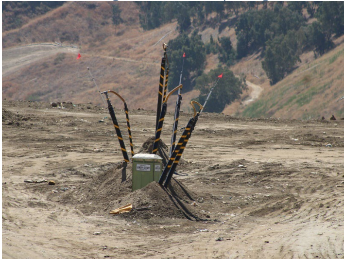
Photo 35: Working Area, CC4 Part 1/2: August 19, 2024
