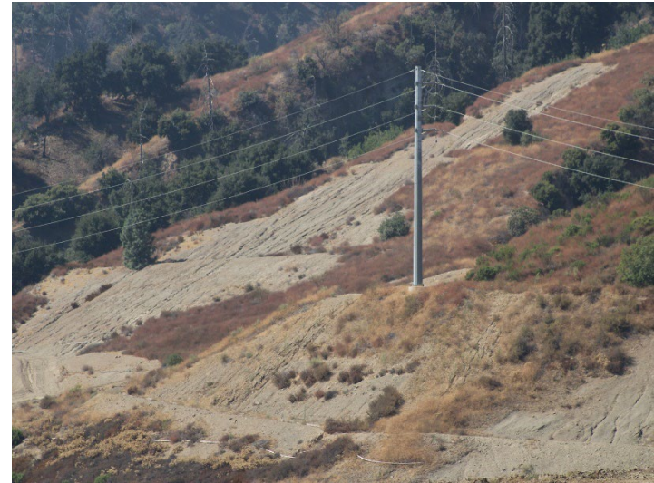
Photo 138: County Sage Mitigation Area and Westside Drainage Channels : September 24, 2024
