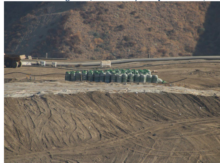
Photo 60: Working Area, CC4 Part 1/2: September 24, 2024
