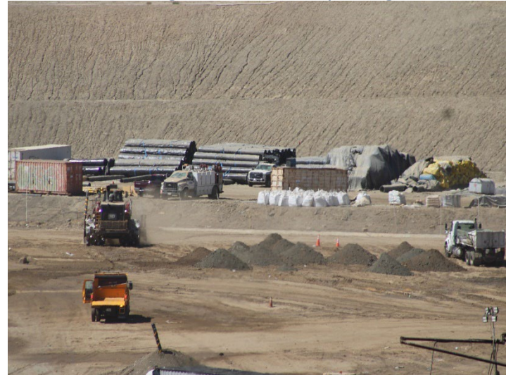
Photo 44: Working Area, CC4 Part 1/2: August 19, 2024
