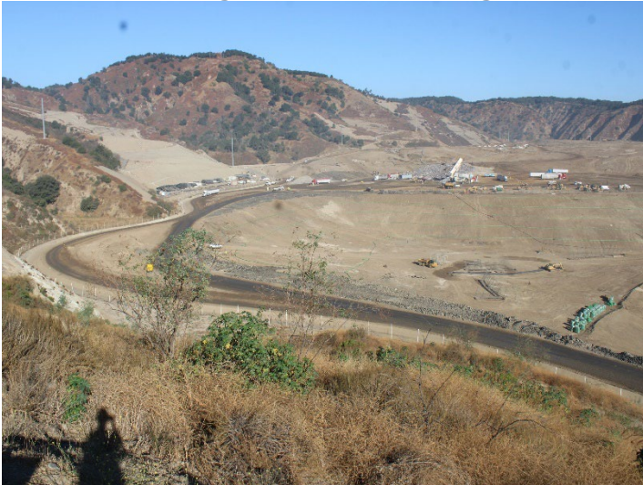
Photo 79: Working Area, CC-4 Part 3: September 24, 2024
