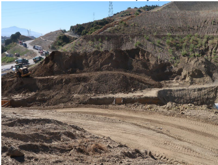
Photo 319: General Site: July 3, 2024
