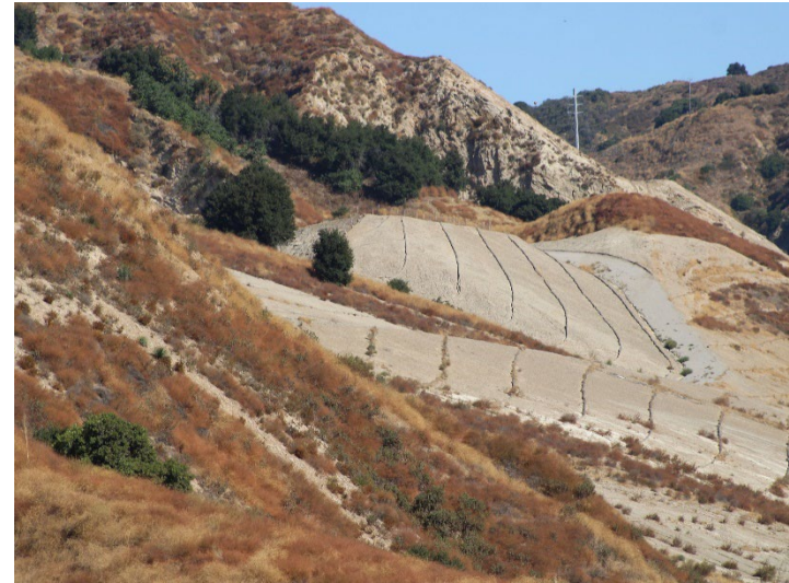
Photo 130: County Sage Mitigation Area and Westside Drainage Channels : August 19, 2024
