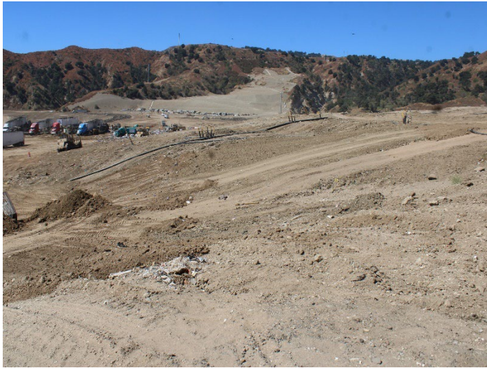
Photo 29: Working Area, CC4 Part 1/2: August 19, 2024
