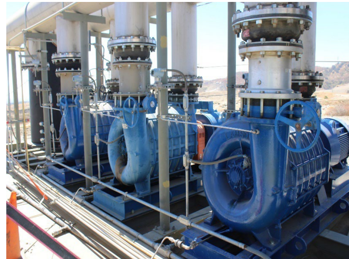
Photo 154: Flares 9, 10, 11 and Gas-to-Energy Facility: August 19, 2024
