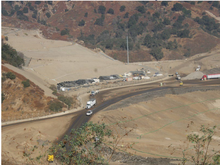
Photo 83: Working Area, CC-4 Part 3: September 24, 2024
