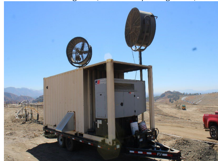
Photo 24: Working Area, CC4 Part 1/2: August 19, 2024
