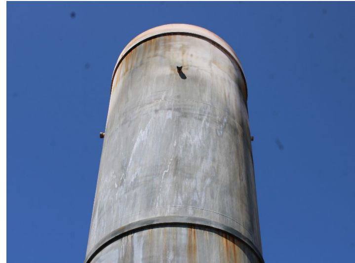
Photo 490: General Site: September 24, 2024
