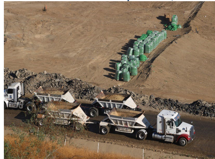
Photo 448: General Site: September 24, 2024
