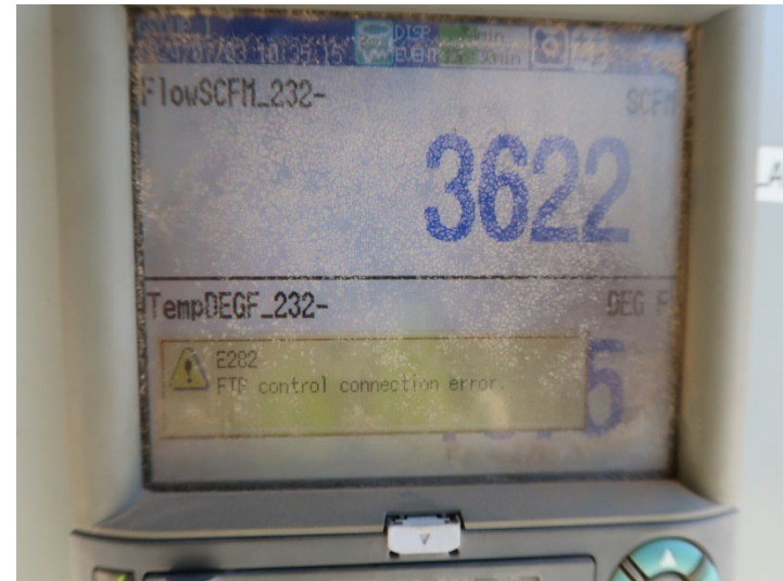
Photo 142: Flares 9, 10, 11 and Gas-to-Energy Facility: July 3, 2024
