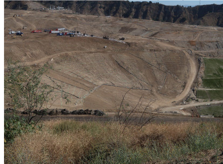
Photo 104: Working Area, CC-4 Part 4/5: July 3, 2024
