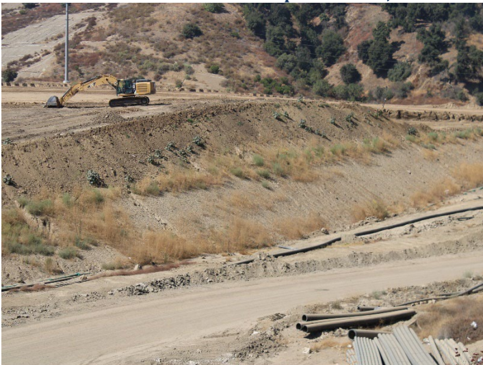
Photo 483: General Site: September 24, 2024
