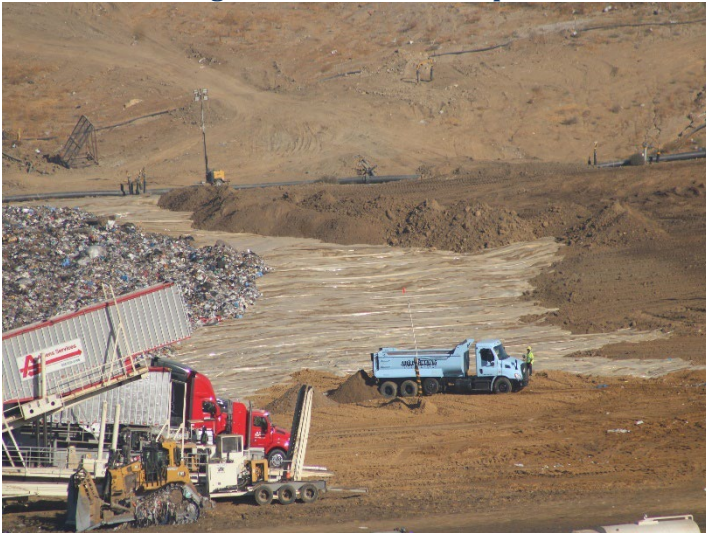
Photo 99: Working Area, CC-4 Part 3: September 24, 2024
