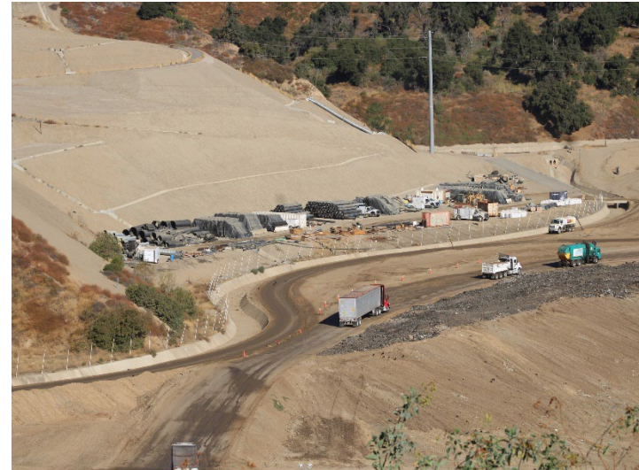
Photo 114: Working Area, CC-4 Part 4/5: August 19, 2024
