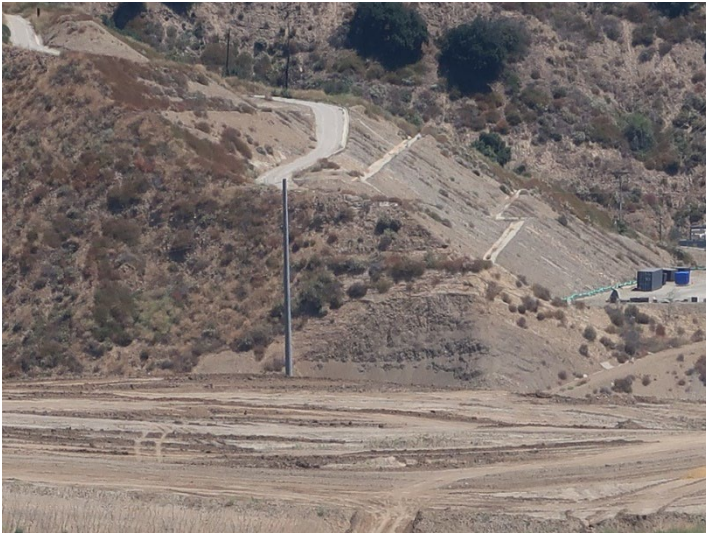
Photo 129: County Sage Mitigation Area and Westside Drainage Channels : July 3, 2024
