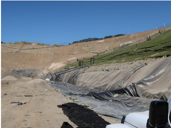
Photo 329: General Site: July 3, 2024
