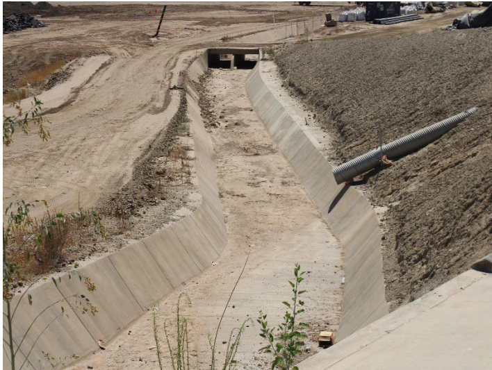
Photo 137: County Sage Mitigation Area and Westside Drainage Channels : August 19, 2024
