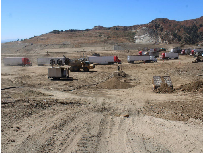
Photo 27: Working Area, CC4 Part 1/2: August 19, 2024
