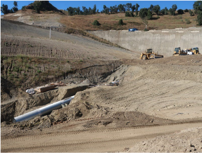
Photo 321: General Site: July 3, 2024
