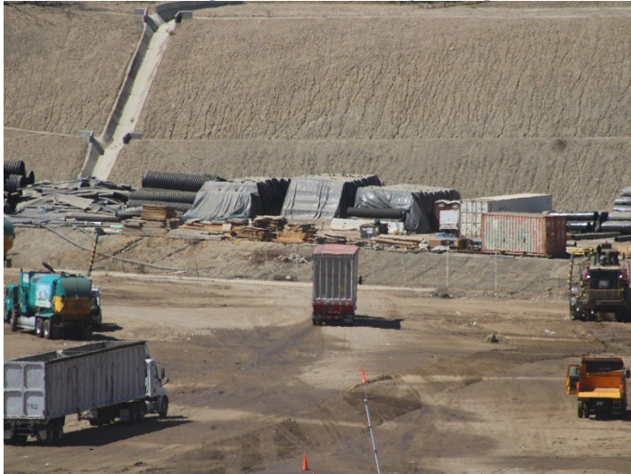
Photo 43: Working Area, CC4 Part 1/2: August 19, 2024
