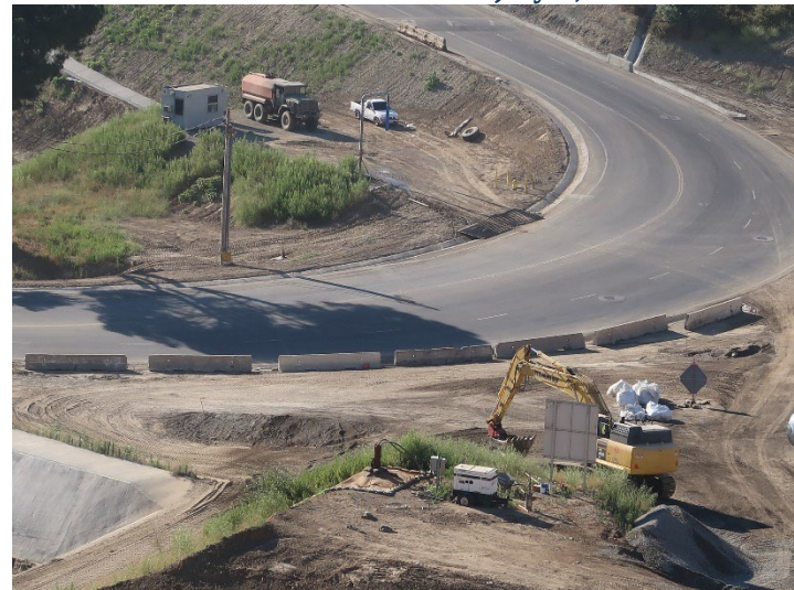
Photo 304: General Site: July 3, 2024
