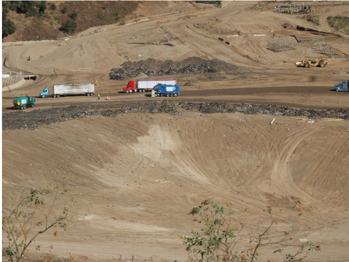
Photo 115: Working Area, CC-4 Part 4/5: August 19, 2024
