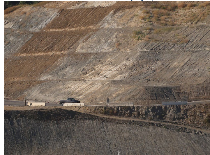
Photo 308: General Site: July 3, 2024
