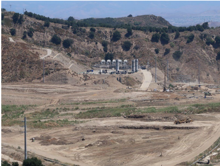
Photo 349: General Site: July 3, 2024
