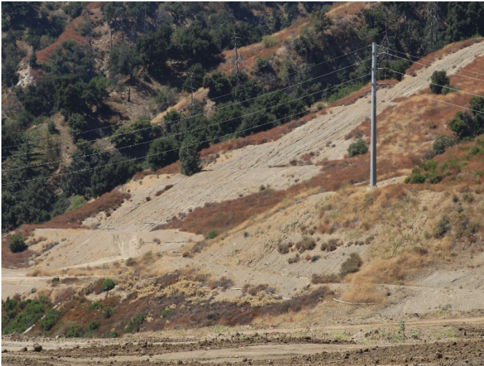
Photo 133: County Sage Mitigation Area and Westside Drainage Channels : August 19, 2024
