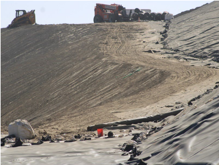
Photo 469: General Site: September 24, 2024
