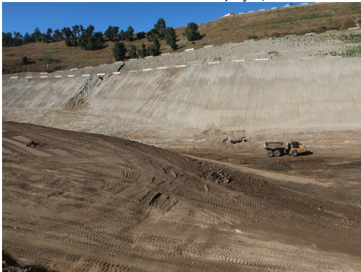
Photo 315: General Site: July 3, 2024
