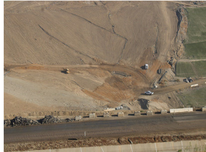
Photo 86: Working Area, CC-4 Part 3: September 24, 2024
