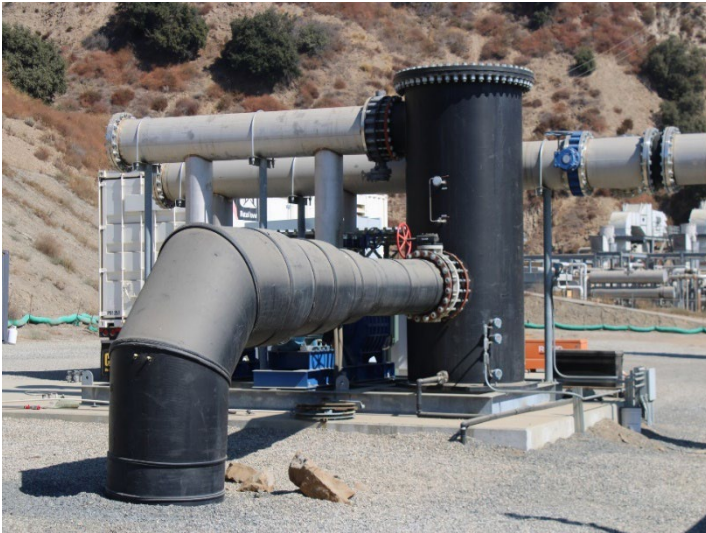
Photo 173: Flares 9, 10, 11 and Gas-to-Energy Facility: September 24, 2024
