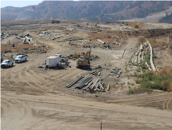
Photo 481: General Site: September 24, 2024
