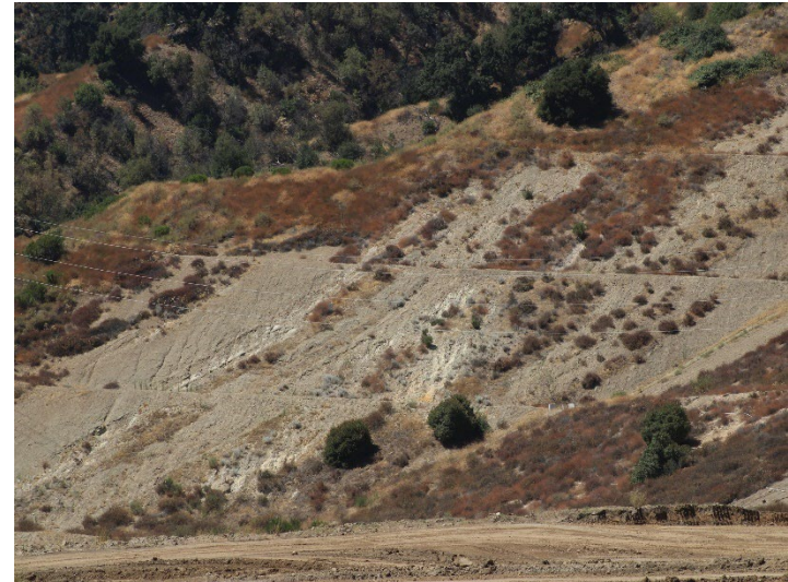
Photo 134: County Sage Mitigation Area and Westside Drainage Channels : August 19, 2024
