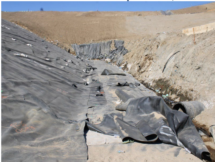
Photo 459: General Site: September 24, 2024
