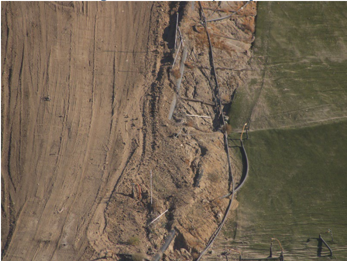
Photo 63: Working Area, CC4 Part 1/2: September 24, 2024
