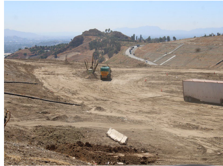
Photo 30: Working Area, CC4 Part 1/2: August 19, 2024
