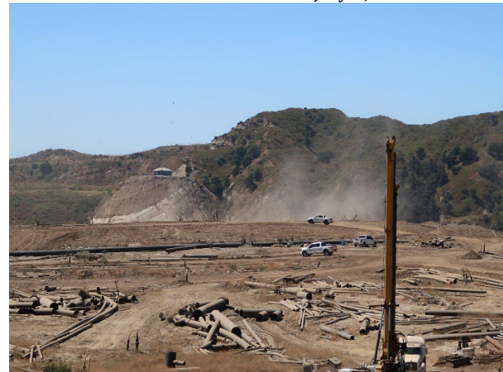
Photo 340: General Site: July 3, 2024
