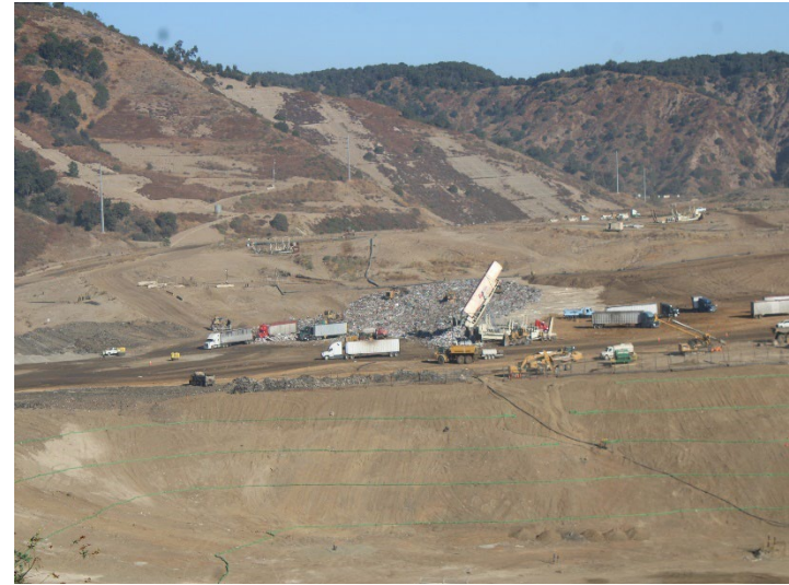
Photo 54: Working Area, CC4 Part 1/2: September 24, 2024
