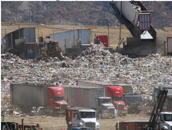
Photo 51: Working Area, CC4 Part 1/2: August 19, 2024
