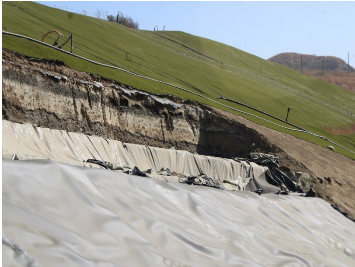
Photo 477: General Site: September 24, 2024
