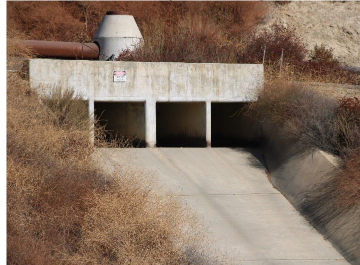
Photo 212: Eastside Drainage Channel: September 24, 2024
