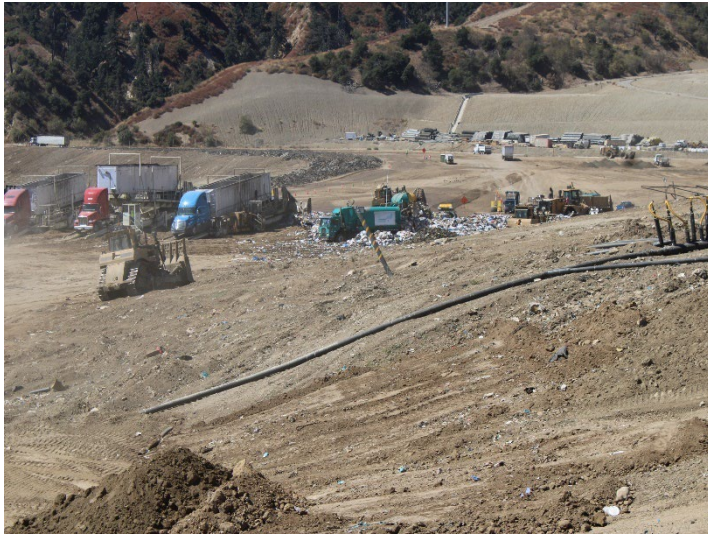
Photo 33: Working Area, CC4 Part 1/2: August 19, 2024
