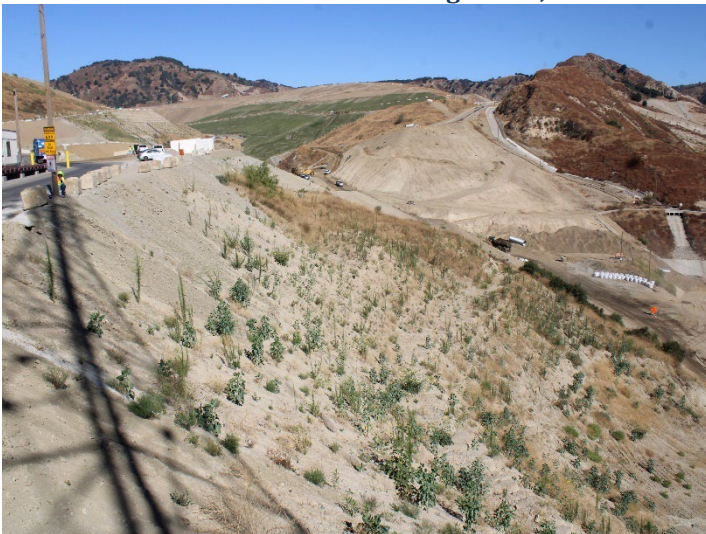
Photo 367: General Site: August 19, 2024
