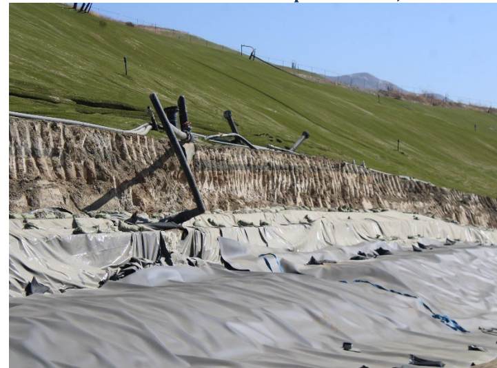
Photo 476: General Site: September 24, 2024
