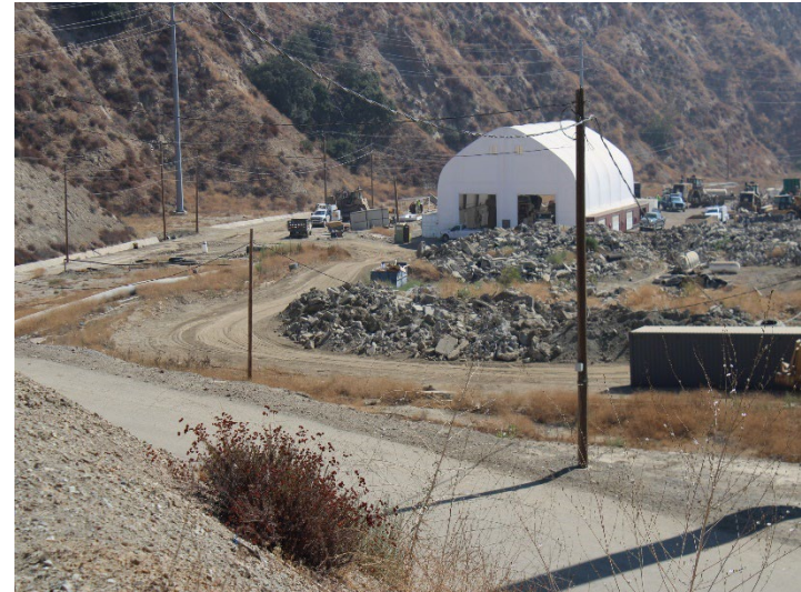
Photo 478: General Site: September 24, 2024
