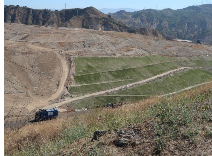
Photo 116: Closure Turf: July 3, 2024
