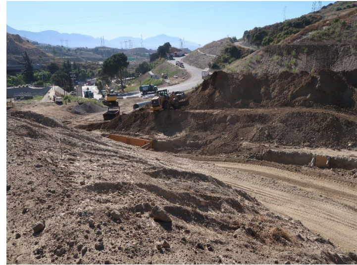
Photo 318: General Site: July 3, 2024
