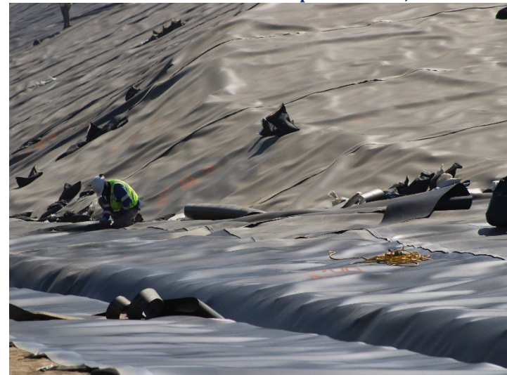
Photo 468: General Site: September 24, 2024
