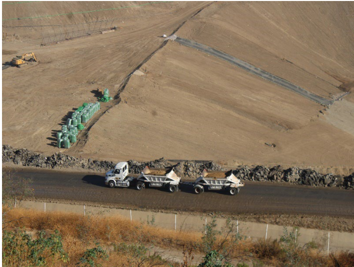
Photo 85: Working Area, CC-4 Part 3: September 24, 2024
