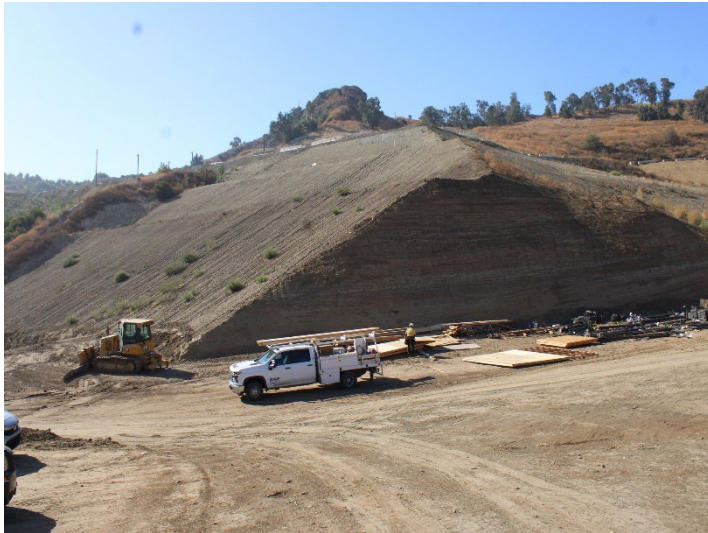
Photo 453: General Site: September 24, 2024
