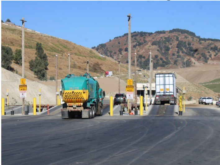
Photo 127: Office and Scales Location: August 19, 2024
