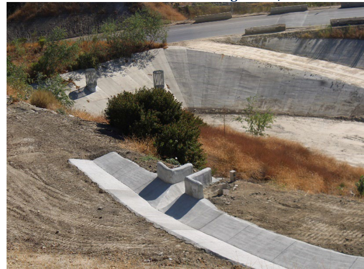
Photo 356: General Site: August 19, 2024
