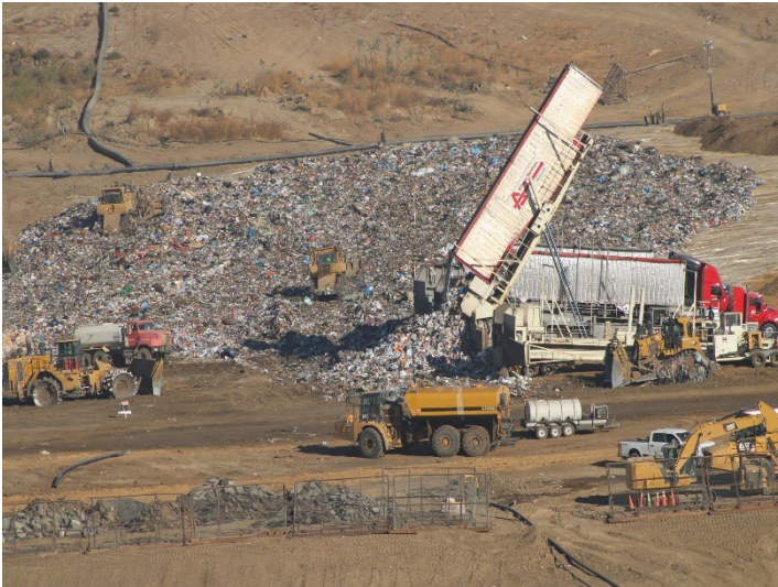
Photo 93: Working Area, CC-4 Part 3: September 24, 2024
