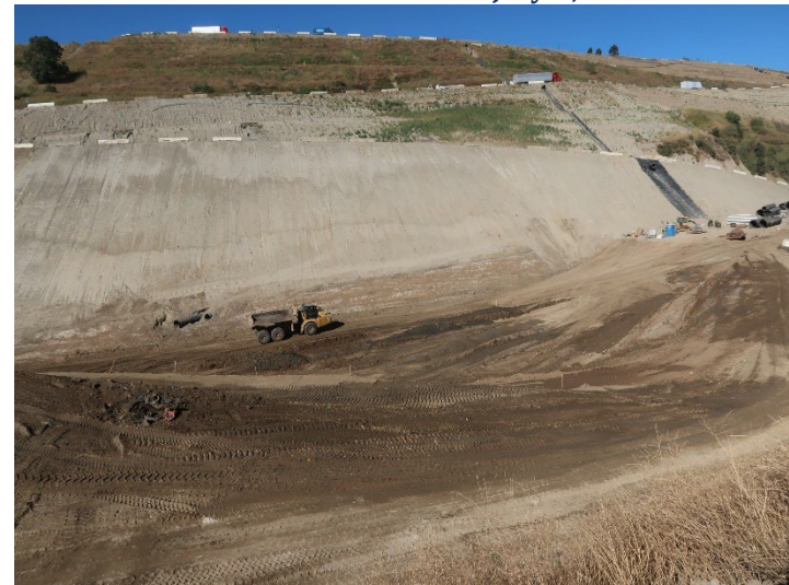
Photo 316: General Site: July 3, 2024
