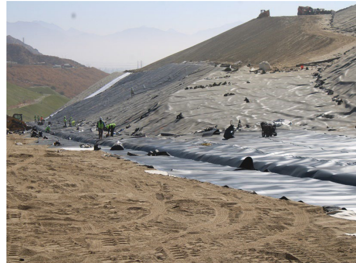
Photo 466: General Site: September 24, 2024
