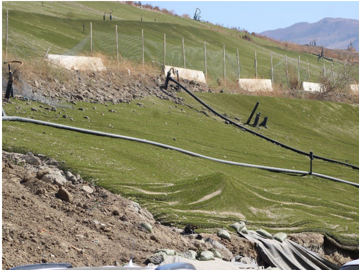
Photo 473: General Site: September 24, 2024
