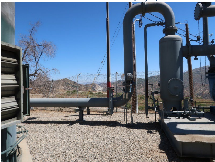
Photo 343: General Site: July 3, 2024
