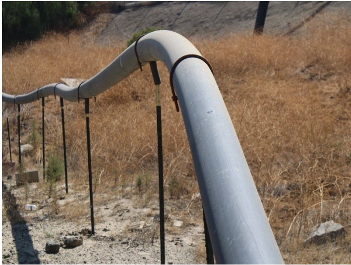
Photo 493: General Site: September 24, 2024
