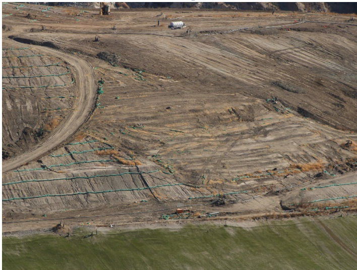
Photo 19: Working Area, CC4 Part 1/2: August 19, 2024
