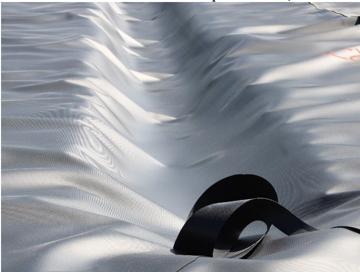
Photo 471: General Site: September 24, 2024
