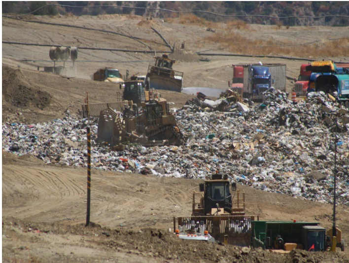
Photo 49: Working Area, CC4 Part 1/2: August 19, 2024
