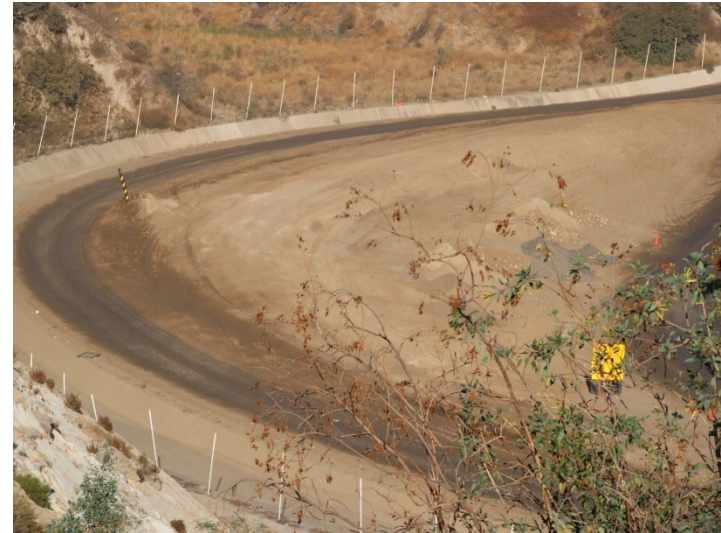
Photo 446: General Site: September 24, 2024
