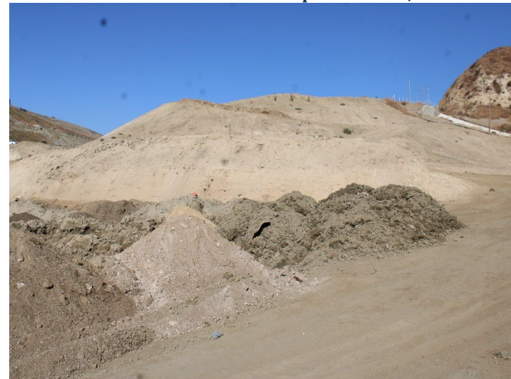
Photo 456: General Site: September 24, 2024
