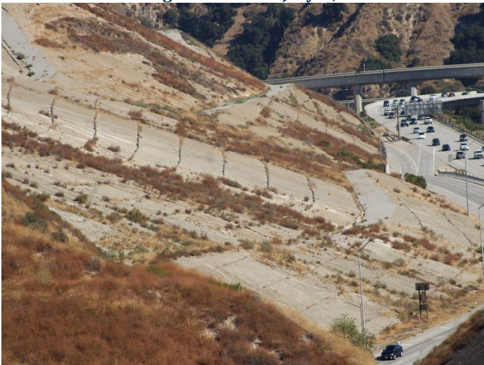
Photo 131: County Sage Mitigation Area and Westside Drainage Channels : August 19, 2024
