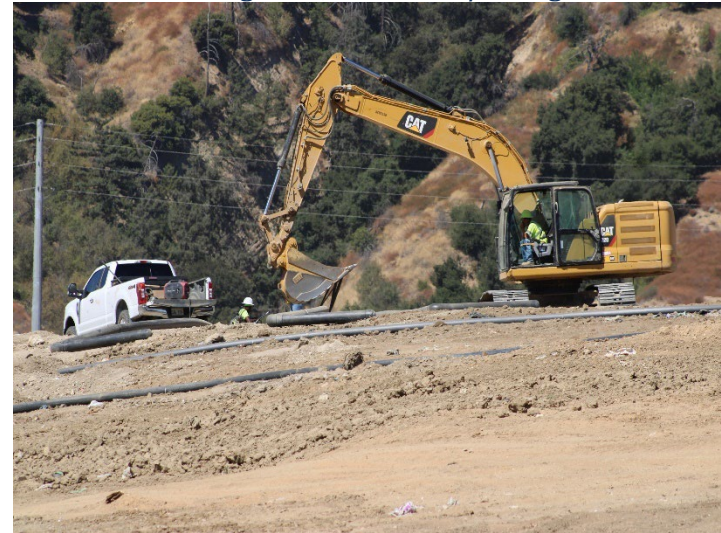
Photo 40: Working Area, CC4 Part 1/2: August 19, 2024
