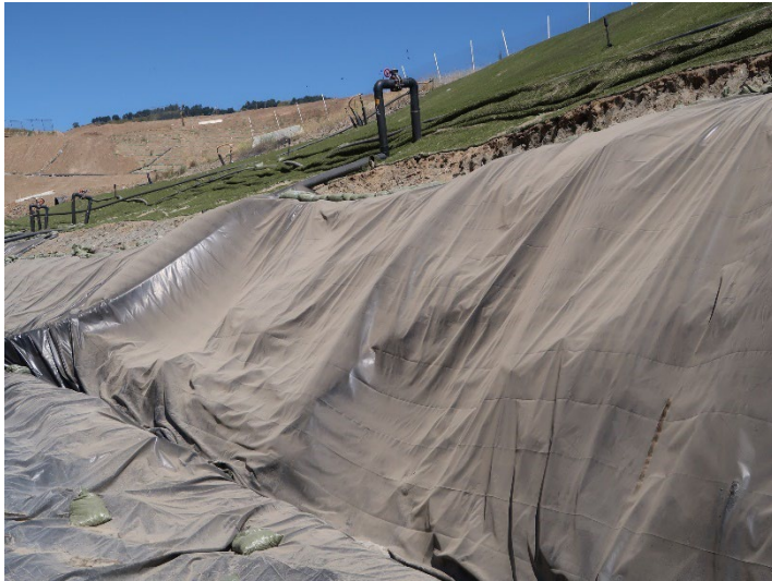
Photo 325: General Site: July 3, 2024
