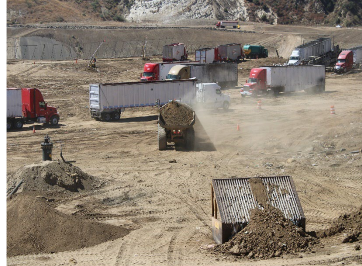
Photo 32: Working Area, CC4 Part 1/2: August 19, 2024
