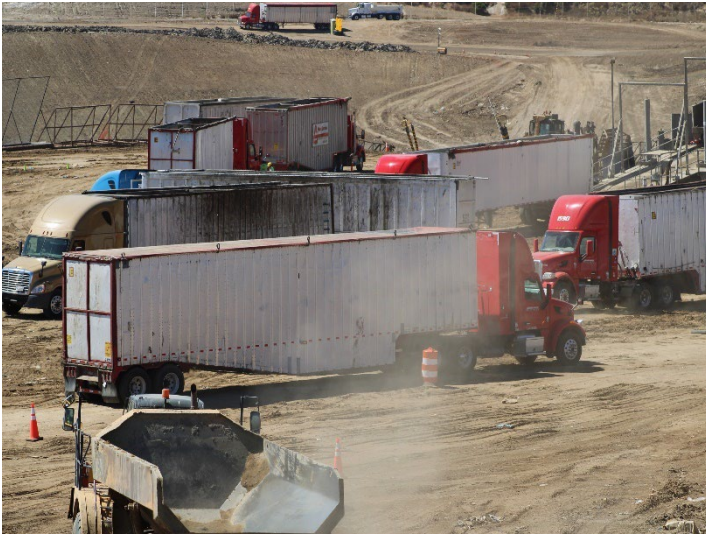
Photo 37: Working Area, CC4 Part 1/2: August 19, 2024
