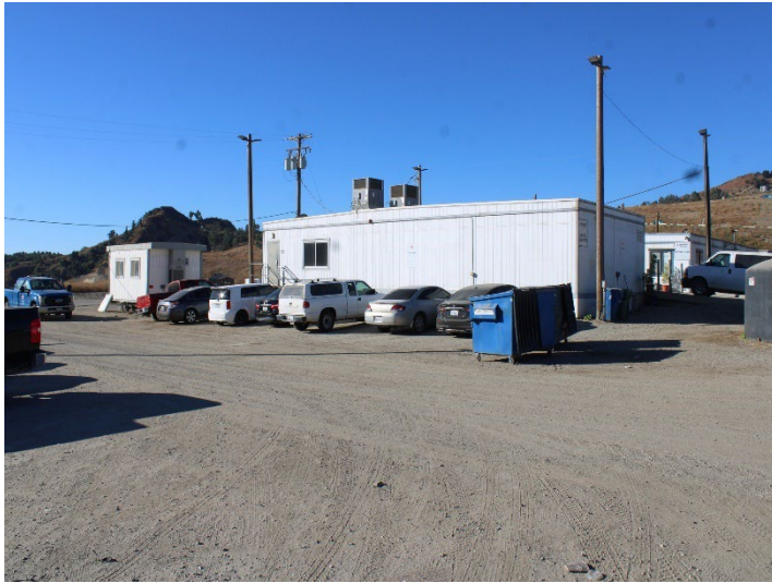
Photo 125: Office and Scales Location: August 19, 2024
