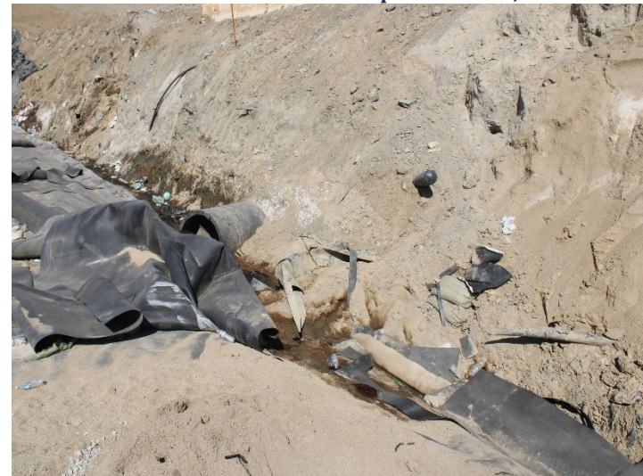
Photo 460: General Site: September 24, 2024
