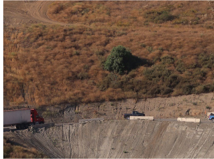
Photo 310: General Site: July 3, 2024
