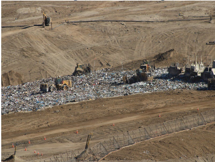
Photo 67: Working Area, CC-4 Part 3: August 19, 2024
