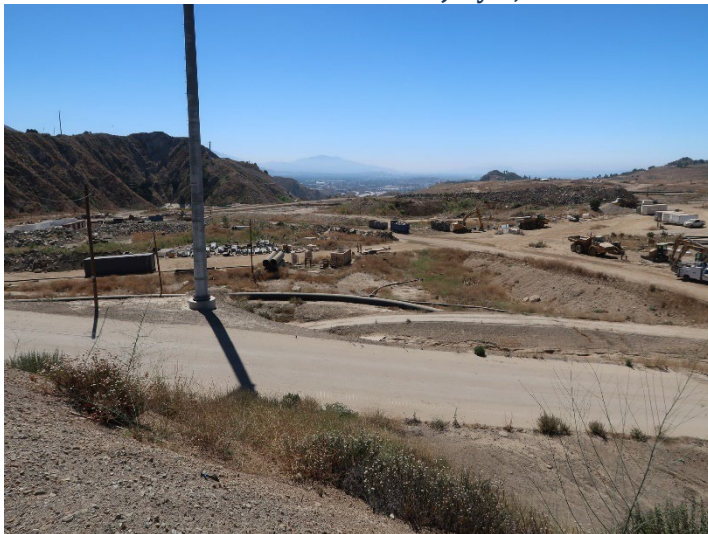
Photo 335: General Site: July 3, 2024
