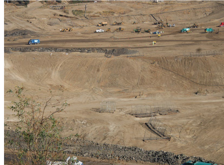
Photo 112: Working Area, CC-4 Part 4/5: August 19, 2024
