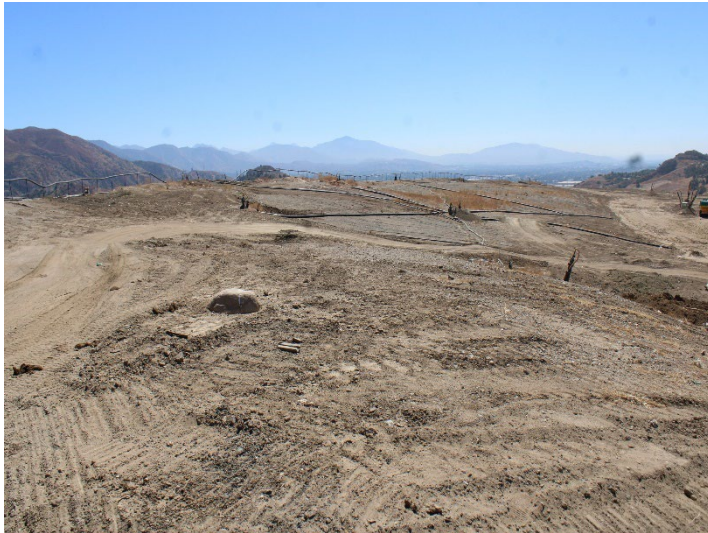
Photo 25: Working Area, CC4 Part 1/2: August 19, 2024
