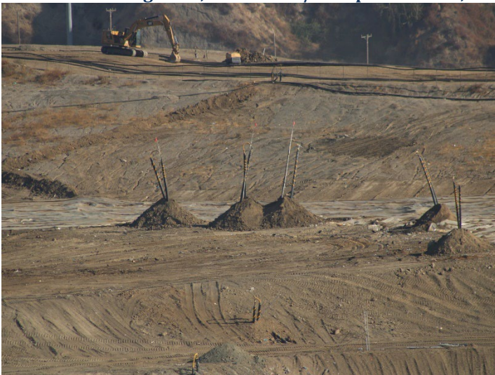
Photo 59: Working Area, CC4 Part 1/2: September 24, 2024
