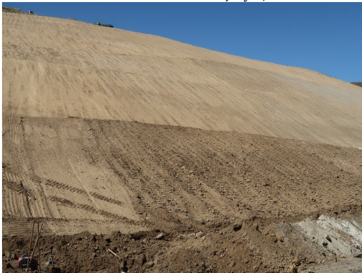
Photo 327: General Site: July 3, 2024
