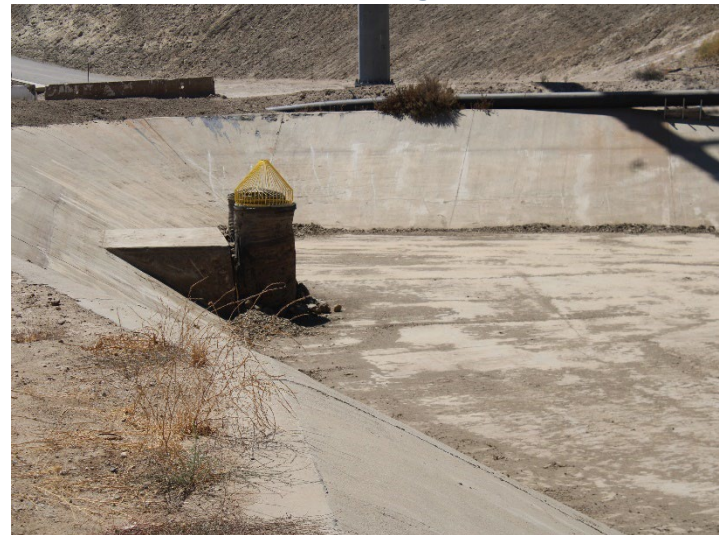
Photo 12: Basin A: August 19, 2024
