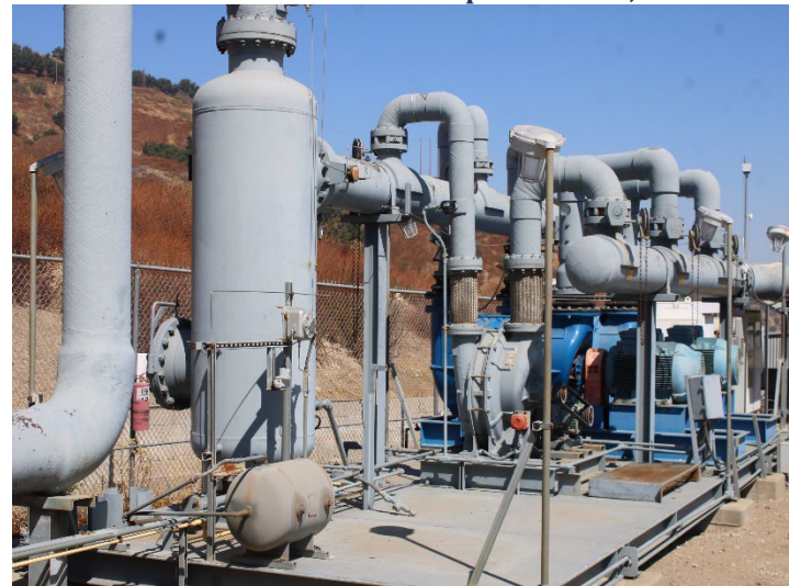
Photo 488: General Site: September 24, 2024
