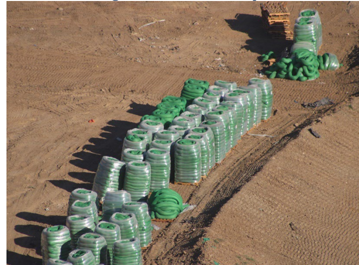
Photo 100: Working Area, CC-4 Part 3: September 24, 2024
