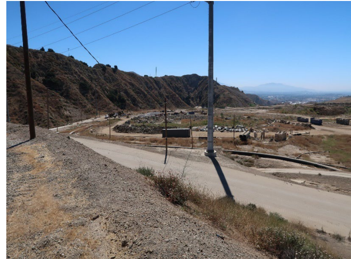
Photo 334: General Site: July 3, 2024
