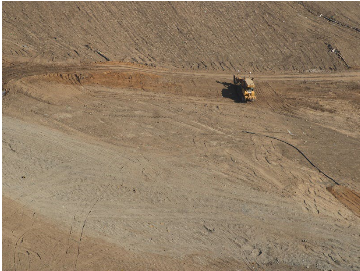
Photo 89: Working Area, CC-4 Part 3: September 24, 2024
