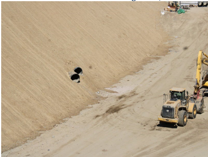
Photo 403: General Site: August 19, 2024
