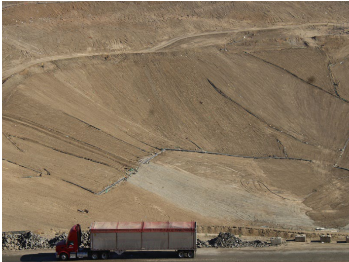
Photo 113: Working Area, CC-4 Part 4/5: August 19, 2024
