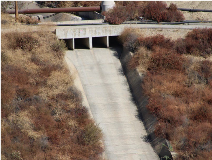
Photo 209: Eastside Drainage Channel: August 19, 2024
