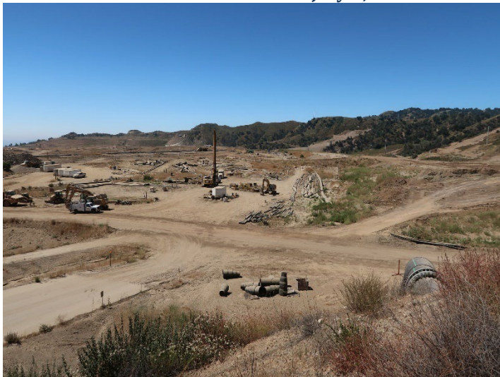
Photo 339: General Site: July 3, 2024
