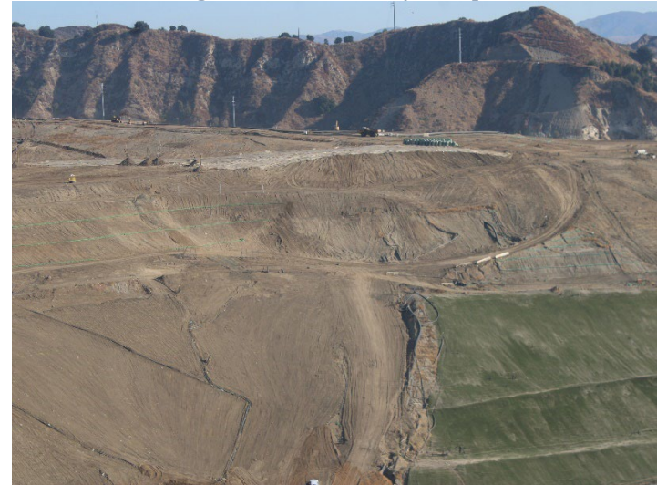
Photo 56: Working Area, CC4 Part 1/2: September 24, 2024
