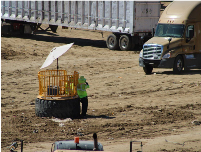
Photo 41: Working Area, CC4 Part 1/2: August 19, 2024
