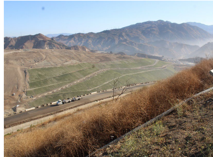
Photo 82: Working Area, CC-4 Part 3: September 24, 2024
