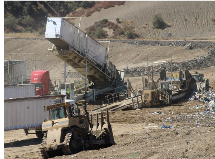
Photo 38: Working Area, CC4 Part 1/2: August 19, 2024
