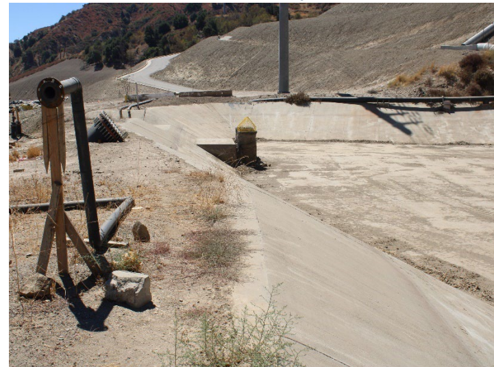
Photo 8: Basin A: August 19, 2024
