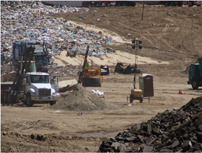
Photo 53: Working Area, CC4 Part 1/2: August 19, 2024
