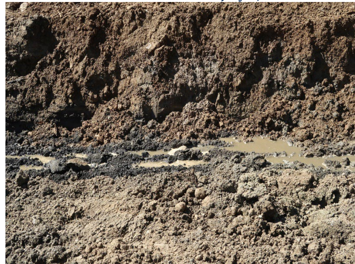
Photo 332: General Site: July 3, 2024
