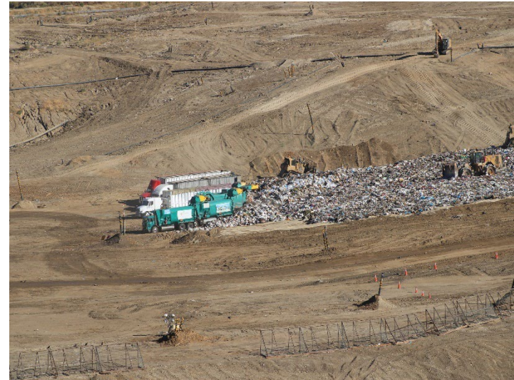
Photo 66: Working Area, CC-4 Part 3: August 19, 2024
