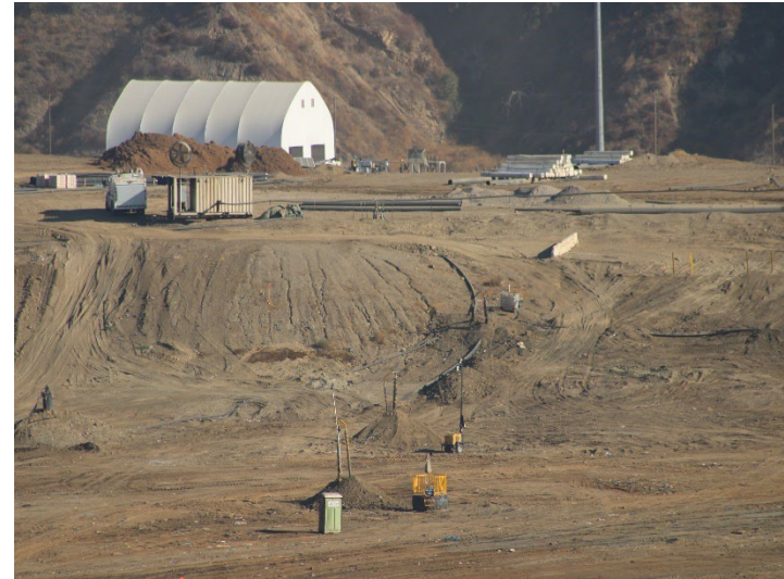
Photo 58: Working Area, CC4 Part 1/2: September 24, 2024
