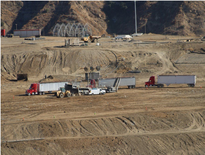
Photo 69: Working Area, CC-4 Part 3: August 19, 2024
