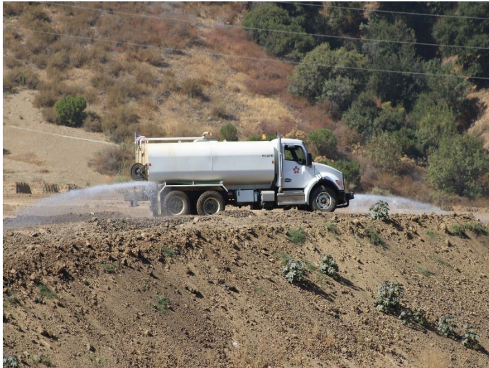
Photo 485: General Site: September 24, 2024
