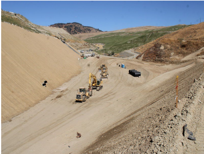
Photo 401: General Site: August 19, 2024
