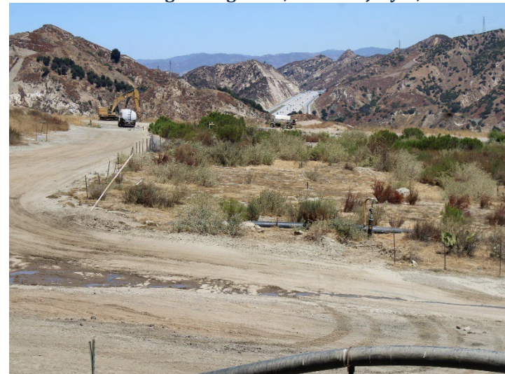
Photo 288: Sage Mitigation, Deck B: August 19, 2024
