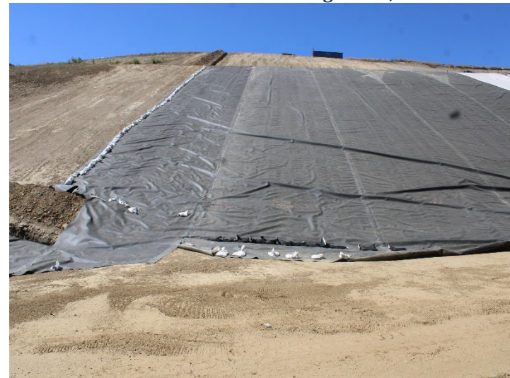
Photo 420: General Site: August 19, 2024
