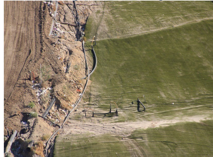
Photo 76: Working Area, CC-4 Part 3: August 19, 2024
