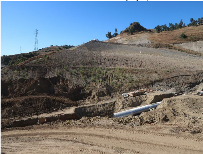
Photo 323: General Site: July 3, 2024
