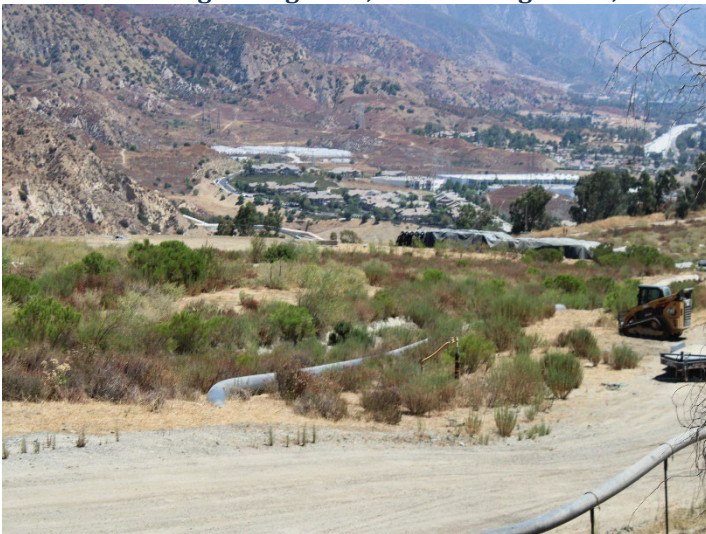
Photo 291: Sage Mitigation, Deck B: August 19, 2024
