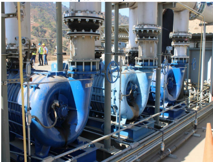
Photo 167: Flares 9, 10, 11 and Gas-to-Energy Facility: September 24, 2024
