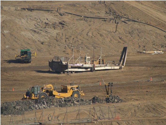
Photo 57: Working Area, CC4 Part 1/2: September 24, 2024
