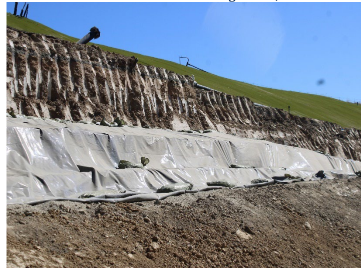
Photo 416: General Site: August 19, 2024
