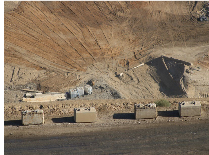
Photo 90: Working Area, CC-4 Part 3: September 24, 2024
