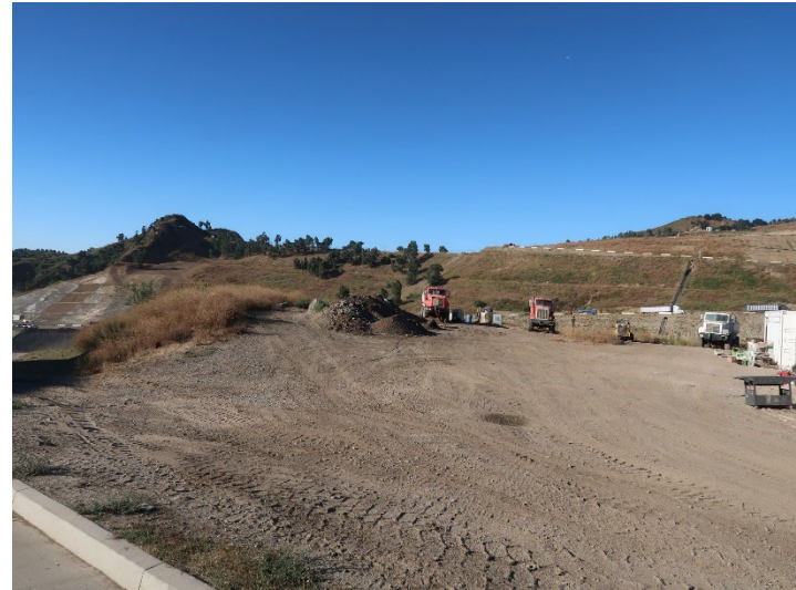
Photo 298: General Site: July 3, 2024
