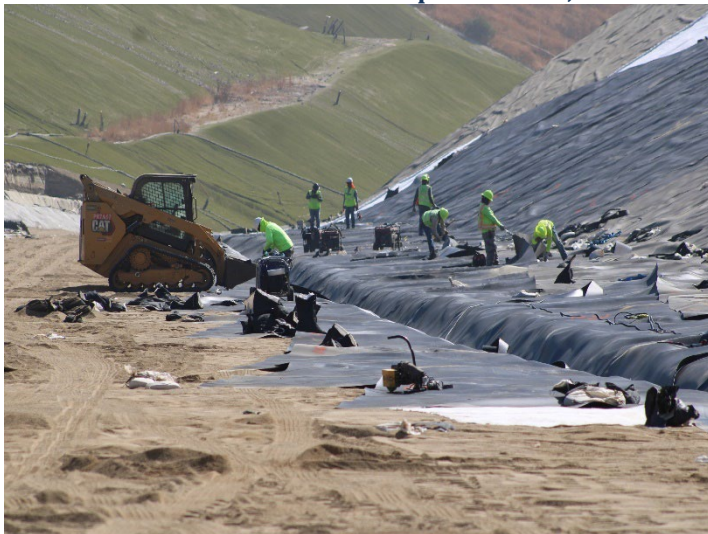
Photo 467: General Site: September 24, 2024
