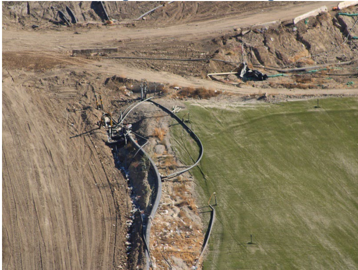
Photo 75: Working Area, CC-4 Part 3: August 19, 2024
