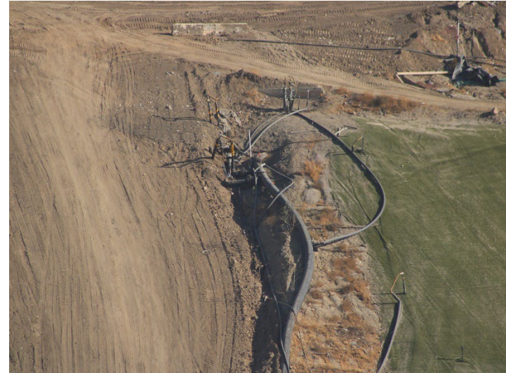
Photo 62: Working Area, CC4 Part 1/2: September 24, 2024
