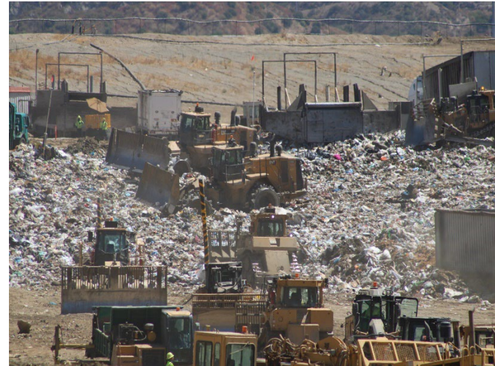
Photo 50: Working Area, CC4 Part 1/2: August 19, 2024
