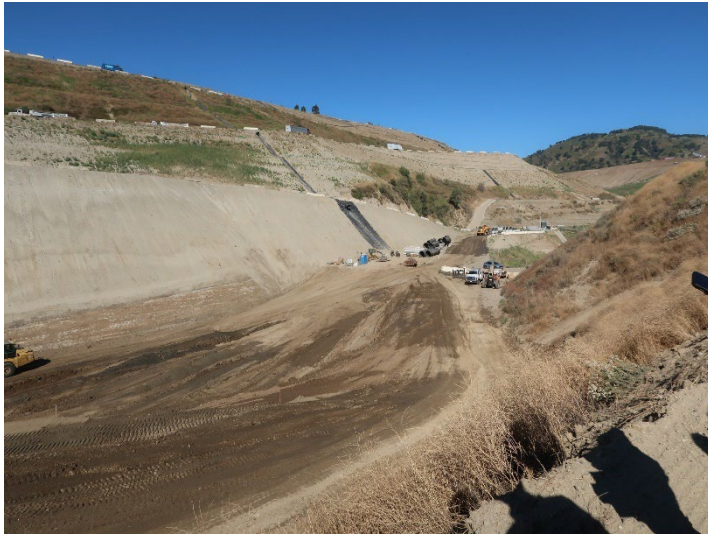
Photo 317: General Site: July 3, 2024
