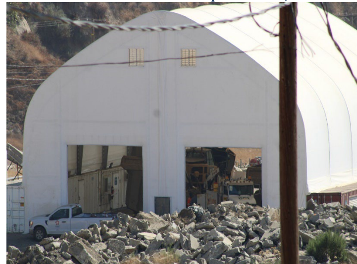
Photo 484: General Site: September 24, 2024
