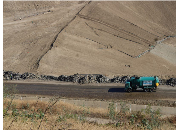
Photo 110: Working Area, CC-4 Part 4/5: August 19, 2024
