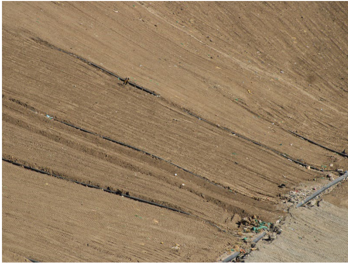
Photo 73: Working Area, CC-4 Part 3: August 19, 2024
