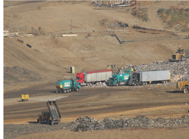
Photo 92: Working Area, CC-4 Part 3: September 24, 2024
