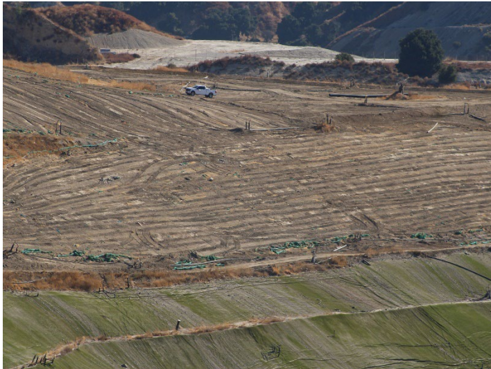
Photo 21: Working Area, CC4 Part 1/2: August 19, 2024
