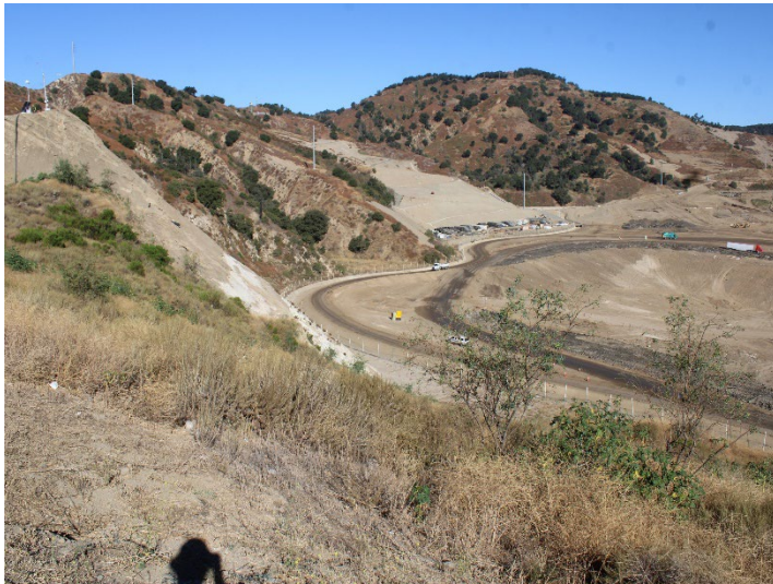
Photo 105: Working Area, CC-4 Part 4/5: August 19, 2024
