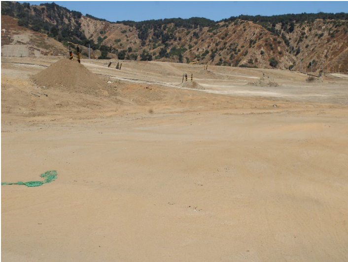
Photo 181: County Top Deck: August 19, 2024
