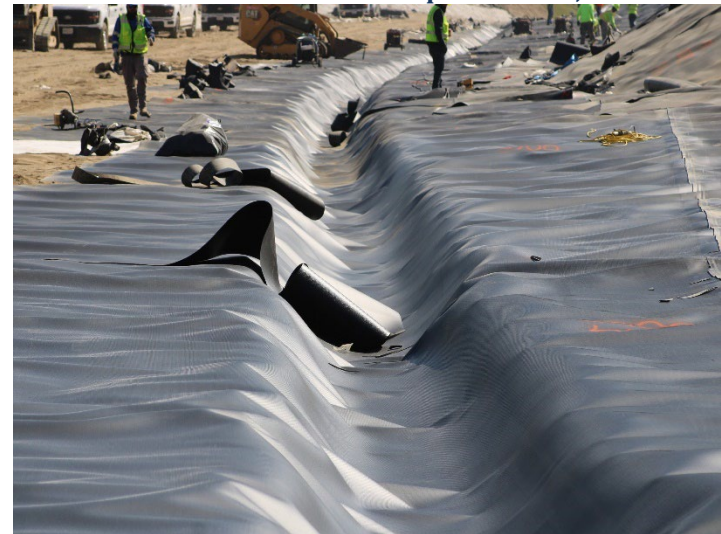
Photo 472: General Site: September 24, 2024
