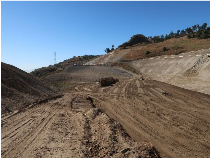
Photo 313: General Site: July 3, 2024
