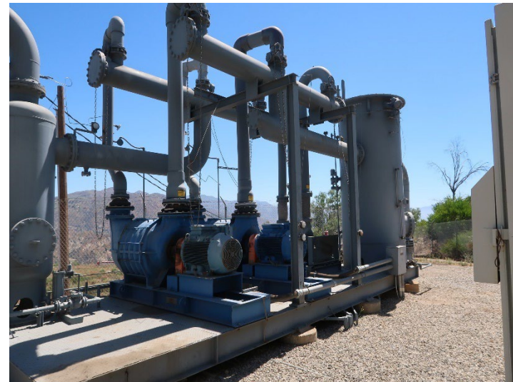
Photo 342: General Site: July 3, 2024
