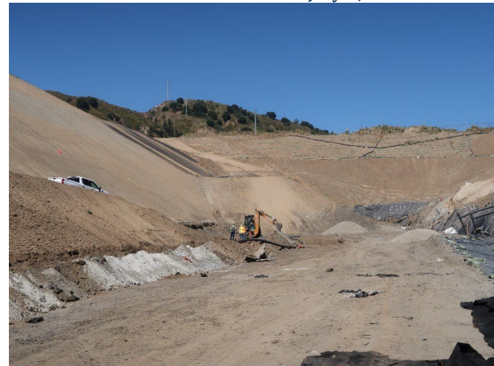
Photo 328: General Site: July 3, 2024
