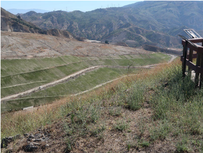
Photo 117: Closure Turf: July 3, 2024
