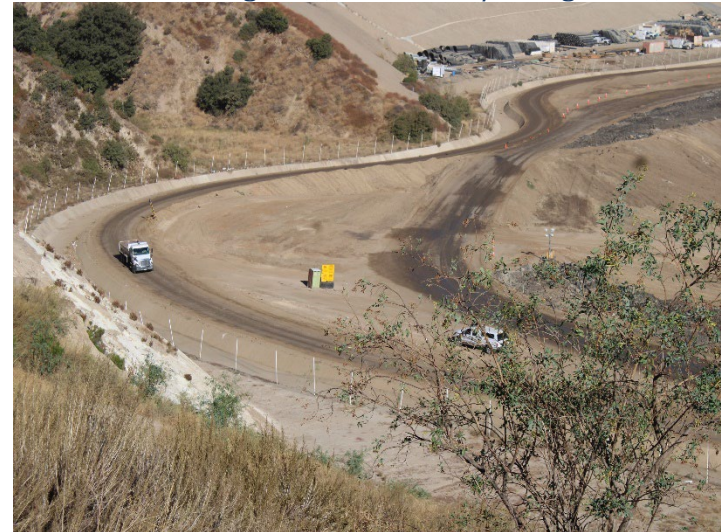
Photo 108: Working Area, CC-4 Part 4/5: August 19, 2024
