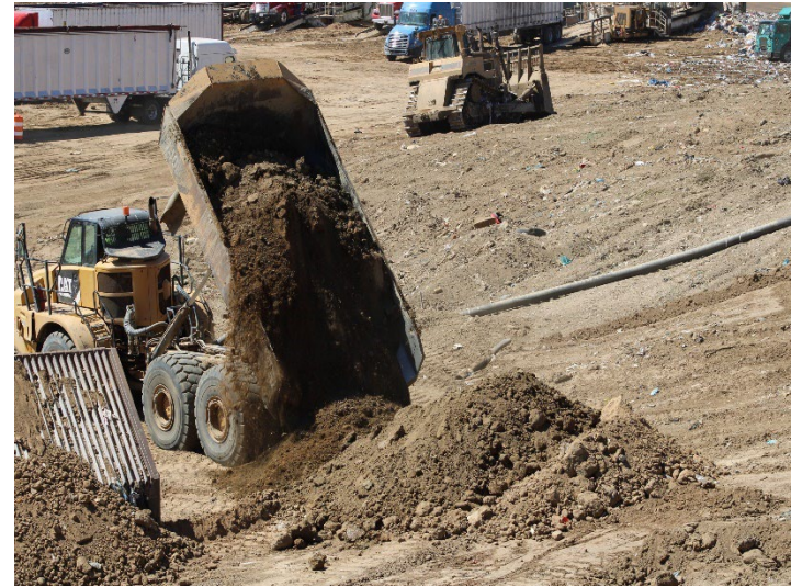
Photo 34: Working Area, CC4 Part 1/2: August 19, 2024
