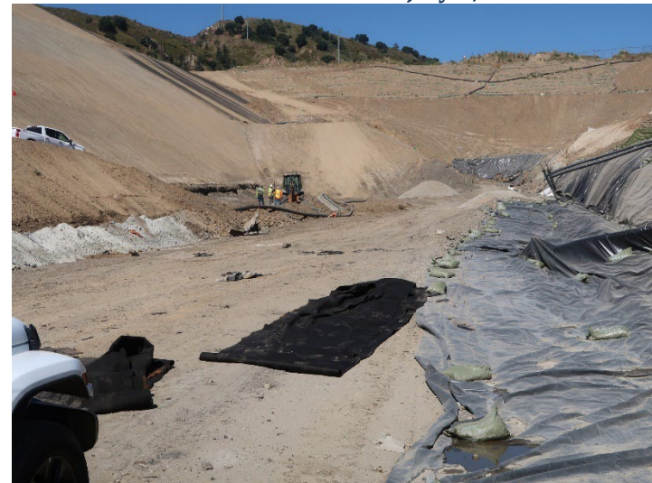
Photo 324: General Site: July 3, 2024
