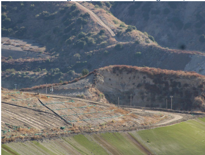
Photo 23: Working Area, CC4 Part 1/2: August 19, 2024
