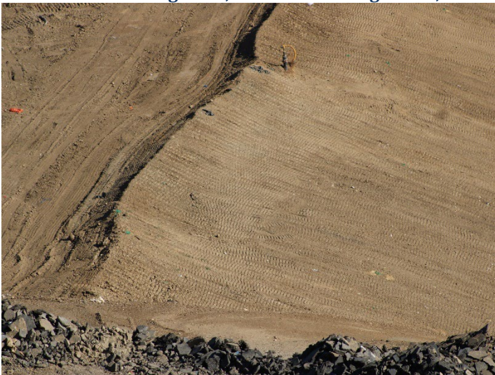
Photo 71: Working Area, CC-4 Part 3: August 19, 2024
