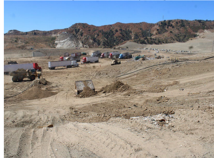
Photo 28: Working Area, CC4 Part 1/2: August 19, 2024
