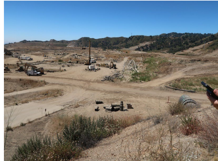
Photo 338: General Site: July 3, 2024
