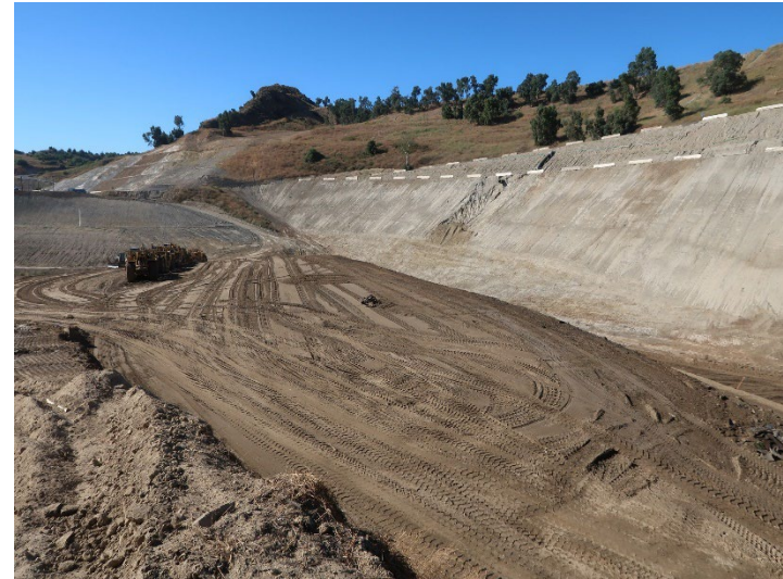
Photo 314: General Site: July 3, 2024
