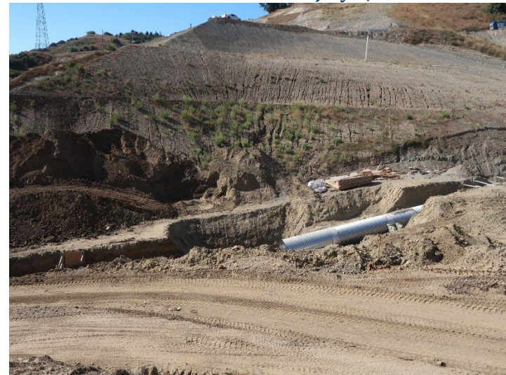
Photo 320: General Site: July 3, 2024
