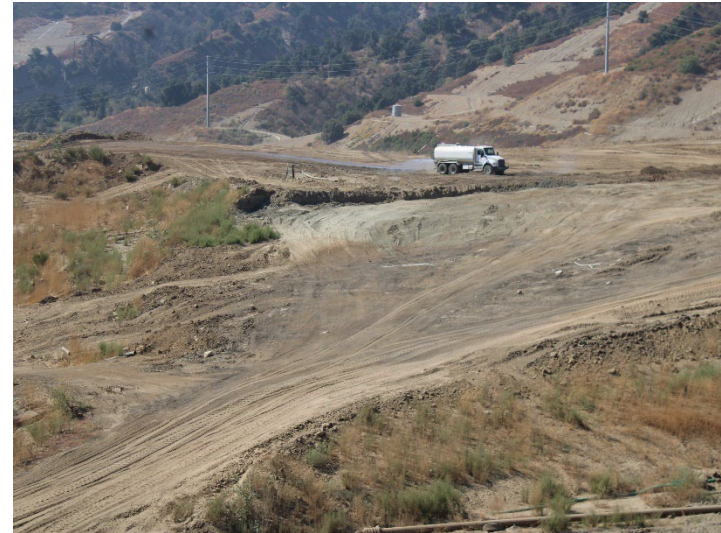
Photo 482: General Site: September 24, 2024
