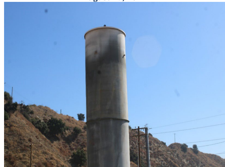
Photo 160: Flares 9, 10, 11 and Gas-to-Energy Facility: September 24, 2024
