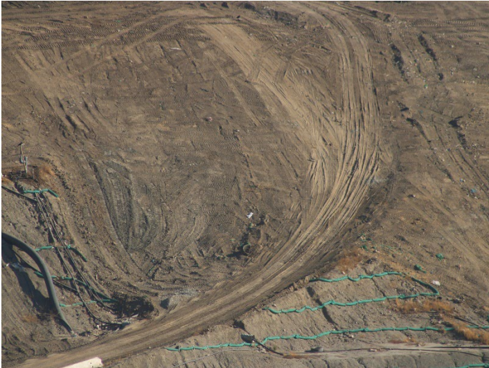
Photo 61: Working Area, CC4 Part 1/2: September 24, 2024
