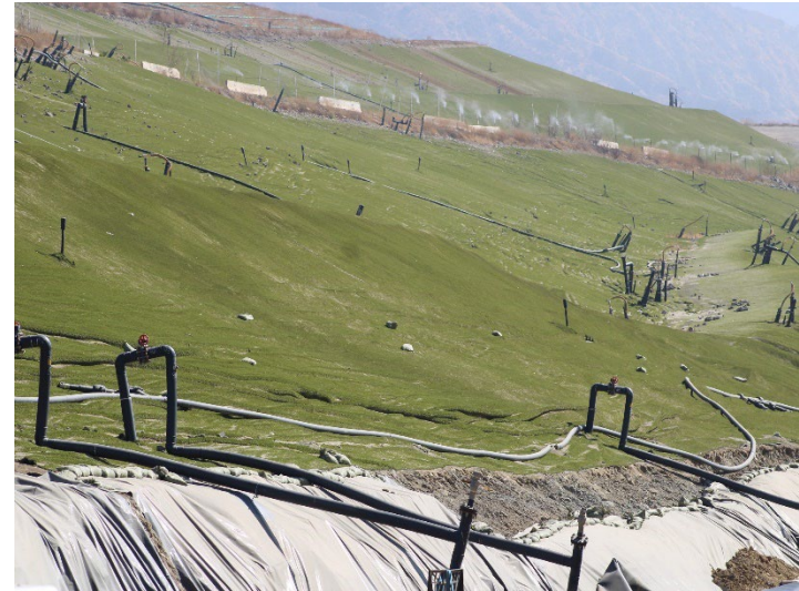
Photo 474: General Site: September 24, 2024
