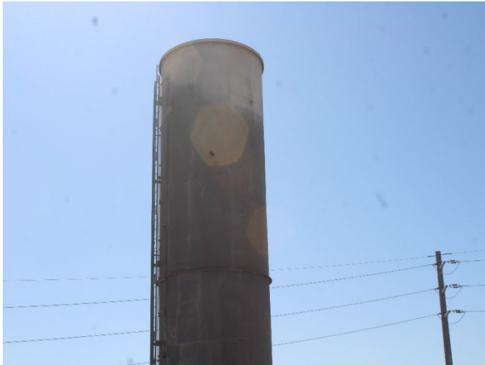
Photo 161: Flares 9, 10, 11 and Gas-to-Energy Facility: September 24, 2024
