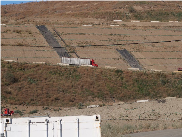
Photo 301: General Site: July 3, 2024
