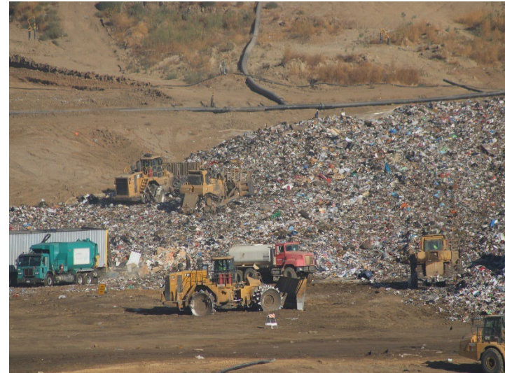
Photo 98: Working Area, CC-4 Part 3: September 24, 2024
