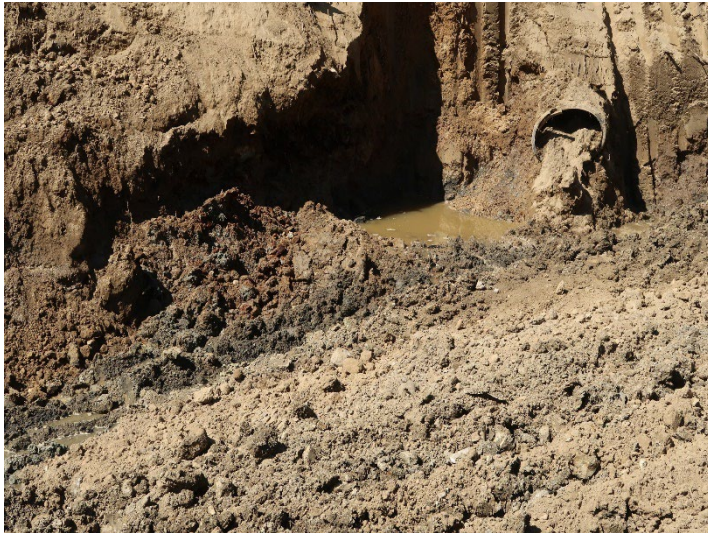
Photo 333: General Site: July 3, 2024
