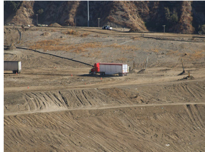
Photo 70: Working Area, CC-4 Part 3: August 19, 2024
