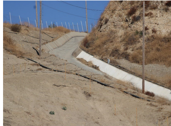
Photo 210: Eastside Drainage Channel: September 24, 2024
