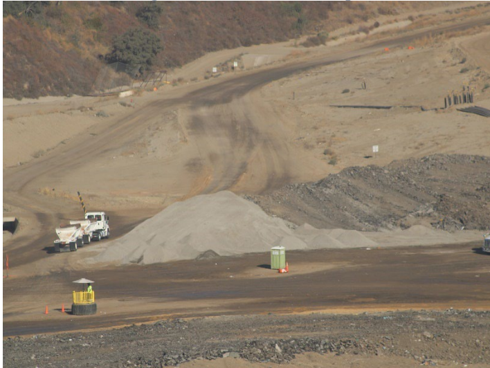
Photo 91: Working Area, CC-4 Part 3: September 24, 2024
