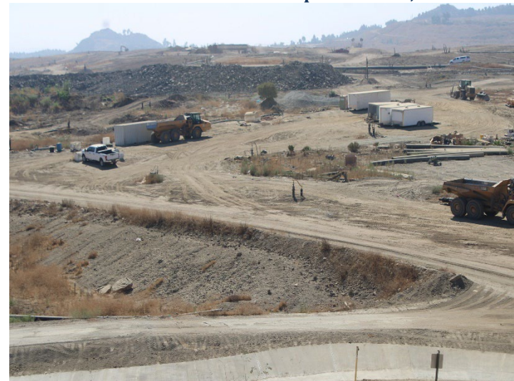
Photo 480: General Site: September 24, 2024
