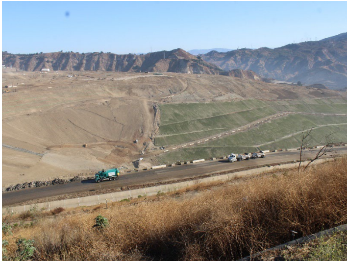
Photo 81: Working Area, CC-4 Part 3: September 24, 2024
