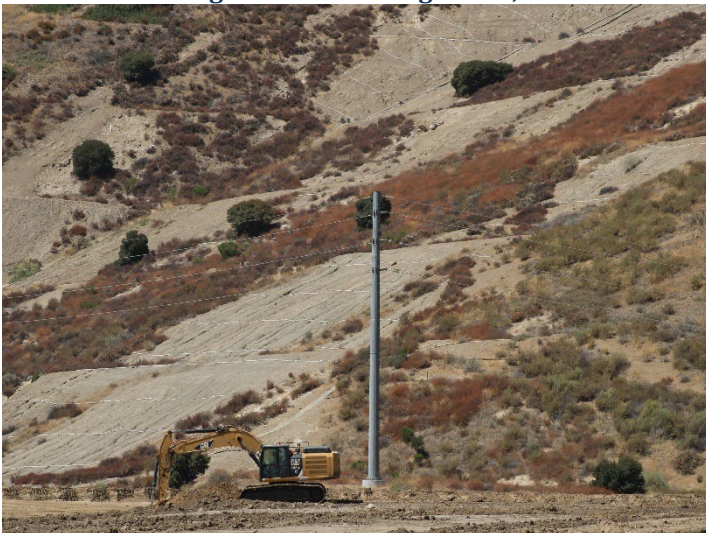
Photo 135: County Sage Mitigation Area and Westside Drainage Channels : August 19, 2024
