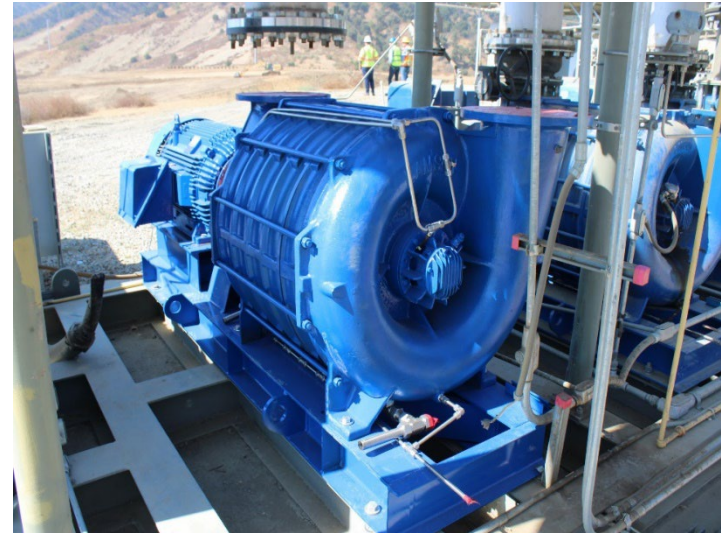
Photo 166: Flares 9, 10, 11 and Gas-to-Energy Facility: September 24, 2024
