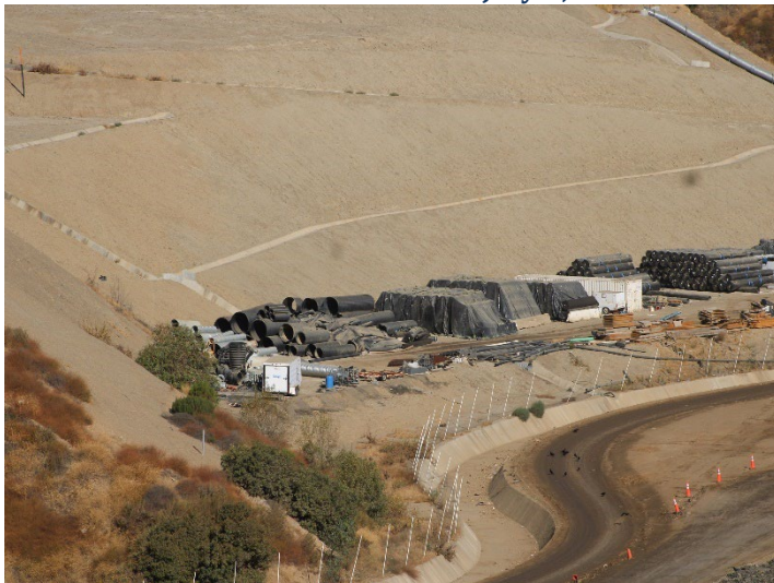
Photo 351: General Site: August 19, 2024
