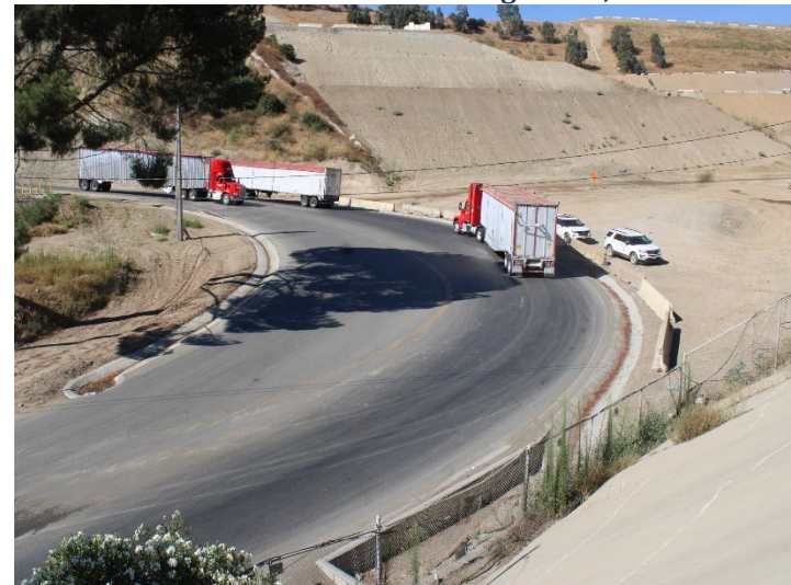
Photo 380: General Site: August 19, 2024
