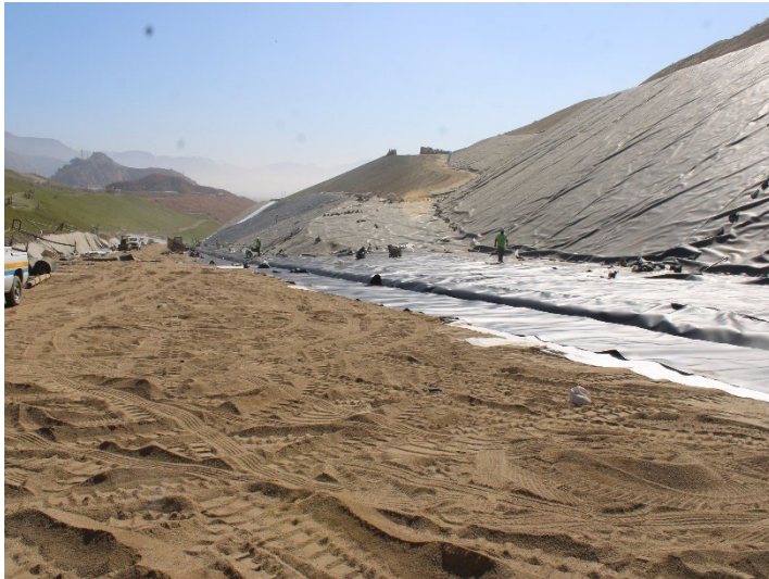
Photo 465: General Site: September 24, 2024
