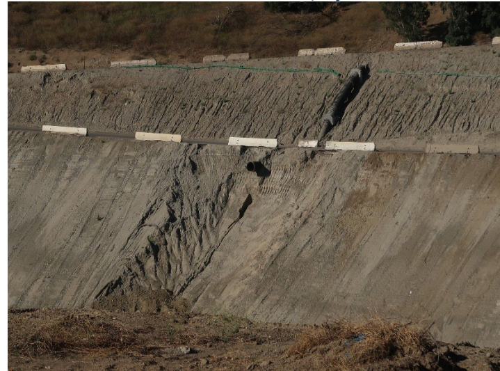
Photo 312: General Site: July 3, 2024
