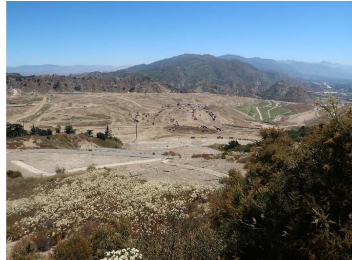
Photo 346: General Site: July 3, 2024
