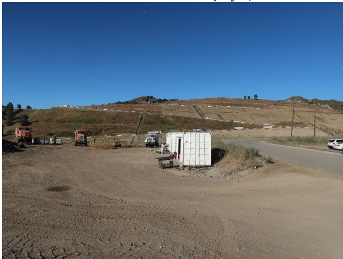
Photo 299: General Site: July 3, 2024
