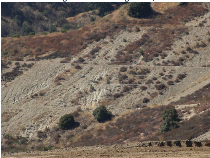
Photo 139: County Sage Mitigation Area and Westside Drainage Channels : September 24, 2024
