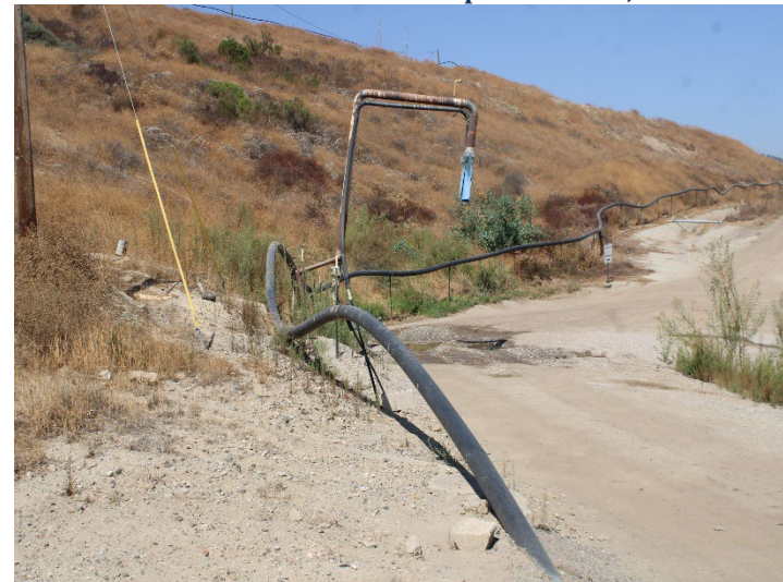
Photo 492: General Site: September 24, 2024
