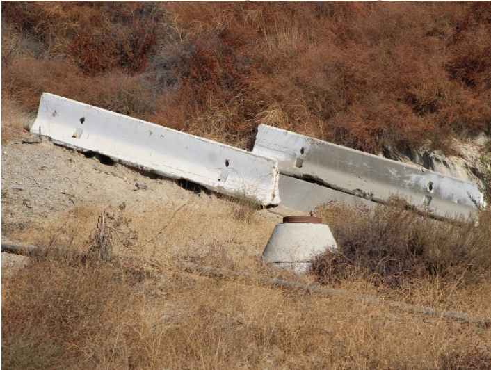
Photo 211: Eastside Drainage Channel: September 24, 2024
