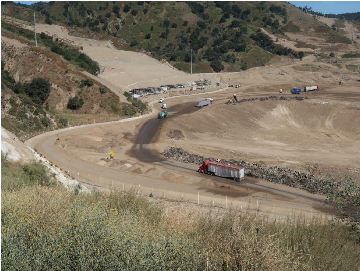
Photo 101: Working Area, CC-4 Part 4/5: July 3, 2024
