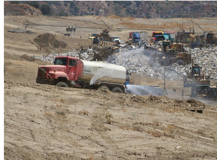
Photo 48: Working Area, CC4 Part 1/2: August 19, 2024
