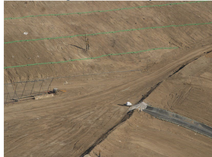
Photo 88: Working Area, CC-4 Part 3: September 24, 2024
