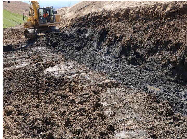
Photo 330: General Site: July 3, 2024
