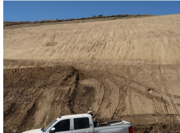
Photo 326: General Site: July 3, 2024
