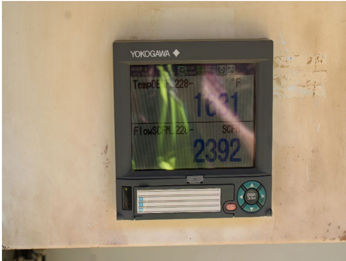
Photo 489: General Site: September 24, 2024
