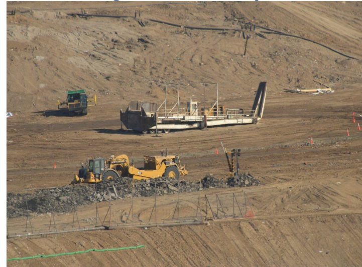
Photo 96: Working Area, CC-4 Part 3: September 24, 2024
