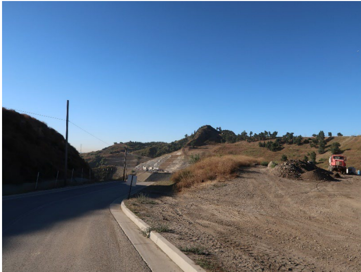
Photo 297: General Site: July 3, 2024
