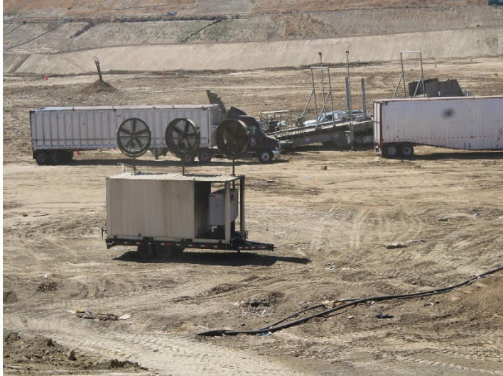
Photo 31: Working Area, CC4 Part 1/2: August 19, 2024
