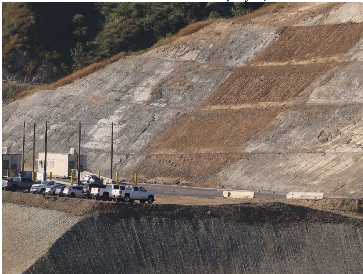
Photo 307: General Site: July 3, 2024
