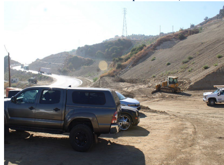
Photo 452: General Site: September 24, 2024
