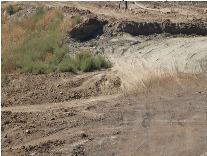
Photo 487: General Site: September 24, 2024
