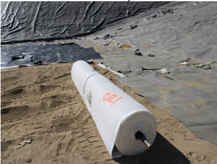
Photo 463: General Site: September 24, 2024
