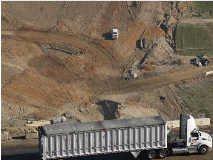
Photo 449: General Site: September 24, 2024
