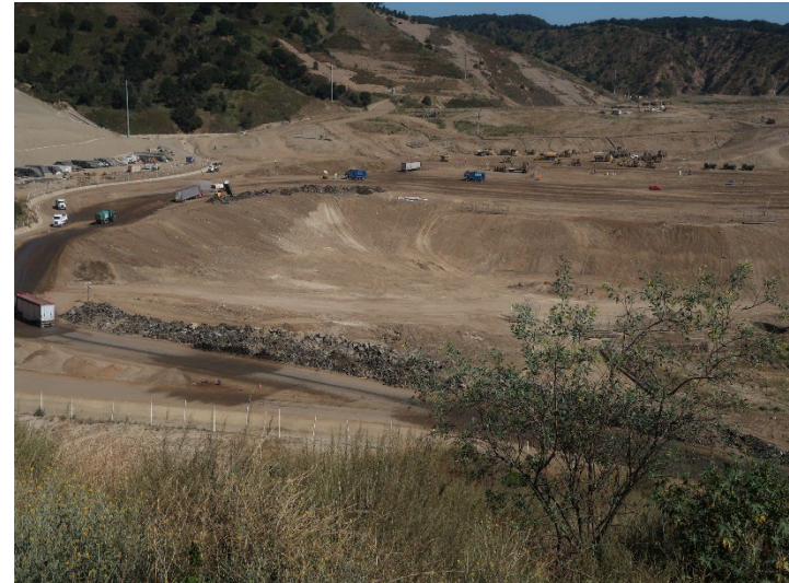
Photo 102: Working Area, CC-4 Part 4/5: July 3, 2024
