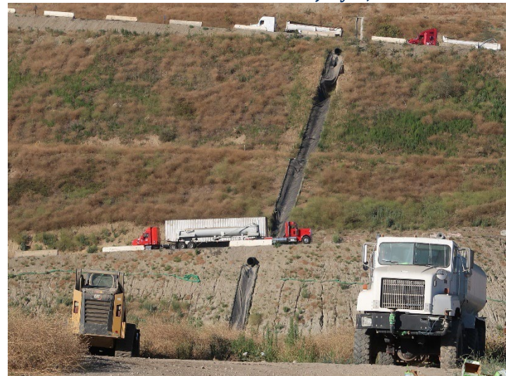
Photo 300: General Site: July 3, 2024
