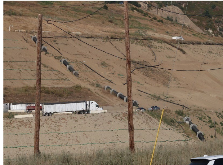
Photo 302: General Site: July 3, 2024
