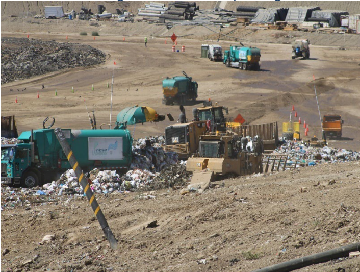
Photo 39: Working Area, CC4 Part 1/2: August 19, 2024
