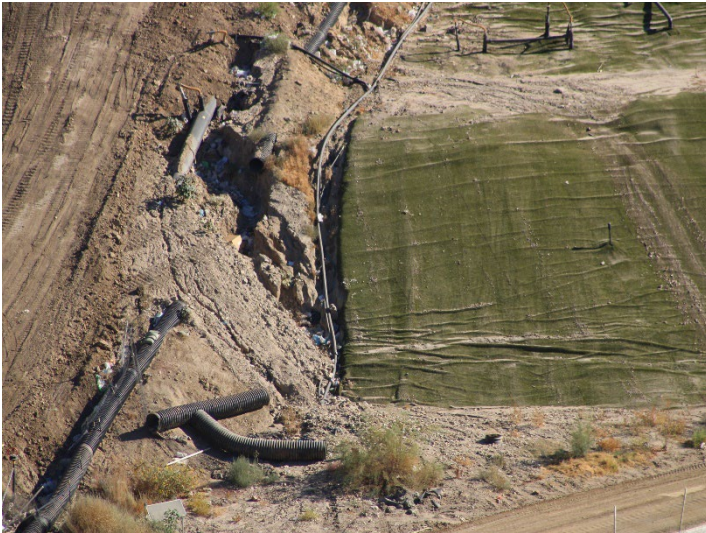
Photo 77: Working Area, CC-4 Part 3: August 19, 2024
