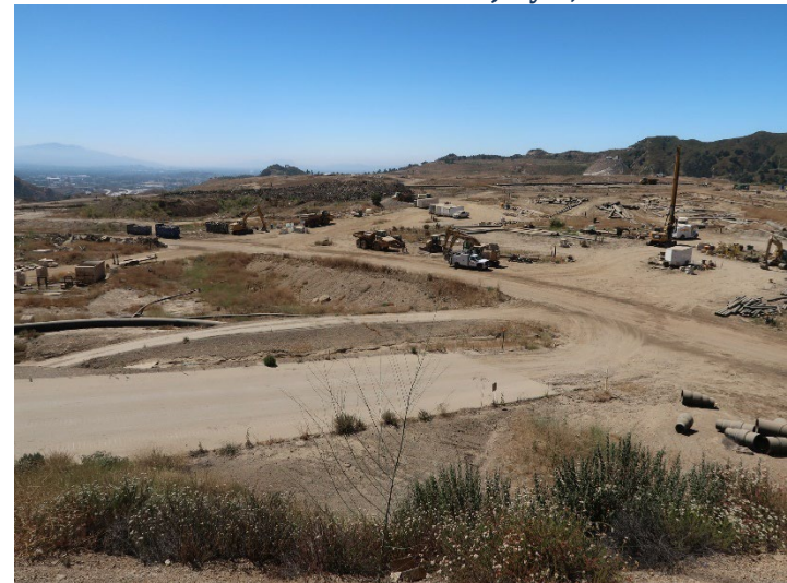
Photo 336: General Site: July 3, 2024
