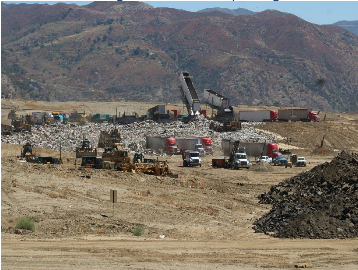
Photo 47: Working Area, CC4 Part 1/2: August 19, 2024
