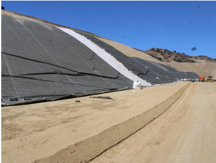
Photo 421: General Site: August 19, 2024
