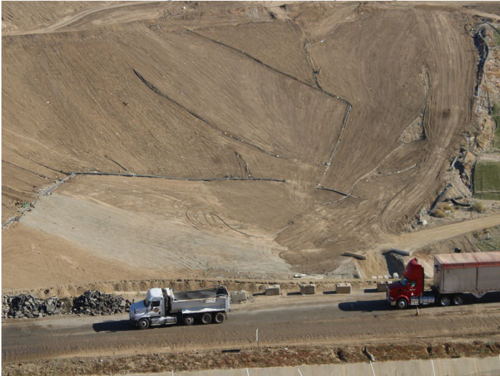
Photo 111: Working Area, CC-4 Part 4/5: August 19, 2024
