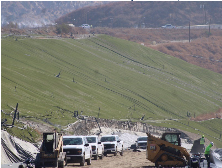
Photo 475: General Site: September 24, 2024
