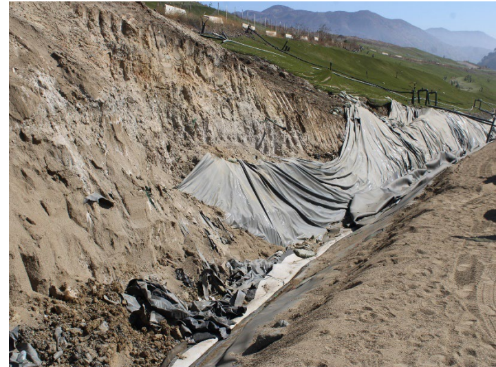
Photo 462: General Site: September 24, 2024
