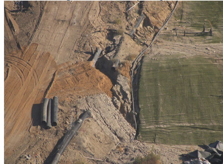
Photo 64: Working Area, CC4 Part 1/2: September 24, 2024
