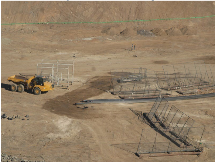
Photo 87: Working Area, CC-4 Part 3: September 24, 2024
