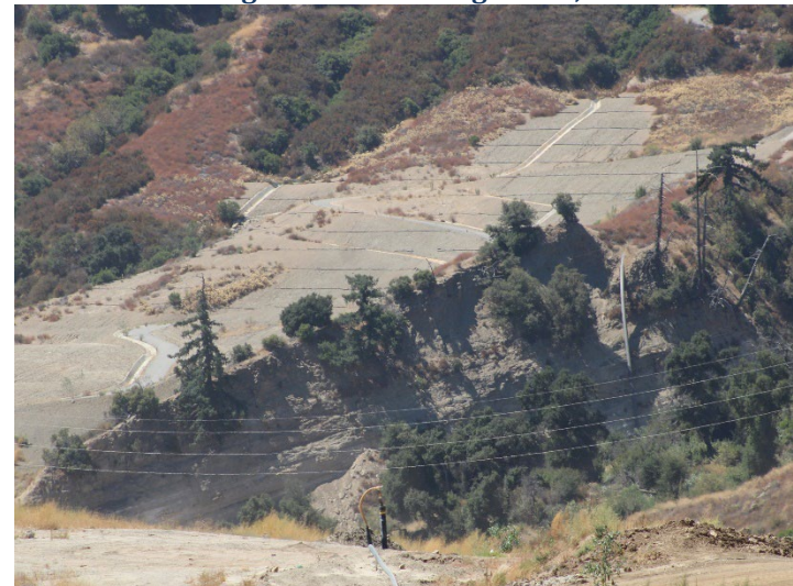
Photo 132: County Sage Mitigation Area and Westside Drainage Channels : August 19, 2024
