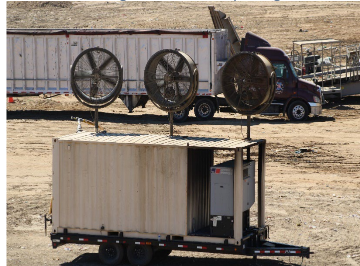
Photo 36: Working Area, CC4 Part 1/2: August 19, 2024
