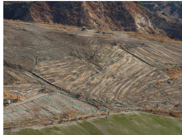
Photo 20: Working Area, CC4 Part 1/2: August 19, 2024
