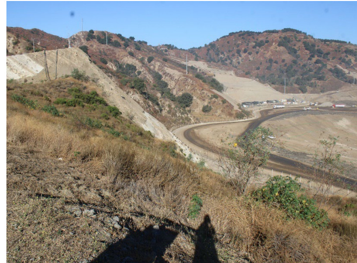
Photo 78: Working Area, CC-4 Part 3: September 24, 2024
