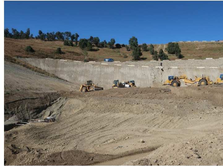
Photo 322: General Site: July 3, 2024
