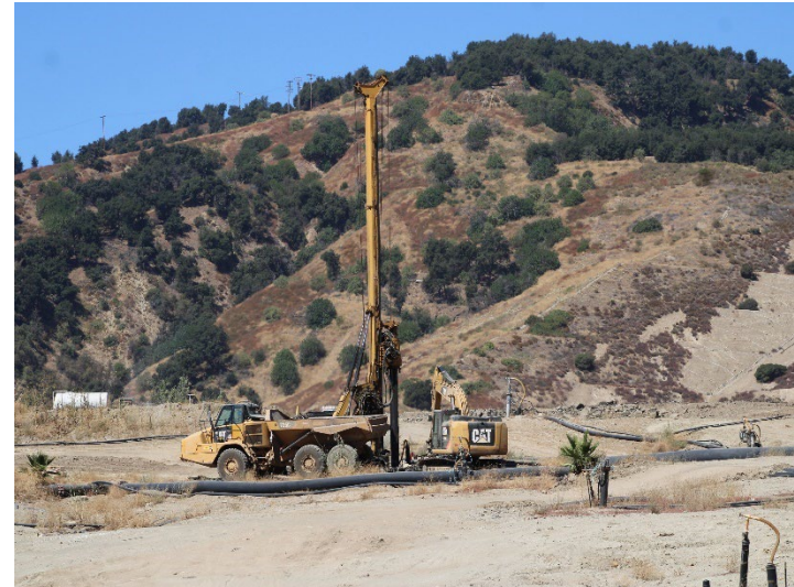
Photo 178: County Top Deck: August 19, 2024
