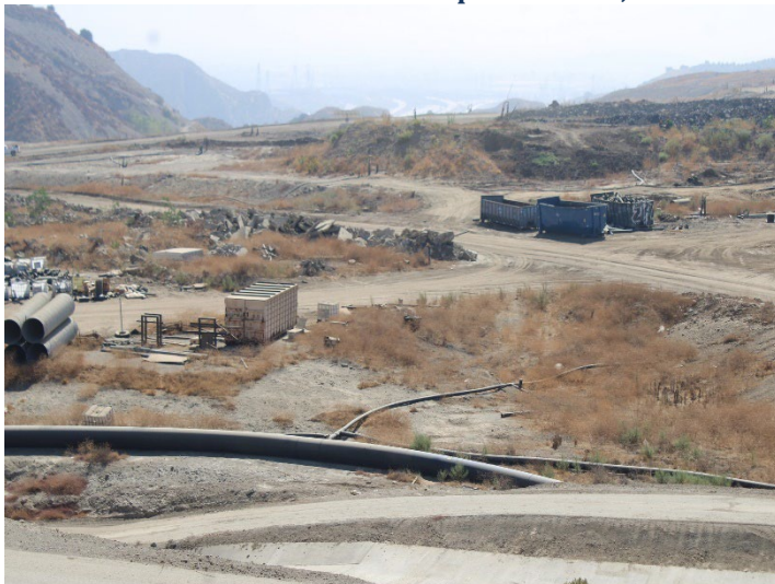
Photo 479: General Site: September 24, 2024
