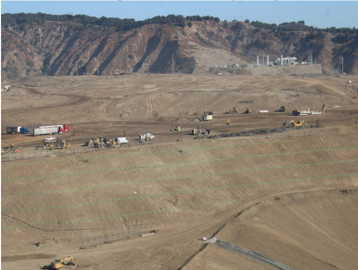
Photo 55: Working Area, CC4 Part 1/2: September 24, 2024
