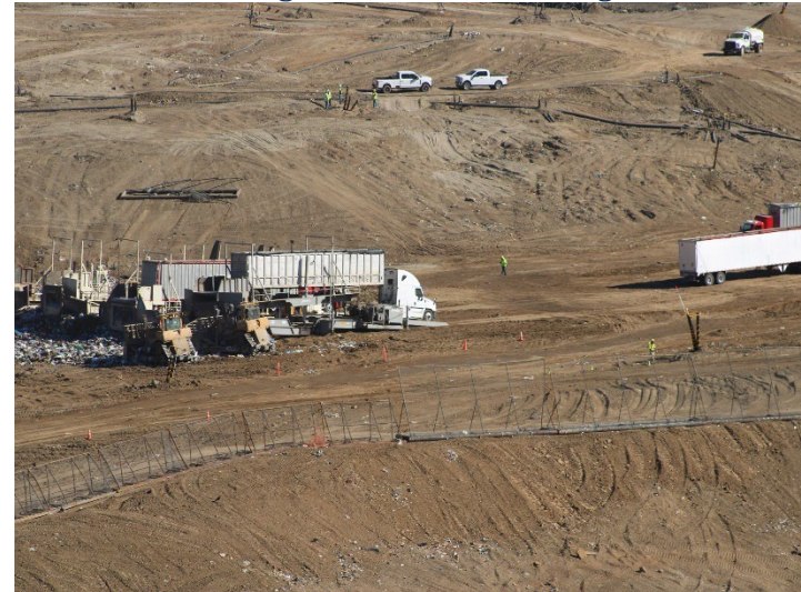
Photo 68: Working Area, CC-4 Part 3: August 19, 2024
