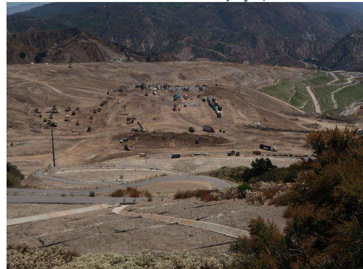
Photo 348: General Site: July 3, 2024
