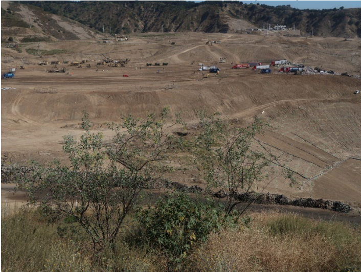
Photo 103: Working Area, CC-4 Part 4/5: July 3, 2024
