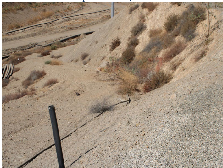
Photo 171: Flares 9, 10, 11 and Gas-to-Energy Facility: September 24, 2024
