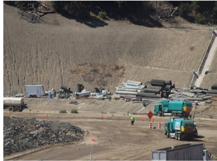
Photo 42: Working Area, CC4 Part 1/2: August 19, 2024
