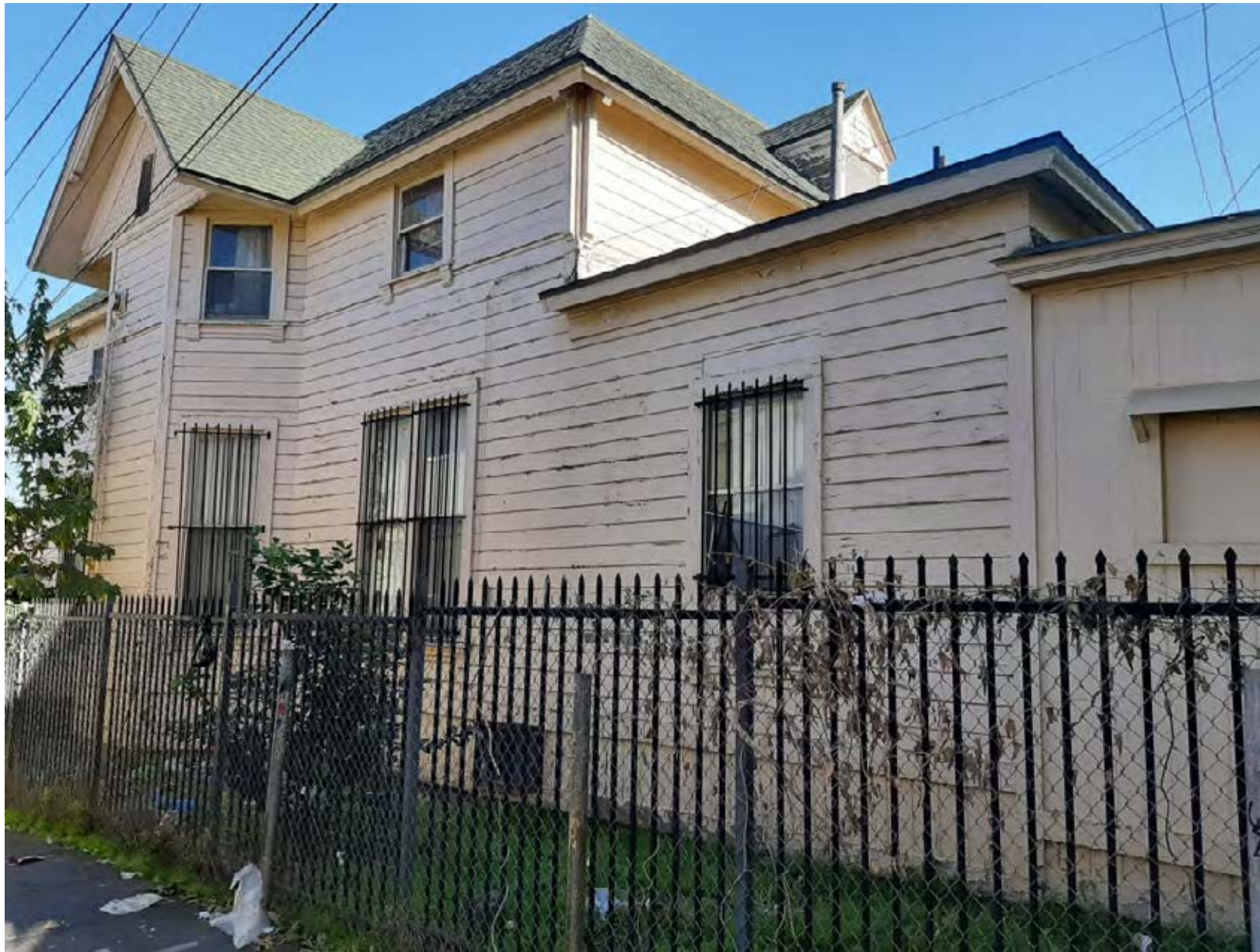
Secondary (west) elevation, facing northeast. Photo by Andrea Griego.
