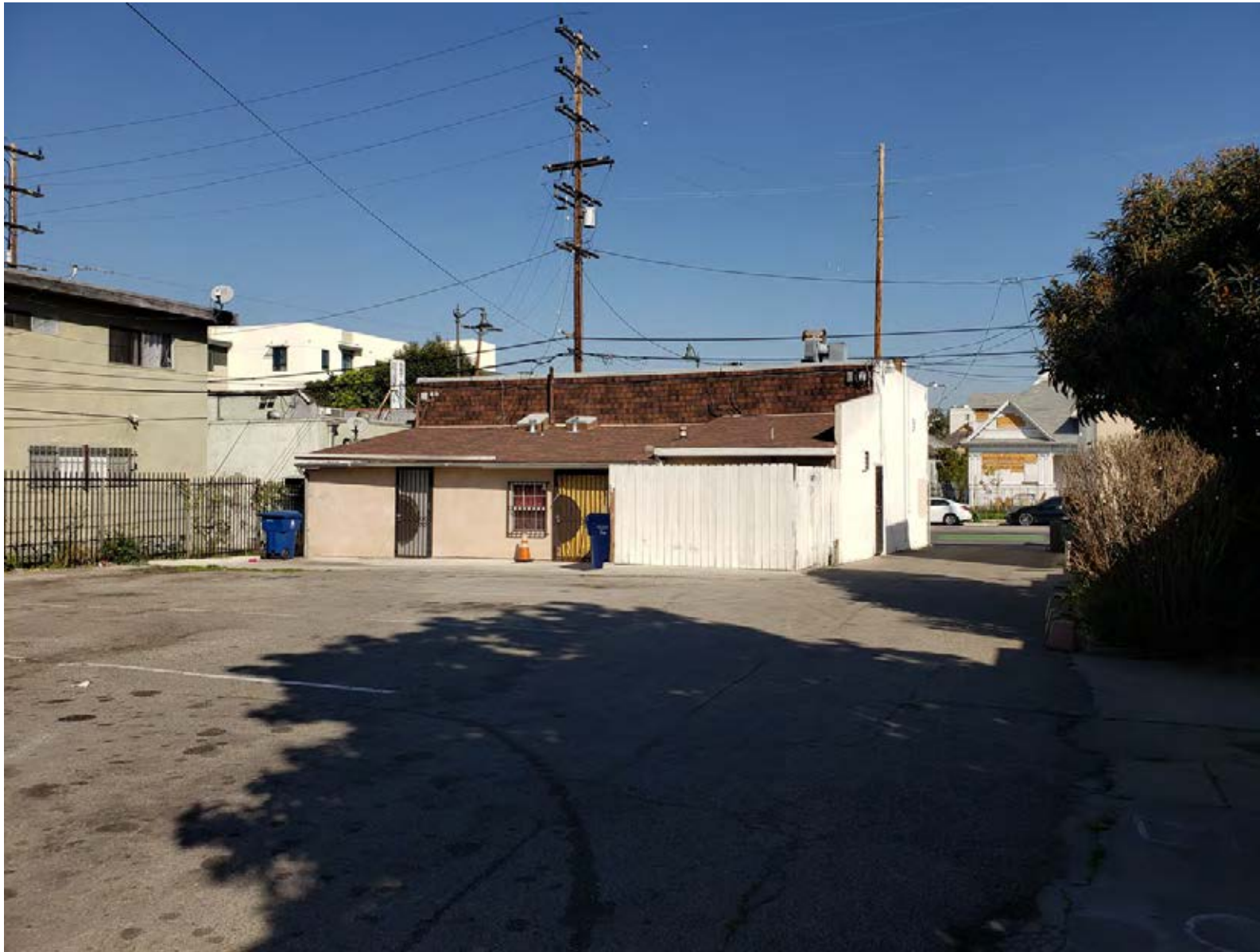
Rear (south) elevation of 2504-2506½ East First Street, facing northwest. Photo by M. Rosalind Sagara.
