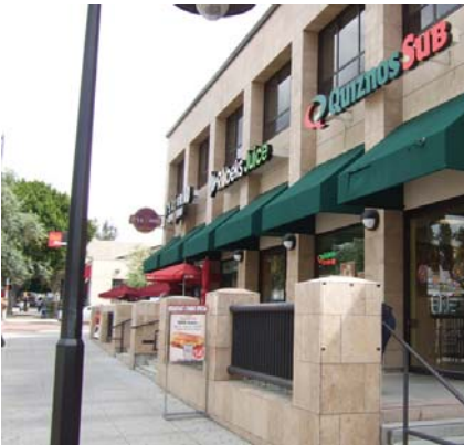
The structural bay pattern and simple profile make this building appropriate to an historic streetscape.
