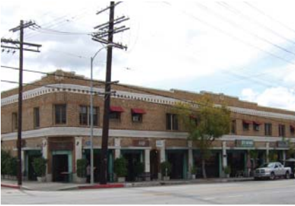
The upper-floor windows have not been filled-in and maintain a cohesive fenestration pattern.
