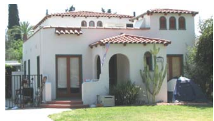
This second-story addition is set-back and preserves the look and scale of the original bungalow.
