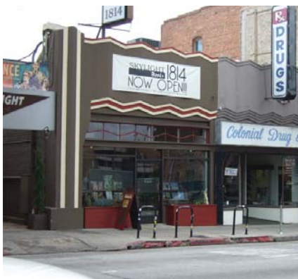
An appropriate paint scheme can showcase a building's original architectural features.
