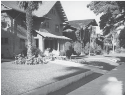
Hobart Boulevard streetscape showing homes in the Craftsman and Shingle styles.
