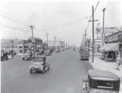
1927 view looking at Washington Blvd, west from 3rd Ave. There are numerous buildings advertising everything from auto supplies, dry goods, a pharmacy, used cars, real estate, overstuffed furniture sale, etc.
