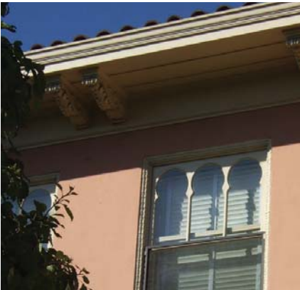
Smooth, hand-trowled stucco is an appropriate finish for this Italian Renaissance Revival home.
