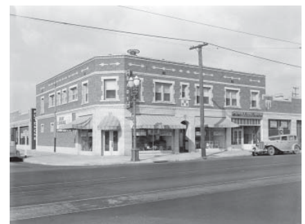
Exterior view of a brick retail building with residences on the second floor, located at 2225 West Washington Blvd. at Manhattan Place. Retail stores on the first floor include a baby shop and Perret Fine Arts.
