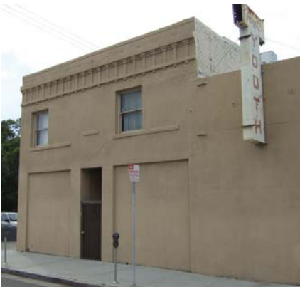
Filling-in windows creates an obvious impact to historic buildings.
