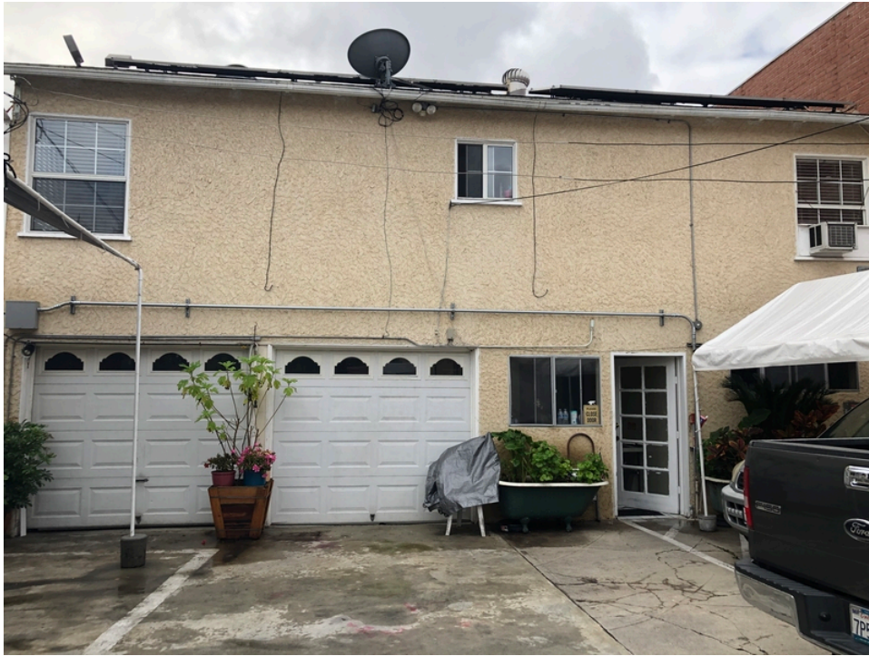
13. View of residence and commissary office at 3812 Oakwood Avenue, north elevation.
