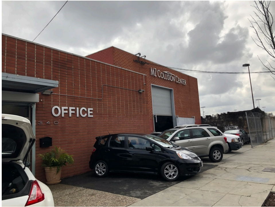
37. View of south-adjacent MZ Collision Center at 340 North Juanita Avenue.
