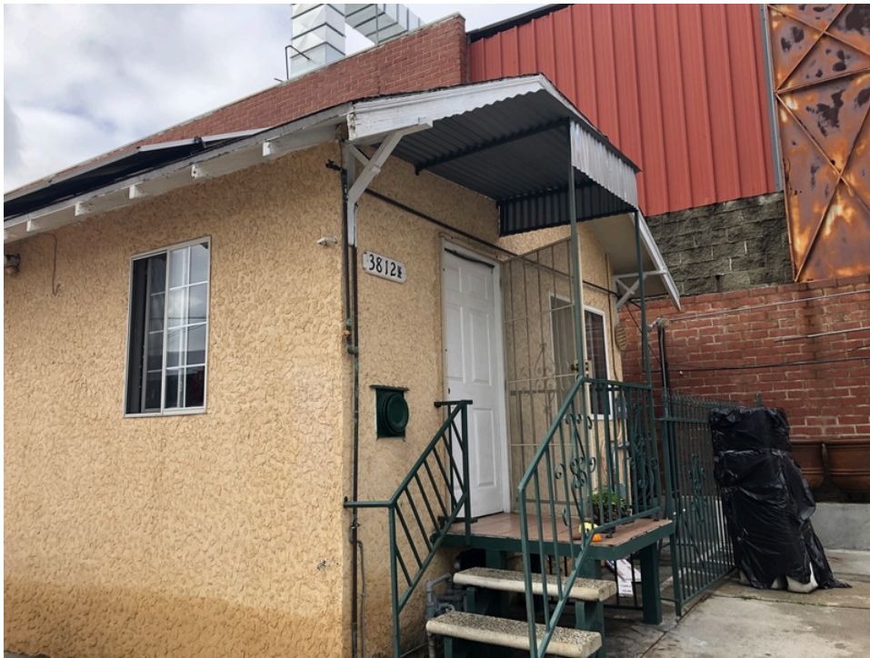
10. View of residential cottage at 3812 1/2 Oakwood Avenue.
