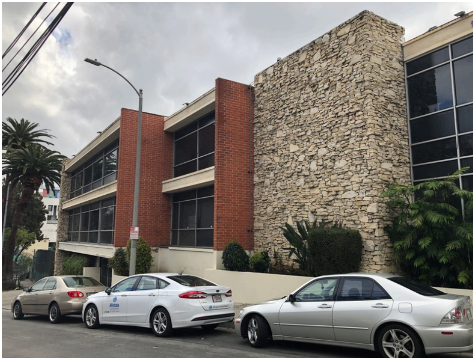
22. View of Mackintosh & Mackintosh office at 3820-3838 Oakwood Avenue, north elevation.
