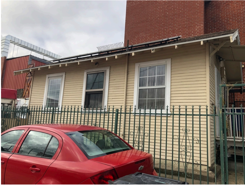
1. View of residential cottage at 3814 1/2 Oakwood Avenue.
