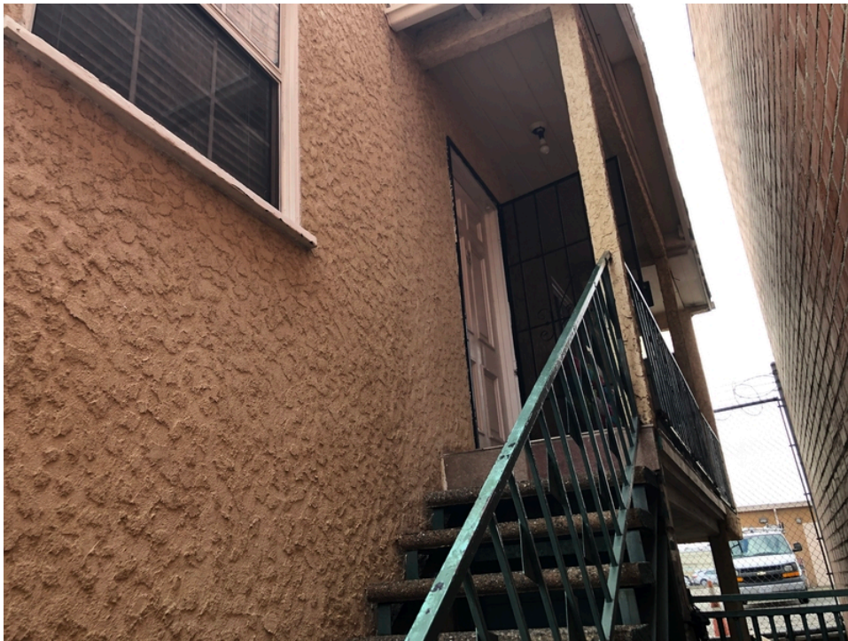
14. View of west elevation.
