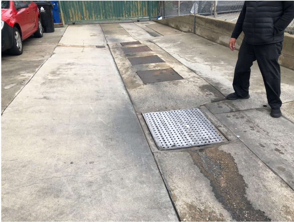
9. View of stormwater drain by interceptor.
