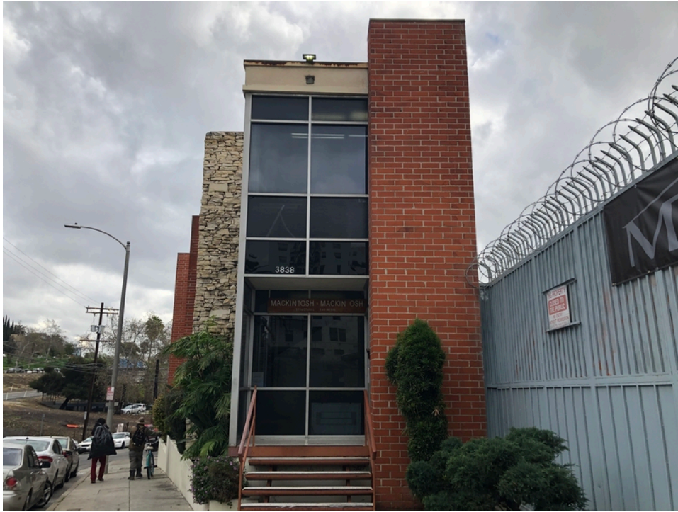
23. View of west elevation.
