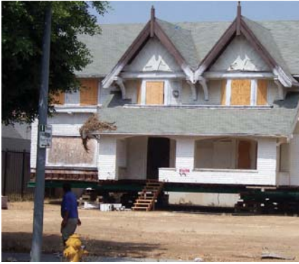
This home is being relocated to an HPOZ in Pico-Union.
