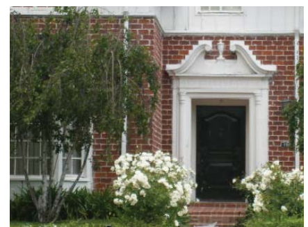
The pilasters, pediment and crown shown are typical to the Colonial Revival style.
