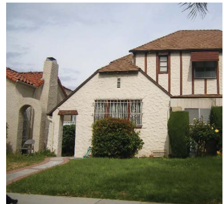
The use of highly textured stucco is a modern look and inappropriate on an historic home. Adding faux historic features, such as the timbering and stone on this front facade, is inappropriate.
