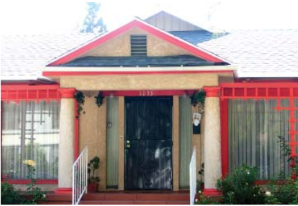
This doorway has been altered with a metal gate and plate glass sidelights.
