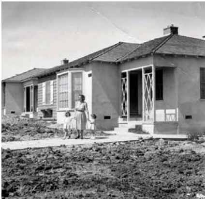
The Post-War building boom brought inexpensive and plentiful housing to the San Fernando Valley.
