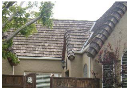
The wood shingles, curved detail of the roof and the extended rafter tails add character to this historic home.
