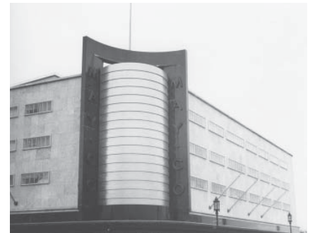
Formerly the May Company, the building at Fairfax and Wilshire epitomizes the Miracle Mile aesthetic.
