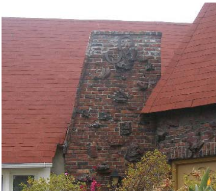
The clinker brick on this chimney adds character to this structure.
