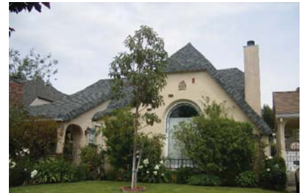
The notched gable ends and complex roof shape are defining features of this historic home..
