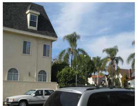
The massing of this building along with its mansard roof and dormer have little to do with the surrounding context.
