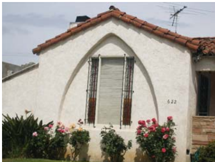
This window has been replaced with an ill-fitted window that diminishes the historic integrity of the house.
