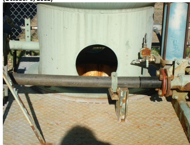
Photo 160: Condensate Drain at Flare 1 Discharge Knockout (December 7, 2012)
