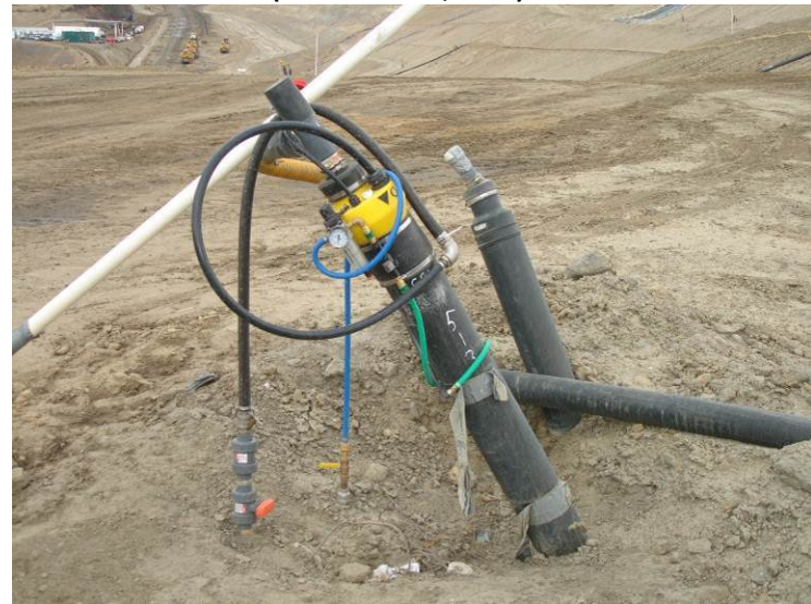
Photo 220: Cell CC2A Gas Well Liquid Removal Piping (November 15, 2012)
