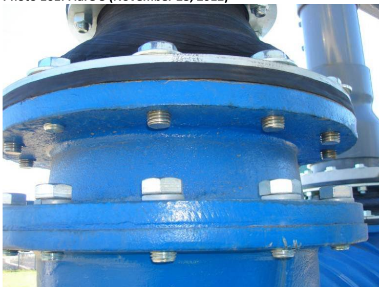
Photo 163: Flare 8 – Blower C Discharge Flange (December 7, 2012)
