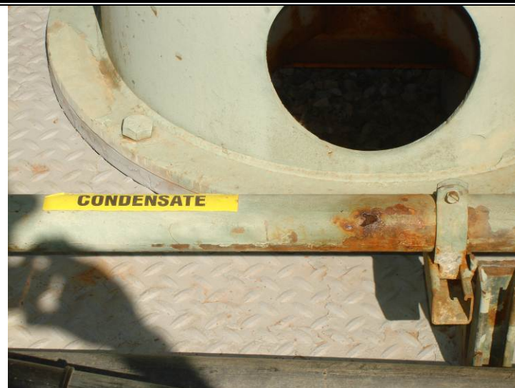
Photo 158: Condensate Drain at Flare 1 Discharge Knockout (October 9, 2012)
