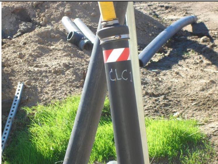
Photo 97: Abandoned Gas Collection Pipeline (December 19, 2012)
