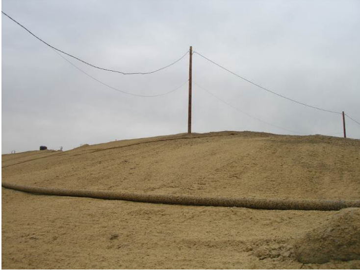
Photo 225: City North New Seed Mix Hydroseeding (November 15, 2012)
