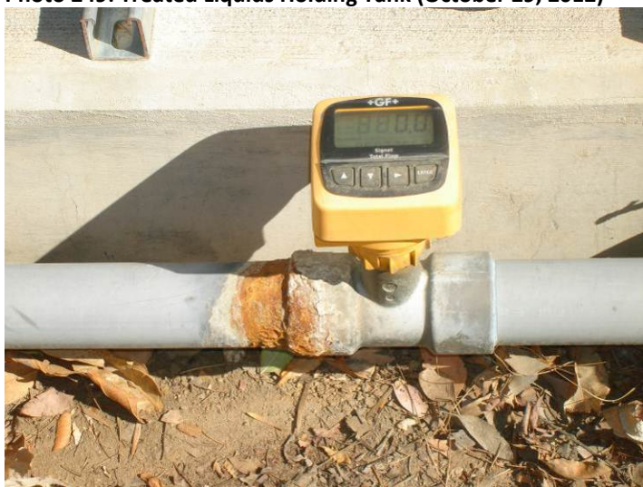
Photo 251: Treated Liquids Flow Meter (October 29, 2012)
