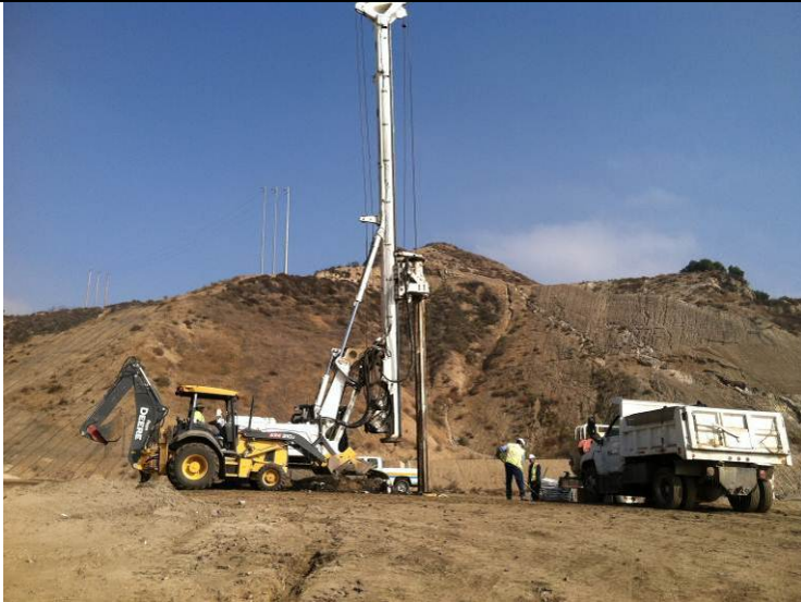
Photo 165: Well Drilling - County (November 28, 2012)
