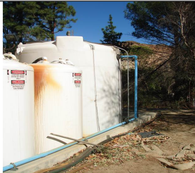
Photo 250: Treated Liquids Holding Tank (October 29, 2012)
