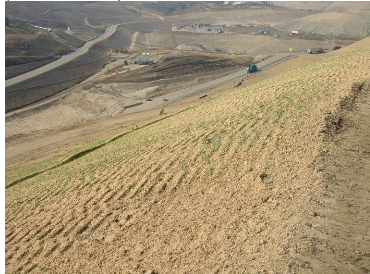
Photo 228: City North New Seed Mix Hydroseeding (November 28, 2012)
