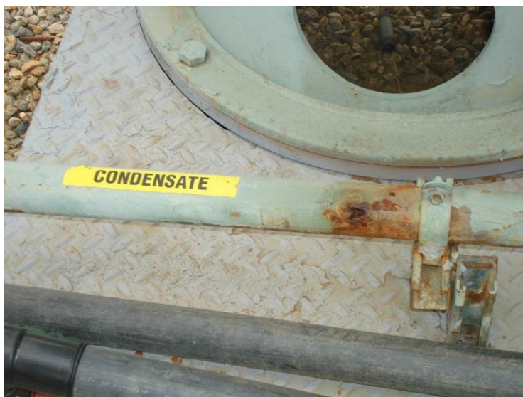
Photo 159: Condensate Drain at Flare 1 Discharge Knockout (November 15, 2012)
