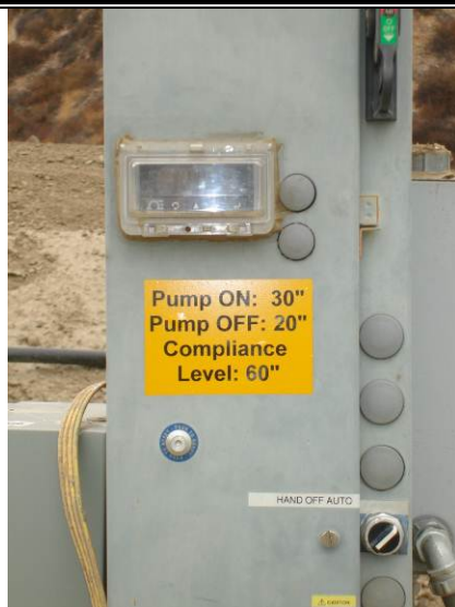
Photo 153: Leachate Sump Control Panel (November 15, 2012)
