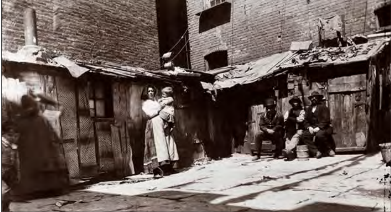
Urban planners sought to avoid the conditions found in places like the tenements of New York's Lower East Side, as documented by urban reformer Jacob Riis. Photo circa 1890. (Photo courtesy of the Museum of the City of New York)
