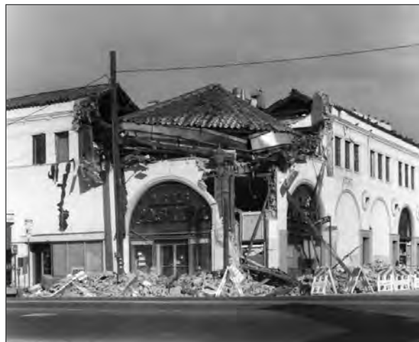
Damage sustained to a commercial building on Hollywood Boulevard as a result of the Northridge earthquake in 1994. (Photo courtesy of Los Angeles Public Library)
