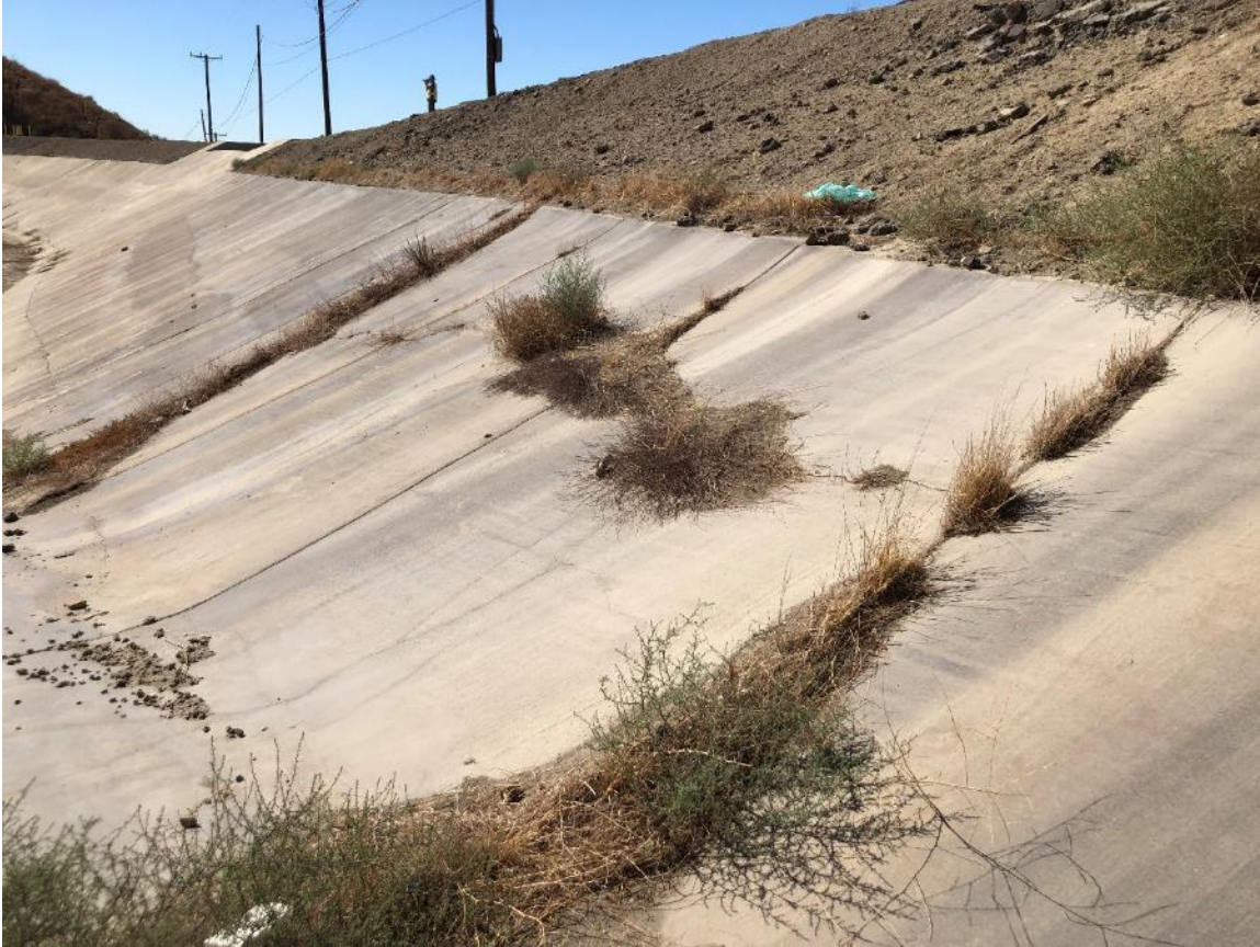
Photo 6: Vegetation growing in cracks at Basin B wall
