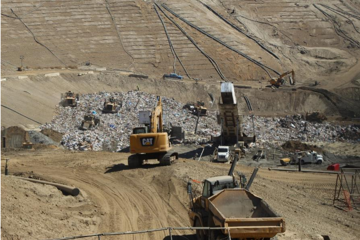
Photo 3: Waste disposal on top of Cell CC4 Phase 4
