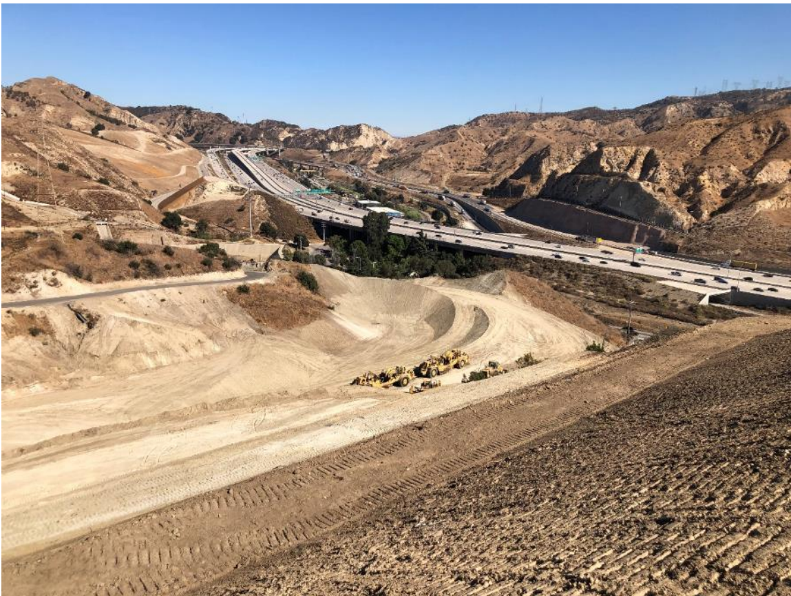
Photo 9: New sedimentation basin on new access road
