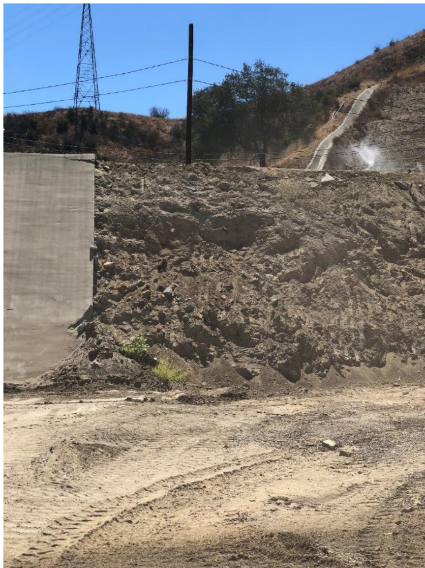
Photo 5: Exposed soil slope at terminal basin
