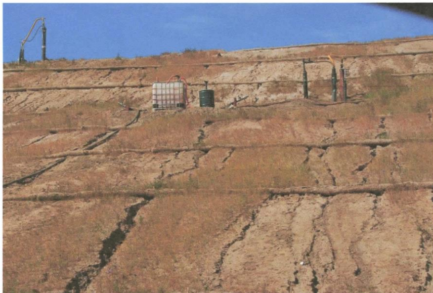
Photo 4: Erosion on north facing slope of Cell CC3
