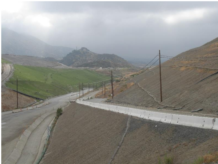
Photo 211: Closure Turf and Posi Shell: May 22, 2018
