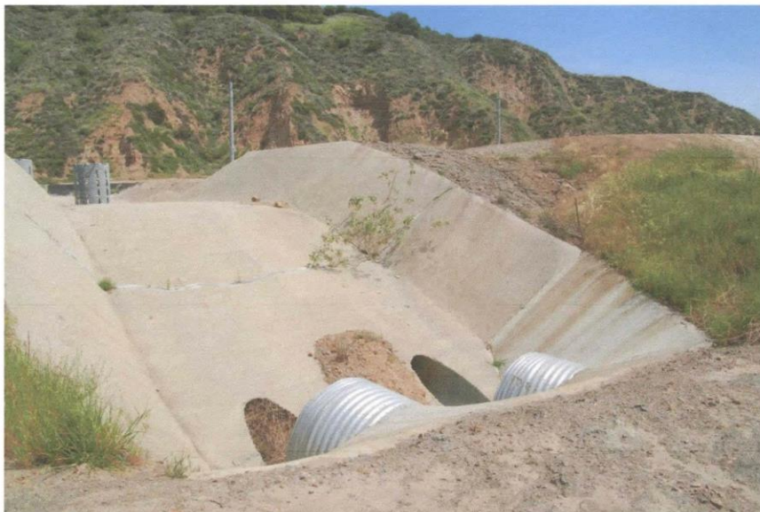
Photo 8: Cracked concrete spillway between two parts of Basin D and vegetation in crack
