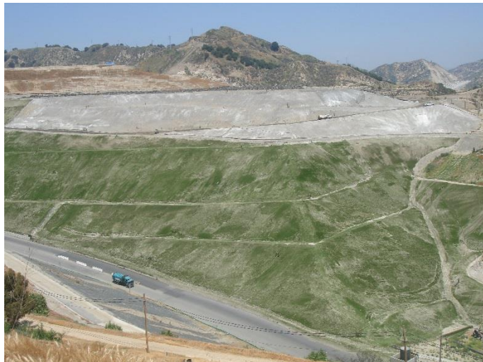
Photo 203: Closure Turf and Posi Shell: May 10, 2018
