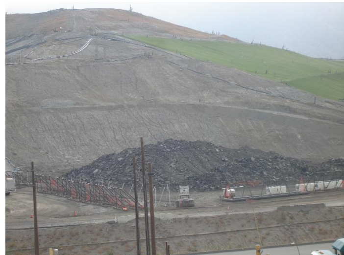
Photo 212: Closure Turf and Posi Shell: May 22, 2018
