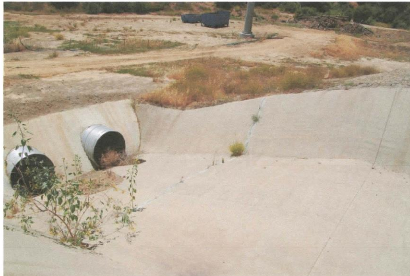
Photo 9: Cracked concrete spillway between two parts of Basin D and vegetation in crack
