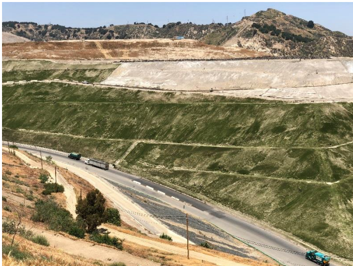
Photo 207: Closure Turf and Posi Shell: May 10, 2018
