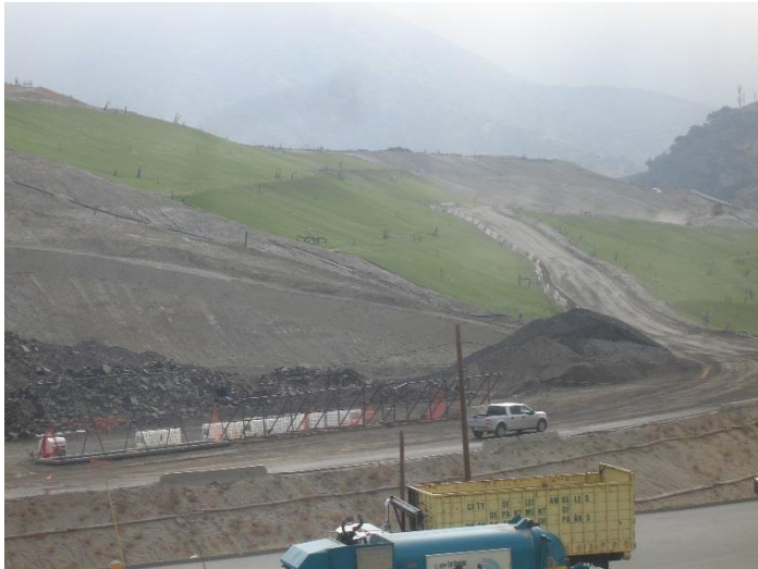
Photo 213: Closure Turf and Posi Shell: May 22, 2018
