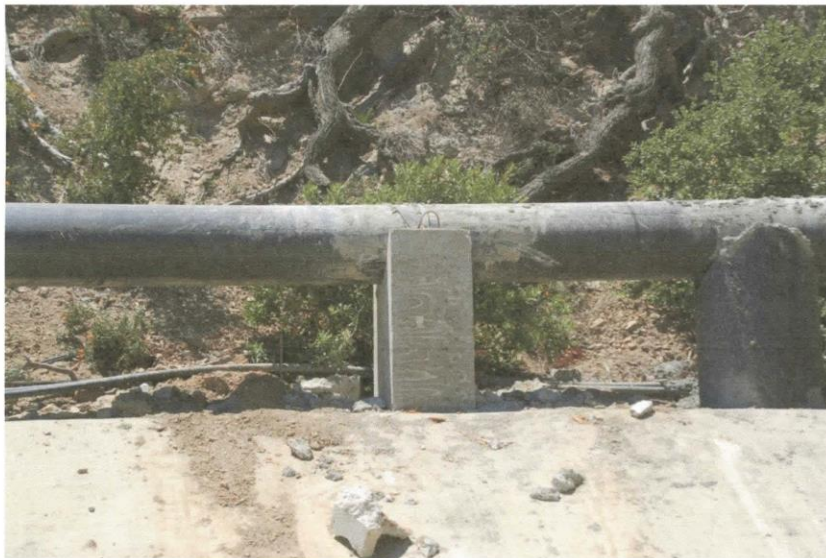
Photo 8: Concrete support for gas header to Flare 3
