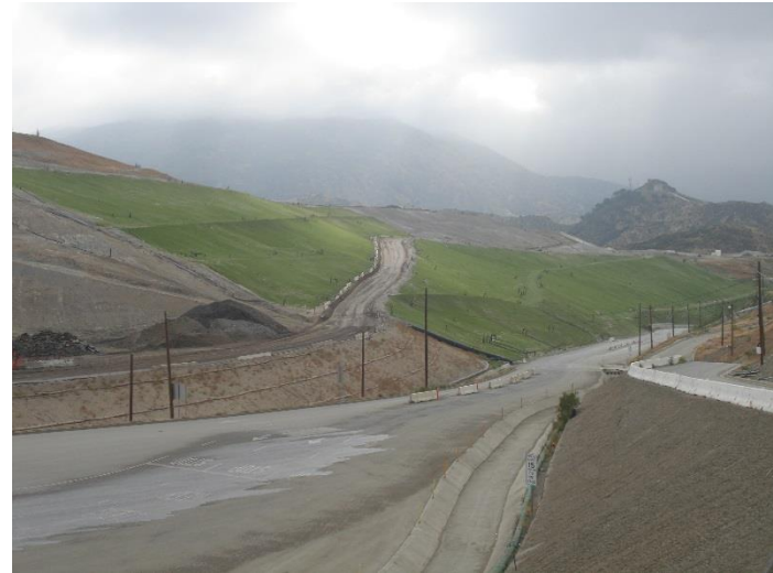
Photo 210: Closure Turf and Posi Shell: May 22, 2018
