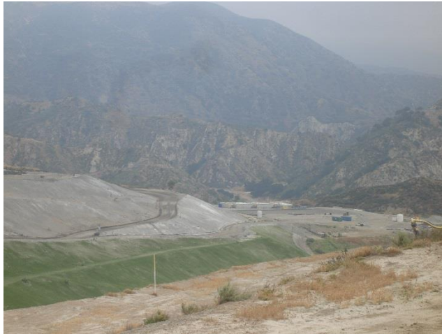
Photo 217: Closure Turf and Posi Shell: May 22, 2018
