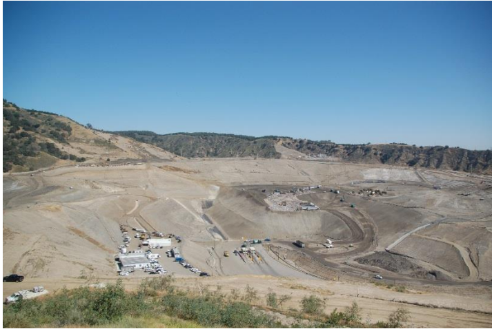
Photo 181: Site Working Area CC4A Part 3 Buttress Excavation: June 12, 2018
