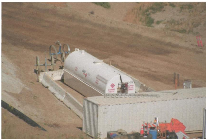
Photo 1: Petroleum product tank on city landfill bench – no drip pan under nozzle
