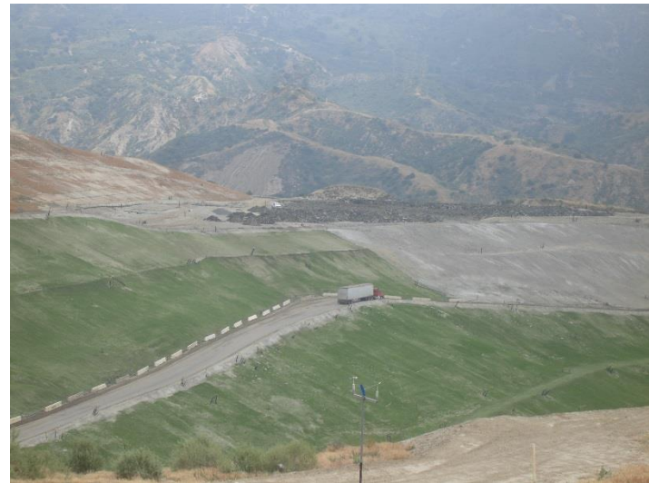
Photo 216: Closure Turf and Posi Shell: May 22, 2018
