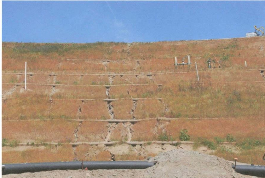
Photo 3: Erosion on east facing slope of Cell CC3
