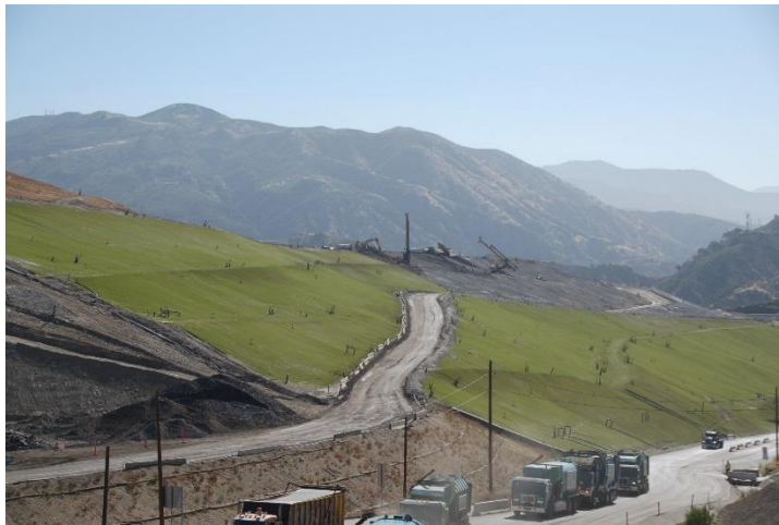
Photo 223: Closure Turf and Posi Shell: June 12, 2018
