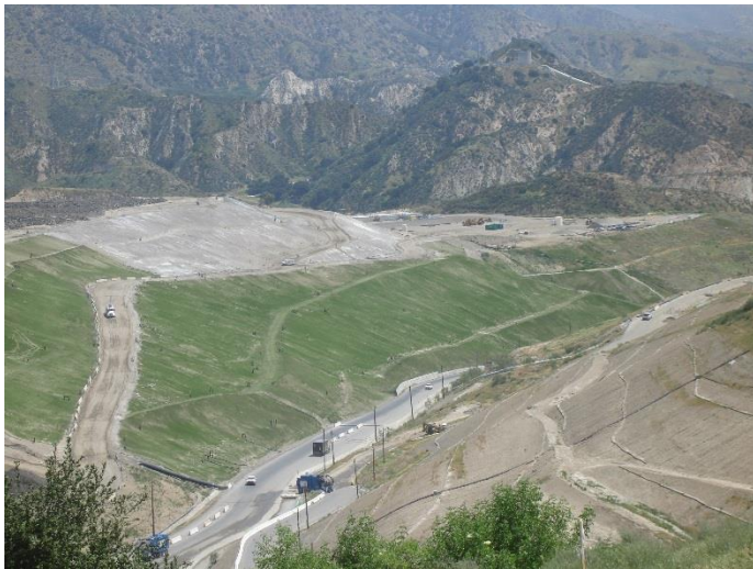
Photo 199: Closure Turf and Posi Shell: April 24, 2018
