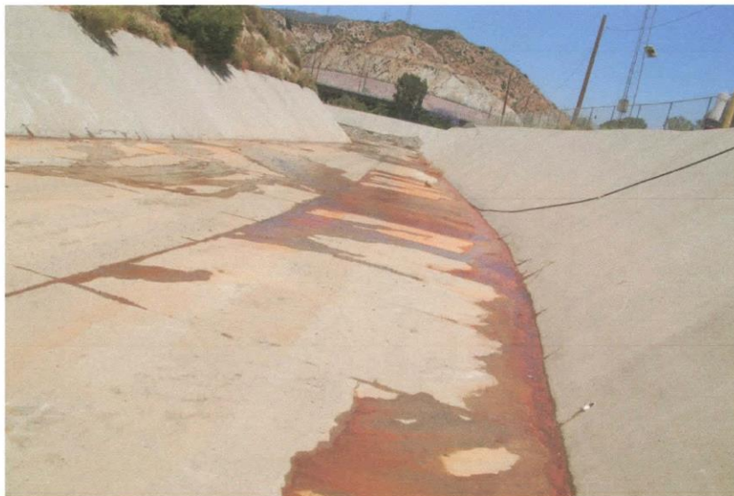
Photo 6: Reddish water oozing at intersection of bottom slab and slope slabs at terminal Basin
