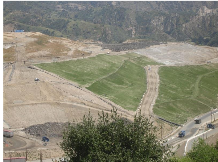
Photo 198: Closure Turf and Posi Shell: April 24, 2018
