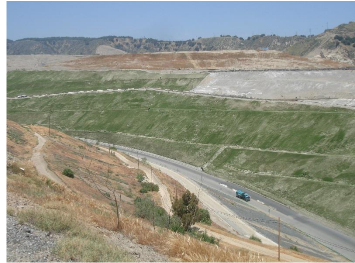
Photo 202: Closure Turf and Posi Shell: May 10, 2018
