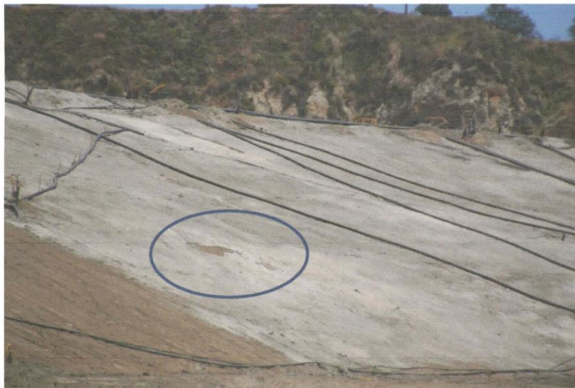
Photo 4: Bold spots on PosiShell on slope of Cell CC3
