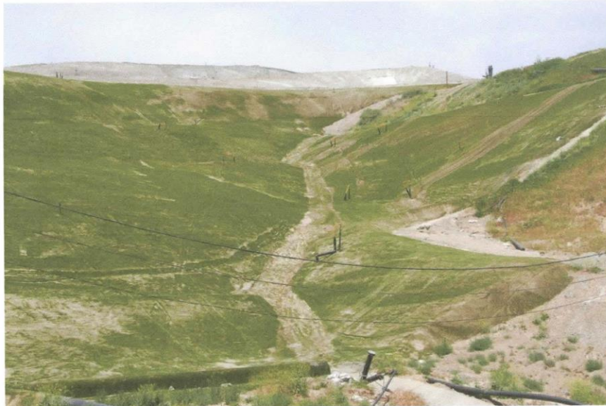
Photo 13: Sand washed out of the ClosureTurf in drainage path
