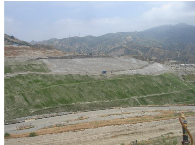
Photo 218: Closure Turf and Posi Shell: May 22, 2018
