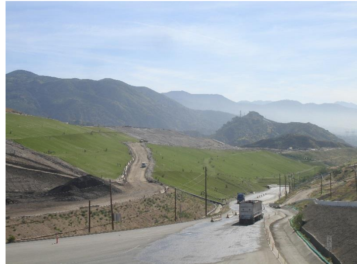
Photo 194: Closure Turf and Posi Shell: April 24, 2018
