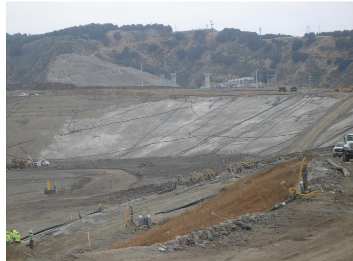
Photo 220: Closure Turf and Posi Shell: May 22, 2018
