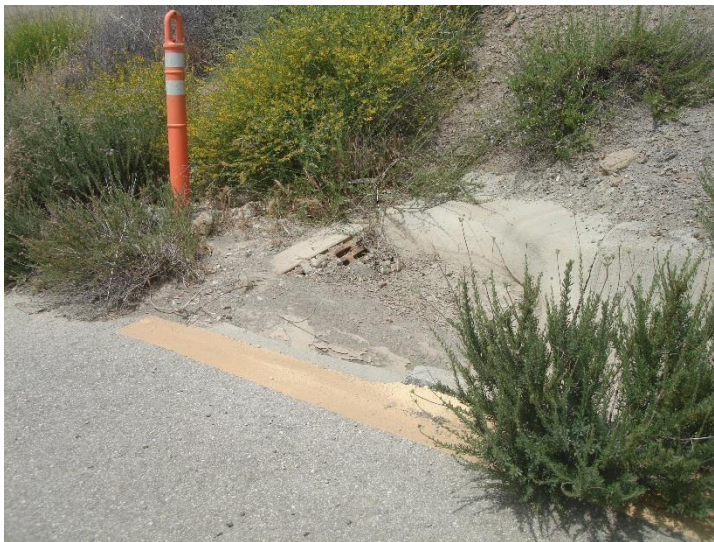
Photo 419: Buried Drain at Flare 9 Access Road: May 22, 2018
