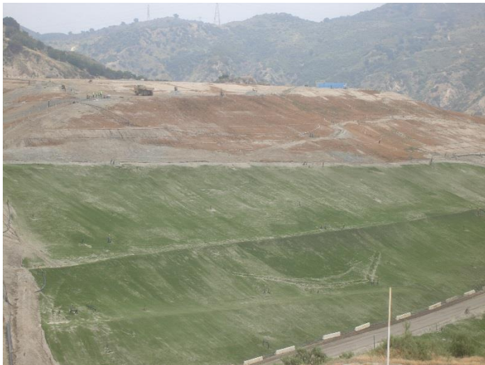
Photo 215: Closure Turf and Posi Shell: May 22, 2018
