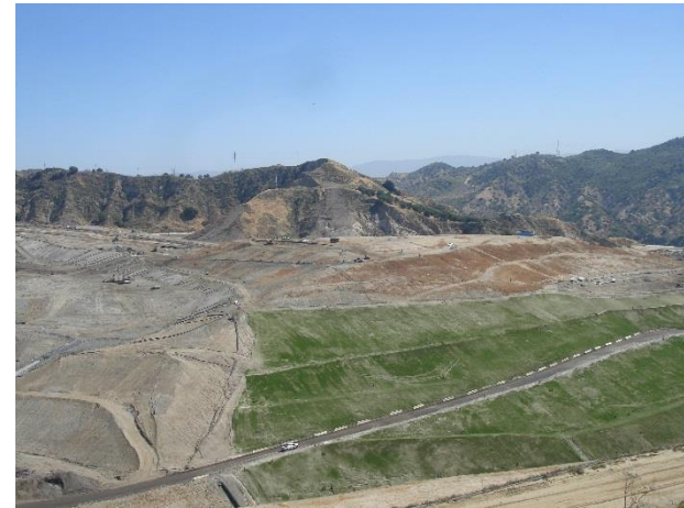
Photo 222: Closure Turf and Posi Shell: June 12, 2018
