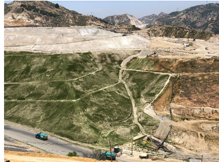
Photo 208: Closure Turf and Posi Shell: May 10, 2018
