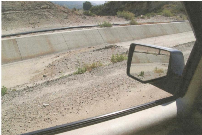
Photo 10: Sediments accumulation against asphalt berm in northern portion of main channel to terminal Basin
