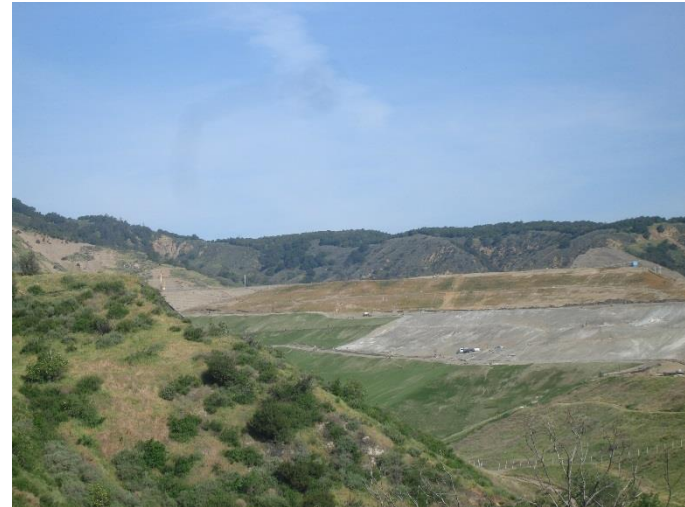
Photo 196: Closure Turf and Posi Shell: April 24, 2018
