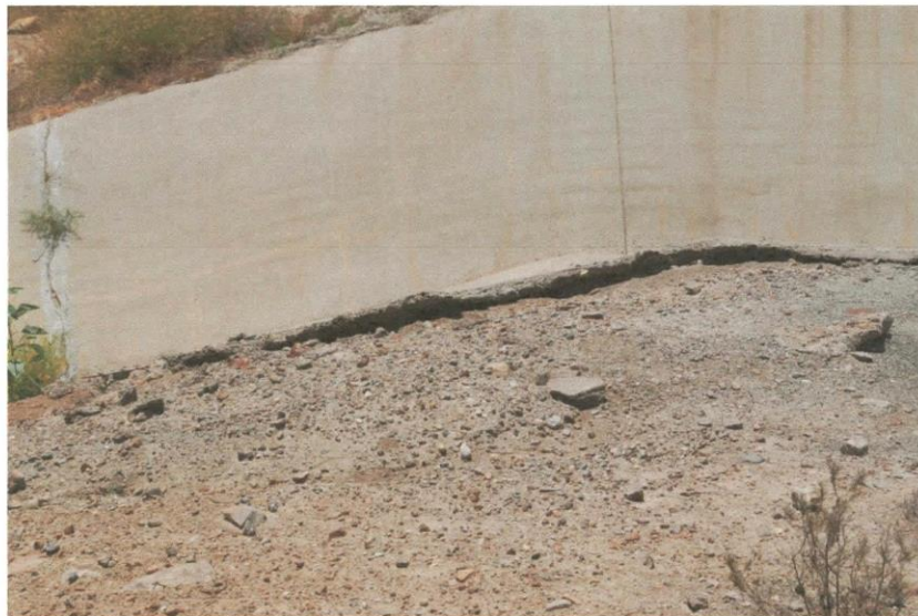
Photo 10: Separation between soil and spillway concrete at Basin D
