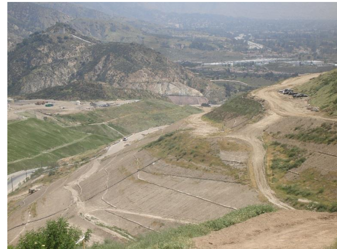
Photo 200: Closure Turf and Posi Shell: April 24, 2018
