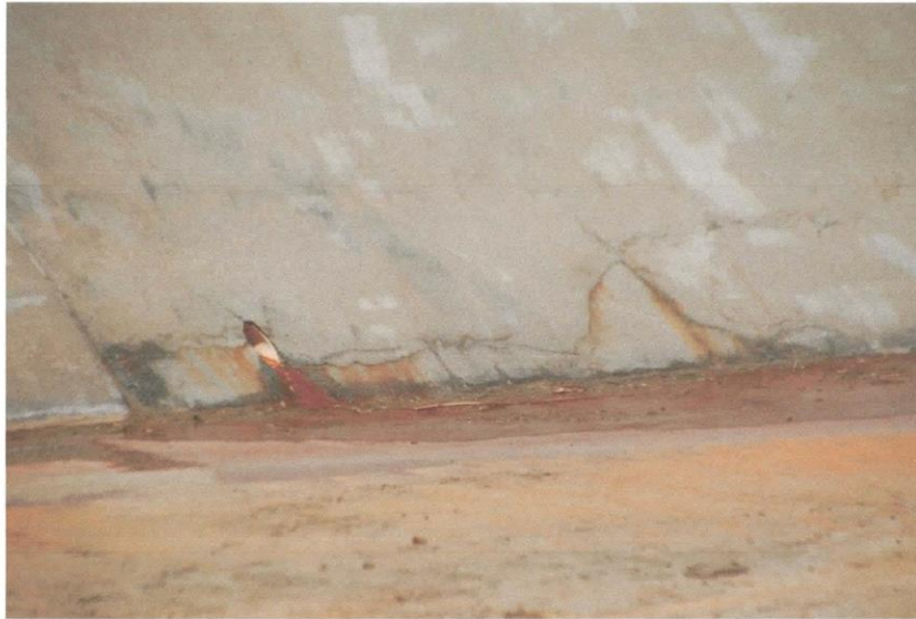
Photo 7: Reddish water oozing from weep hole in slope slabs at terminal Basin
