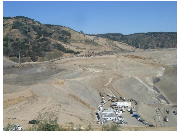
Photo 176: Site Working Area CC4A Part 3 Buttress Excavation: June 12, 2018
