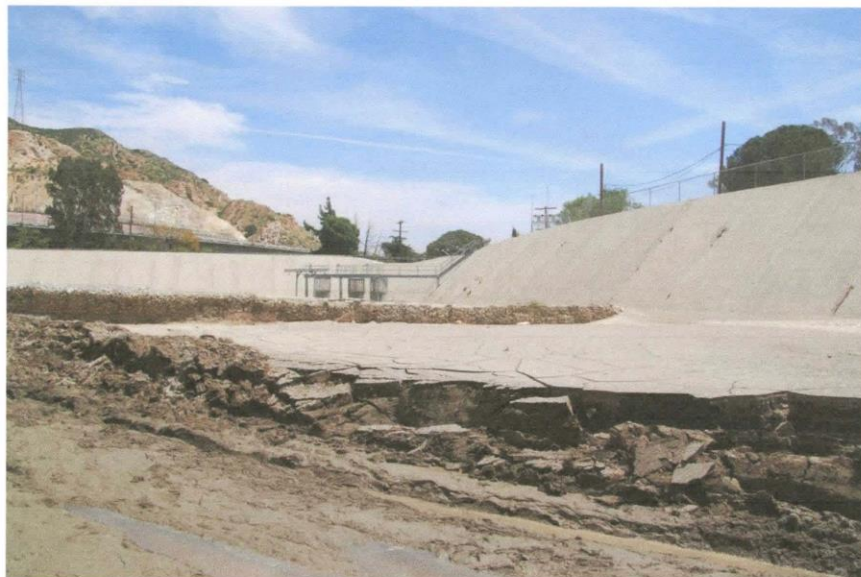
Photo 6: Sediments in Terminal Basin Upstream of Gabion Wall
