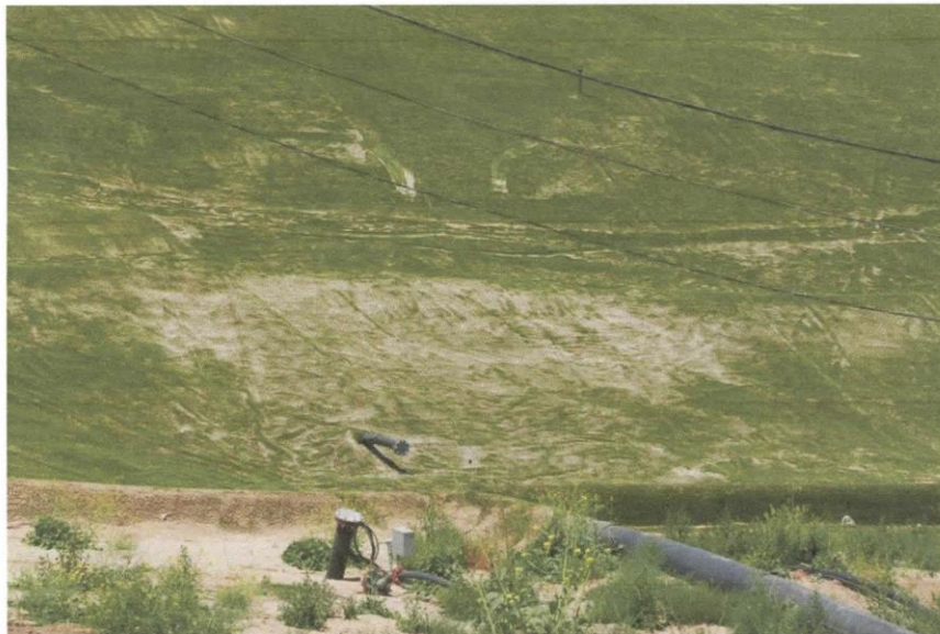
Photo 12: Sand washed out of the ClosureTurf on steep slope
