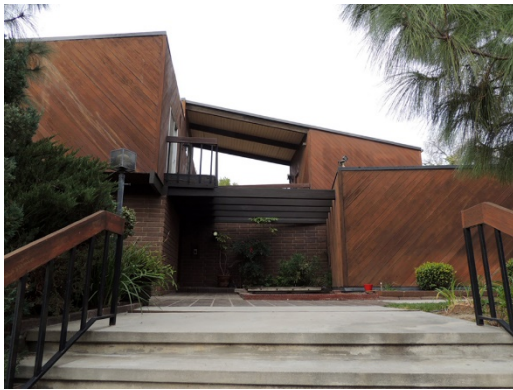
Address: 12069 Susan Drive Architect: H.C. Dixon Date: 1974
