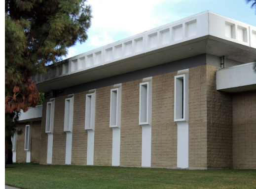
Address: 11254 Gothic Avenue Name: John F. Kennedy High School Architect: Stewart S. Granger & Associates Date: 1971
