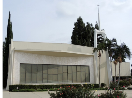
Address: 15950 Chatsworth Street Name: St. Stephen's Lutheran Church Architect: Orr, Strange, Inslee & Senefeld Date: 1966
