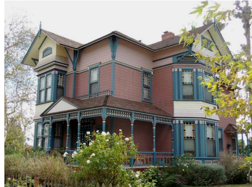
Address: 17410 Mayerling Street Architect: Joseph Cather Newsom Date: 1887
