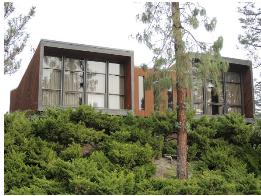
Address: 12069 Susan Drive Architect: H.C. Dixon Date: 1974
