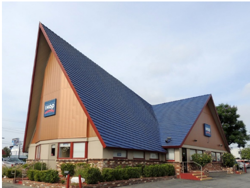
Address: 16943 Devonshire Street Name: International House of Pancakes Architect: Neil Johnson Date: 1962
