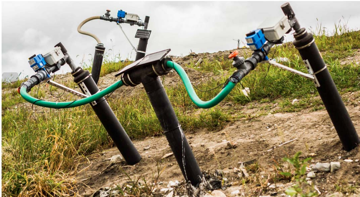
Photo 3- Loci Controls WellWatcher monitoring & control system used to automatically adjust and monitor each landfill gas well.
