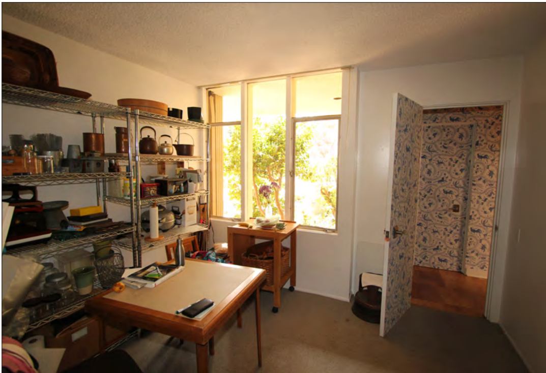
Image 52: Service area, view north (Chattel, 2019)
