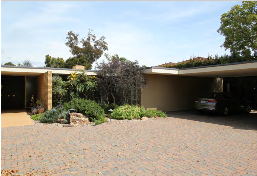
Image 9: Front entrance and carport, view southeast (Chattel, 2019)
