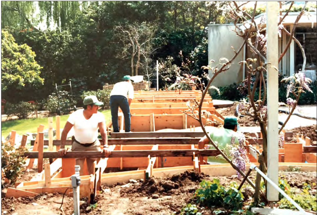
Image 37: Garden, coy pond construction (Ray Borun, 1985)
