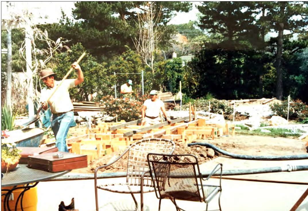
Image 25: Garden renovations (Ray Borun, 1985)
