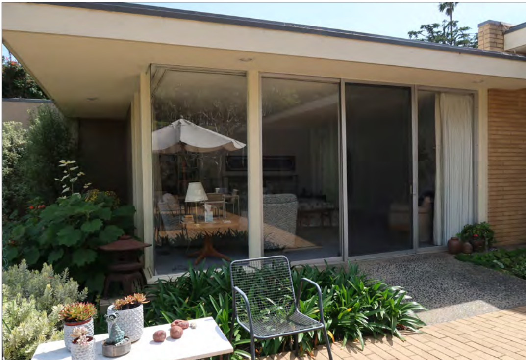
Image 18: East elevation, view south (Chattel, 2019)
