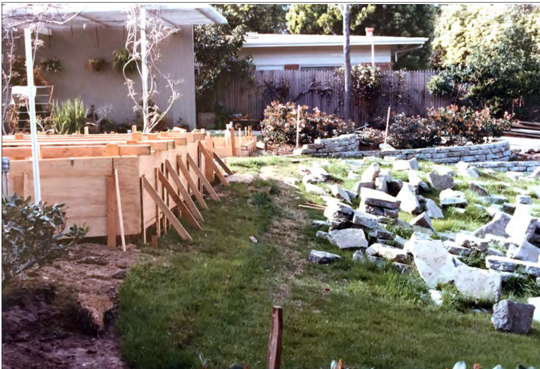
Image 42: Garden renovations (Ray Borun, 1985)
