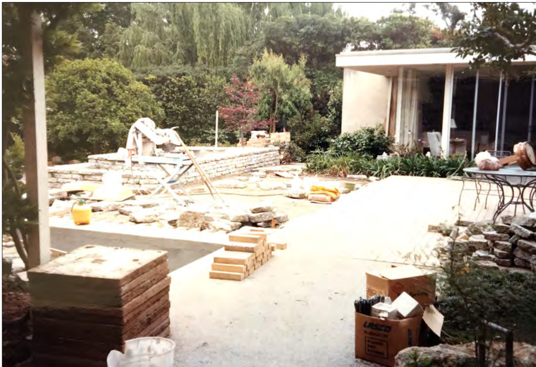
Image 44: Garden, coy pond construction (Ray Borun, 1985)
