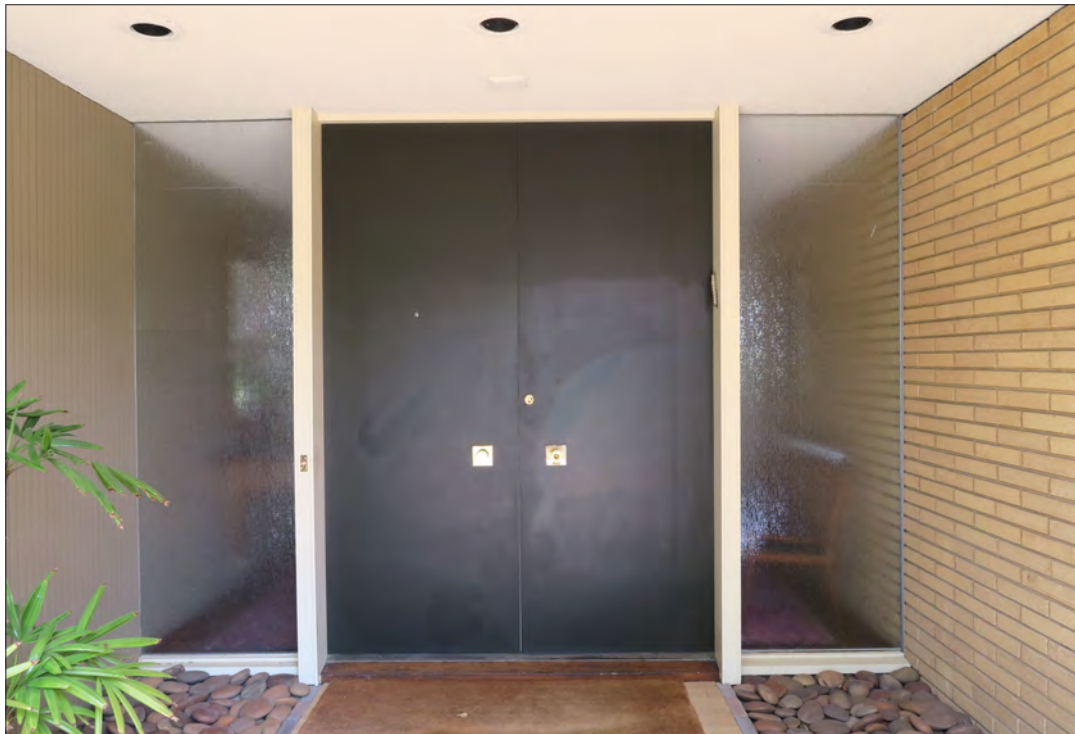
Image 14: Front entrance doors, view east (Chattel, 2019)
