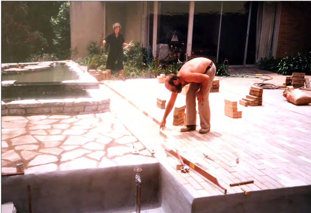
Image 43: Garden, coy pond construction (Ray Borun, 1985)
