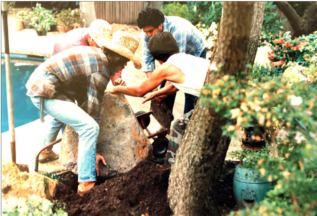
Image 58: Garden renovations (Ray Borun, 1985)
