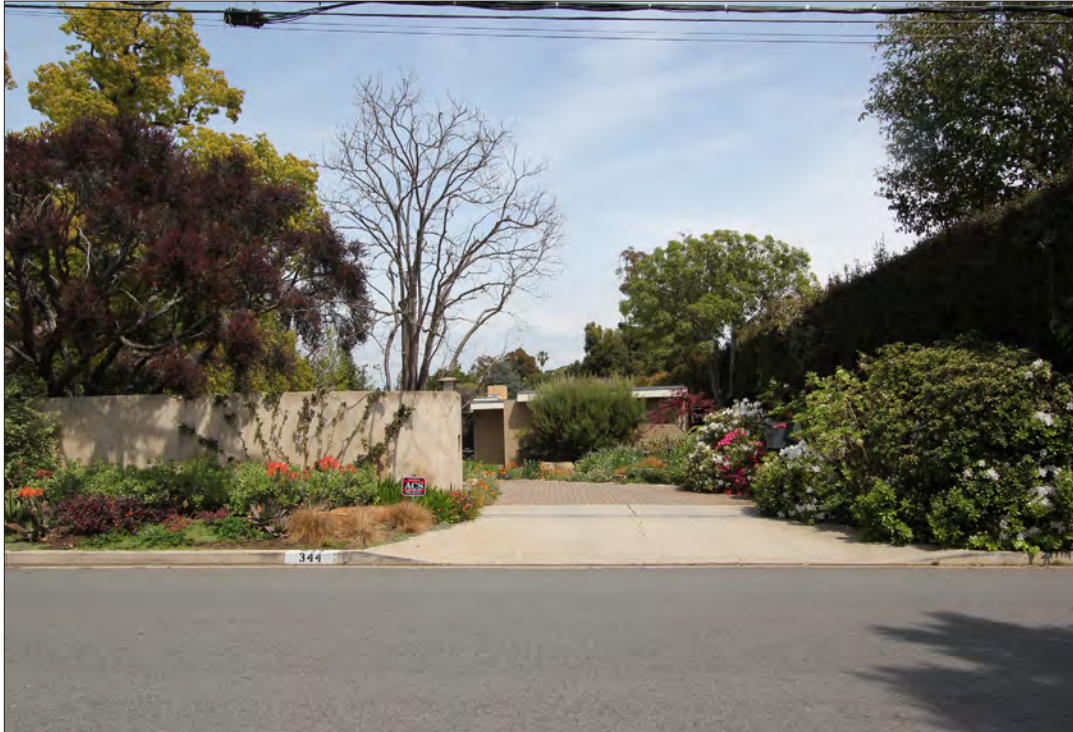
Image 3: Borun House and driveway, view east (Chattel, 2019)
