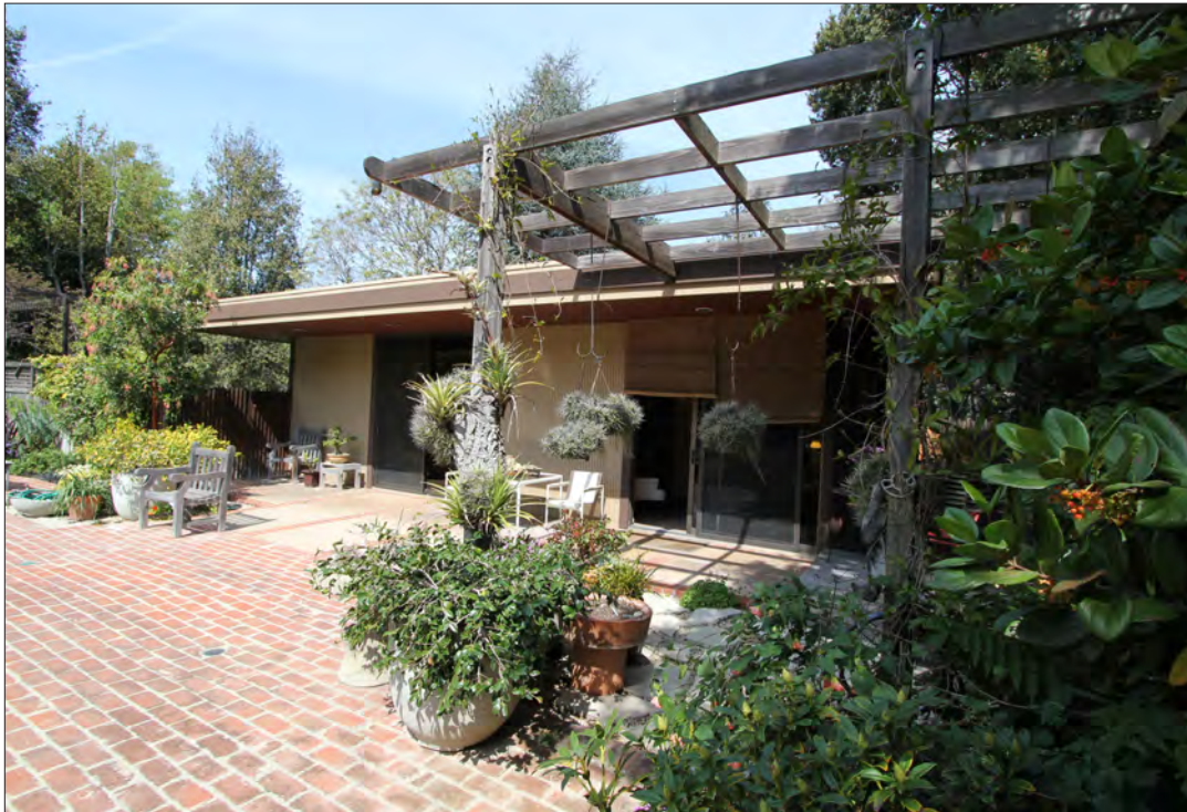
Image 61: Accessory Building, west elevation, view northeast (Chattel, 2019)
