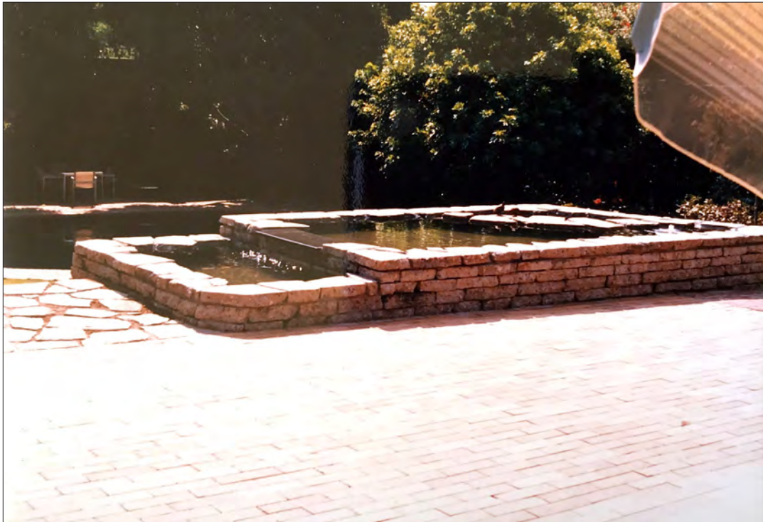
Image 45: Garden, coy pond construction (Ray Borun, 1985)
