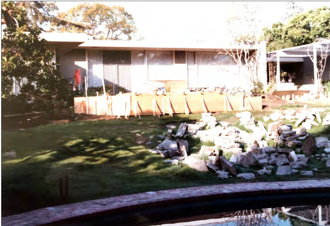
Image 41: Garden renovations (Ray Borun, 1985)
