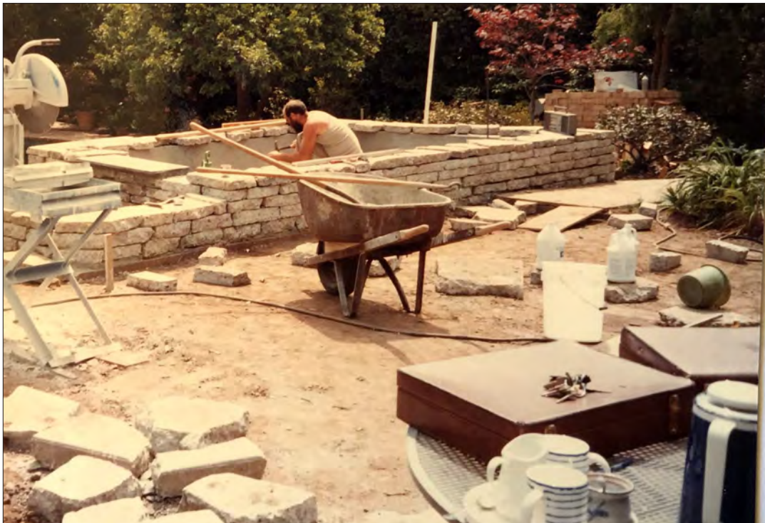
Image 48: Garden, coy pond construction (Ray Borun, 1985)
