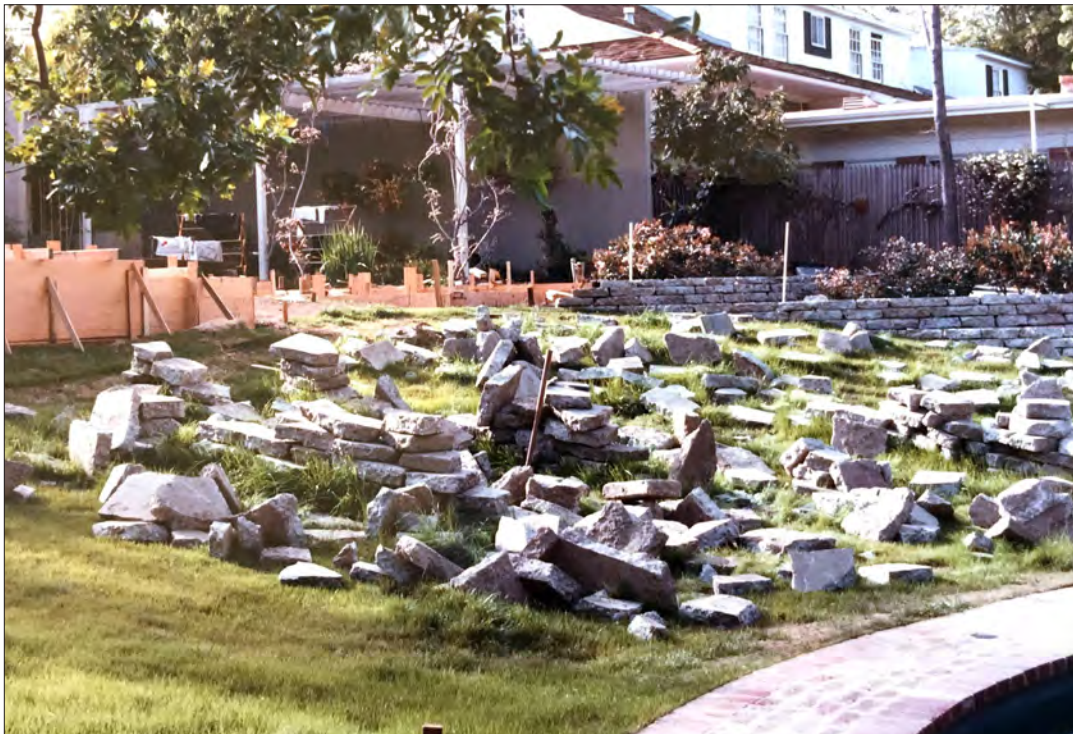
Image 40: Garden renovations (Ray Borun, 1985)
