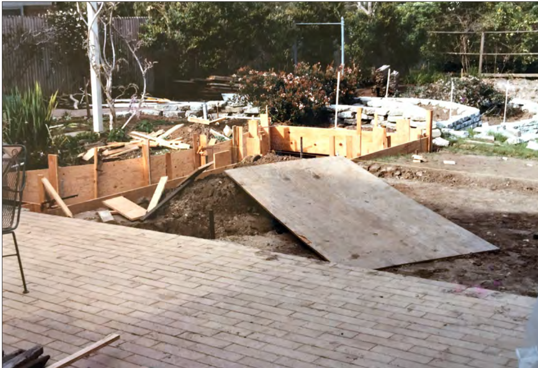
Image 28: Garden, coy pond construction (Ray Borun, 1985)
