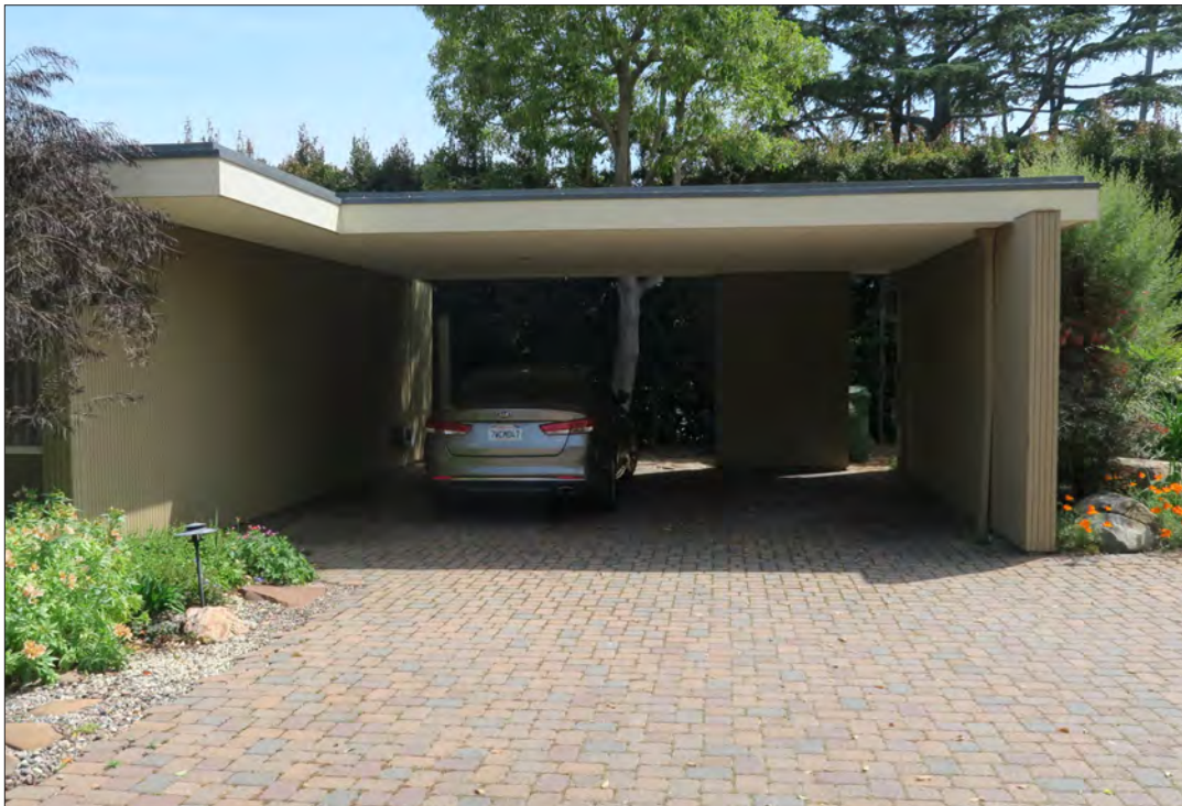
Image 10: Carport, view south (Chattel, 2019)
