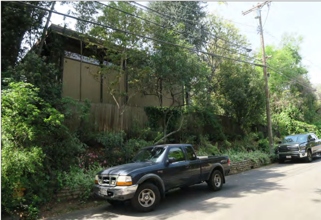
Image 65: Accessory Building, east elevation, view west (Chattel, 2019)
