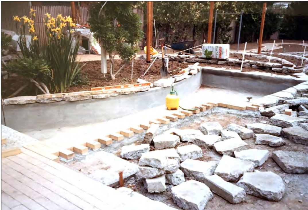
Image 34: Garden, coy pond construction (Ray Borun, 1985)
