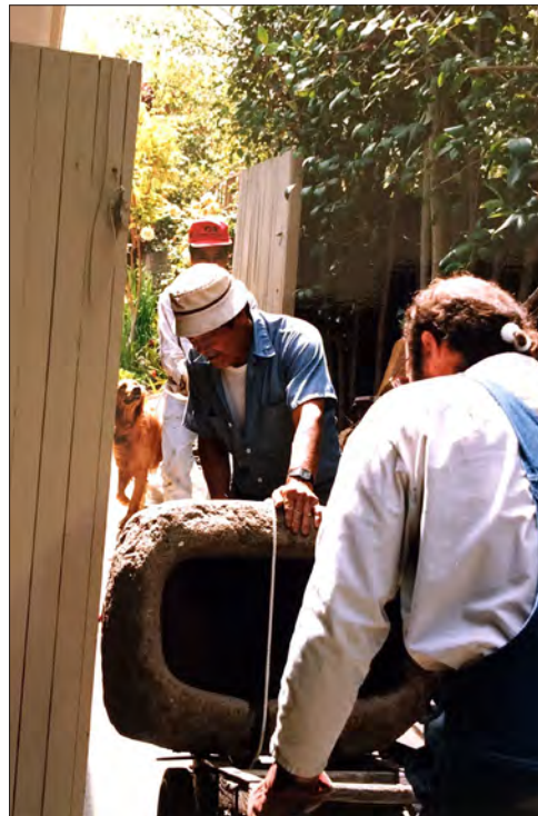
Image 54: Garden renovations (Ray Borun, 1985)
