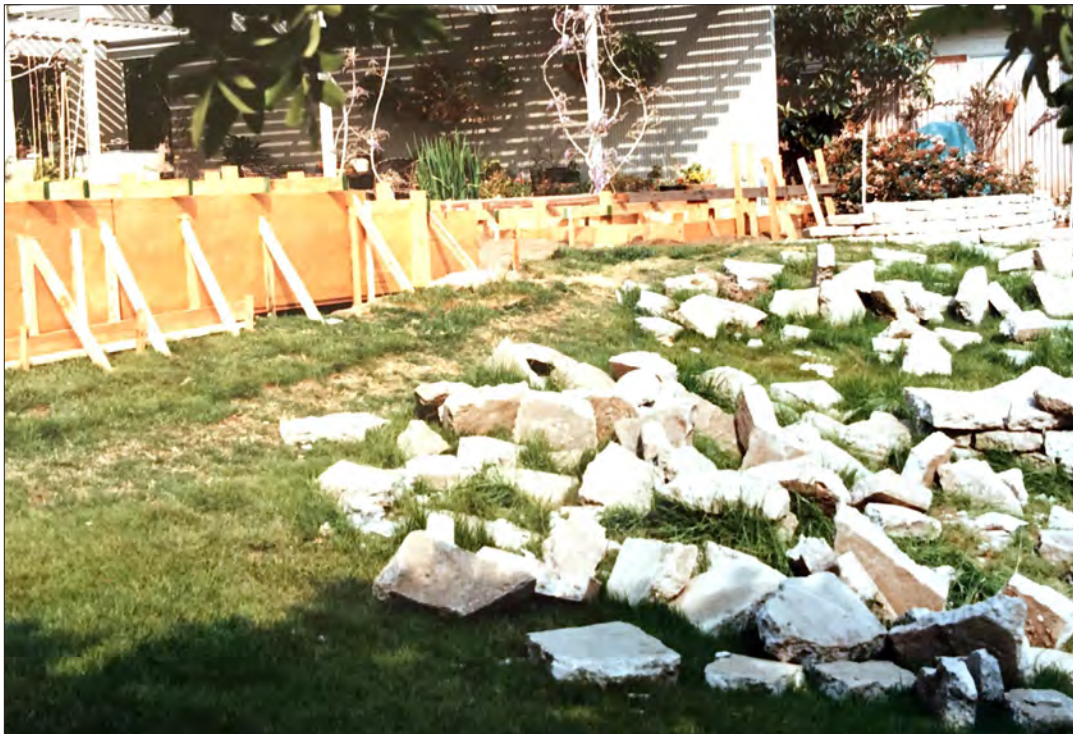
Image 36: Garden renovations (Ray Borun, 1985)
