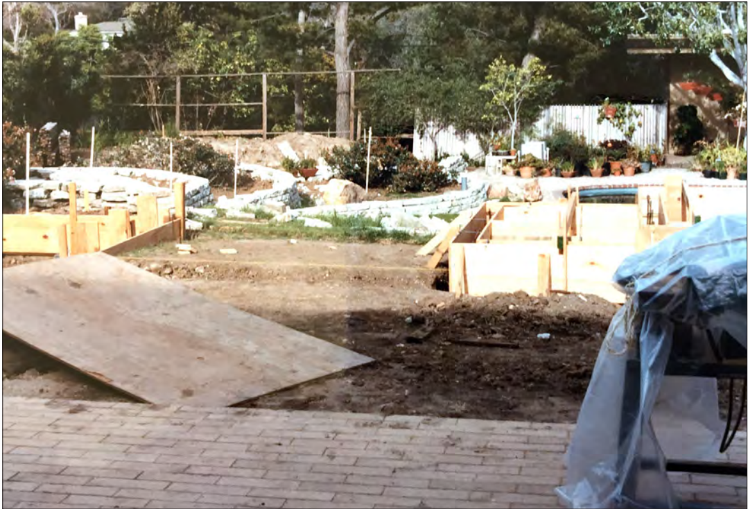
Image 38: Garden, coy pond construction (Ray Borun, 1985)
