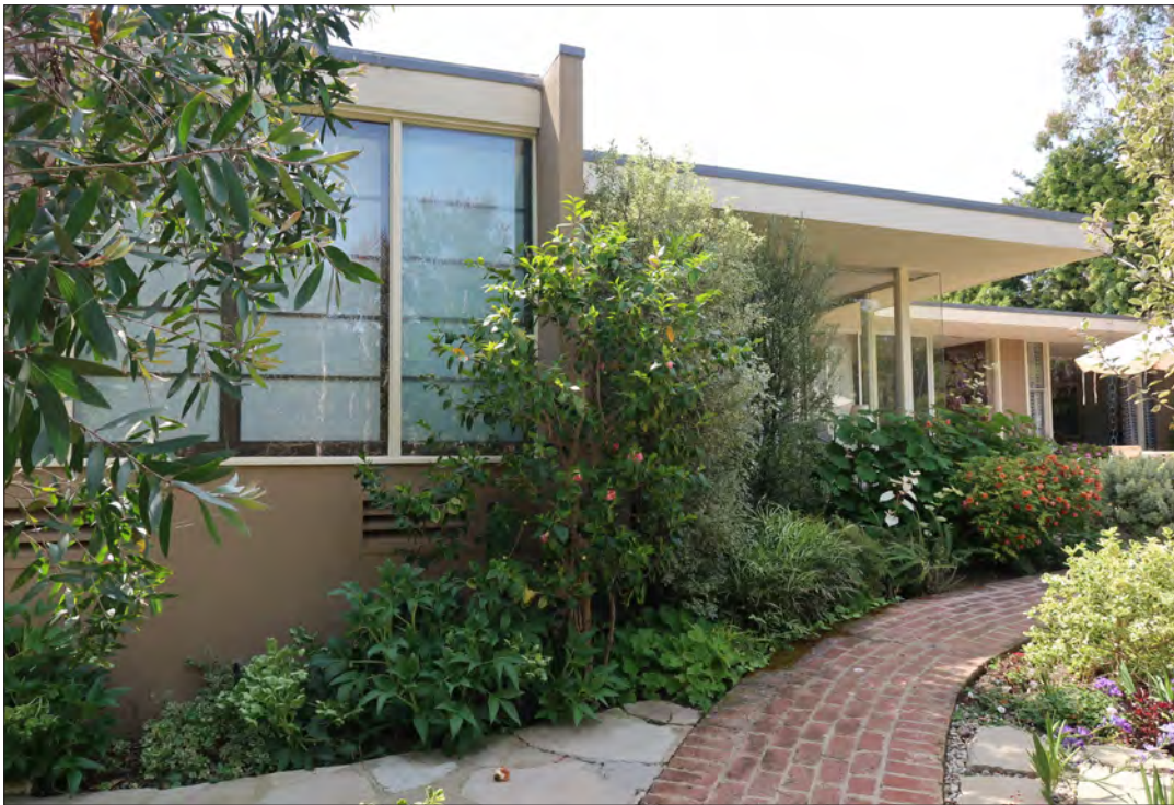
Image 16: East elevation, view northwest (Chattel, 2019)
