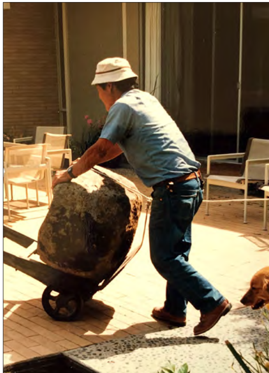
Image 60: Garden renovations (Ray Borun, 1985)
