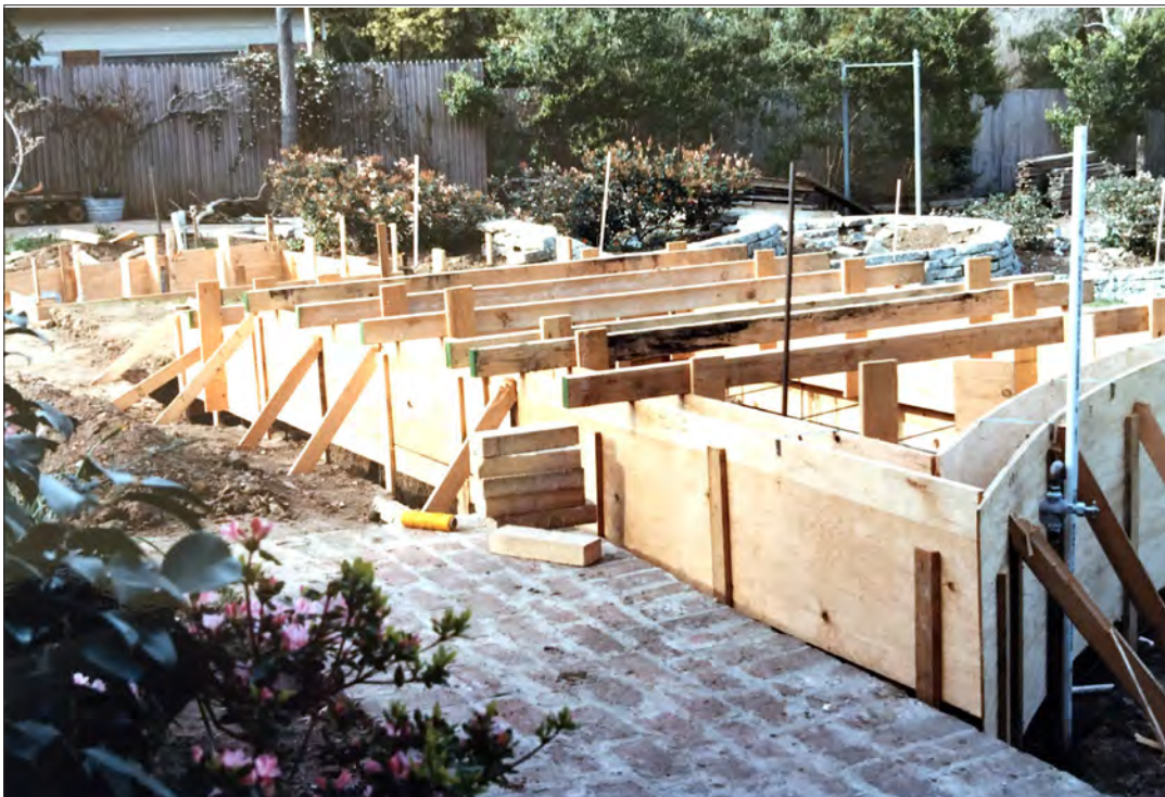
Image 27: Garden, coy pond construction (Ray Borun, 1985)
