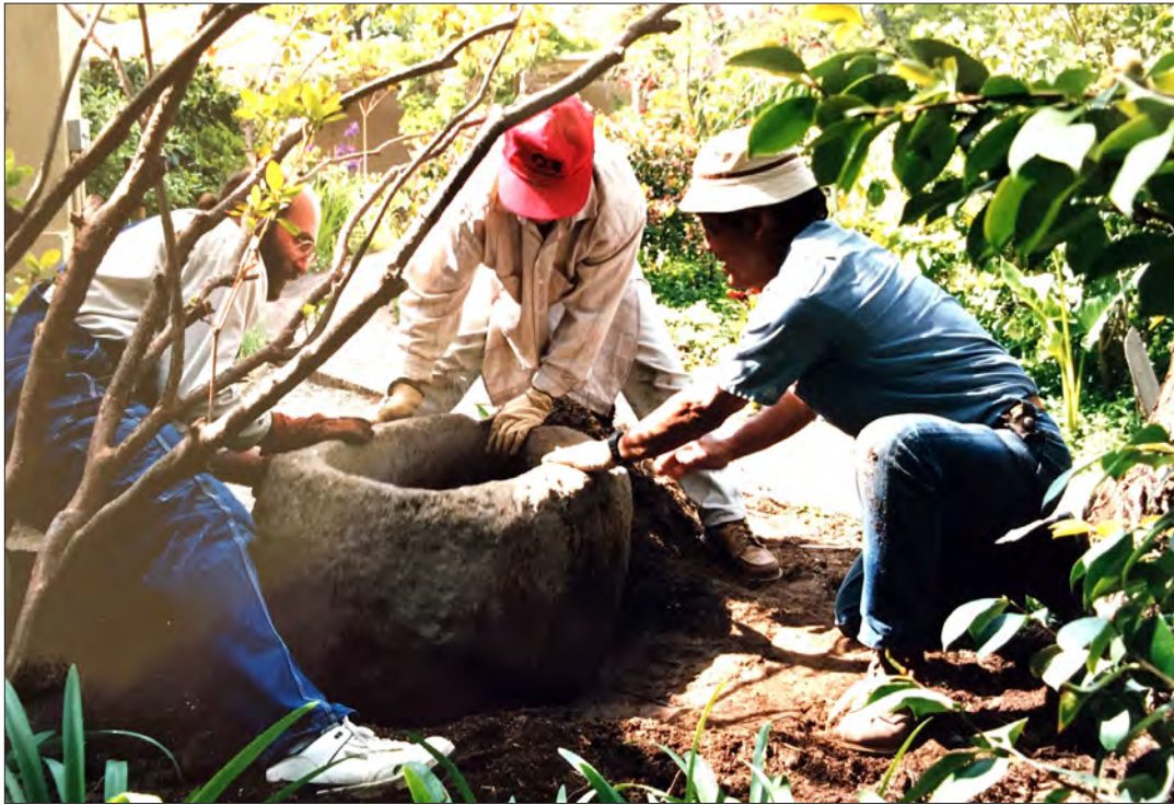
Image 55: Garden renovations (Ray Borun, 1985)
