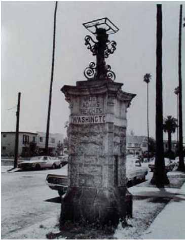
Stone marker placed by West Adams Heights tract realtors at Washington Boulevard. The top portion of the marker has an intricate street lamp with its base made up of steel scrolls.
