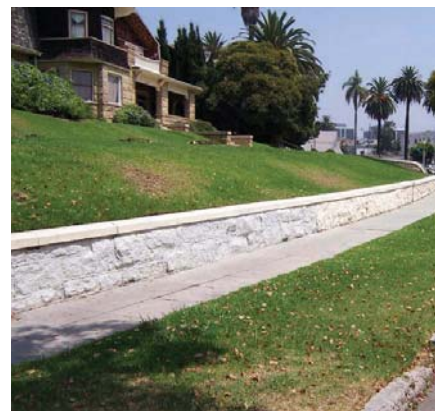
Retaining walls are an important part of the neighborhood streetscape.
