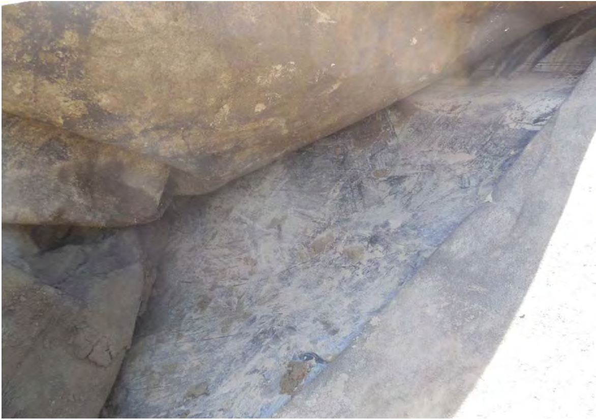
Photo 9 - The liner surface was inspected to confirm that the liner was undamaged.
