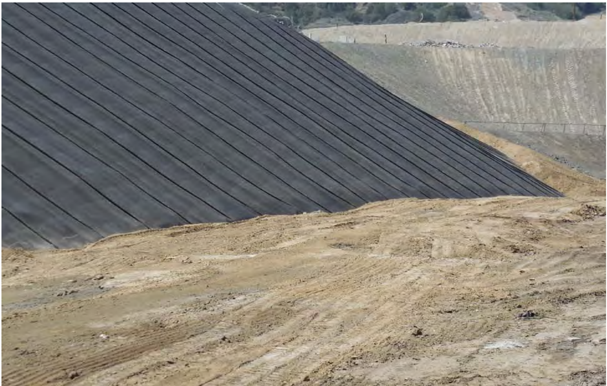
Photo 12 - The protective soil was replaced.
