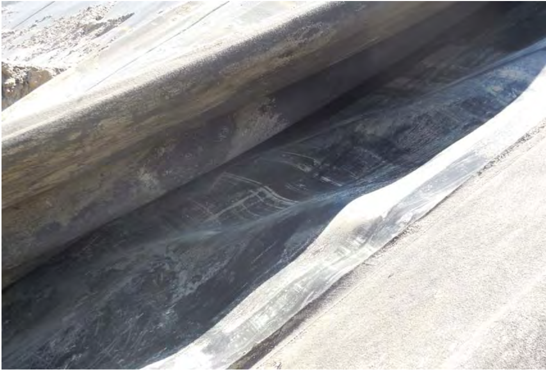
Photo 7 - The liner surface was inspected to confirm that the liner was undamaged.
