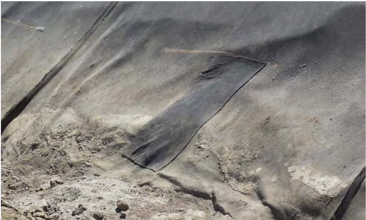
Photo 10 - The geotextile was repaired.
