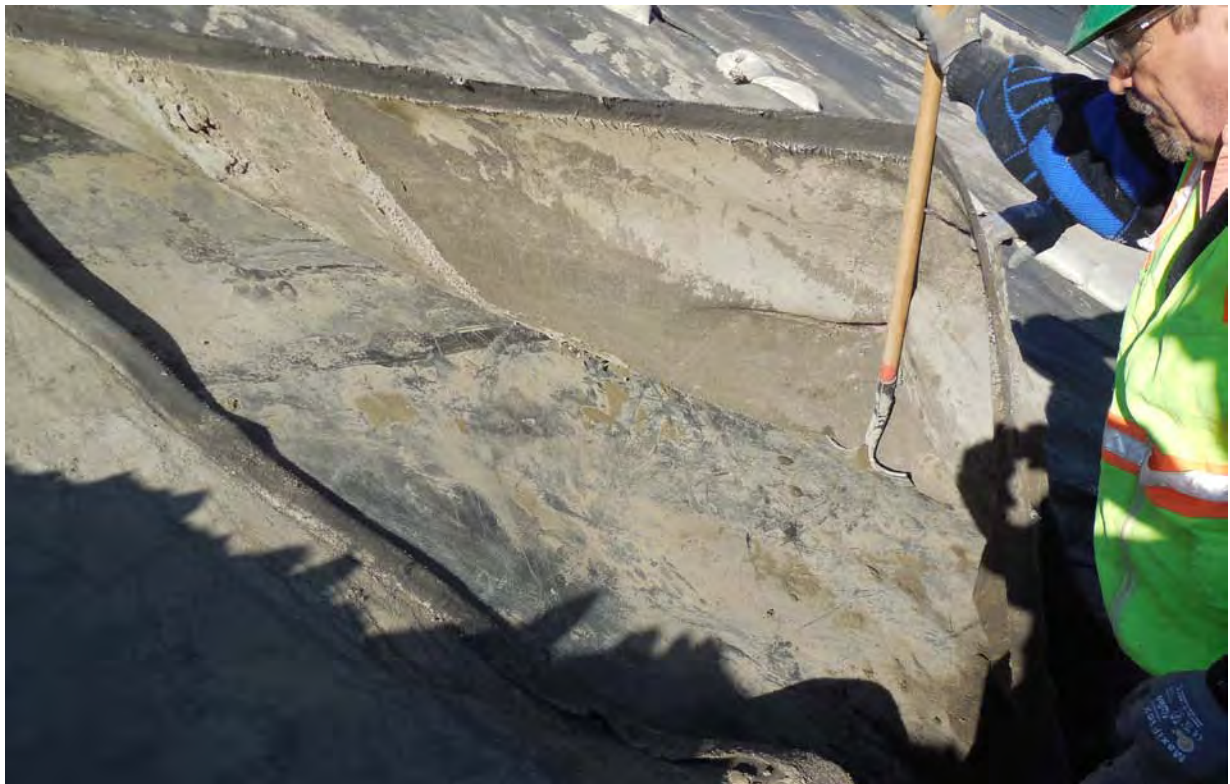
Photo 8 - The liner surface was inspected to confirm that the liner was undamaged.
