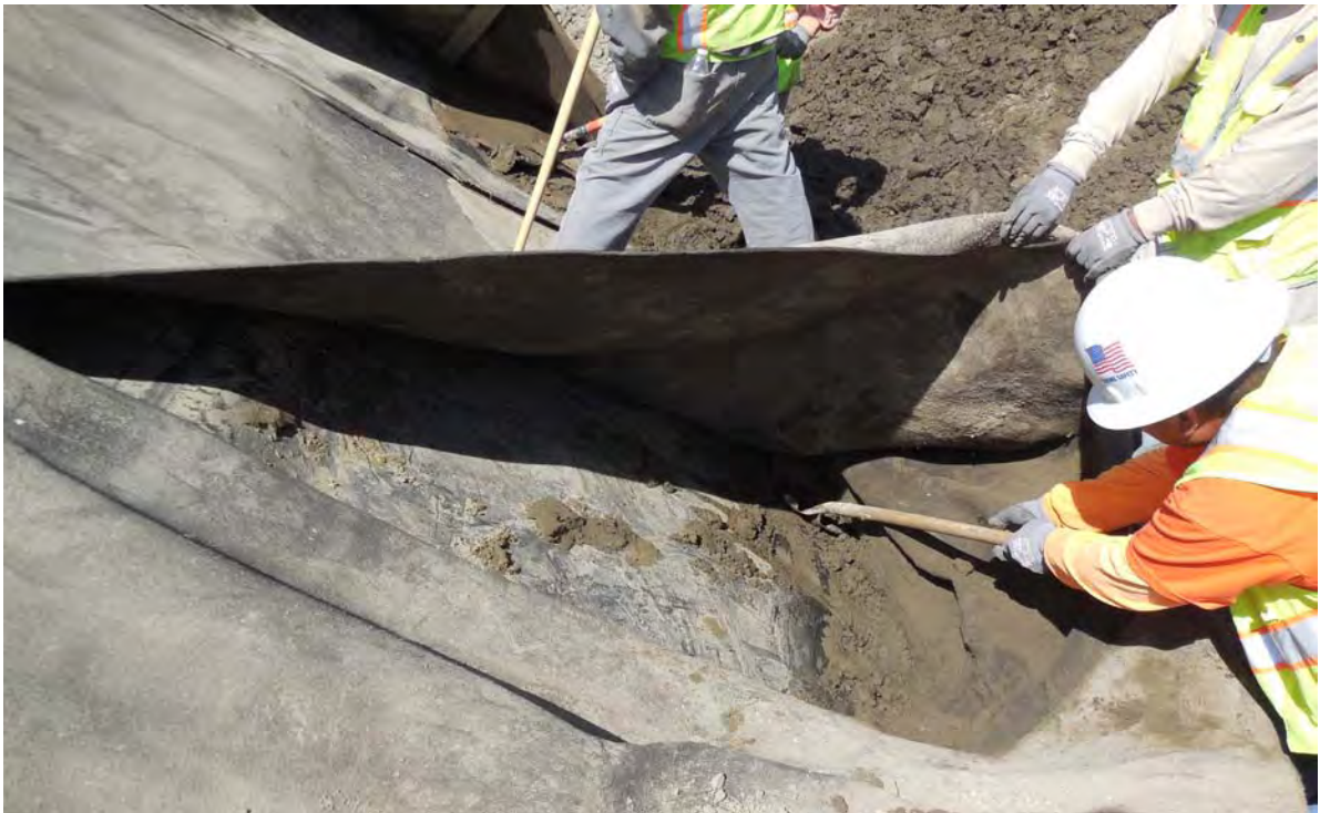
Photo 6 - Fine-grained soils were removed.
