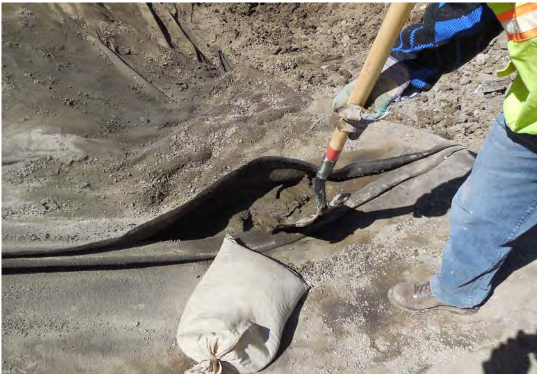
Photo 4 - Fine-grained soils were observed under the geotextile.
