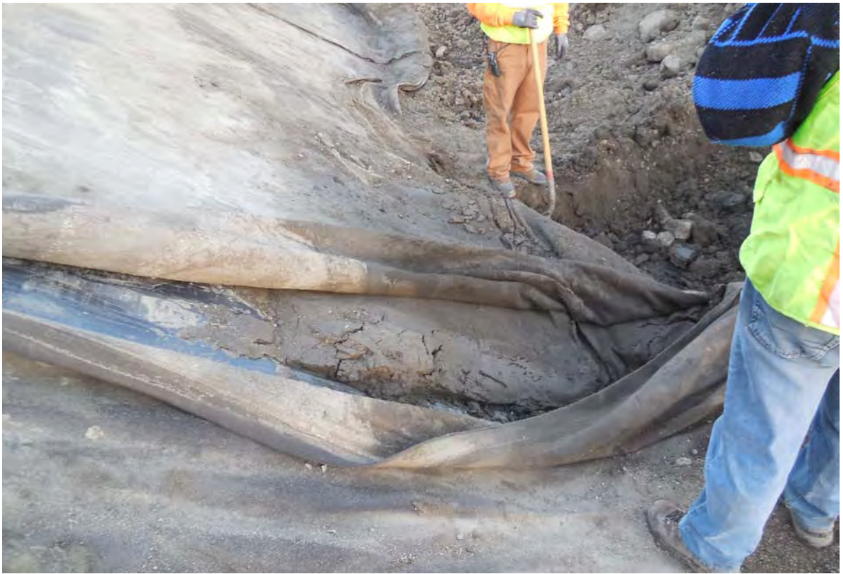
Photo 5 - Fine-grained soils were observed under the geotextile.
