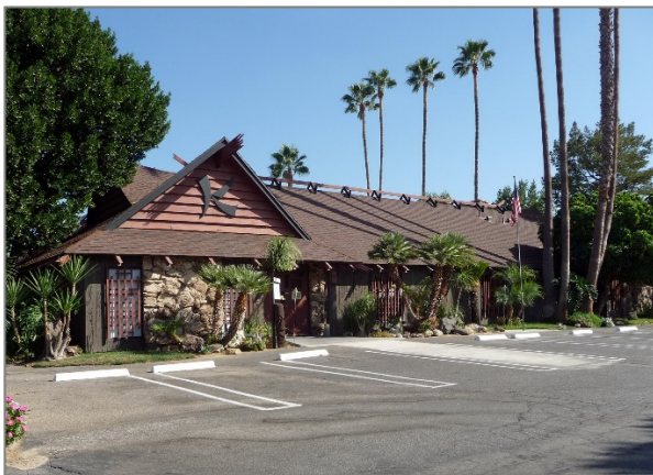
Name: Kona Kai Village (recreation building)
