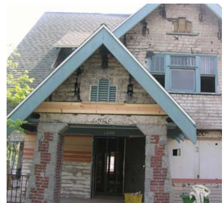
This house has recently been emancipated from a layer of stucco, exposing ornate and beautiful materials.
