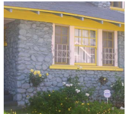
Stone and masonry should always be left to exhibit their natural finish qualities. Painting over the Arroyo stone on this house has muted the stone's texture.
