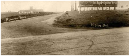
Wilshire Boulevard and Rimpau Boulevard, 1919.
