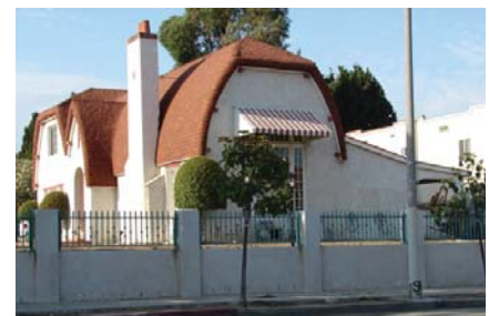
The pitch, rolled-eaves, brackets, and unique materials are all components of this roof that should be preserved.
