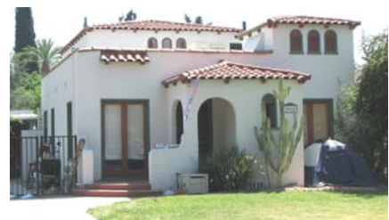
This second-story addition is set-back and preserving the look and scale of the original bungalow.
