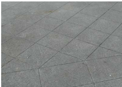
Original concrete texture and score patterns are an important part of the neighborhood.
