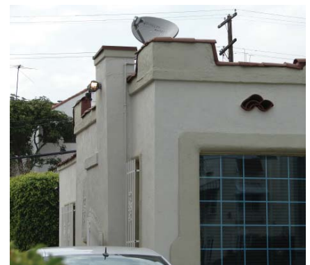
Television antennae and satellite dishes create an unnecessary visual obstruction and should be placed out of sight-
