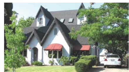
This second-story addition, with its noticeable dormers, calls attention to itself, overwhelming the original cottage.
