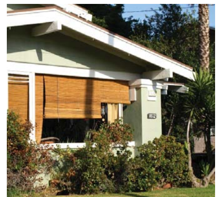
Non-permanent devices such as this bamboo screen may effectively screen a porch without altering the home and disrupting the streetscape.
