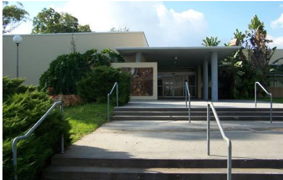
Address: 1111 South Figueroa Place Name: Harbor College Administration Building Date: 1963
