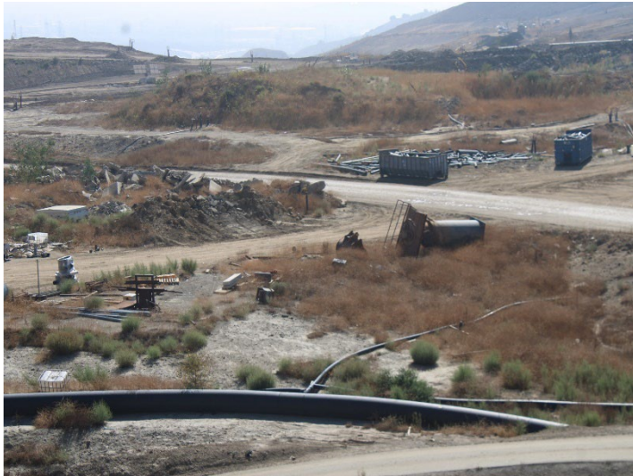
Photo 497: General Site: October 8, 2025
