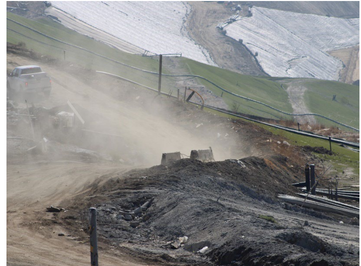
Photo 488: General Site: October 8, 2025
