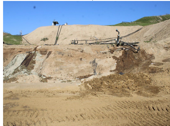
Photo 76: Working Area, CC-4 Part 4/5, CC-5A: October 8, 2025
