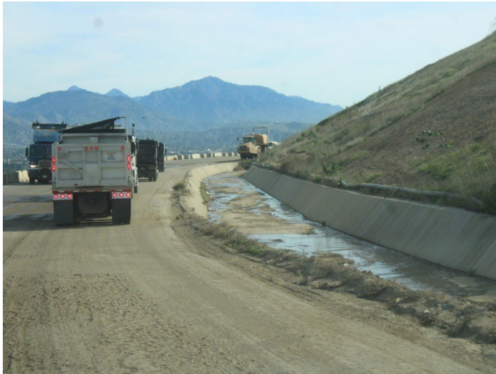
Photo 249: County Sage Mitigation Area and Westside Drainage Channels: December 18, 2025
