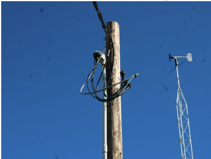
Photo 543: General Site: November 6, 2025
