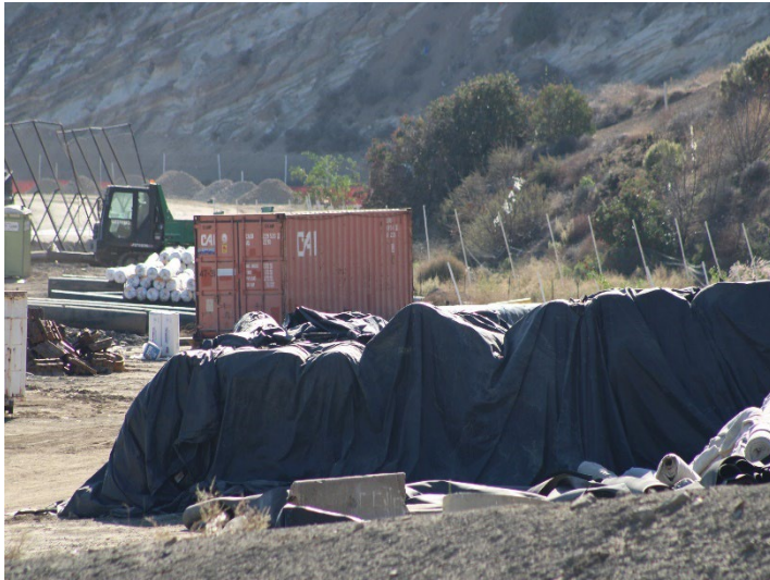
Photo 529: General Site: November 6, 2025
