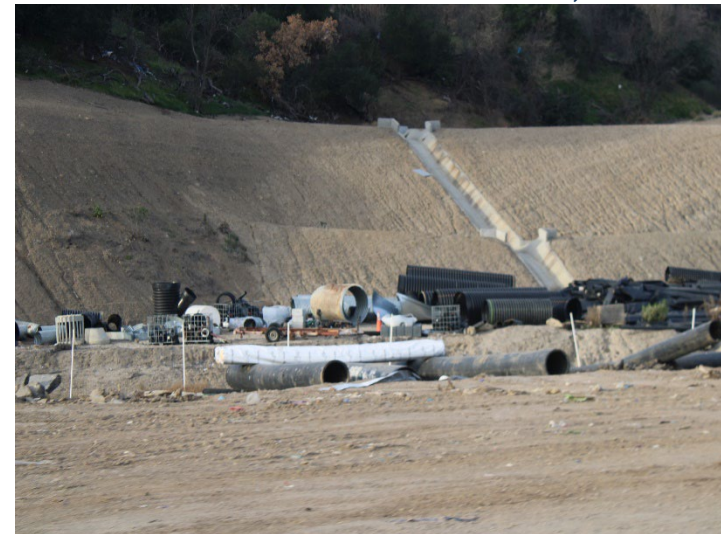
Photo 560: General Site: December 18, 2025
