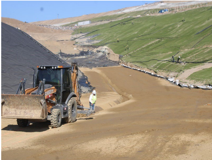
Photo 97: Working Area, CC-4 Part 4/5, CC-5A: October 8, 2025
