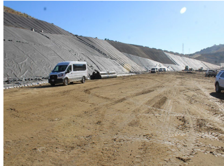
Photo 146: Working Area, CC-4 Part 4/5, CC-5A: November 6, 2025
