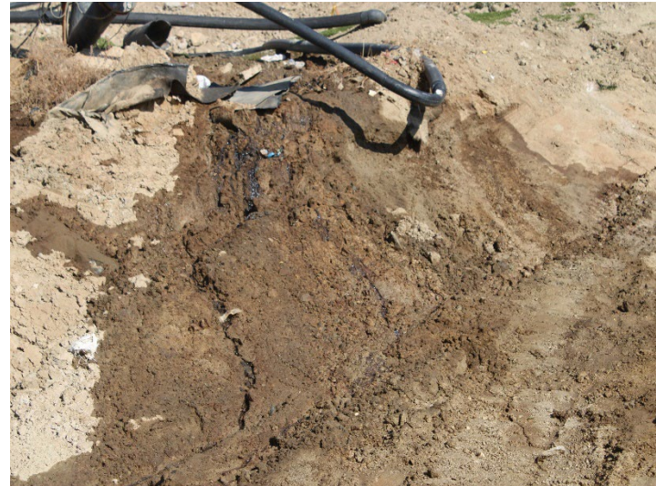
Photo 78: Working Area, CC-4 Part 4/5, CC-5A: October 8, 2025
