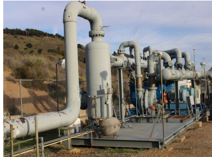
Photo 562: General Site: December 18, 2025
