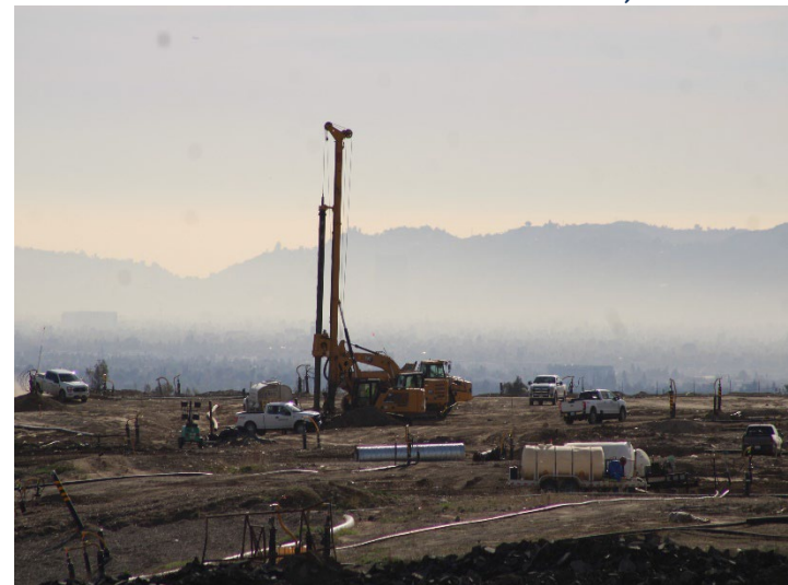
Photo 608: General Site: December 18, 2025
