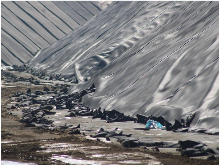
Photo 93: Working Area, CC-4 Part 4/5, CC-5A: October 8, 2025
