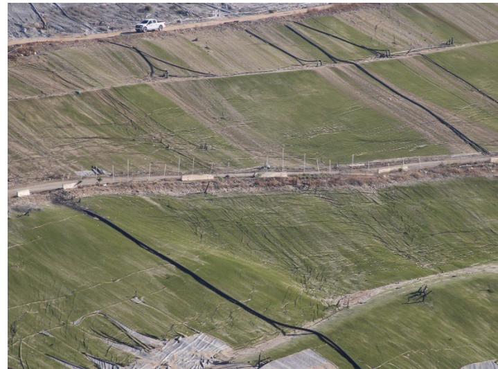
Photo 212: Closure Turf: October 8, 2025
