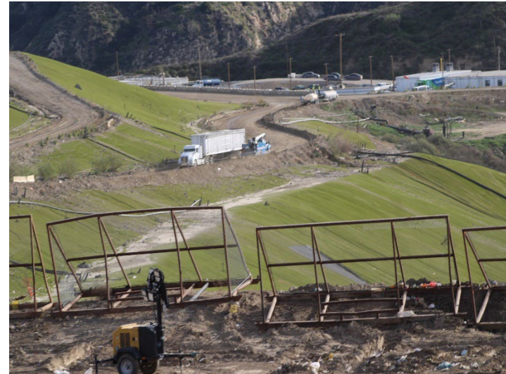
Photo 586: General Site: December 18, 2025
