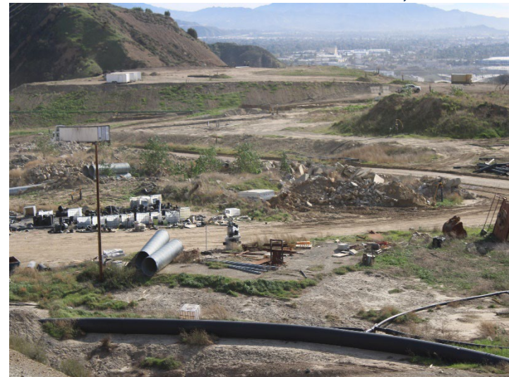
Photo 600: General Site: December 18, 2025
