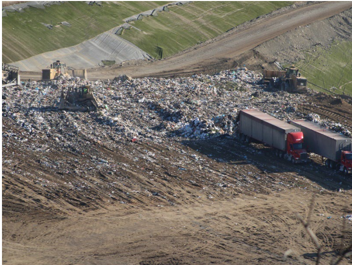
Photo 69: Working Area, CC-4 Part 4/5, CC-5A: October 8, 2025
