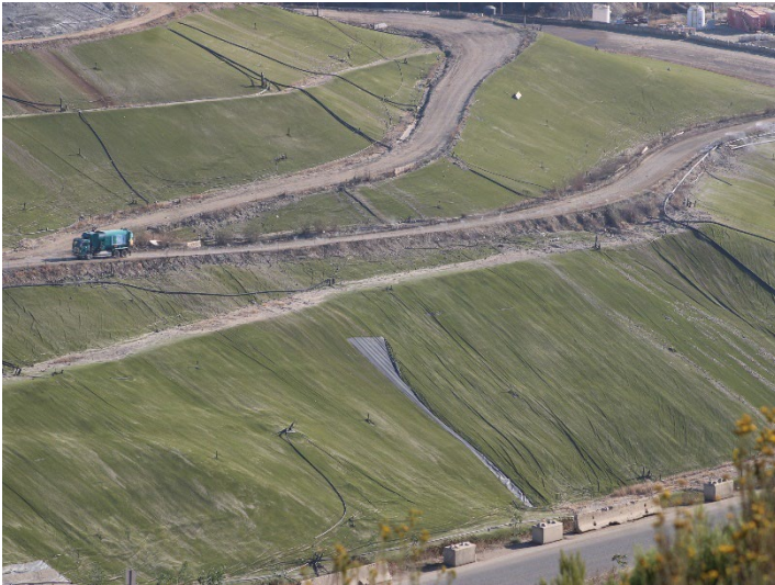
Photo 213: Closure Turf: October 8, 2025
