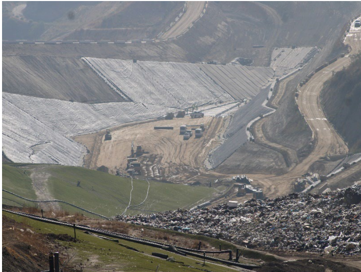
Photo 113: Working Area, CC-4 Part 4/5, CC-5A: October 8, 2025
