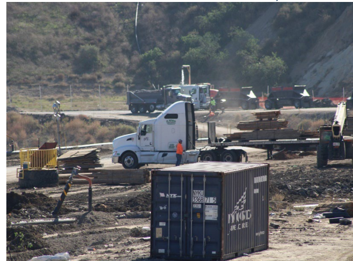
Photo 528: General Site: November 6, 2025
