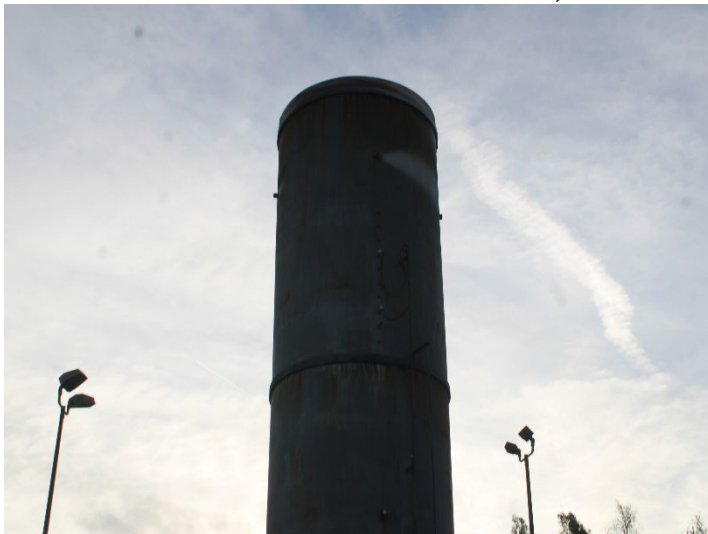
Photo 555: General Site: December 18, 2025
