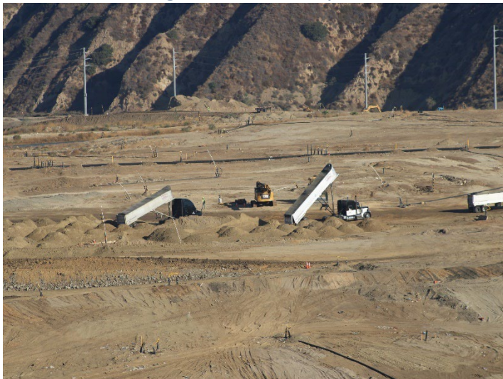
Photo 19: Working Area, CC4 Part 1/2: October 8, 2025
