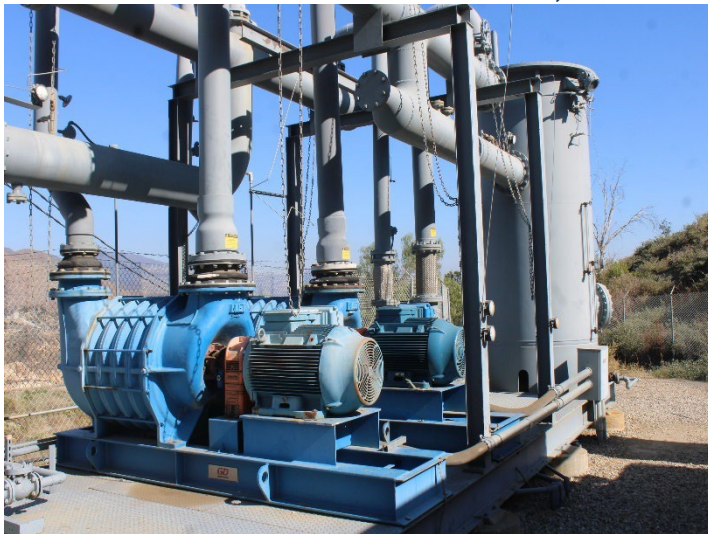
Photo 551: General Site: November 6, 2025
