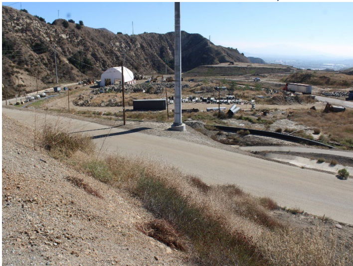
Photo 531: General Site: November 6, 2025
