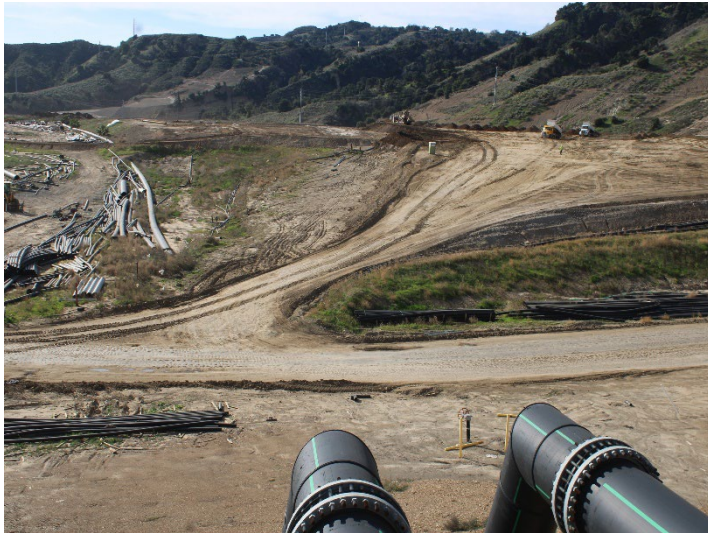
Photo 597: General Site: December 18, 2025
