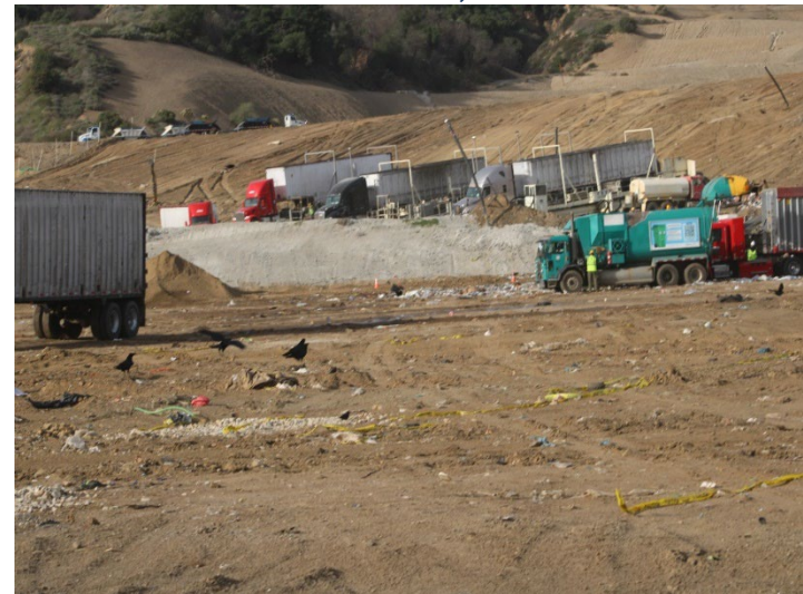
Photo 180: Working Area, CC-4 Part 4/5, CC-5A: December 18, 2025
