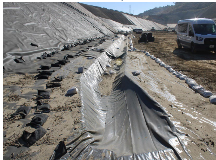
Photo 148: Working Area, CC-4 Part 4/5, CC-5A: November 6, 2025
