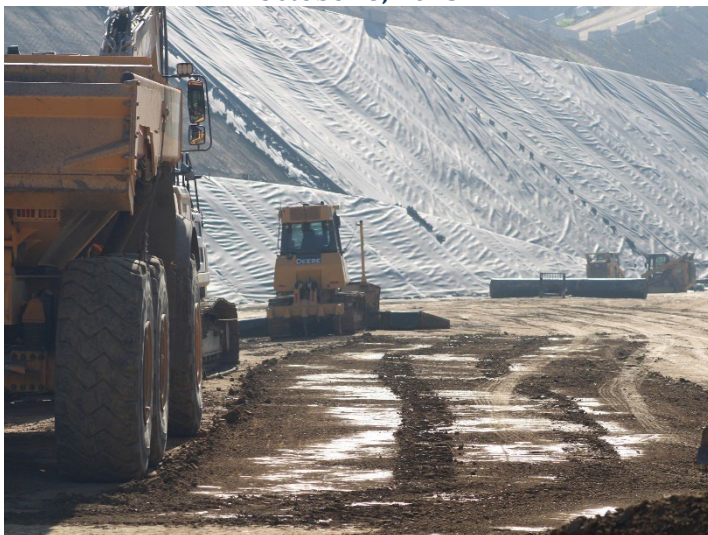
Photo 91: Working Area, CC-4 Part 4/5, CC-5A: October 8, 2025
