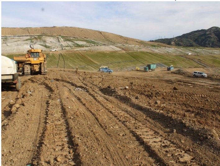
Photo 579: General Site: December 18, 2025
