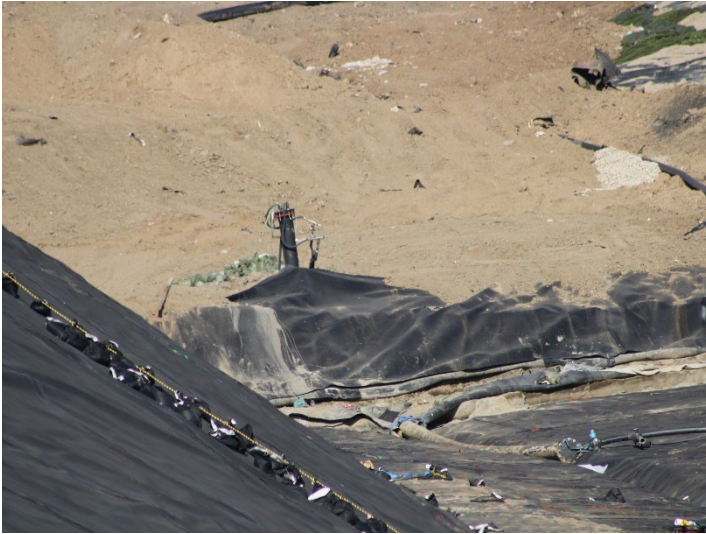
Photo 109: Working Area, CC-4 Part 4/5, CC-5A: October 8, 2025
