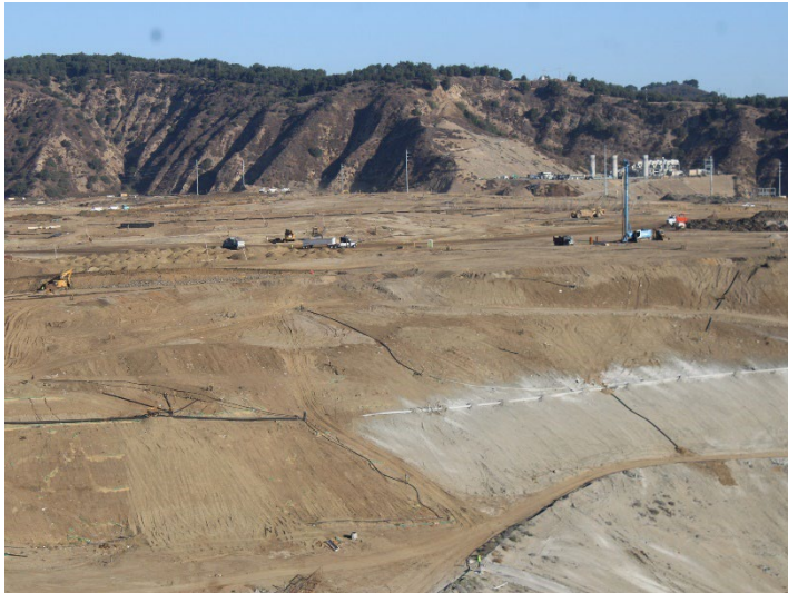
Photo 57: Working Area, CC-4 Part 4/5, CC-5A: October 8, 2025
