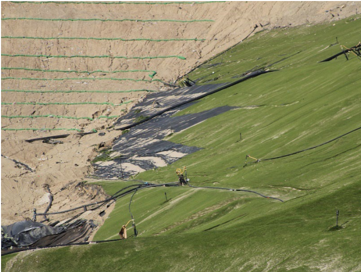
Photo 221: Closure Turf: December 18, 2025
