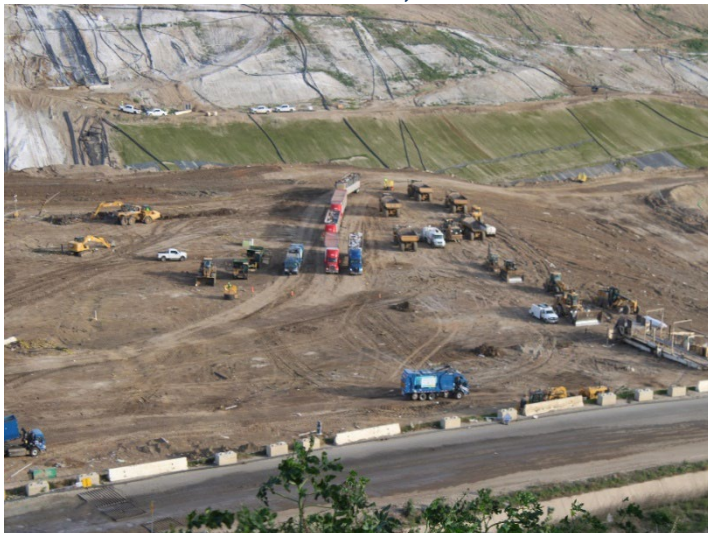
Photo 167: Working Area, CC-4 Part 4/5, CC-5A: December 18, 2025
