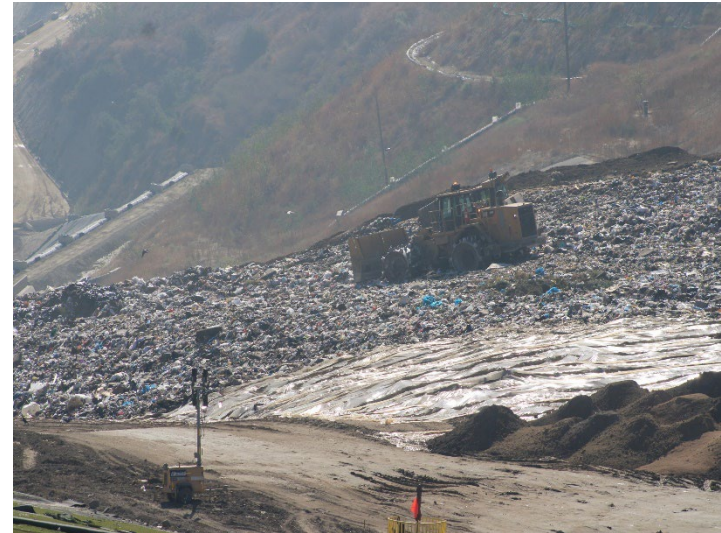
Photo 114: Working Area, CC-4 Part 4/5, CC-5A: October 8, 2025
