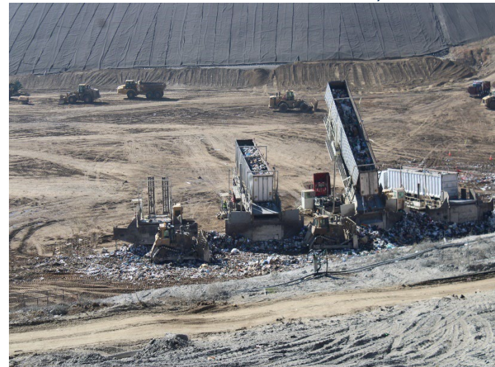
Photo 484: General Site: October 8, 2025
