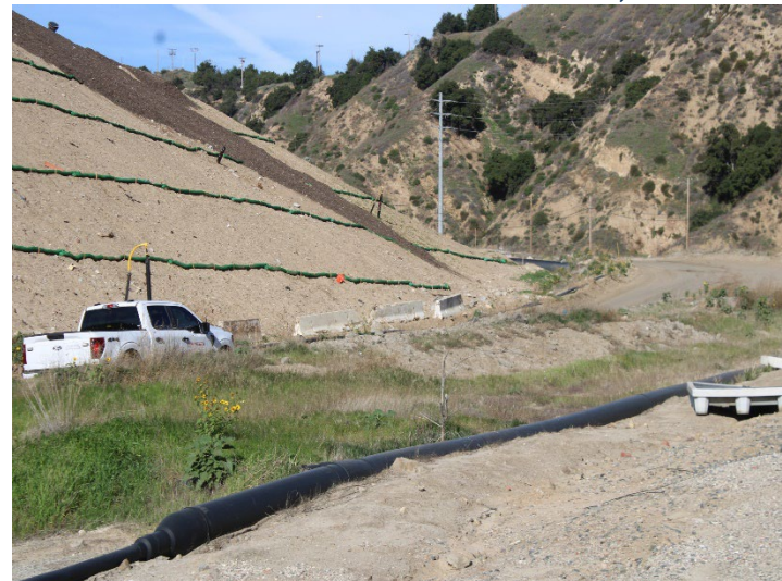
Photo 592: General Site: December 18, 2025
