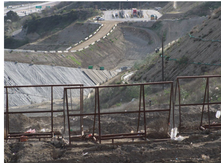
Photo 184: Working Area, CC-4 Part 4/5, CC-5A: December 18, 2025
