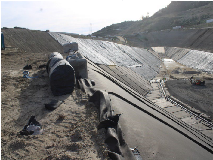
Photo 187: Working Area, CC-4 Part 4/5, CC-5A: December 18, 2025
