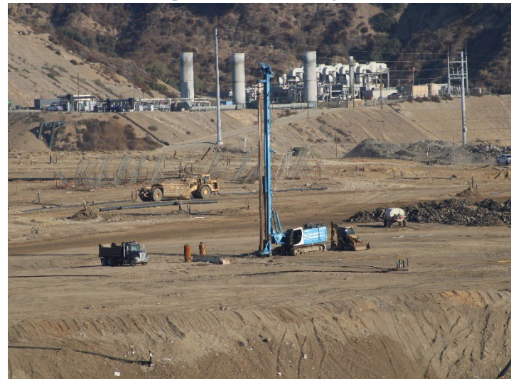
Photo 20: Working Area, CC4 Part 1/2: October 8, 2025
