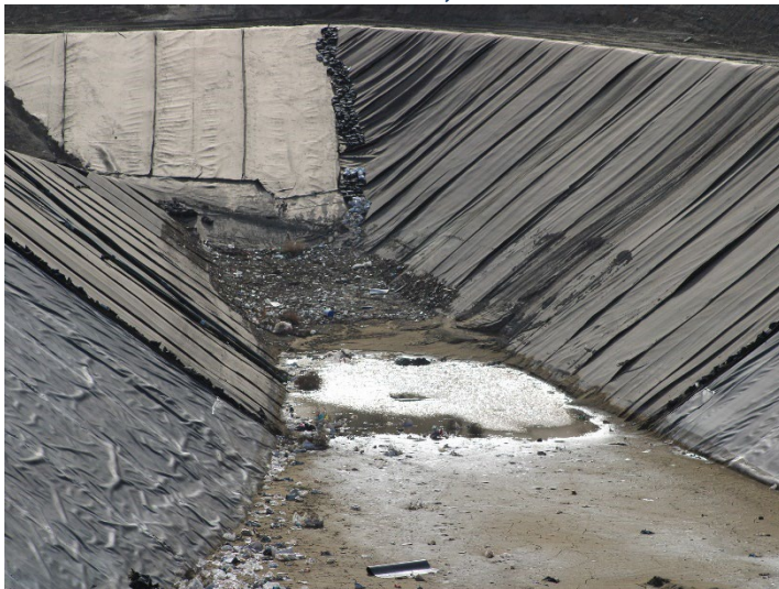
Photo 203: Working Area, CC-4 Part 4/5, CC-5A: December 18, 2025
