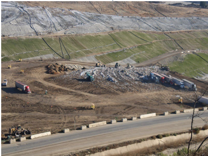
Photo 55: Working Area, CC-4 Part 4/5, CC-5A: October 8, 2025
