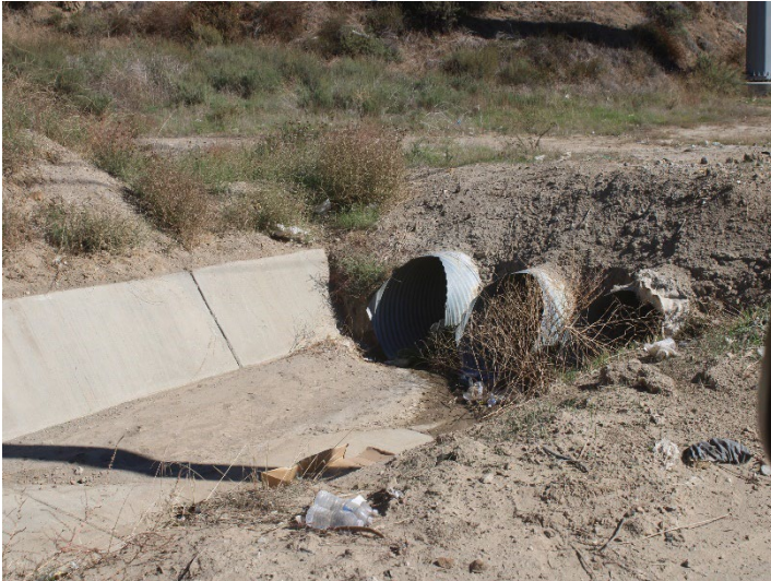
Photo 359: Eastside Drainage Channel: November 6, 2025
