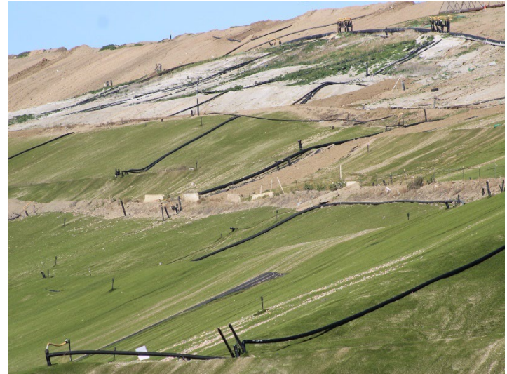
Photo 222: Closure Turf: December 18, 2025
