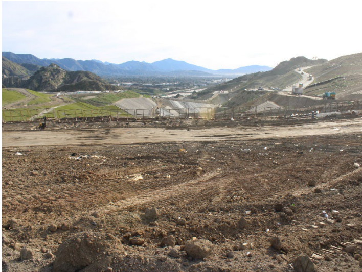
Photo 581: General Site: December 18, 2025
