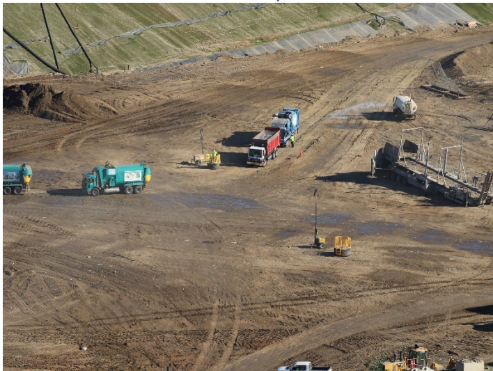
Photo 139: Working Area, CC-4 Part 4/5, CC-5A: November 6, 2025
