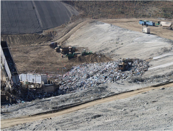
Photo 485: General Site: October 8, 2025
