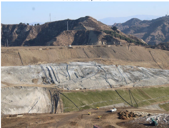
Photo 59: Working Area, CC-4 Part 4/5, CC-5A: October 8, 2025
