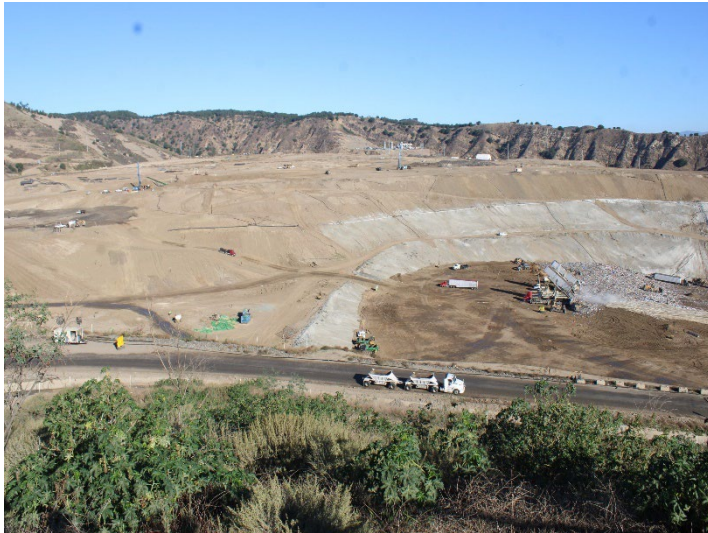
Photo 525: General Site: November 6, 2025
