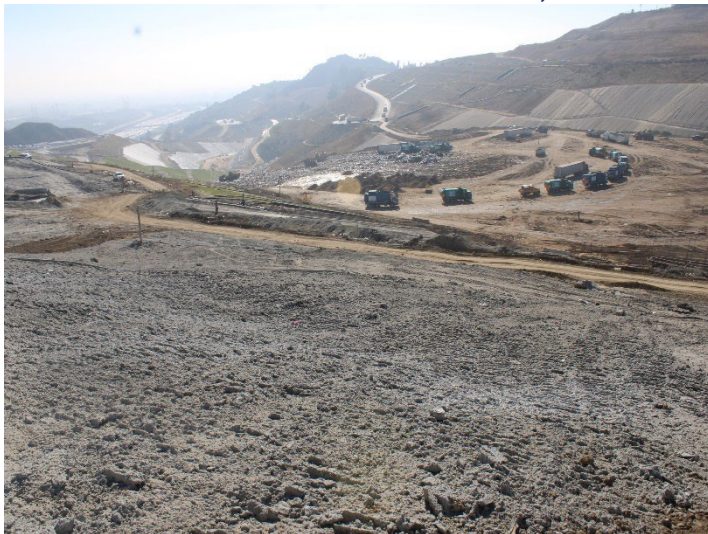
Photo 475: General Site: October 8, 2025
