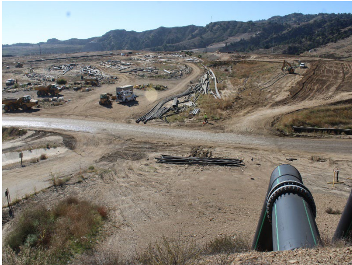
Photo 533: General Site: November 6, 2025
