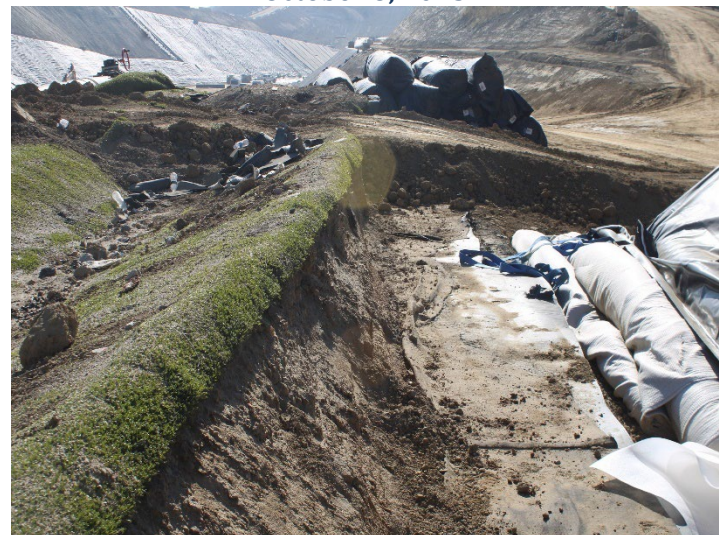
Photo 100: Working Area, CC-4 Part 4/5, CC-5A: October 8, 2025
