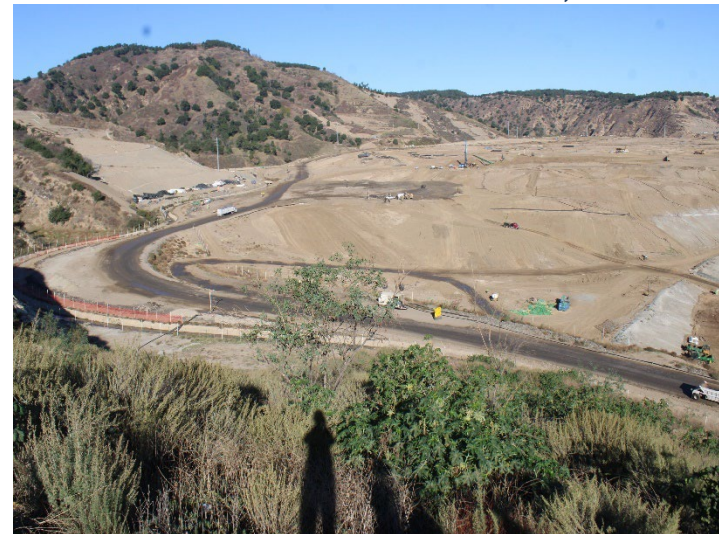
Photo 524: General Site: November 6, 2025
