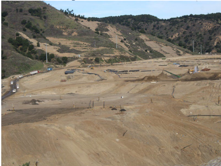
Photo 47: Working Area, CC-4 Part 3: December 18, 2025
