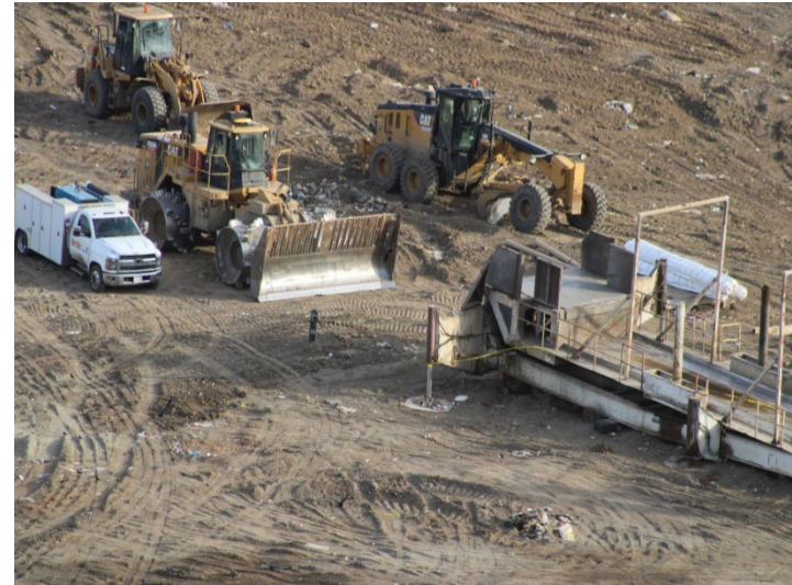
Photo 178: Working Area, CC-4 Part 4/5, CC-5A: December 18, 2025
