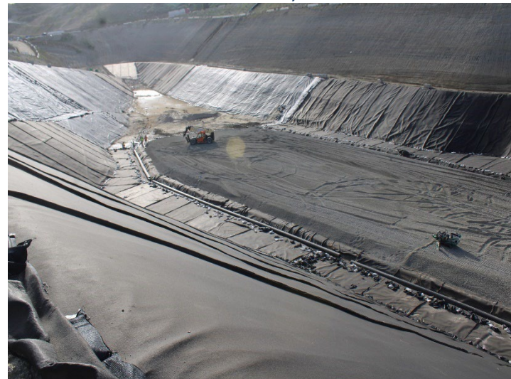
Photo 188: Working Area, CC-4 Part 4/5, CC-5A: December 18, 2025
