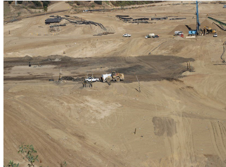
Photo 134: Working Area, CC-4 Part 4/5, CC-5A: November 6, 2025
