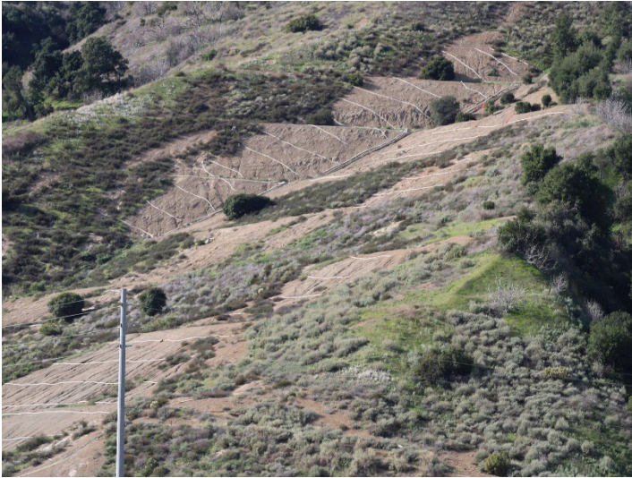
Photo 245: County Sage Mitigation Area and Westside Drainage Channels: December 18, 2025
