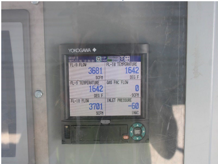
Photo 267: Flares 9, 10, 11 and Gas-to-Energy Facility: November 6, 2025
