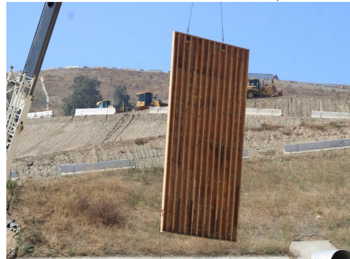
Photo 396: Terminal Basin: October 8, 2025
