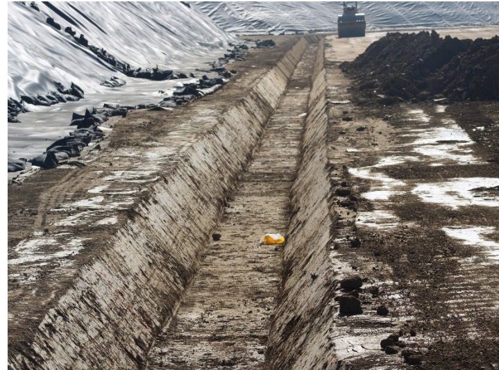
Photo 94: Working Area, CC-4 Part 4/5, CC-5A: October 8, 2025
