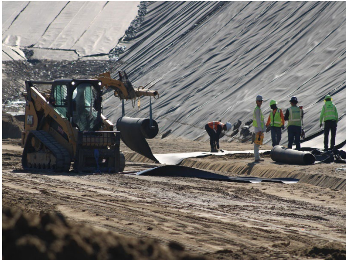
Photo 161: Working Area, CC-4 Part 4/5, CC-5A: November 6, 2025
