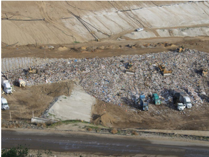
Photo 165: Working Area, CC-4 Part 4/5, CC-5A: December 18, 2025
