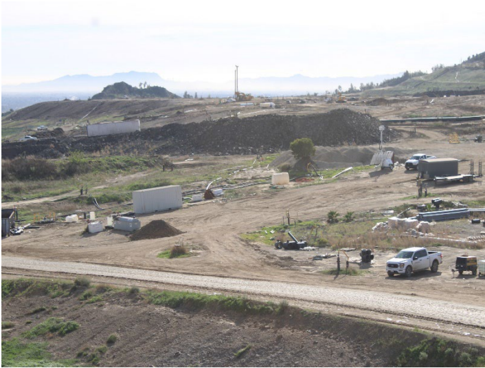
Photo 601: General Site: December 18, 2025
