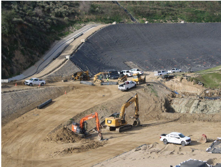
Photo 197: Working Area, CC-4 Part 4/5, CC-5A: December 18, 2025
