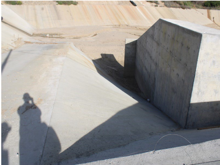
Photo 417: Terminal Basin: December 18, 2025
