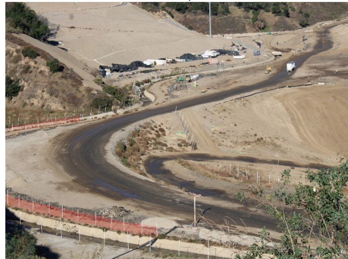
Photo 128: Working Area, CC-4 Part 4/5, CC-5A: November 6, 2025
