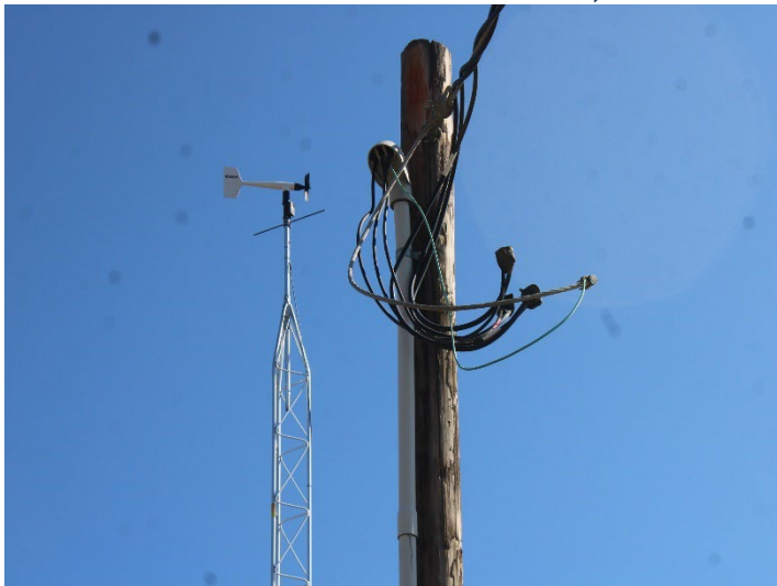
Photo 511: General Site: October 8, 2025
