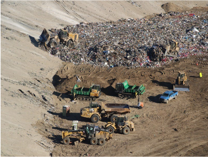
Photo 65: Working Area, CC-4 Part 4/5, CC-5A: October 8, 2025
