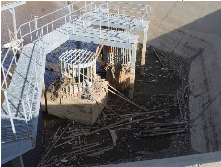
Photo 423: Terminal Basin: December 18, 2025
