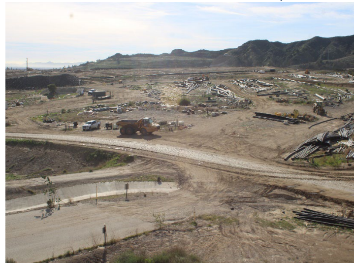
Photo 596: General Site: December 18, 2025
