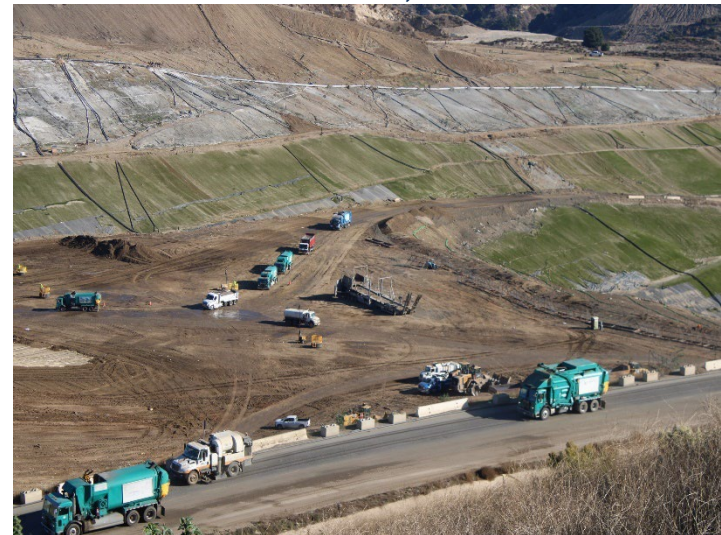
Photo 132: Working Area, CC-4 Part 4/5, CC-5A: November 6, 2025
