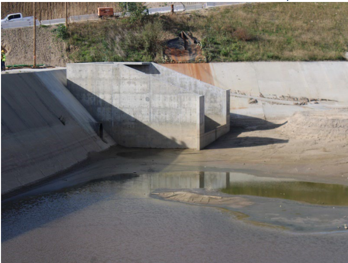
Photo 427: Terminal Basin: December 18, 2025
