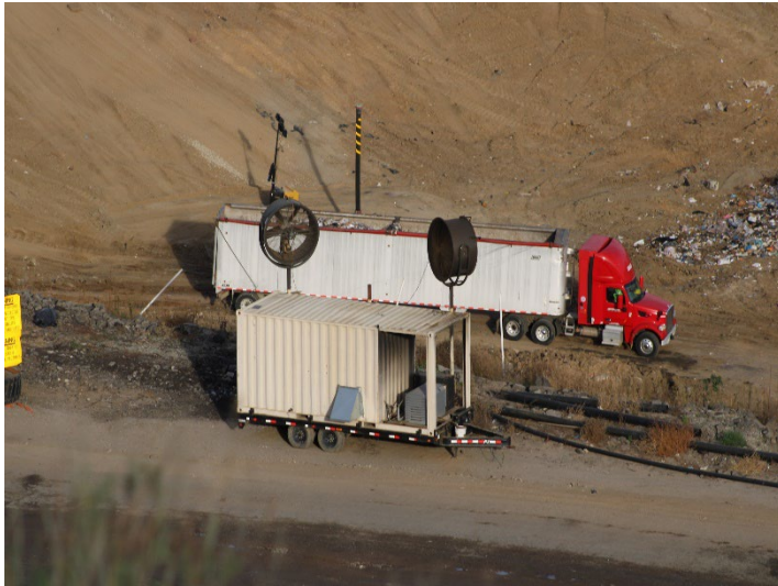
Photo 577: General Site: December 18, 2025
