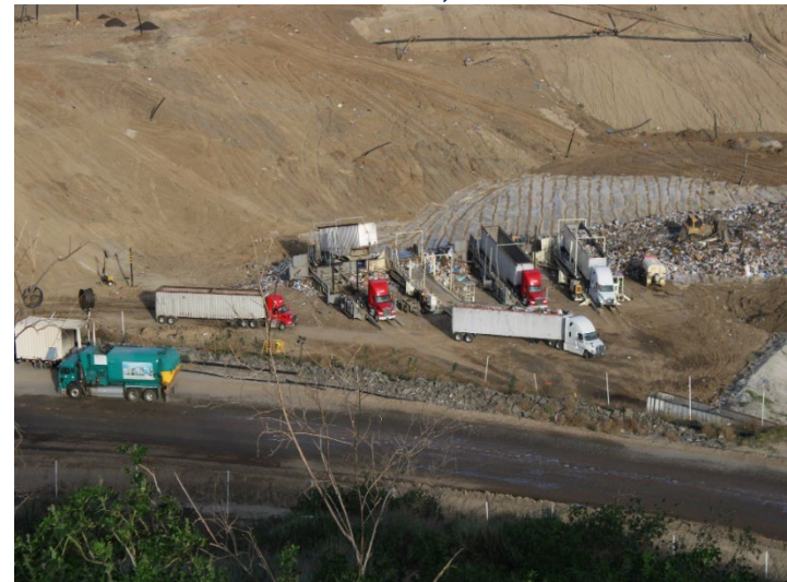
Photo 164: Working Area, CC-4 Part 4/5, CC-5A: December 18, 2025
