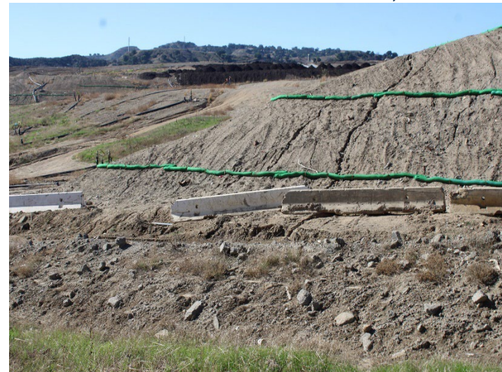
Photo 548: General Site: November 6, 2025
