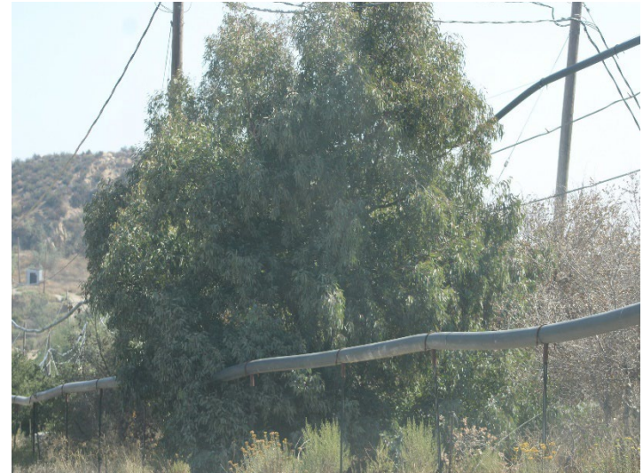
Photo 454: Southern Ownership Buffer: October 8, 2025
