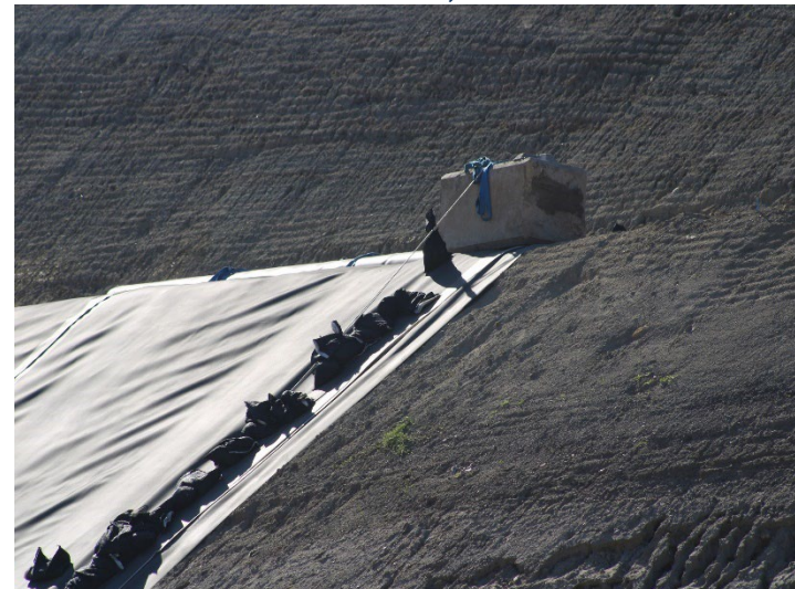
Photo 160: Working Area, CC-4 Part 4/5, CC-5A: November 6, 2025
