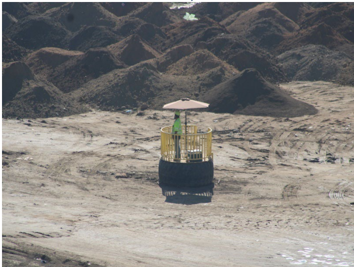
Photo 127: Working Area, CC-4 Part 4/5, CC-5A: October 8, 2025
