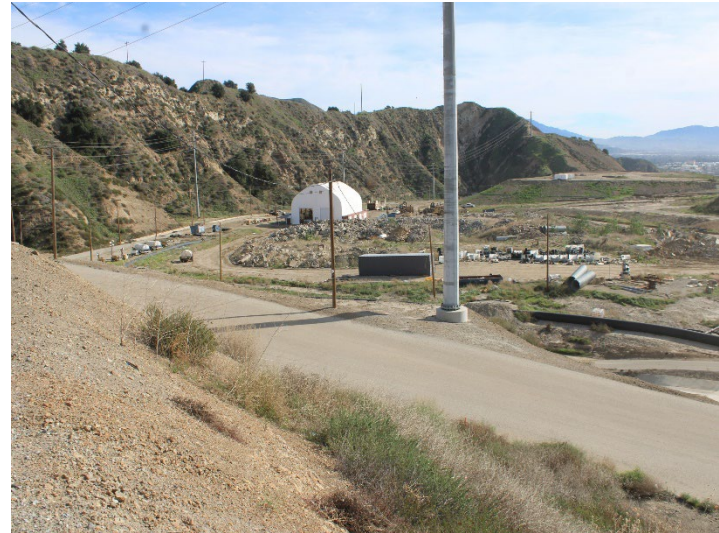
Photo 594: General Site: December 18, 2025
