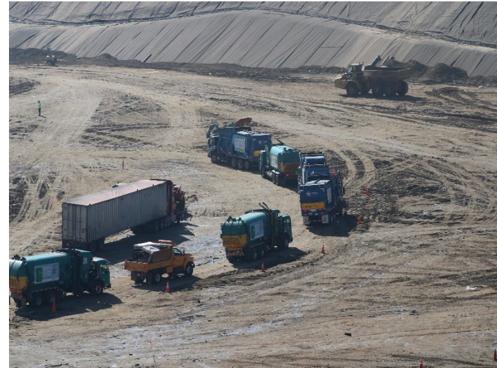
Photo 118: Working Area, CC-4 Part 4/5, CC-5A: October 8, 2025
