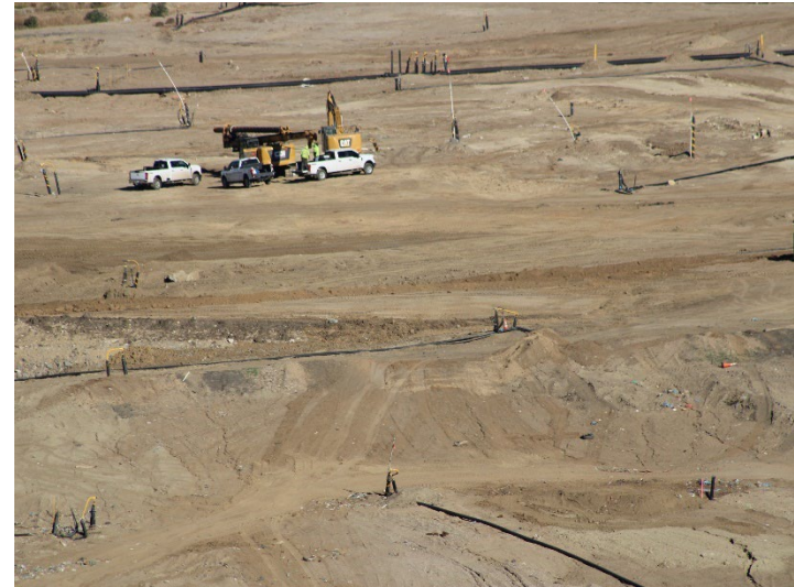
Photo 42: Working Area, CC-4 Part 3: November 6, 2025
