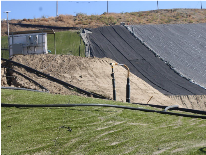
Photo 101: Working Area, CC-4 Part 4/5, CC-5A: October 8, 2025
