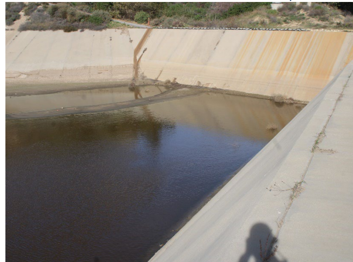
Photo 424: Terminal Basin: December 18, 2025
