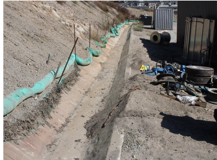
Photo 262: Flares 9, 10, 11 and Gas-to-Energy Facility: October 8, 2025
