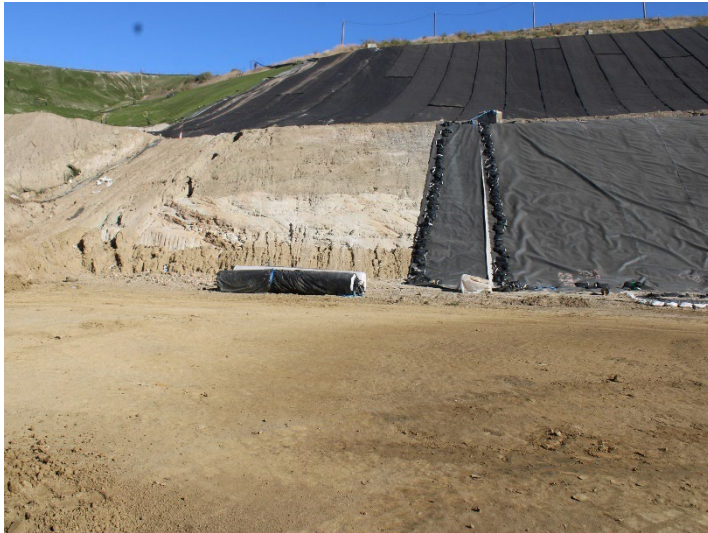
Photo 145: Working Area, CC-4 Part 4/5, CC-5A: November 6, 2025
