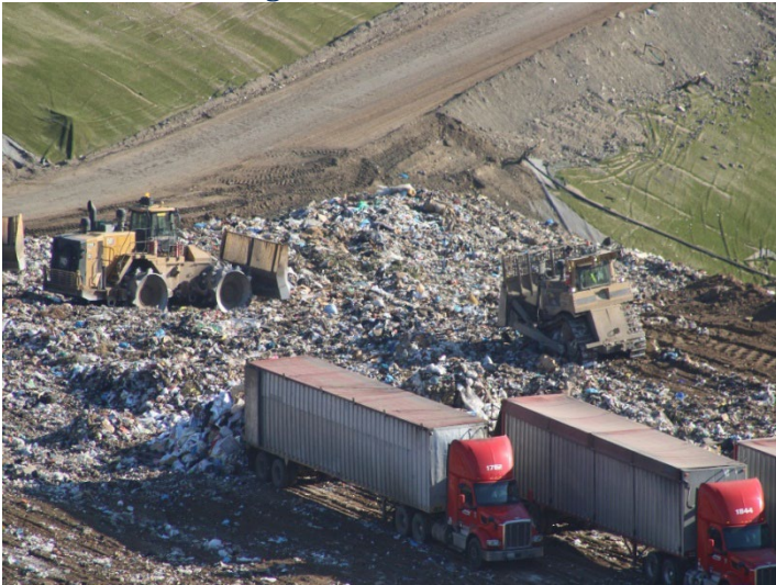
Photo 35: Working Area, CC-4 Part 3: October 8, 2025
