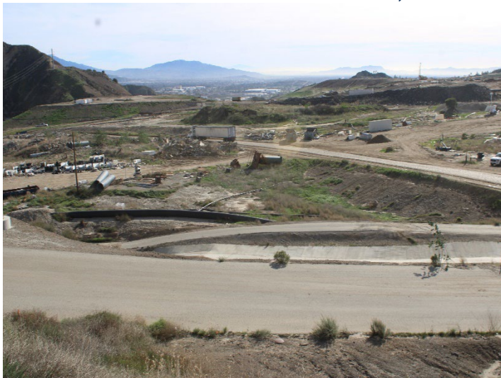
Photo 595: General Site: December 18, 2025
