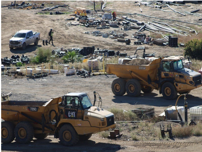
Photo 537: General Site: November 6, 2025
