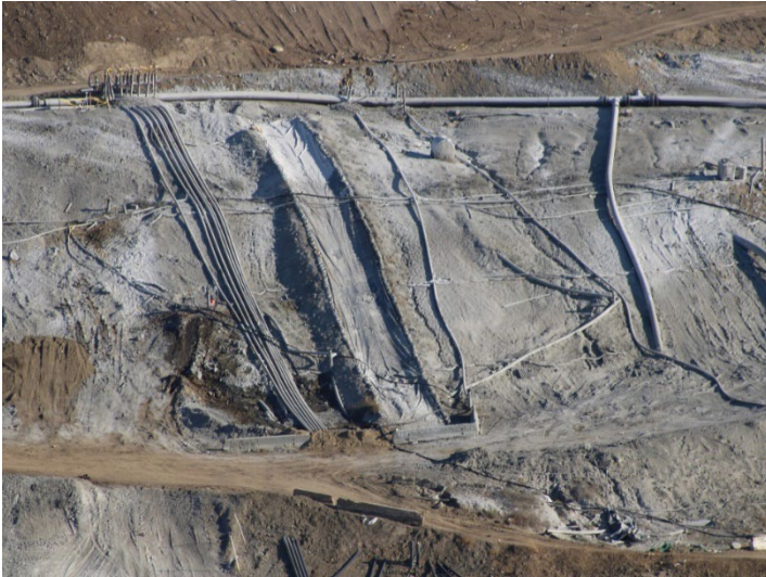
Photo 31: Working Area, CC-4 Part 3: October 8, 2025
