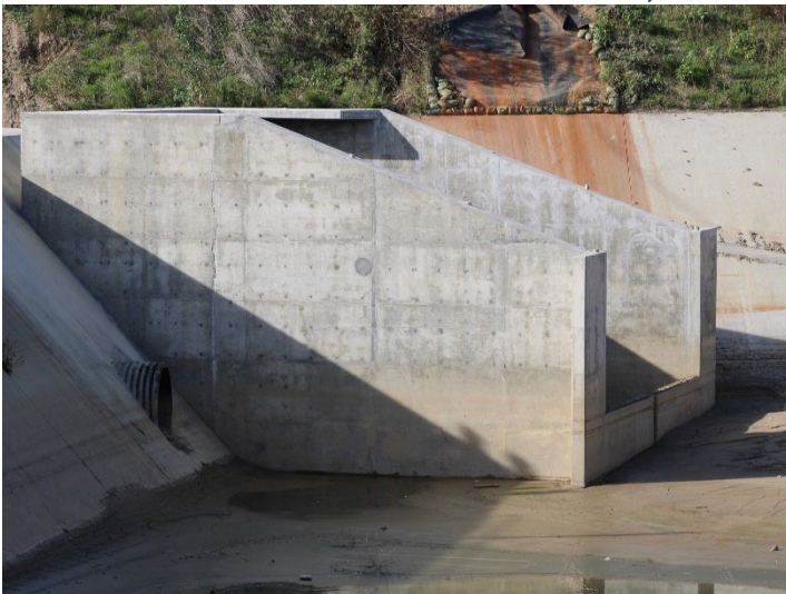
Photo 431: Terminal Basin: December 18, 2025
