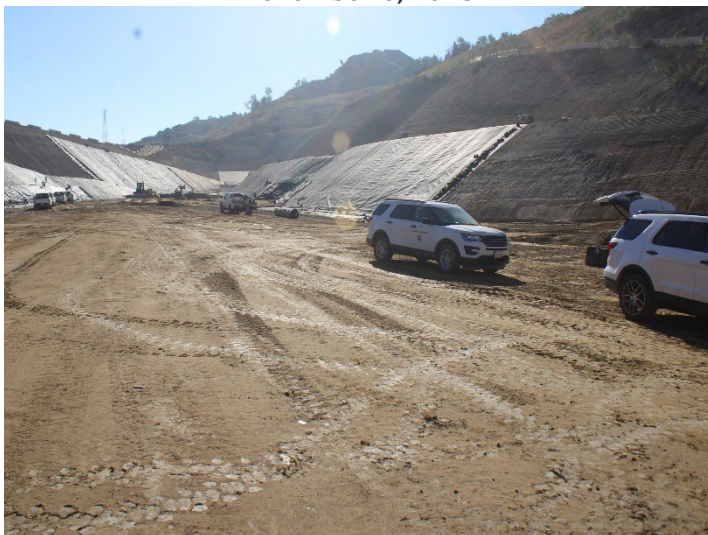
Photo 147: Working Area, CC-4 Part 4/5, CC-5A: November 6, 2025
