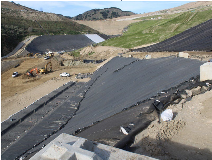
Photo 191: Working Area, CC-4 Part 4/5, CC-5A: December 18, 2025
