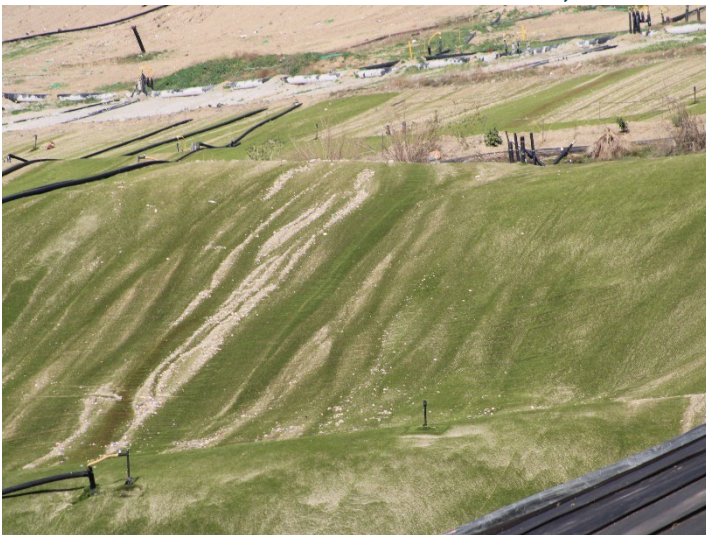
Photo 223: Closure Turf: December 18, 2025
