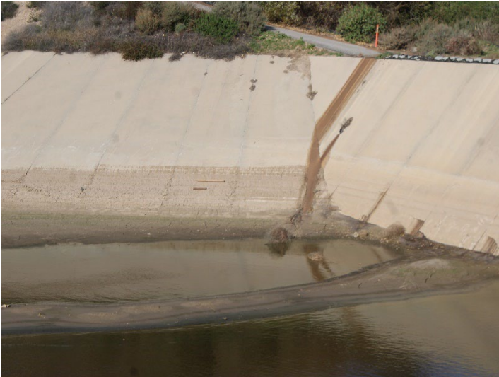
Photo 429: Terminal Basin: December 18, 2025
