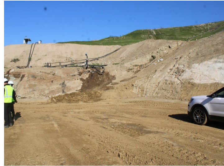
Photo 82: Working Area, CC-4 Part 4/5, CC-5A: October 8, 2025
