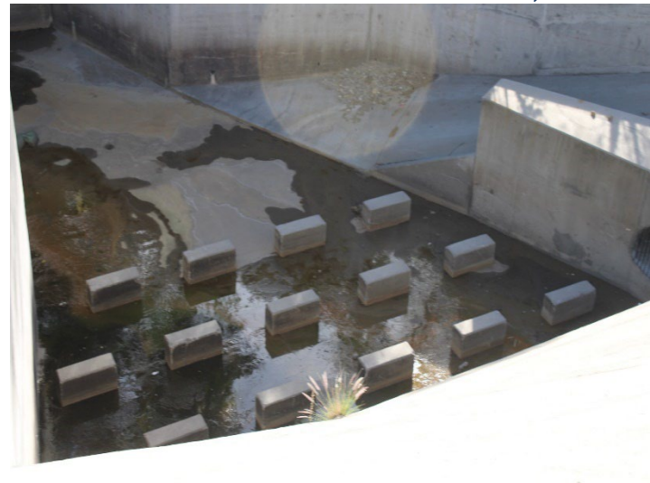
Photo 436: Terminal Basin: December 18, 2025
