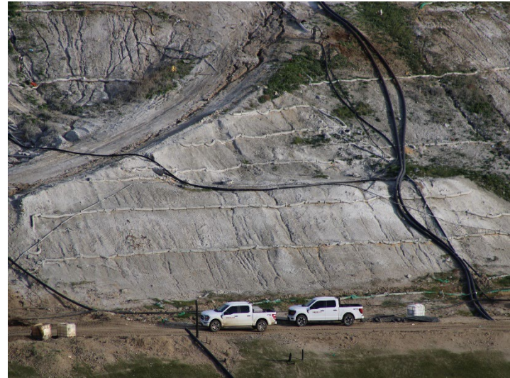
Photo 574: General Site: December 18, 2025
