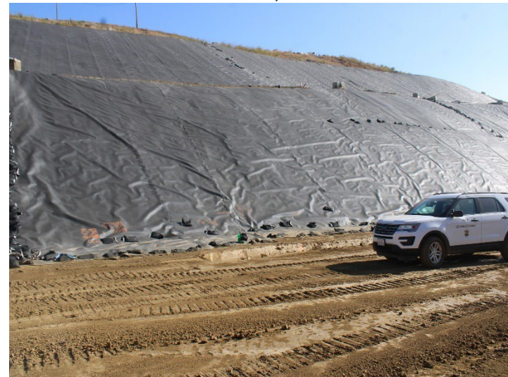
Photo 84: Working Area, CC-4 Part 4/5, CC-5A: October 8, 2025
