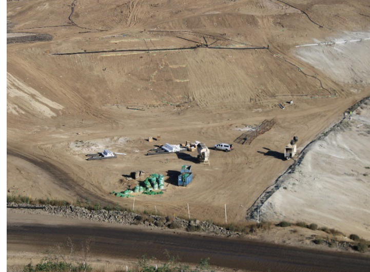
Photo 52: Working Area, CC-4 Part 4/5, CC-5A: October 8, 2025
