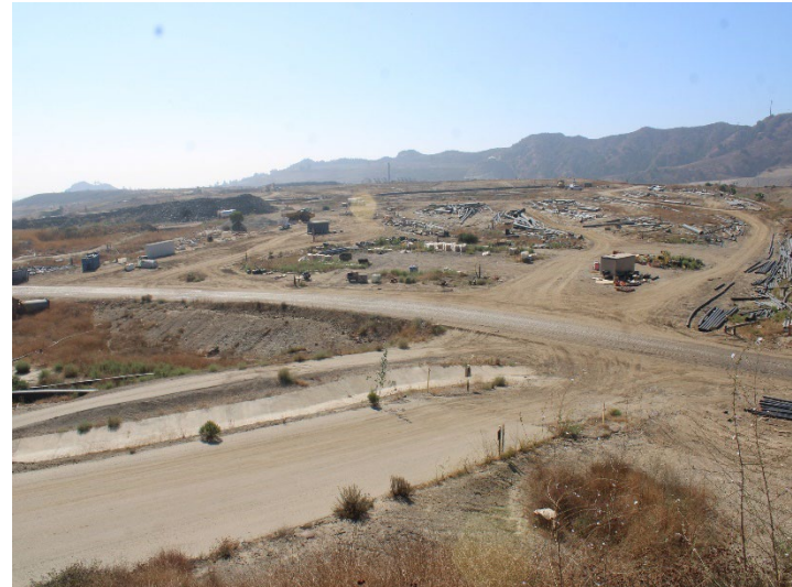
Photo 494: General Site: October 8, 2025
