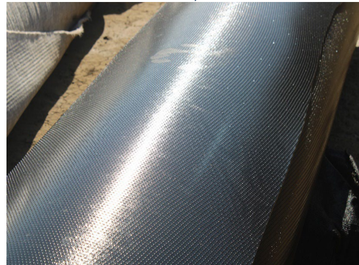
Photo 104: Working Area, CC-4 Part 4/5, CC-5A: October 8, 2025
