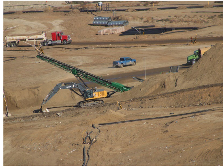
Photo 22: Working Area, CC4 Part 1/2: October 8, 2025
