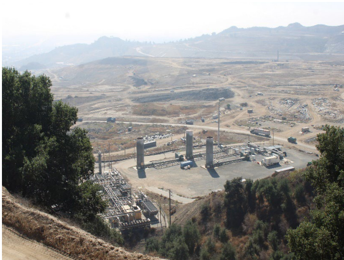
Photo 513: General Site: October 8, 2025
