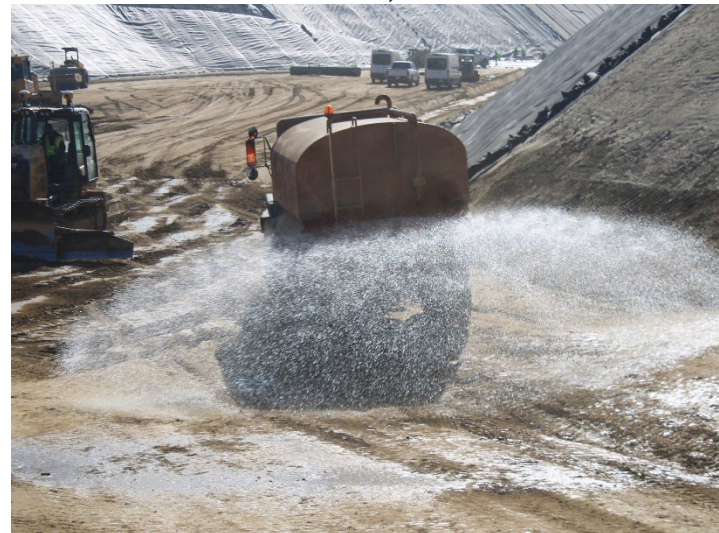
Photo 96: Working Area, CC-4 Part 4/5, CC-5A: October 8, 2025
