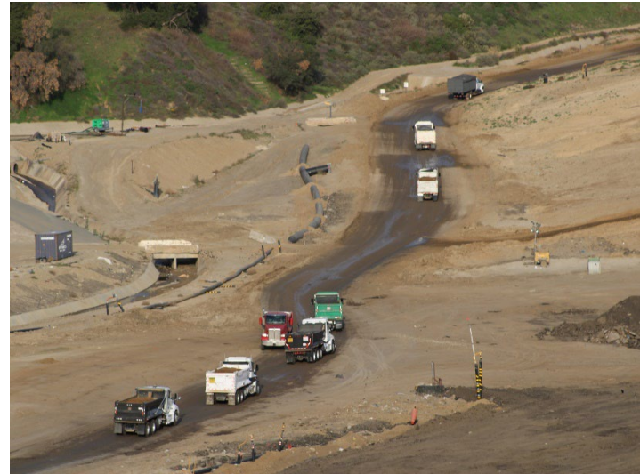
Photo 578: General Site: December 18, 2025
