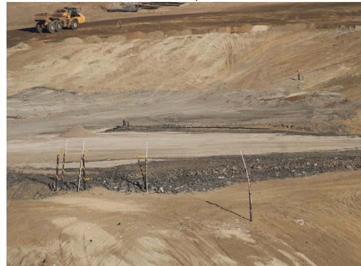
Photo 72: Working Area, CC-4 Part 4/5, CC-5A: October 8, 2025
