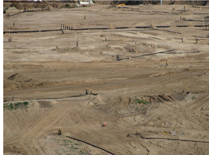
Photo 28: Working Area, CC4 Part 1/2: December 18, 2025
