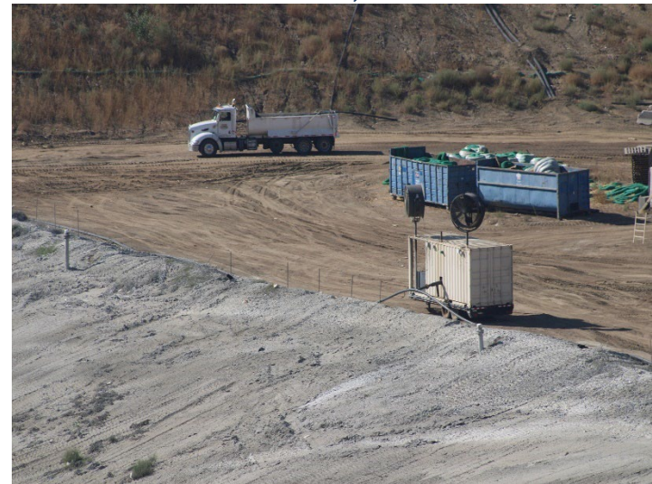
Photo 124: Working Area, CC-4 Part 4/5, CC-5A: October 8, 2025
