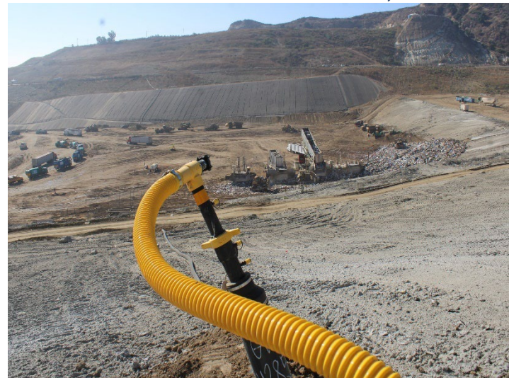
Photo 476: General Site: October 8, 2025
