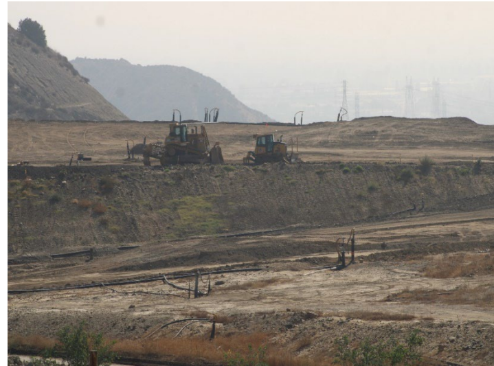
Photo 502: General Site: October 8, 2025
