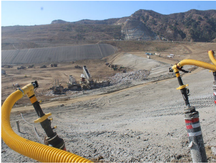
Photo 477: General Site: October 8, 2025
