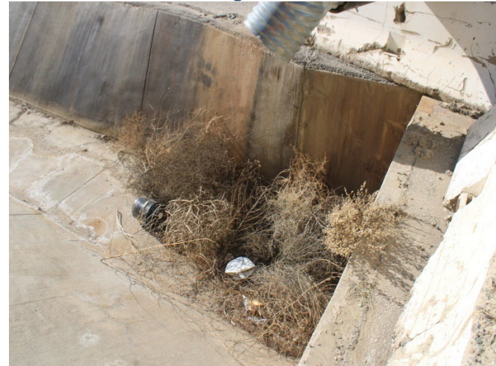
Photo 372: Eastside Drainage Channel: December 18, 2025
