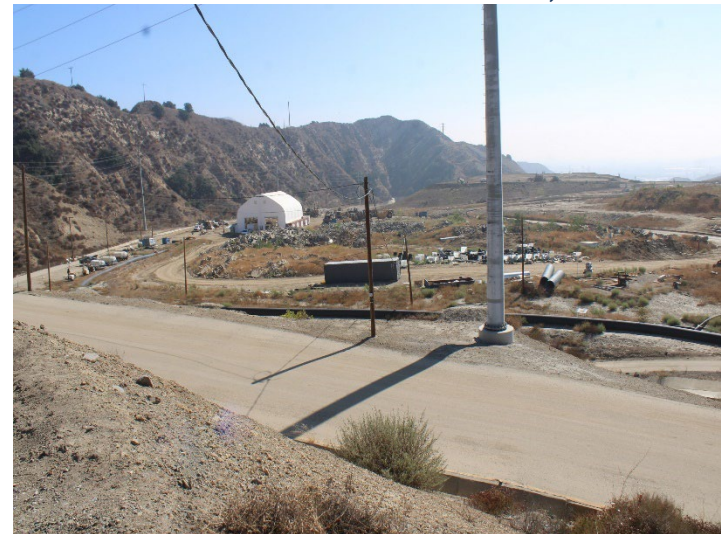
Photo 492: General Site: October 8, 2025
