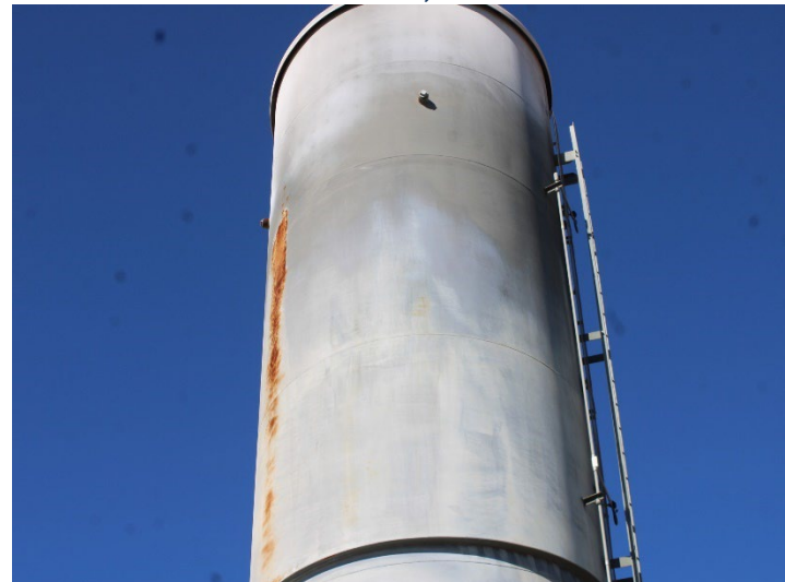
Photo 264: Flares 9, 10, 11 and Gas-to-Energy Facility: November 6, 2025
