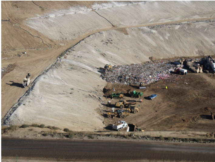
Photo 53: Working Area, CC-4 Part 4/5, CC-5A: October 8, 2025
