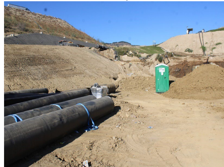
Photo 144: Working Area, CC-4 Part 4/5, CC-5A: November 6, 2025
