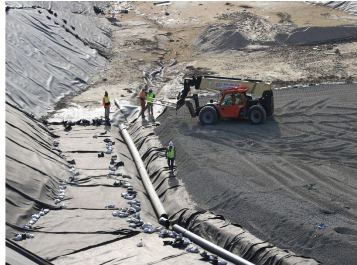
Photo 202: Working Area, CC-4 Part 4/5, CC-5A: December 18, 2025
