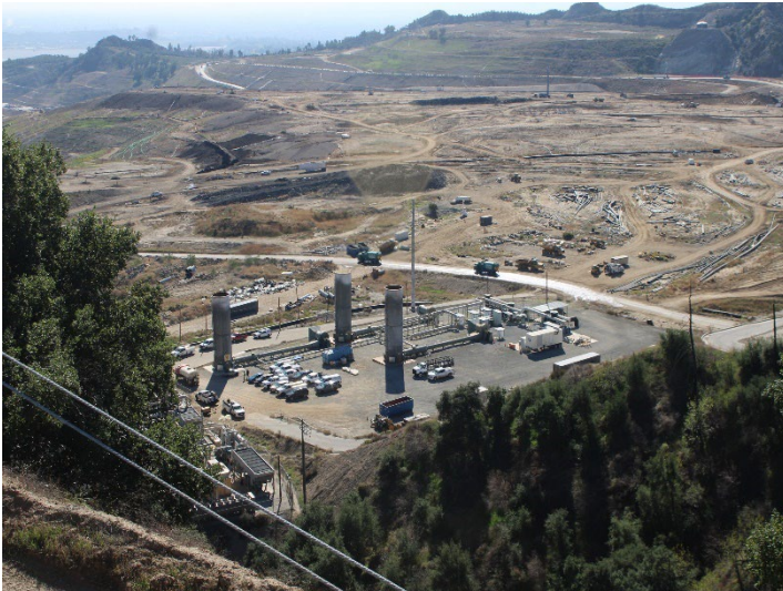
Photo 545: General Site: November 6, 2025
