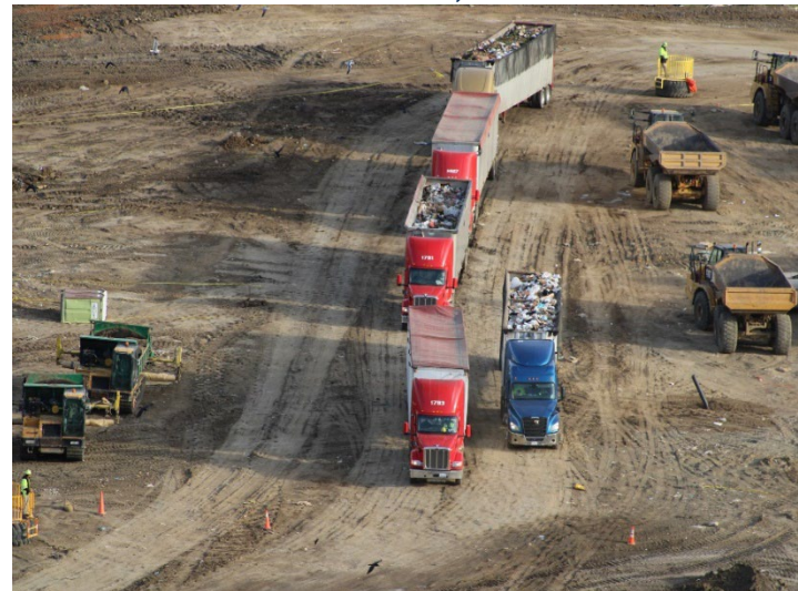
Photo 176: Working Area, CC-4 Part 4/5, CC-5A: December 18, 2025
