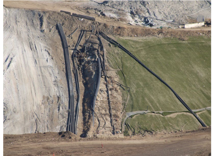
Photo 32: Working Area, CC-4 Part 3: October 8, 2025
