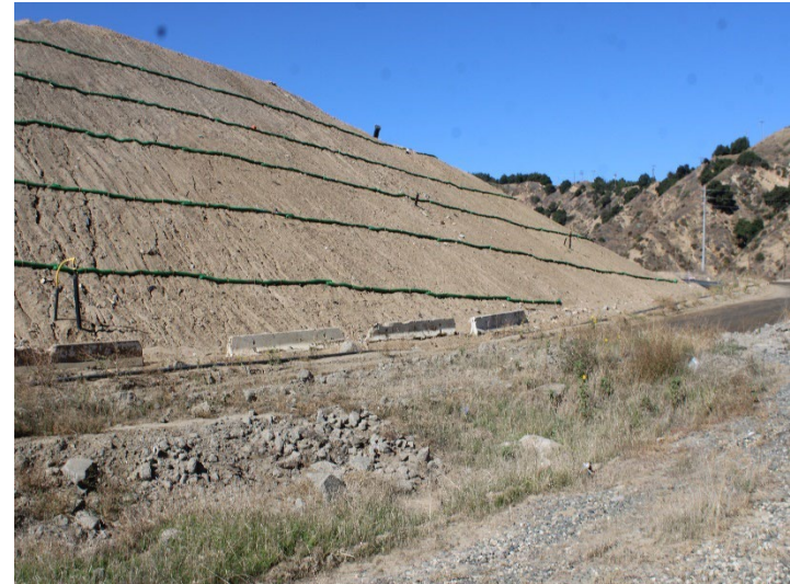
Photo 550: General Site: November 6, 2025
