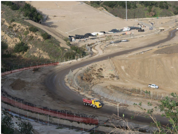
Photo 163: Working Area, CC-4 Part 4/5, CC-5A: December 18, 2025
