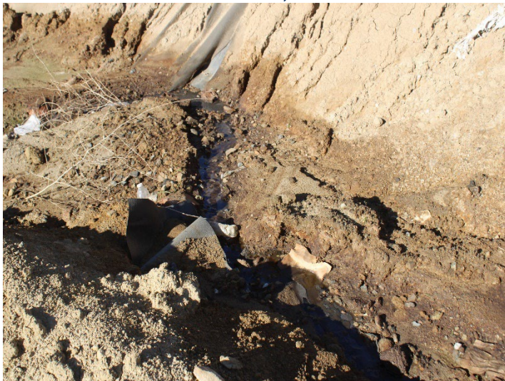
Photo 151: Working Area, CC-4 Part 4/5, CC-5A: November 6, 2025
