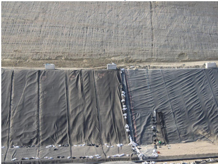
Photo 199: Working Area, CC-4 Part 4/5, CC-5A: December 18, 2025
