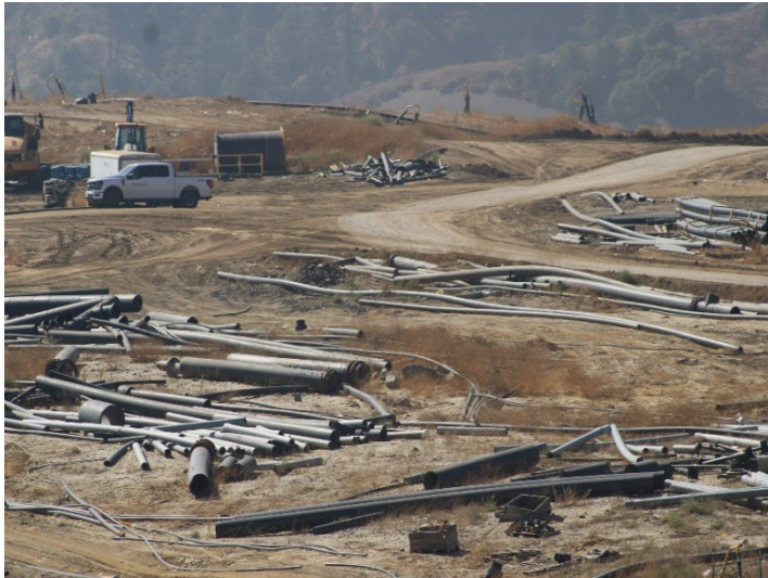
Photo 509: General Site: October 8, 2025
