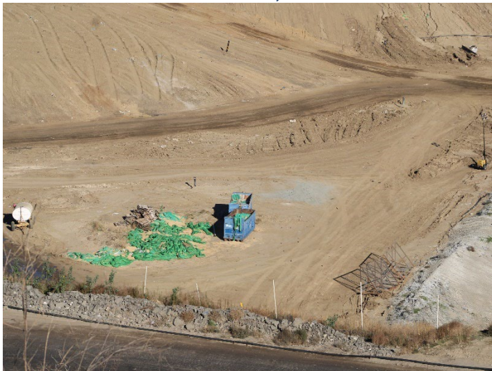
Photo 135: Working Area, CC-4 Part 4/5, CC-5A: November 6, 2025
