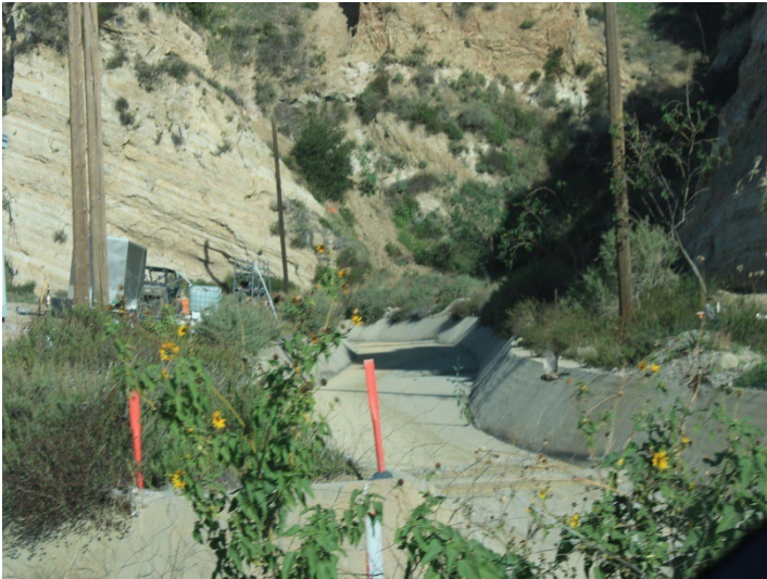
Photo 369: Eastside Drainage Channel: December 18, 2025
