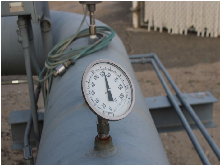
Photo 557: General Site: December 18, 2025
