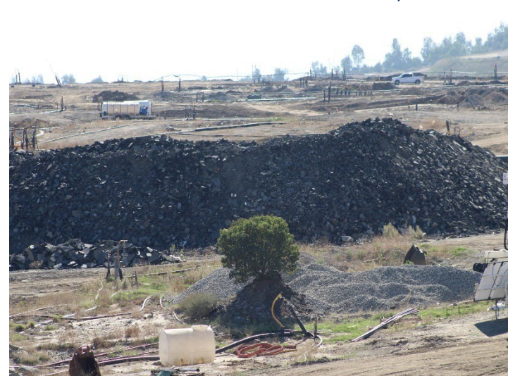
Photo 536: General Site: November 6, 2025
