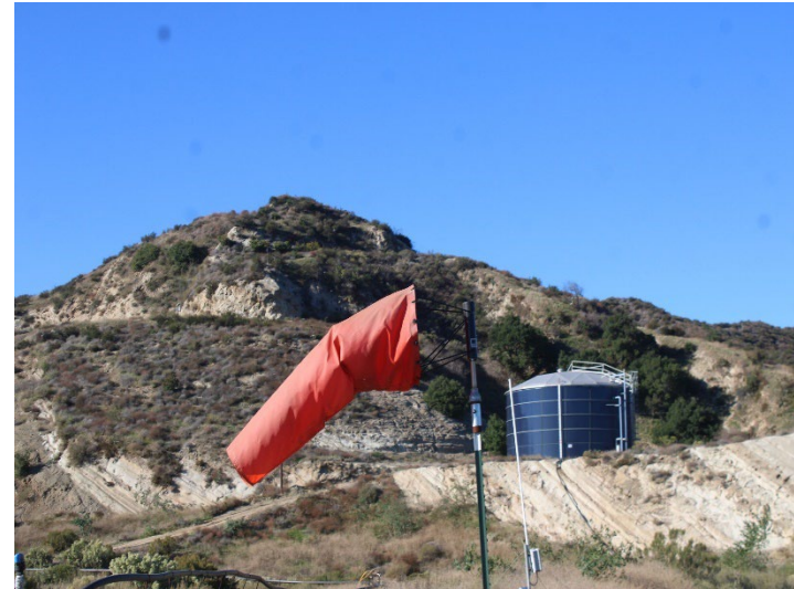
Photo 522: General Site: November 6, 2025
