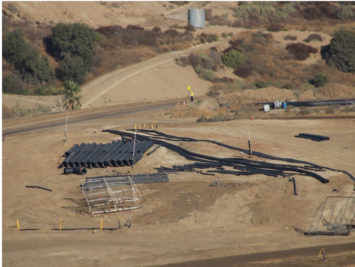
Photo 17: Working Area, CC4 Part 1/2: October 8, 2025
