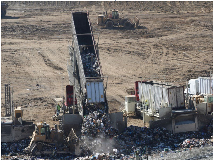
Photo 119: Working Area, CC-4 Part 4/5, CC-5A: October 8, 2025
