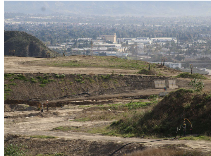
Photo 606: General Site: December 18, 2025
