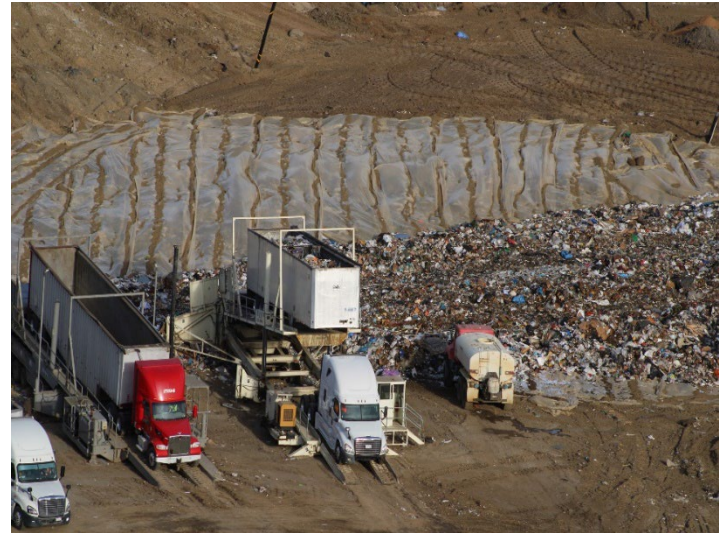
Photo 170: Working Area, CC-4 Part 4/5, CC-5A: December 18, 2025
