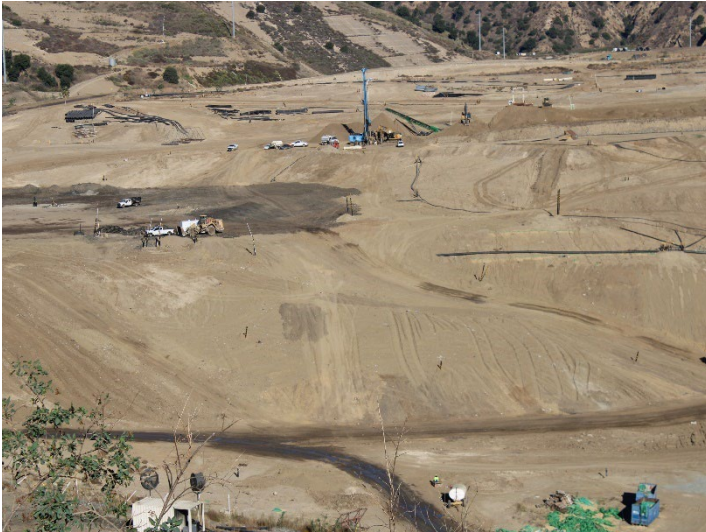
Photo 129: Working Area, CC-4 Part 4/5, CC-5A: November 6, 2025
