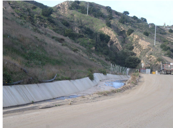
Photo 234: County Sage Mitigation Area and Westside Drainage Channels: December 18, 2025
