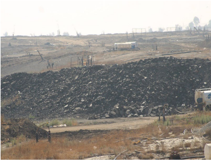
Photo 505: General Site: October 8, 2025
