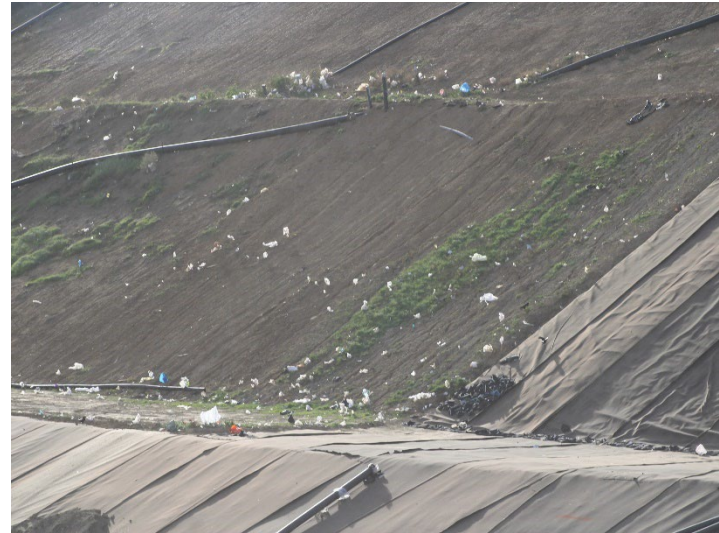
Photo 186: Working Area, CC-4 Part 4/5, CC-5A: December 18, 2025
