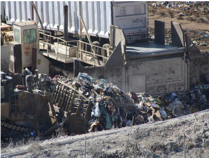
Photo 123: Working Area, CC-4 Part 4/5, CC-5A: October 8, 2025
