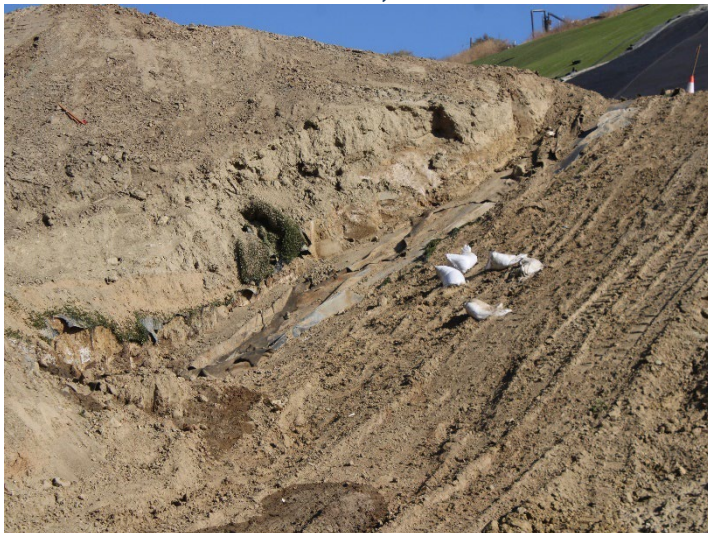
Photo 79: Working Area, CC-4 Part 4/5, CC-5A: October 8, 2025
