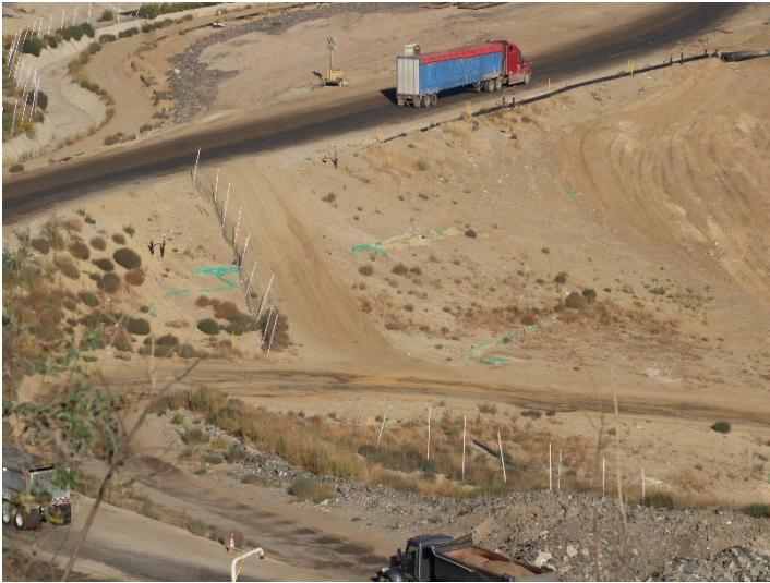
Photo 61: Working Area, CC-4 Part 4/5, CC-5A: October 8, 2025
