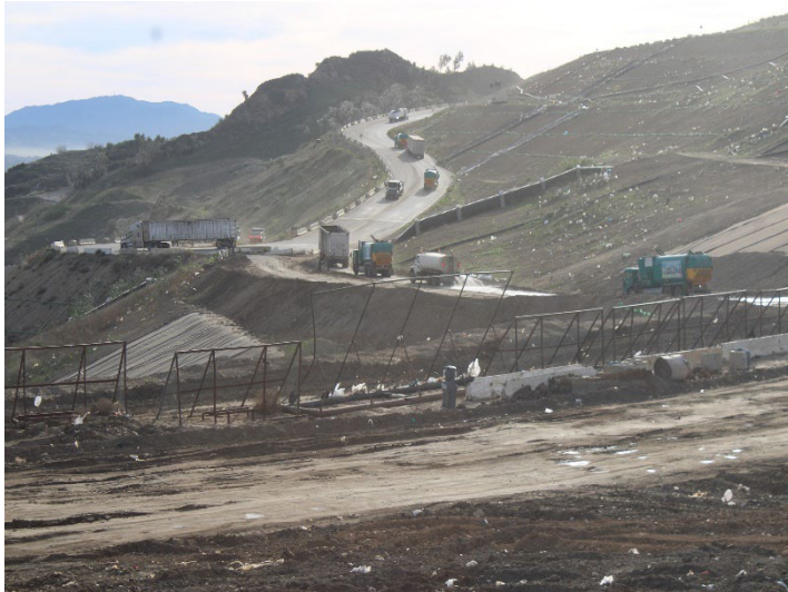
Photo 585: General Site: December 18, 2025
