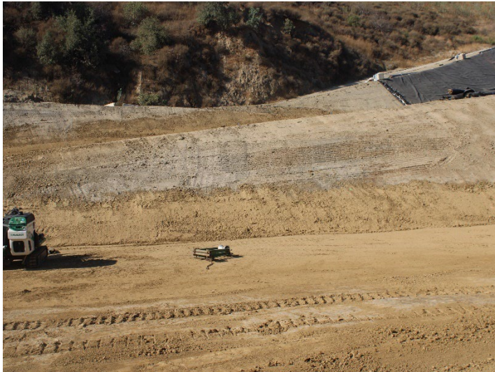
Photo 89: Working Area, CC-4 Part 4/5, CC-5A: October 8, 2025
