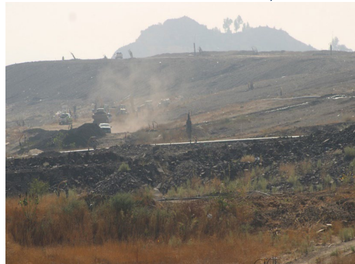
Photo 504: General Site: October 8, 2025
