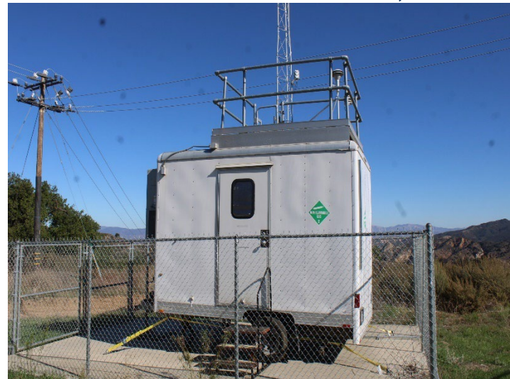
Photo 544: General Site: November 6, 2025
