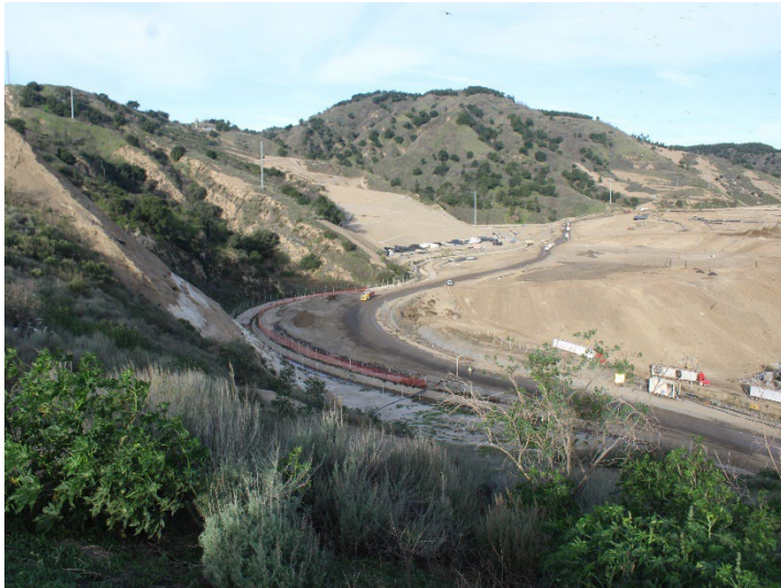
Photo 565: General Site: December 18, 2025
