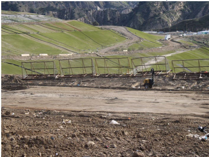
Photo 583: General Site: December 18, 2025
