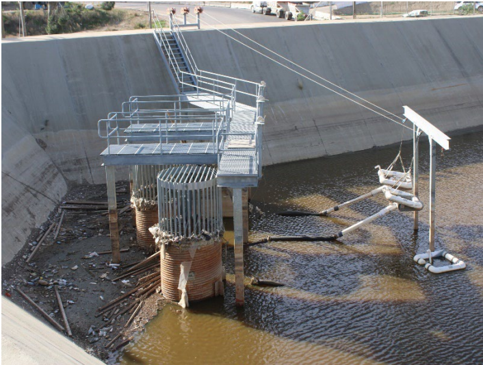
Photo 425: Terminal Basin: December 18, 2025
