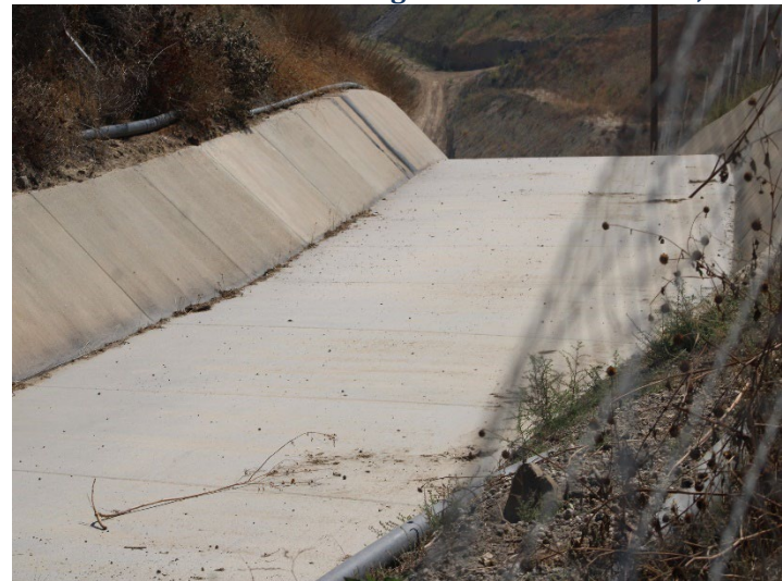
Photo 356: Eastside Drainage Channel: October 8, 2025
