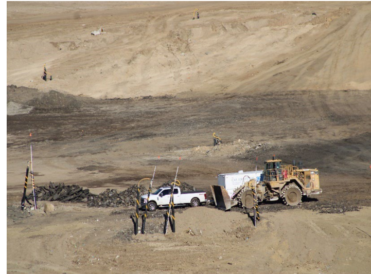
Photo 38: Working Area, CC-4 Part 3: November 6, 2025
