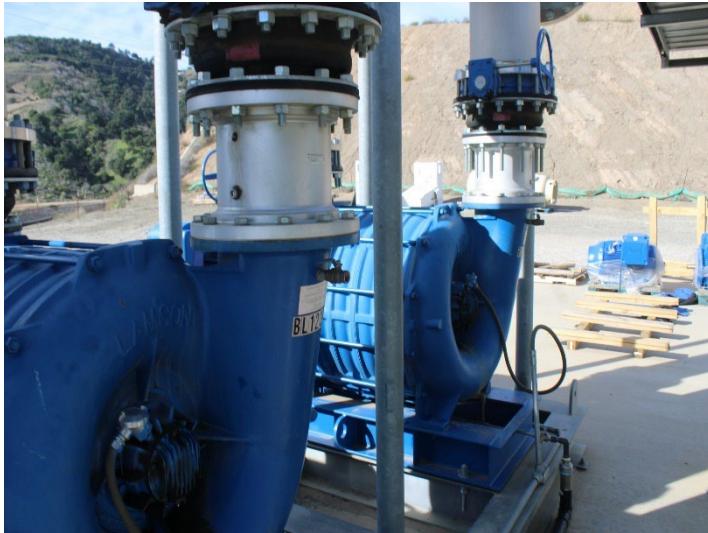
Photo 285: Flares 9, 10, 11 and Gas-to-Energy Facility: December 18, 2025
