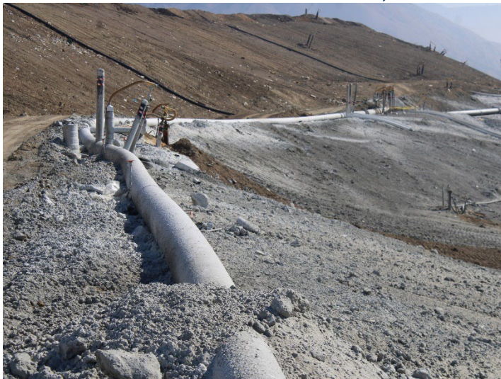
Photo 479: General Site: October 8, 2025
