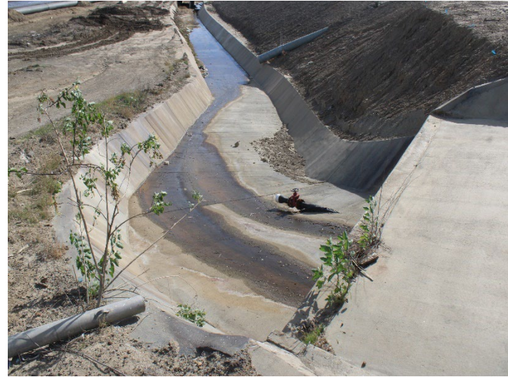
Photo 246: County Sage Mitigation Area and Westside Drainage Channels: December 18, 2025
