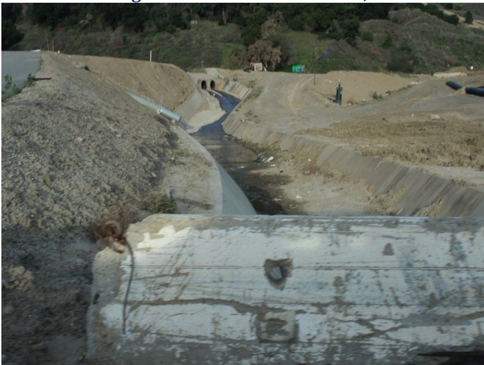
Photo 239: County Sage Mitigation Area and Westside Drainage Channels: December 18, 2025
