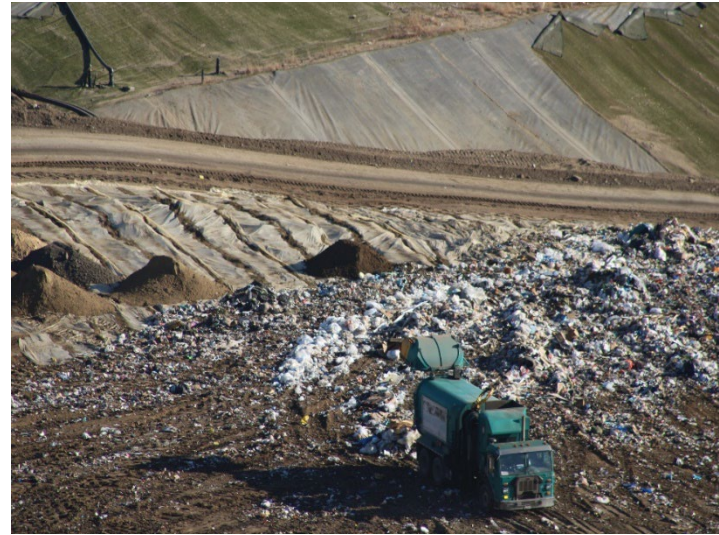
Photo 34: Working Area, CC-4 Part 3: October 8, 2025
