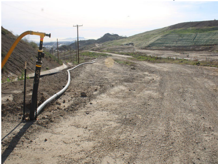
Photo 587: General Site: December 18, 2025
