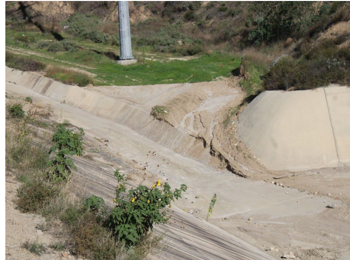
Photo 346: Basin B: December 18, 2025
