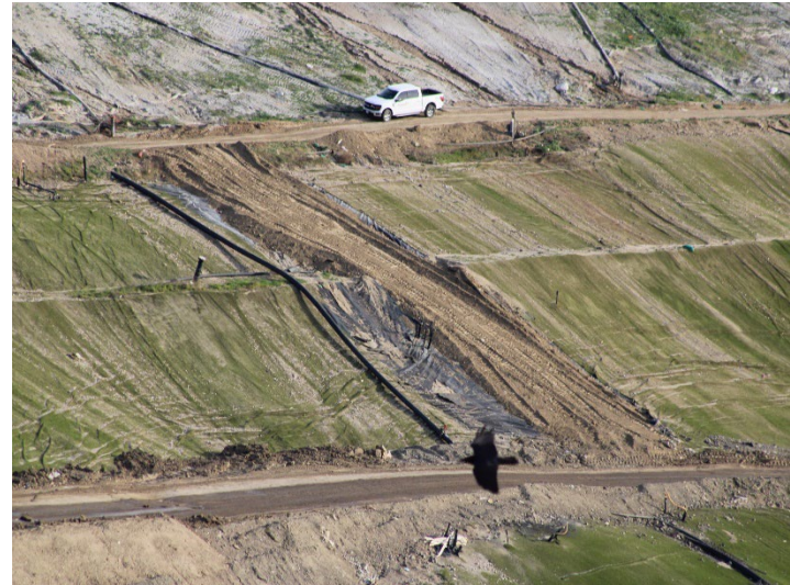
Photo 218: Closure Turf: December 18, 2025
