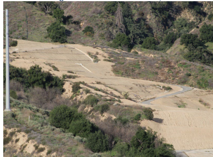
Photo 240: County Sage Mitigation Area and Westside Drainage Channels: December 18, 2025
