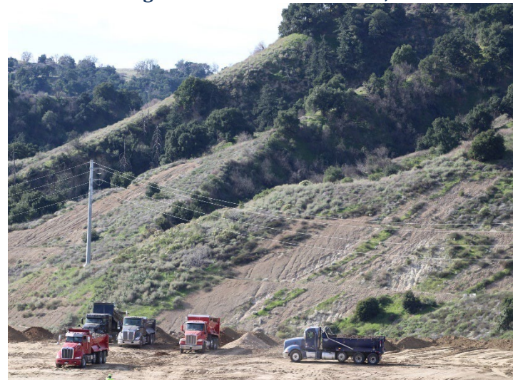
Photo 244: County Sage Mitigation Area and Westside Drainage Channels: December 18, 2025
