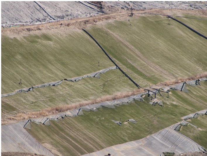
Photo 211: Closure Turf: October 8, 2025
