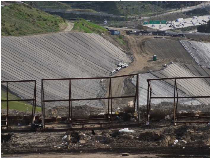
Photo 183: Working Area, CC-4 Part 4/5, CC-5A: December 18, 2025
