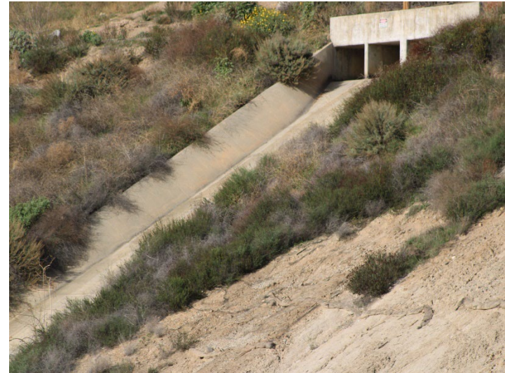
Photo 366: Eastside Drainage Channel: December 18, 2025
