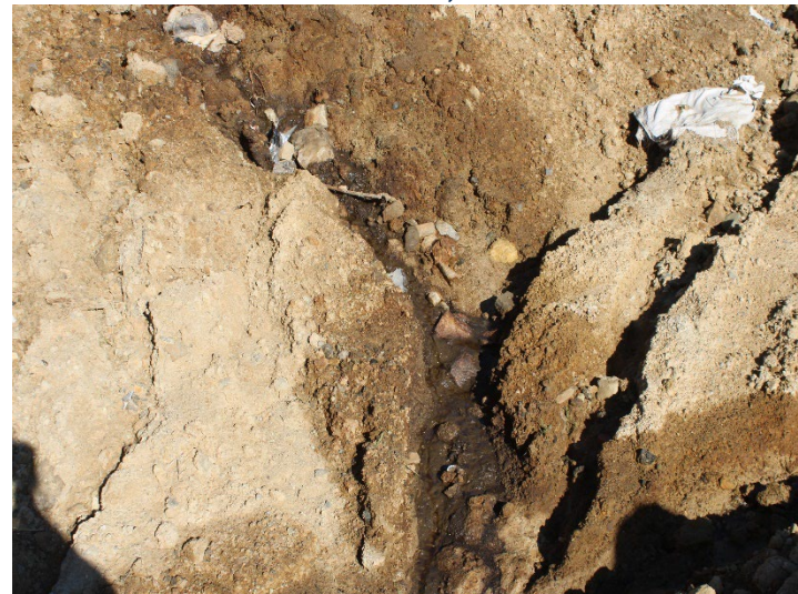
Photo 152: Working Area, CC-4 Part 4/5, CC-5A: November 6, 2025
