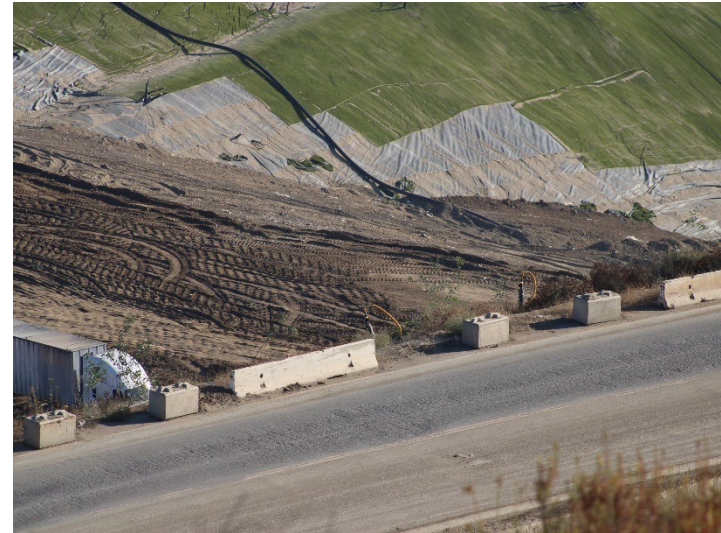
Photo 70: Working Area, CC-4 Part 4/5, CC-5A: October 8, 2025
