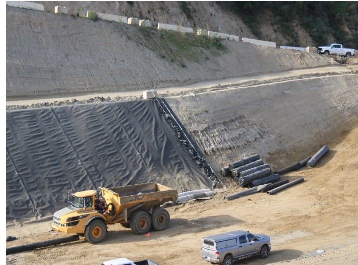
Photo 198: Working Area, CC-4 Part 4/5, CC-5A: December 18, 2025
