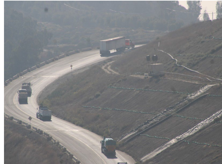
Photo 490: General Site: October 8, 2025
