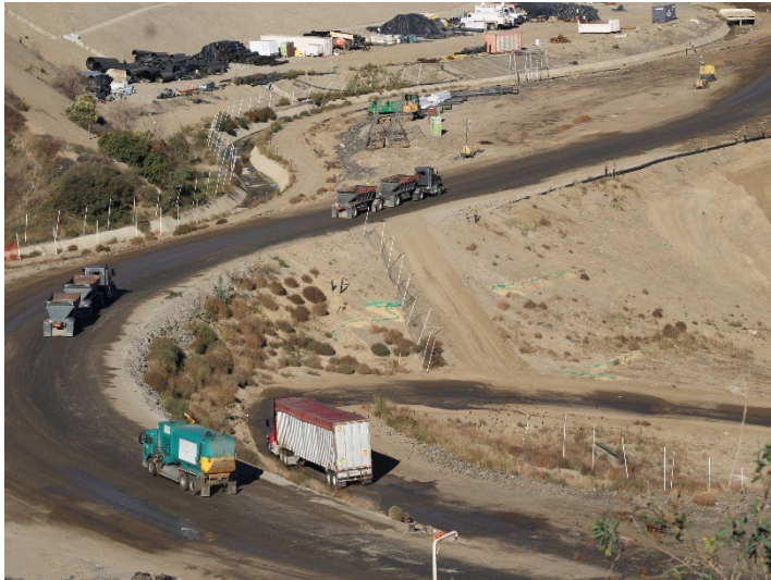
Photo 133: Working Area, CC-4 Part 4/5, CC-5A: November 6, 2025
