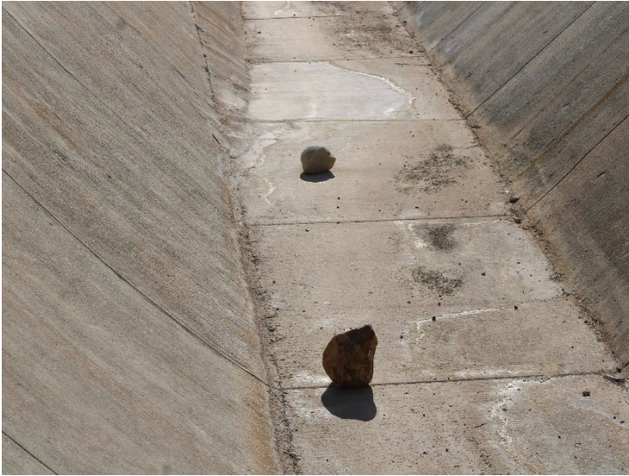
Photo 373: Eastside Drainage Channel: December 18, 2025
