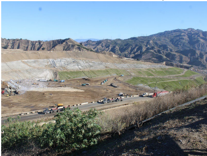
Photo 527: General Site: November 6, 2025
