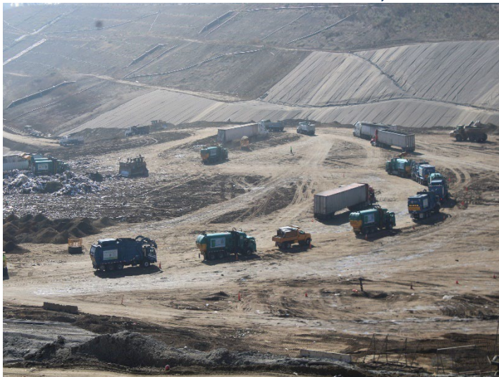
Photo 483: General Site: October 8, 2025
