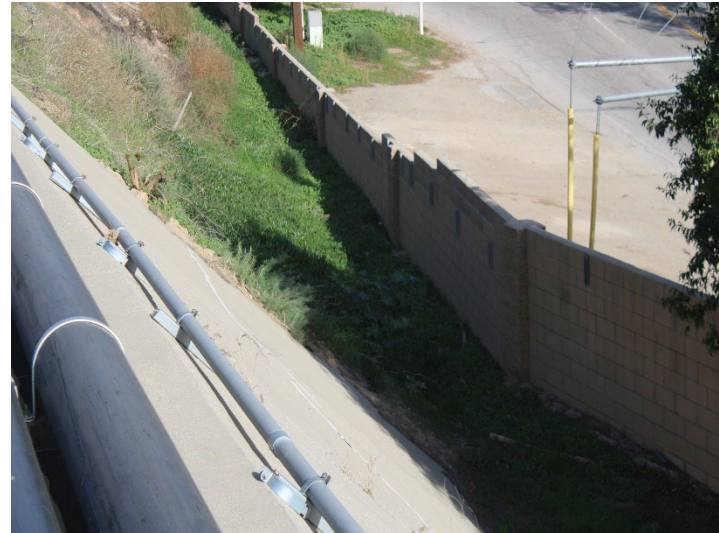
Photo 434: Terminal Basin: December 18, 2025
