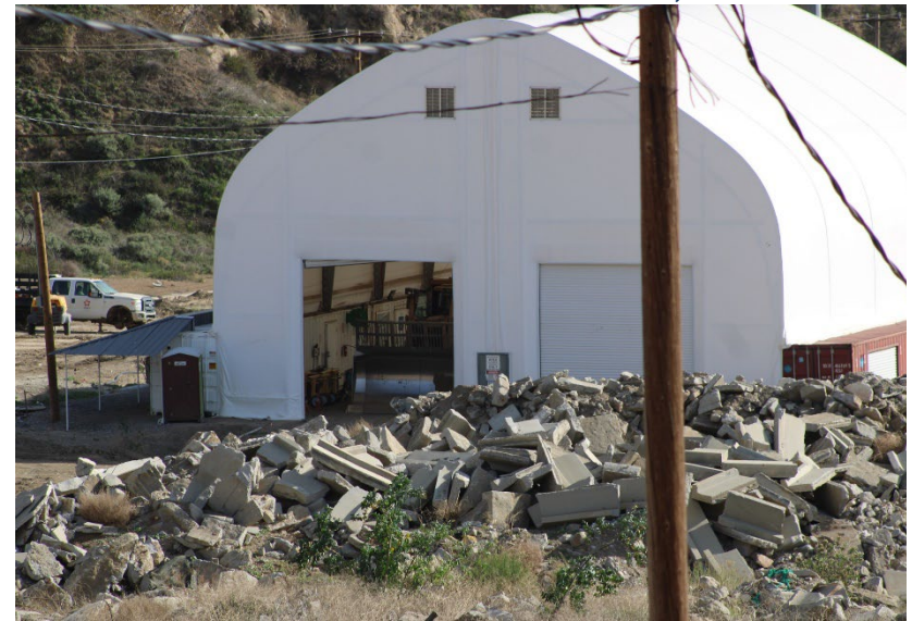
Photo 604: General Site: December 18, 2025
