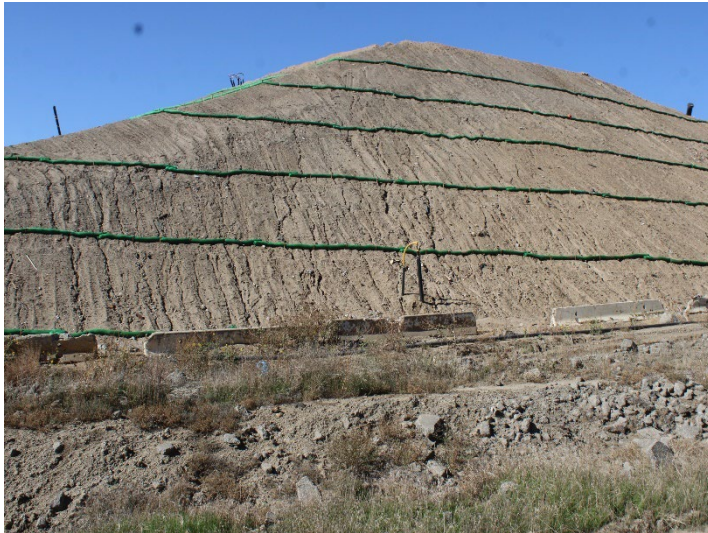
Photo 549: General Site: November 6, 2025
