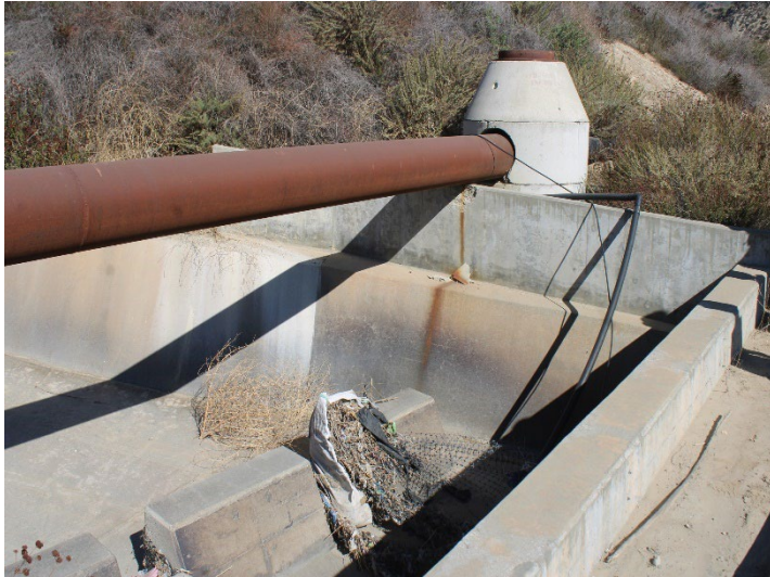
Photo 363: Eastside Drainage Channel: November 6, 2025
