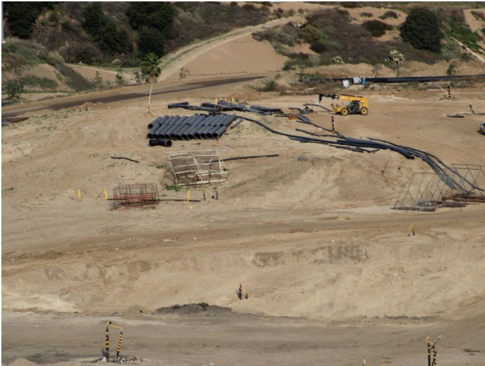
Photo 25: Working Area, CC4 Part 1/2: December 18, 2025
