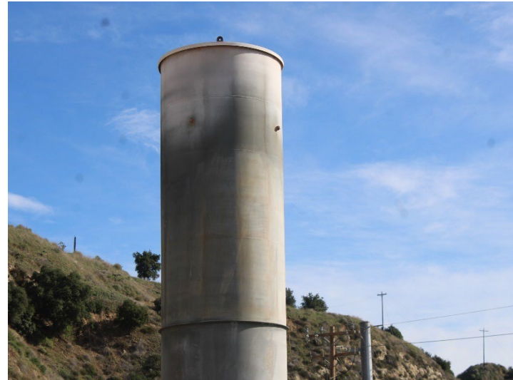
Photo 278: Flares 9, 10, 11 and Gas-to-Energy Facility: December 18, 2025
