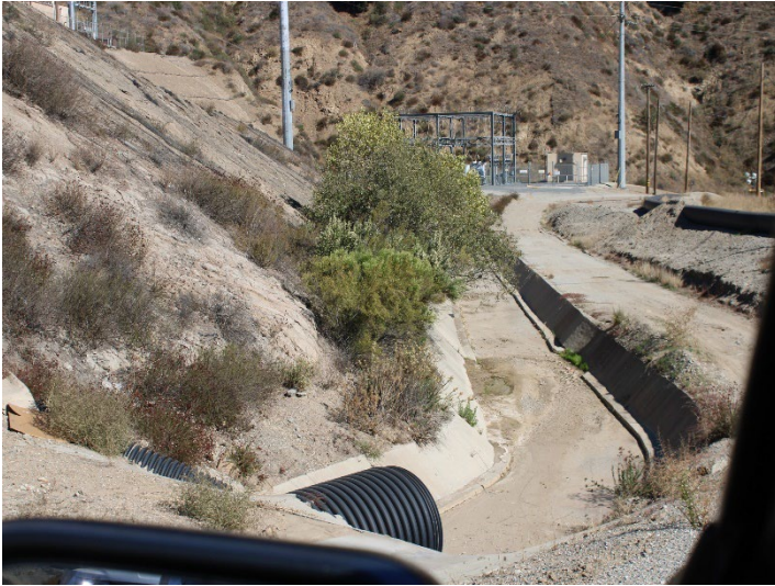
Photo 357: Eastside Drainage Channel: November 6, 2025
