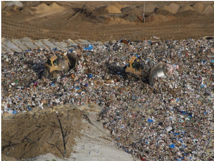
Photo 171: Working Area, CC-4 Part 4/5, CC-5A: December 18, 2025
