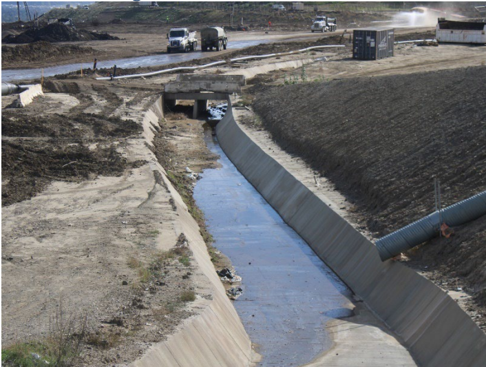
Photo 247: County Sage Mitigation Area and Westside Drainage Channels: December 18, 2025
