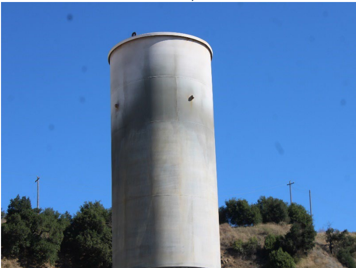
Photo 263: Flares 9, 10, 11 and Gas-to-Energy Facility: November 6, 2025
