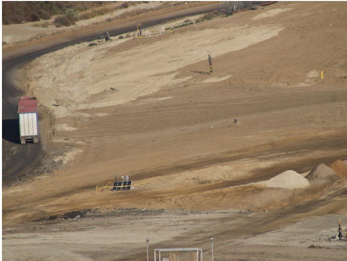
Photo 73: Working Area, CC-4 Part 4/5, CC-5A: October 8, 2025
