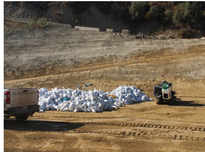
Photo 88: Working Area, CC-4 Part 4/5, CC-5A: October 8, 2025
