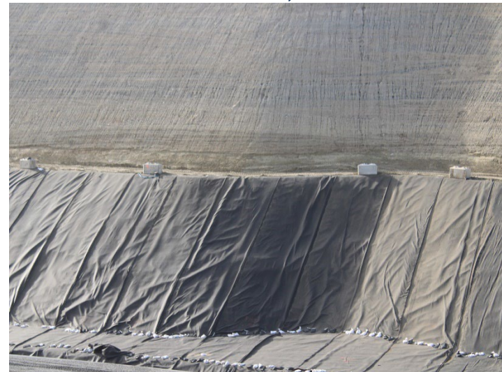
Photo 200: Working Area, CC-4 Part 4/5, CC-5A: December 18, 2025
