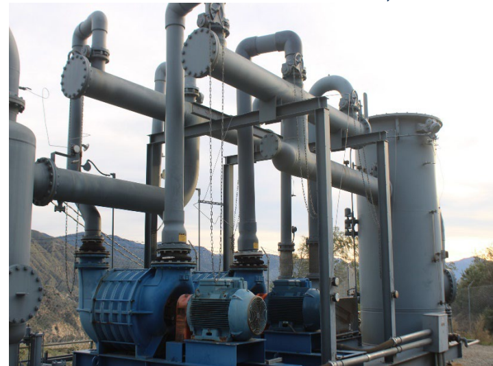
Photo 556: General Site: December 18, 2025
