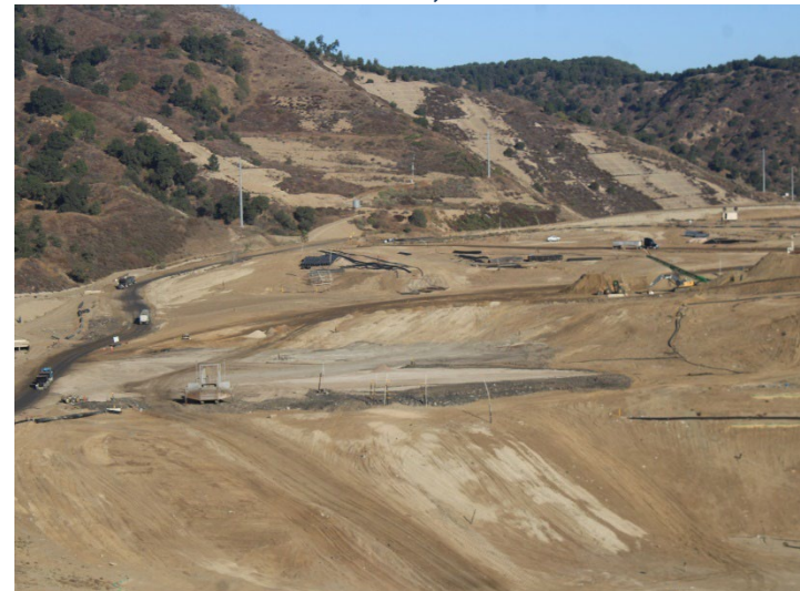
Photo 56: Working Area, CC-4 Part 4/5, CC-5A: October 8, 2025
