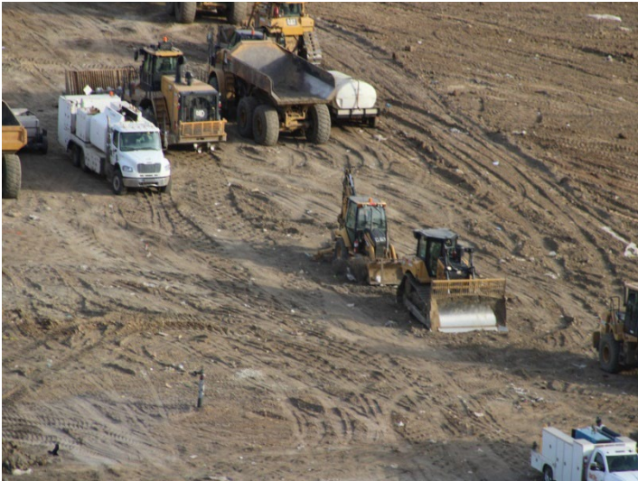
Photo 177: Working Area, CC-4 Part 4/5, CC-5A: December 18, 2025
