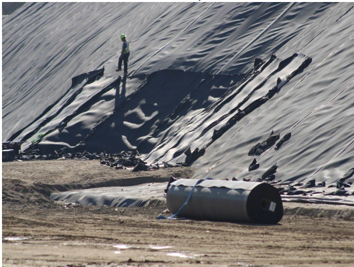
Photo 159: Working Area, CC-4 Part 4/5, CC-5A: November 6, 2025
