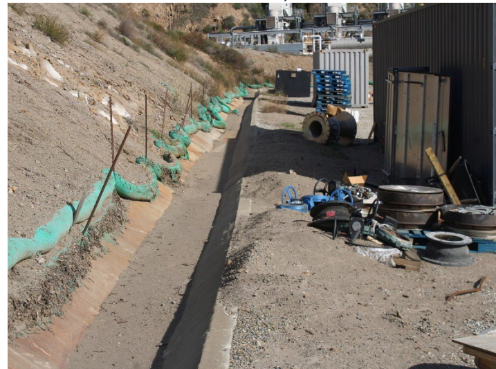
Photo 288: Flares 9, 10, 11 and Gas-to-Energy Facility: December 18, 2025
