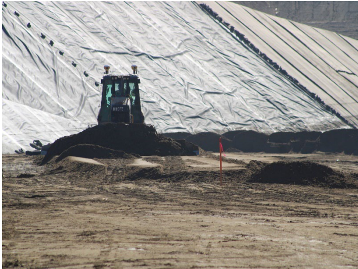
Photo 157: Working Area, CC-4 Part 4/5, CC-5A: November 6, 2025
