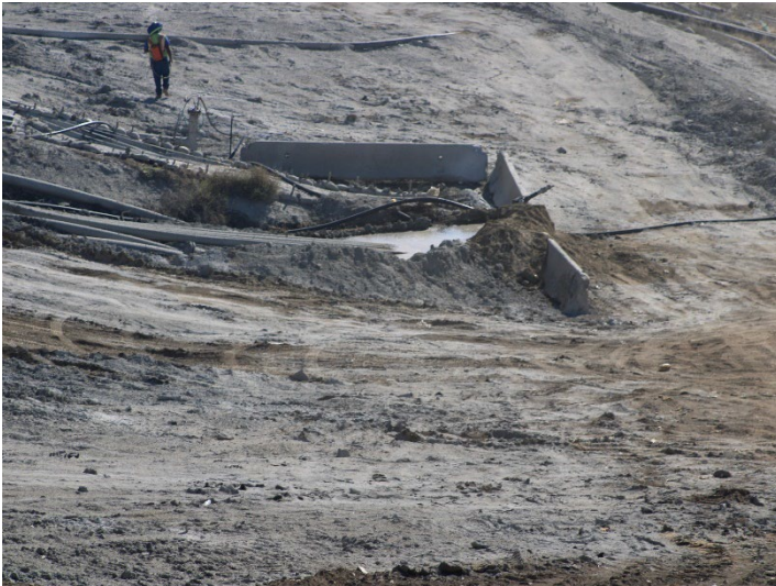
Photo 487: General Site: October 8, 2025
