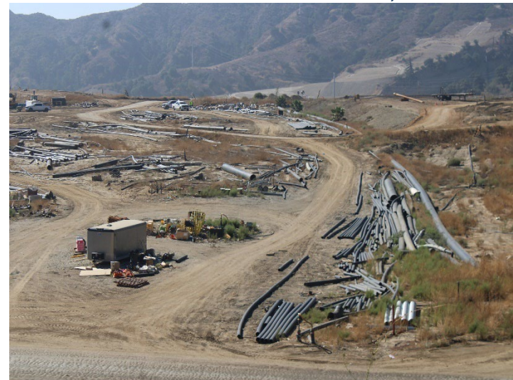
Photo 500: General Site: October 8, 2025
