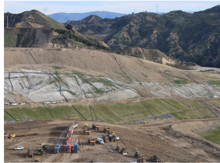
Photo 50: Working Area, CC-4 Part 3: December 18, 2025
