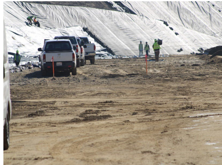
Photo 156: Working Area, CC-4 Part 4/5, CC-5A: November 6, 2025
