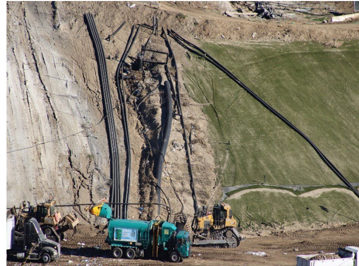
Photo 142: Working Area, CC-4 Part 4/5, CC-5A: November 6, 2025
