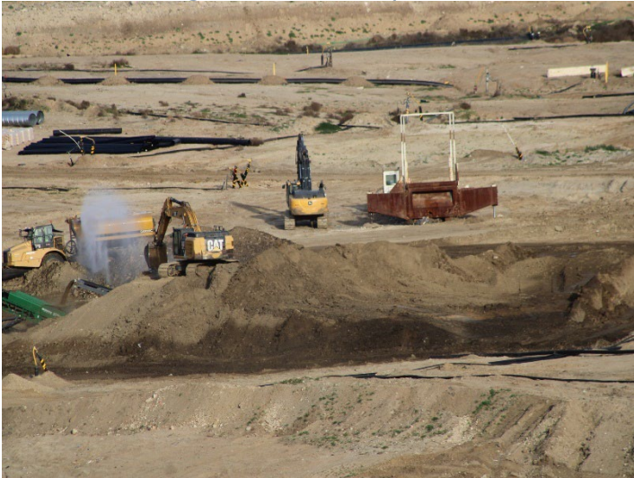
Photo 27: Working Area, CC4 Part 1/2: December 18, 2025
