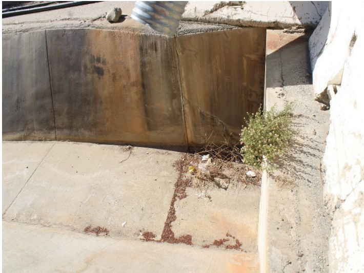
Photo 361: Eastside Drainage Channel: November 6, 2025
