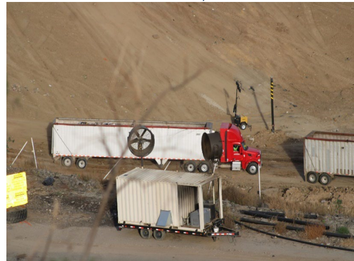
Photo 168: Working Area, CC-4 Part 4/5, CC-5A: December 18, 2025
