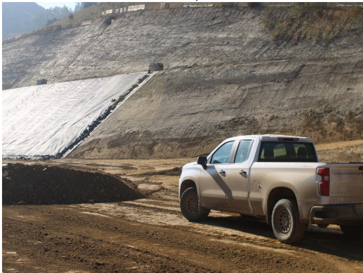
Photo 87: Working Area, CC-4 Part 4/5, CC-5A: October 8, 2025
