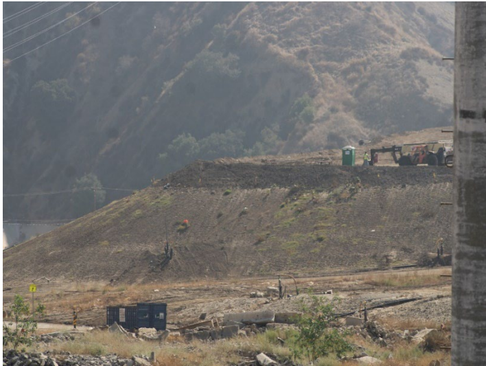
Photo 501: General Site: October 8, 2025
