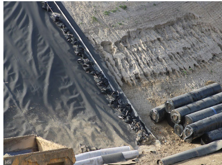
Photo 204: Working Area, CC-4 Part 4/5, CC-5A: December 18, 2025
