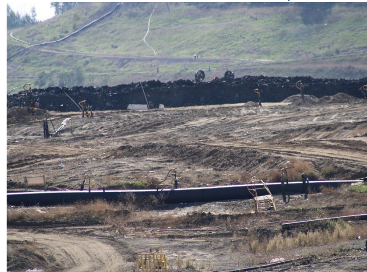
Photo 540: General Site: November 6, 2025
