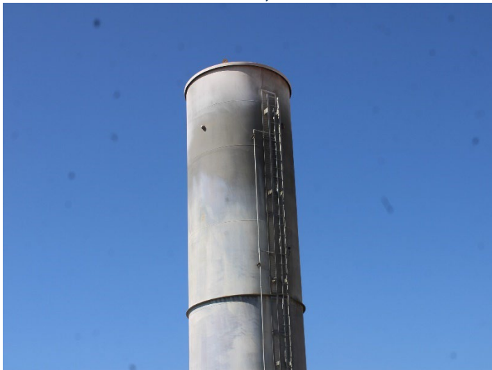
Photo 255: Flares 9, 10, 11 and Gas-to-Energy Facility: October 8, 2025
