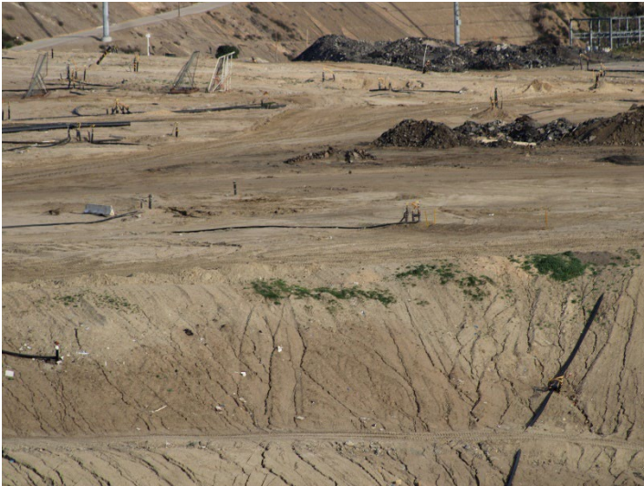
Photo 29: Working Area, CC4 Part 1/2: December 18, 2025
