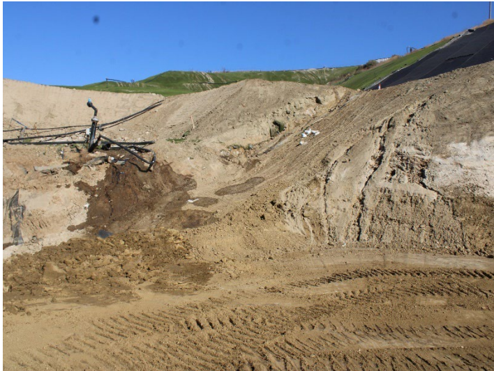
Photo 77: Working Area, CC-4 Part 4/5, CC-5A: October 8, 2025
