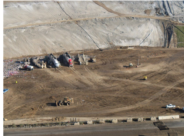
Photo 54: Working Area, CC-4 Part 4/5, CC-5A: October 8, 2025
