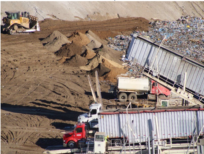
Photo 143 Working Area, CC-4 Part 4/5, CC-5A: November 6, 2025
