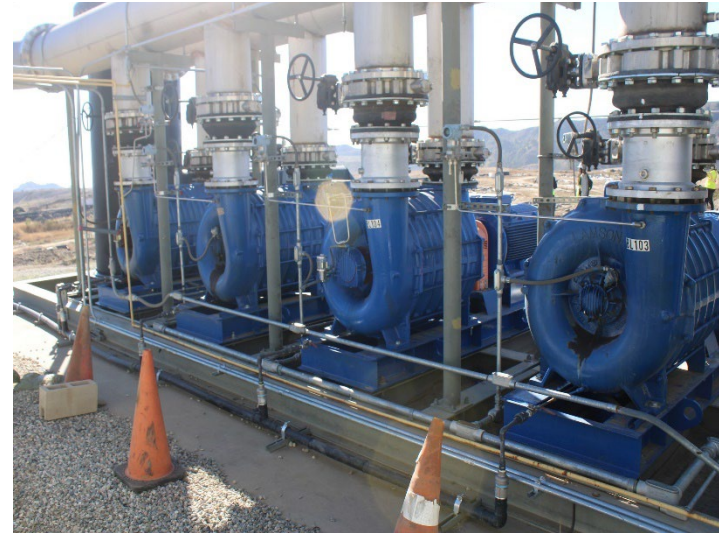
Photo 266: Flares 9, 10, 11 and Gas-to-Energy Facility: November 6, 2025
