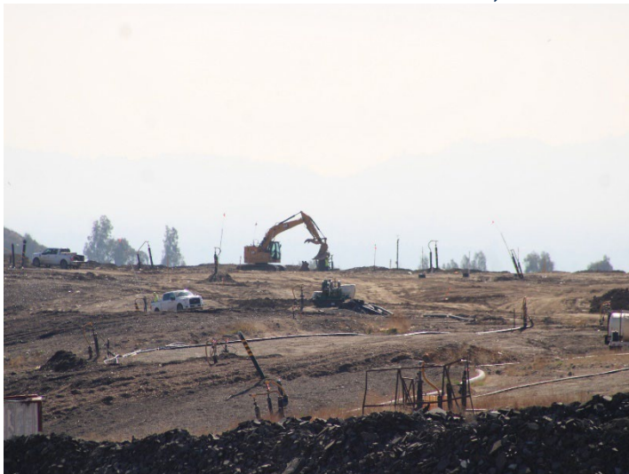
Photo 539: General Site: November 6, 2025
