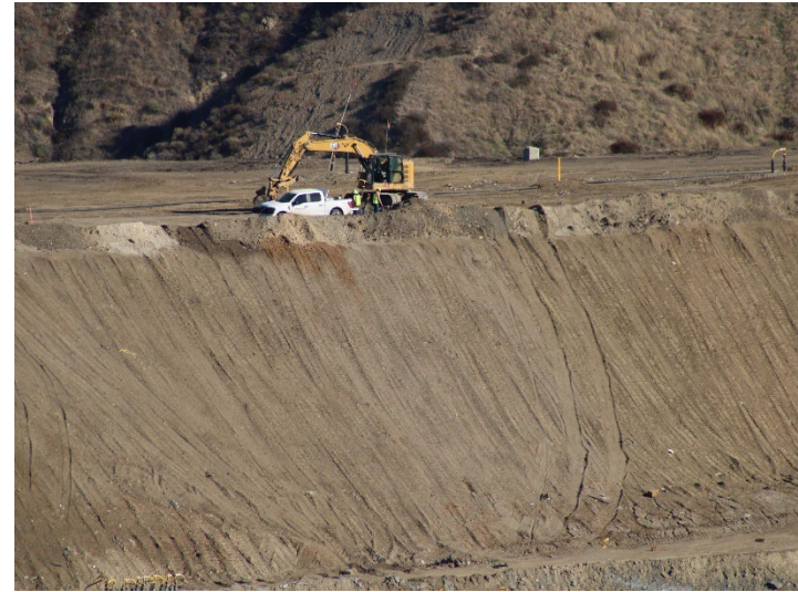
Photo 46: Working Area, CC-4 Part 3: November 6, 2025
