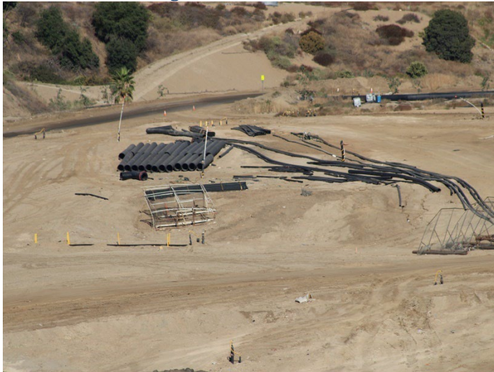
Photo 39: Working Area, CC-4 Part 3: November 6, 2025
