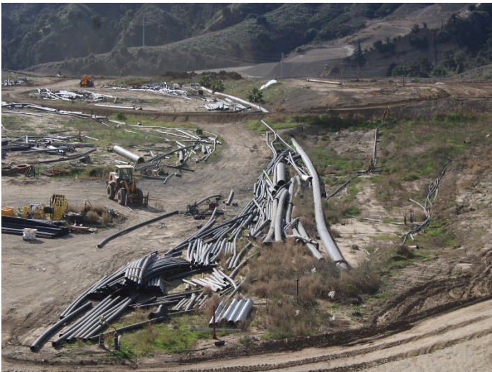
Photo 603: General Site: December 18, 2025
