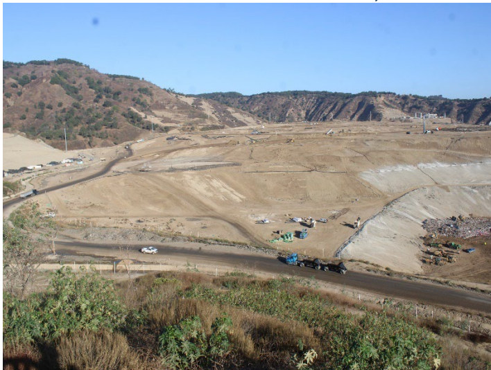
Photo 467: General Site: October 8, 2025
