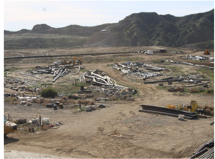
Photo 602: General Site: December 18, 2025
