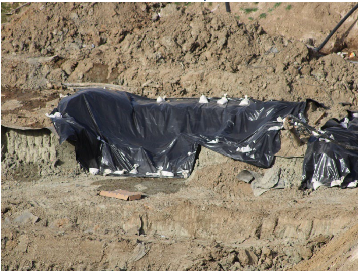
Photo 207: Working Area, CC-4 Part 4/5, CC-5A: December 18, 2025
