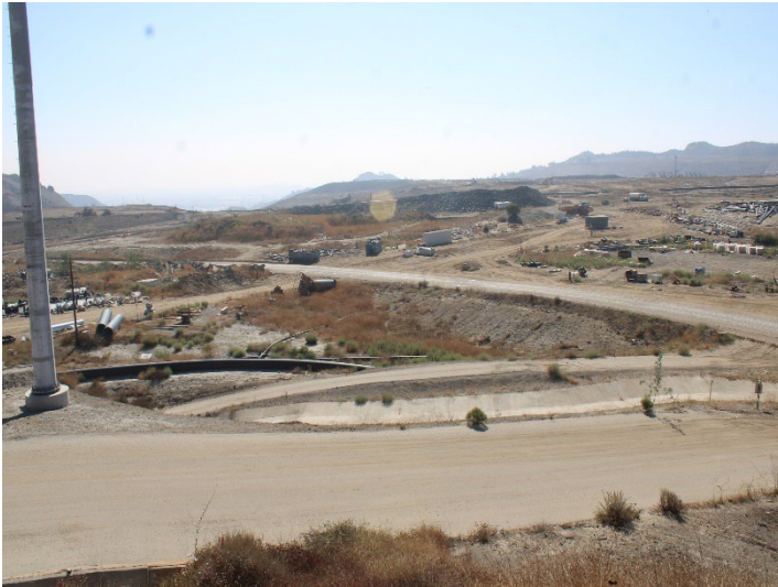
Photo 493: General Site: October 8, 2025
