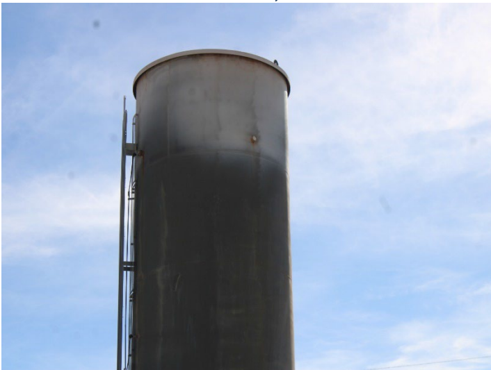
Photo 279: Flares 9, 10, 11 and Gas-to-Energy Facility: December 18, 2025
