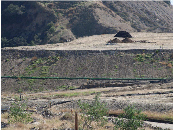
Photo 541: General Site: November 6, 2025
