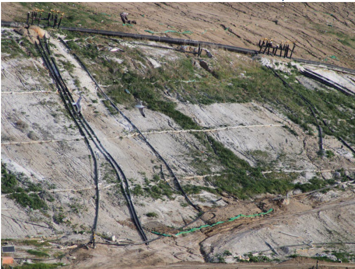
Photo 575: General Site: December 18, 2025
