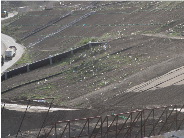
Photo 185: Working Area, CC-4 Part 4/5, CC-5A: December 18, 2025
