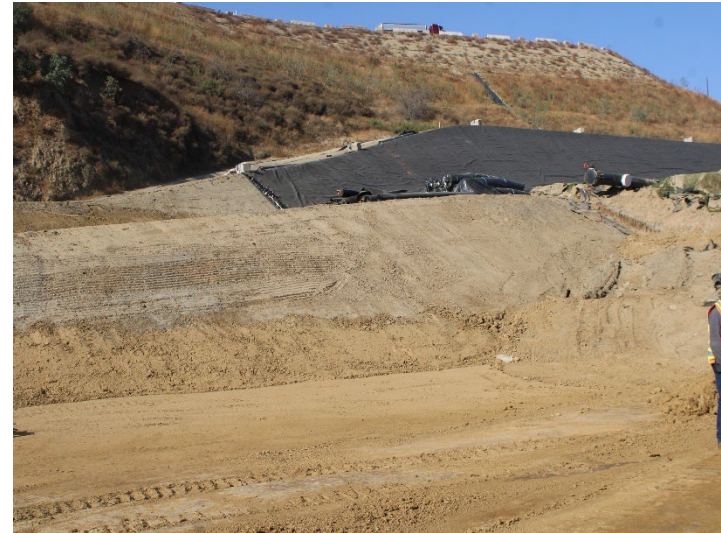
Photo 90: Working Area, CC-4 Part 4/5, CC-5A: October 8, 2025
