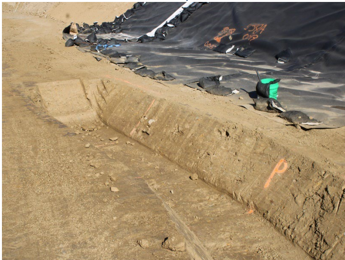
Photo 95: Working Area, CC-4 Part 4/5, CC-5A: October 8, 2025
