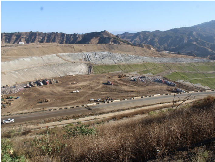
Photo 469: General Site: October 8, 2025
