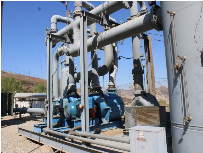
Photo 519: General Site: October 8, 2025
