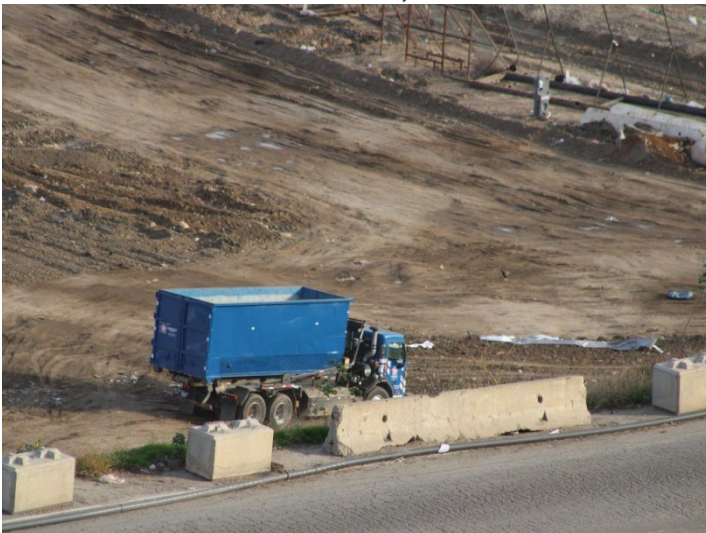
Photo 179: Working Area, CC-4 Part 4/5, CC-5A: December 18, 2025
