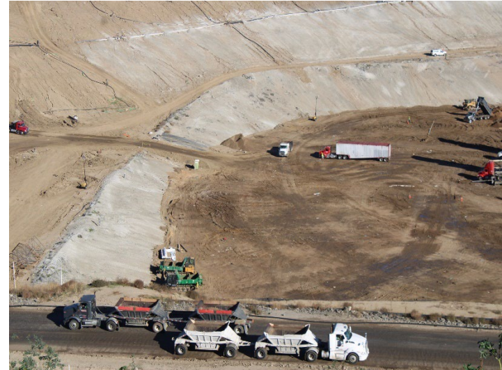
Photo 130: Working Area, CC-4 Part 4/5, CC-5A: November 6, 2025
