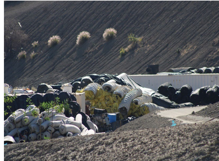
Photo 530: General Site: November 6, 2025
