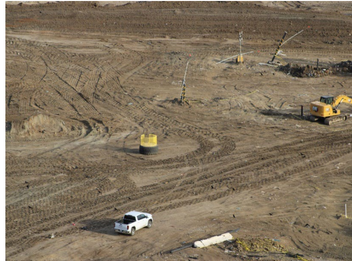
Photo 174: Working Area, CC-4 Part 4/5, CC-5A: December 18, 2025
