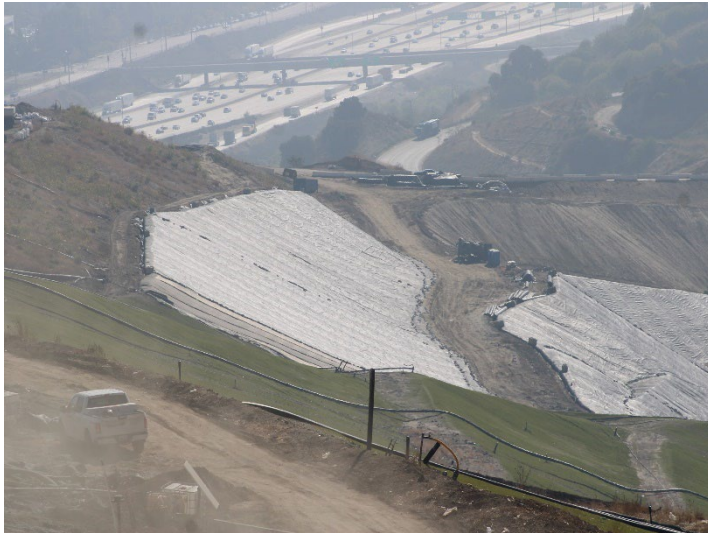
Photo 489: General Site: October 8, 2025
