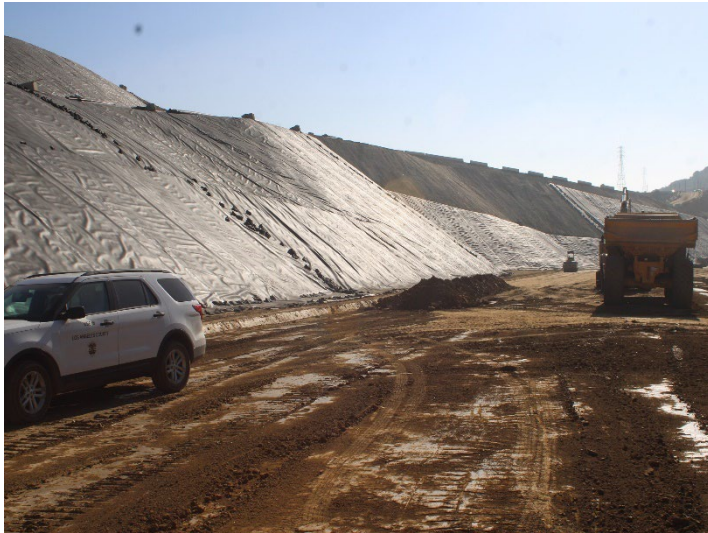
Photo 85: Working Area, CC-4 Part 4/5, CC-5A: October 8, 2025
