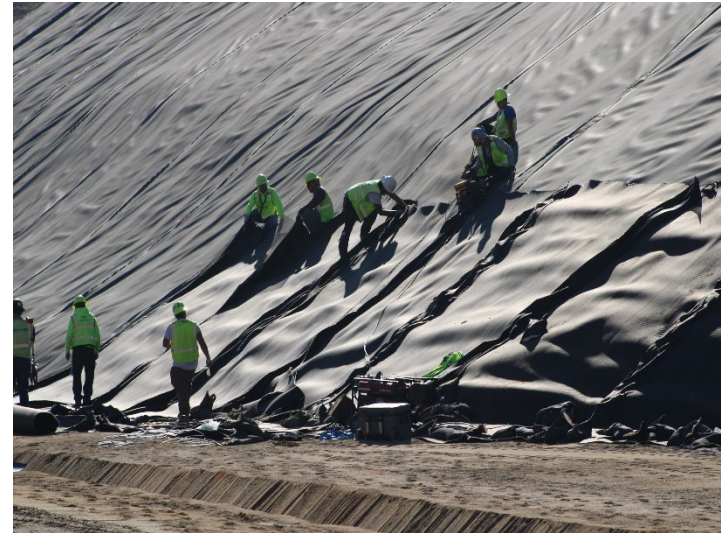
Photo 162: Working Area, CC-4 Part 4/5, CC-5A: November 6, 2025
