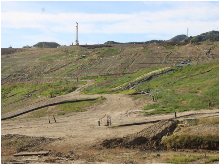
Photo 589: General Site: December 18, 2025
