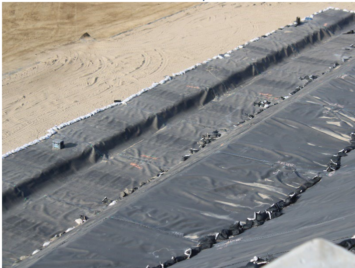
Photo 195: Working Area, CC-4 Part 4/5, CC-5A: December 18, 2025
