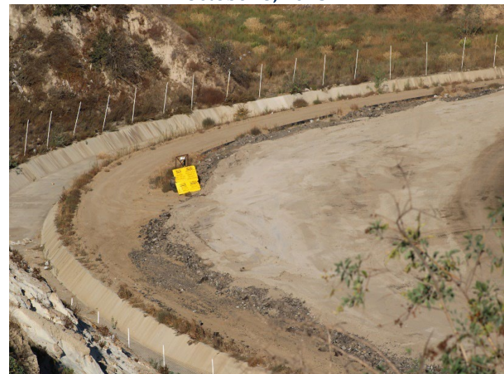
Photo 60: Working Area, CC-4 Part 4/5, CC-5A: October 8, 2025
