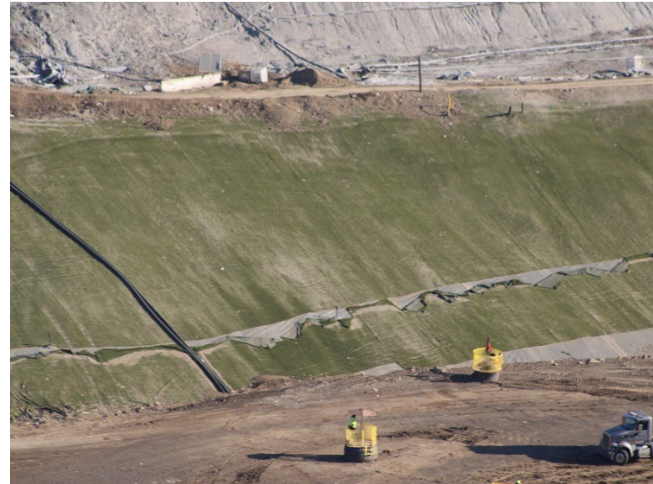
Photo 210: Closure Turf: October 8, 2025
