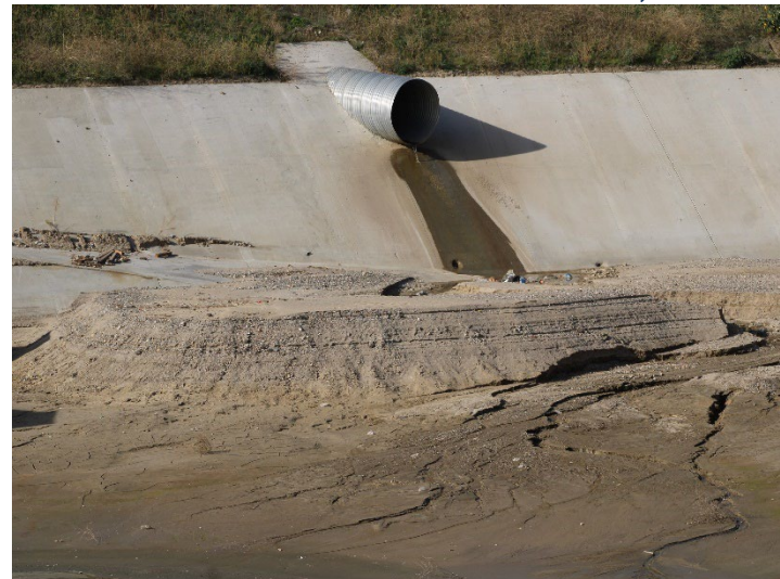
Photo 432: Terminal Basin: December 18, 2025
