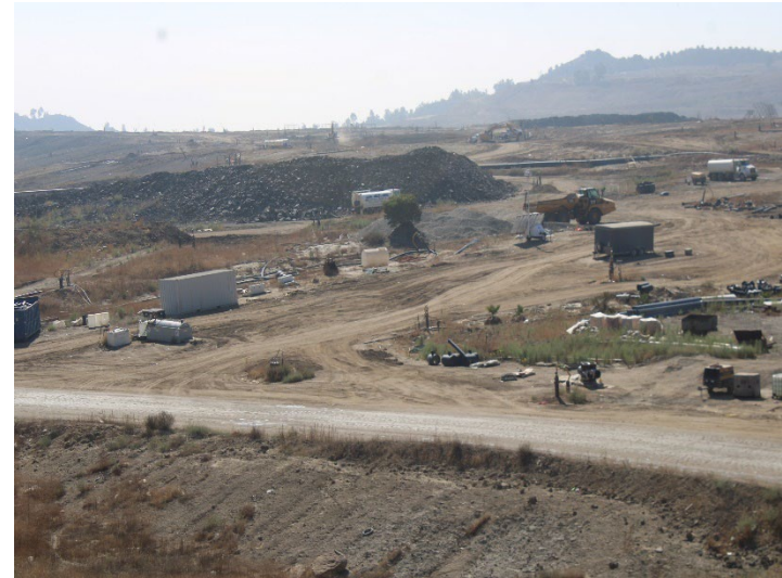
Photo 498: General Site: October 8, 2025
