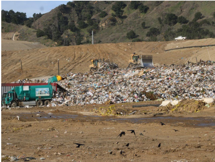
Photo 181: Working Area, CC-4 Part 4/5, CC-5A: December 18, 2025
