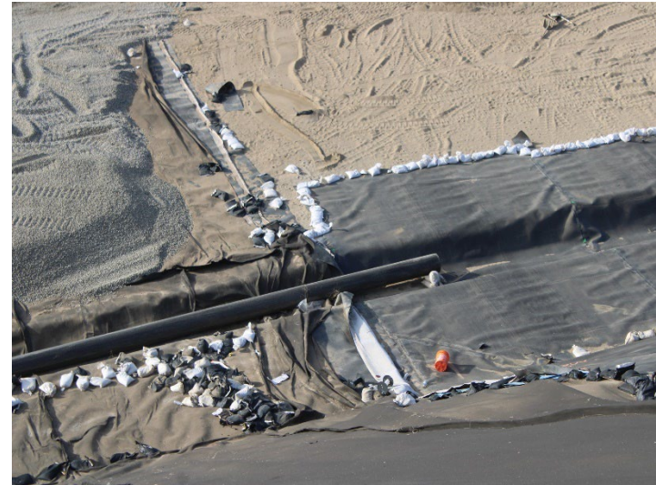
Photo 194: Working Area, CC-4 Part 4/5, CC-5A: December 18, 2025
