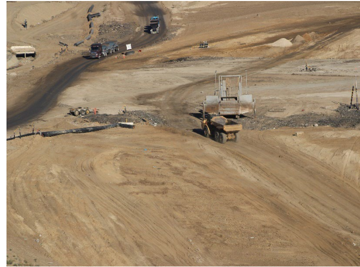
Photo 62: Working Area, CC-4 Part 4/5, CC-5A: October 8, 2025
