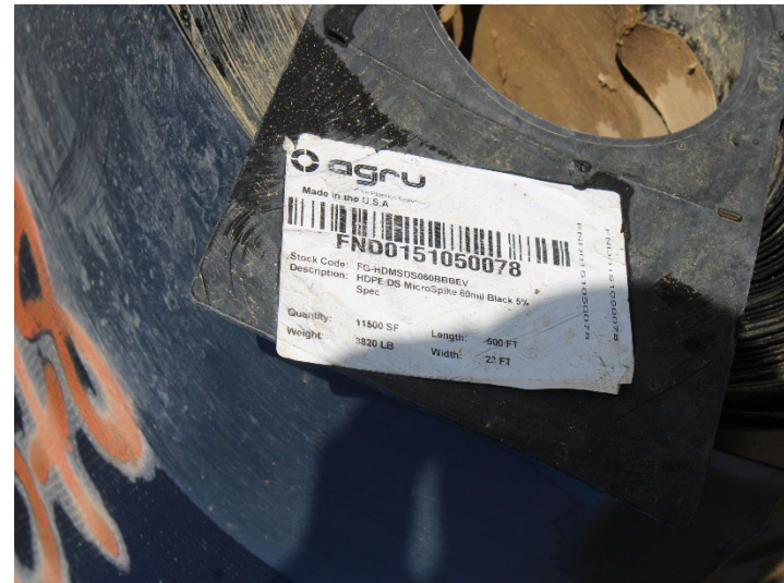
Photo 106: Working Area, CC-4 Part 4/5, CC-5A: October 8, 2025
