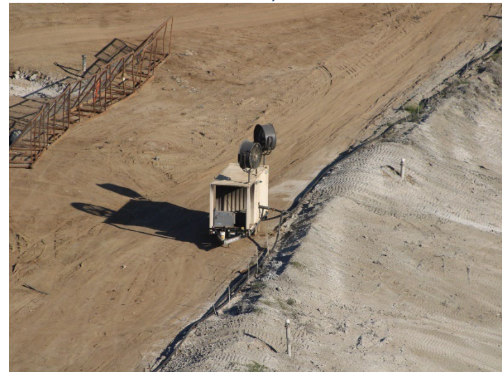
Photo 64: Working Area, CC-4 Part 4/5, CC-5A: October 8, 2025
