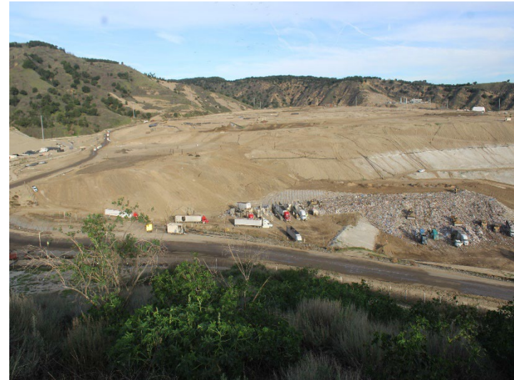
Photo 566: General Site: December 18, 2025
