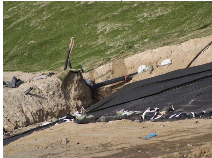
Photo 208: Working Area, CC-4 Part 4/5, CC-5A: December 18, 2025
