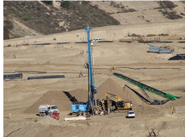
Photo 40: Working Area, CC-4 Part 3: November 6, 2025
