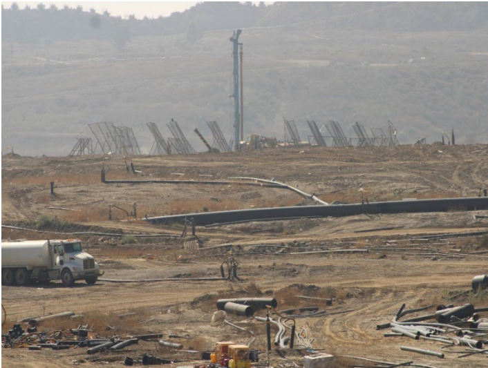
Photo 507: General Site: October 8, 2025
