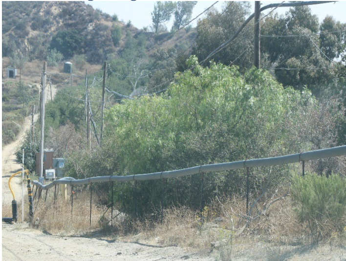
Photo 454: Southern Ownership Buffer: October 8, 2025
