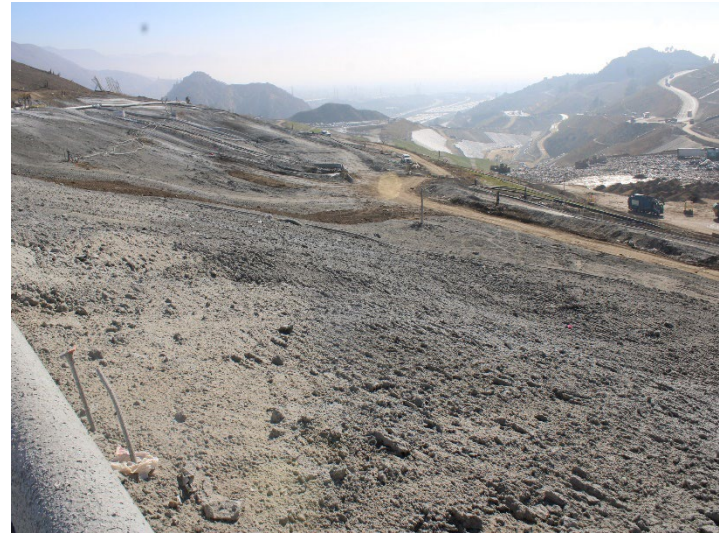
Photo 474: General Site: October 8, 2025
