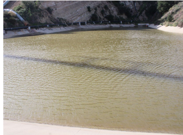
Photo 14: Basin A: December 18, 2025
