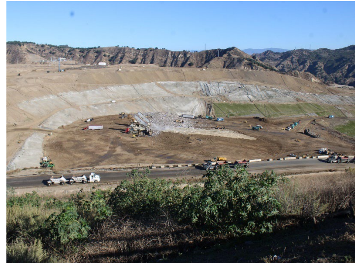
Photo 526: General Site: November 6, 2025
