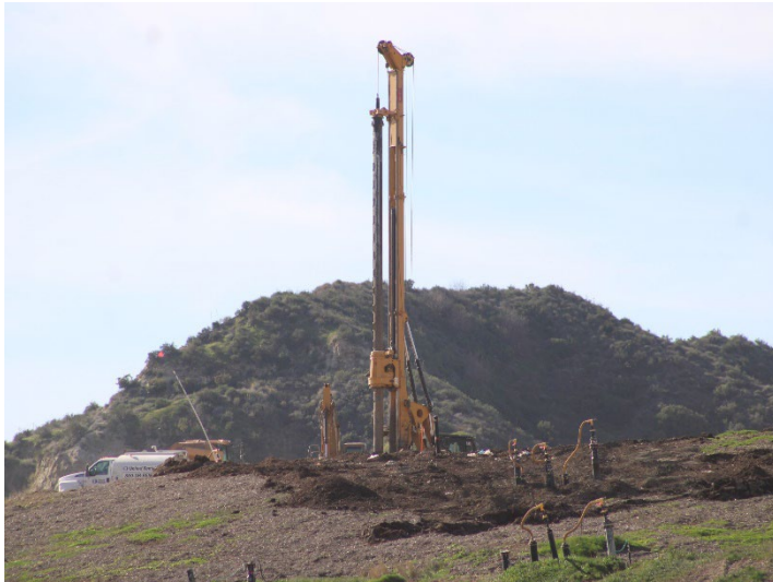
Photo 593: General Site: December 18, 2025
