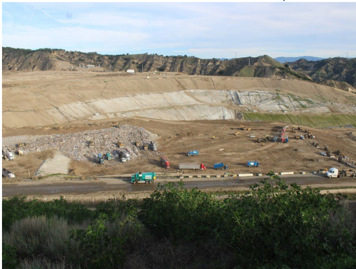
Photo 567: General Site: December 18, 2025
