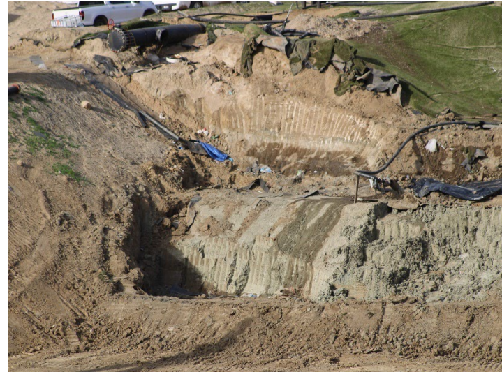
Photo 206: Working Area, CC-4 Part 4/5, CC-5A: December 18, 2025
