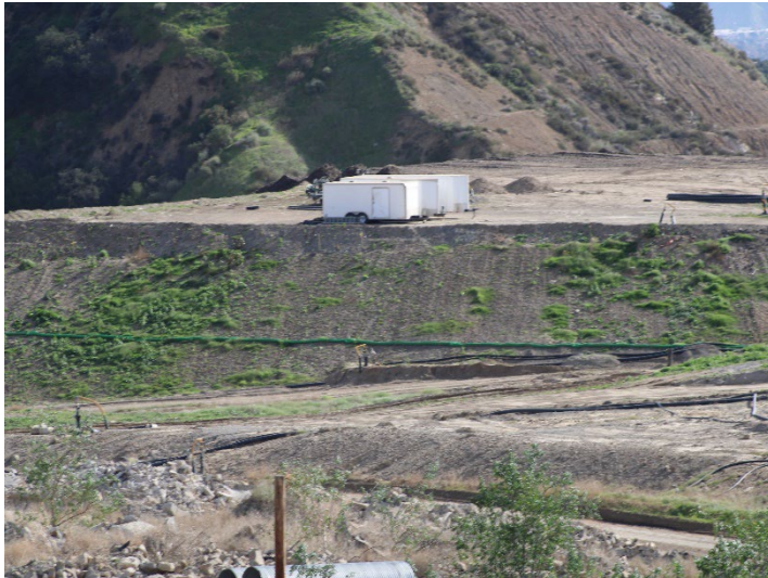
Photo 605: General Site: December 18, 2025
