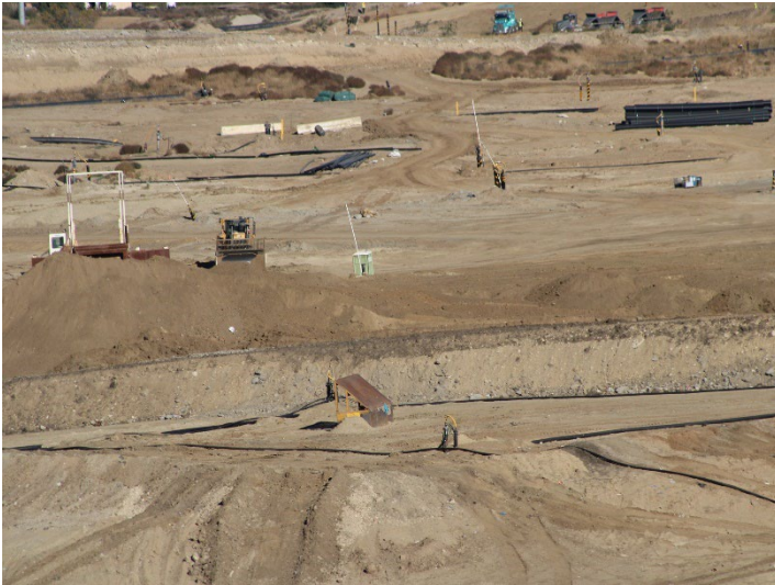
Photo 41: Working Area, CC-4 Part 3: November 6, 2025
