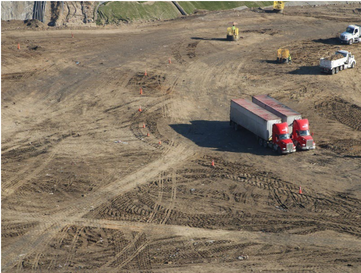
Photo 67: Working Area, CC-4 Part 4/5, CC-5A: October 8, 2025
