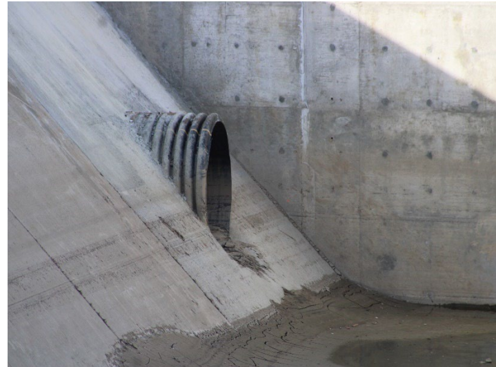
Photo 430: Terminal Basin: December 18, 2025
