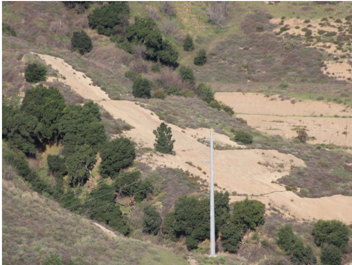
Photo 241: County Sage Mitigation Area and Westside Drainage Channels: December 18, 2025
