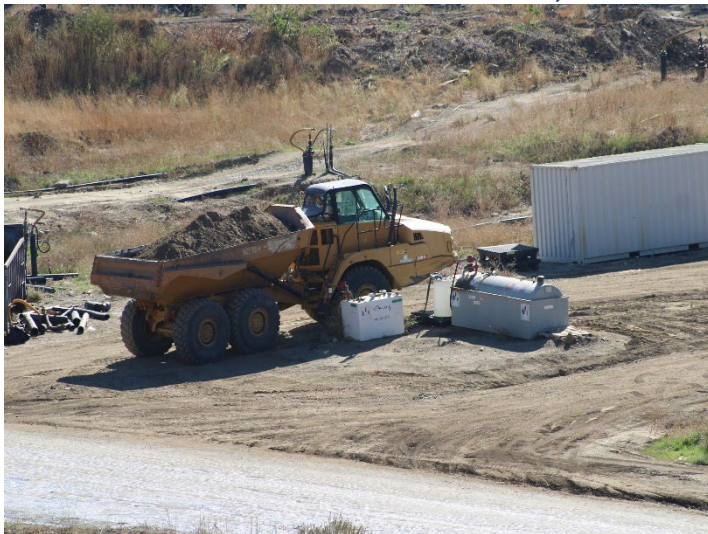
Photo 535: General Site: November 6, 2025
