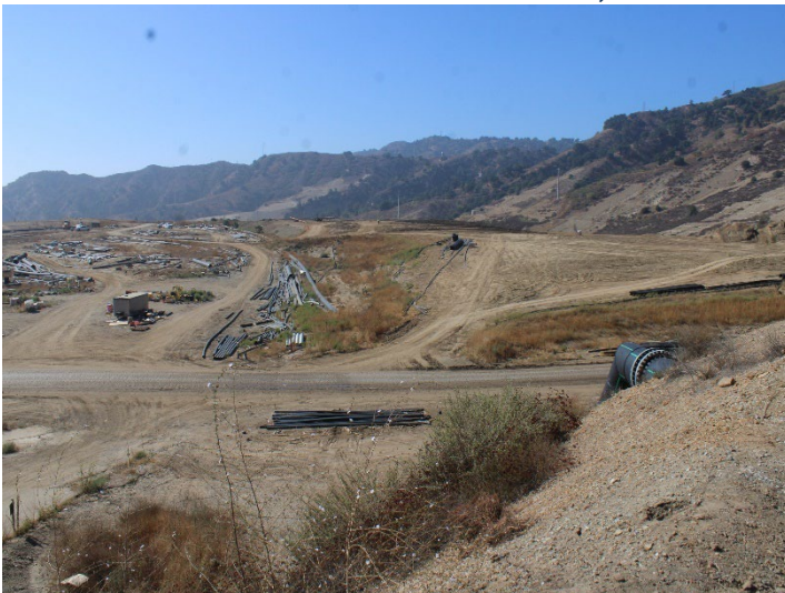
Photo 495: General Site: October 8, 2025
