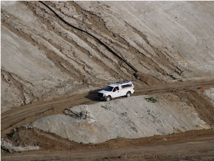
Photo 569: General Site: December 18, 2025
