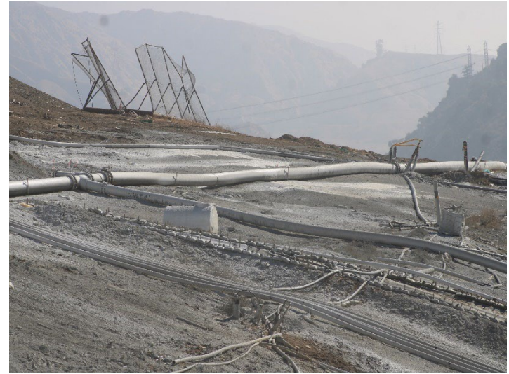
Photo 486: General Site: October 8, 2025
