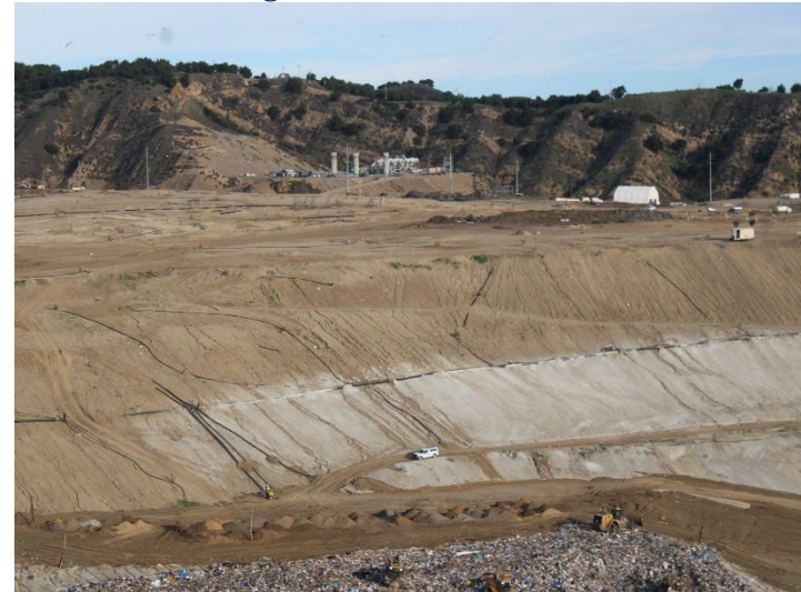
Photo 48: Working Area, CC-4 Part 3: December 18, 2025
