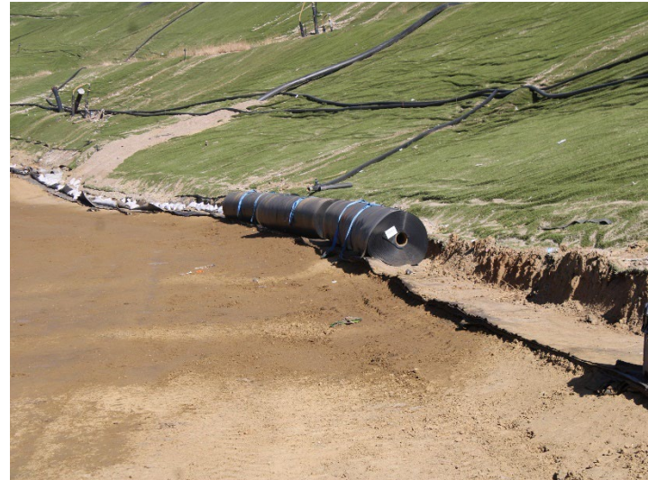
Photo 98: Working Area, CC-4 Part 4/5, CC-5A: October 8, 2025
