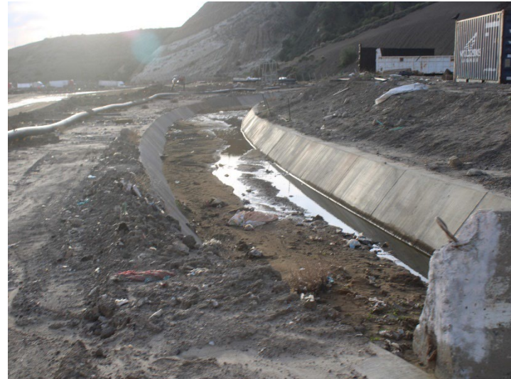
Photo 238: County Sage Mitigation Area and Westside Drainage Channels: December 18, 2025
