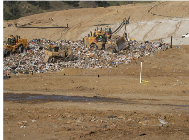
Photo 182: Working Area, CC-4 Part 4/5, CC-5A: December 18, 2025
