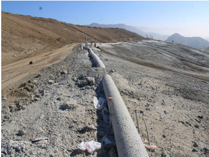
Photo 473: General Site: October 8, 2025
