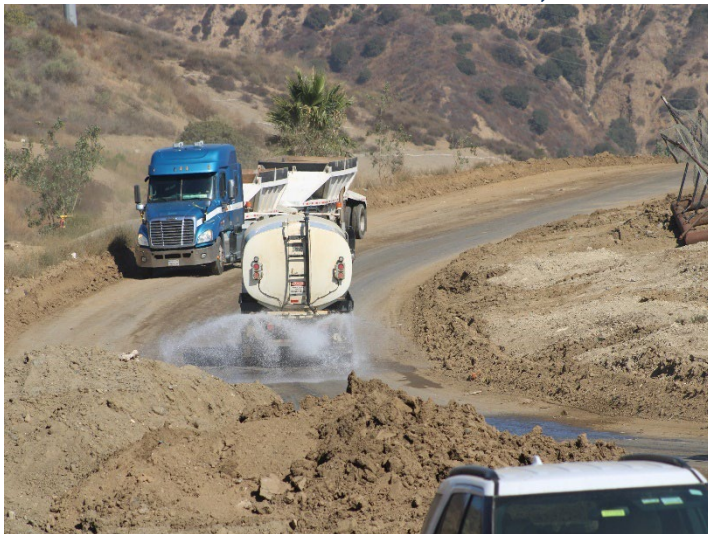
Photo 491: General Site: October 8, 2025
