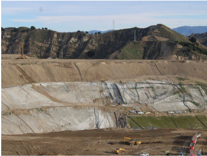
Photo 49: Working Area, CC-4 Part 3: December 18, 2025
