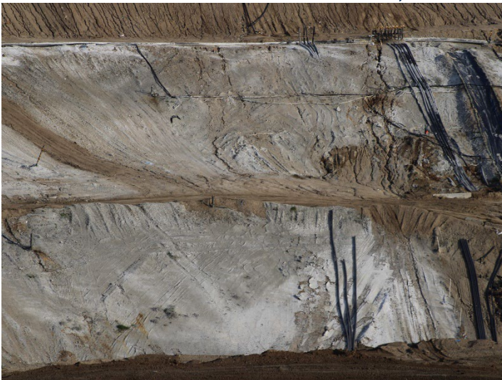
Photo 571: General Site: December 18, 2025
