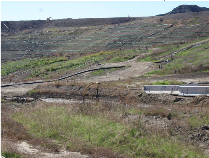
Photo 547: General Site: November 6, 2025
