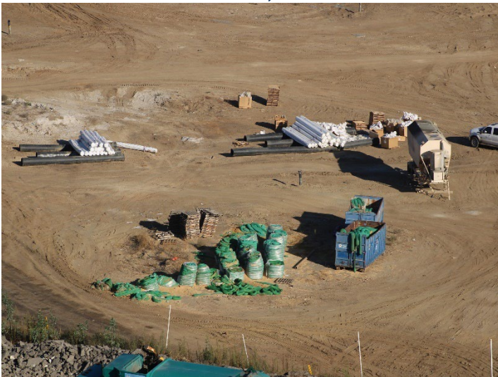
Photo 63: Working Area, CC-4 Part 4/5, CC-5A: October 8, 2025
