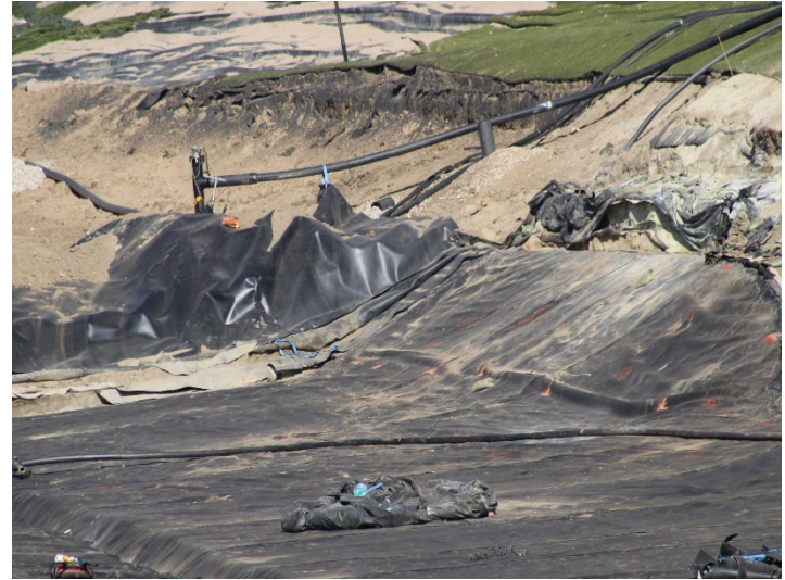
Photo 110: Working Area, CC-4 Part 4/5, CC-5A: October 8, 2025
