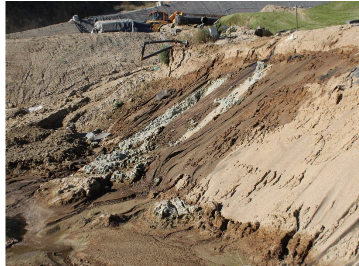
Photo 150: Working Area, CC-4 Part 4/5, CC-5A: November 6, 2025
