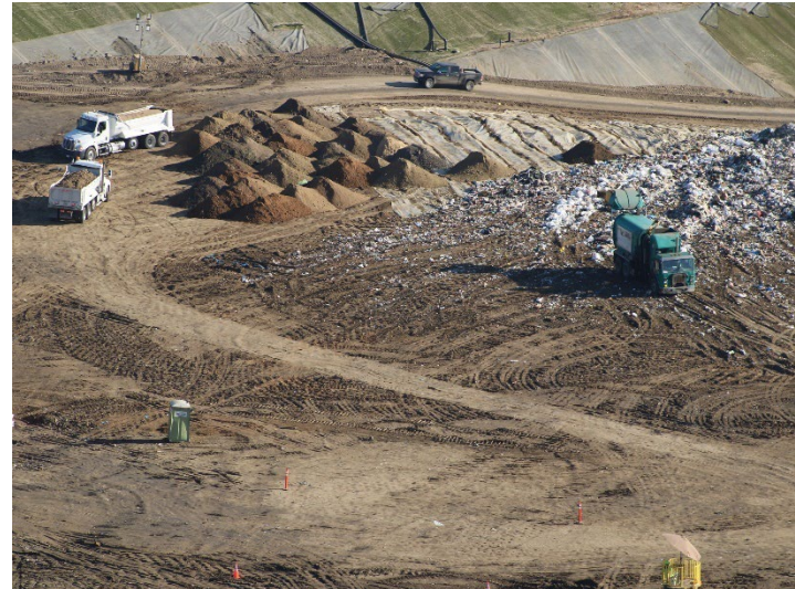
Photo 68: Working Area, CC-4 Part 4/5, CC-5A: October 8, 2025
