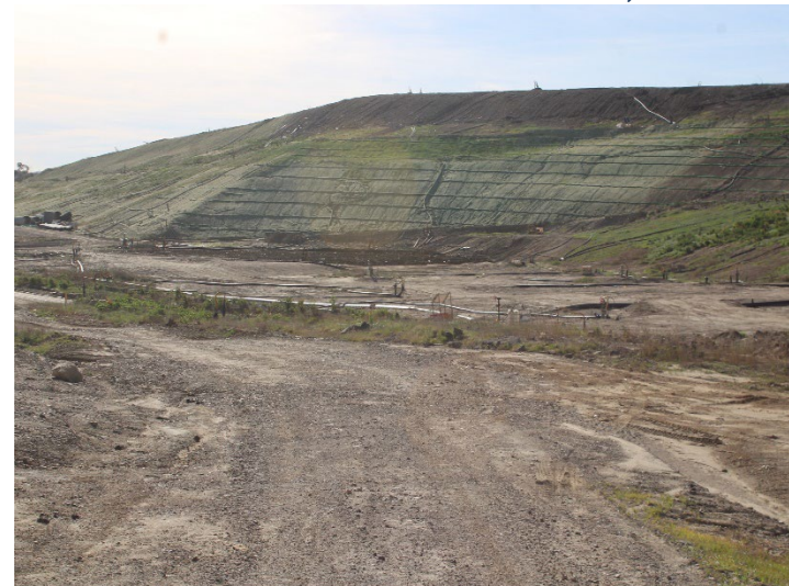
Photo 588: General Site: December 18, 2025
