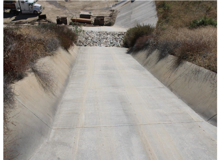
Photo 364: Eastside Drainage Channel: November 6, 2025
