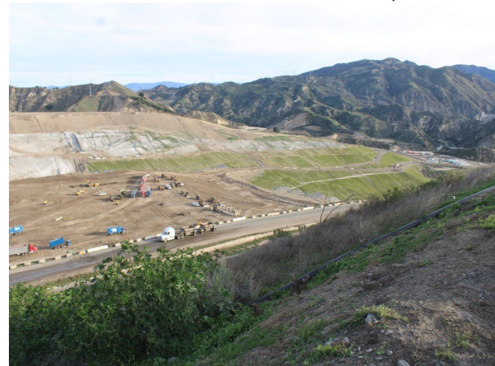
Photo 568: General Site: December 18, 2025
