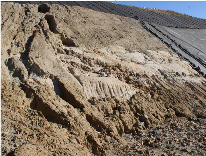
Photo 155: Working Area, CC-4 Part 4/5, CC-5A: November 6, 2025
