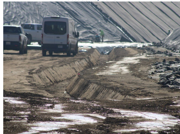
Photo 92: Working Area, CC-4 Part 4/5, CC-5A: October 8, 2025
