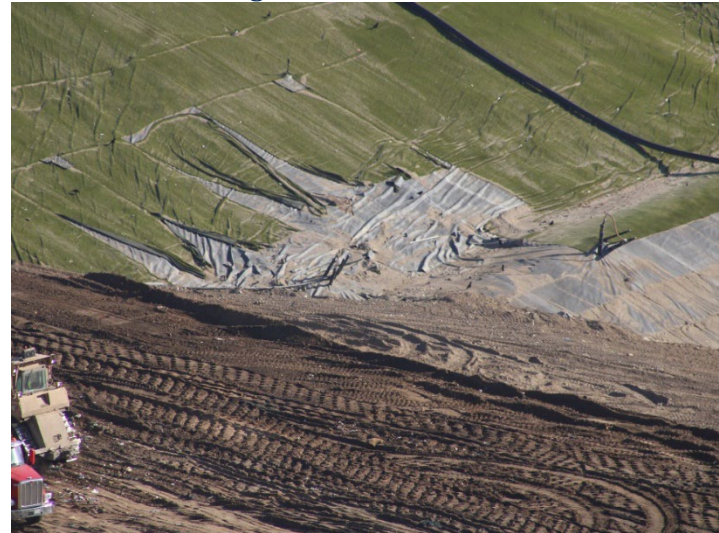
Photo 36: Working Area, CC-4 Part 3: October 8, 2025
