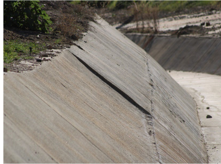
Photo 374: Eastside Drainage Channel: December 18, 2025
