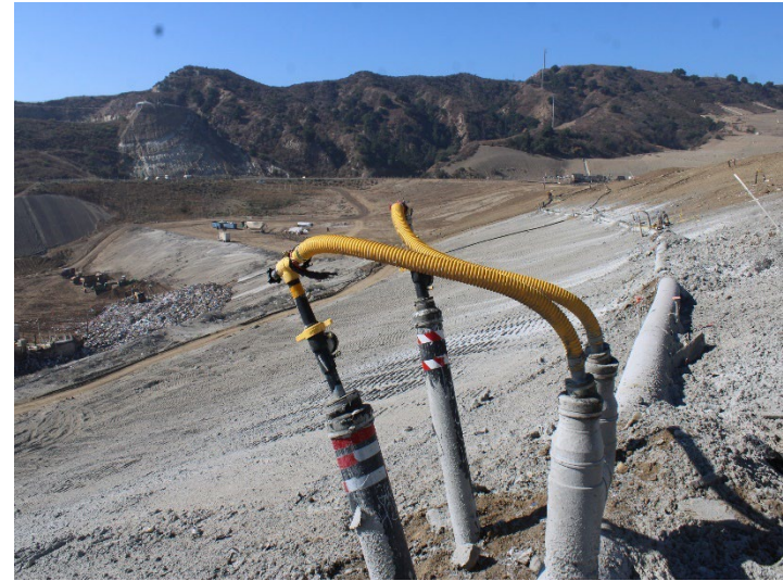
Photo 478: General Site: October 8, 2025
