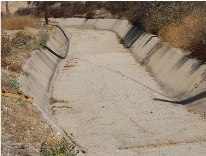
Photo 355: Eastside Drainage Channel: October 8, 2025
