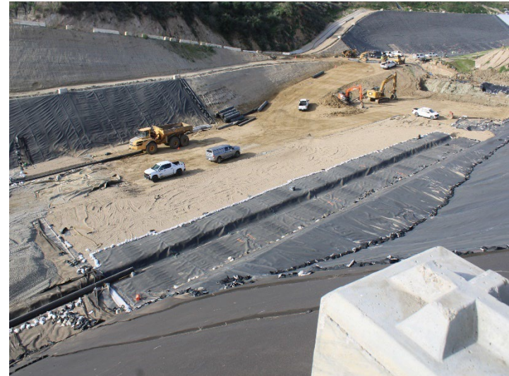
Photo 190: Working Area, CC-4 Part 4/5, CC-5A: December 18, 2025
