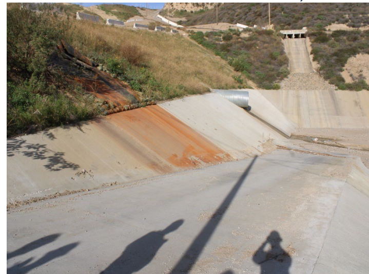
Photo 416: Terminal Basin: December 18, 2025
