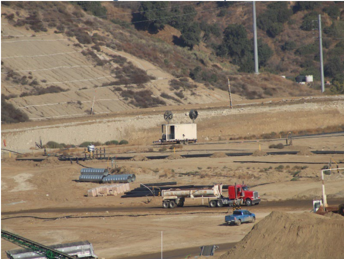
Photo 23: Working Area, CC4 Part 1/2: October 8, 2025
