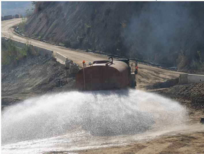
Photo 471: General Site: October 8, 2025
