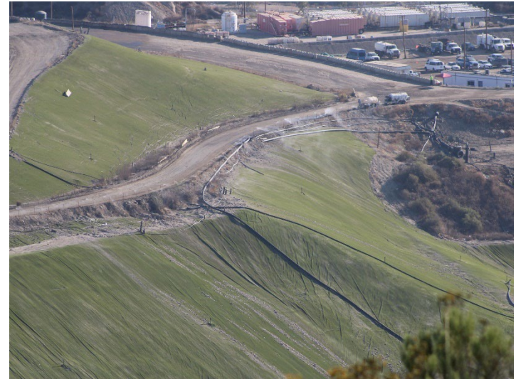
Photo 214: Closure Turf: October 8, 2025
