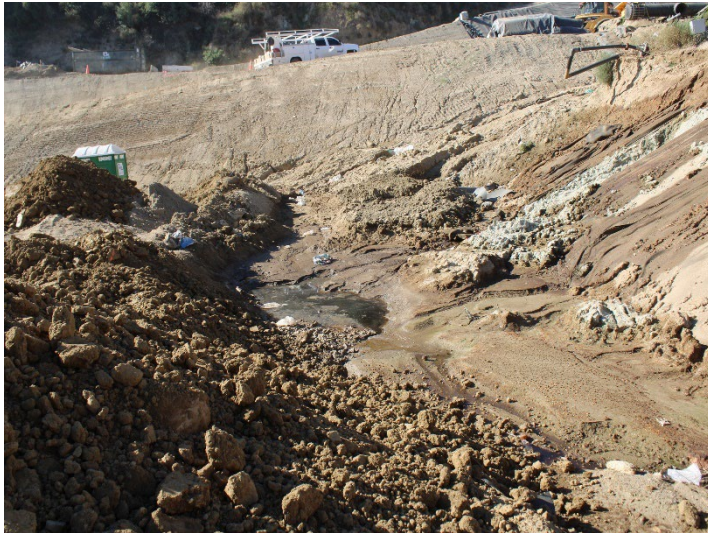
Photo 149: Working Area, CC-4 Part 4/5, CC-5A: November 6, 2025
