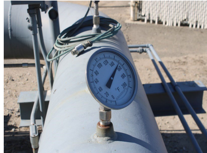
Photo 554: General Site: November 6, 2025
