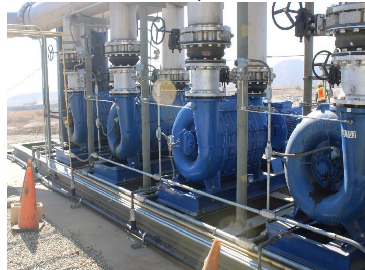
Photo 256: Flares 9, 10, 11 and Gas-to-Energy Facility: October 8, 2025
