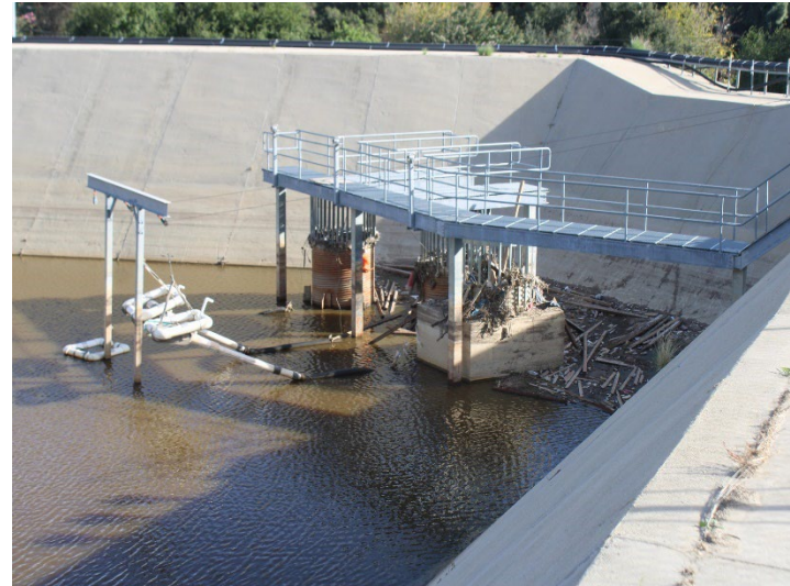
Photo 422: Terminal Basin: December 18, 2025
