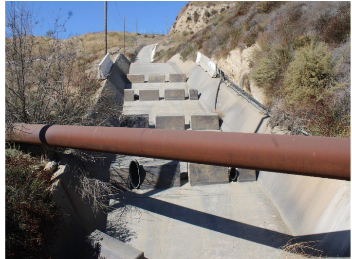
Photo 362: Eastside Drainage Channel: November 6, 2025
