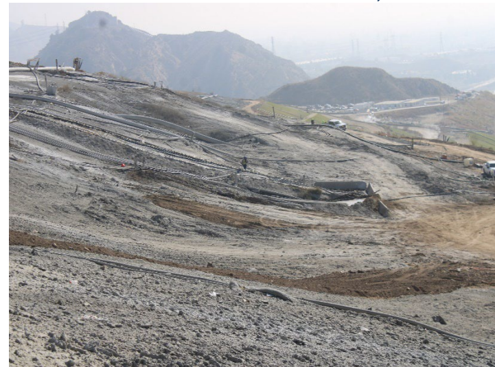
Photo 480: General Site: October 8, 2025
