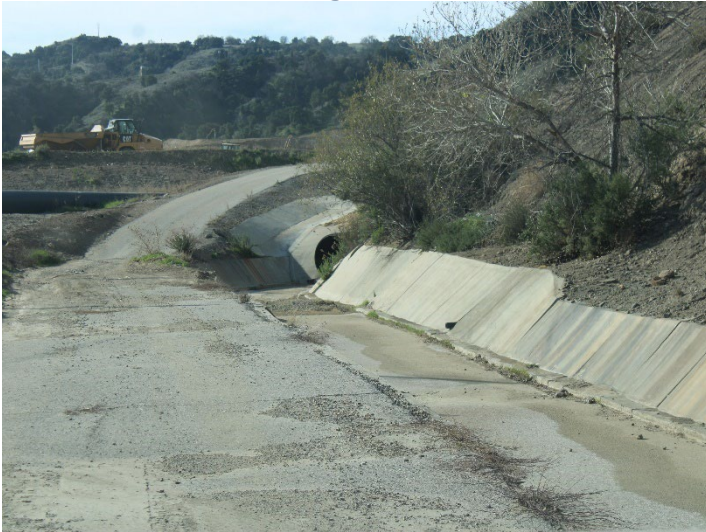
Photo 375: Eastside Drainage Channel: December 18, 2025
