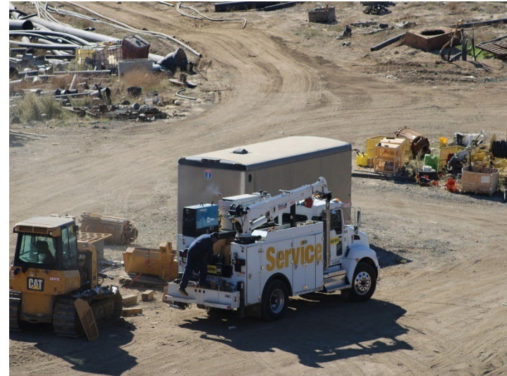
Photo 538: General Site: November 6, 2025
