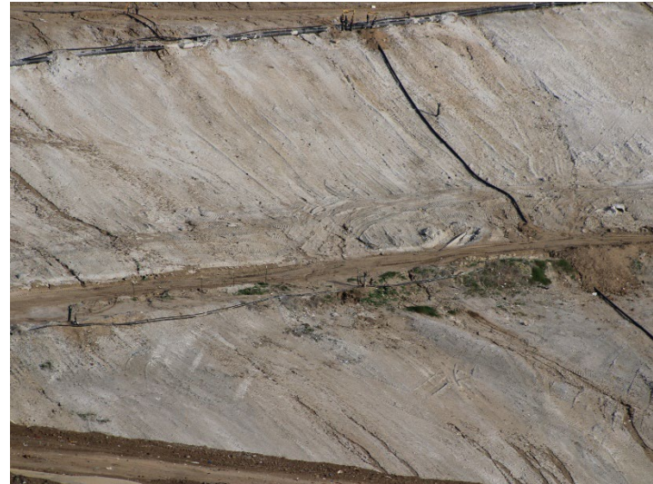
Photo 570: General Site: December 18, 2025
