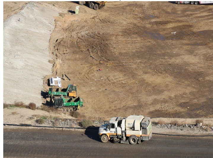
Photo 136: Working Area, CC-4 Part 4/5, CC-5A: November 6, 2025
