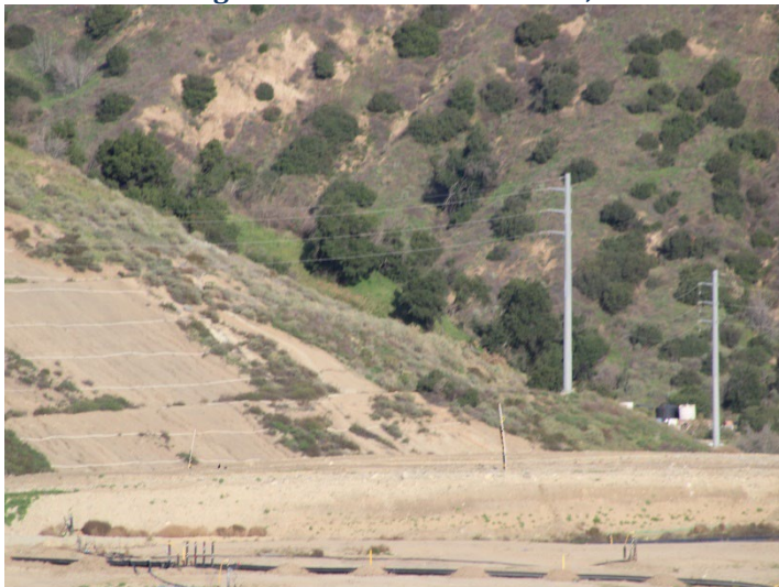
Photo 243: County Sage Mitigation Area and Westside Drainage Channels: December 18, 2025
