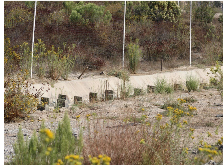
Photo 450: Sage Mitigation, Deck B: October 8, 2025
