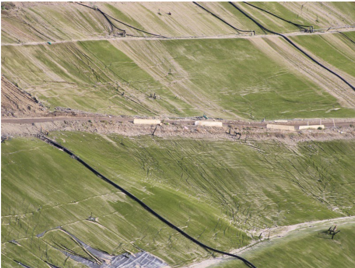
Photo 219: Closure Turf: December 18, 2025
