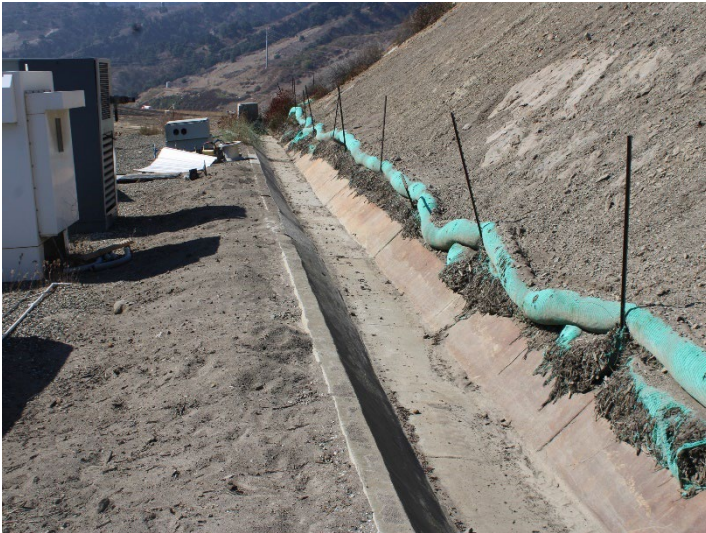
Photo 261: Flares 9, 10, 11 and Gas-to-Energy Facility: October 8, 2025
