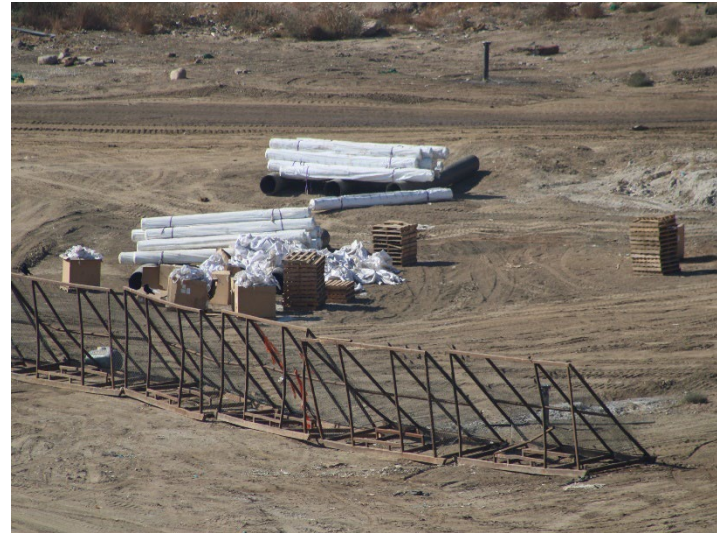
Photo 126: Working Area, CC-4 Part 4/5, CC-5A: October 8, 2025
