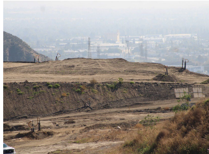
Photo 542: General Site: November 6, 2025
