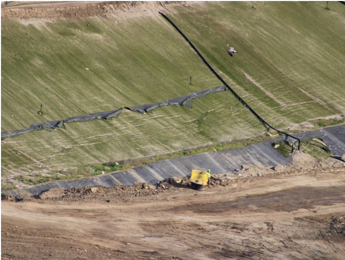
Photo 217: Closure Turf: December 18, 2025
