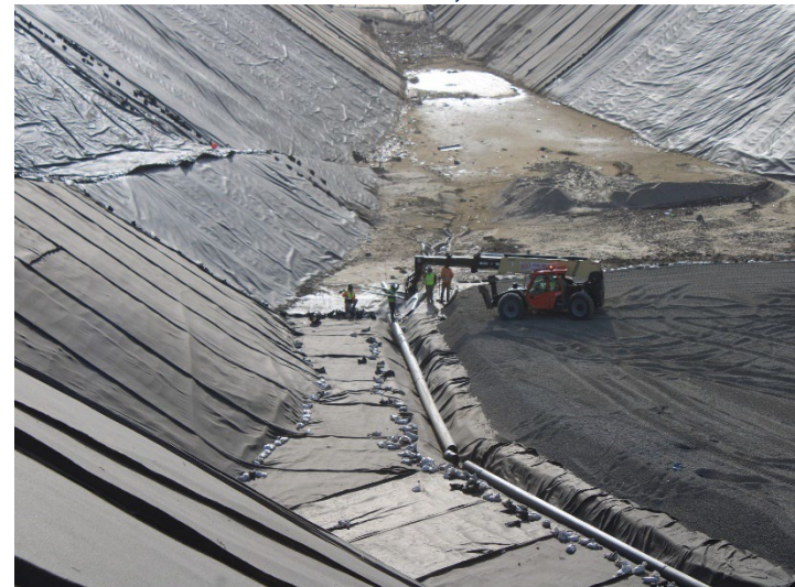
Photo 192: Working Area, CC-4 Part 4/5, CC-5A: December 18, 2025
