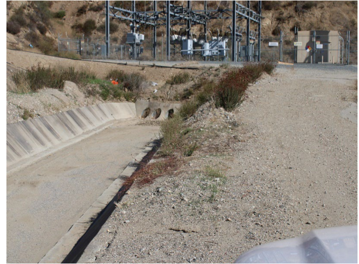
Photo 358: Eastside Drainage Channel: November 6, 2025
