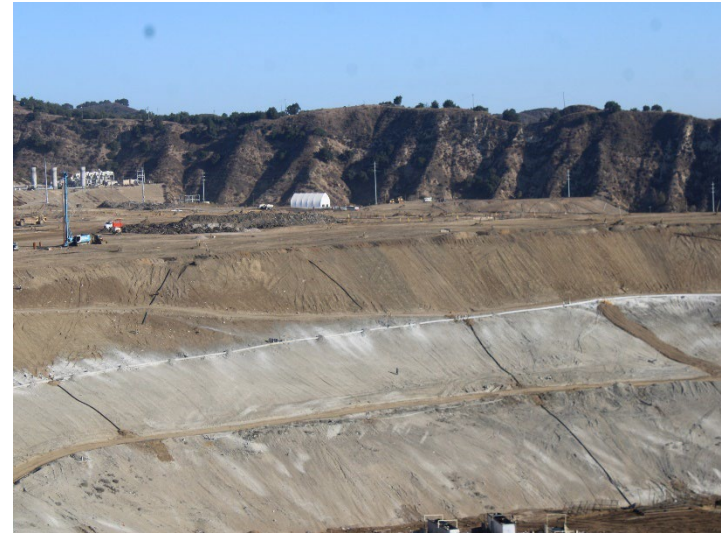
Photo 58: Working Area, CC-4 Part 4/5, CC-5A: October 8, 2025
