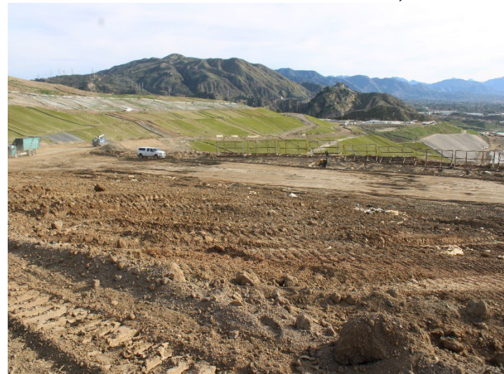
Photo 580: General Site: December 18, 2025
