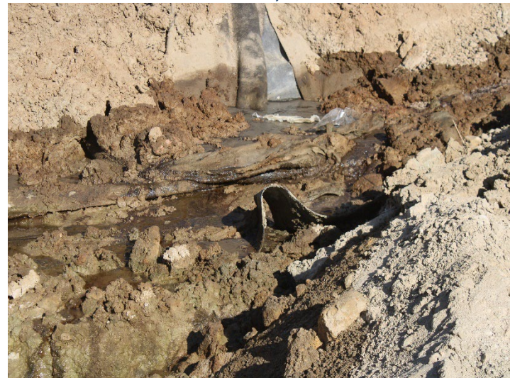
Photo 80: Working Area, CC-4 Part 4/5, CC-5A: October 8, 2025
