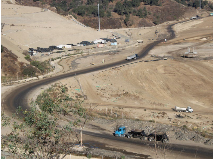
Photo 51: Working Area, CC-4 Part 4/5, CC-5A: October 8, 2025
