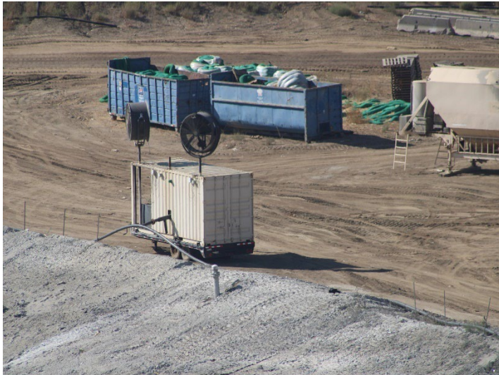
Photo 125: Working Area, CC-4 Part 4/5, CC-5A: October 8, 2025
