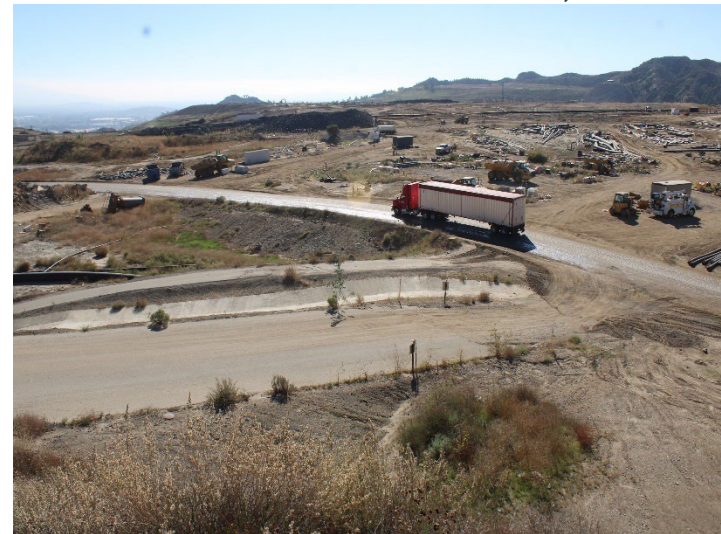
Photo 532: General Site: November 6, 2025
