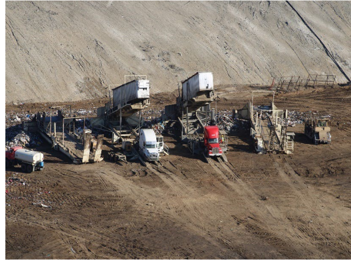
Photo 66: Working Area, CC-4 Part 4/5, CC-5A: October 8, 2025
