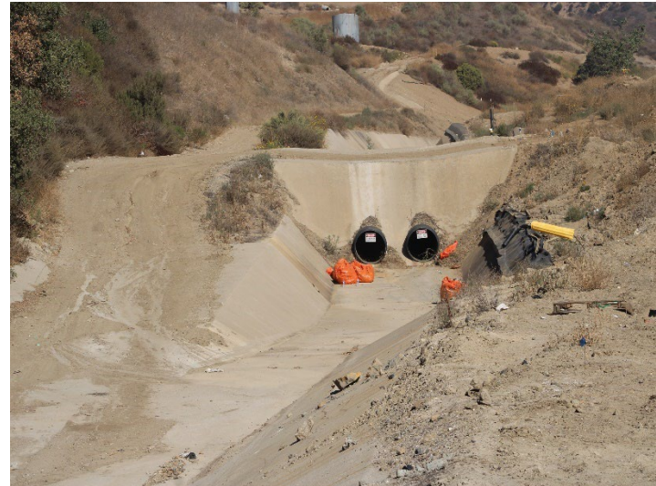
Photo 354: Eastside Drainage Channel: October 8, 2025
