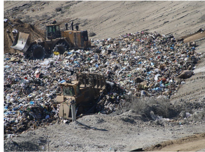
Photo 122: Working Area, CC-4 Part 4/5, CC-5A: October 8, 2025
