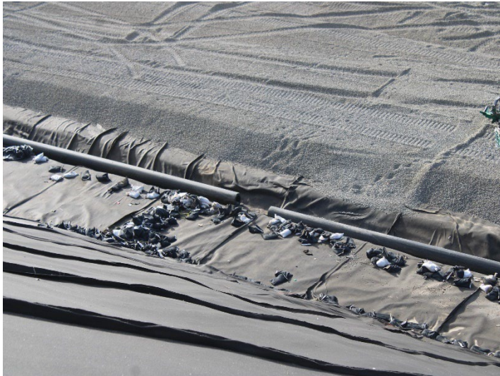
Photo 193: Working Area, CC-4 Part 4/5, CC-5A: December 18, 2025
