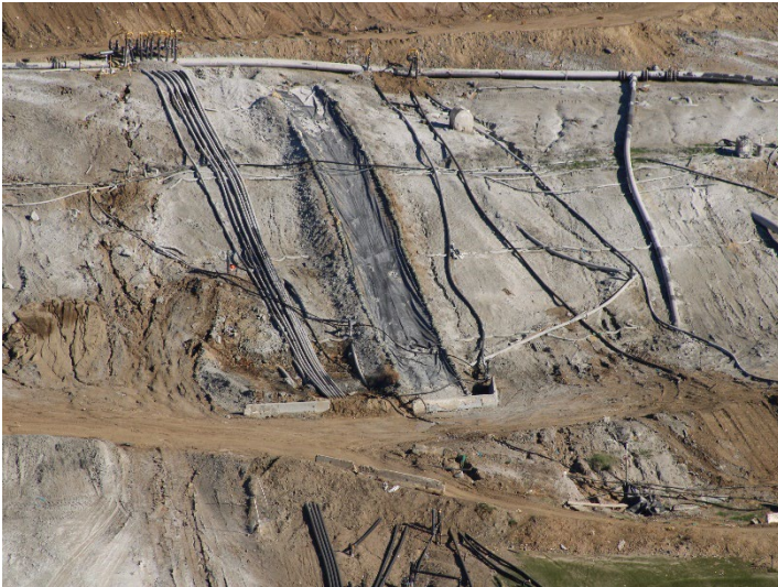
Photo 141: Working Area, CC-4 Part 4/5, CC-5A: November 6, 2025
