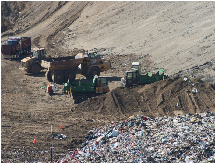
Photo 121: Working Area, CC-4 Part 4/5, CC-5A: October 8, 2025
