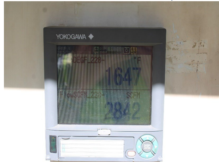
Photo 552: General Site: November 6, 2025
