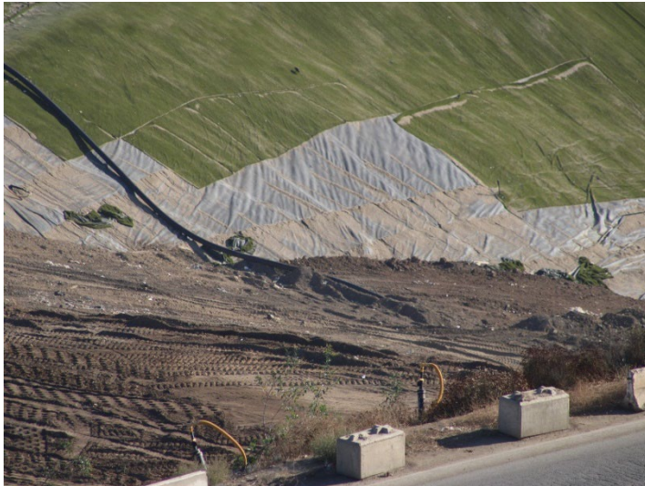
Photo 37: Working Area, CC-4 Part 3: October 8, 2025
