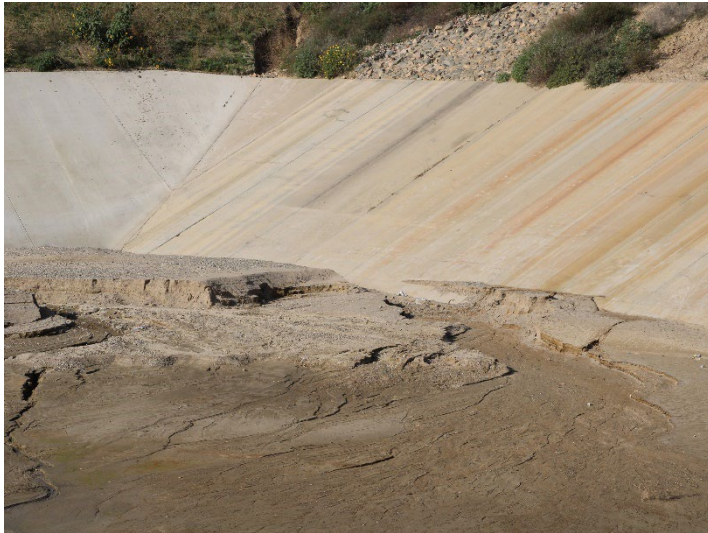
Photo 433: Terminal Basin: December 18, 2025
