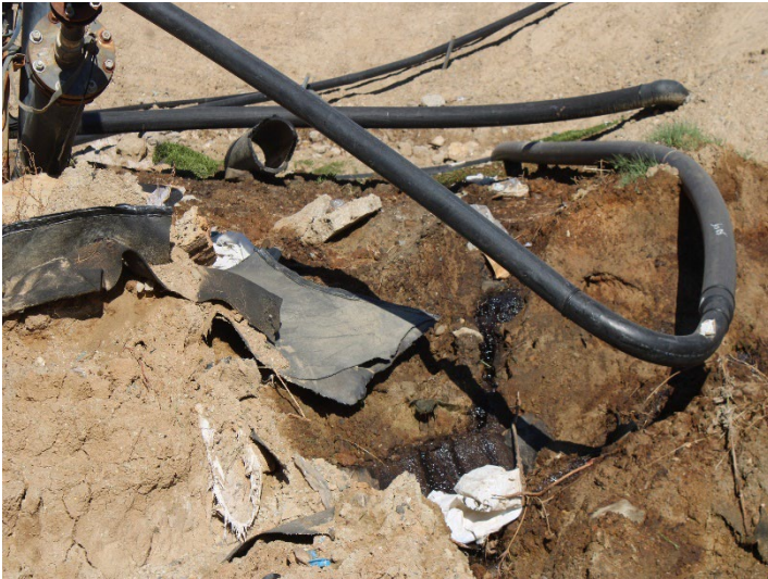
Photo 153: Working Area, CC-4 Part 4/5, CC-5A: November 6, 2025
