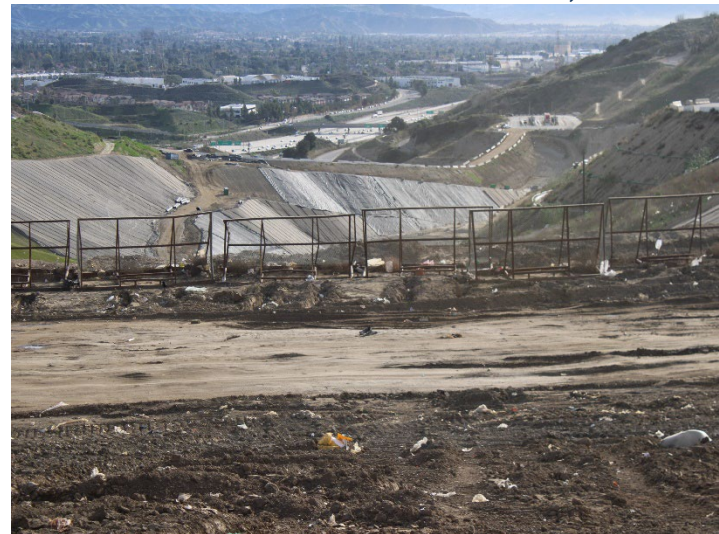
Photo 584: General Site: December 18, 2025
