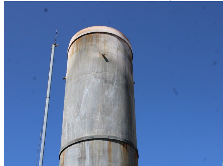
Photo 520: General Site: October 8, 2025
