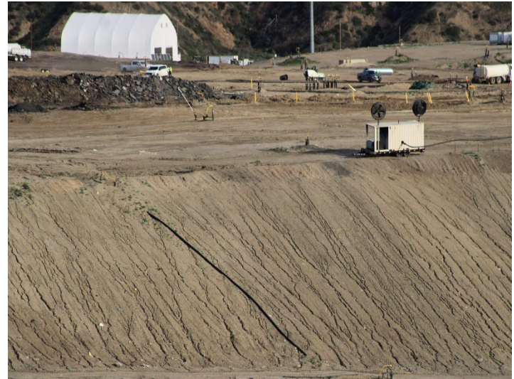
Photo 30: Working Area, CC4 Part 1/2: December 18, 2025
