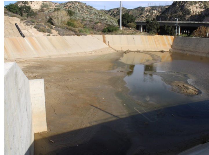
Photo 420: Terminal Basin: December 18, 2025
