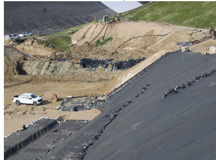
Photo 196: Working Area, CC-4 Part 4/5, CC-5A: December 18, 2025
