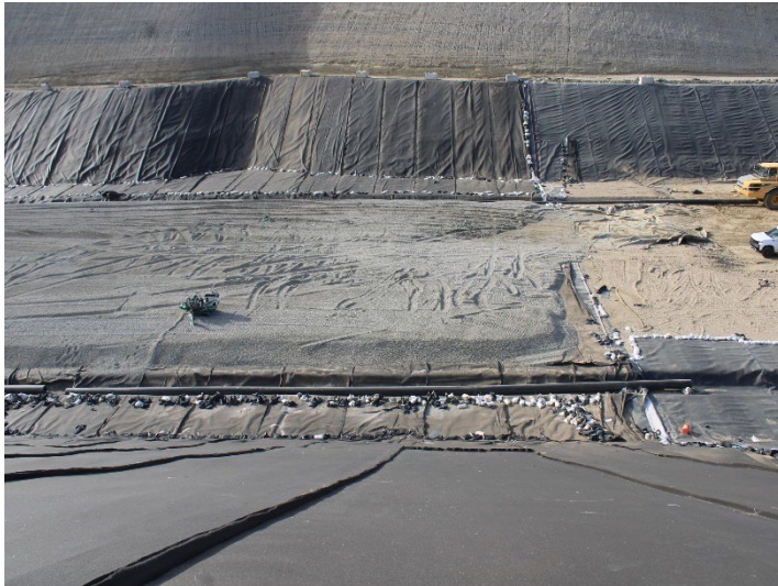
Photo 189: Working Area, CC-4 Part 4/5, CC-5A: December 18, 2025
