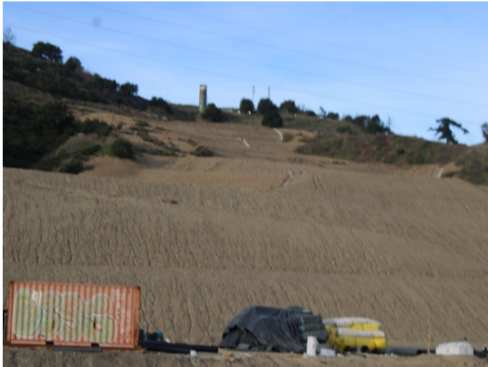
Photo 561: General Site: December 18, 2025
