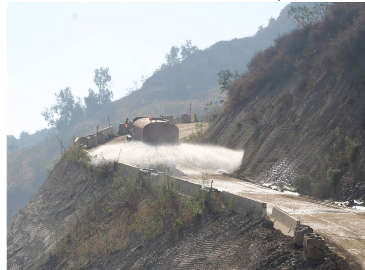
Photo 472: General Site: October 8, 2025
