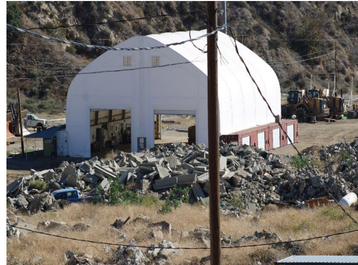
Photo 534: General Site: November 6, 2025
