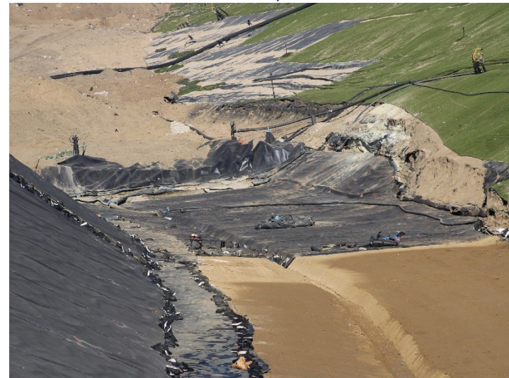
Photo 108: Working Area, CC-4 Part 4/5, CC-5A: October 8, 2025
