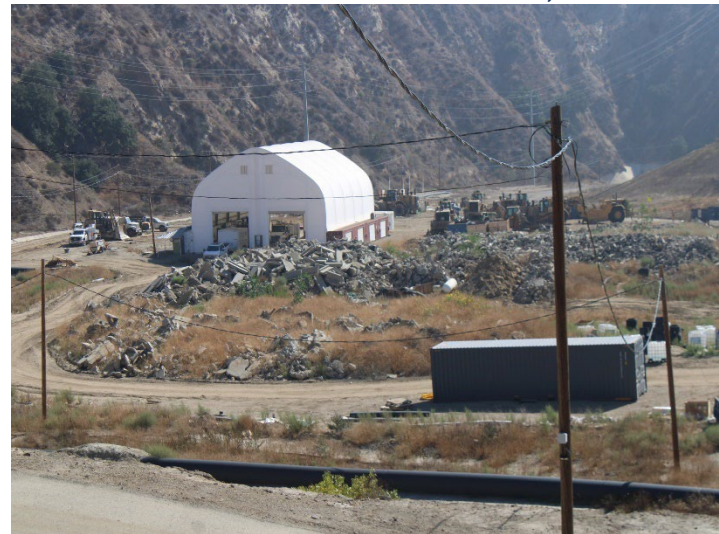
Photo 496: General Site: October 8, 2025
