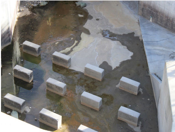
Photo 437: Terminal Basin: December 18, 2025
