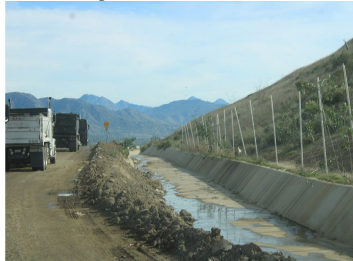
Photo 248: County Sage Mitigation Area and Westside Drainage Channels: December 18, 2025
