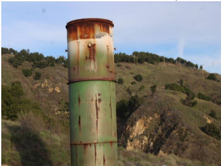
Photo 563: General Site: December 18, 2025
