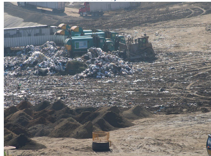
Photo 116: Working Area, CC-4 Part 4/5, CC-5A: October 8, 2025
