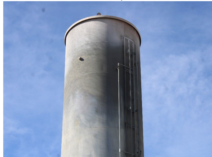
Photo 280: Flares 9, 10, 11 and Gas-to-Energy Facility: December 18, 2025
