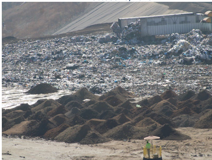
Photo 115: Working Area, CC-4 Part 4/5, CC-5A: October 8, 2025
