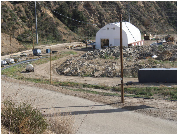
Photo 599: General Site: December 18, 2025
