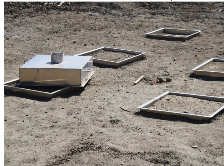
Photo 516: General Site: October 8, 2025
