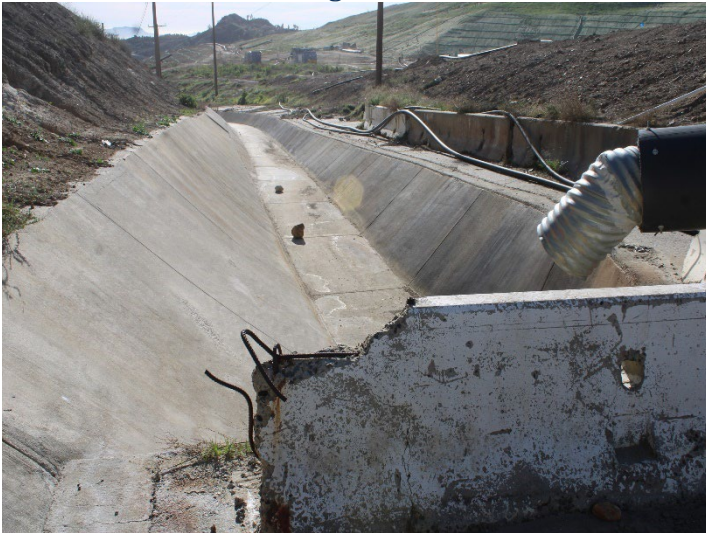
Photo 371: Eastside Drainage Channel: December 18, 2025
