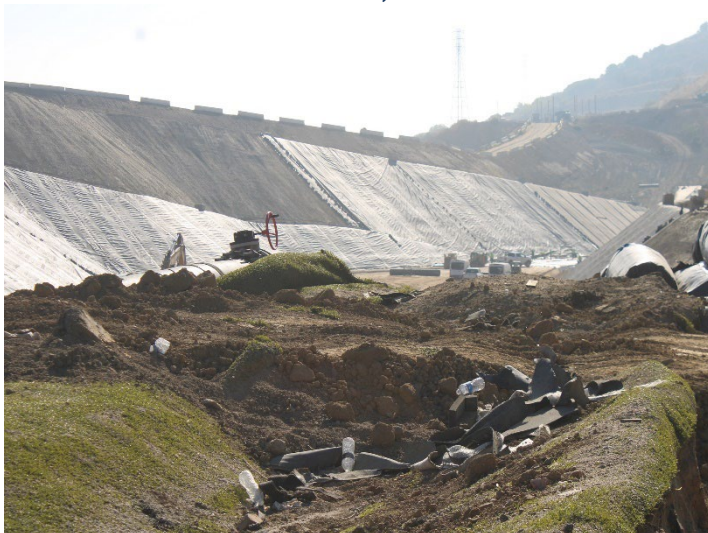
Photo 103: Working Area, CC-4 Part 4/5, CC-5A: October 8, 2025
