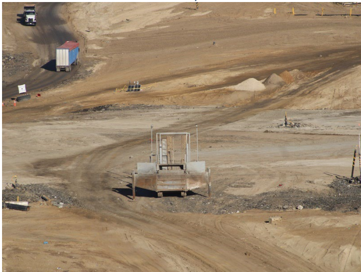
Photo 71: Working Area, CC-4 Part 4/5, CC-5A: October 8, 2025
