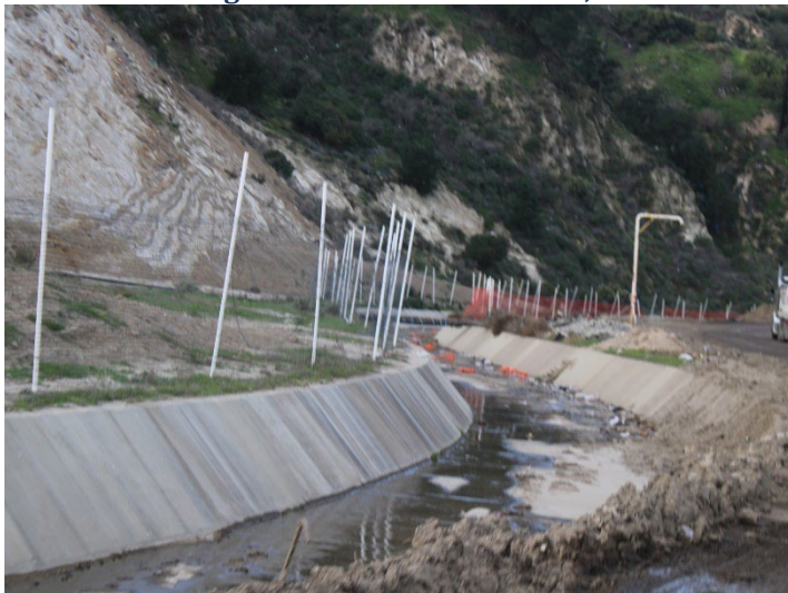
Photo 235: County Sage Mitigation Area and Westside Drainage Channels: December 18, 2025
