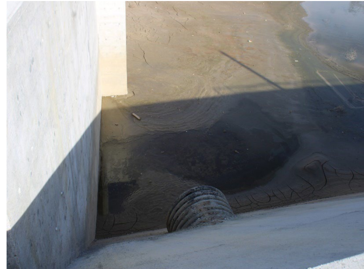
Photo 418: Terminal Basin: December 18, 2025
