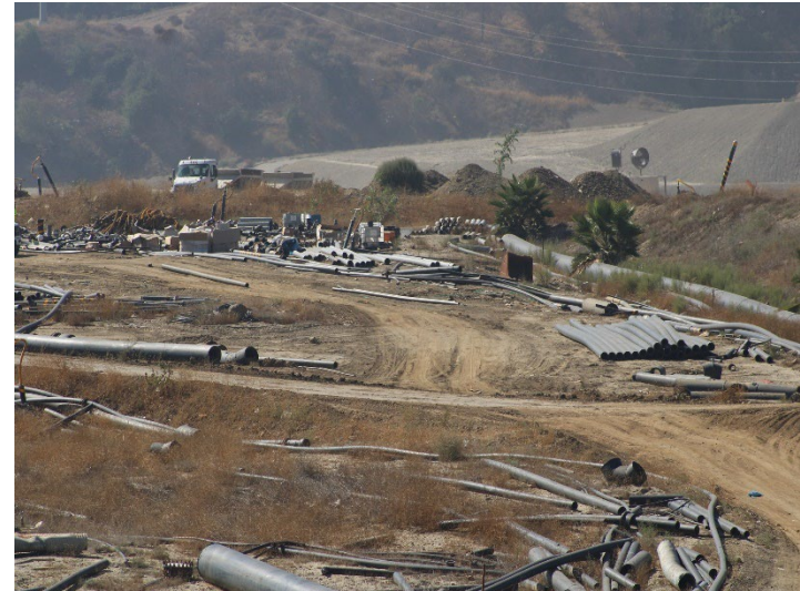
Photo 510: General Site: October 8, 2025
