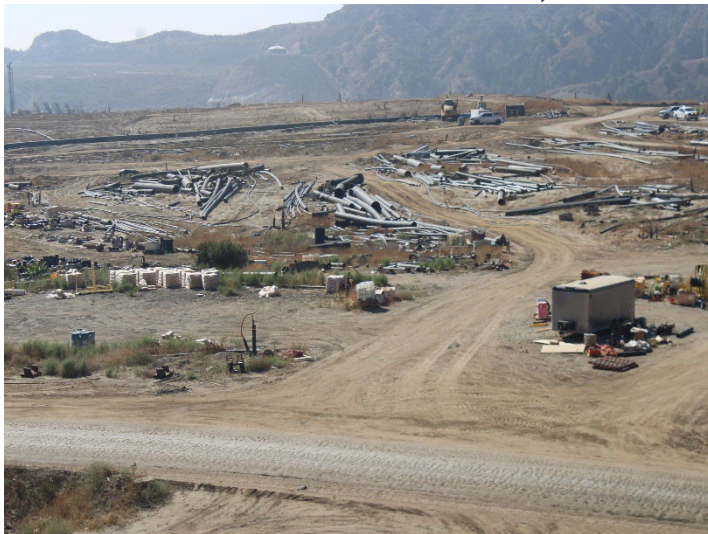
Photo 499: General Site: October 8, 2025
