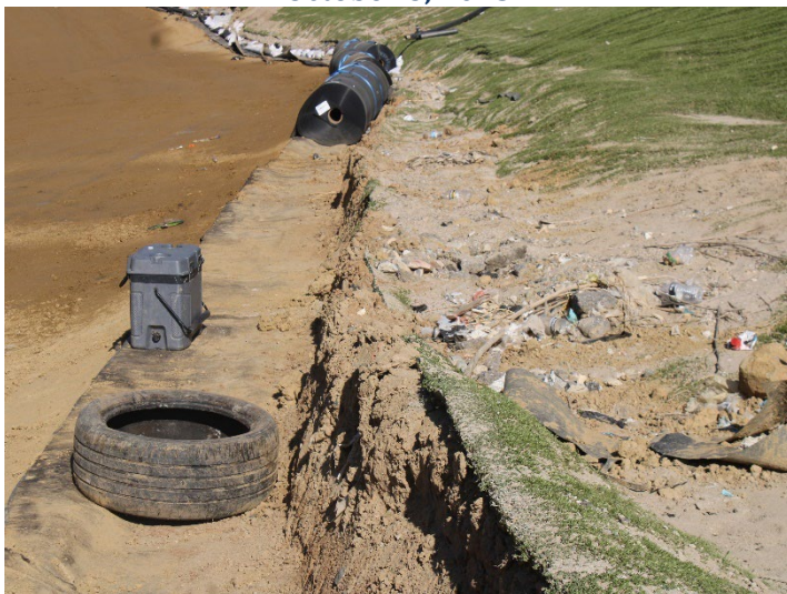
Photo 99: Working Area, CC-4 Part 4/5, CC-5A: October 8, 2025
