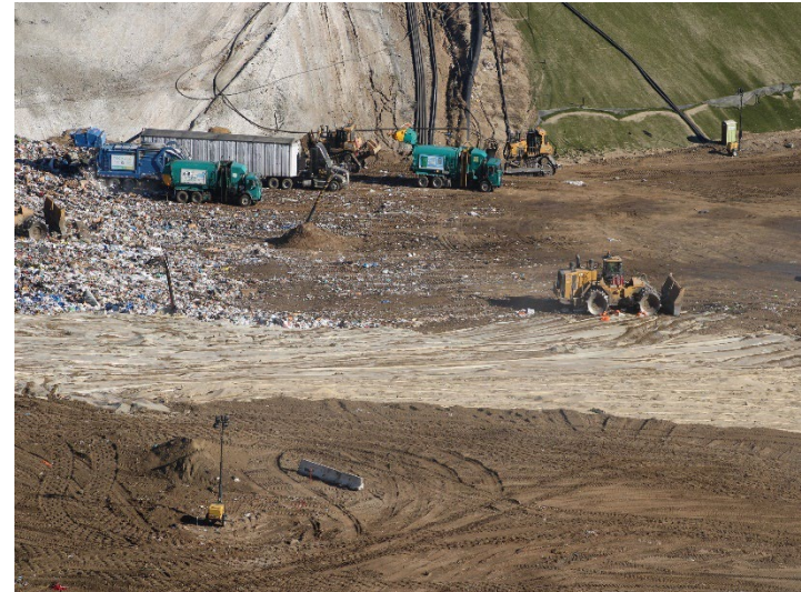
Photo 138: Working Area, CC-4 Part 4/5, CC-5A: November 6, 2025
