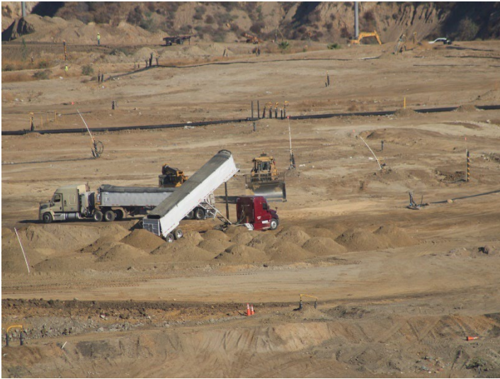
Photo 21: Working Area, CC4 Part 1/2: October 8, 2025
