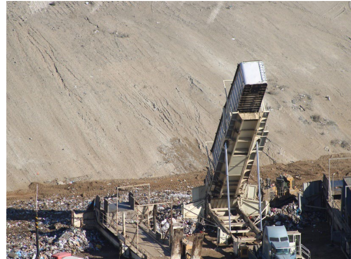
Photo 74: Working Area, CC-4 Part 4/5, CC-5A: October 8, 2025
