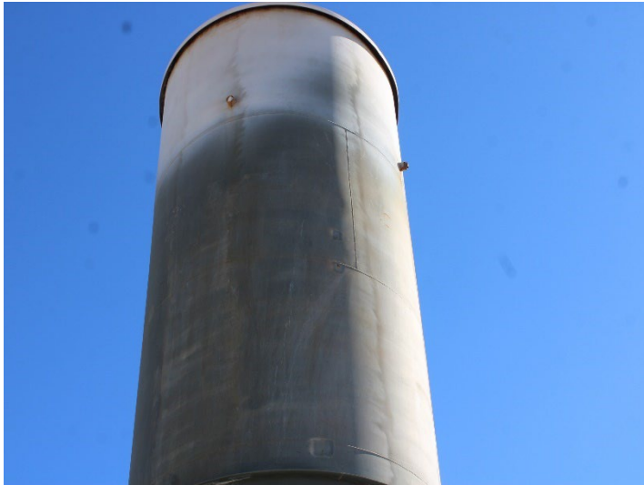
Photo 265: Flares 9, 10, 11 and Gas-to-Energy Facility: November 6, 2025
