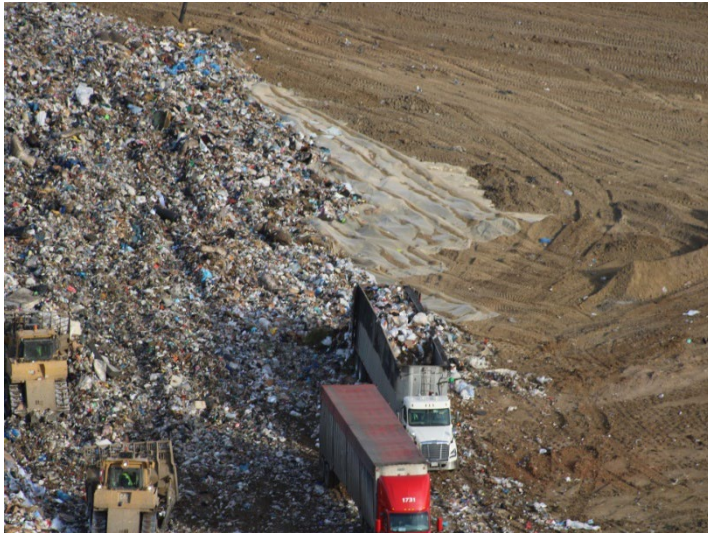
Photo 173: Working Area, CC-4 Part 4/5, CC-5A: December 18, 2025
