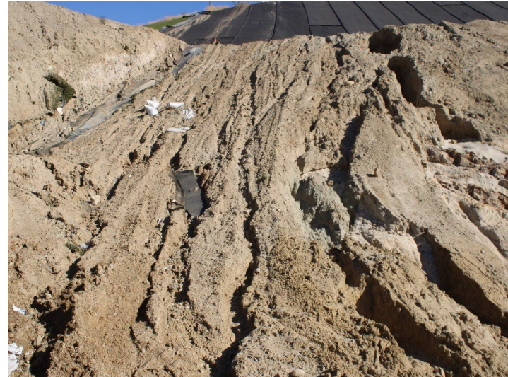
Photo 154: Working Area, CC-4 Part 4/5, CC-5A: November 6, 2025
