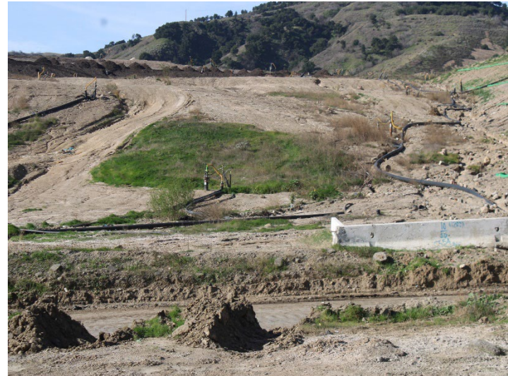
Photo 590: General Site: December 18, 2025
