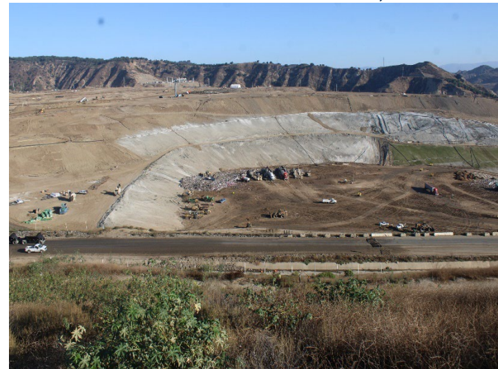
Photo 468: General Site: October 8, 2025
