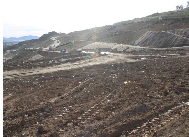
Photo 582: General Site: December 18, 2025
