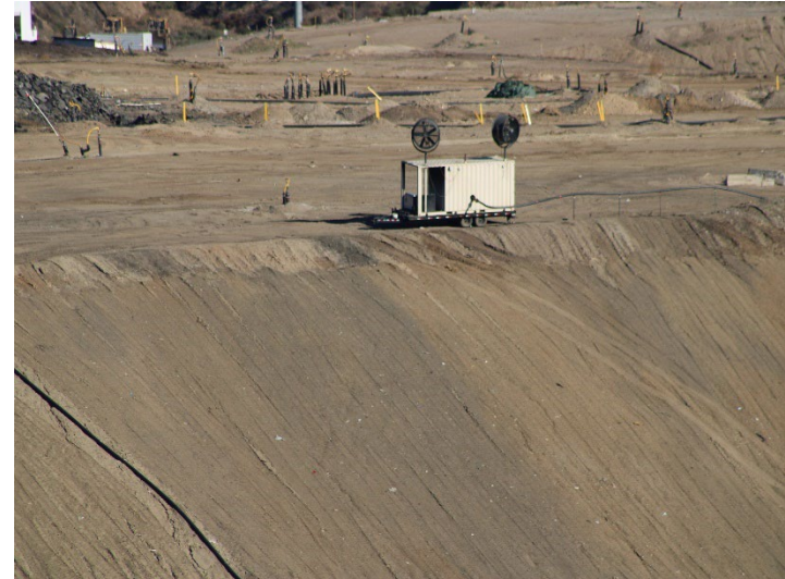
Photo 44: Working Area, CC-4 Part 3: November 6, 2025
