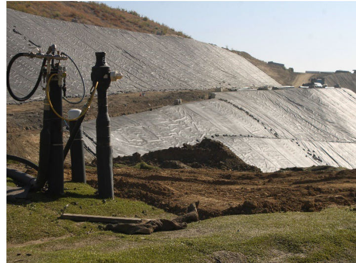
Photo 102: Working Area, CC-4 Part 4/5, CC-5A: October 8, 2025
