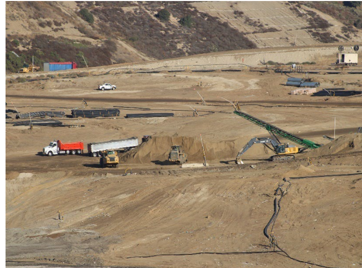
Photo 18: Working Area, CC4 Part 1/2: October 8, 2025
