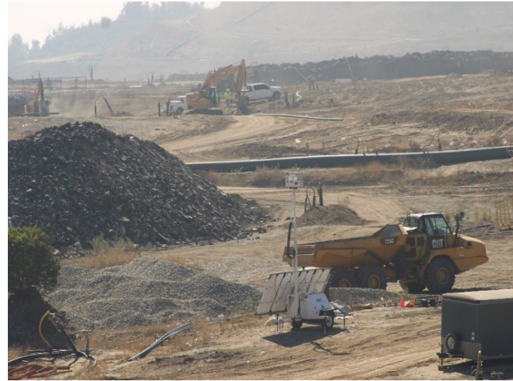
Photo 506: General Site: October 8, 2025
