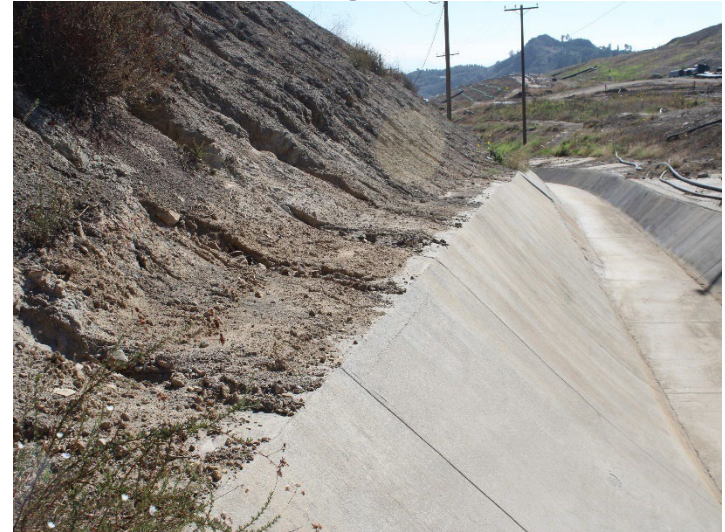
Photo 360: Eastside Drainage Channel: November 6, 2025
