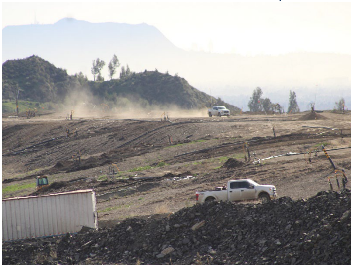
Photo 607: General Site: December 18, 2025
