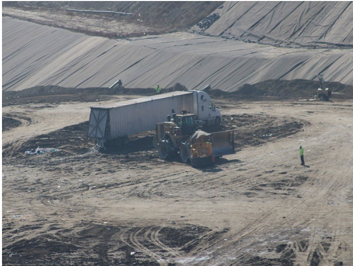
Photo 117: Working Area, CC-4 Part 4/5, CC-5A: October 8, 2025
