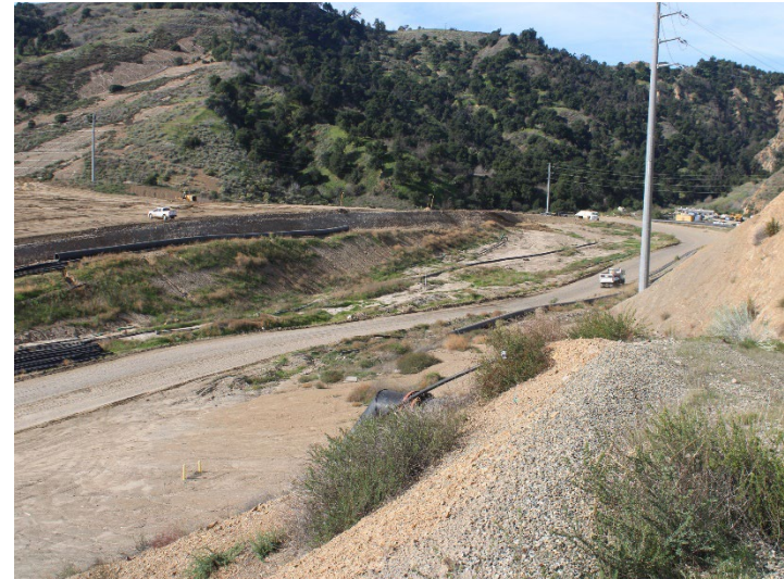
Photo 598: General Site: December 18, 2025
