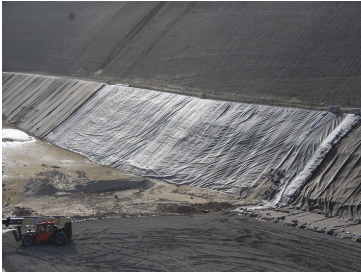
Photo 201: Working Area, CC-4 Part 4/5, CC-5A: December 18, 2025
