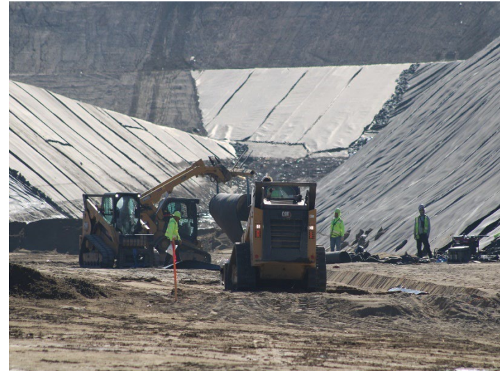
Photo 158: Working Area, CC-4 Part 4/5, CC-5A: November 6, 2025
