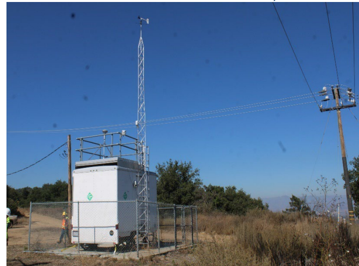
Photo 512: General Site: October 8, 2025
