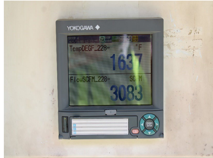
Photo 518: General Site: October 8, 2025
