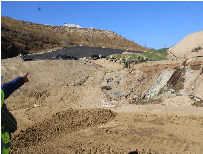
Photo 75: Working Area, CC-4 Part 4/5, CC-5A: October 8, 2025
