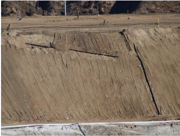
Photo 45: Working Area, CC-4 Part 3: November 6, 2025
