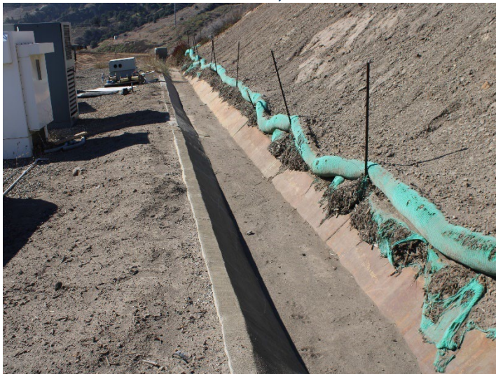
Photo 271: Flares 9, 10, 11 and Gas-to-Energy Facility: November 6, 2025
