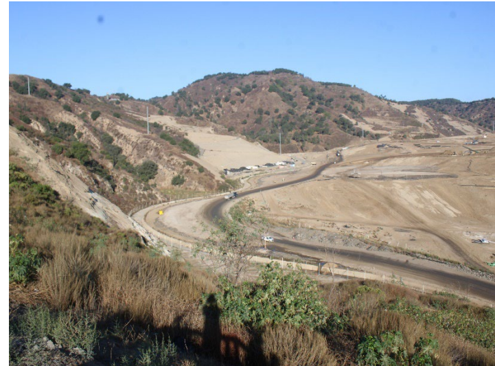
Photo 466: General Site: October 8, 2025
