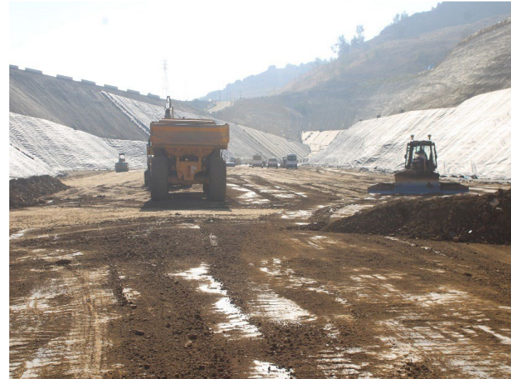
Photo 86: Working Area, CC-4 Part 4/5, CC-5A: October 8, 2025
