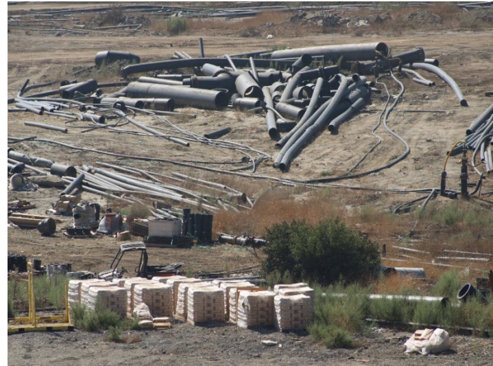
Photo 508: General Site: October 8, 2025
