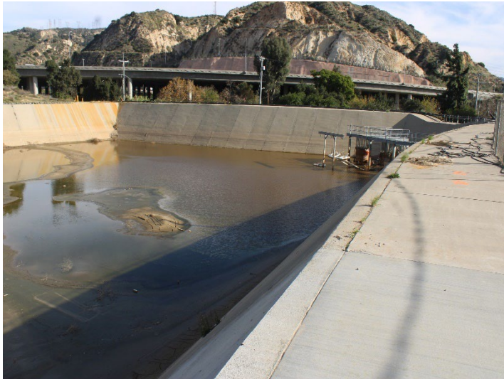
Photo 421: Terminal Basin: December 18, 2025
