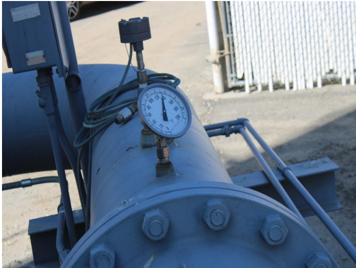
Photo 517: General Site: October 8, 2025
