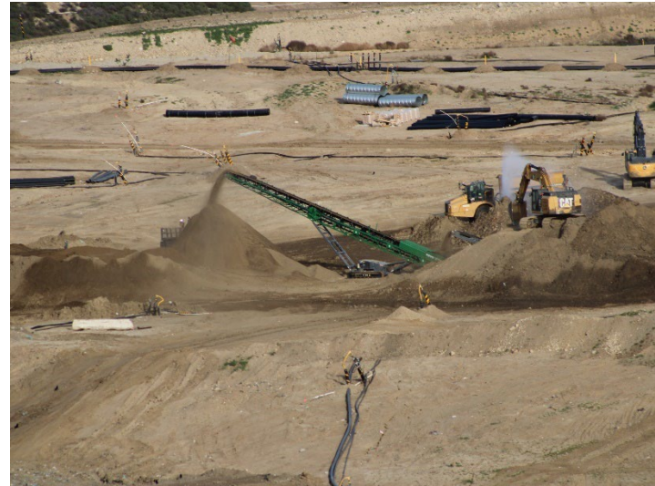
Photo 26: Working Area, CC4 Part 1/2: December 18, 2025
