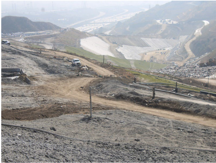
Photo 481: General Site: October 8, 2025
