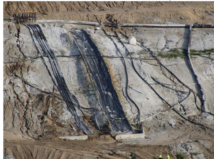
Photo 572: General Site: December 18, 2025
