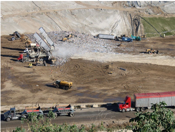
Photo 131: Working Area, CC-4 Part 4/5, CC-5A: November 6, 2025
