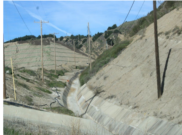
Photo 370: Eastside Drainage Channel: December 18, 2025
