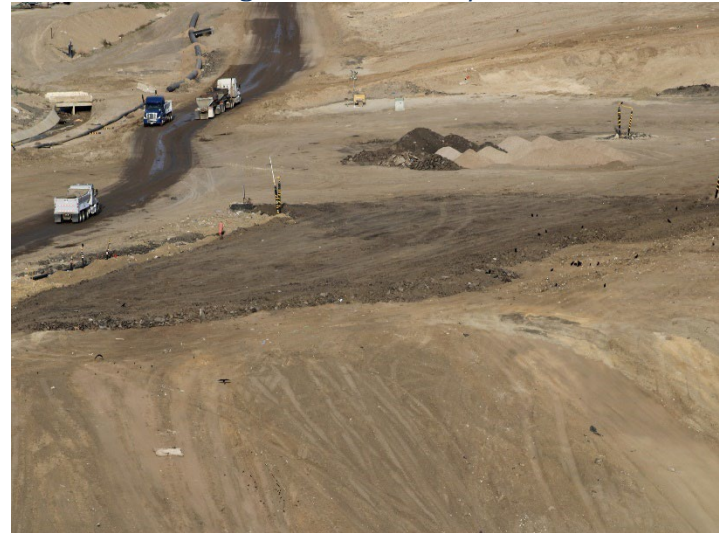
Photo 24: Working Area, CC4 Part 1/2: December 18, 2025
