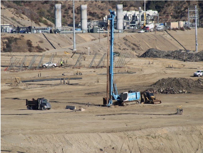
Photo 43: Working Area, CC-4 Part 3: November 6, 2025
