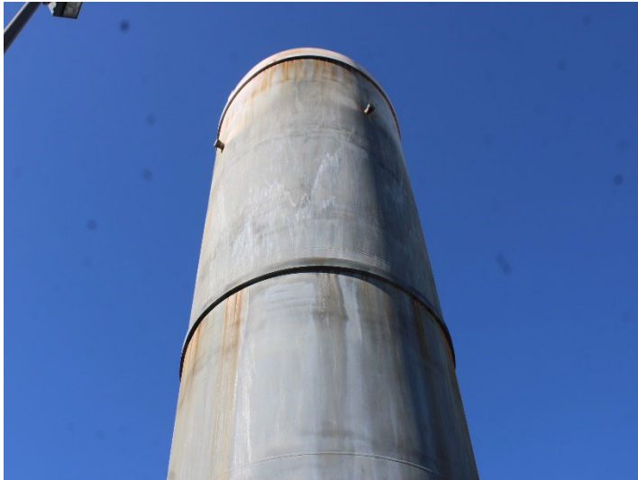
Photo 553: General Site: November 6, 2025
