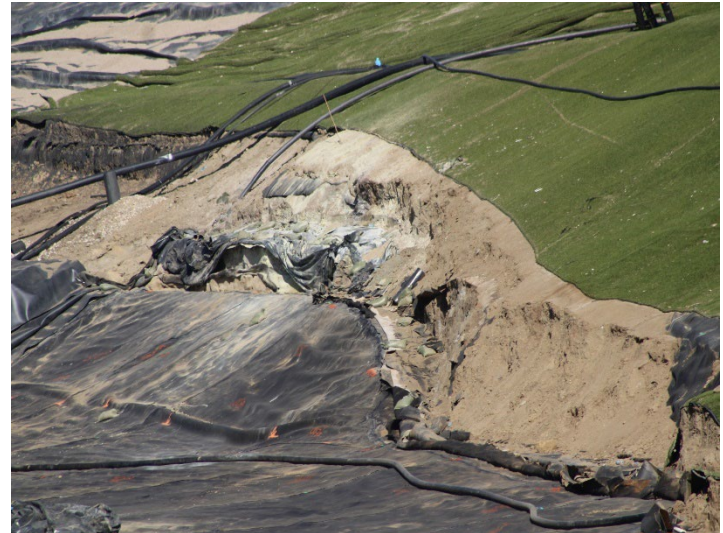
Photo 112: Working Area, CC-4 Part 4/5, CC-5A: October 8, 2025
