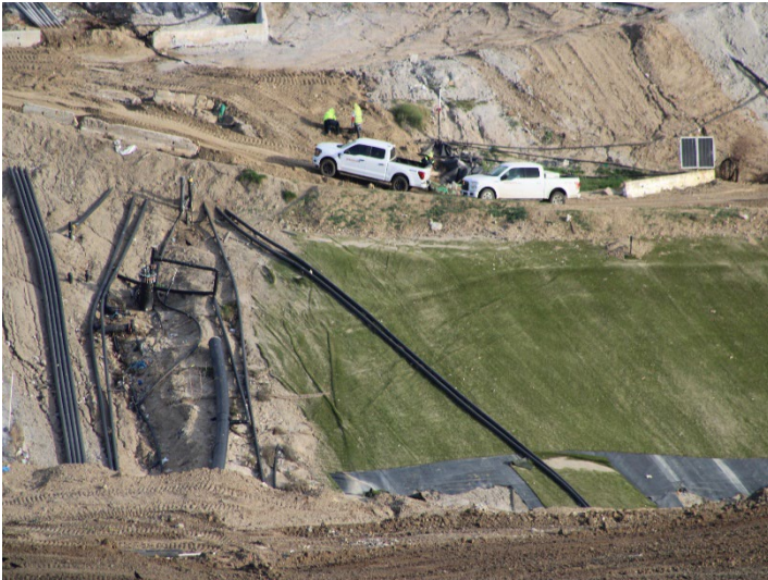
Photo 573: General Site: December 18, 2025
