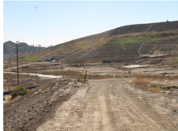
Photo 546: General Site: November 6, 2025
