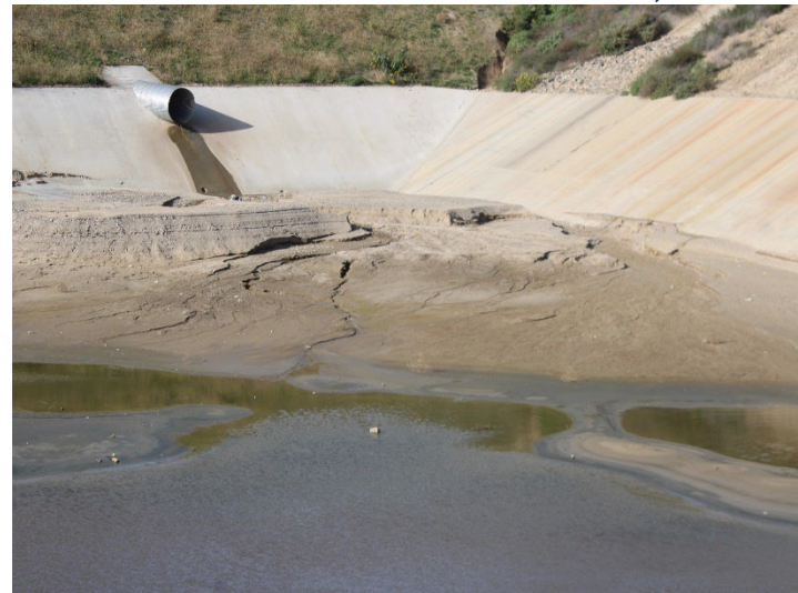
Photo 428: Terminal Basin: December 18, 2025
