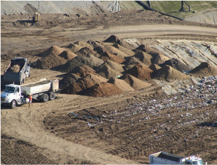
Photo 33: Working Area, CC-4 Part 3: October 8, 2025
