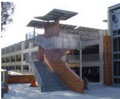
Solar panels on top of parking structure
