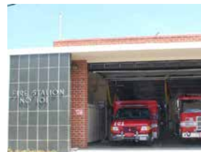
Fire Station 101 on W. 25th Street
