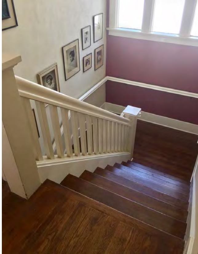
Staircase, viewed from second floor landing, looking down and toward north
