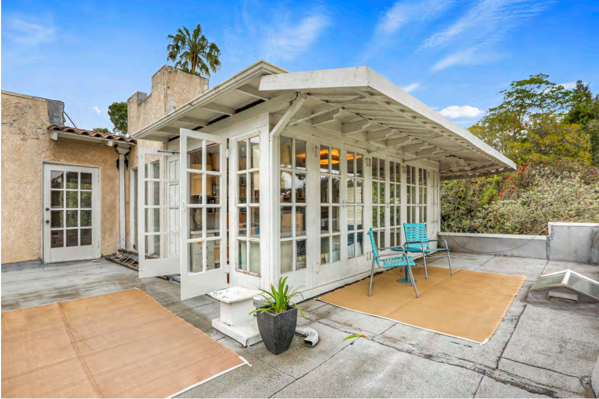
Sunroom, viewed from northwest toward southeast.
