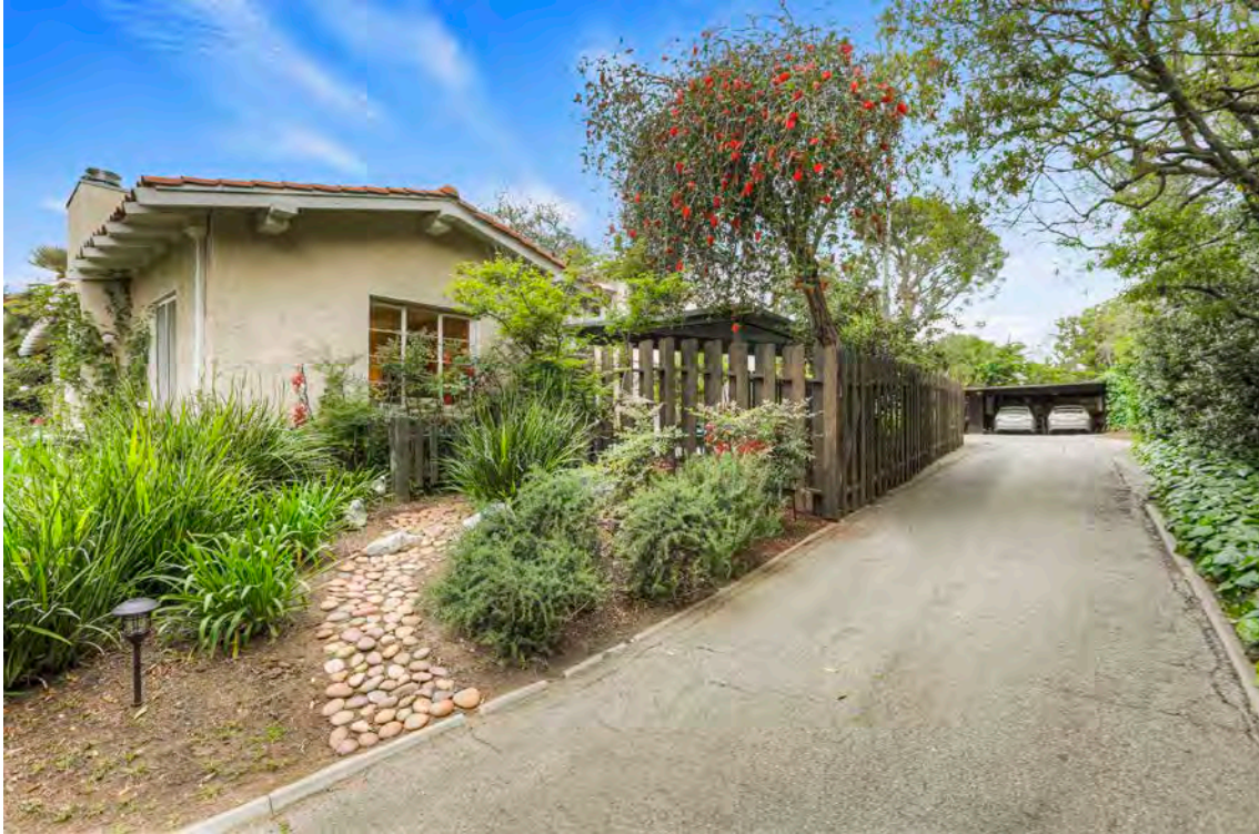
West wing of house/south elevation viewed from driveway looking northeast
