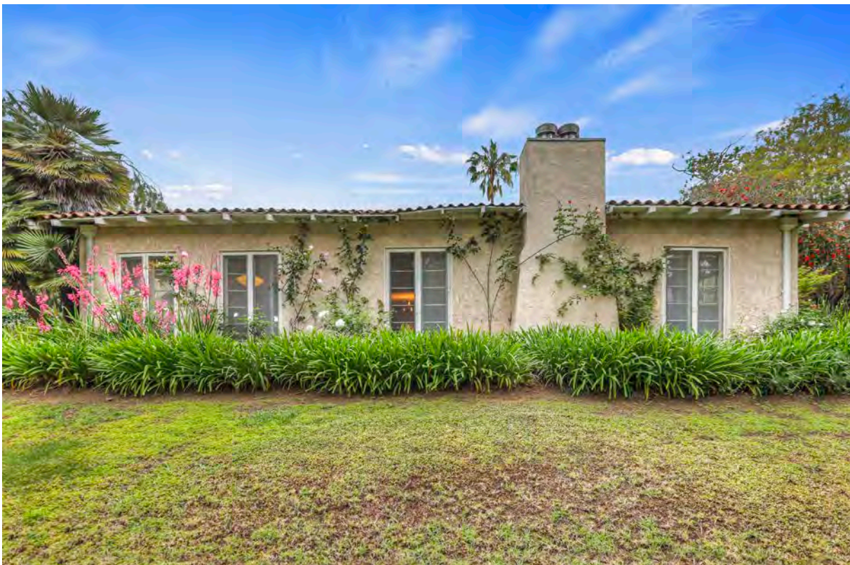
West wing/west-facing elevation – French doors to living room to right, dining room to left
