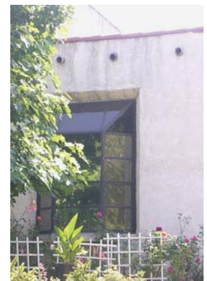
Despite their utility, garden-box windows such as this did not exist during this home's Period of Significance.
