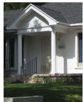
Metal security gates obscure a house's door.
