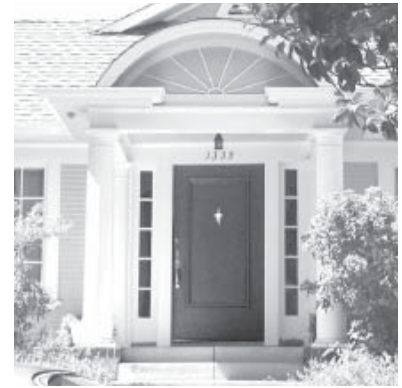
This simple door with a single panel, original hardware and side-lights is appropriate for a Colonial Revival house.
