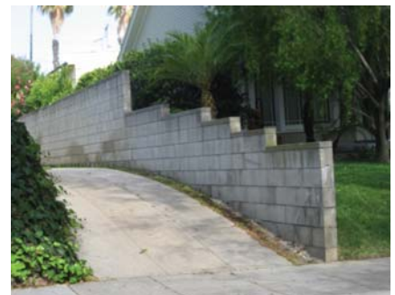
Concrete block walls can appear massive and unsightly.
