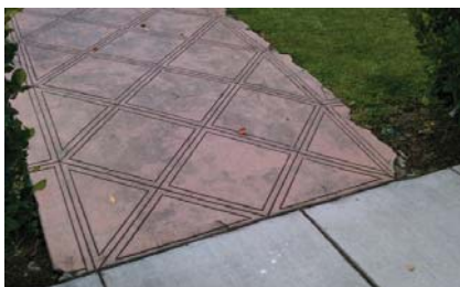
Scored concrete may be successfully used in some instances in lieu of tile or pavers.
