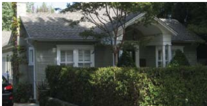
This Colonial Revival house features a gabled roof, with a hipped cross gable, and is finished with simple asphalt shingles.
