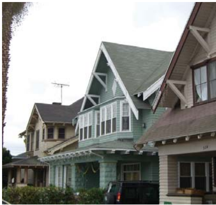
This street presents a consistent roof pattern that should be replicated on new construction.
