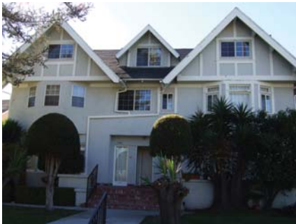
The modern windows that have been added to this home are poorly scaled and dramatically alter the home's original appearance.
