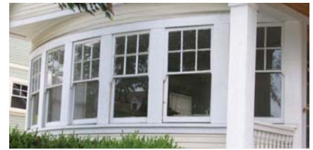
A curved bay of double-hung windows is shown.
