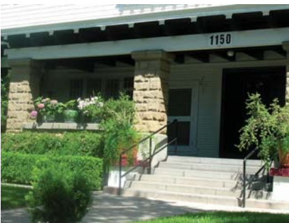
The sandstone porch columns are left to display their natural finish quality.
