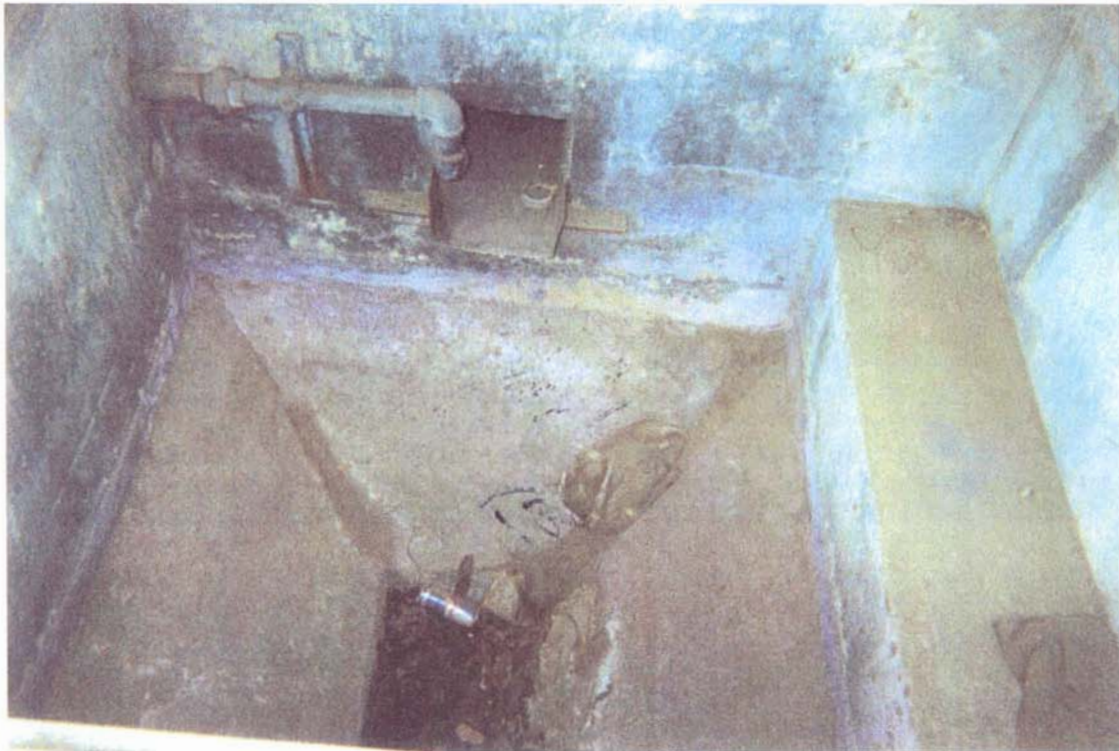
16. A view of the inside of the pit. A pipe appears to be plumbed to the pit. The bottom of the pit appears to be soil. Purple staining is visible in the pit.
