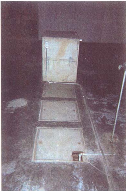
17. A view of the 2,000 gallon clarifier located on the eastern side of the inside of the Site building. The clarifier appears to be 3-stages. .
