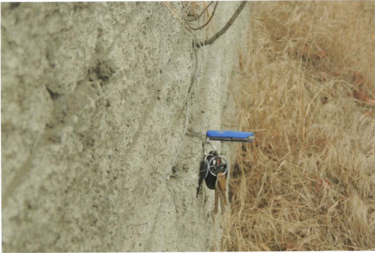
Photo 5: Blocks off alignment on wall along San Fernando Road
