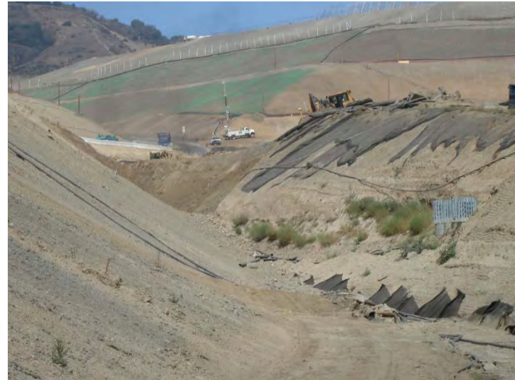
Photo 214: Construction Low Point Drain to Terminal Basin: August 26, 2015
