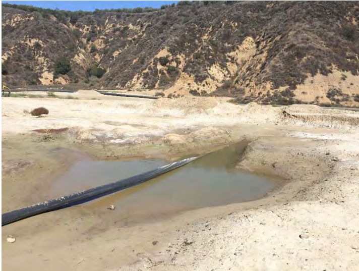
Photo 113: County Top Deck Low Point Ponding: September 23, 2015
