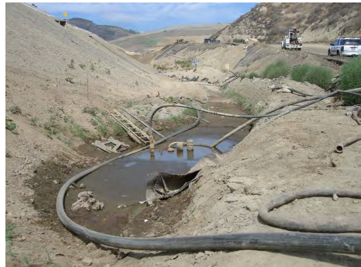
Photo 216: Construction Low Point Drain to Terminal Basin: August 26, 2015
