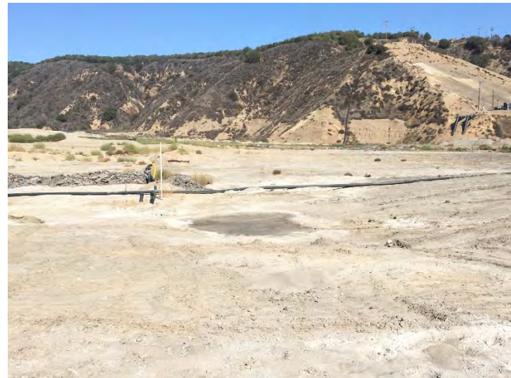
Photo 108: County Top Deck Low Point Ponding: September 23, 2015
