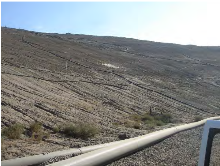
Photo 383: City Slope with no Erosion Control: August 26, 2015
