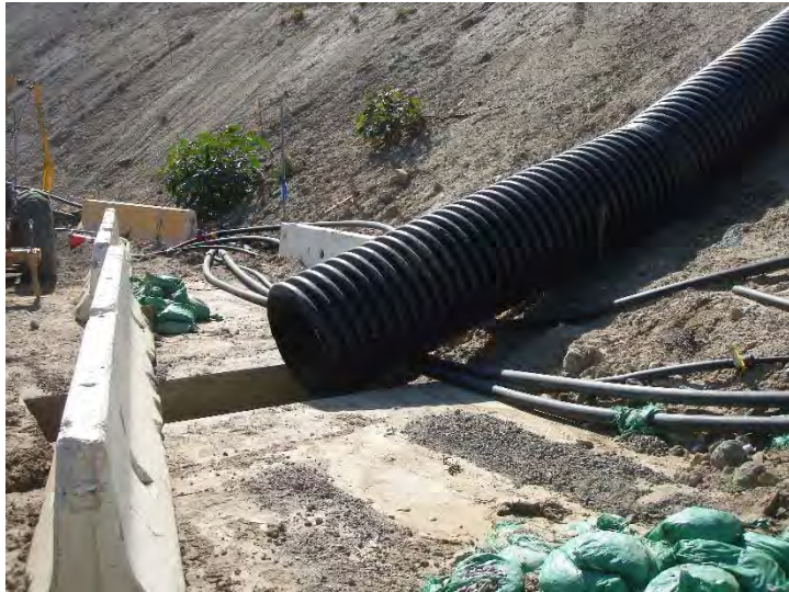
Photo 221: Water Inlet to Terminal Basin: September 23, 2015
