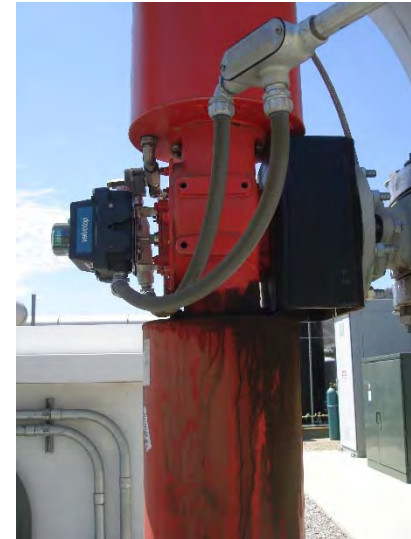
Photo 386: Hydraulic Oil Leak on Gas to Plant Shutoff Valve: August 26, 2015
