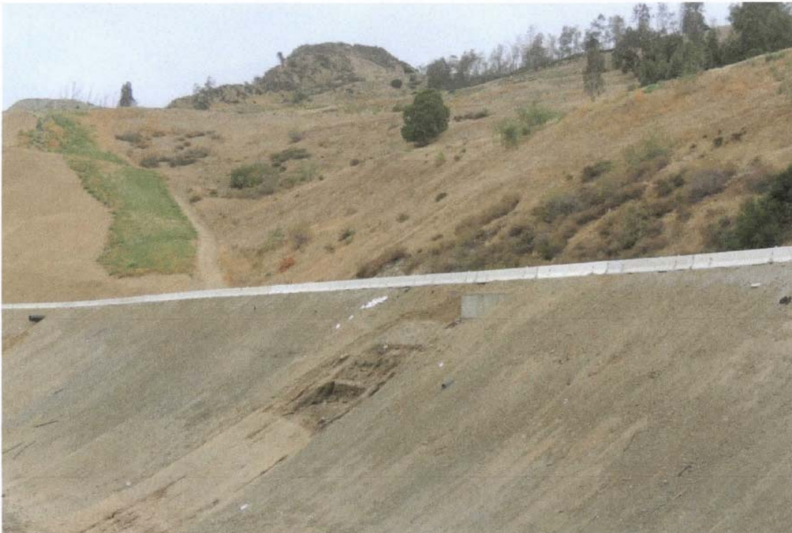
Photo 2: Damage under box culvert on new access road
