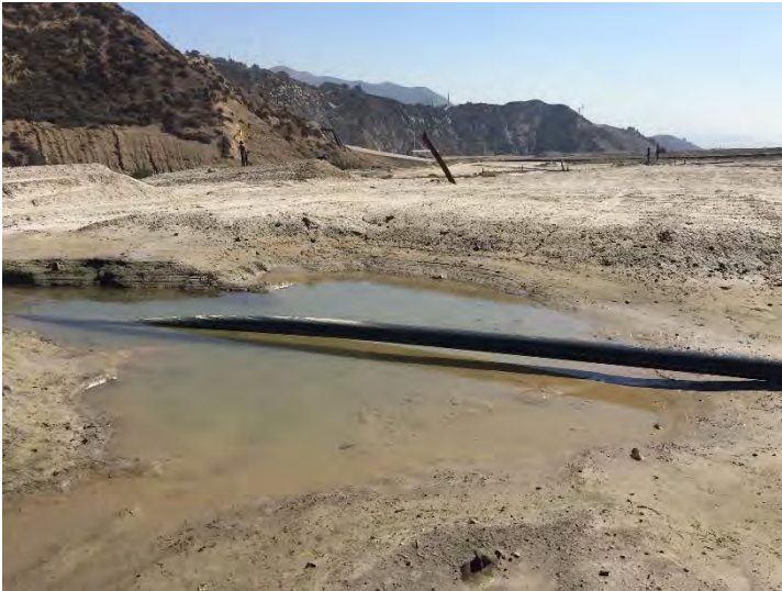
Photo 111: County Top Deck Low Point Ponding: September 23, 2015
