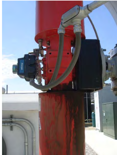
Photo 123: Photo 65 Hydraulic Oil Leak on Gas to Plant Shutoff Valve: August 26, 2015
