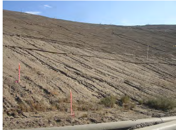
Photo 382: City Slope with no Erosion Control: August 26, 2015
