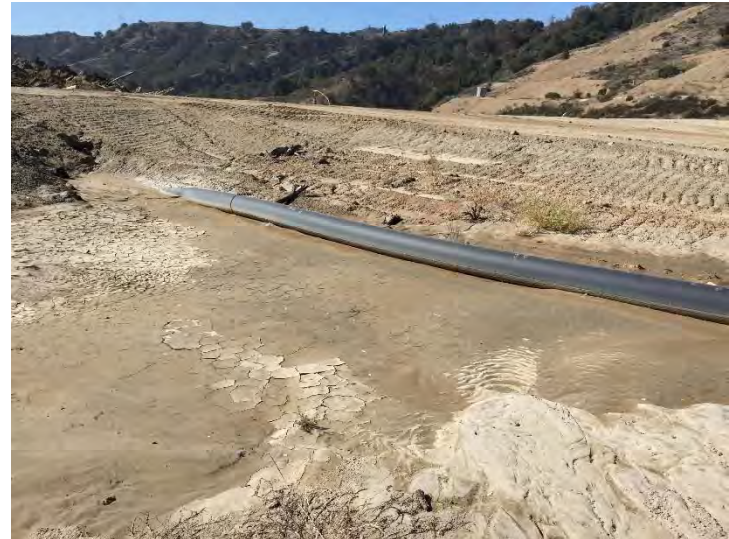
Photo 106: County Top Deck Low Point Ponding: September 23, 2015
