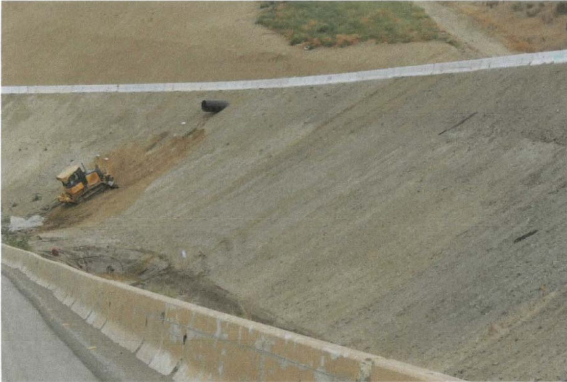
Photo 1: Damage repair at drainage pipe under new access road
