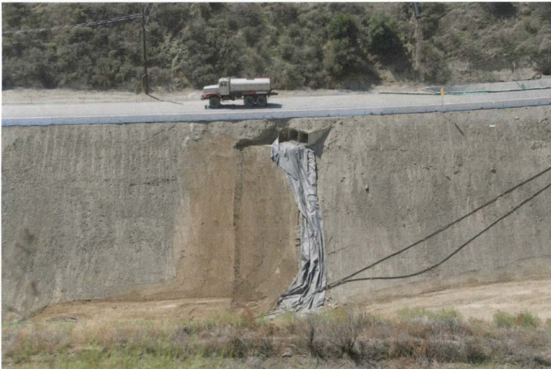
Photo 4: Geomembrane at Box Culver on Access Road
