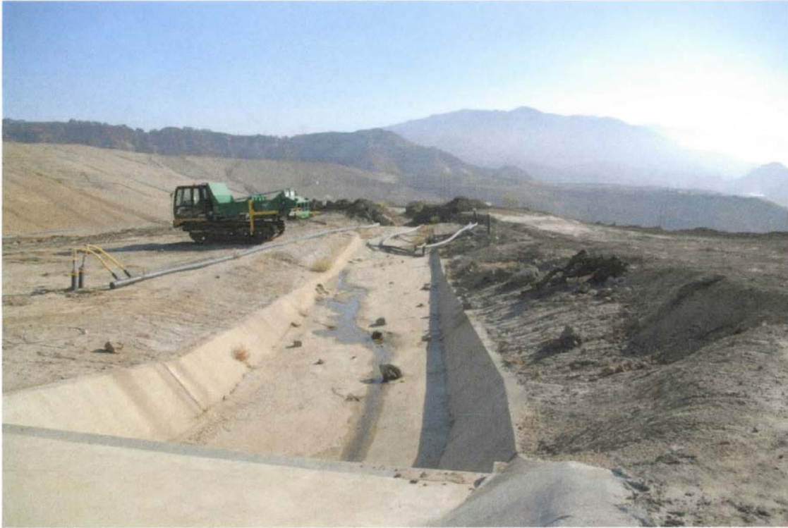
Figure 3: Channel out of Basin A Partially Blocked
