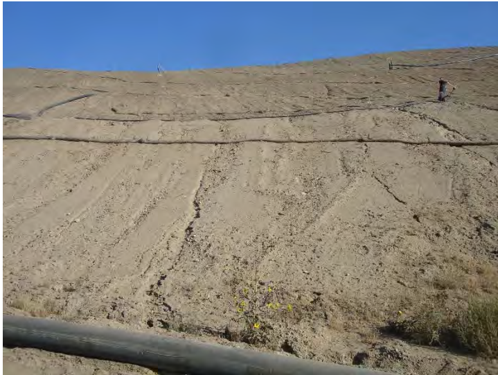
Photo 381: City Slope with no Erosion Control: August 26, 2015
