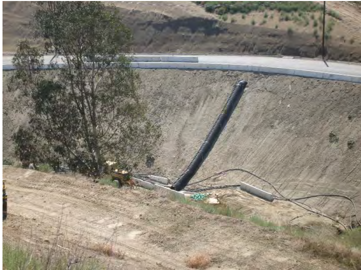
Photo 219: Access Road Drainage to Terminal Basin: September 23, 2015
