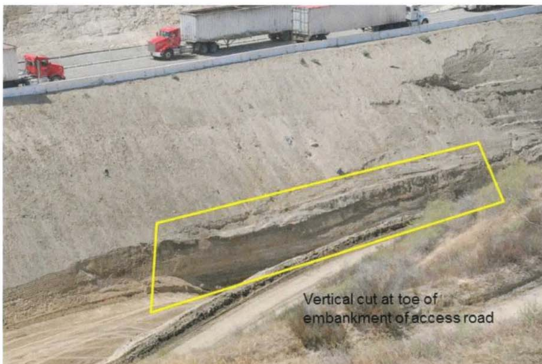
Photo 1: Vertical Cut at Toe of Access Road Embankment
