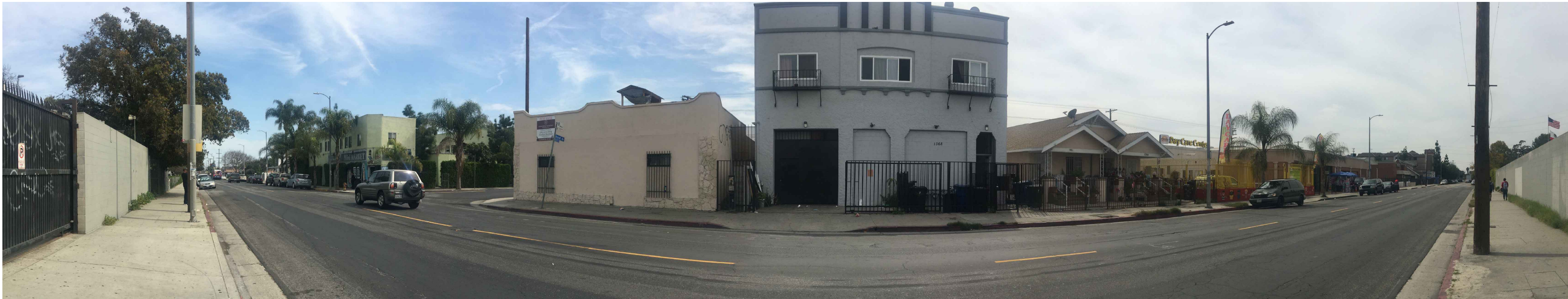
41 ST STREET (VIEW LOOKING SOUTH)
