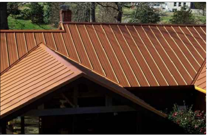
COPPER COLORED STANDING SEAM ROOF
