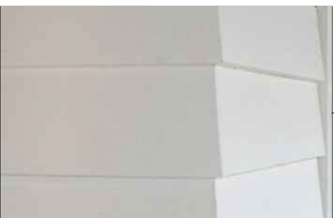
SHINGLED COMPOSITE SIDING PAINTED WHITE
