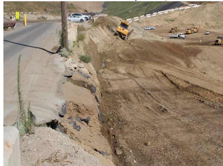
Photo 608: General Site: June 11, 2026
