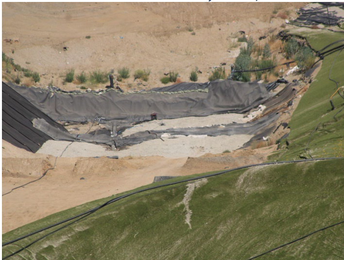
Photo 647: General Site: June 11, 2026
