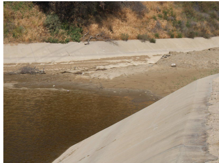
Photo 8: Basin A: April 9, 2026
