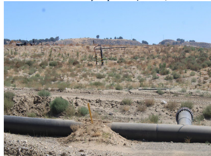
Photo 260: County Top Deck: June 11, 2026
