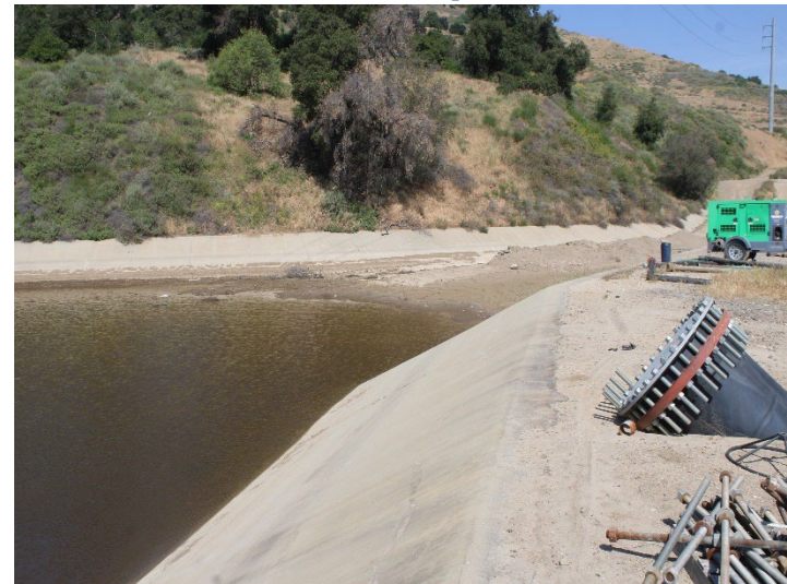
Photo 4: Basin A: April 9, 2026
