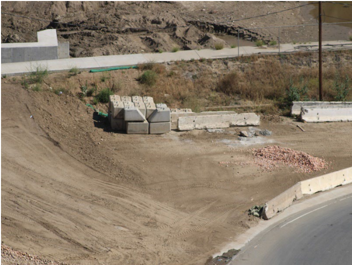
Photo 497: General Site: May 21, 2026
