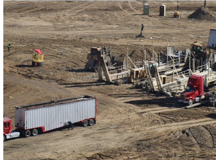
Photo 116: Working Area, CC-4 Part 4/5, CC-5A: May 21, 2026
