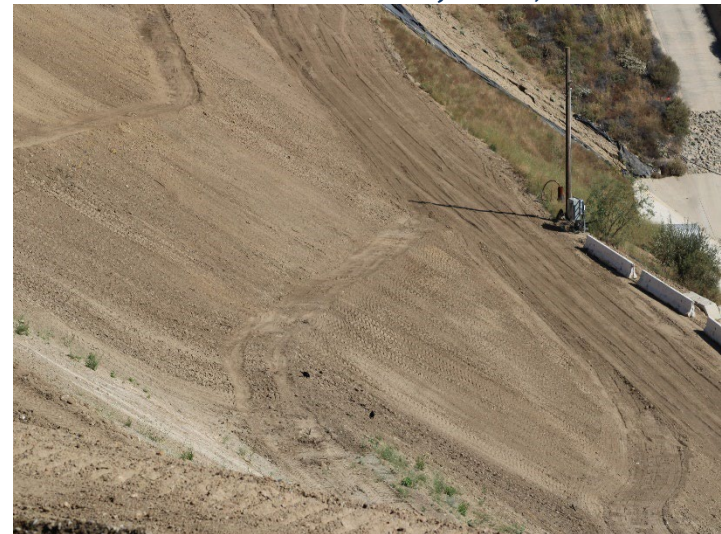
Photo 612: General Site: June 11, 2026
