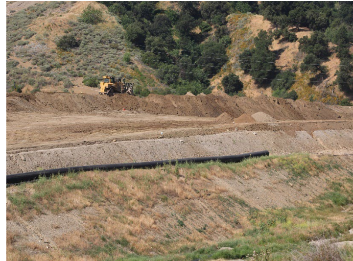
Photo 250: County Top Deck: April 9, 2026
