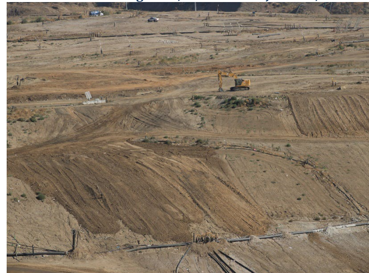
Photo 60: Working Area, CC-4 Part 3: June 11, 2026
