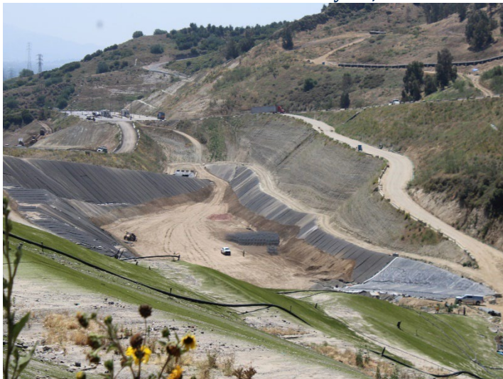
Photo 575: General Site: May 21, 2026
