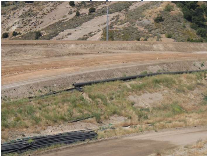
Photo 255: County Top Deck: May 21, 2026
