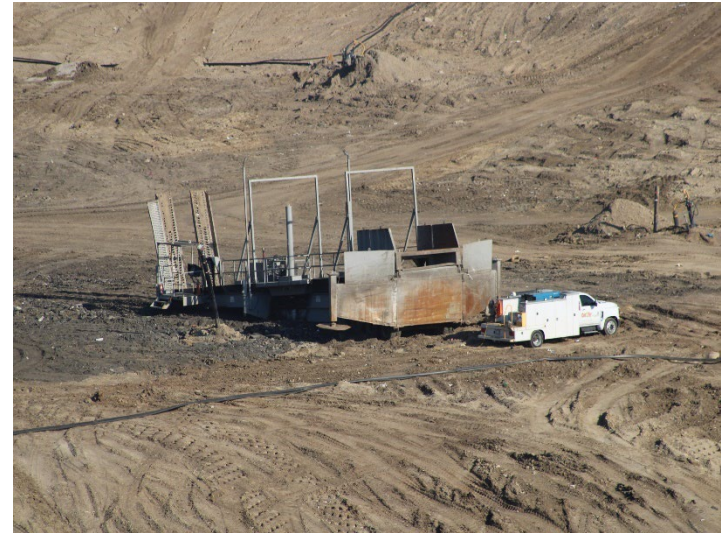
Photo 82: Working Area, CC-4 Part 4/5, CC-5A: April 9, 2026
