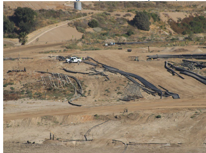
Photo 64: Working Area, CC-4 Part 3: June 11, 2026
