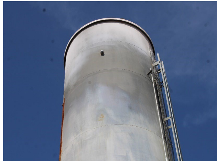
Photo 216: Flares 9, 10, 11 and Gas-to-Energy Facility: April 9, 2026
