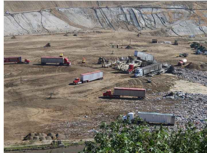
Photo 94: Working Area, CC-4 Part 4/5, CC-5A: May 21, 2026
