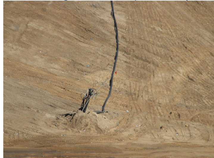
Photo 104: Working Area, CC-4 Part 4/5, CC-5A: May 21, 2026
