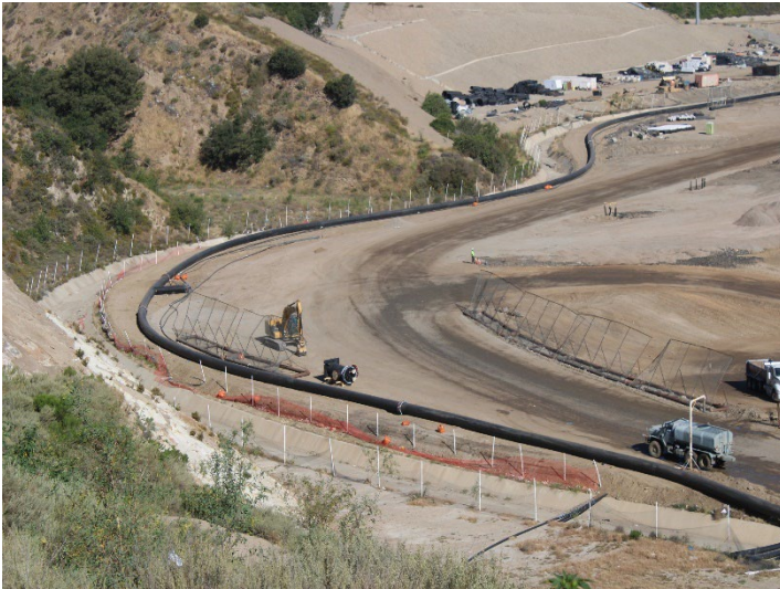
Photo 89: Working Area, CC-4 Part 4/5, CC-5A: May 21, 2026
