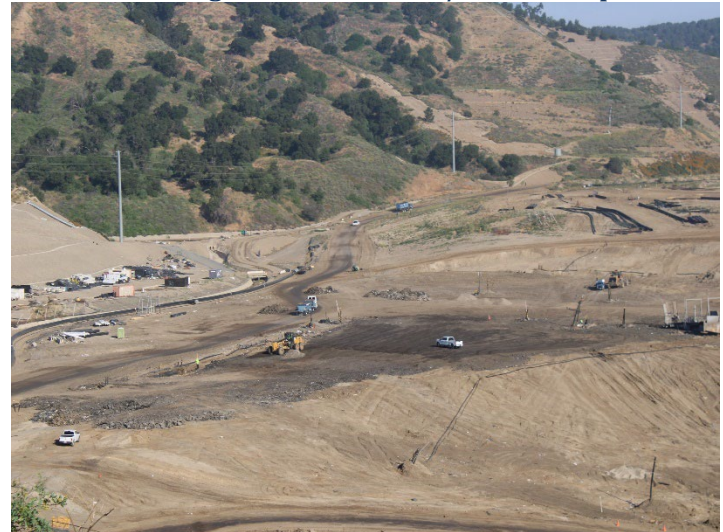
Photo 72: Working Area, CC-4 Part 4/5, CC-5A: April 9, 2026
