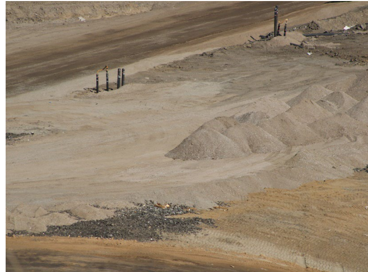
Photo 102: Working Area, CC-4 Part 4/5, CC-5A: May 21, 2026
