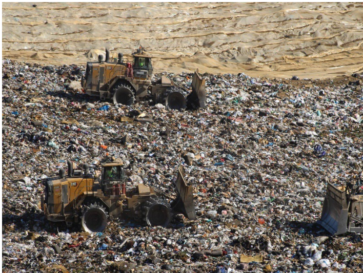
Photo 135: Working Area, CC-4 Part 4/5, CC-5A: June 11, 2026
