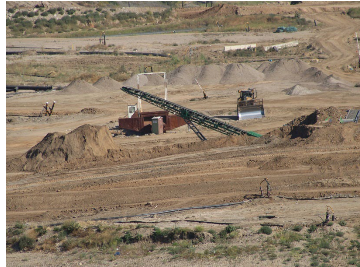
Photo 34: Working Area, CC4 Part 1/2: May 21, 2026
