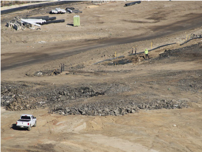
Photo 79: Working Area, CC-4 Part 4/5, CC-5A: April 9, 2026
