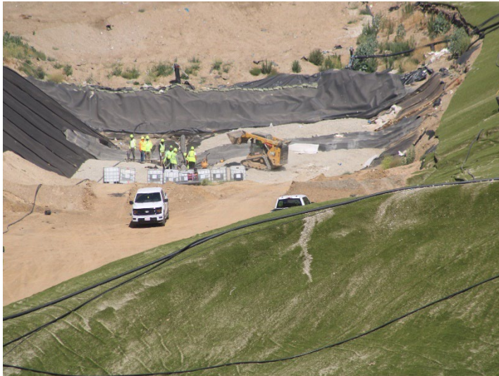
Photo 533: General Site: May 21, 2026
