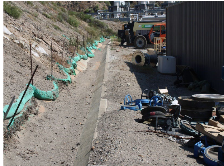
Photo 224: Flares 9, 10, 11 and Gas-to-Energy Facility: April 9, 2026
