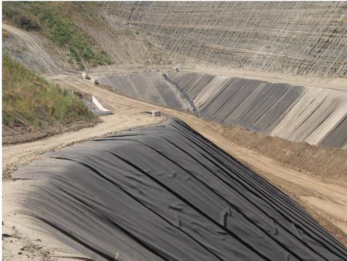
Photo 513: General Site: May 21, 2026
