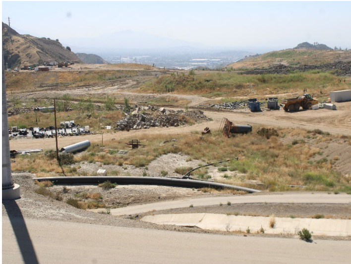
Photo 553: General Site: May 21, 2026
