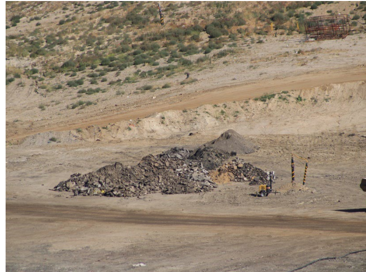
Photo 106: Working Area, CC-4 Part 4/5, CC-5A: May 21, 2026
