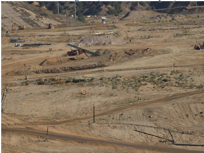
Photo 59: Working Area, CC-4 Part 3: June 11, 2026
