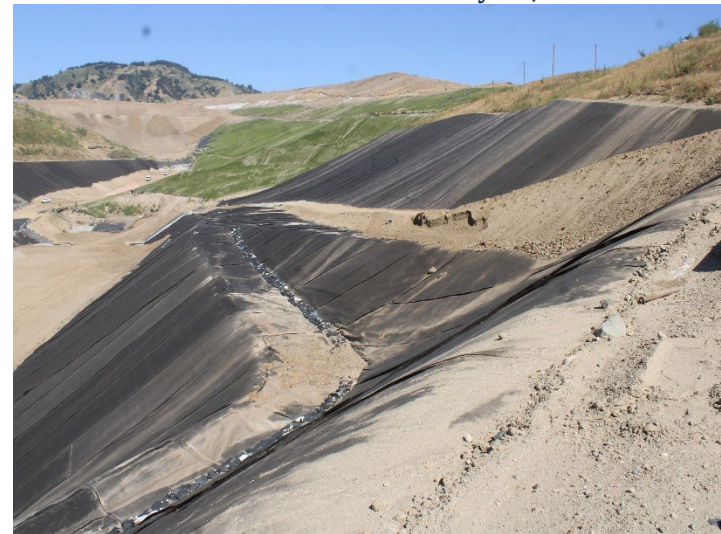
Photo 512: General Site: May 21, 2026
