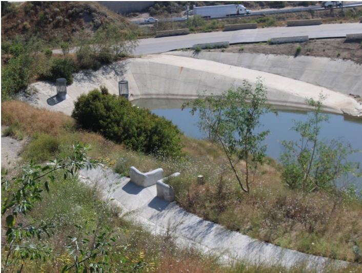
Photo 501: General Site: May 21, 2026
