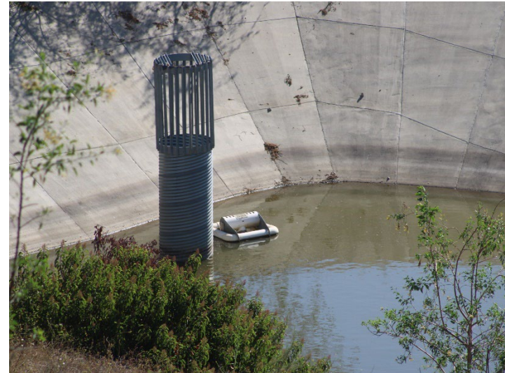
Photo 602: General Site: June 11, 2026
