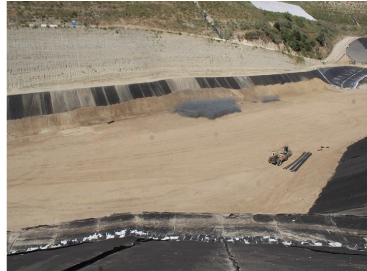
Photo 510: General Site: May 21, 2026
