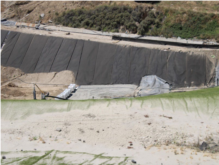
Photo 577: General Site: May 21, 2026
