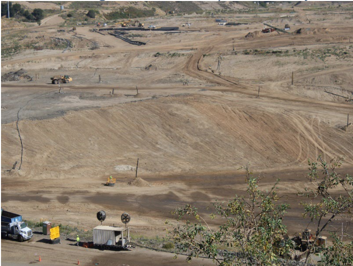
Photo 91: Working Area, CC-4 Part 4/5, CC-5A: May 21, 2026
