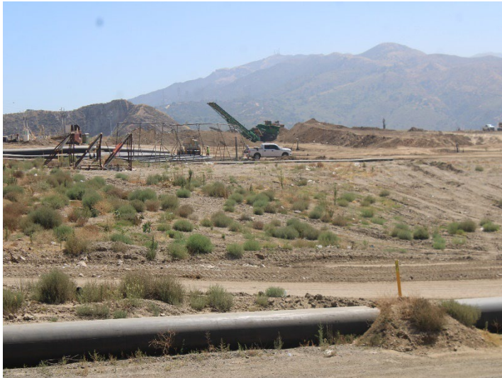
Photo 261: County Top Deck: June 11, 2026
