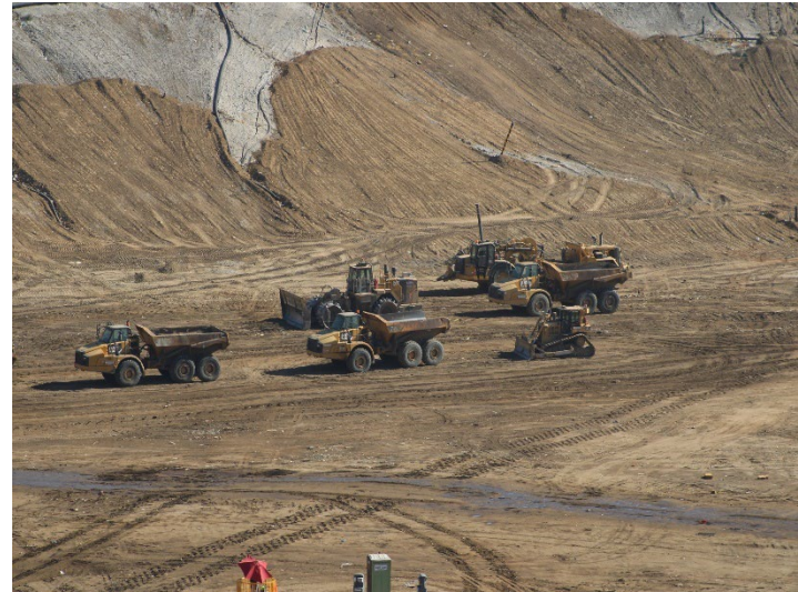
Photo 62: Working Area, CC-4 Part 3: June 11, 2026
