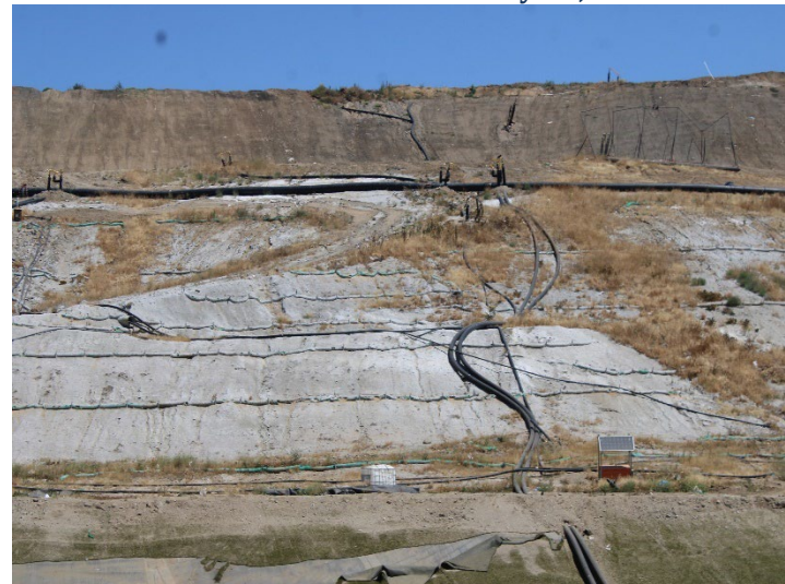
Photo 572: General Site: May 21, 2026
