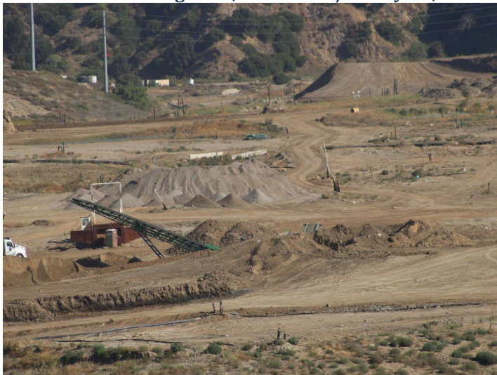
Photo 39: Working Area, CC4 Part 1/2: June 11, 2026
