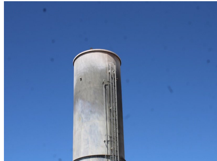
Photo 240: Flares 9, 10, 11 and Gas-to-Energy Facility: June 11, 2026
