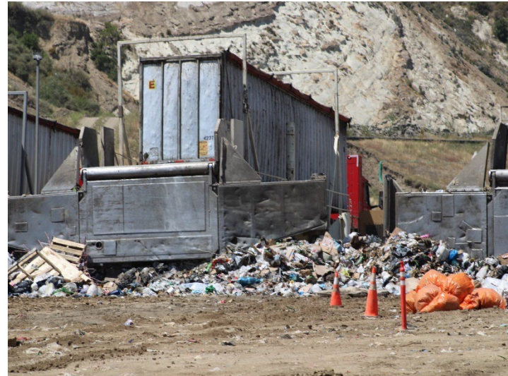
Photo 122: Working Area, CC-4 Part 4/5, CC-5A: May 21, 2026
