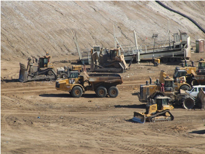
Photo 109: Working Area, CC-4 Part 4/5, CC-5A: May 21, 2026
