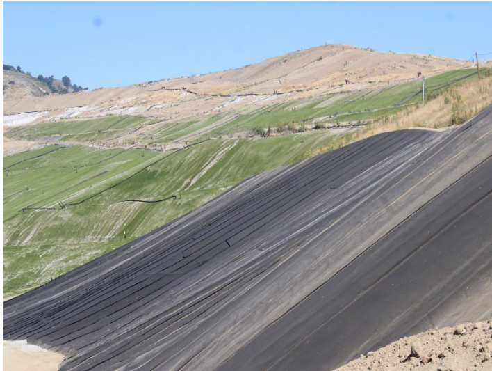
Photo 541: General Site: May 21, 2026
