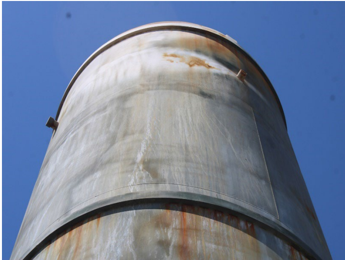
Photo 557: General Site: May 21, 2026
