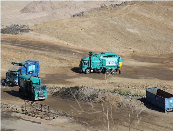
Photo 99: Working Area, CC-4 Part 4/5, CC-5A: May 21, 2026
