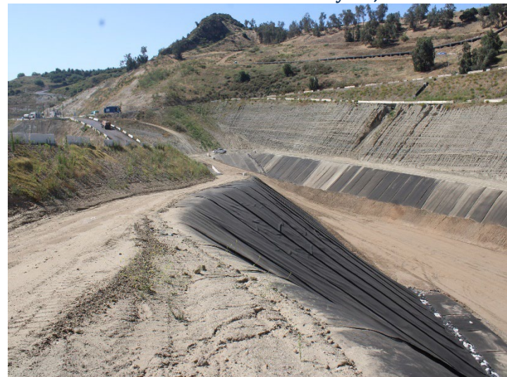
Photo 508: General Site: May 21, 2026
