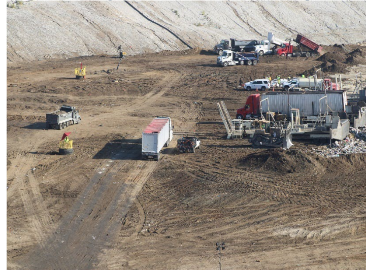
Photo 84: Working Area, CC-4 Part 4/5, CC-5A: April 9, 2026
