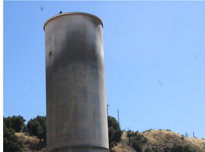
Photo 226: Flares 9, 10, 11 and Gas-to-Energy Facility: May 21, 2026
