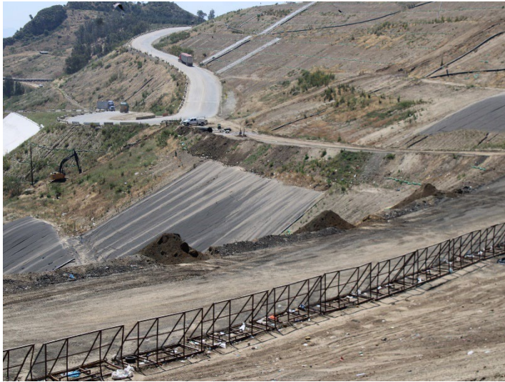
Photo 569: General Site: May 21, 2026
