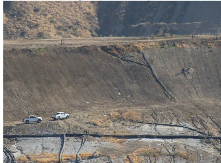
Photo 44: Working Area, CC4 Part 1/2: June 11, 2026
