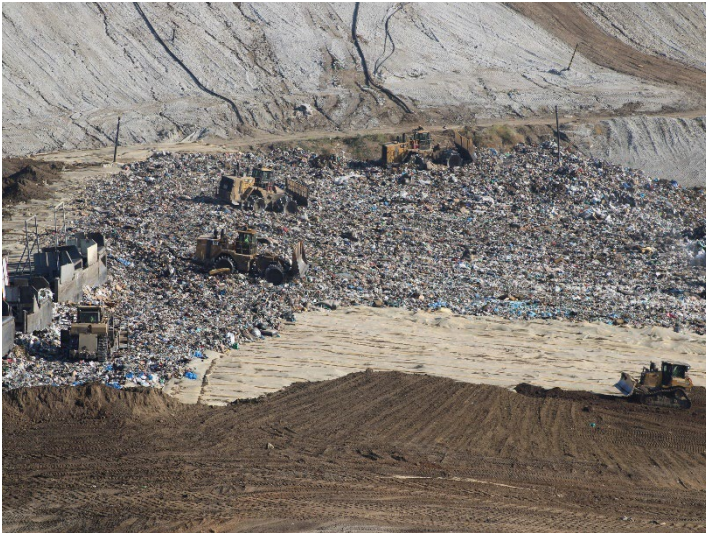
Photo 85: Working Area, CC-4 Part 4/5, CC-5A: April 9, 2026
