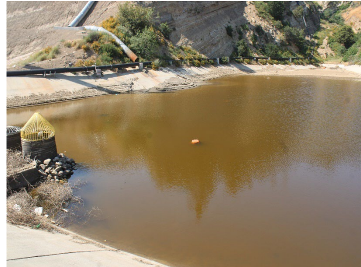
Photo 2: Basin A: April 9, 2026
