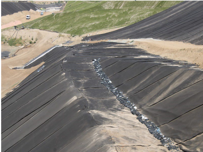
Photo 519: General Site: May 21, 2026
