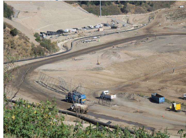
Photo 128: Working Area, CC-4 Part 4/5, CC-5A: June 11, 2026
