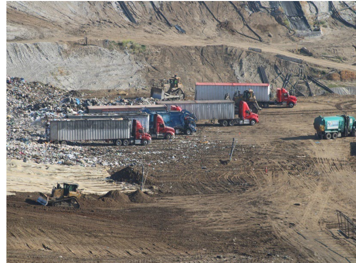
Photo 86: Working Area, CC-4 Part 4/5, CC-5A: April 9, 2026
