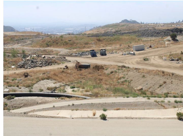
Photo 654: General Site: June 11, 2026
