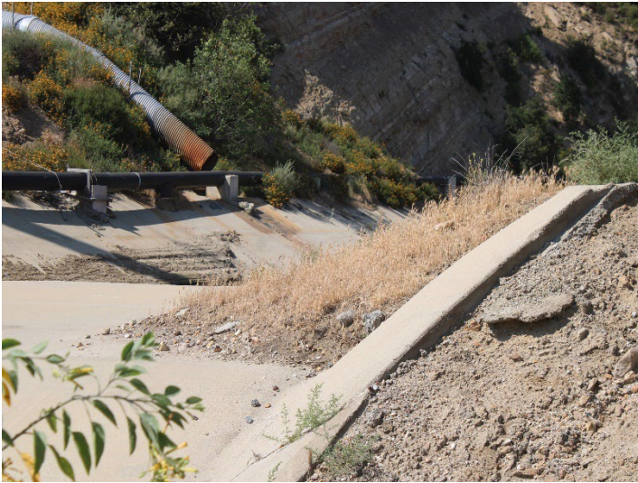
Photo 9: Basin A: April 9, 2026
