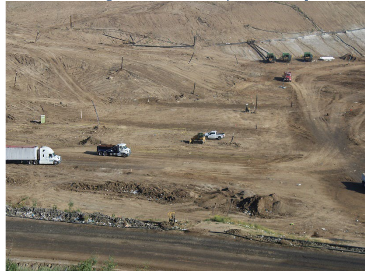
Photo 68: Working Area, CC-4 Part 4/5, CC-5A: April 9, 2026
