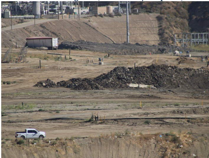
Photo 35: Working Area, CC4 Part 1/2: May 21, 2026
