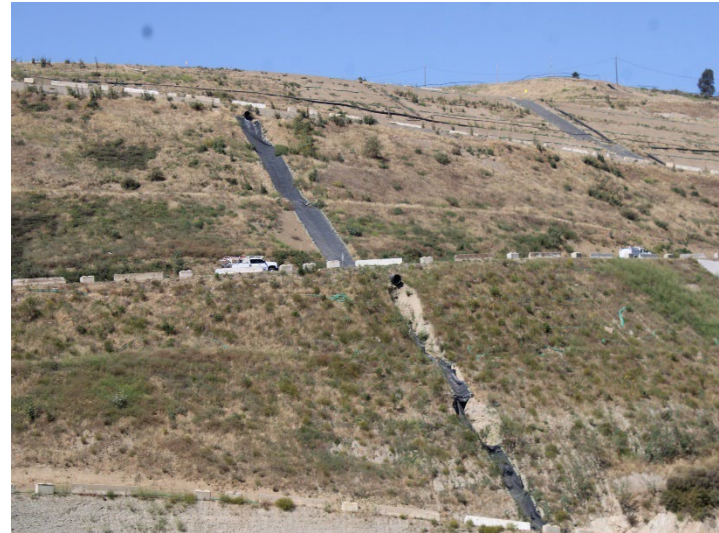
Photo 538: General Site: May 21, 2026
