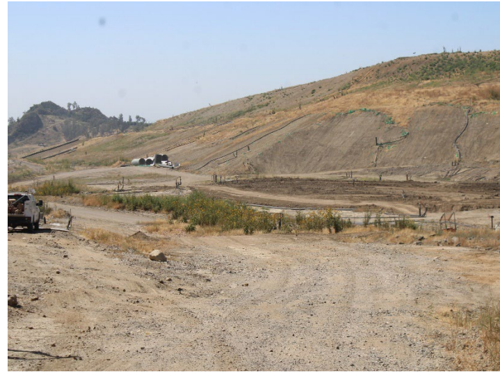
Photo 546: General Site: May 21, 2026
