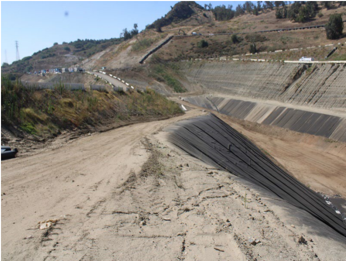
Photo 617: General Site: June 11, 2026
