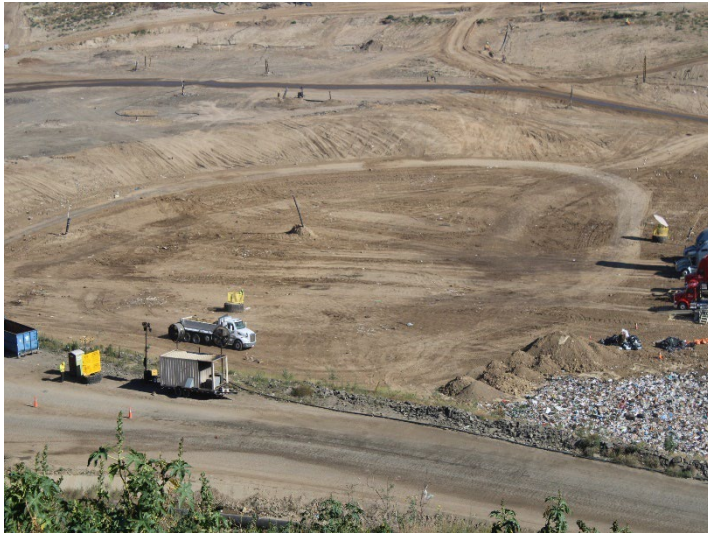
Photo 129: Working Area, CC-4 Part 4/5, CC-5A: June 11, 2026
