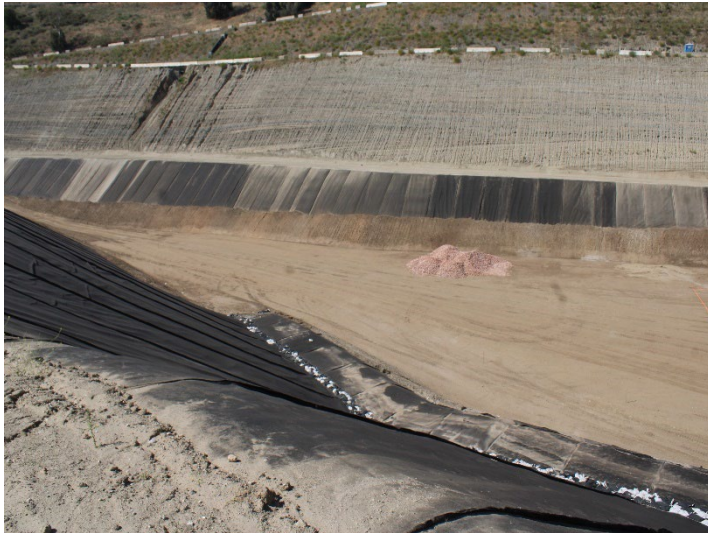
Photo 509: General Site: May 21, 2026
