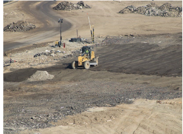
Photo 80: Working Area, CC-4 Part 4/5, CC-5A: April 9, 2026
