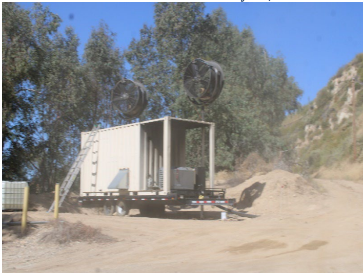
Photo 483: General Site: May 21, 2026
