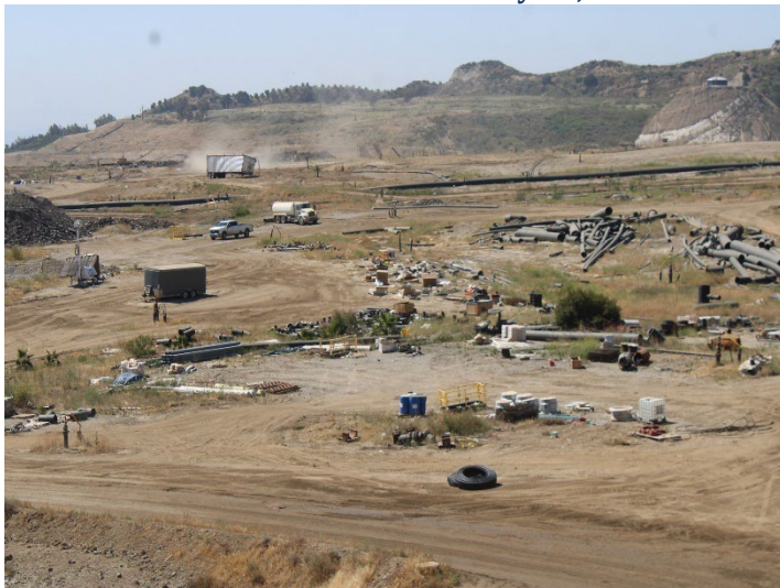
Photo 555: General Site: May 21, 2026
