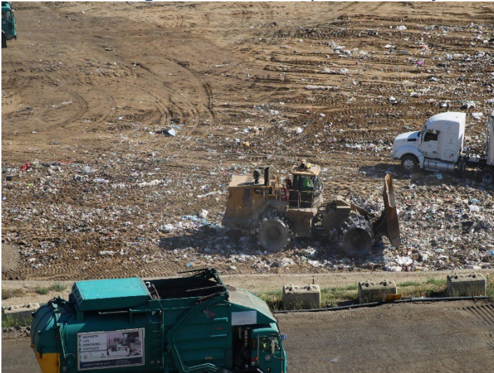
Photo 111: Working Area, CC-4 Part 4/5, CC-5A: May 21, 2026
