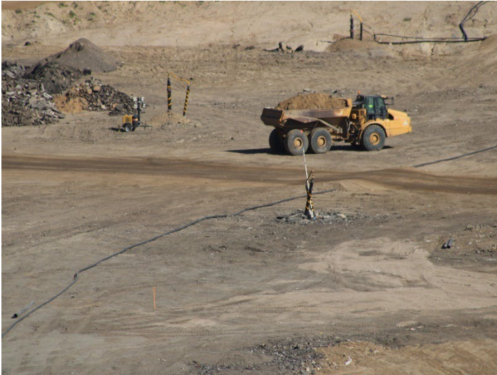
Photo 105: Working Area, CC-4 Part 4/5, CC-5A: May 21, 2026
