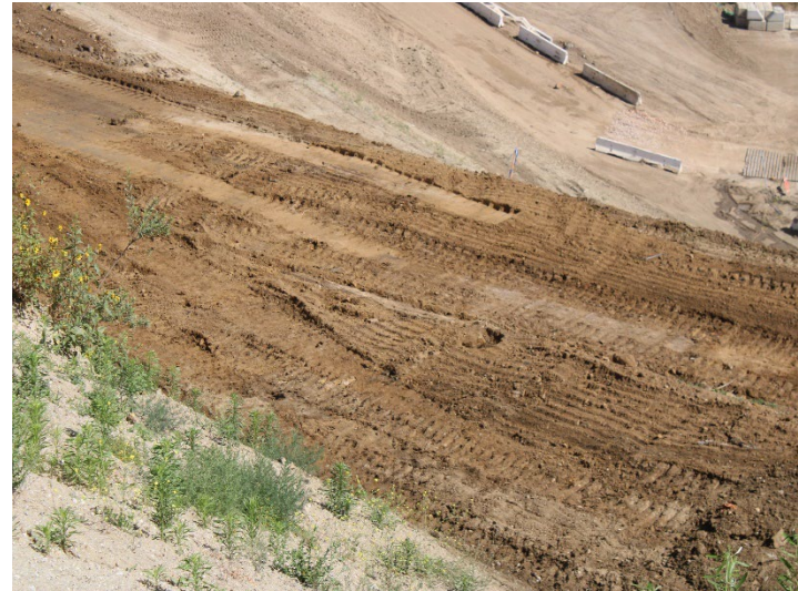
Photo 490: General Site: May 21, 2026
