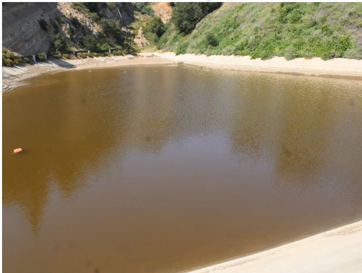
Photo 3: Basin A: April 9, 2026
