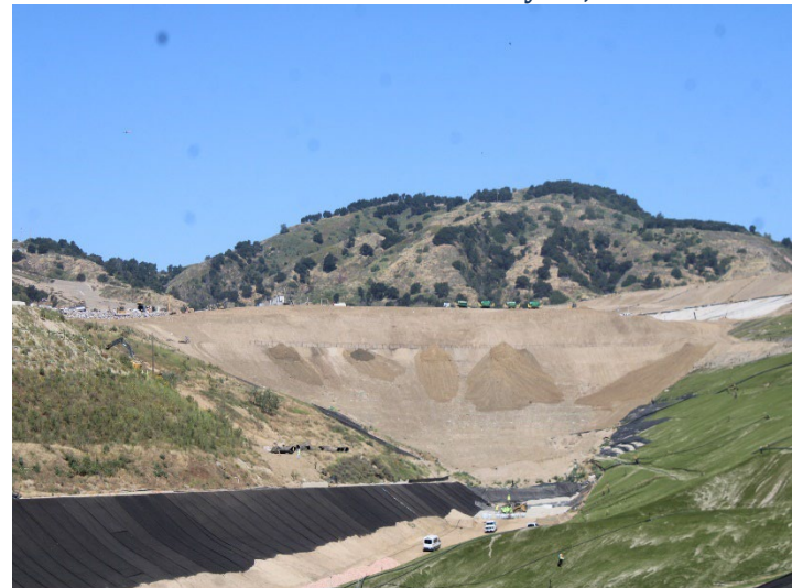
Photo 540: General Site: May 21, 2026
