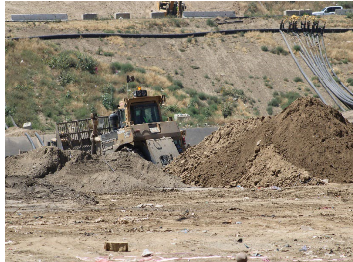
Photo 574: General Site: May 21, 2026
