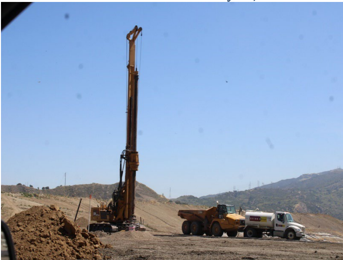
Photo 563: General Site: May 21, 2026
