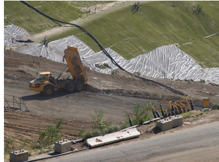
Photo 38: Working Area, CC4 Part 1/2: May 21, 2026
