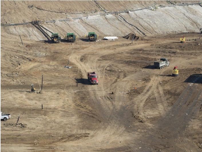
Photo 83: Working Area, CC-4 Part 4/5, CC-5A: April 9, 2026
