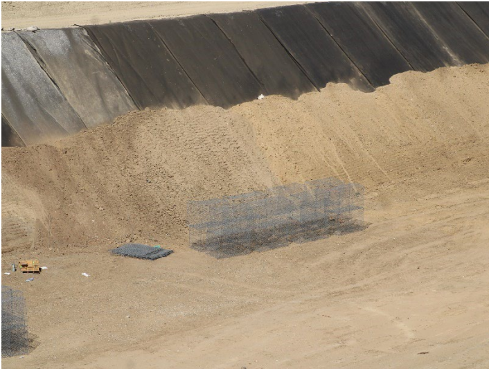
Photo 529: General Site: May 21, 2026
