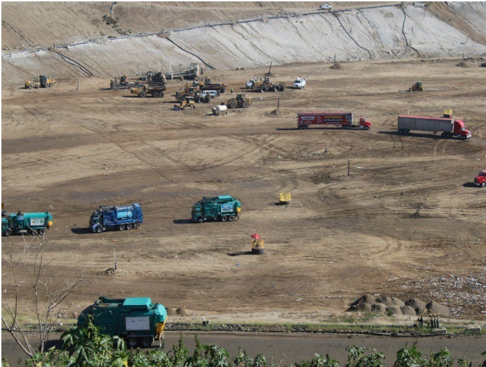
Photo 93: Working Area, CC-4 Part 4/5, CC-5A: May 21, 2026
