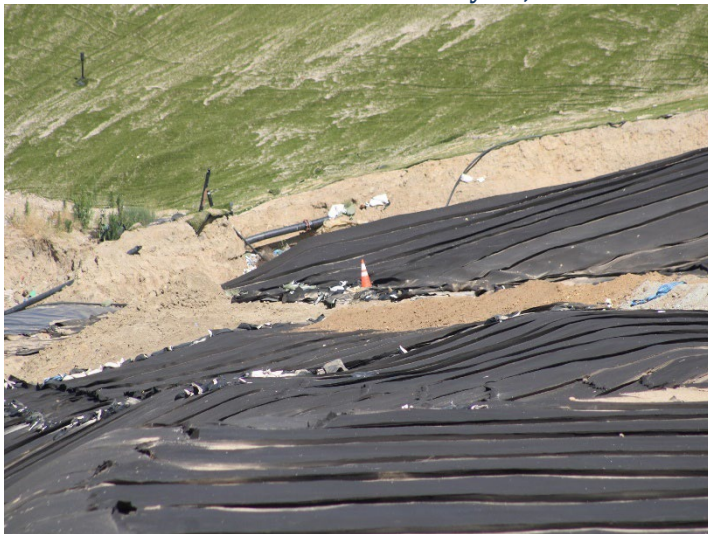
Photo 535: General Site: May 21, 2026
