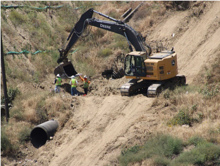
Photo 589: General Site: May 21, 2026
