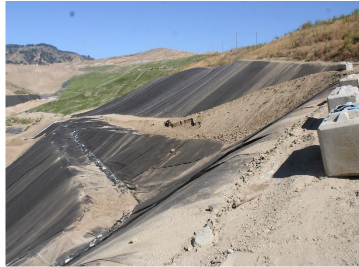
Photo 622: General Site: June 11, 2026
