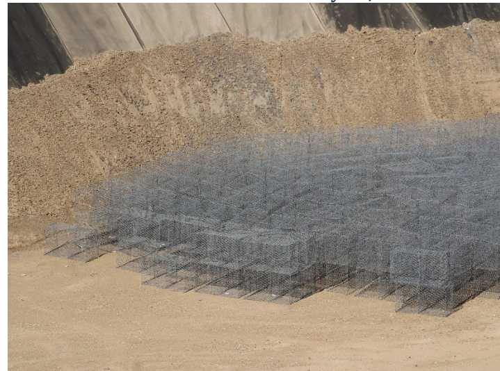
Photo 528: General Site: May 21, 2026
