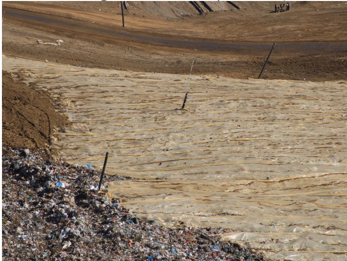
Photo 139: Working Area, CC-4 Part 4/5, CC-5A: June 11, 2026
