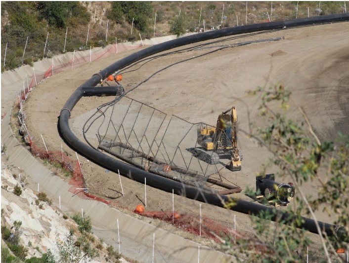
Photo 97: Working Area, CC-4 Part 4/5, CC-5A: May 21, 2026
