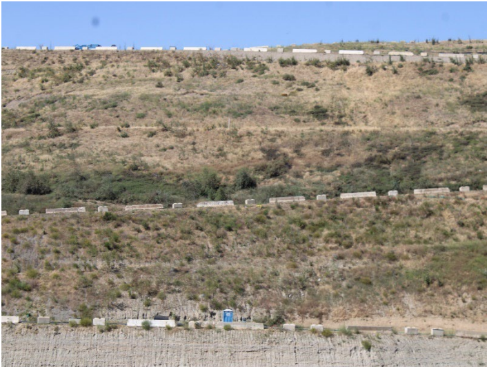
Photo 537: General Site: May 21, 2026
