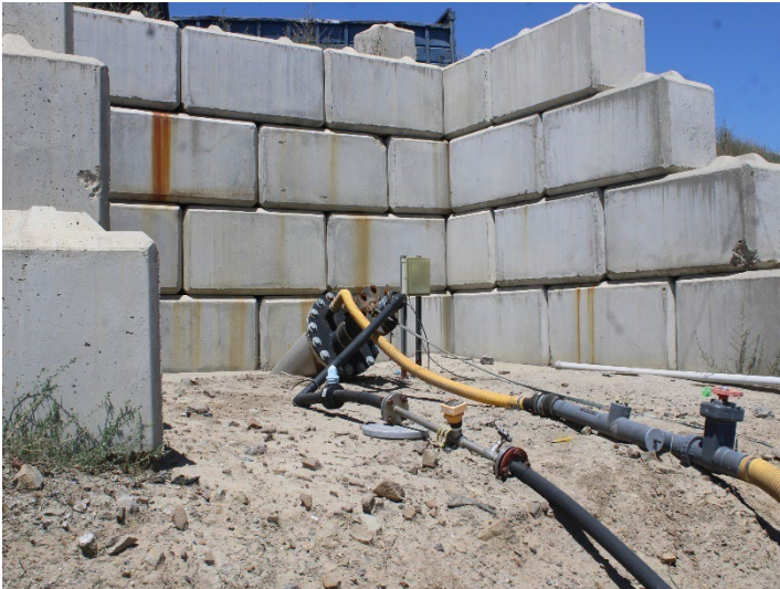
Photo 593: General Site: May 21, 2026
