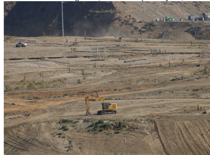
Photo 40: Working Area, CC4 Part 1/2: June 11, 2026
