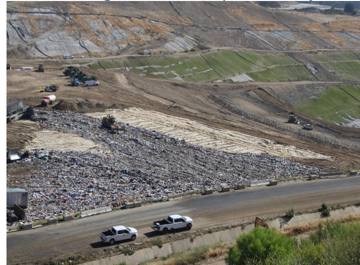
Photo 96: Working Area, CC-4 Part 4/5, CC-5A: May 21, 2026
