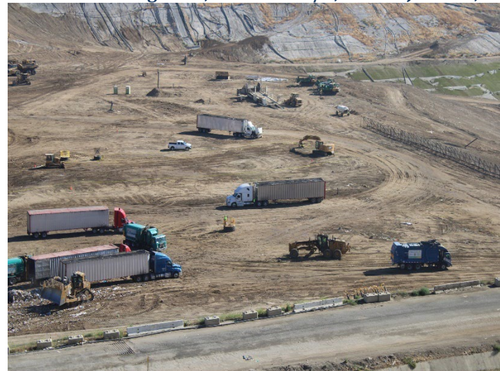
Photo 132: Working Area, CC-4 Part 4/5, CC-5A: June 11, 2026
