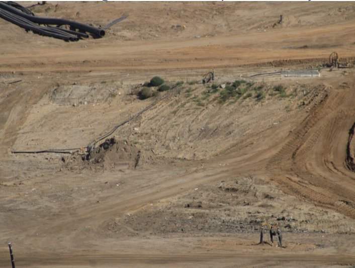
Photo 107: Working Area, CC-4 Part 4/5, CC-5A: May 21, 2026
