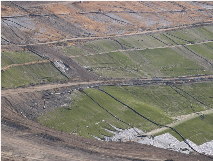
Photo 145: Closure Turf: June 11, 2026
