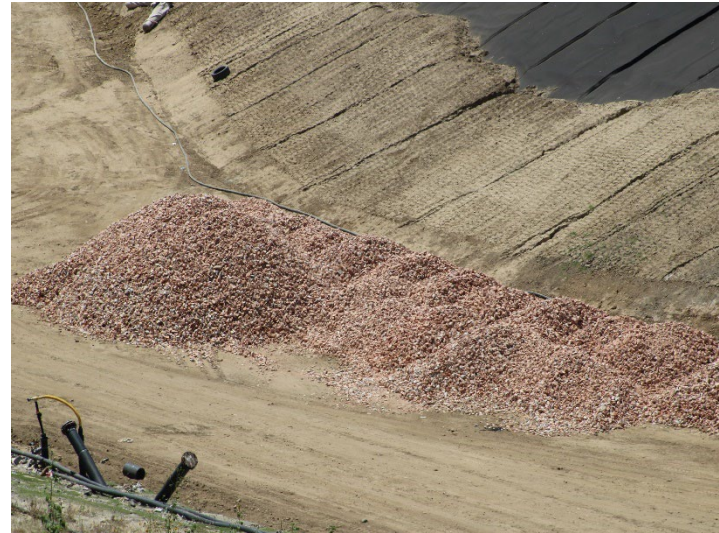
Photo 582: General Site: May 21, 2026
