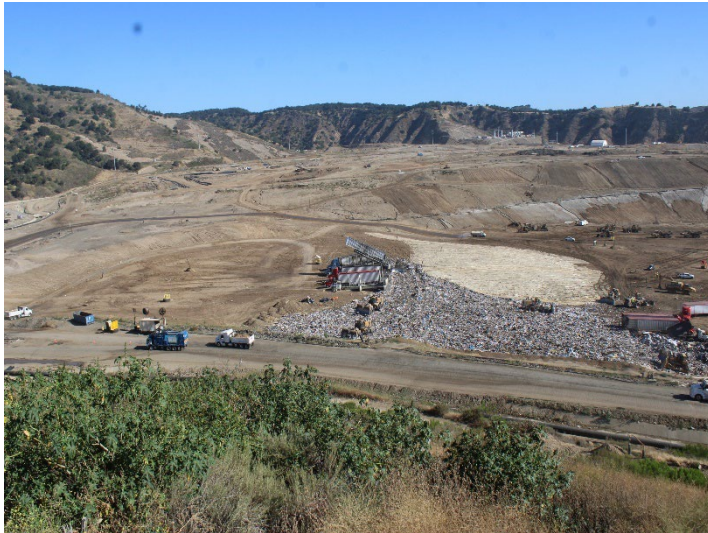
Photo 125: Working Area, CC-4 Part 4/5, CC-5A: June 11, 2026
