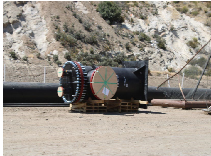
Photo 562: General Site: May 21, 2026
