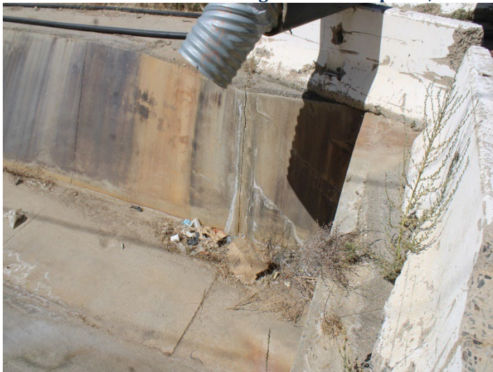
Photo 303: Eastside Drainage Channel: May 21, 2026
