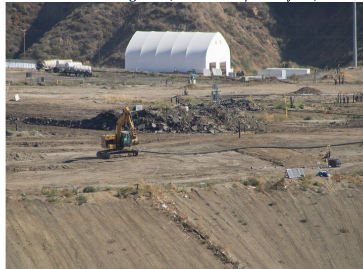
Photo 36: Working Area, CC4 Part 1/2: May 21, 2026
