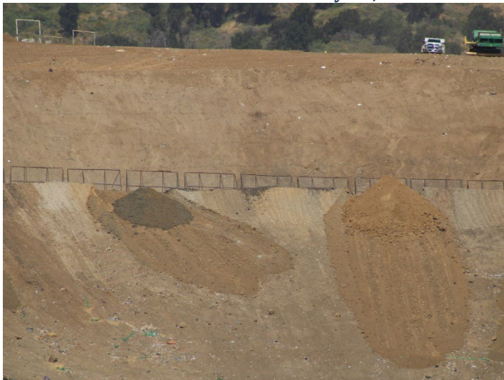
Photo 543: General Site: May 21, 2026
