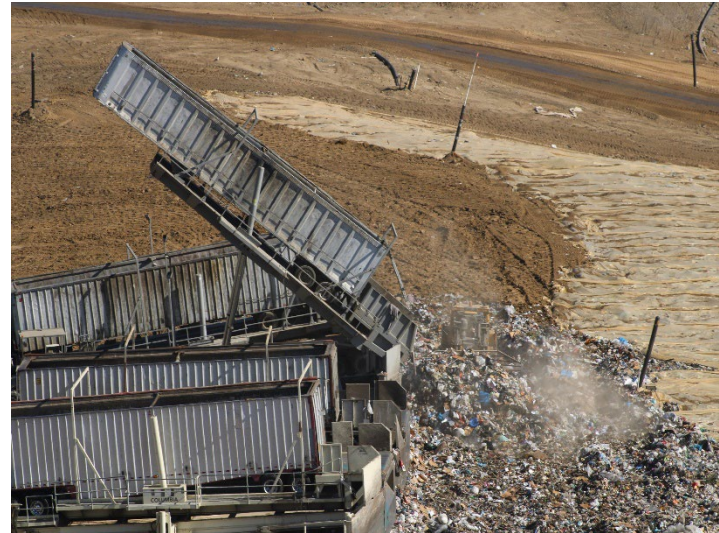
Photo 134: Working Area, CC-4 Part 4/5, CC-5A: June 11, 2026
