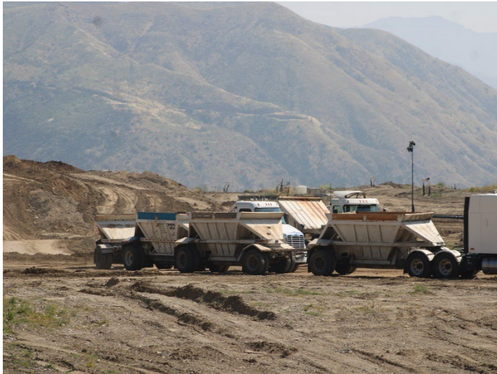
Photo 253: County Top Deck: April 9, 2026
