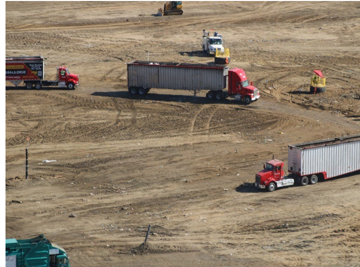
Photo 110: Working Area, CC-4 Part 4/5, CC-5A: May 21, 2026
