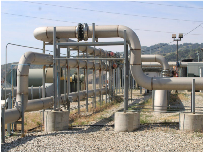
Photo 217: Flares 9, 10, 11 and Gas-to-Energy Facility: April 9, 2026
