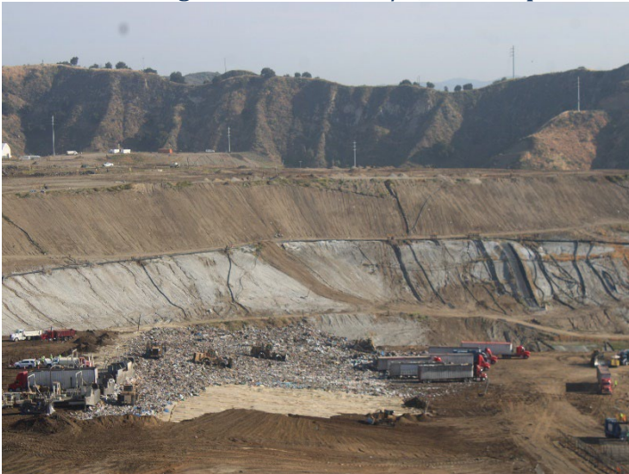
Photo 75: Working Area, CC-4 Part 4/5, CC-5A: April 9, 2026
