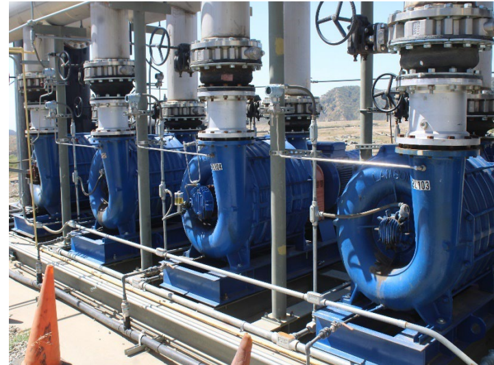
Photo 230: Flares 9, 10, 11 and Gas-to-Energy Facility: May 21, 2026
