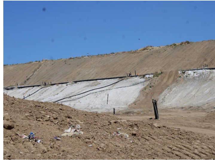
Photo 570: General Site: May 21, 2026
