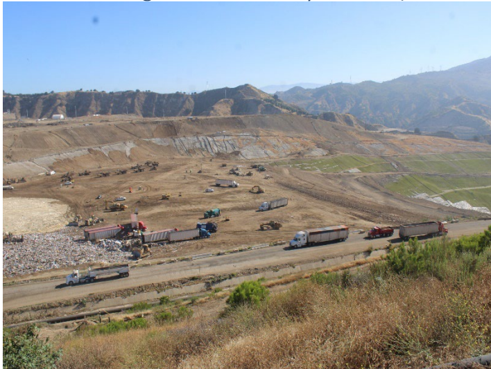
Photo 127: Working Area, CC-4 Part 4/5, CC-5A: June 11, 2026
