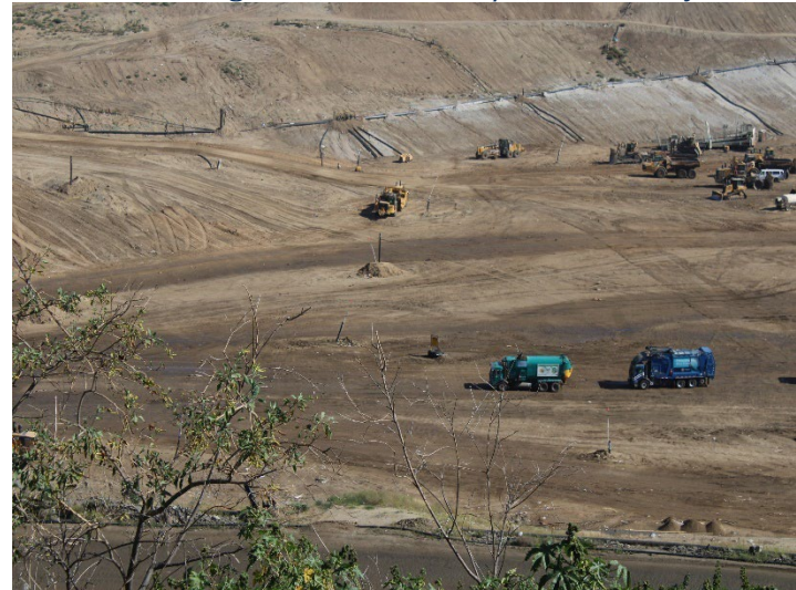
Photo 92: Working Area, CC-4 Part 4/5, CC-5A: May 21, 2026
