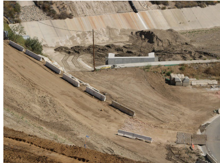
Photo 494: General Site: May 21, 2026
