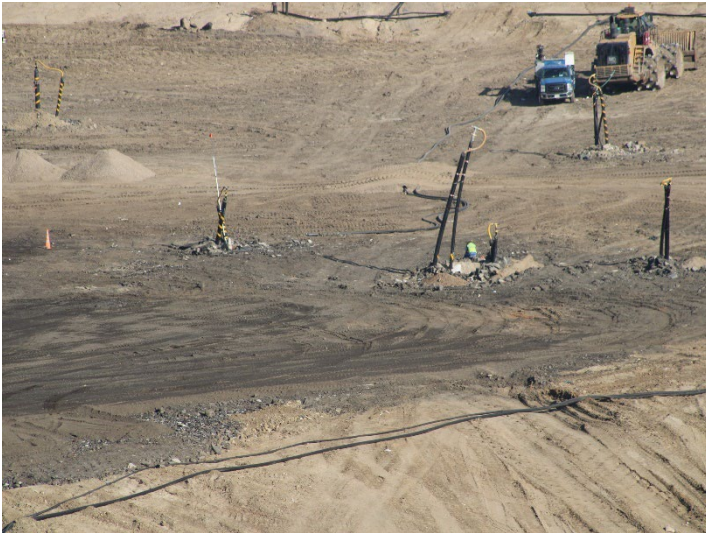
Photo 81: Working Area, CC-4 Part 4/5, CC-5A: April 9, 2026
