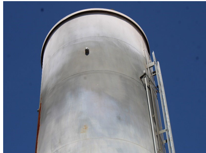
Photo 228: Flares 9, 10, 11 and Gas-to-Energy Facility: May 21, 2026
