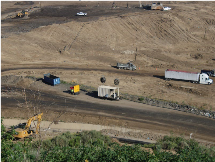
Photo 67: Working Area, CC-4 Part 4/5, CC-5A: April 9, 2026
