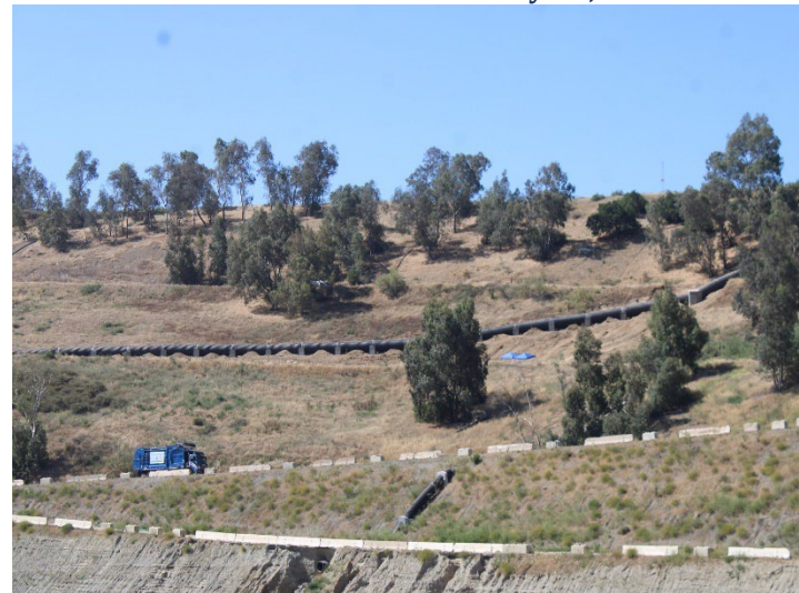
Photo 536: General Site: May 21, 2026
