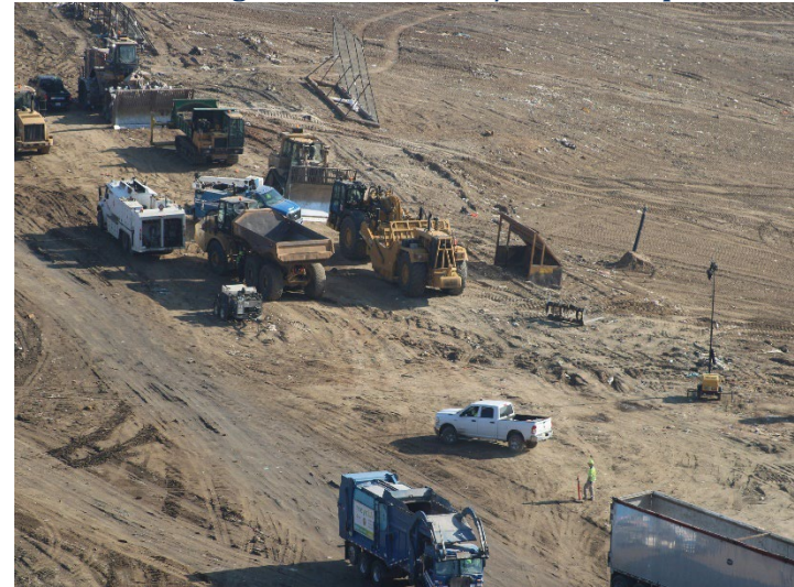
Photo 88: Working Area, CC-4 Part 4/5, CC-5A: April 9, 2026
