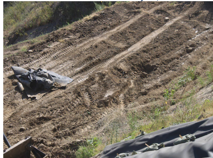
Photo 492: General Site: May 21, 2026
