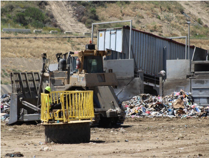
Photo 121: Working Area, CC-4 Part 4/5, CC-5A: May 21, 2026
