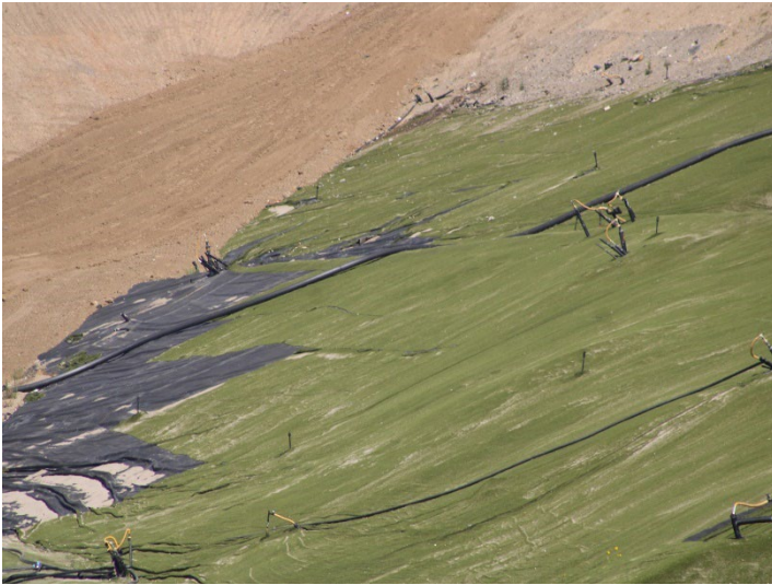
Photo 545: General Site: May 21, 2026
