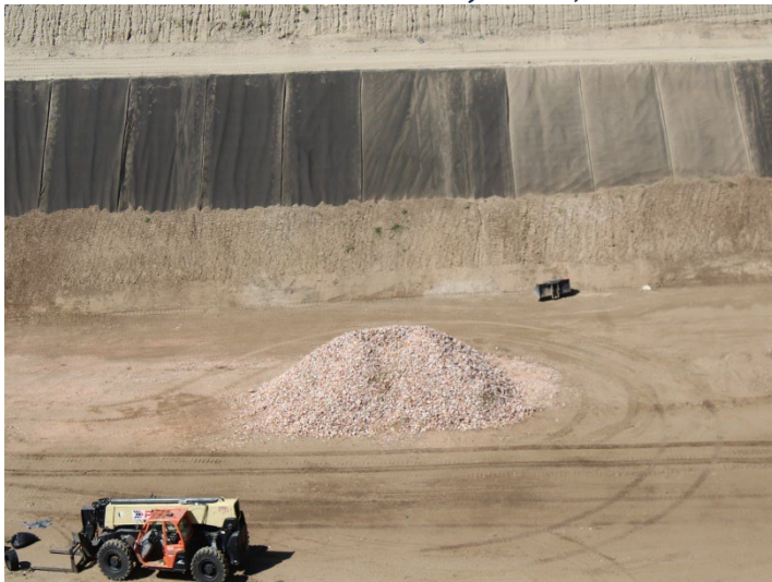
Photo 631: General Site: June 11, 2026
