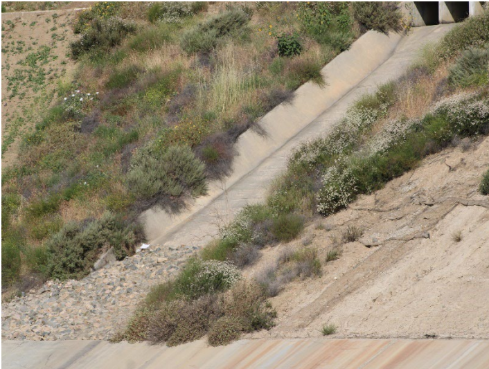
Photo 297: Eastside Drainage Channel: April 9, 2026
