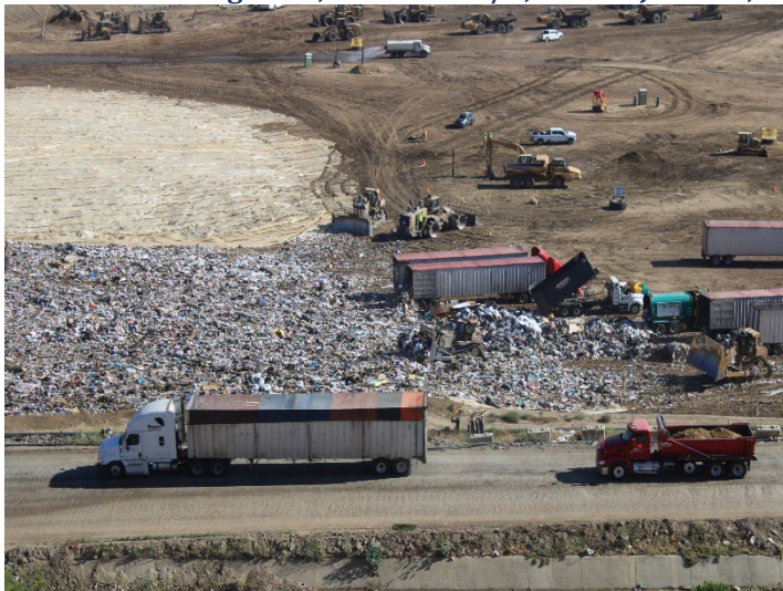
Photo 131: Working Area, CC-4 Part 4/5, CC-5A: June 11, 2026
