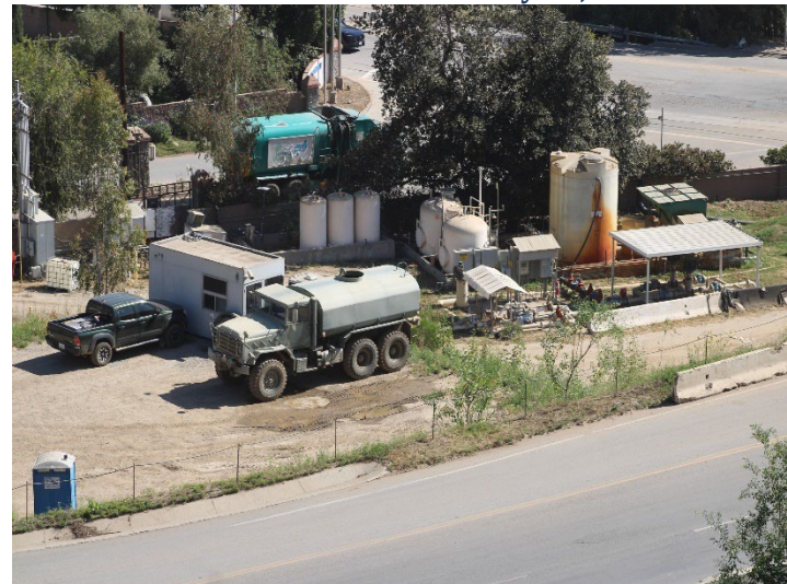
Photo 496: General Site: May 21, 2026
