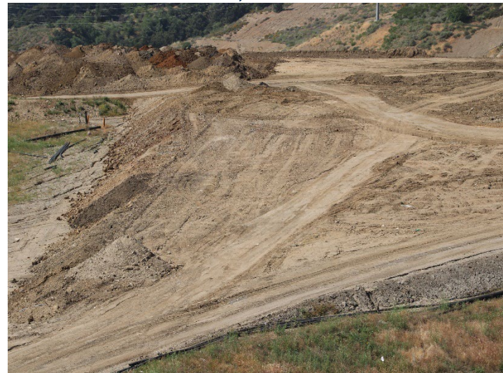
Photo 248: County Top Deck: April 9, 2026
