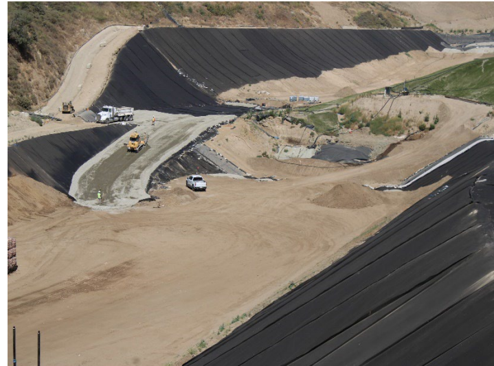
Photo 634: General Site: June 11, 2026
