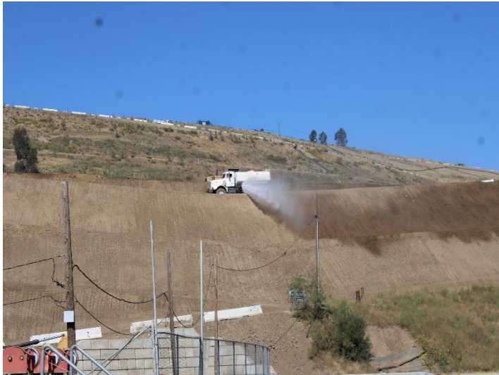
Photo 613: General Site: June 11, 2026
