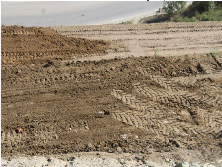
Photo 491: General Site: May 21, 2026
