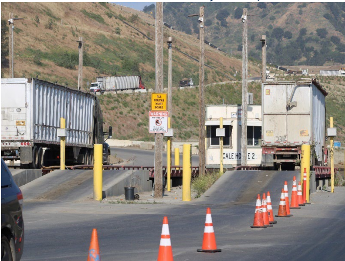
Photo 147: Office and Scales Location: April 9, 2026
