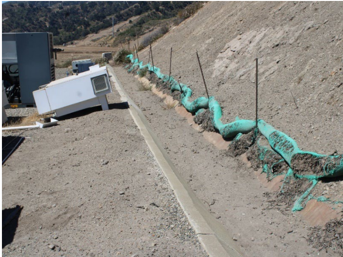
Photo 245: Flares 9, 10, 11 and Gas-to-Energy Facility: June 11, 2026
