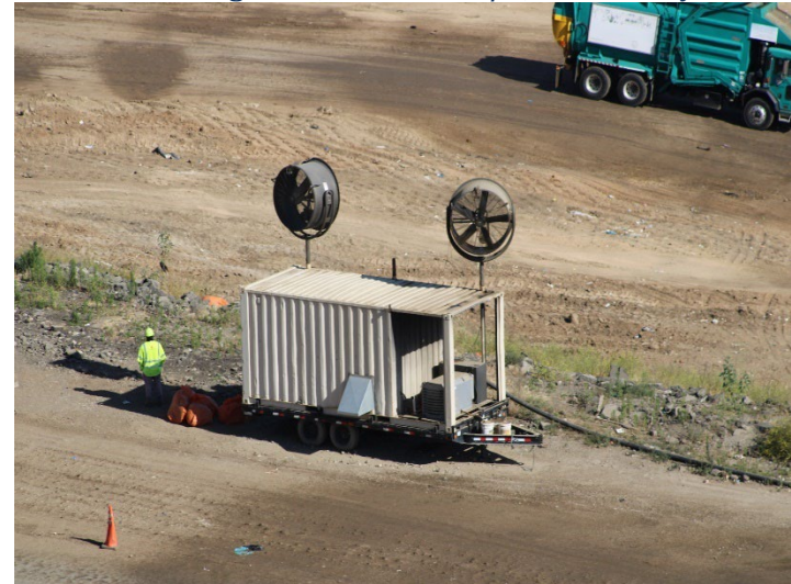
Photo 100: Working Area, CC-4 Part 4/5, CC-5A: May 21, 2026
