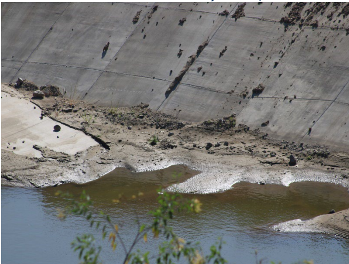
Photo 603: General Site: June 11, 2026
