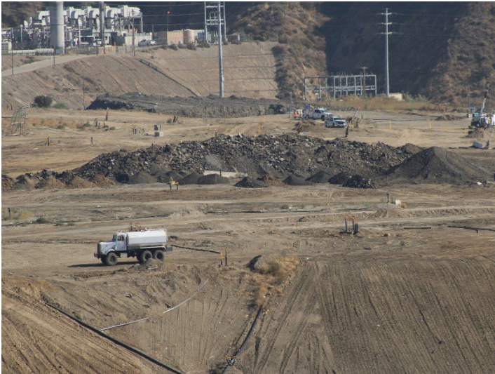
Photo 41: Working Area, CC4 Part 1/2: June 11, 2026
