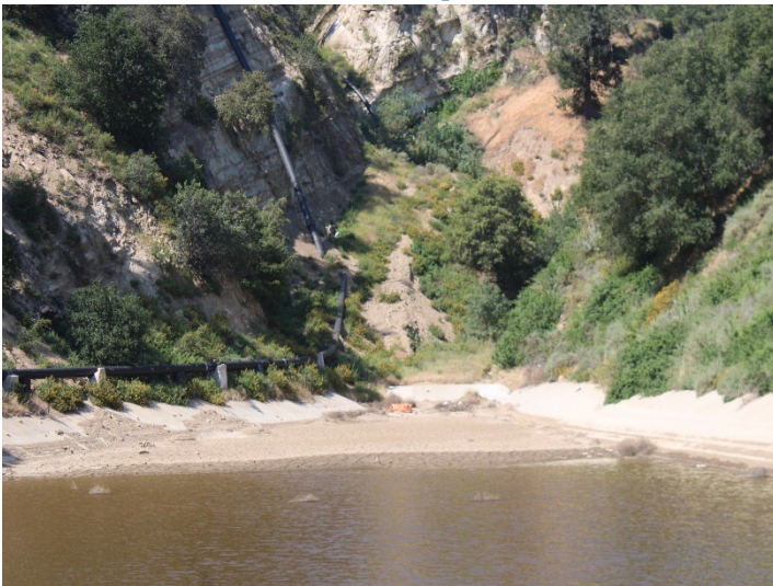
Photo 7: Basin A: April 9, 2026
