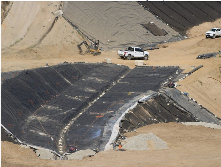
Photo 531: General Site: May 21, 2026
