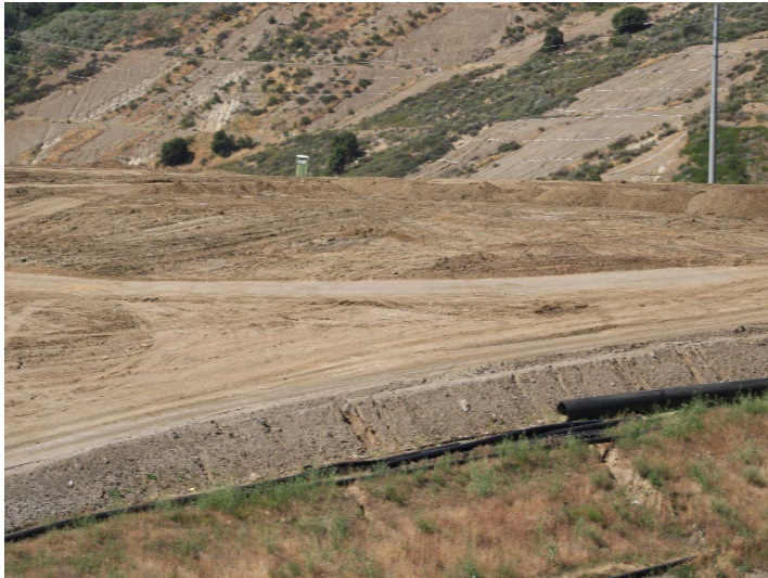
Photo 249: County Top Deck: April 9, 2026
