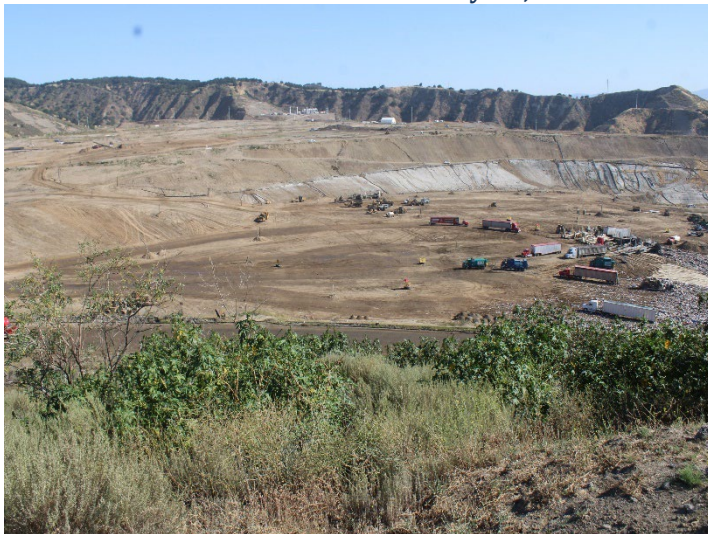
Photo 479: General Site: May 21, 2026
