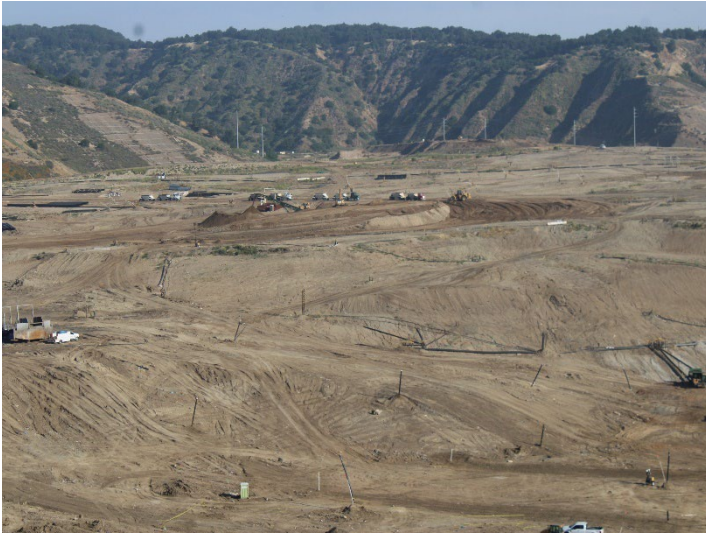
Photo 73: Working Area, CC-4 Part 4/5, CC-5A: April 9, 2026
