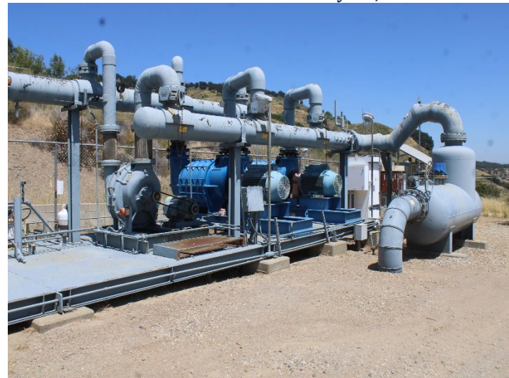
Photo 592: General Site: May 21, 2026
