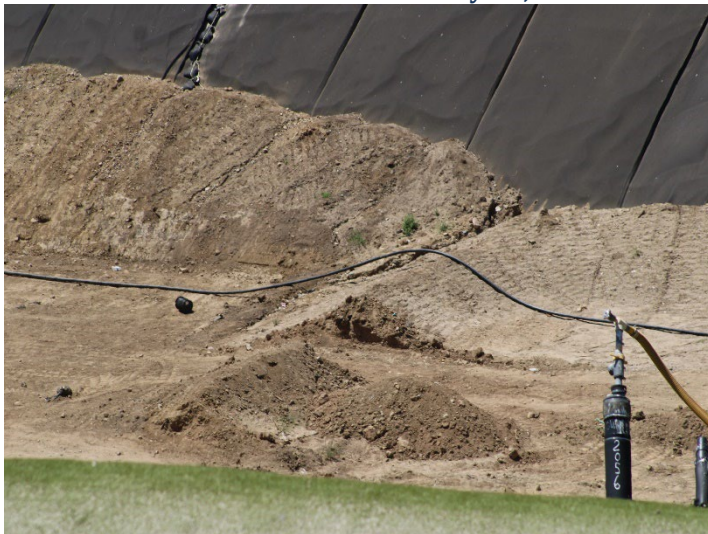
Photo 583: General Site: May 21, 2026
