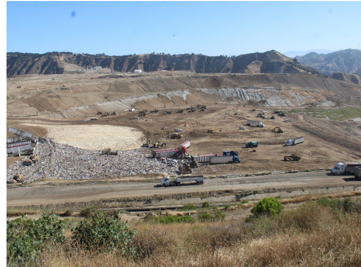
Photo 126: Working Area, CC-4 Part 4/5, CC-5A: June 11, 2026
