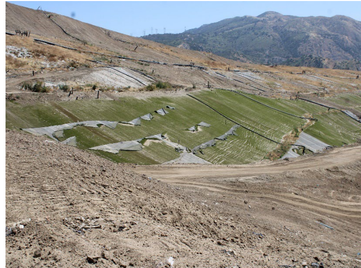
Photo 566: General Site: May 21, 2026
