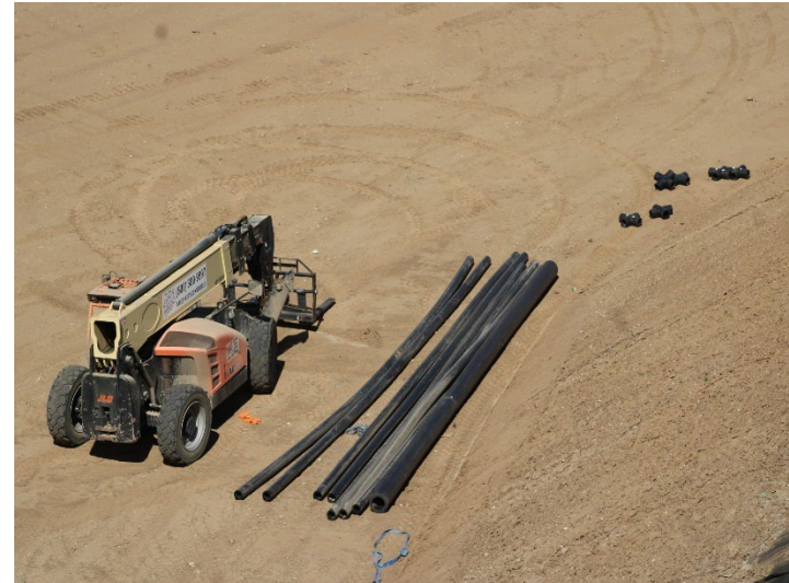
Photo 530: General Site: May 21, 2026
