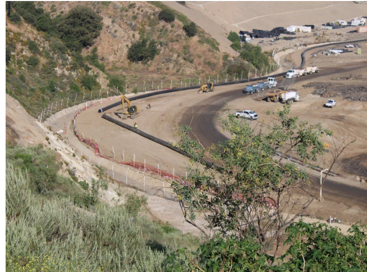
Photo 66: Working Area, CC-4 Part 4/5, CC-5A: April 9, 2026
