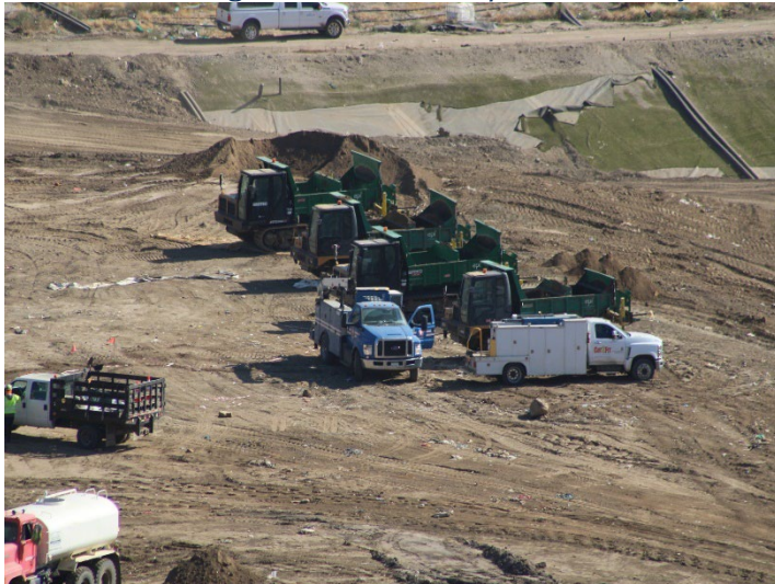
Photo 119: Working Area, CC-4 Part 4/5, CC-5A: May 21, 2026
