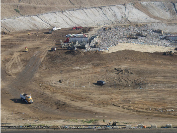
Photo 69: Working Area, CC-4 Part 4/5, CC-5A: April 9, 2026
