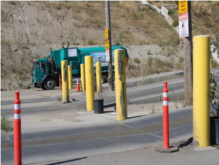
Photo 149: Office and Scales Location: May 21, 2026
