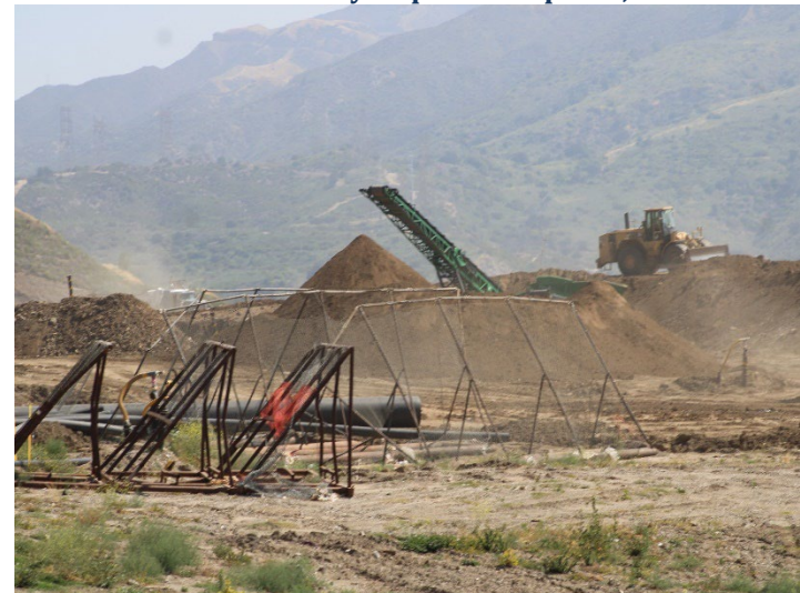
Photo 252: County Top Deck: April 9, 2026
