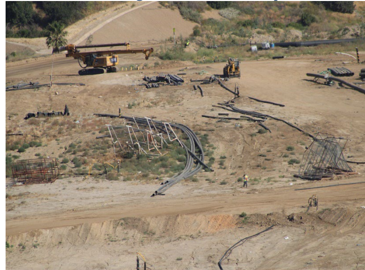
Photo 56: Working Area, CC-4 Part 3: May 21, 2026
