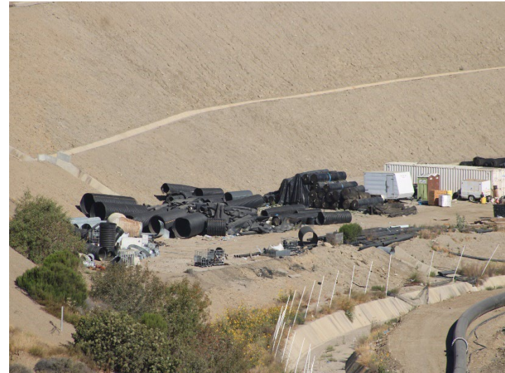
Photo 594: General Site: June 11, 2026
