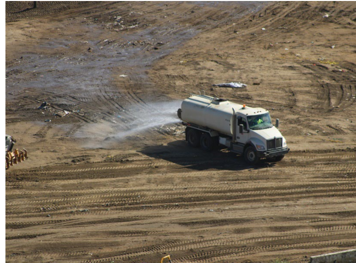
Photo 138: Working Area, CC-4 Part 4/5, CC-5A: June 11, 2026
