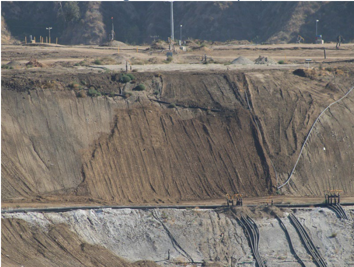
Photo 43: Working Area, CC4 Part 1/2: June 11, 2026
