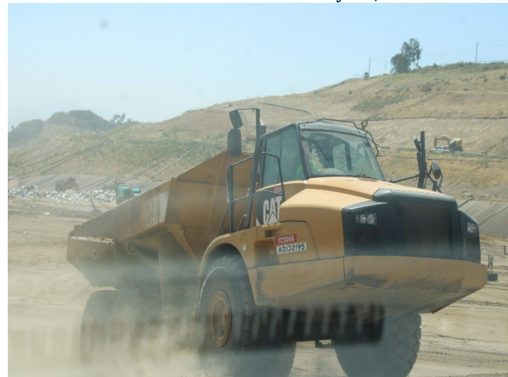
Photo 564: General Site: May 21, 2026
