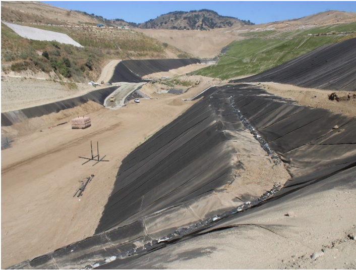
Photo 621: General Site: June 11, 2026
