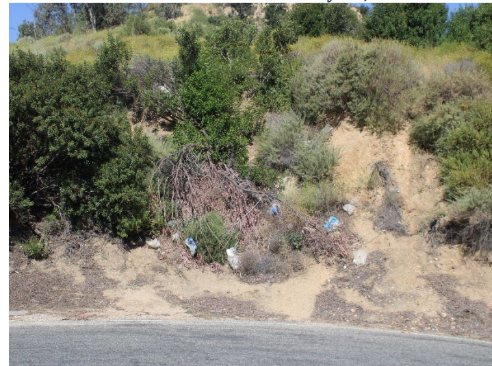
Photo 484: General Site: May 21, 2026
