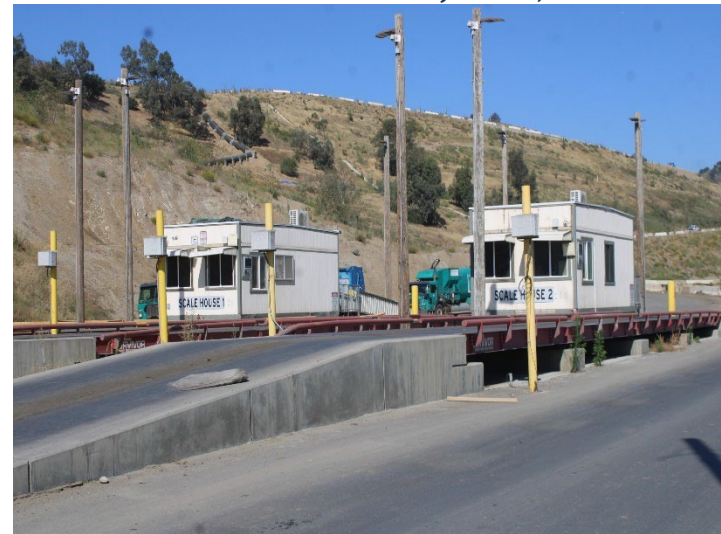
Photo 148: Office and Scales Location: May 21, 2026
