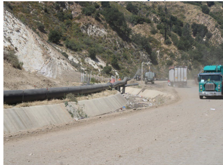
Photo 560: General Site: May 21, 2026
