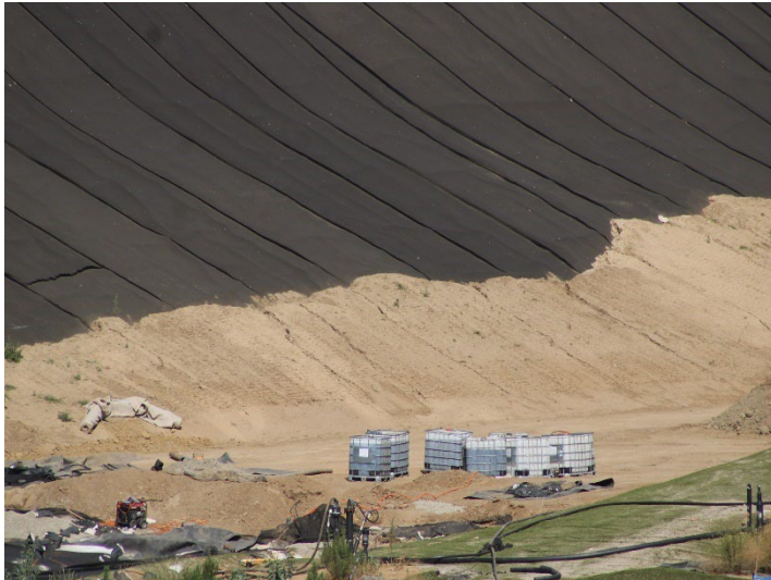
Photo 645: General Site: June 11, 2026
