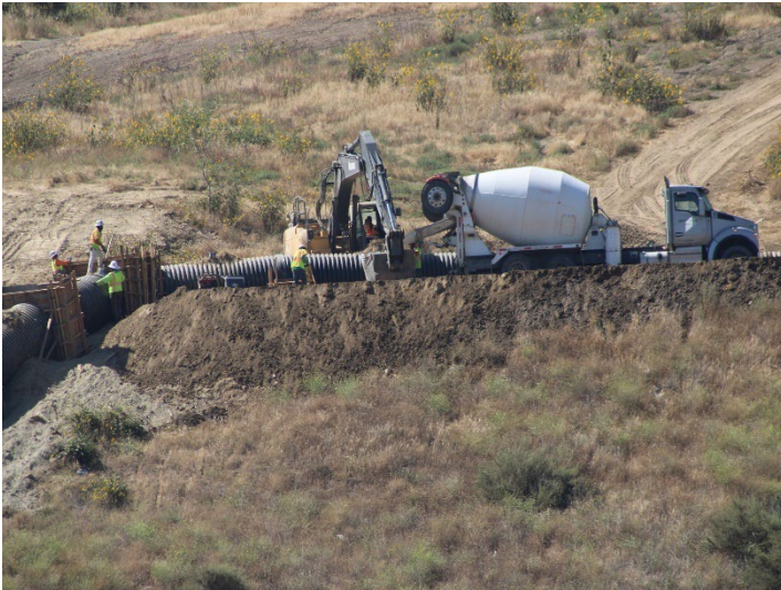
Photo 649: General Site: June 11, 2026
