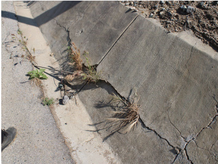
Photo 301: Eastside Drainage Channel: April 9, 2026
