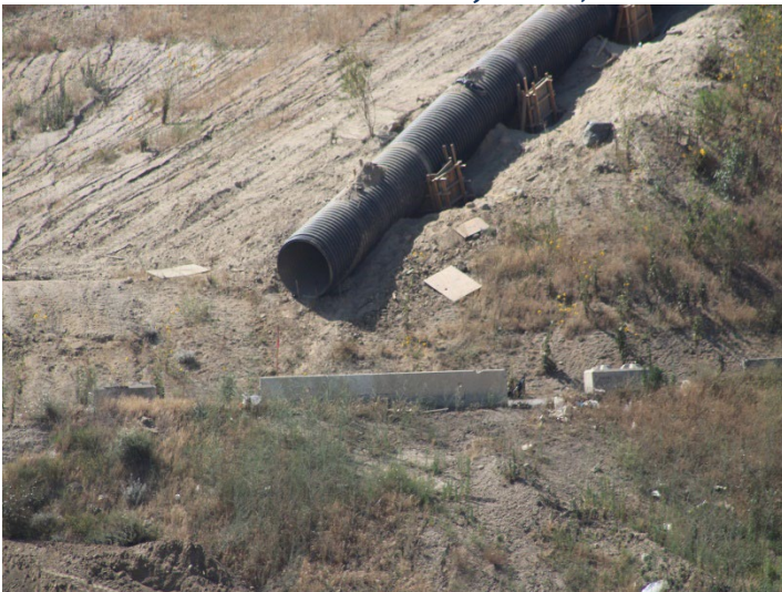
Photo 651: General Site: June 11, 2026
