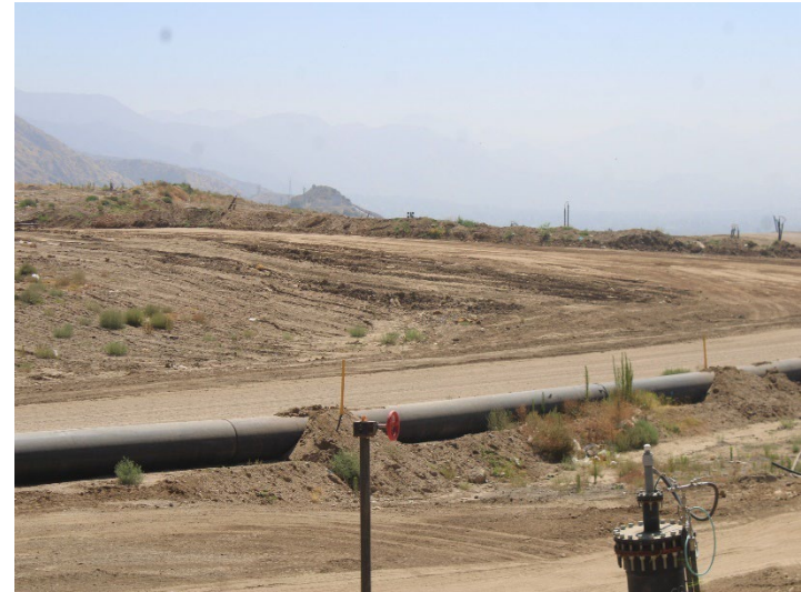
Photo 262: County Top Deck: June 11, 2026
