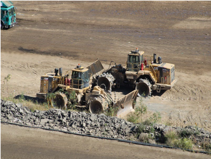
Photo 101: Working Area, CC-4 Part 4/5, CC-5A: May 21, 2026
