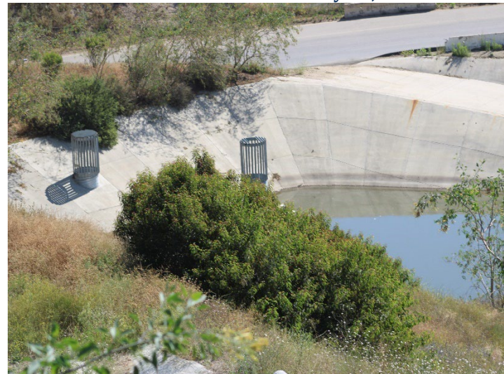
Photo 504: General Site: May 21, 2026
