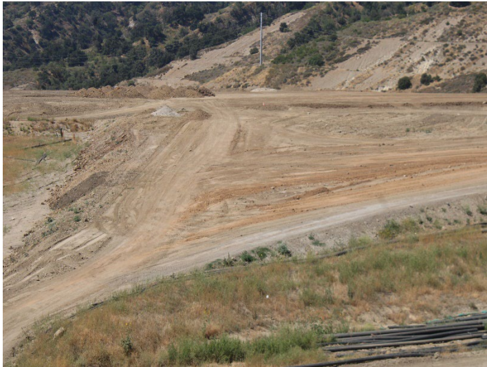
Photo 257: County Top Deck: June 11, 2026
