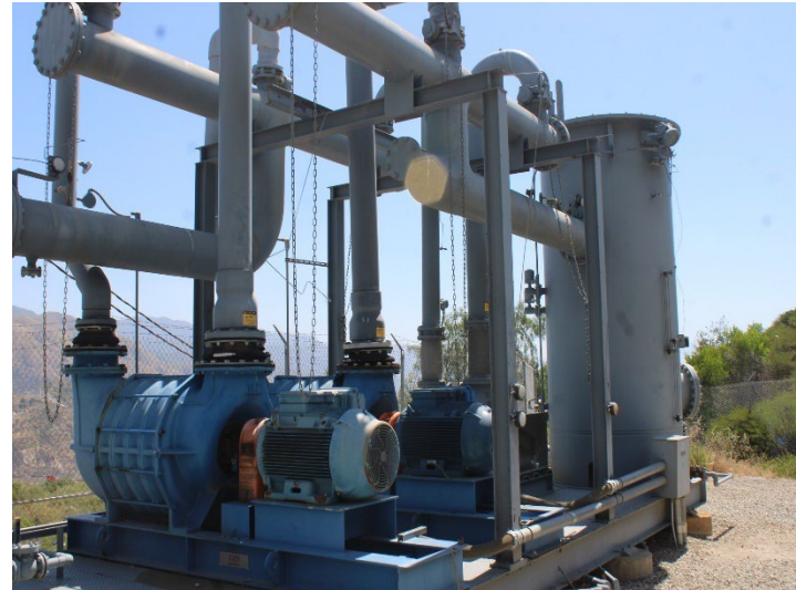
Photo 558: General Site: May 21, 2026
