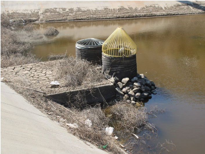
Photo 5: Basin A: April 9, 2026
