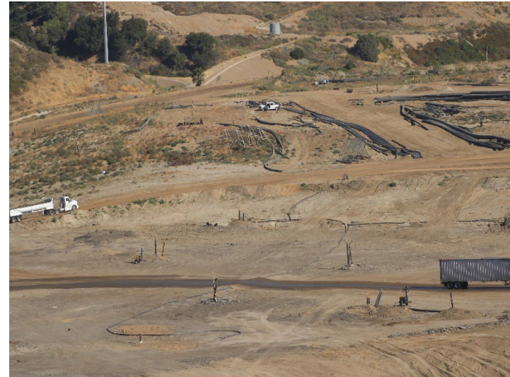
Photo 58: Working Area, CC-4 Part 3: June 11, 2026
