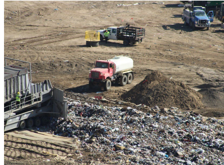
Photo 118: Working Area, CC-4 Part 4/5, CC-5A: May 21, 2026
