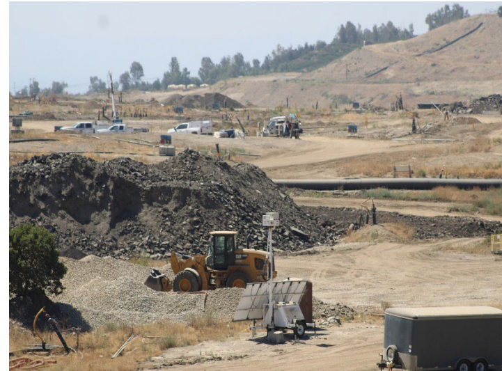
Photo 658: General Site: June 11, 2026
