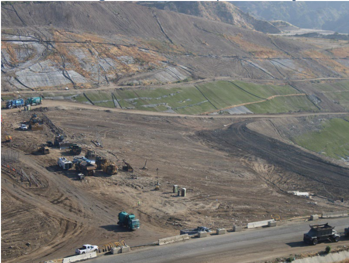
Photo 71: Working Area, CC-4 Part 4/5, CC-5A: April 9, 2026
