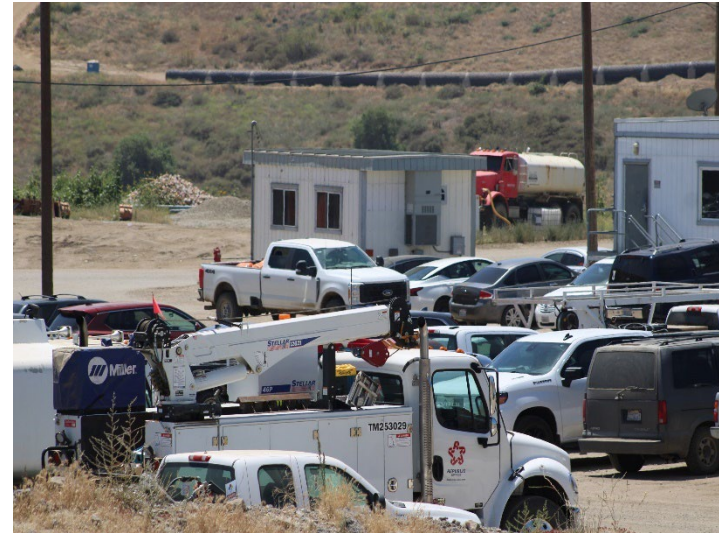
Photo 150: Office and Scales Location: May 21, 2026
