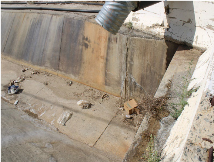
Photo 299: Eastside Drainage Channel: April 9, 2026
