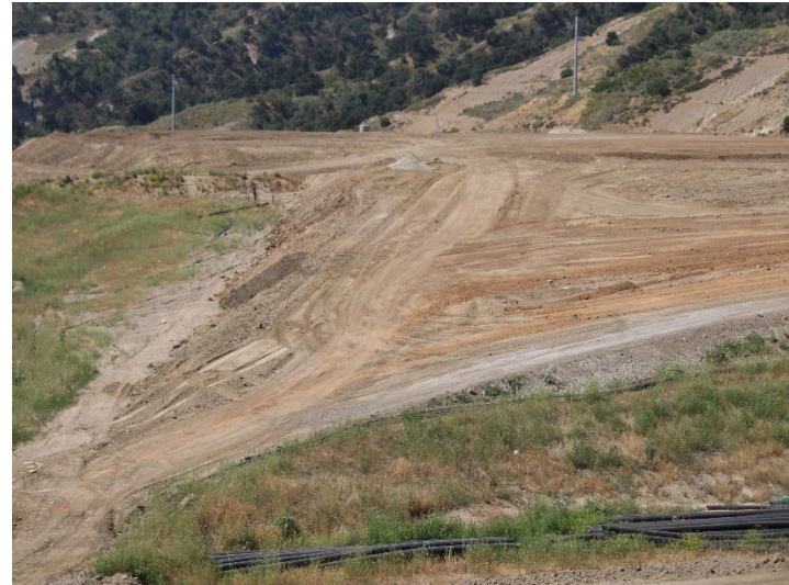
Photo 254: County Top Deck: May 21, 2026
