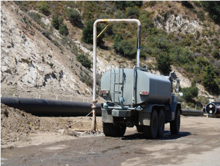
Photo 561: General Site: May 21, 2026
