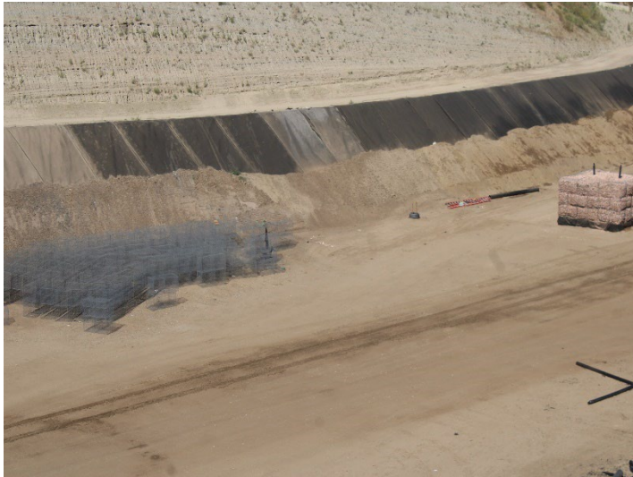
Photo 633: General Site: June 11, 2026
