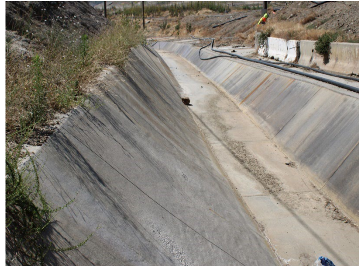
Photo 302: Eastside Drainage Channel: May 21, 2026
