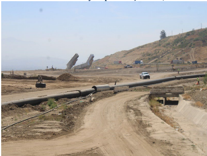
Photo 263: County Top Deck: June 11, 2026
