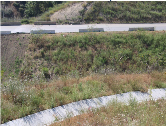
Photo 503: General Site: May 21, 2026
