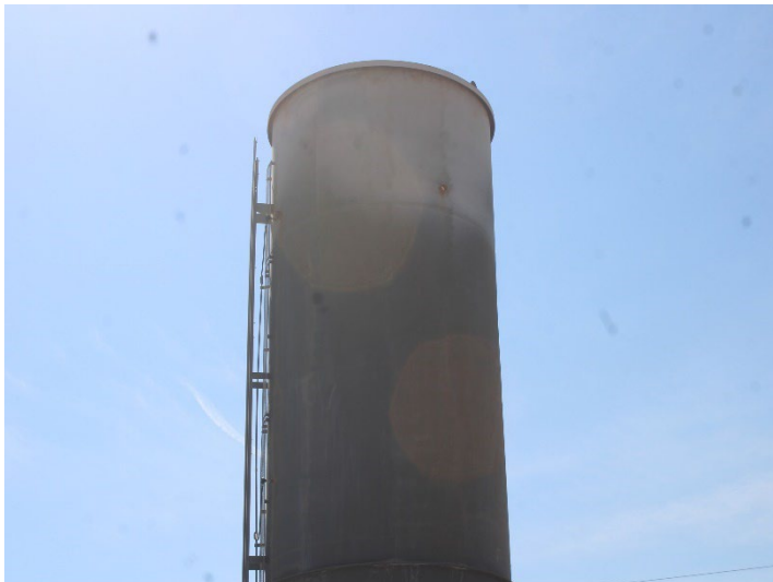
Photo 215: Flares 9, 10, 11 and Gas-to-Energy Facility: April 9, 2026
