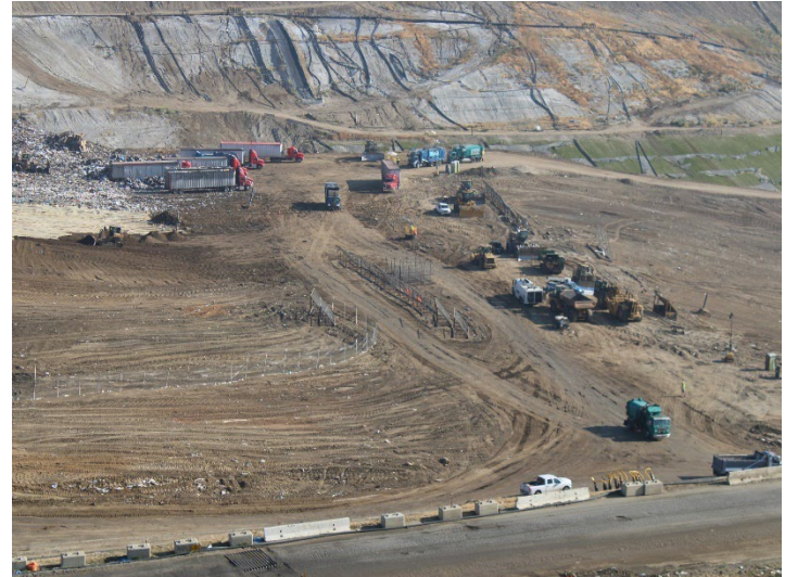
Photo 70: Working Area, CC-4 Part 4/5, CC-5A: April 9, 2026
