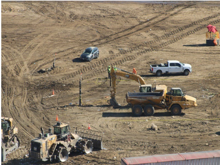
Photo 137: Working Area, CC-4 Part 4/5, CC-5A: June 11, 2026
