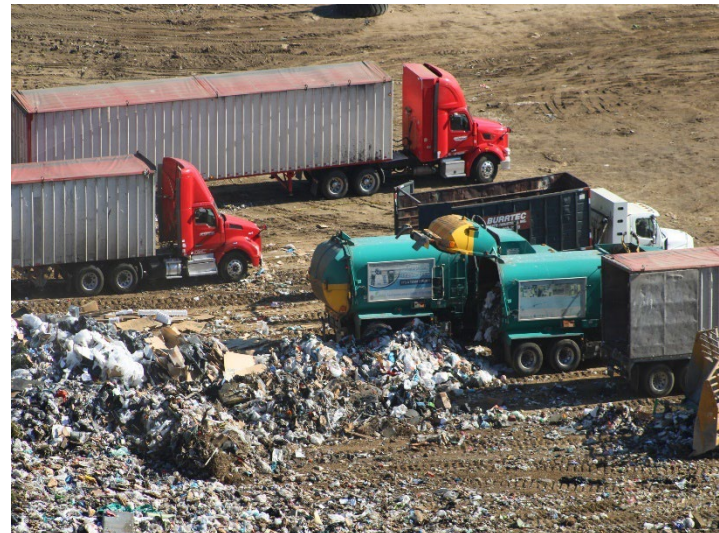
Photo 136: Working Area, CC-4 Part 4/5, CC-5A: June 11, 2026
