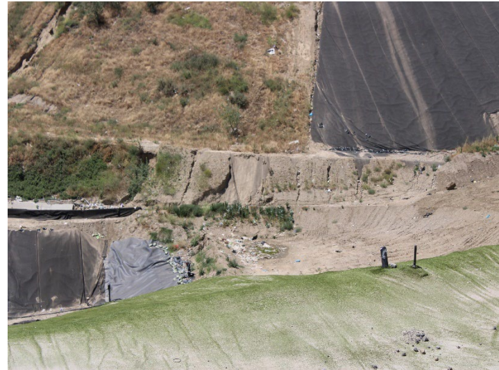
Photo 578: General Site: May 21, 2026
