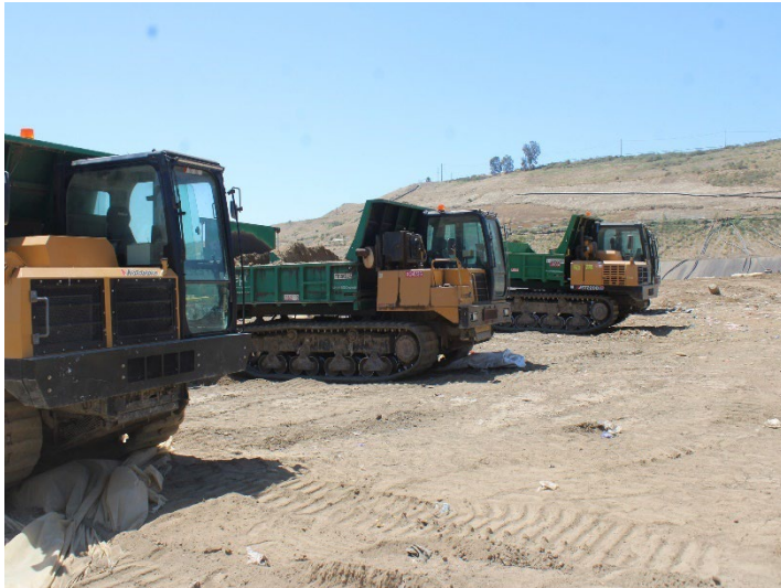
Photo 573: General Site: May 21, 2026
