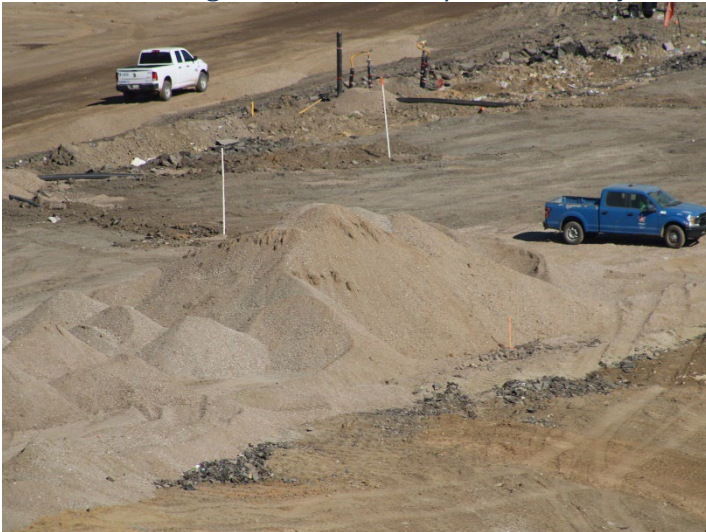
Photo 103: Working Area, CC-4 Part 4/5, CC-5A: May 21, 2026
