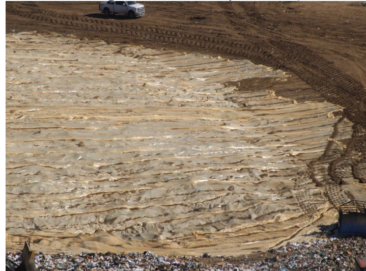
Photo 140: Working Area, CC-4 Part 4/5, CC-5A: June 11, 2026
