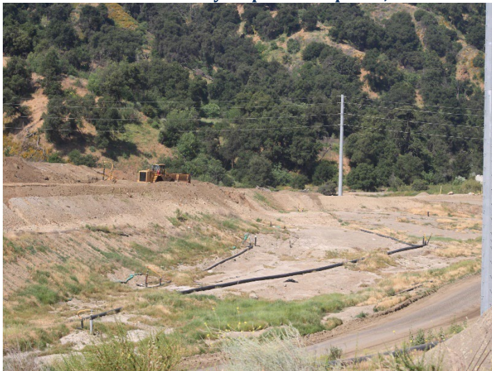
Photo 251: County Top Deck: April 9, 2026
