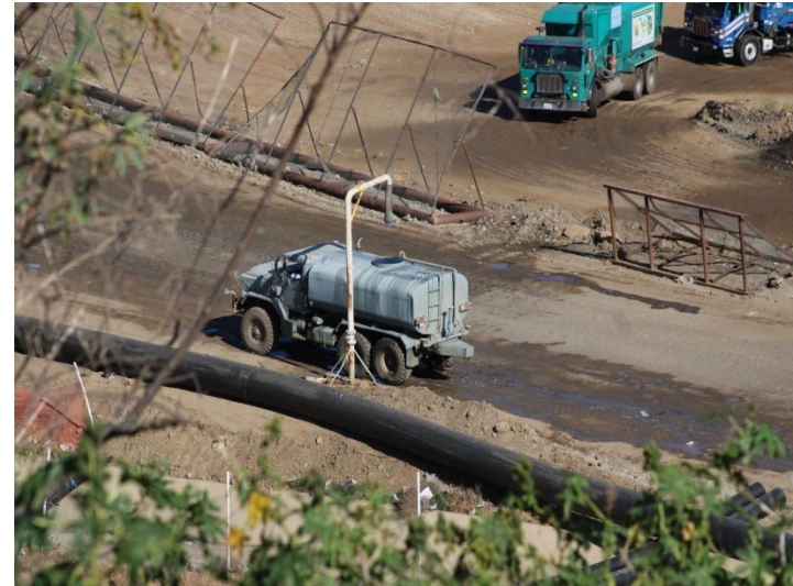
Photo 98: Working Area, CC-4 Part 4/5, CC-5A: May 21, 2026
