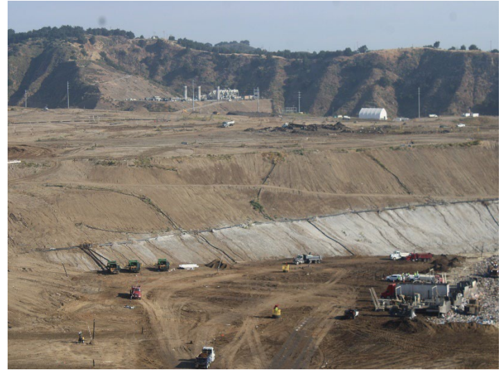
Photo 74: Working Area, CC-4 Part 4/5, CC-5A: April 9, 2026
