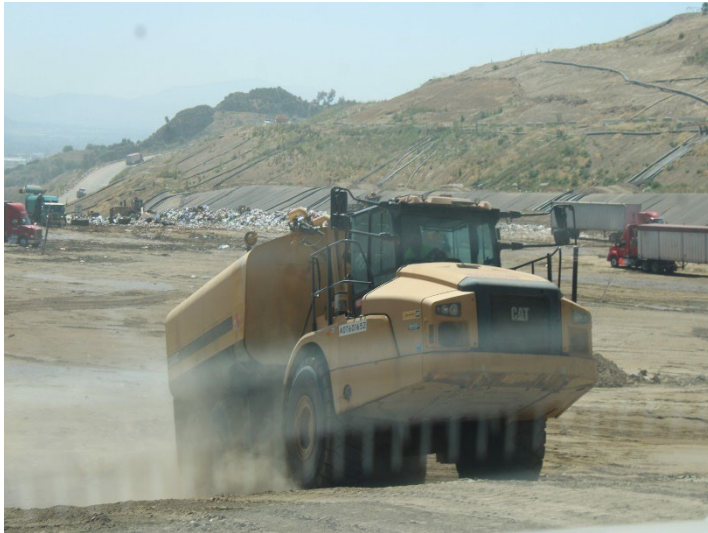
Photo 565: General Site: May 21, 2026
