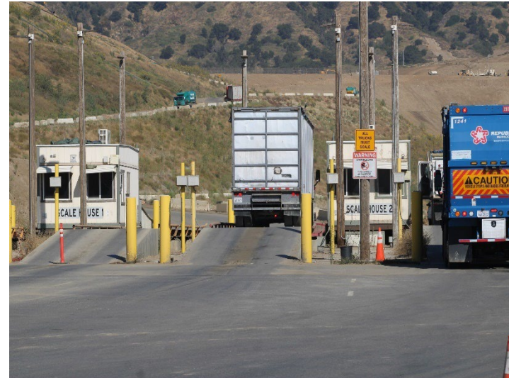
Photo 154: Office and Scales Location: June 11, 2026
