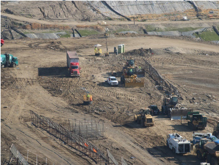
Photo 87: Working Area, CC-4 Part 4/5, CC-5A: April 9, 2026
