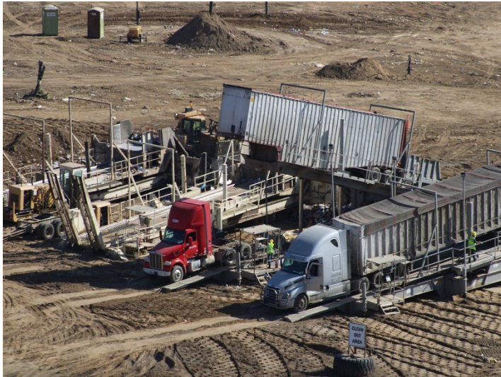
Photo 117: Working Area, CC-4 Part 4/5, CC-5A: May 21, 2026
