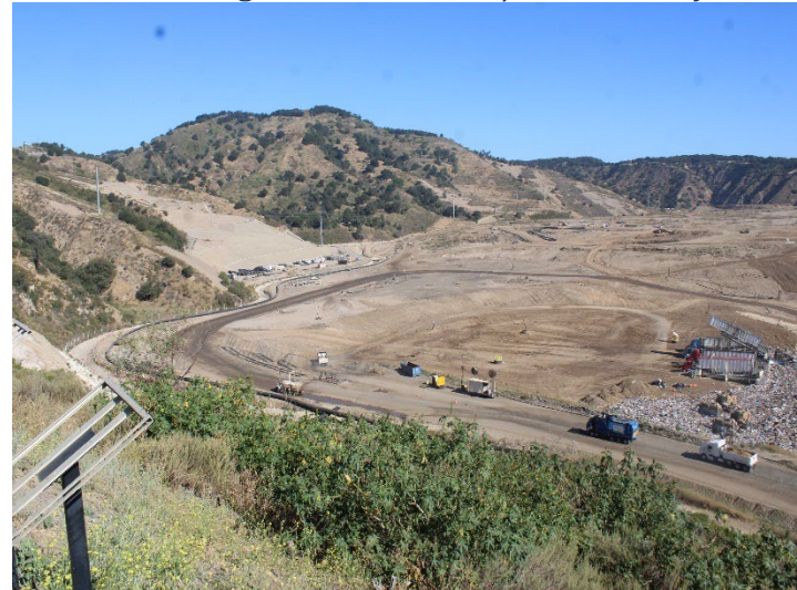
Photo 124: Working Area, CC-4 Part 4/5, CC-5A: June 11, 2026
