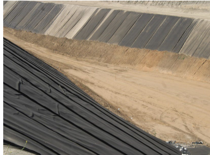
Photo 514: General Site: May 21, 2026
