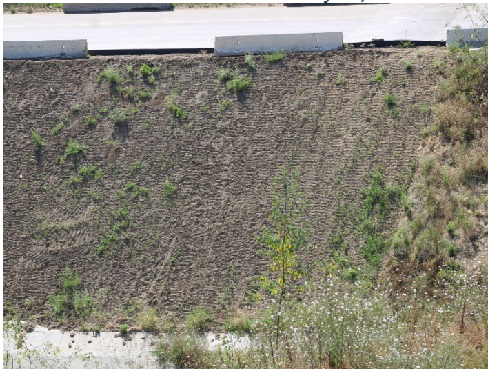
Photo 507: General Site: May 21, 2026
