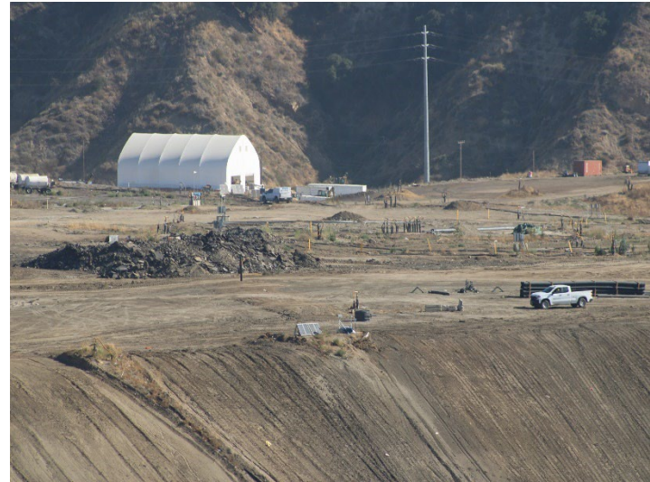
Photo 42: Working Area, CC4 Part 1/2: June 11, 2026
