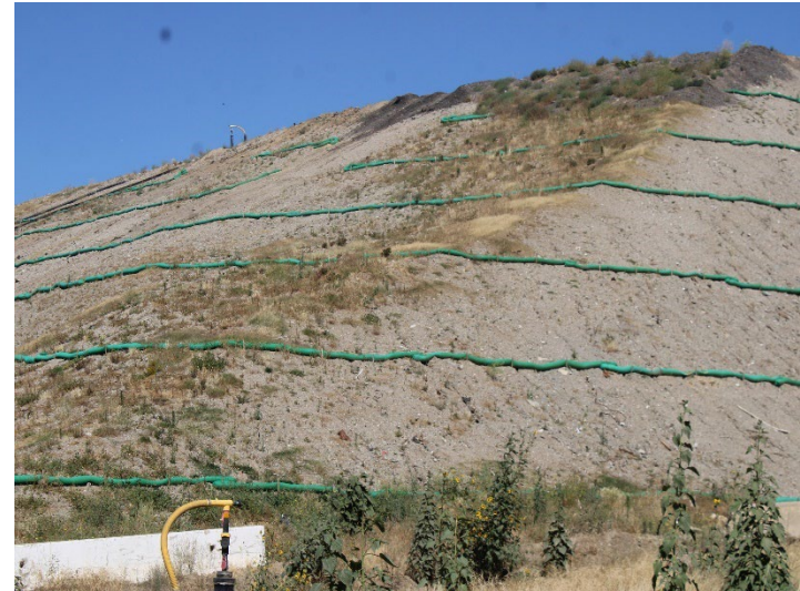
Photo 550: General Site: May 21, 2026
