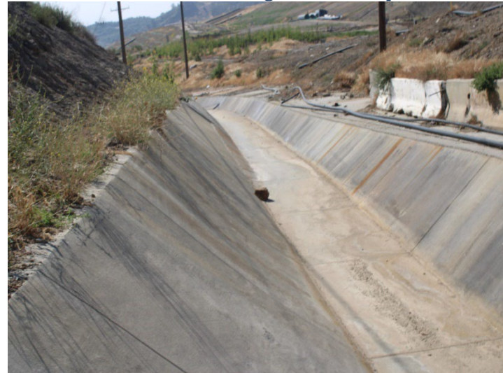
Photo 300: Eastside Drainage Channel: April 9, 2026
