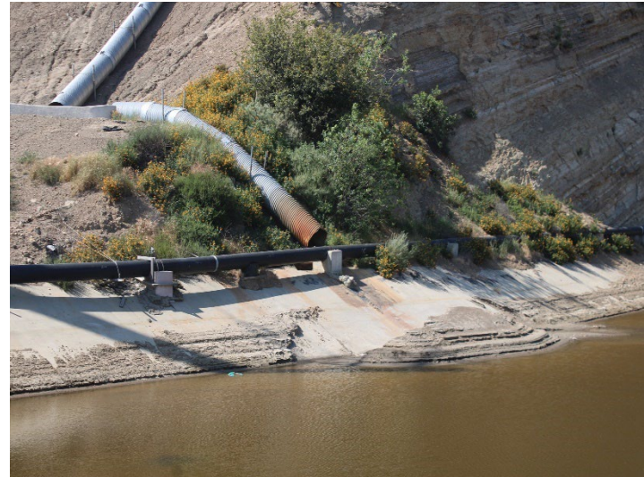
Photo 6: Basin A: April 9, 2026
