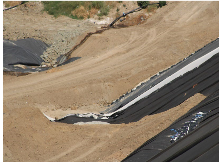
Photo 534: General Site: May 21, 2026
