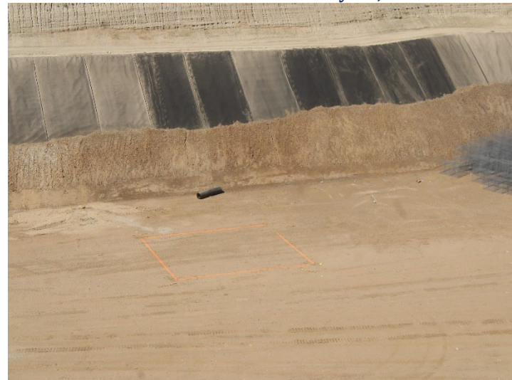
Photo 516: General Site: May 21, 2026
