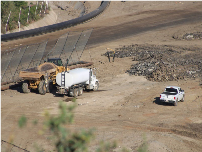
Photo 77: Working Area, CC-4 Part 4/5, CC-5A: April 9, 2026
