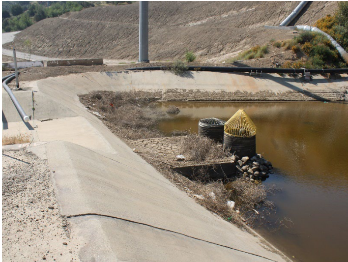
Photo 1: Basin A: April 9, 2026
