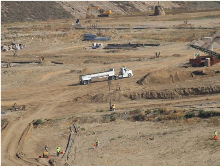
Photo 65: Working Area, CC-4 Part 3: June 11, 2026
