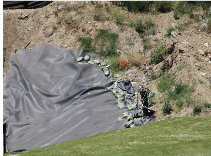
Photo 586: General Site: May 21, 2026
