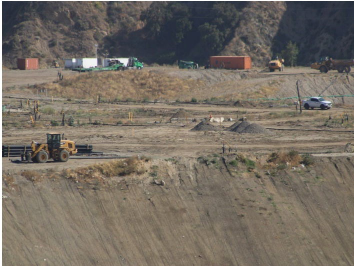
Photo 37: Working Area, CC4 Part 1/2: May 21, 2026
