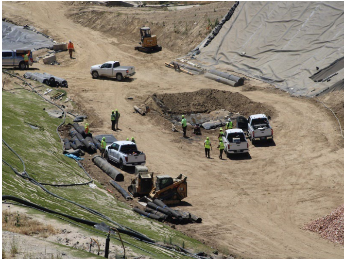
Photo 581: General Site: May 21, 2026
