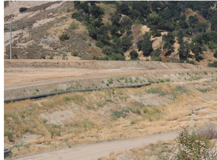
Photo 258: County Top Deck: June 11, 2026
