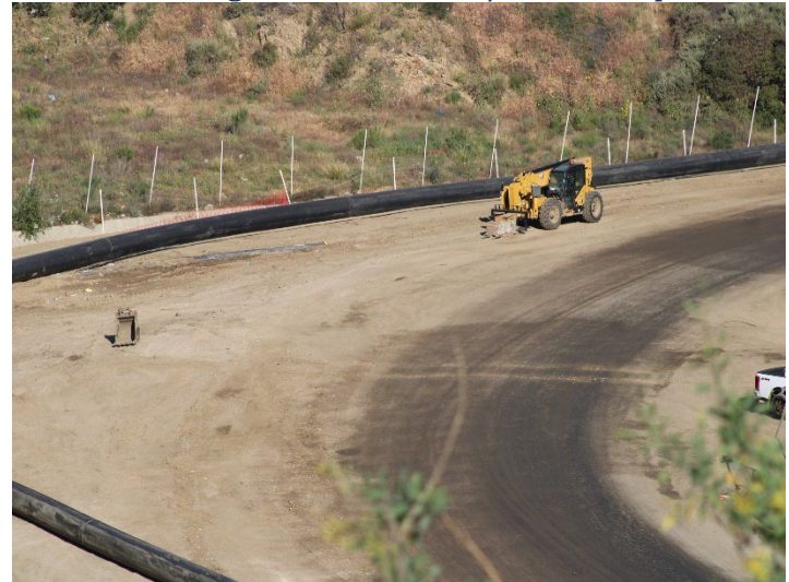
Photo 76: Working Area, CC-4 Part 4/5, CC-5A: April 9, 2026
