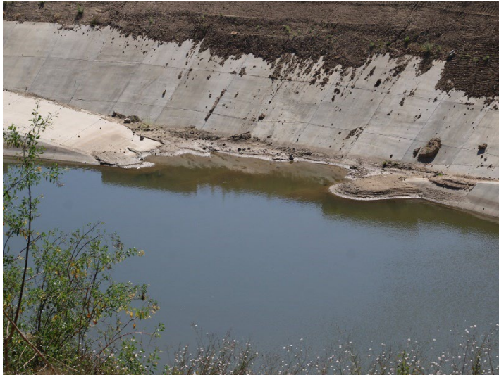
Photo 505: General Site: May 21, 2026
