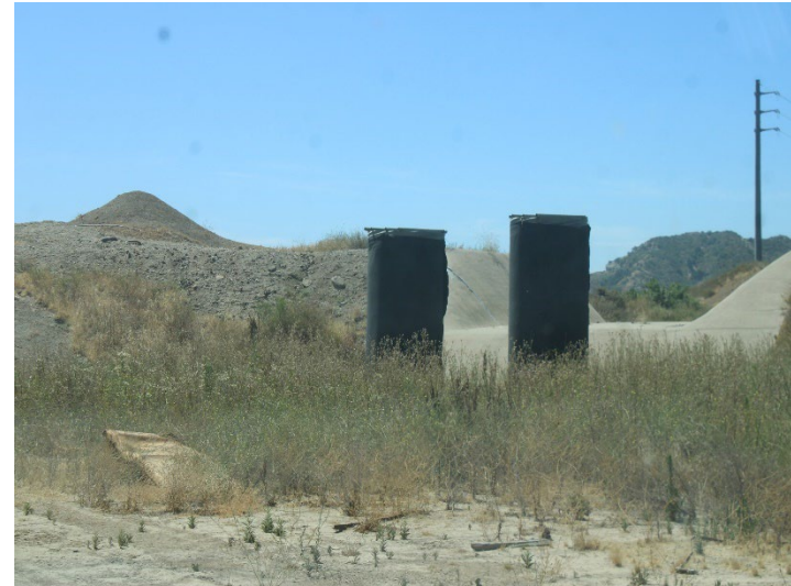
Photo 202: Basin D: June 11, 2026
