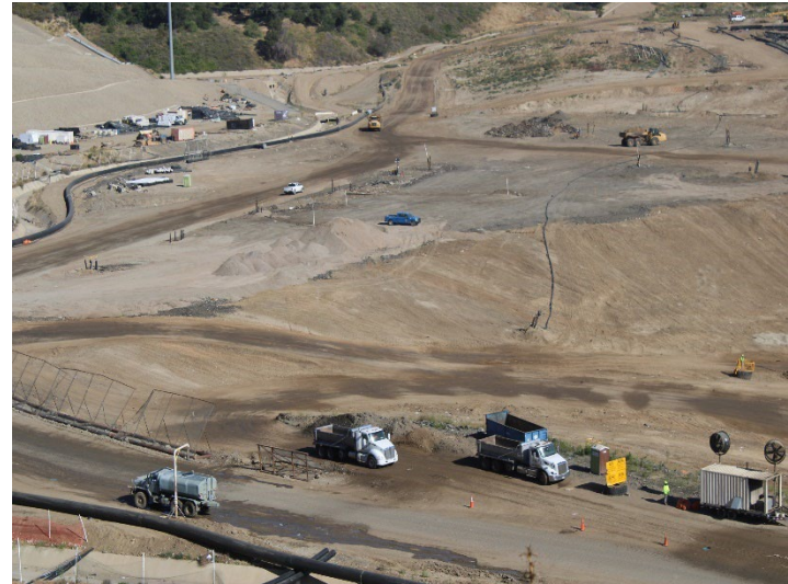
Photo 90: Working Area, CC-4 Part 4/5, CC-5A: May 21, 2026
