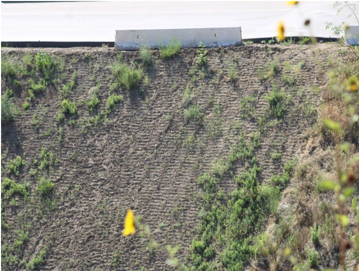
Photo 605: General Site: June 11, 2026
