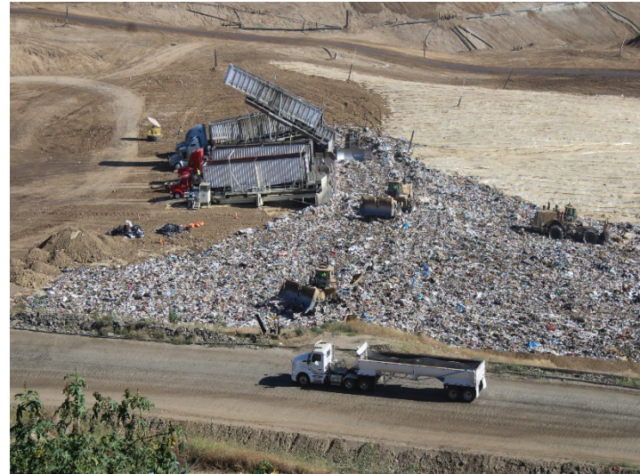
Photo 130: Working Area, CC-4 Part 4/5, CC-5A: June 11, 2026
