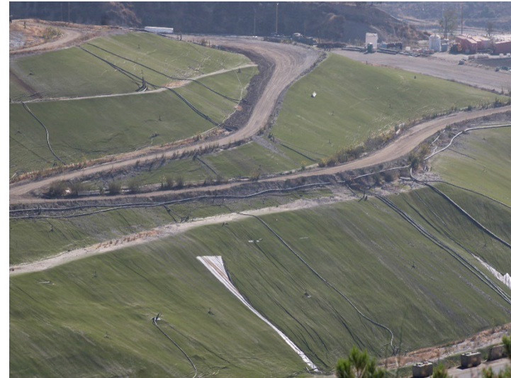
Photo 146: Closure Turf: June 11, 2026
