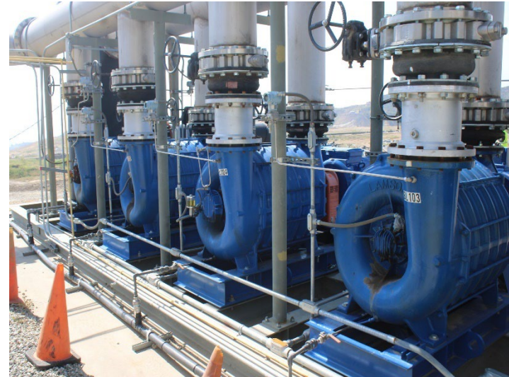
Photo 218: Flares 9, 10, 11 and Gas-to-Energy Facility: April 9, 2026
