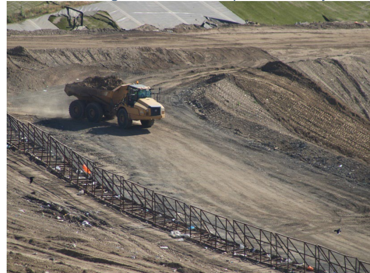
Photo 120: Working Area, CC-4 Part 4/5, CC-5A: May 21, 2026
