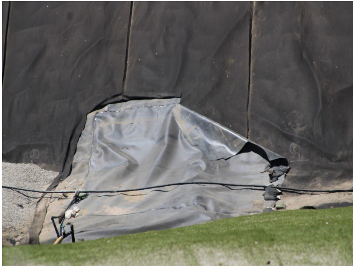
Photo 585: General Site: May 21, 2026
