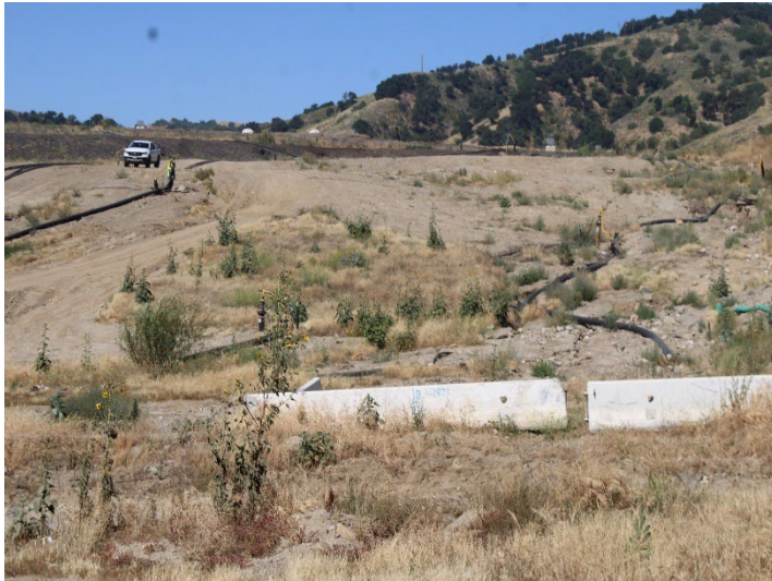
Photo 549: General Site: May 21, 2026
