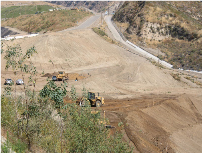
Photo 489: General Site: May 21, 2026
