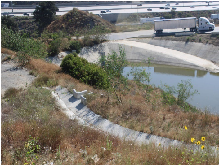
Photo 597: General Site: June 11, 2026
