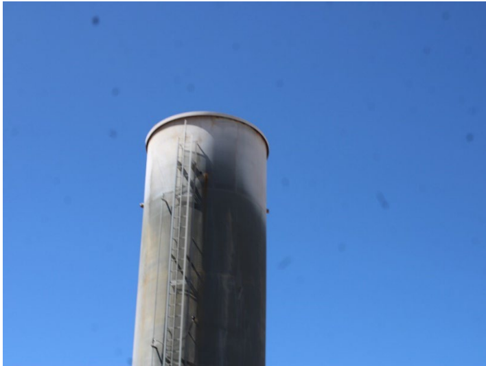
Photo 241: Flares 9, 10, 11 and Gas-to-Energy Facility: June 11, 2026
