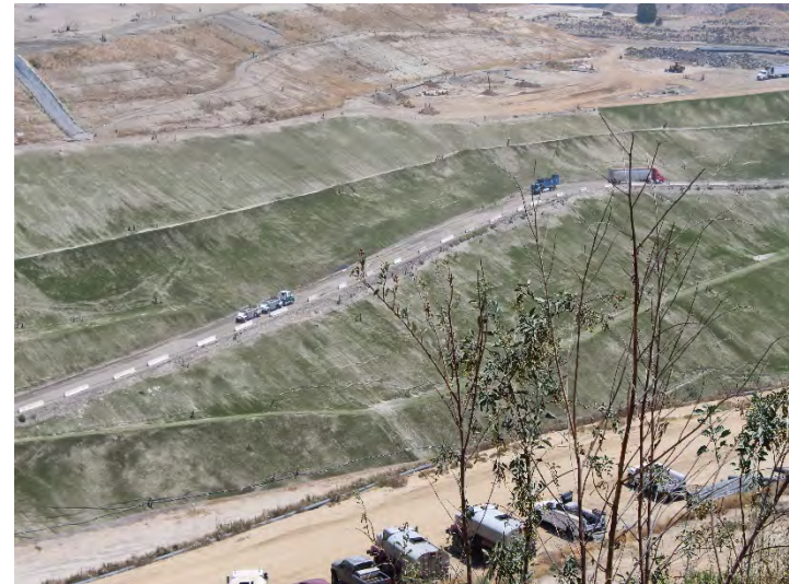
Photo 196: Closure Turf: June 23, 2020
