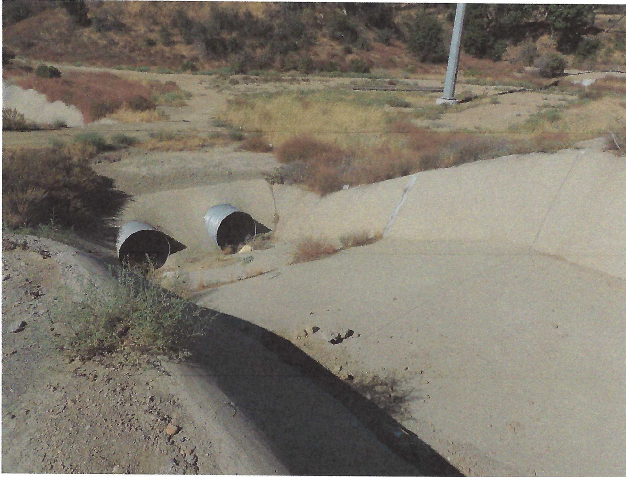
Figure 6: Vegetation in cracks at Basin D spillway
