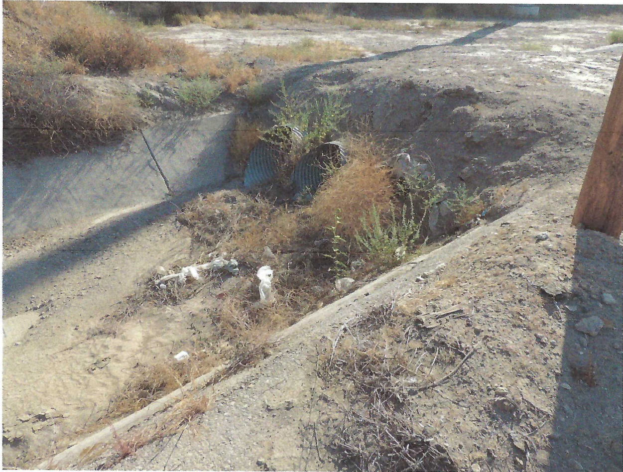
Figure 7: Soil and waste accumulated at intake pipe along channel
