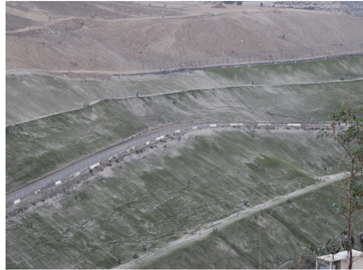
Photo 106: Closure Turf: September 19, 2022
