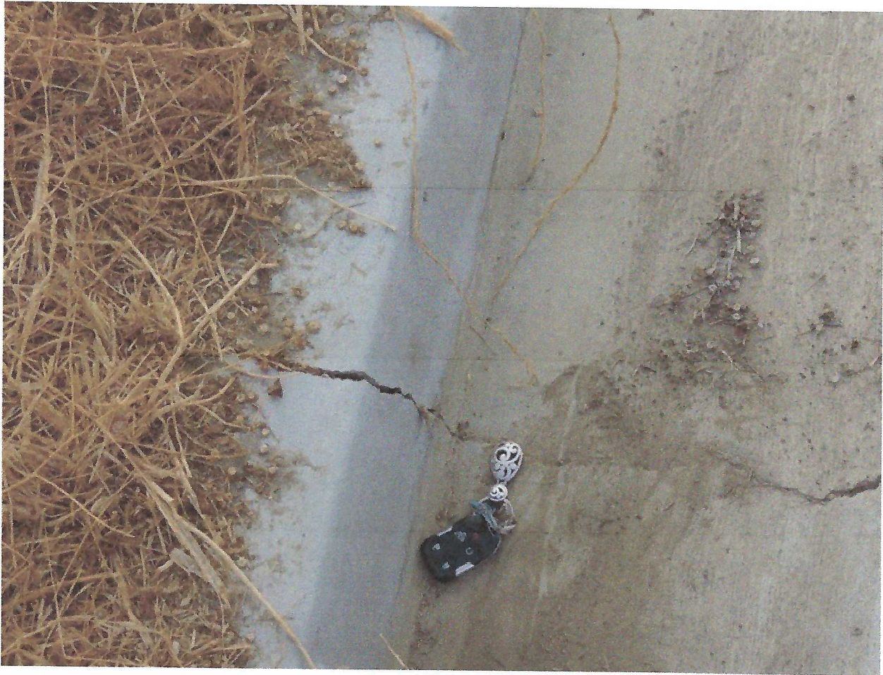
Figure 3: Crack in the curb at end of upper crack – slight vertical offset
