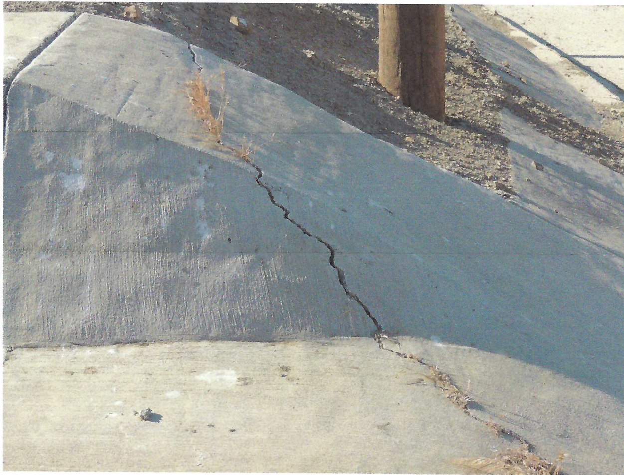
Figure 5: Cracks in spillway at Basin B
