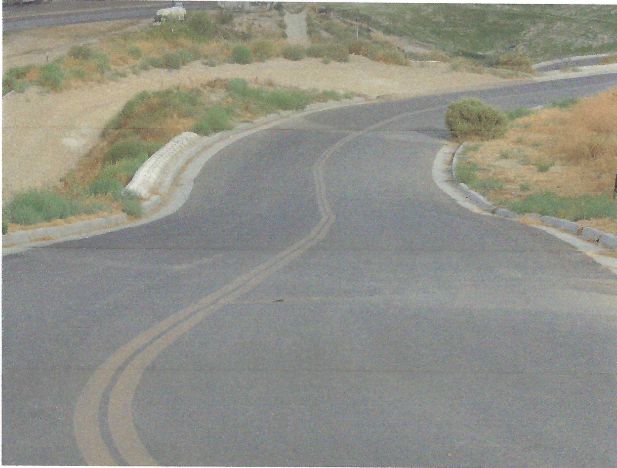
Figure 4 : Slight horizontal offset (yellow lines) at second crack on access road to the administration pad.
