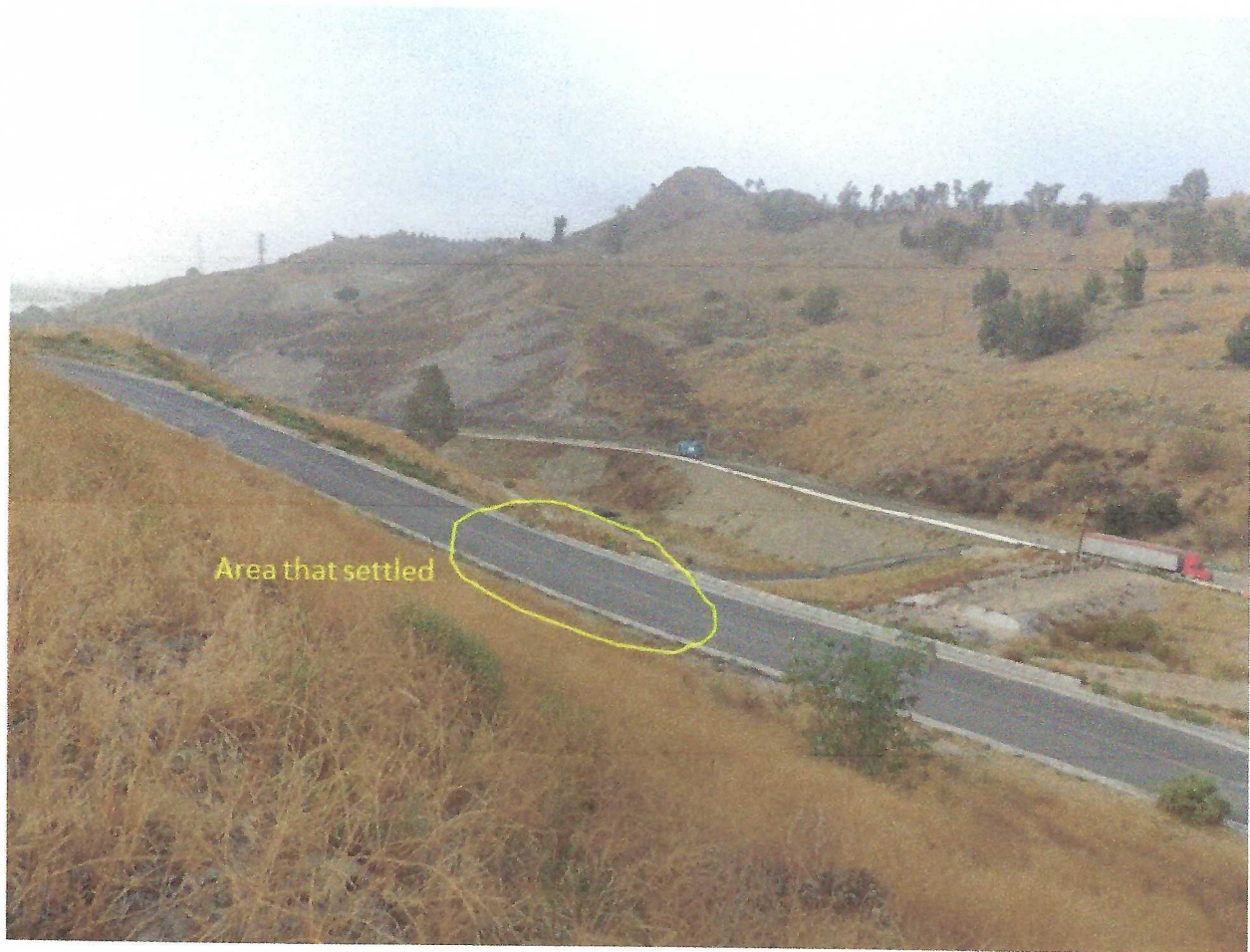
Figure 2 : Slight depression on the road to the administration pad
