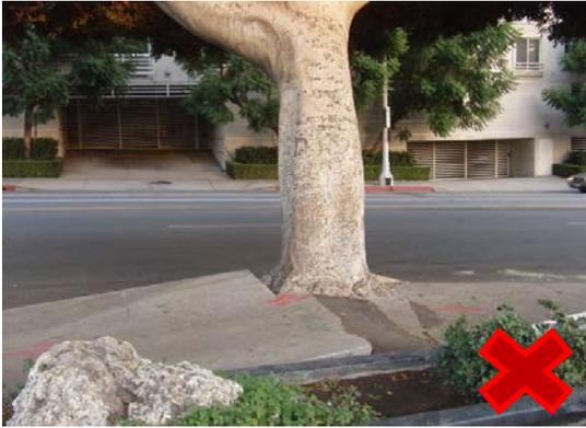
*Poor tree selection, placement, and maintenance can create conditions where tree roots can lift a sidewalk, creating a dangerous conditions and require expensive corrections.*
