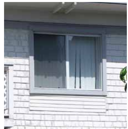
An inappropriately sized aluminum window diminishes the historic value of a house.
