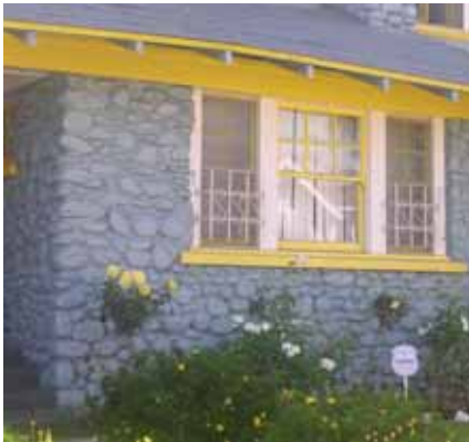
Stone and masonry should always be left to exhibit their natural finish qualities. Painting over the Arroyo stone on this house has muted the stone's texture.
