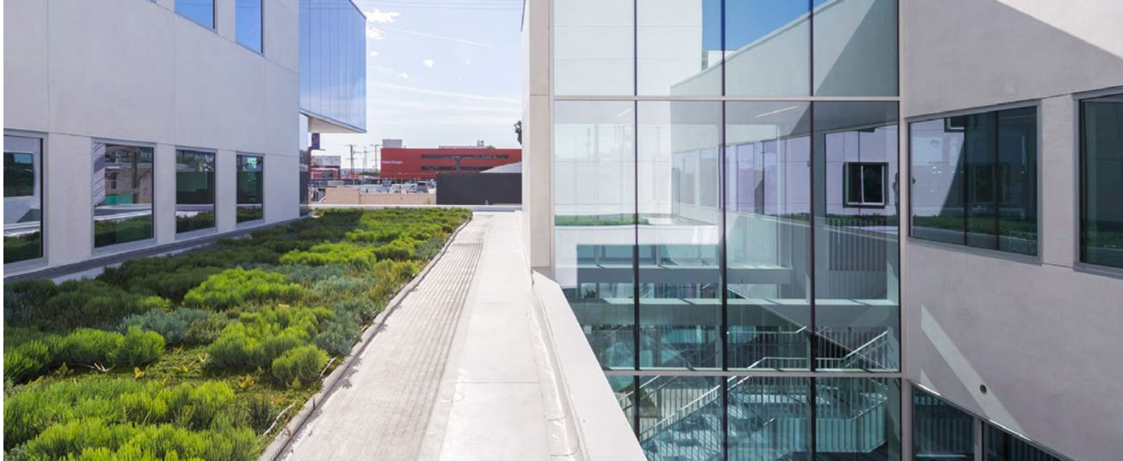
Above: Green roofs can improve stormwater, mitigate the urban heat island and increase urban biodiversity by providing habitat for wildlife. Photo Credit: KFA Architecture, Iwan Baan Photography
