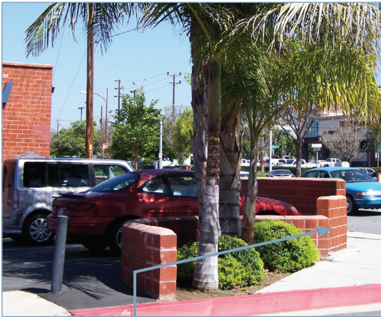
✓ Landscape wall provided to screen headlights
