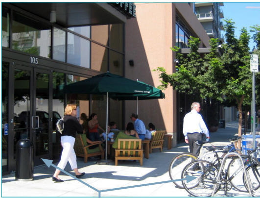
✓ Bicycle racks conveniently located near building entrance
