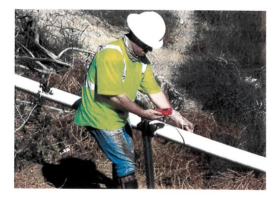
Once pressurized, the system is calibrated to insure even distribution of vapour throughout the covered area. This is accomplished by variation in pipe and outlet sizes.
