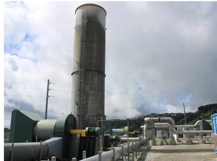
Photo 86: Flares 9, 10, 11 and Gas-to-Energy Facility: March 29, 2023
