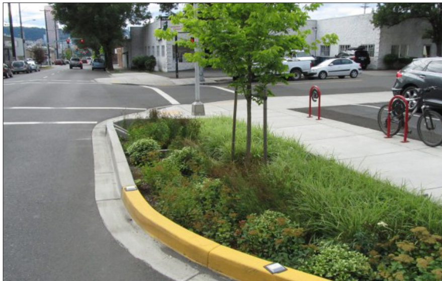
Corner curb extension with optional planting
