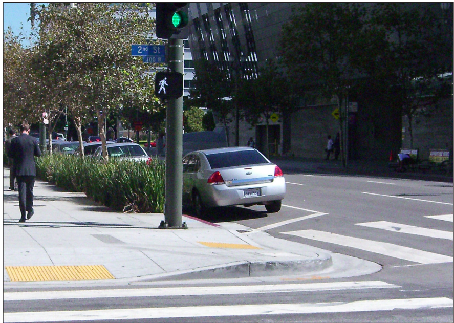
Smaller curb radii create more comfortable conditions for pedestrians.
