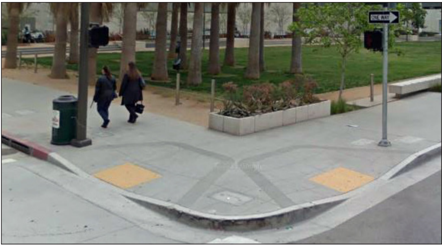
Dual curb ramps with detectable warning surfaces
