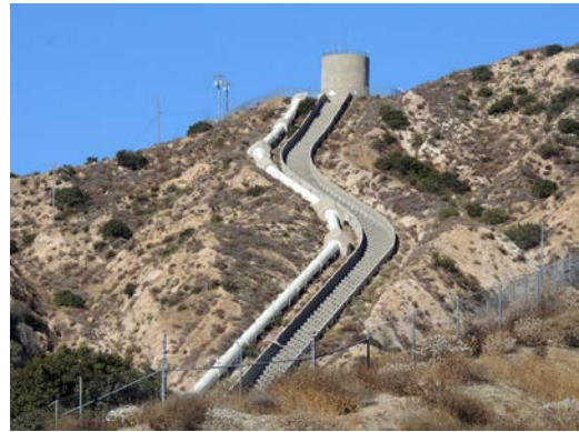
Address: 17001 Foothill Boulevard Name: Second Los Angeles Aqueduct Date: 1970
