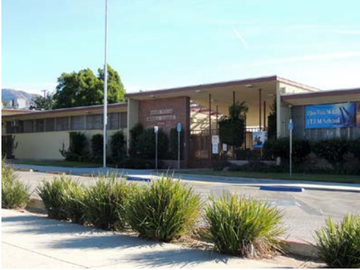
Address: 14600 Tyler Street Name: Olive Vista Middle School Date: 1958
