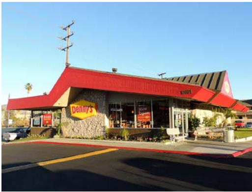
Address: 12861 Encinitas Avenue Name: Denny's Restaurant Architect: Colwell & Ray Date: 1968
