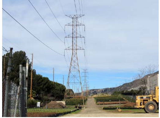
Location: Whitnall Highway Name: Whitnall Highway Power Corridor Date: 1927
