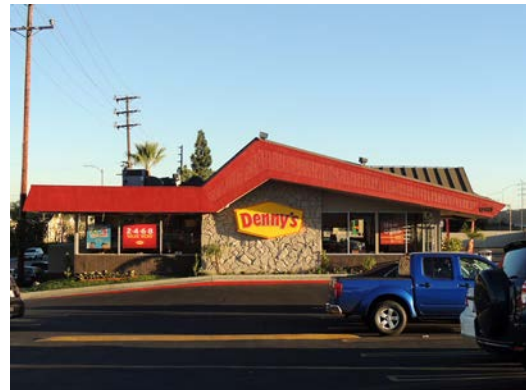
Address: 12861 Encinitas Avenue Name: Denny's Restaurant Architect: Colwell & Ray Date: 1968
