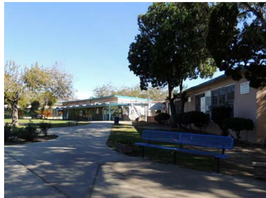
Address: 14500 Dyer Street Name: Dyer Street Elementary School Date: 1953
