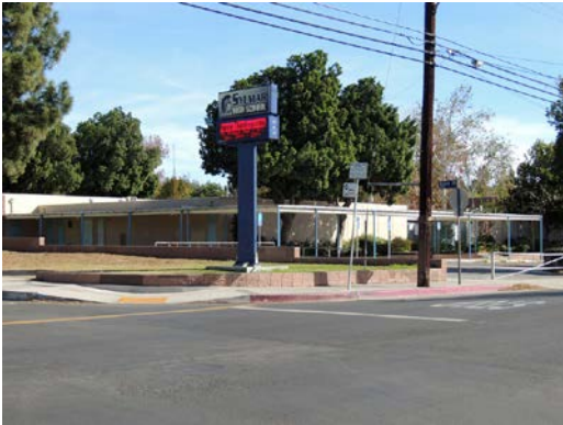
Address: 13050 Borden Avenue Name: Sylmar High School Date: 1961
