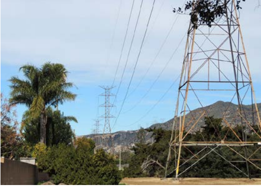
Location: Whitnall Highway Name: Whitnall Highway Power Corridor Date: 1927
