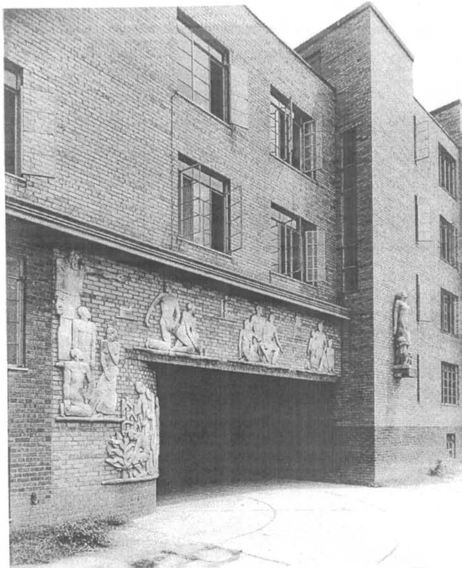
Figure 8 - Detail of building at Langston Terrace in Washington, D.C., a PWA direct-built public housing project completed in 1938, showing typical PWA-era details, including stripped, modern design, brick construction, and casement windows. This complex also featured a significant public art component, a terracotta frieze entitled "The Progress of the Negro Race." (National Register of Historic Places Nomination, 1986)
