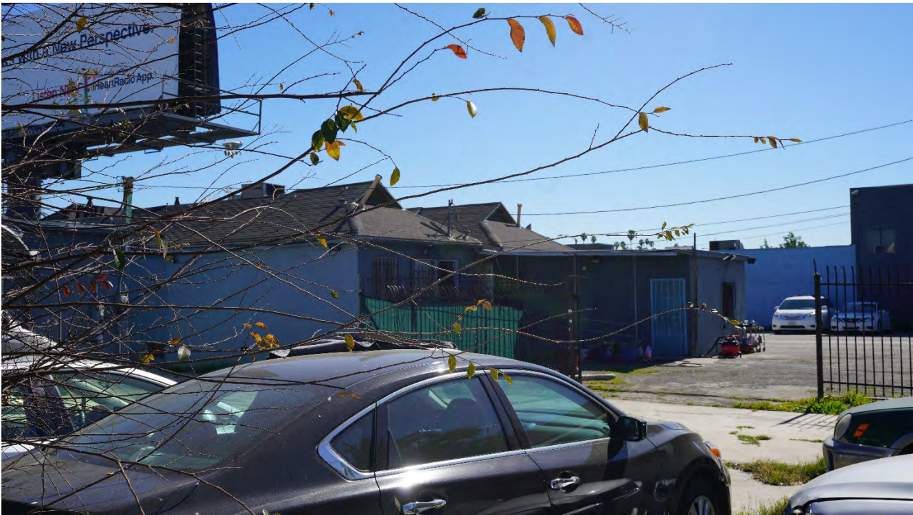
1025-1027 South Crenshaw Boulevard – Crenshaw Women’s Center West elevation Photograph taken: February 18, 2021
