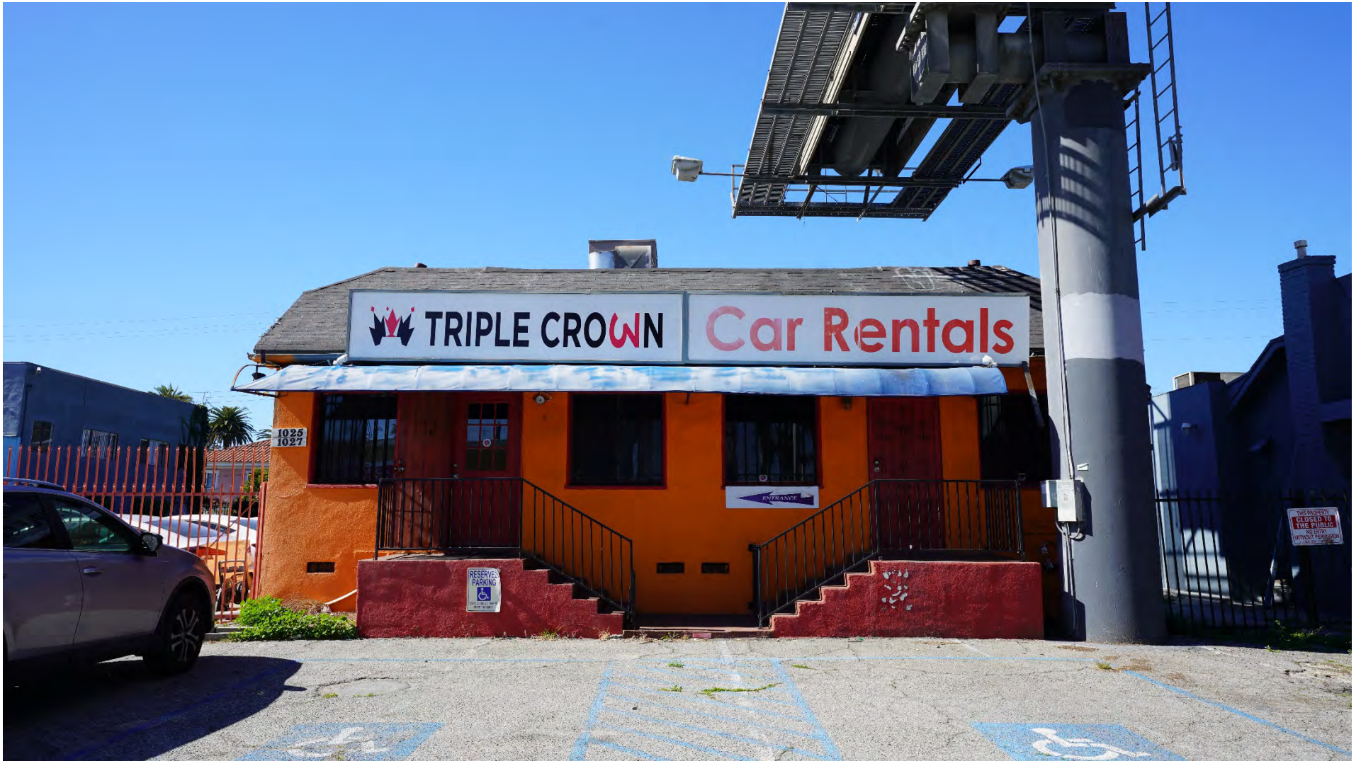
1025-1027 South Crenshaw Boulevard – Women’s Center Main east elevation Photograph taken: February 18, 2021
