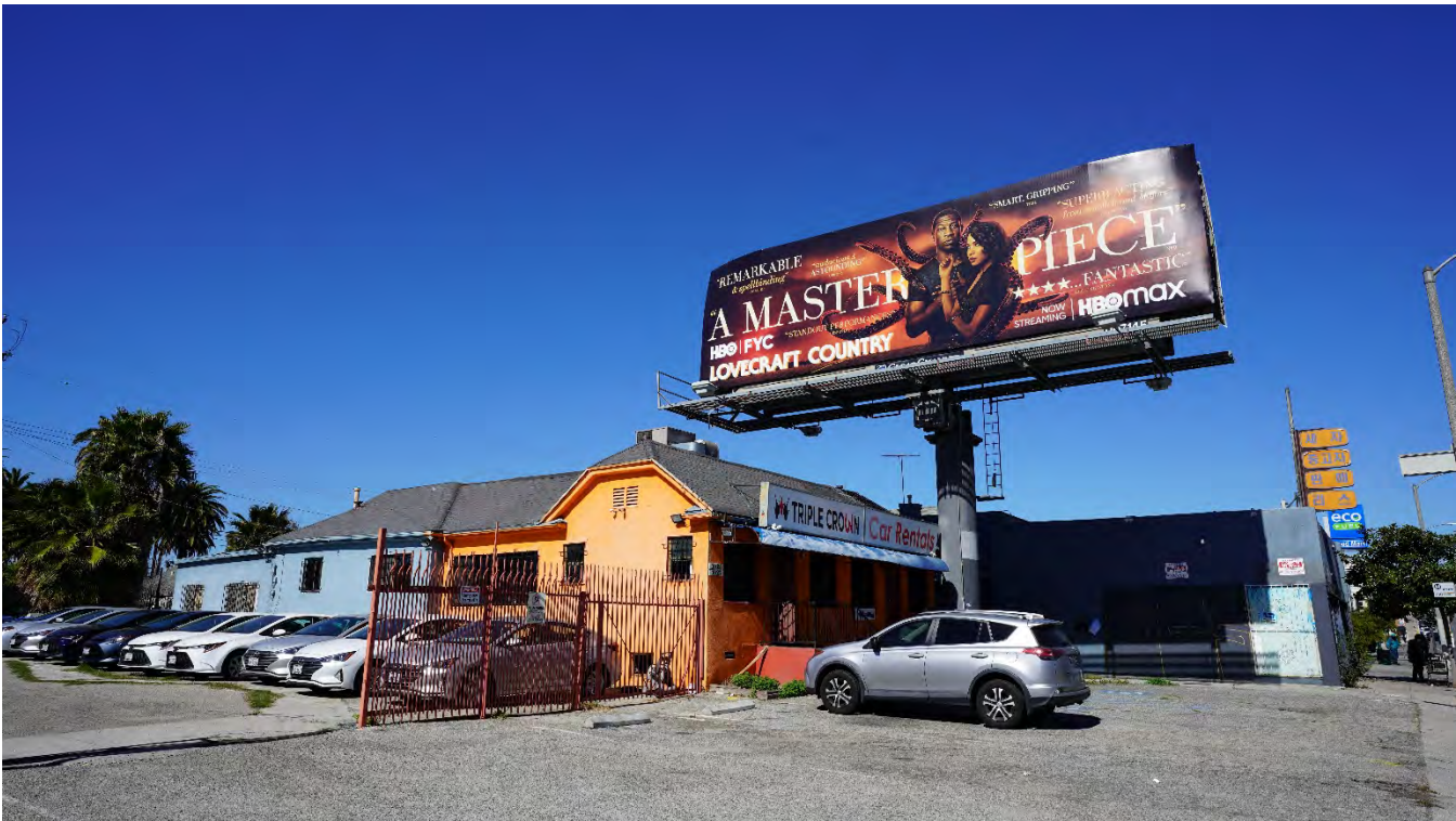
1025-1027 South Crenshaw Boulevard – Crenshaw Women’s Center Main east elevation, south elevation, and surrounding parking Photograph taken: February 18, 2021
