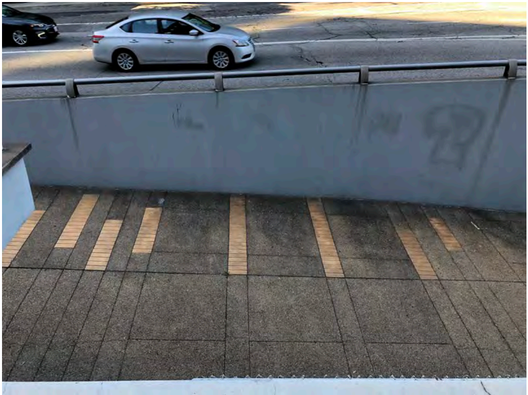
Sidewalk paving along 5th Street, view looking southwest.
