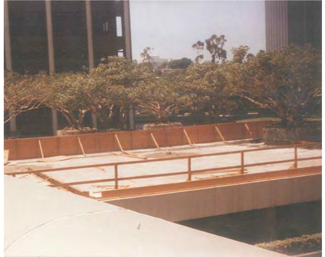
c1990, BEFORE Johnson Fain and Pereira Associates work
