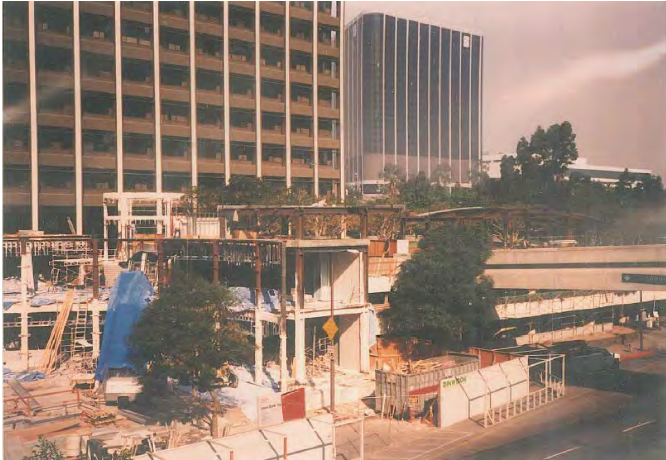
c1990, BEFORE Johnson Fain and Pereira Associates work
