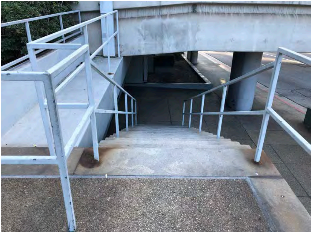
Staircase leading from southern plaza to Fifth Street, view looking southeast.
