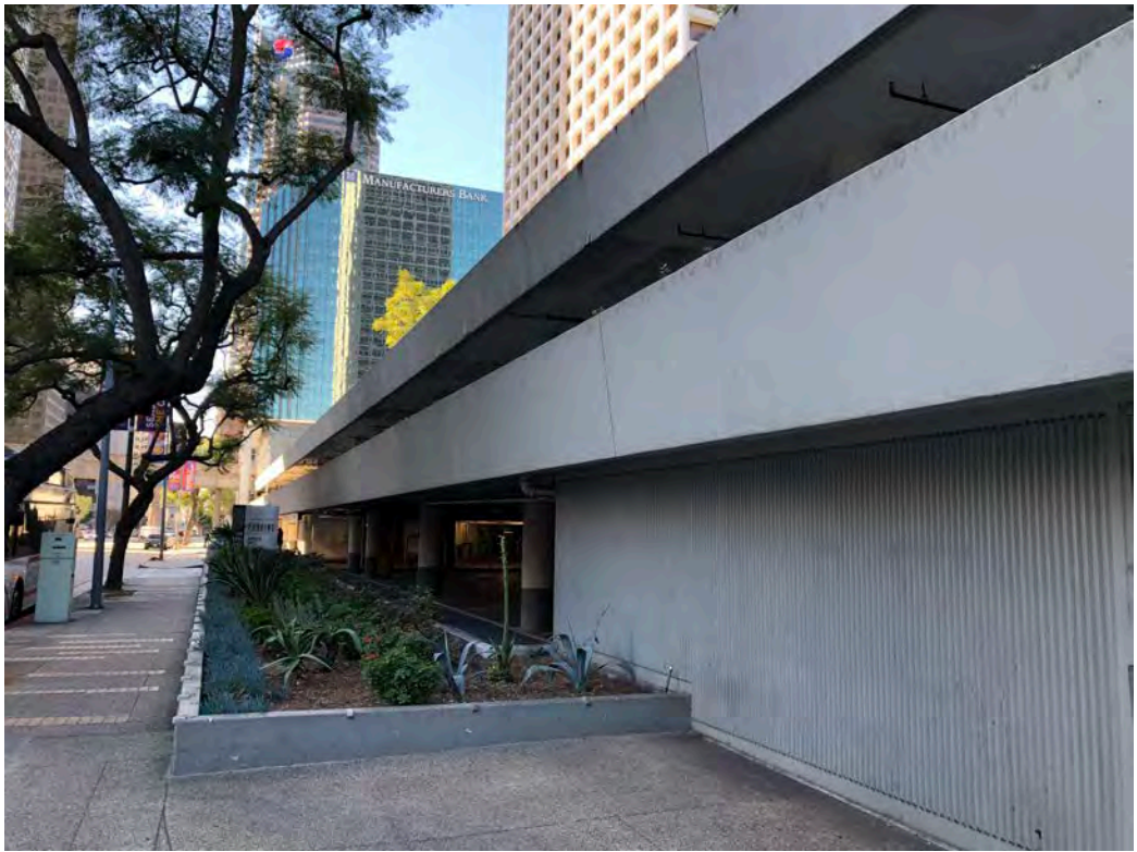
Parking garage, view looking southwest from South Figueroa Street.
