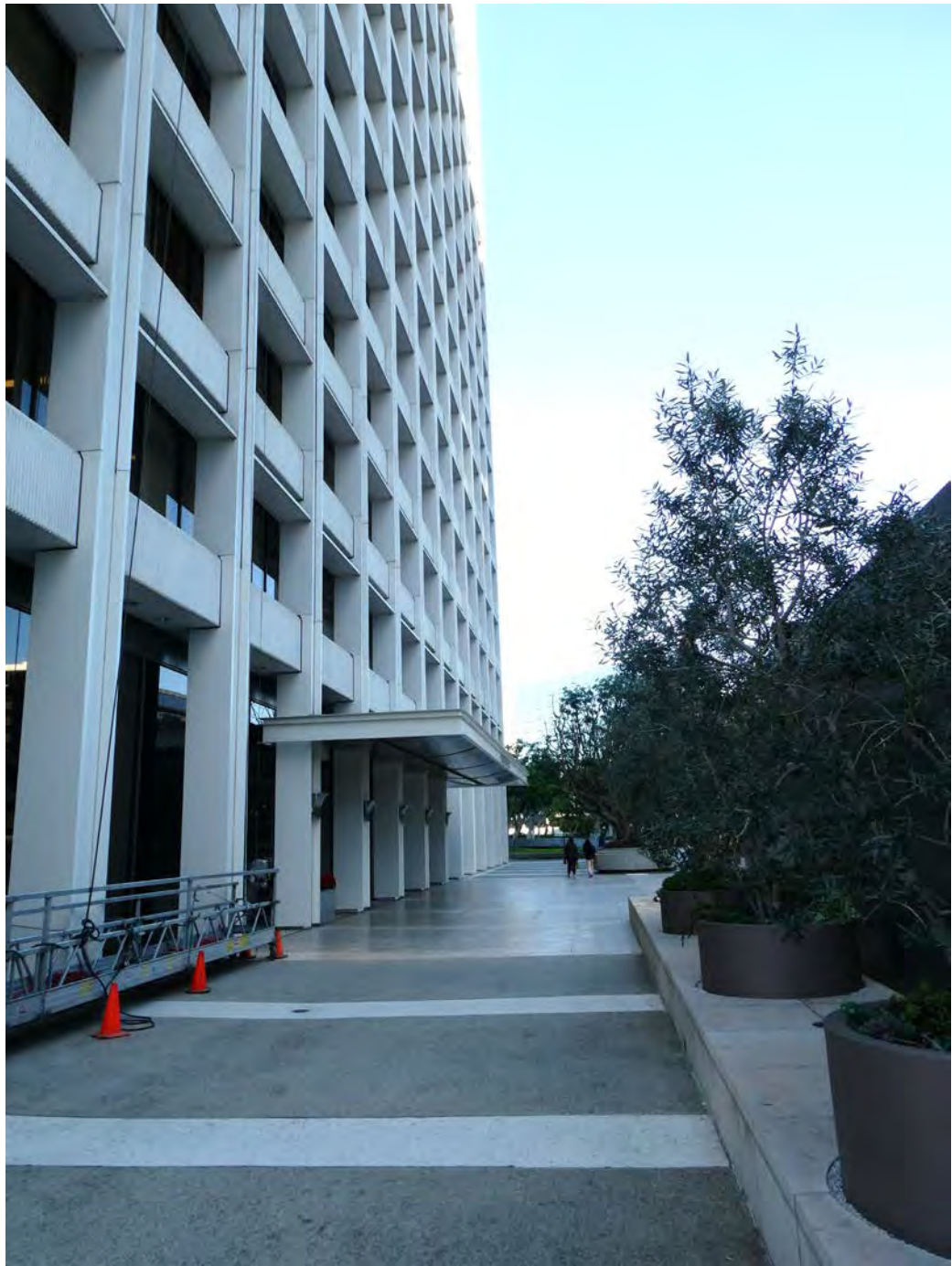
Southern plaza, view looking northeast.
