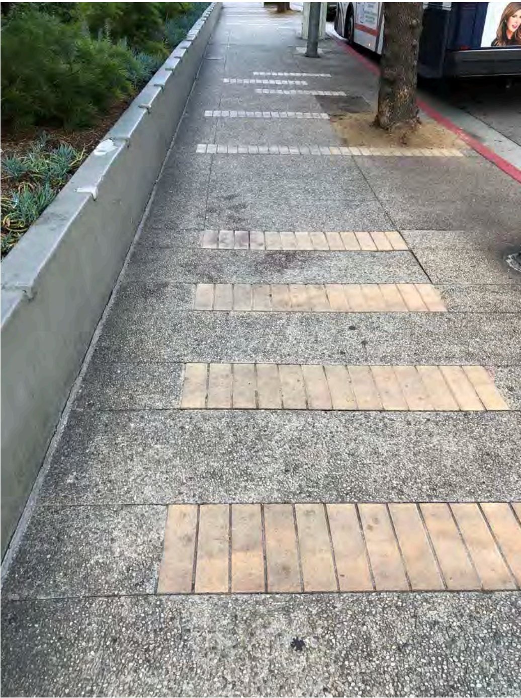
Sidewalk paving along South Figueroa Street, view looking northeast.
