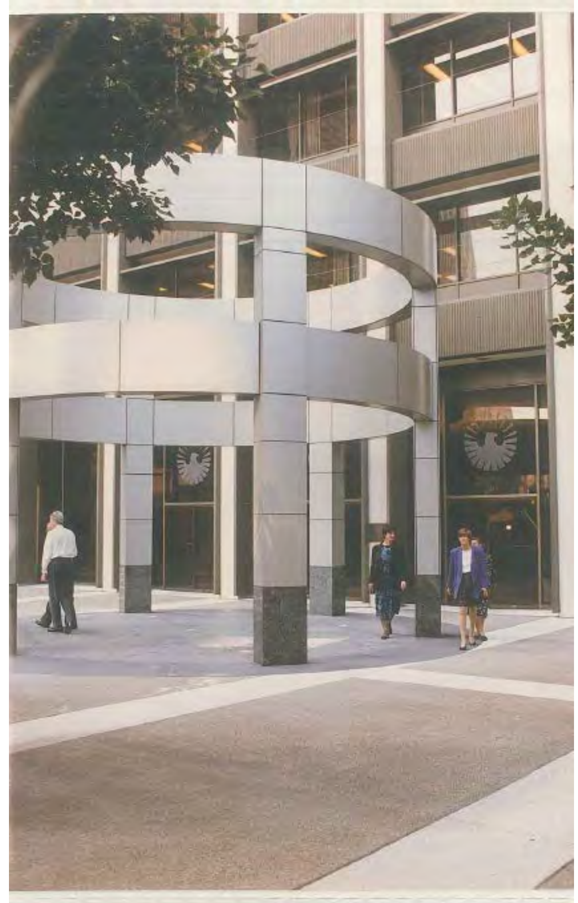
c1990, BEFORE Johnson Fain and Pereira Associates work
