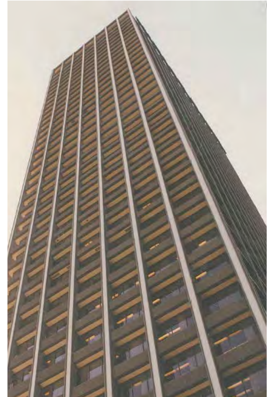
c1990, BEFORE Johnson Fain and Pereira Associates work
