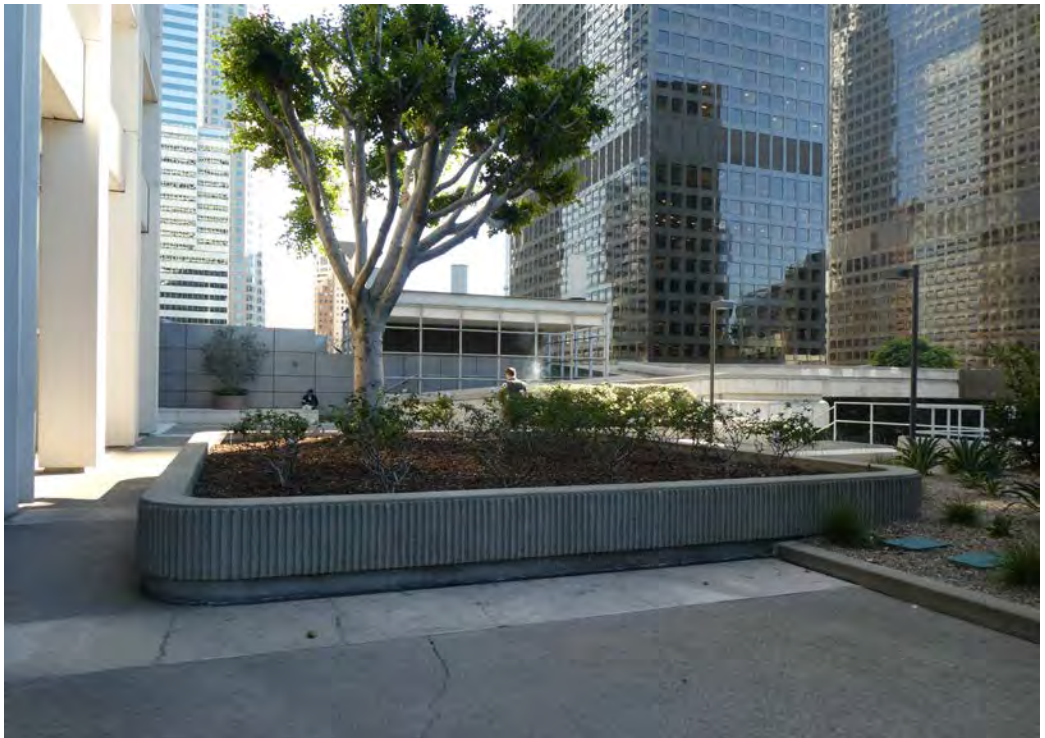
Planter detail, western plaza, view looking southeast.
