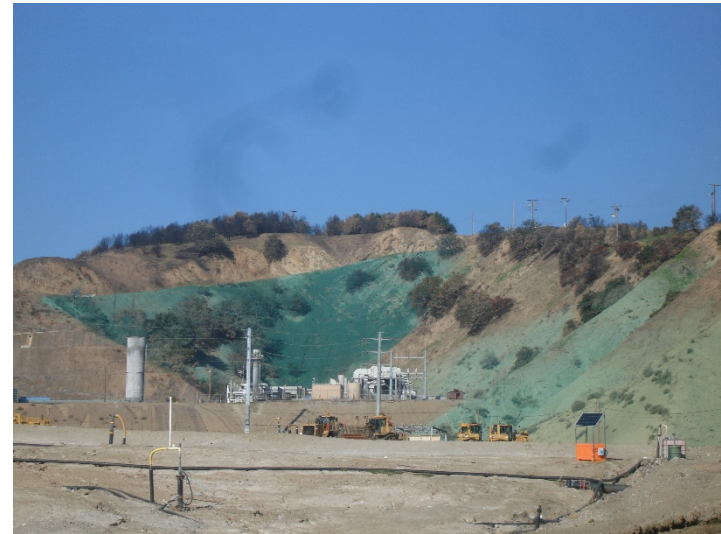
Photo 224: Canyon Eastside Hydroseed Slopes: January 13, 2020
