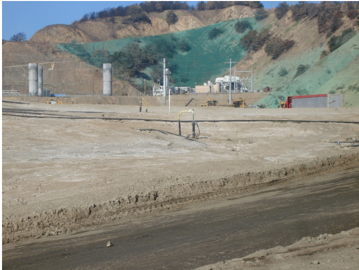
Photo 221: Canyon Eastside Hydroseed Slopes: January 13, 2020
