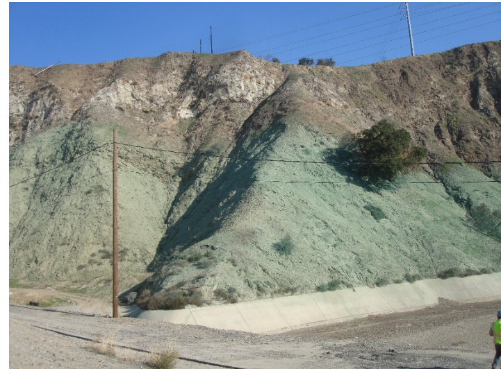
Photo 232: East Ridgeline Slopes Hydroseeding: January 13, 2020
