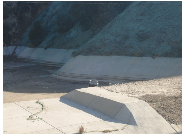
Photo 212: Basin B High Flow Outlet Concrete Cracks: January 13, 2020
