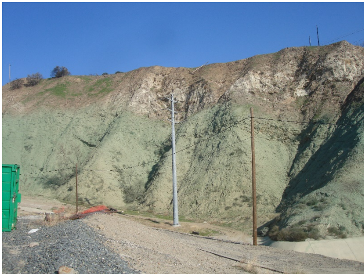
Photo 231: East Ridgeline Slopes Hydroseeding: January 13, 2020
