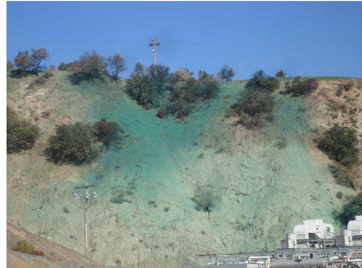
Photo 222: Canyon Eastside Hydroseed Slopes: January 13, 2020
