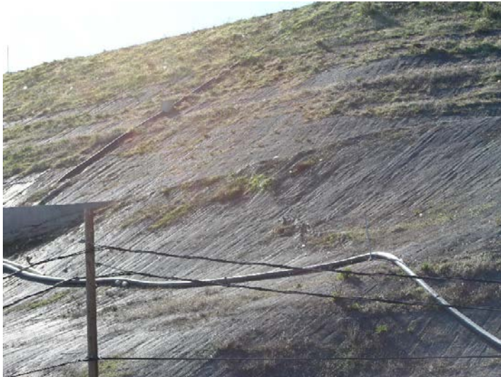
Photo 129: Old City South Stockpiled Soil Slump: February 26, 2020
