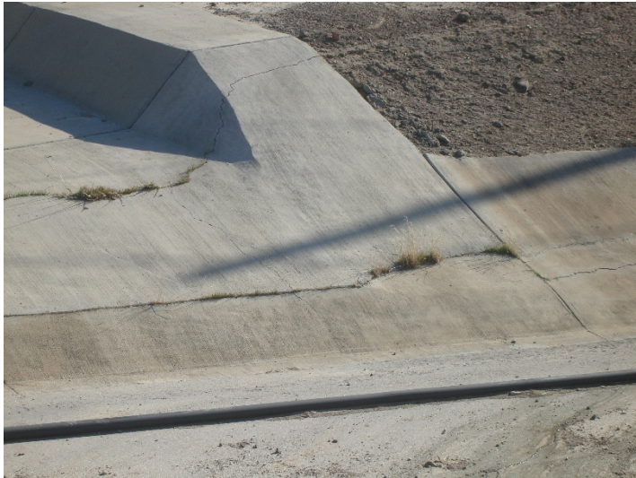
Photo 213: Basin B High Flow Outlet Concrete Cracks: January 13, 2020
