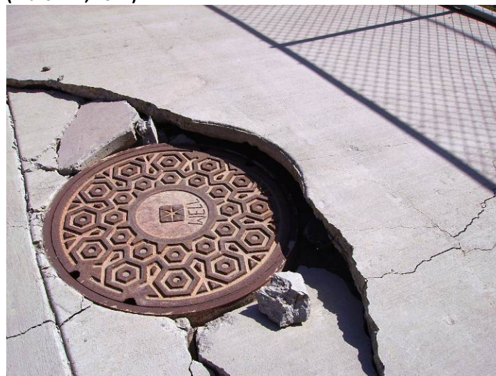
Photo 20: M-4.3.4.1 – 43 Cracked Concrete at Main Basin (March 14, 2012)
