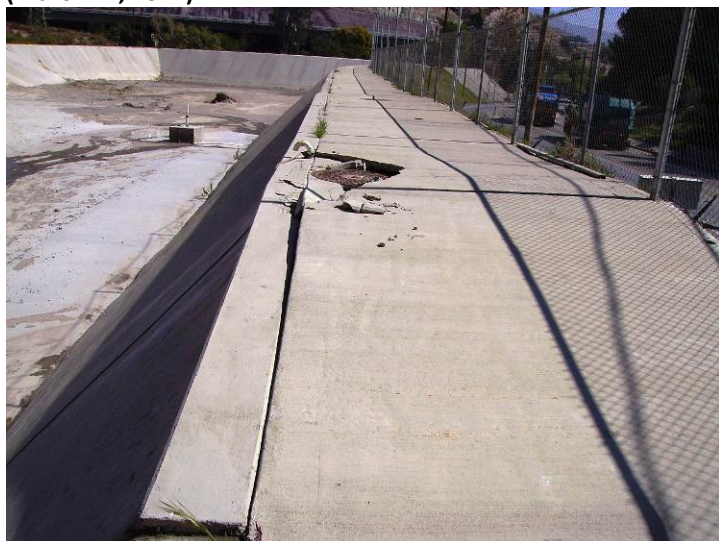
Photo 19: M-4.3.4.1 – 43 Cracked Concrete at Main Basin (March 14, 2012)
