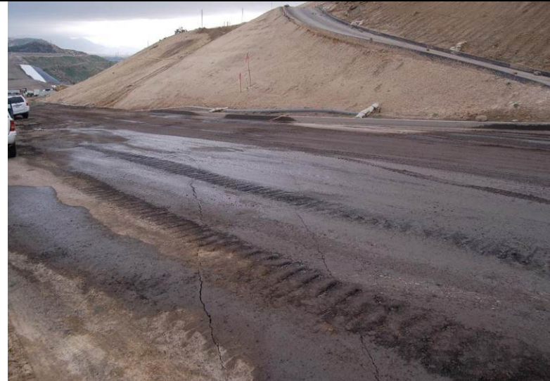
Photo 2: Q.C.3.g February Landslide Cracks - Access Road (February 15, 2012)
