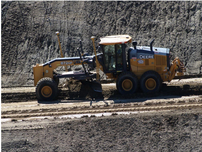
Photo 389: Road Realignment: April 16, 2024
