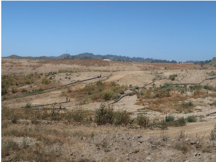
Photo 349: General Site: June 11, 2024
