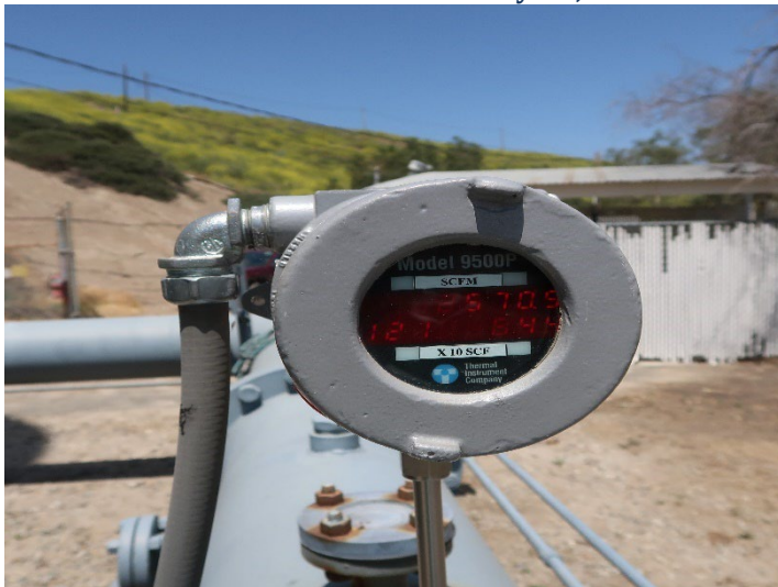
Photo 335: General Site: May 21, 2024
