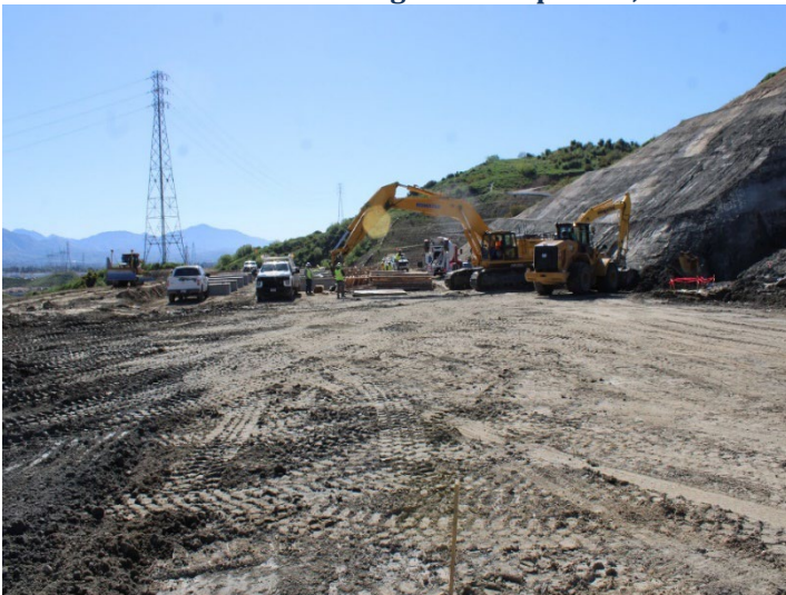
Photo 367: Road Realignment: April 16, 2024
