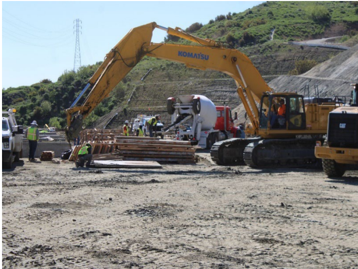
Photo 369: Road Realignment: April 16, 2024
