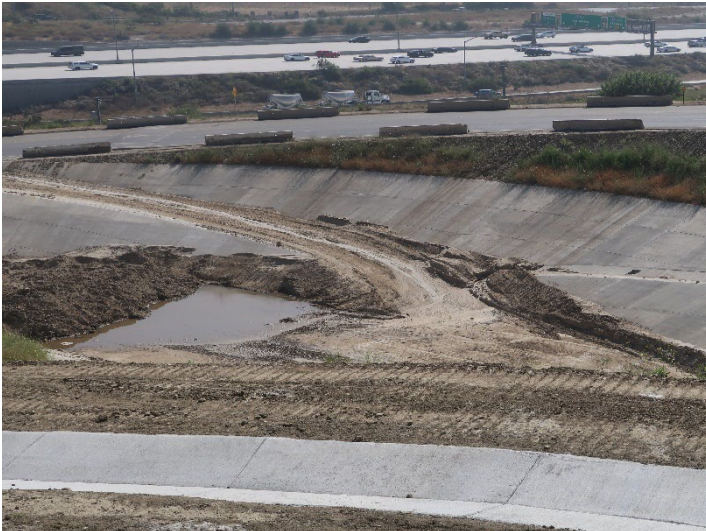
Photo 433: Road Realignment: June 11, 2024
