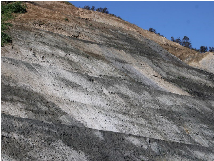
Photo 393: Road Realignment: April 16, 2024
