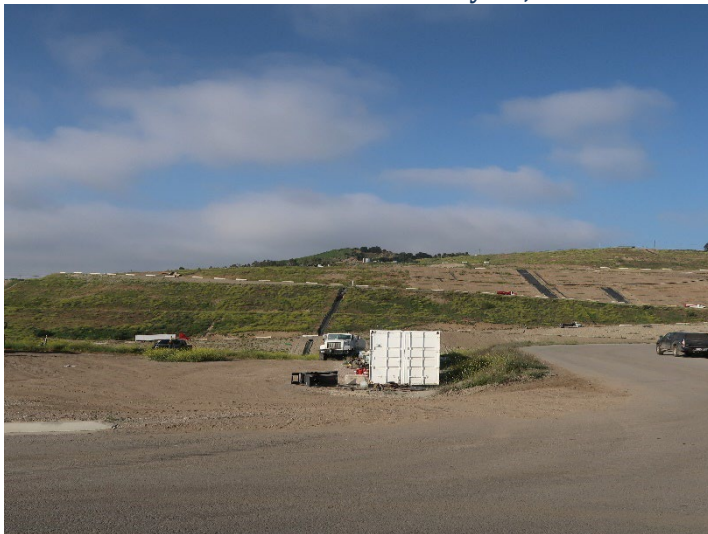
Photo 307: General Site: May 21, 2024
