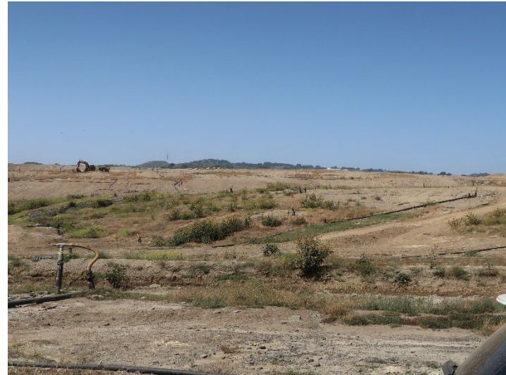
Photo 314: General Site: May 21, 2024
