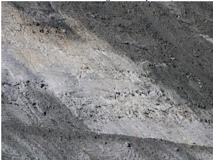
Photo 403: Road Realignment: April 16, 2024
