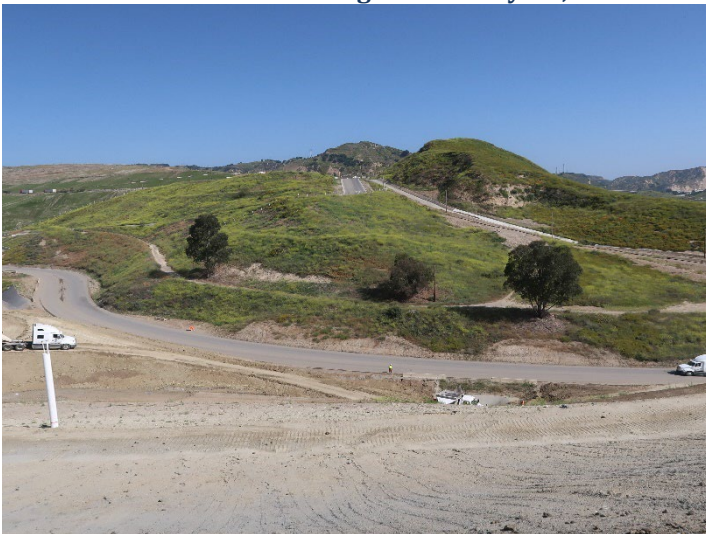
Photo 419: Road Realignment: May 21, 2024
