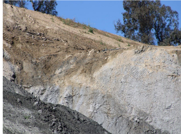
Photo 406: Road Realignment: April 16, 2024
