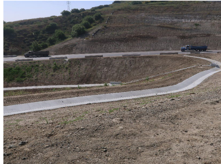
Photo 430: Road Realignment: June 11, 2024
