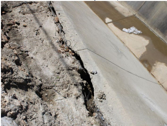
Photo 135: Eastside Drainage Channel: April 16, 2024
