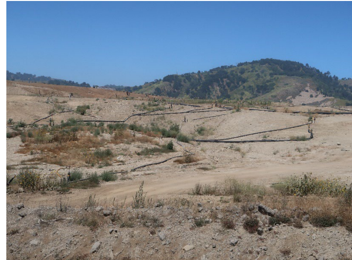
Photo 350: General Site: June 11, 2024
