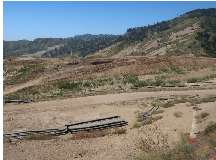
Photo 114: County Top Deck: June 11, 2024
