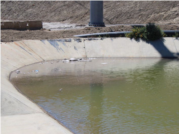
Photo 5: Basin A: April 16, 2024
