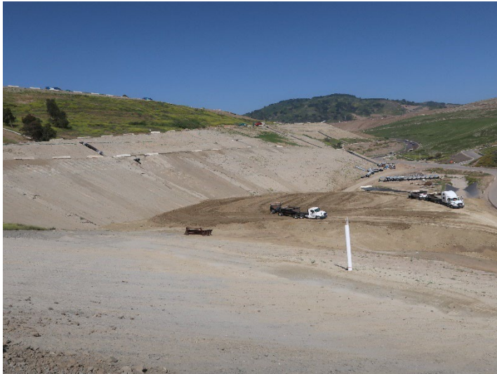
Photo 421: Road Realignment: May 21, 2024
