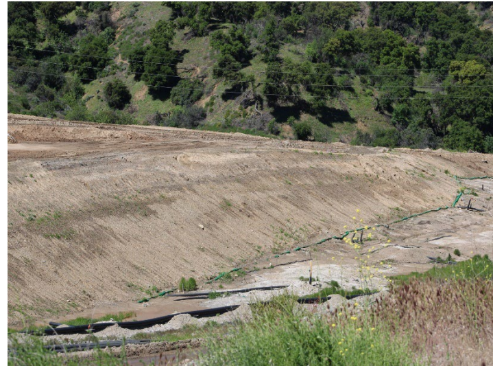
Photo 110: County Top Deck: April 16, 2024
