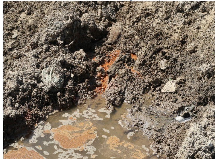
Photo 344: General Site: June 11, 2024
