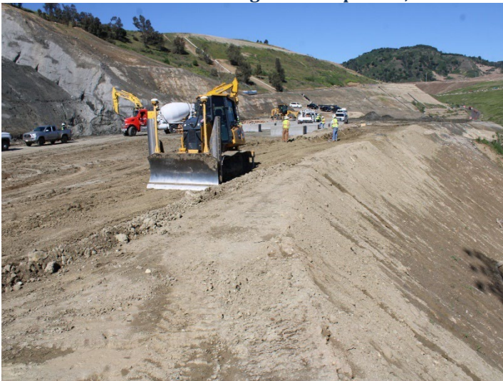
Photo 395: Road Realignment: April 16, 2024
