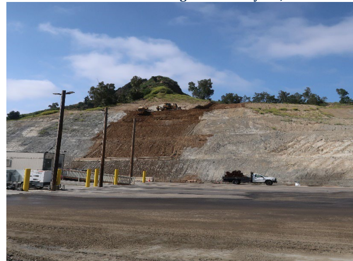
Photo 416: Road Realignment: May 21, 2024
