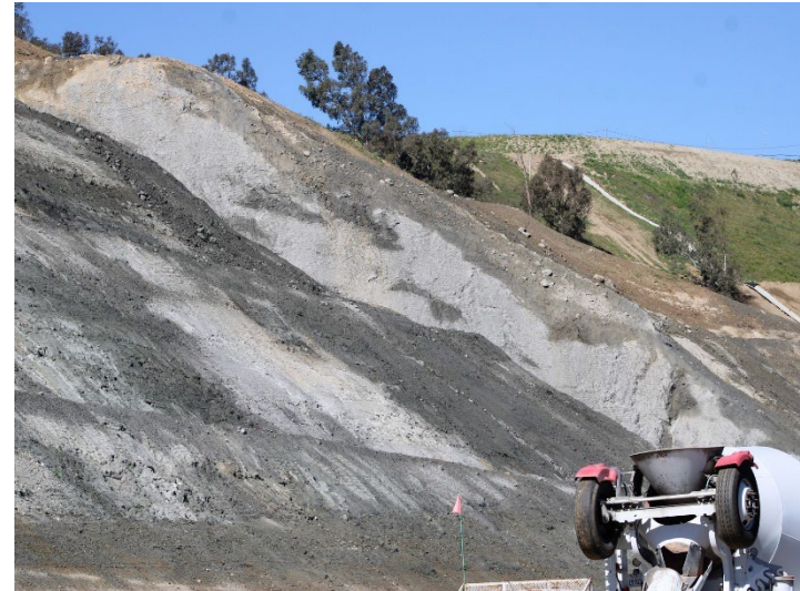
Photo 394: Road Realignment: April 16, 2024
