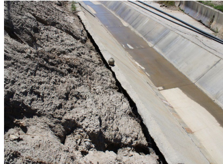
Photo 138: Eastside Drainage Channel: April 16, 2024
