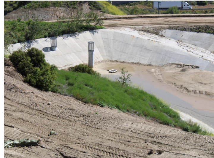
Photo 384: Road Realignment: April 16, 2024
