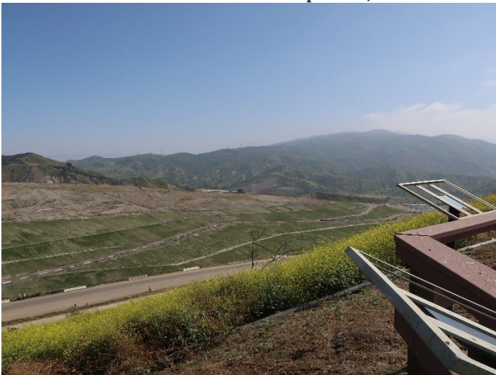
Photo 71: Closure Turf: May 21, 2024
