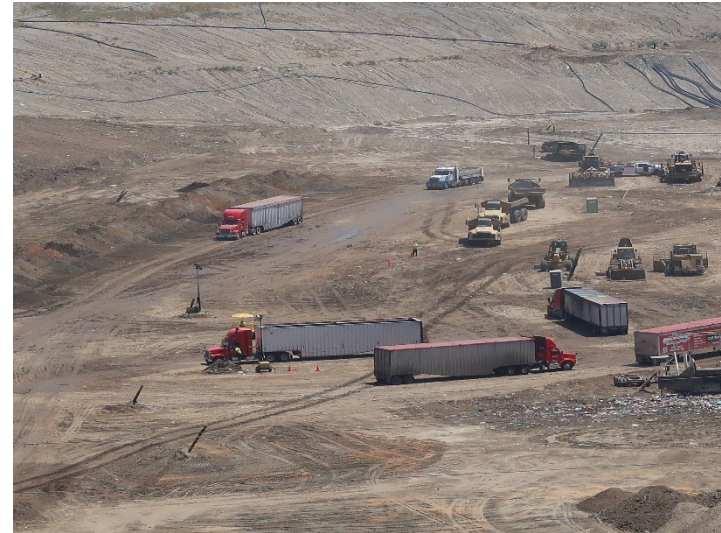
Photo 30: Working Area, CC4 Part 3: May 21, 2024
