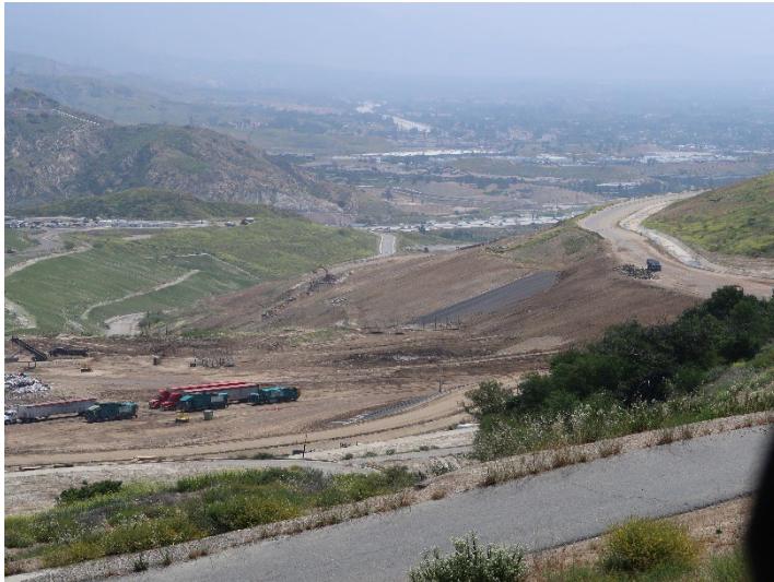
Photo 29: Working Area, CC4 Part 3: May 21, 2024
