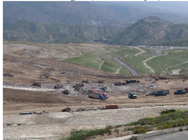
Photo 28: Working Area, CC4 Part 3: May 21, 2024
