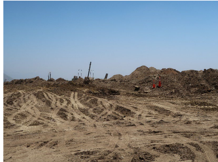
Photo 118: County Top Deck: June 11, 2024
