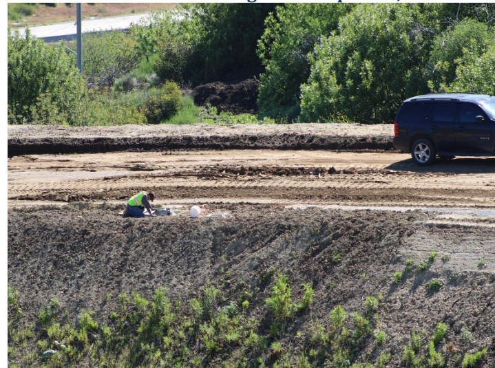
Photo 388: Road Realignment: April 16, 2024
