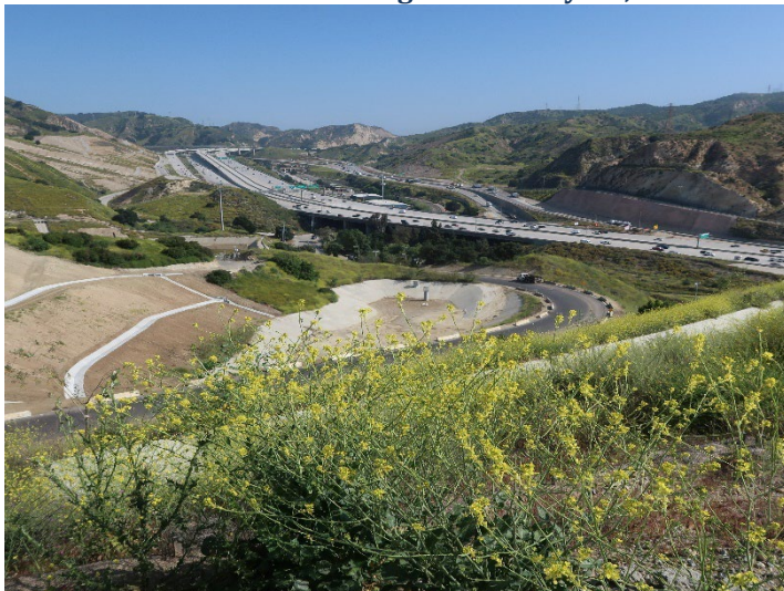
Photo 415: Road Realignment: May 21, 2024
