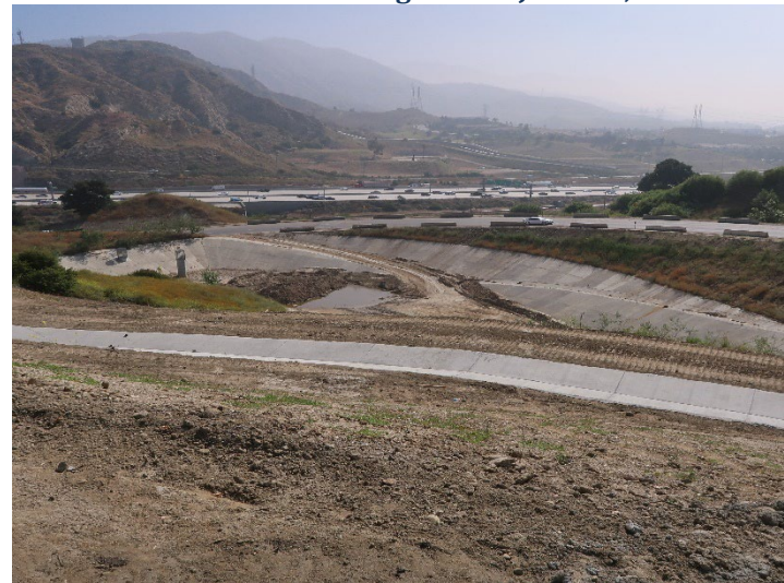
Photo 436: Road Realignment: June 11, 2024
