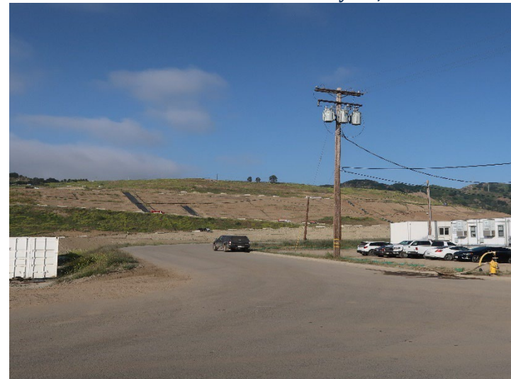
Photo 308: General Site: May 21, 2024
