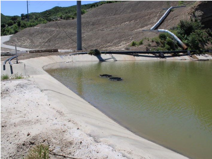
Photo 1: Basin A: April 16, 2024
