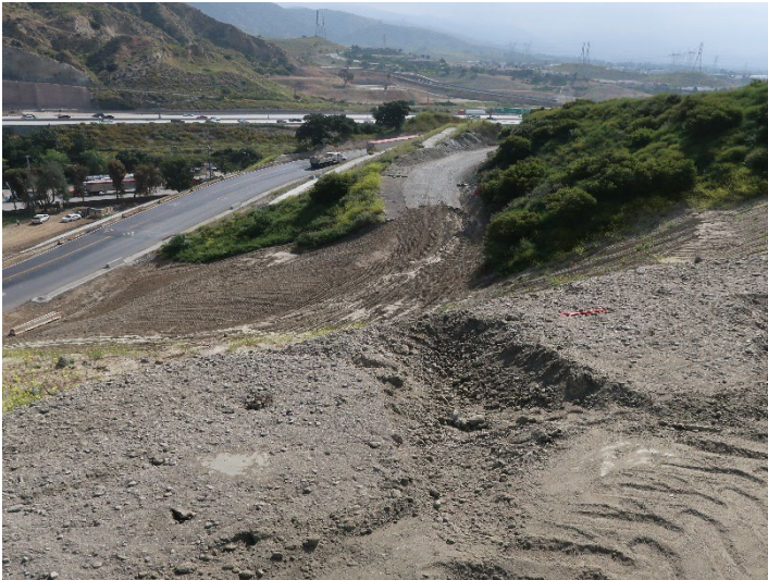
Photo 417: Road Realignment: May 21, 2024
