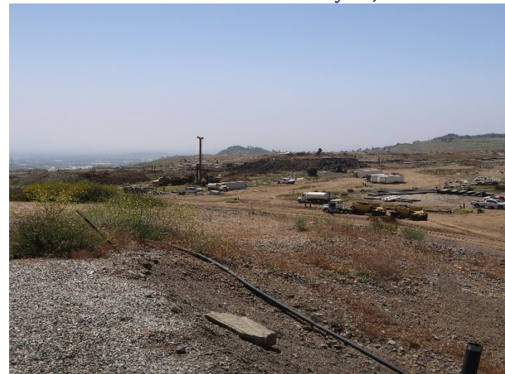
Photo 320: General Site: May 21, 2024
