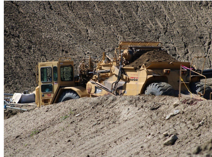
Photo 390: Road Realignment: April 16, 2024
