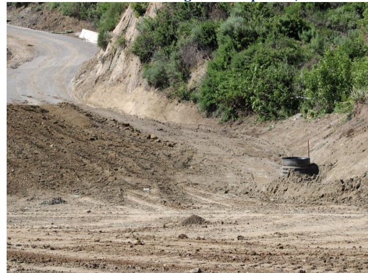
Photo 392: Road Realignment: April 16, 2024
