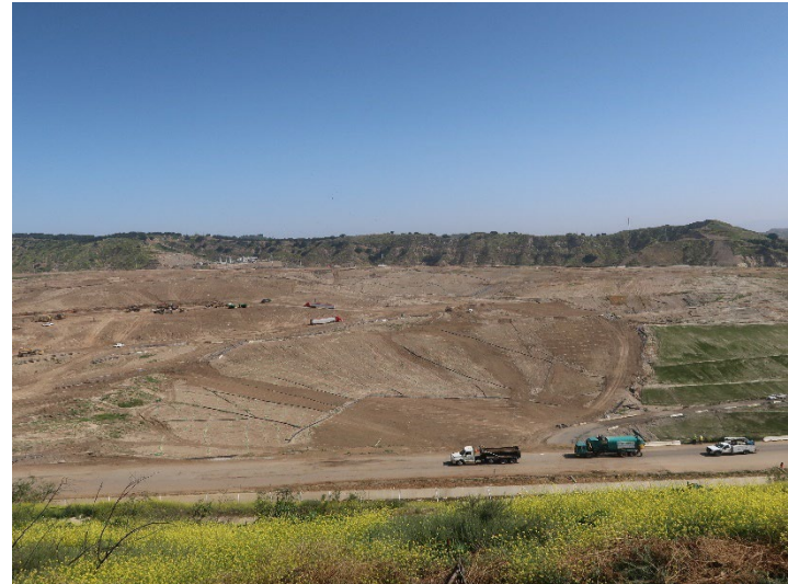
Photo 26: Working Area, CC4 Part 3: May 21, 2024
