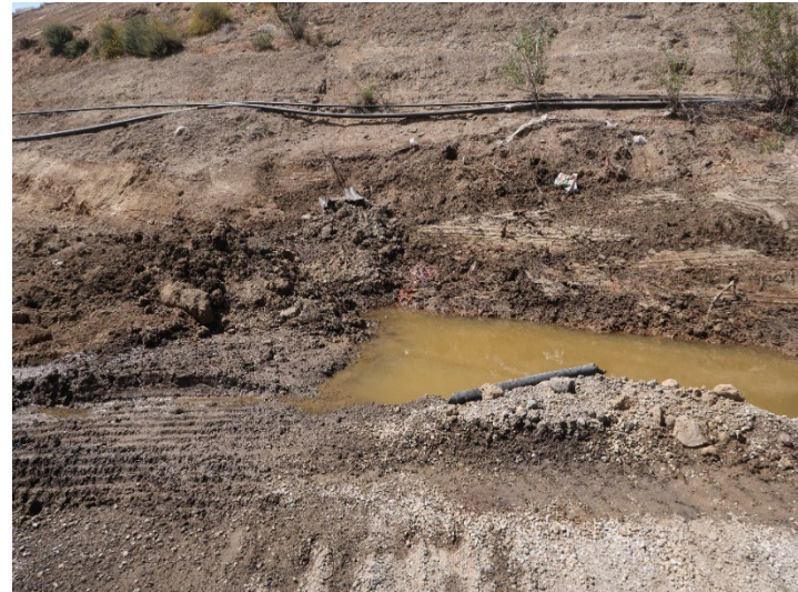
Photo 342: General Site: June 11, 2024
