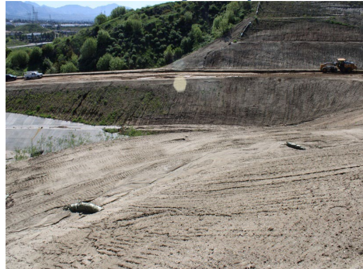
Photo 380: Road Realignment: April 16, 2024
