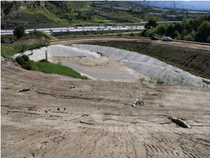
Photo 379: Road Realignment: April 16, 2024
