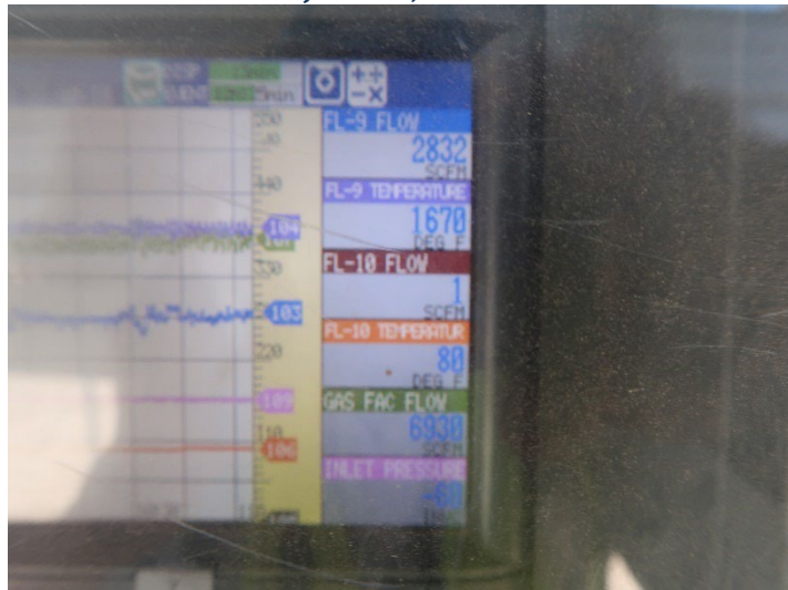
Photo 107: Flares 9, 10, 11 and Gas-to-Energy Facility: June 11, 2024
