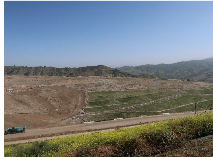
Photo 70: Closure Turf: May 21, 2024
