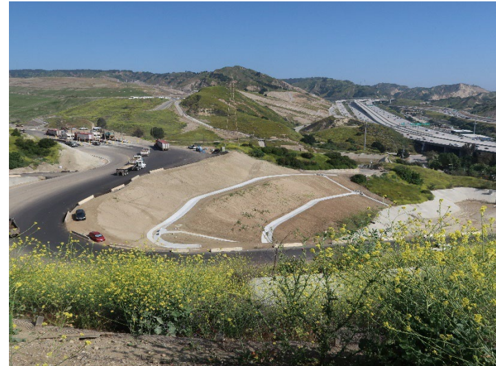
Photo 414: Road Realignment: May 21, 2024
