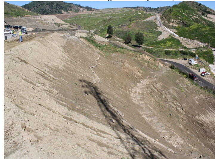
Photo 396: Road Realignment: April 16, 2024
