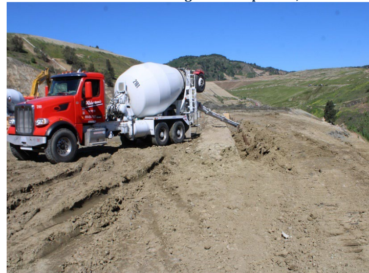
Photo 412: Road Realignment: April 16, 2024
