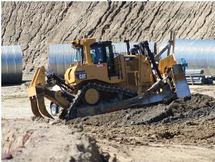
Photo 391: Road Realignment: April 16, 2024
