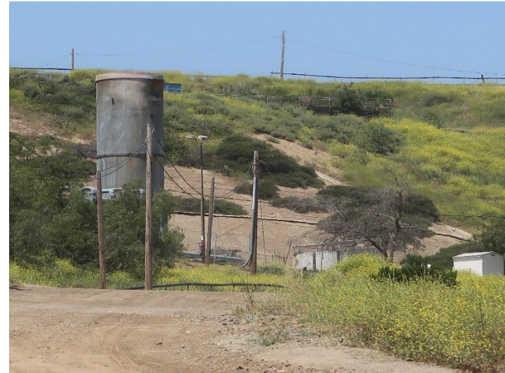
Photo 338: General Site: May 21, 2024
