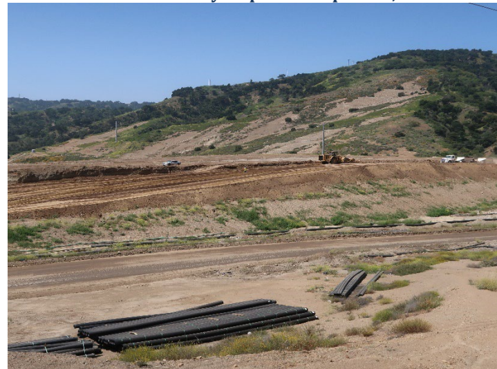
Photo 112: County Top Deck: May 21, 2024
