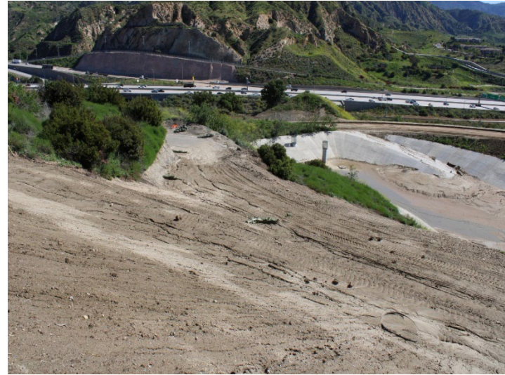
Photo 378: Road Realignment: April 16, 2024
