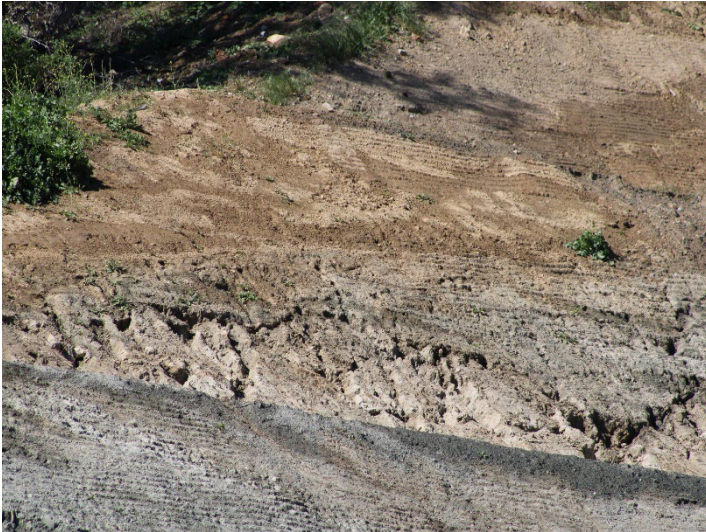
Photo 405: Road Realignment: April 16, 2024
