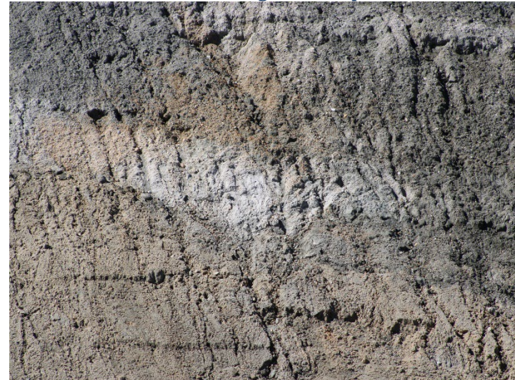
Photo 400: Road Realignment: April 16, 2024
