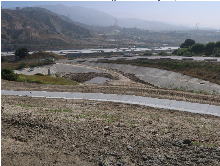
Photo 427: Road Realignment: June 11, 2024
