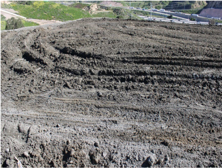
Photo 365: Road Realignment: April 16, 2024
