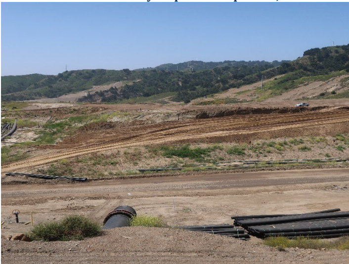
Photo 111: County Top Deck: May 21, 2024
