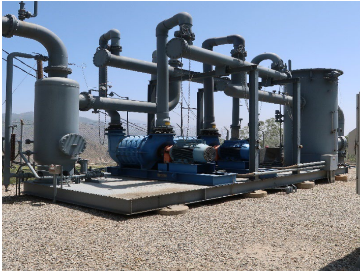
Photo 333: General Site: May 21, 2024
