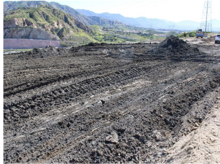
Photo 366: Road Realignment: April 16, 2024
