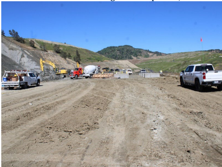
Photo 375: Road Realignment: April 16, 2024
