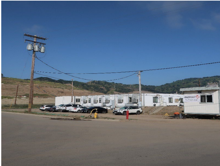
Photo 81: Office and Scales Location: May 21, 2024
