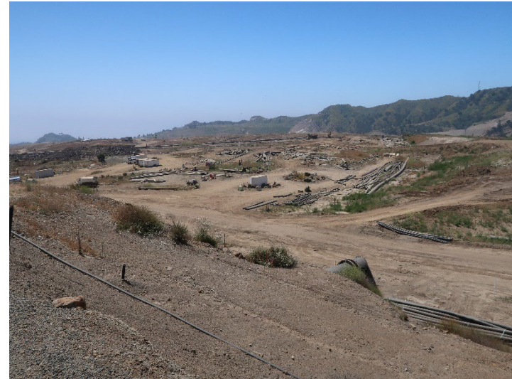
Photo 354: General Site: June 11, 2024
