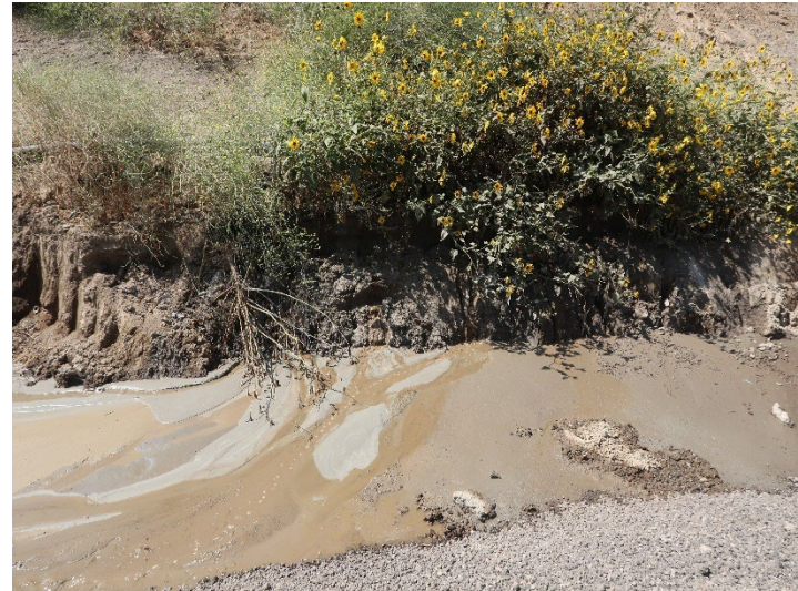
Photo 346: General Site: June 11, 2024
