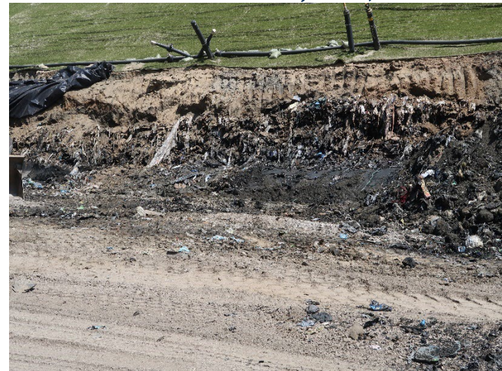
Photo 76: Closure Turf: June 11, 2024
