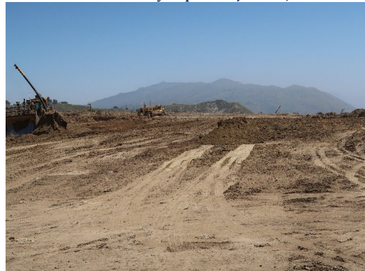
Photo 116: County Top Deck: June 11, 2024
