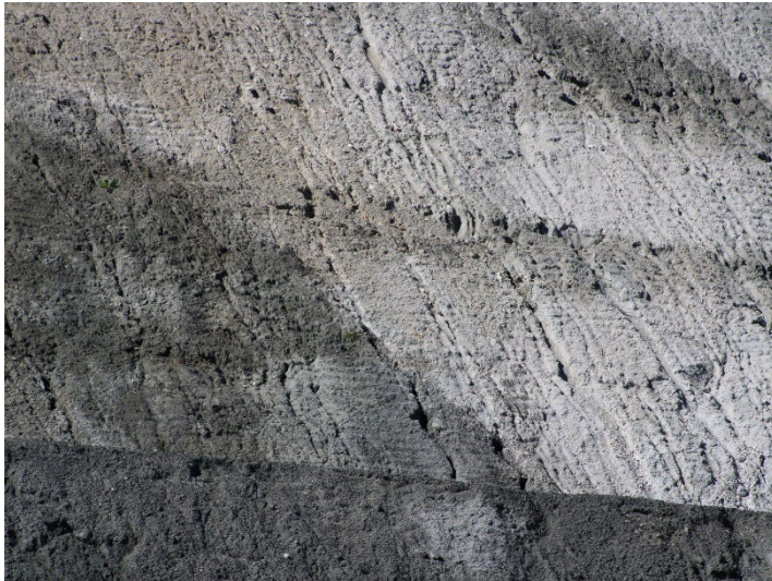
Photo 401: Road Realignment: April 16, 2024
