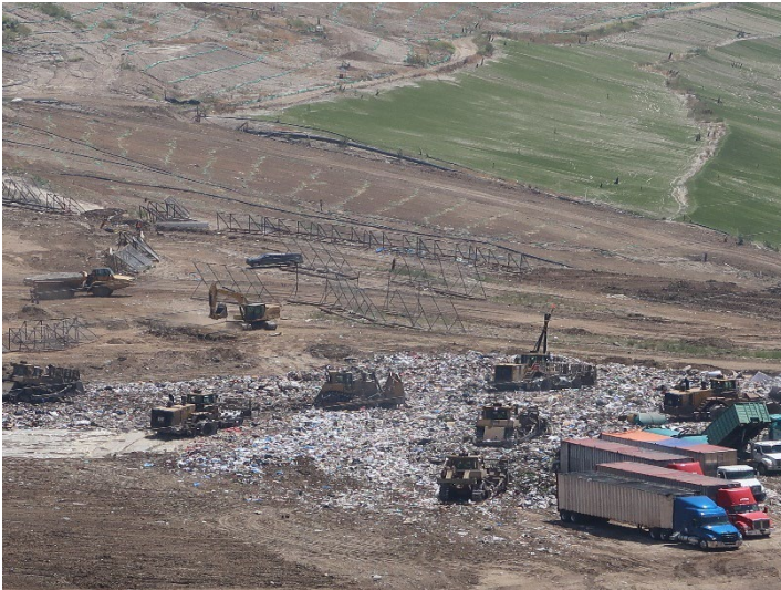
Photo 33: Working Area, CC4 Part 3: May 21, 2024
