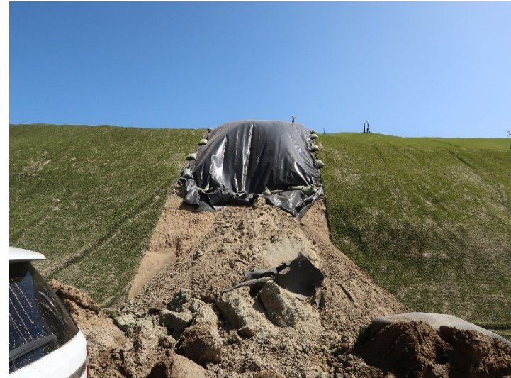
Photo 74: Closure Turf: June 11, 2024
