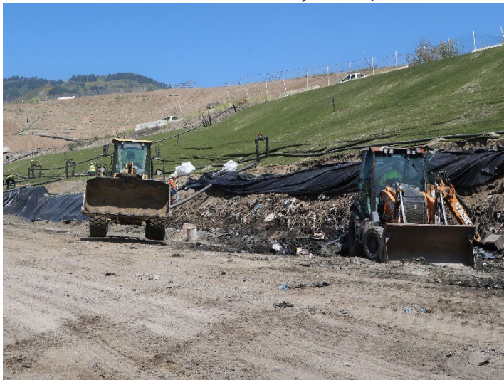
Photo 75: Closure Turf: June 11, 2024
