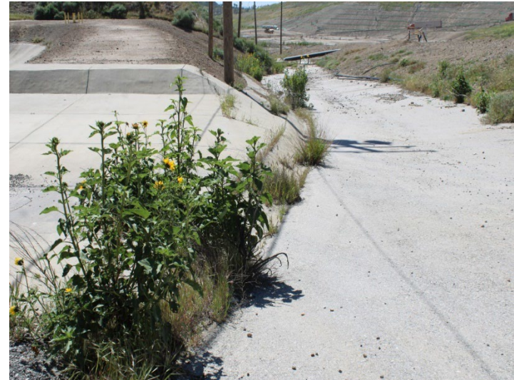
Photo 134: Eastside Drainage Channel: April 16, 2024
