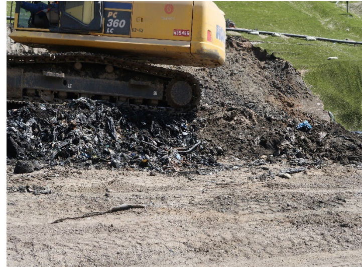
Photo 78: Closure Turf: June 11, 2024
