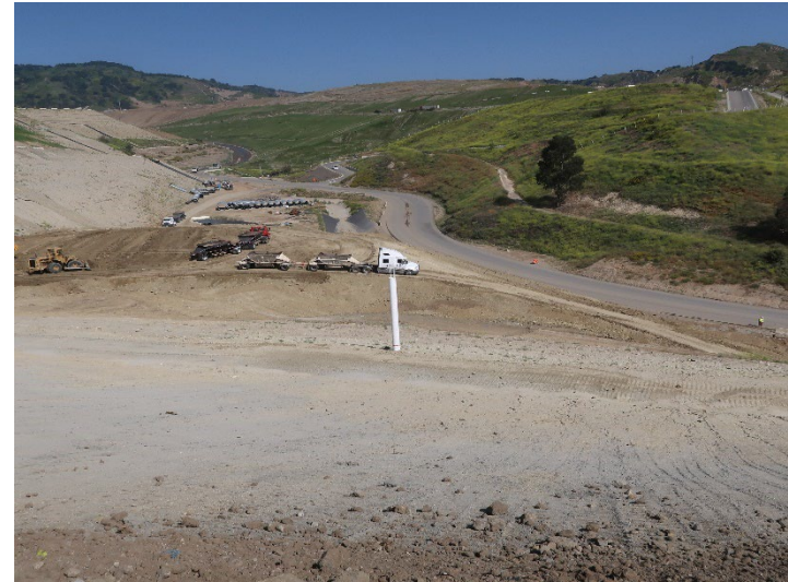
Photo 418: Road Realignment: May 21, 2024
