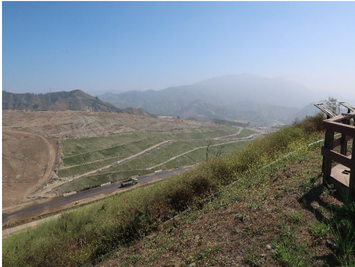
Photo 73: Closure Turf: June 11, 2024
