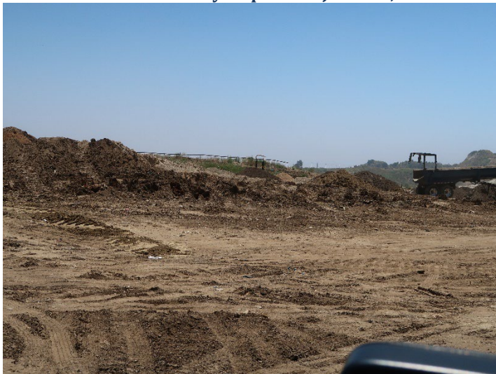
Photo 119: County Top Deck: June 11, 2024
