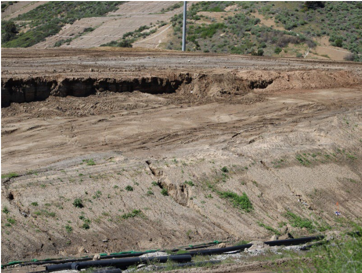
Photo 109: County Top Deck: April 16, 2024
