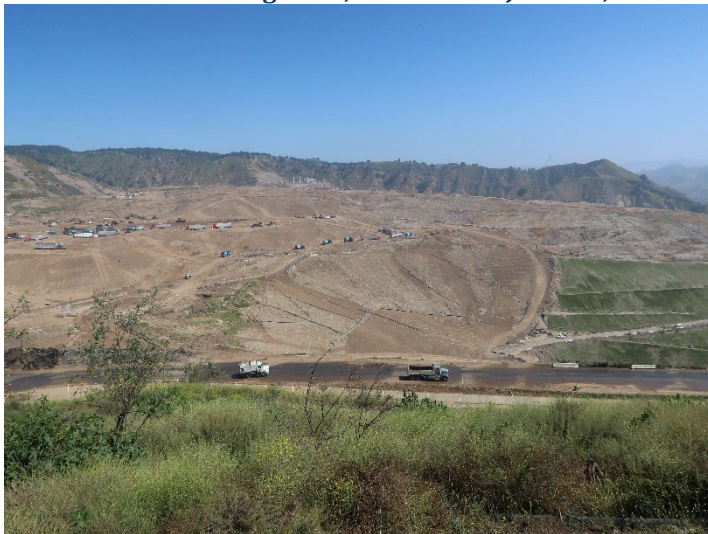
Photo 39: Working Area, CC4 Part 3: June 11, 2024
