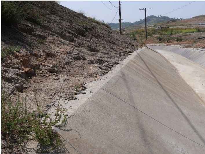
Photo 141: Eastside Drainage Channel: May 21, 2024
