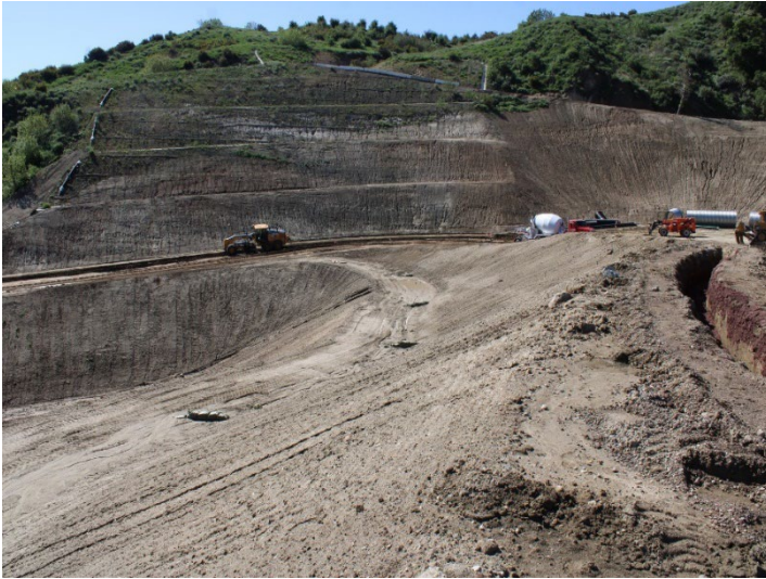
Photo 381: Road Realignment: April 16, 2024
