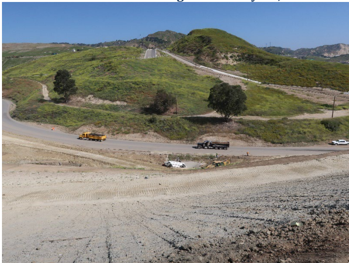
Photo 423: Road Realignment: May 21, 2024
