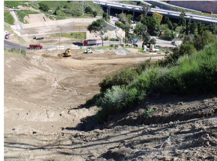
Photo 398: Road Realignment: April 16, 2024
