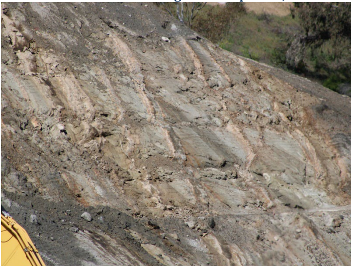
Photo 411: Road Realignment: April 16, 2024
