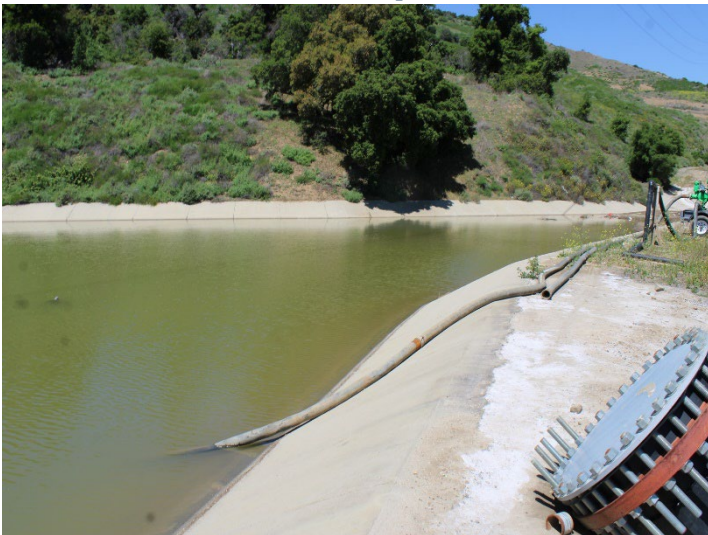
Photo 3: Basin A: April 16, 2024
