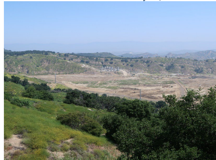
Photo 328: General Site: May 21, 2024
