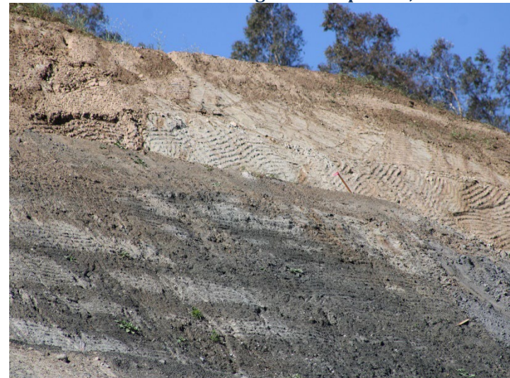
Photo 404: Road Realignment: April 16, 2024
