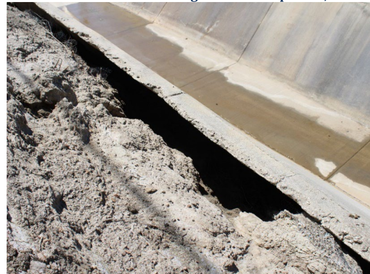
Photo 136: Eastside Drainage Channel: April 16, 2024
