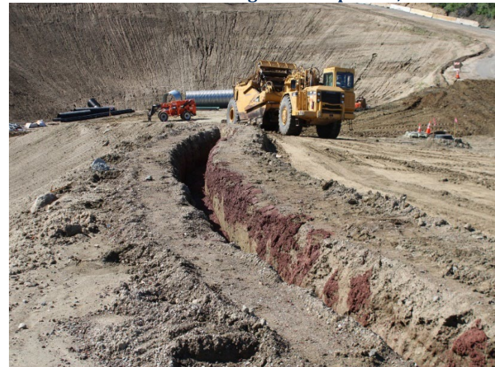
Photo 376: Road Realignment: April 16, 2024
