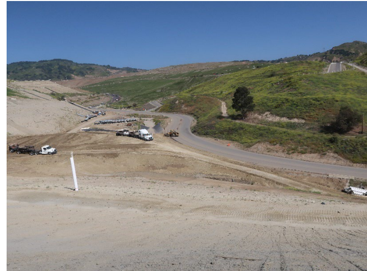
Photo 422: Road Realignment: May 21, 2024
