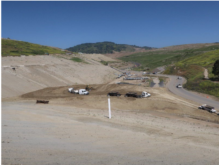
Photo 425: Road Realignment: May 21, 2024
