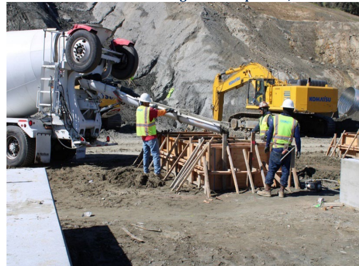
Photo 372: Road Realignment: April 16, 2024
