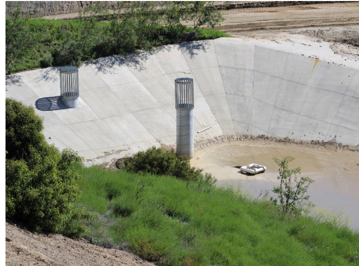
Photo 386: Road Realignment: April 16, 2024
