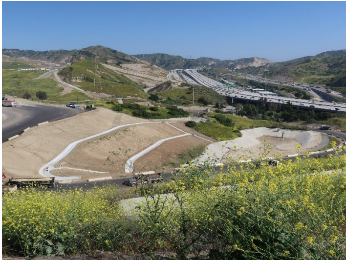
Photo 413: Road Realignment: May 21, 2024
