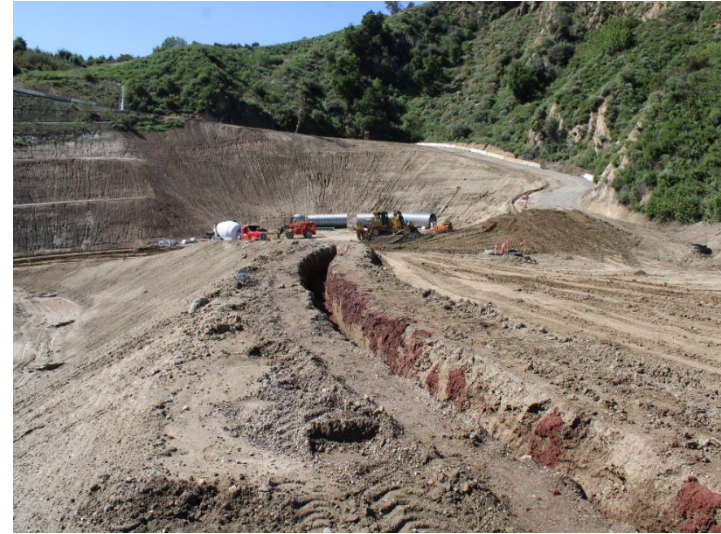
Photo 382: Road Realignment: April 16, 2024
