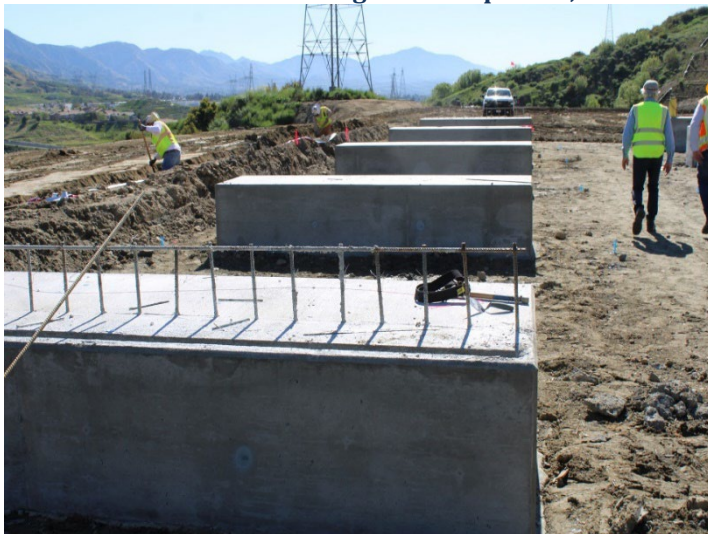
Photo 371: Road Realignment: April 16, 2024
