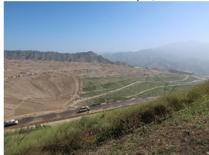
Photo 72: Closure Turf: June 11, 2024
