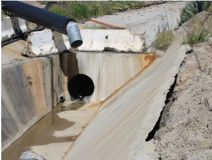
Photo 139: Eastside Drainage Channel: April 16, 2024
