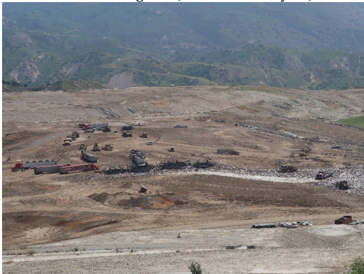
Photo 27: Working Area, CC4 Part 3: May 21, 2024
