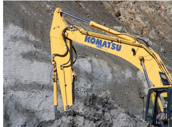
Photo 410: Road Realignment: April 16, 2024
