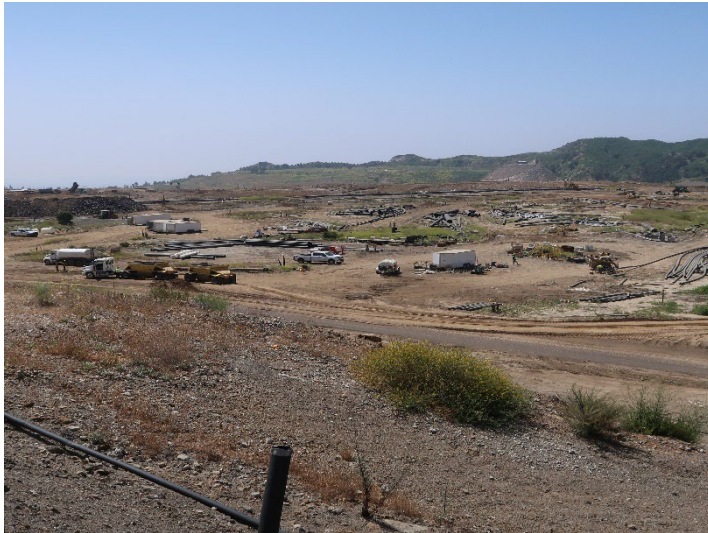
Photo 321: General Site: May 21, 2024
