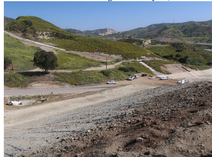
Photo 424: Road Realignment: May 21, 2024
