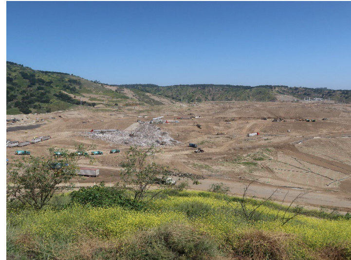
Photo 66: Working Area, CC4 Part 4/5: May 21, 2024
