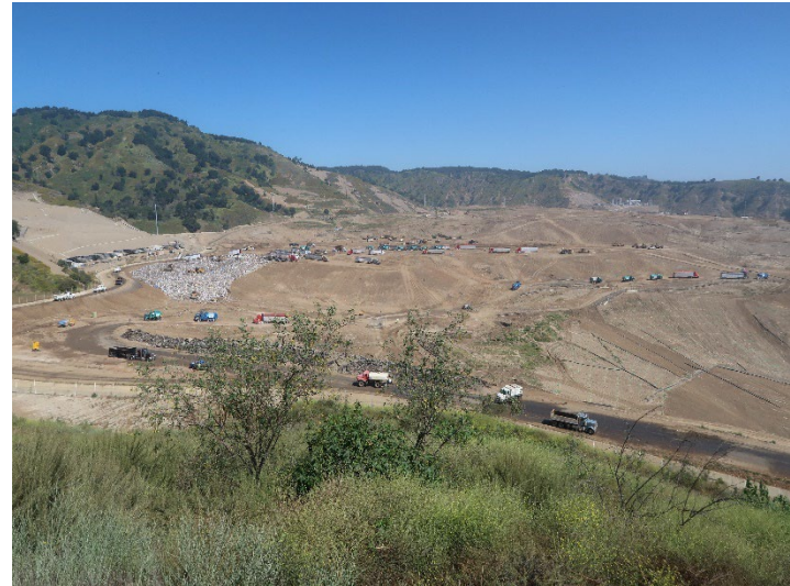
Photo 38: Working Area, CC4 Part 3: June 11, 2024
