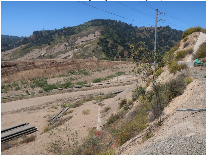
Photo 115: County Top Deck: June 11, 2024
