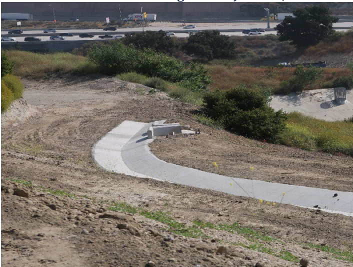
Photo 431: Road Realignment: June 11, 2024
