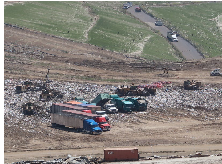
Photo 34: Working Area, CC4 Part 3: May 21, 2024
