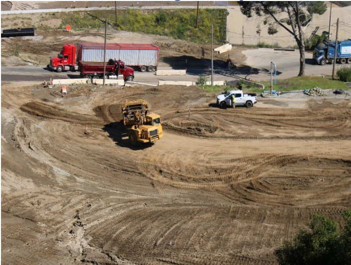
Photo 399: Road Realignment: April 16, 2024
