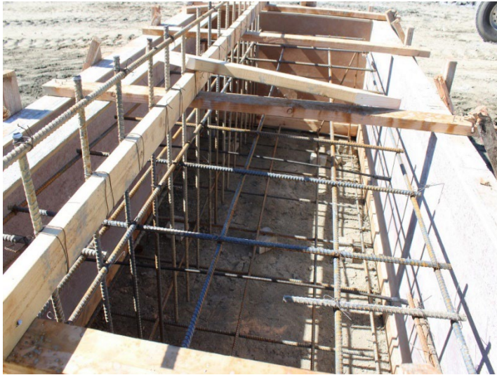
Photo 373: Road Realignment: April 16, 2024
