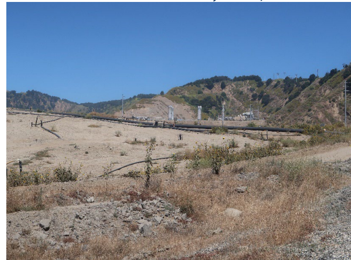
Photo 352: General Site: June 11, 2024
