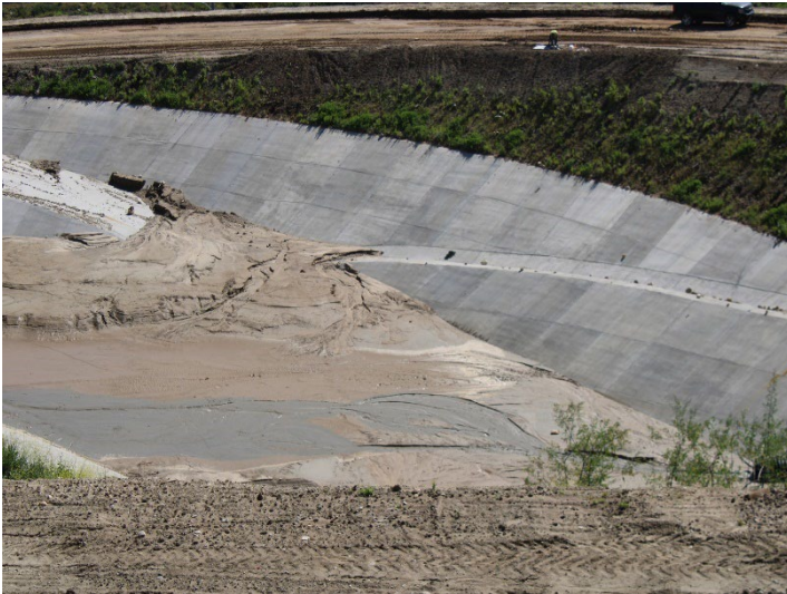
Photo 385: Road Realignment: April 16, 2024
