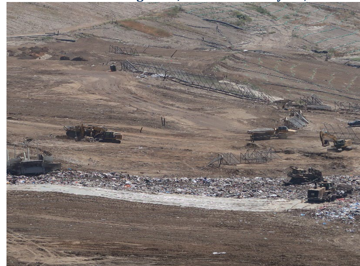
Photo 32: Working Area, CC4 Part 3: May 21, 2024
