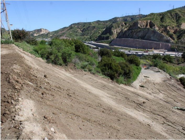
Photo 377: Road Realignment: April 16, 2024
