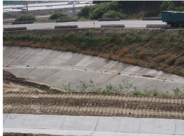
Photo 434: Road Realignment: June 11, 2024
