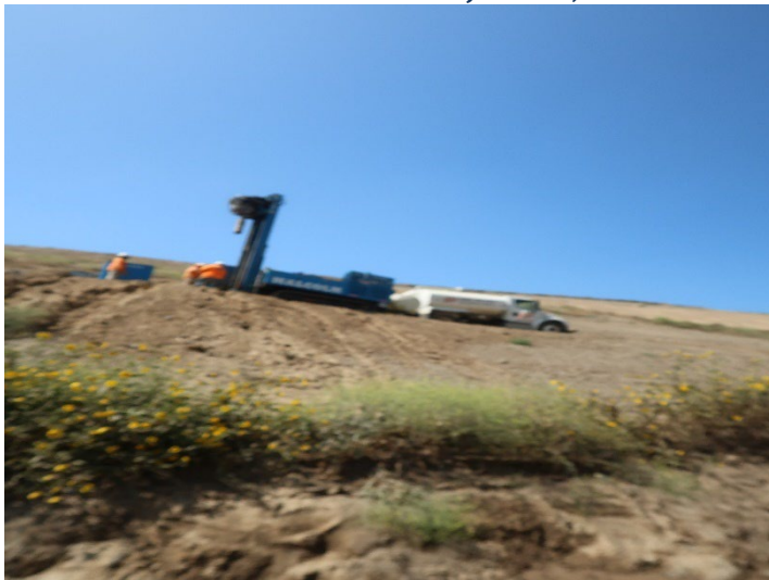
Photo 347: General Site: June 11, 2024
