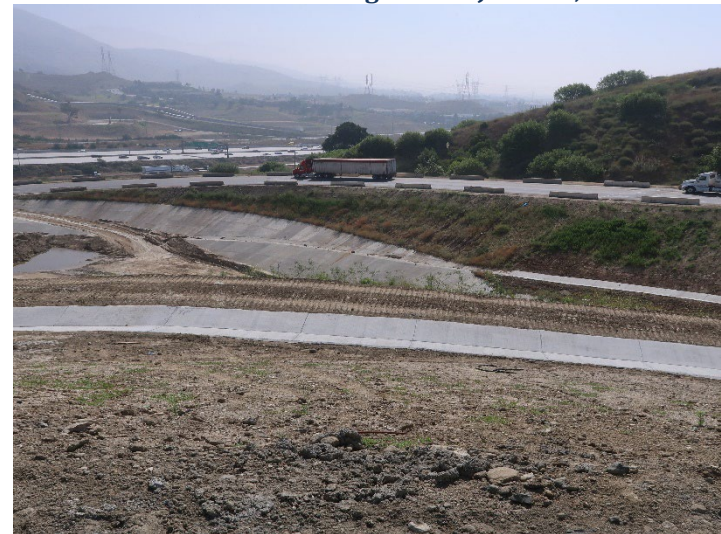
Photo 428: Road Realignment: June 11, 2024
