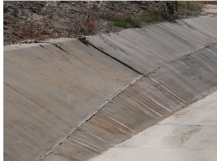
Photo 142: Eastside Drainage Channel: May 21, 2024
