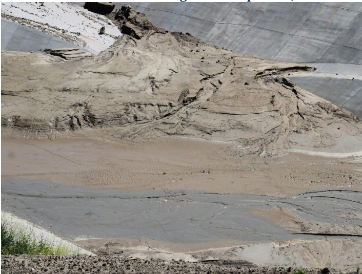
Photo 387: Road Realignment: April 16, 2024
