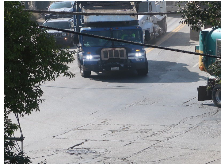
Photo 340: General Site: June 11, 2024
