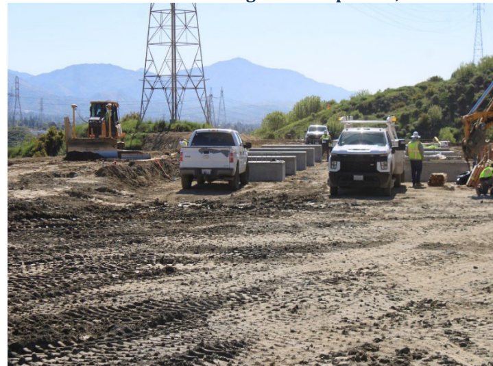
Photo 368: Road Realignment: April 16, 2024
