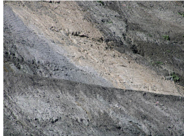
Photo 402: Road Realignment: April 16, 2024
