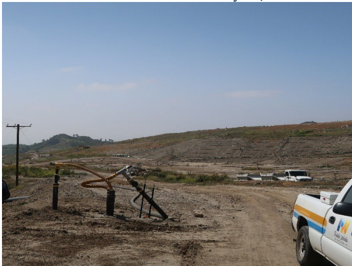
Photo 311: General Site: May 21, 2024
