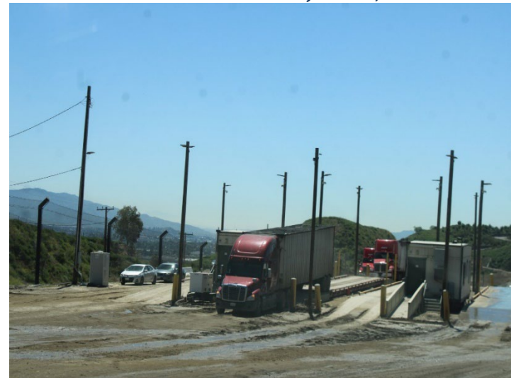
Photo 80: Office and Scales Location: April 16, 2024
