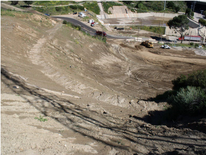
Photo 397: Road Realignment: April 16, 2024
