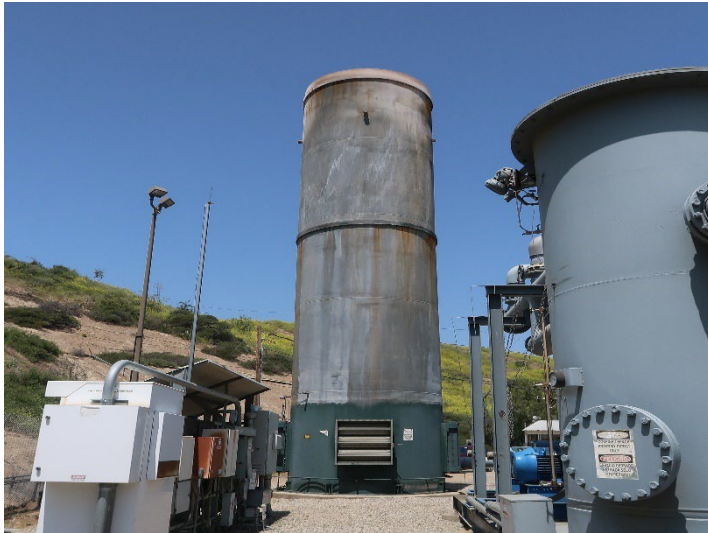
Photo 337: General Site: May 21, 2024
