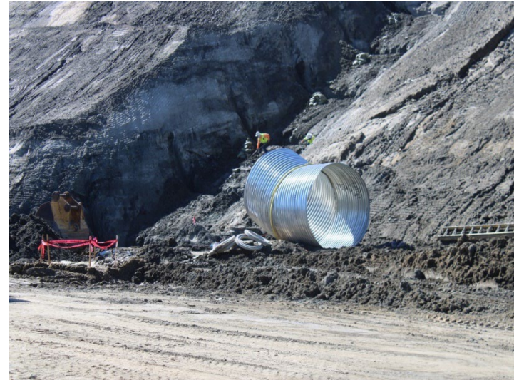
Photo 370: Road Realignment: April 16, 2024
