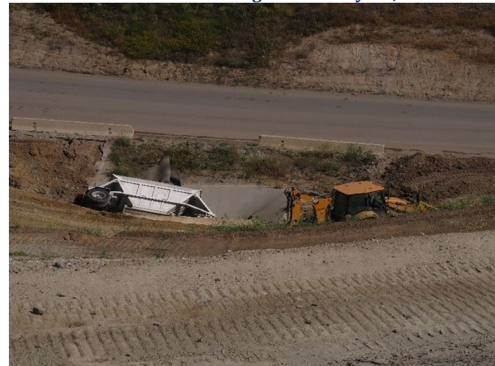
Photo 420: Road Realignment: May 21, 2024
