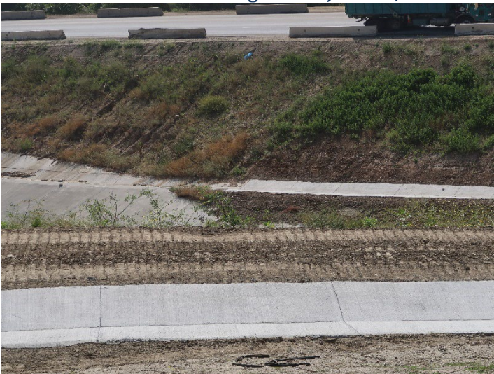
Photo 435: Road Realignment: June 11, 2024
