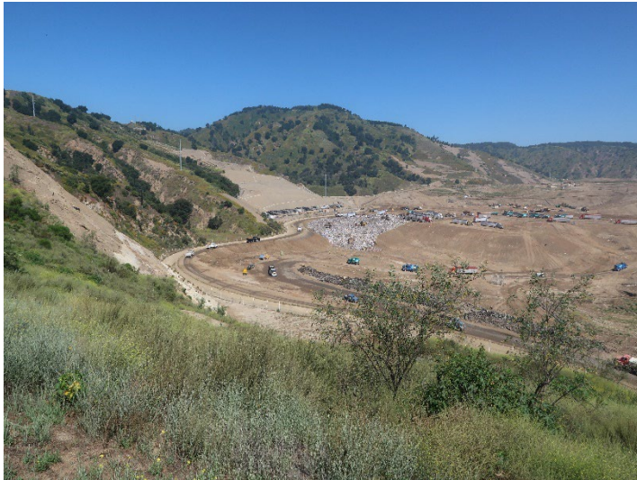
Photo 37: Working Area, CC4 Part 3: June 11, 2024
