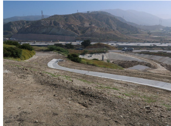
Photo 426: Road Realignment: June 11, 2024
