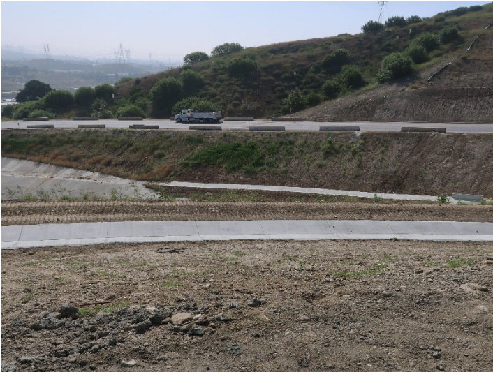
Photo 429: Road Realignment: June 11, 2024
