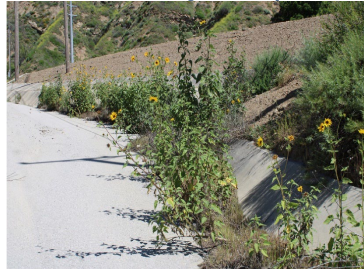
Photo 140: Eastside Drainage Channel: April 16, 2024
