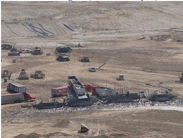
Photo 31: Working Area, CC4 Part 3: May 21, 2024
