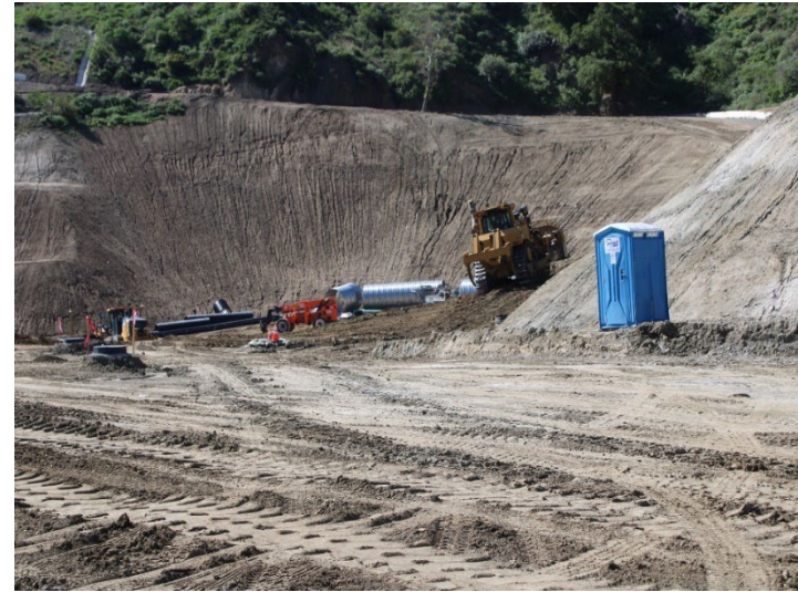
Photo 374: Road Realignment: April 16, 2024
