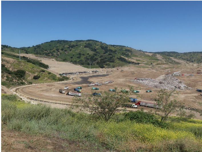
Photo 65: Working Area, CC4 Part 4/5: May 21, 2024
