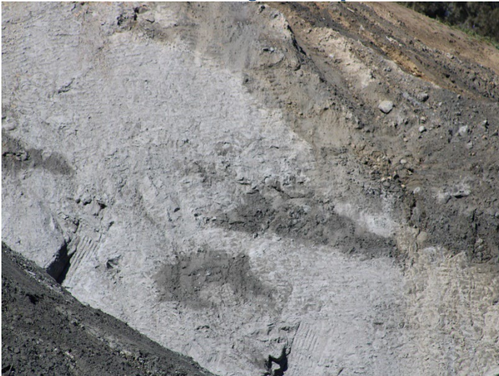
Photo 407: Road Realignment: April 16, 2024
