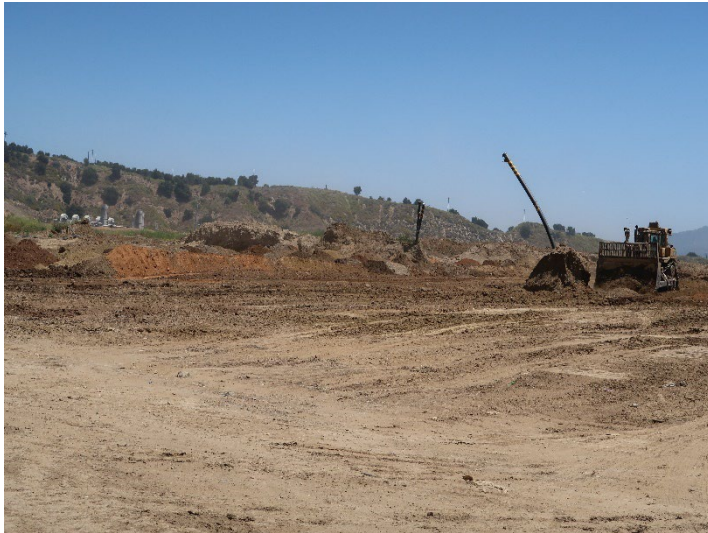
Photo 117: County Top Deck: June 11, 2024
