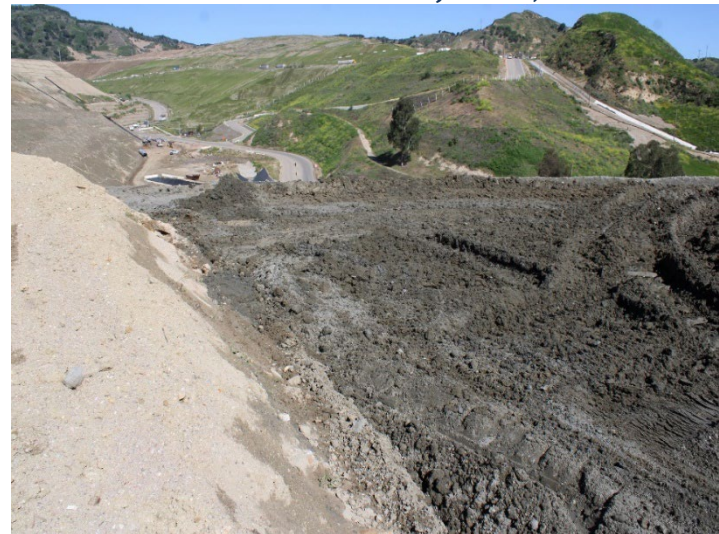
Photo 364: Road Realignment: April 16, 2024
