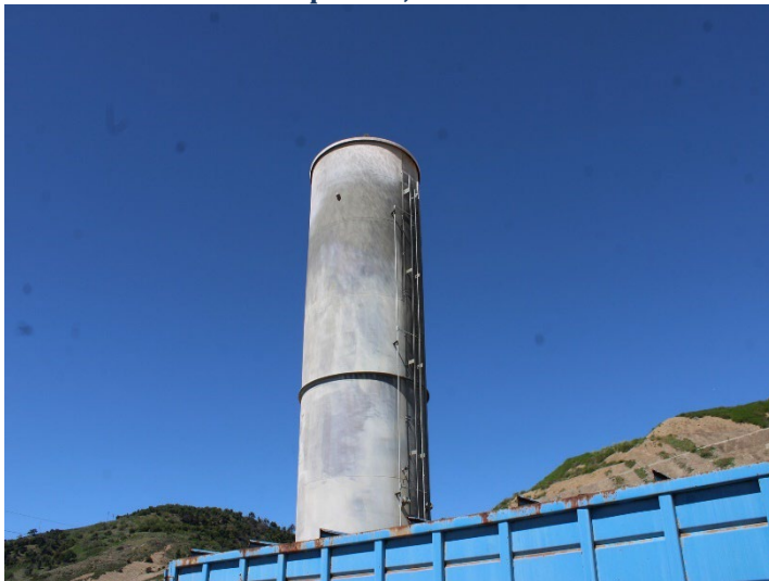
Photo 91: Flares 9, 10, 11 and Gas-to-Energy Facility: April 16, 2024
