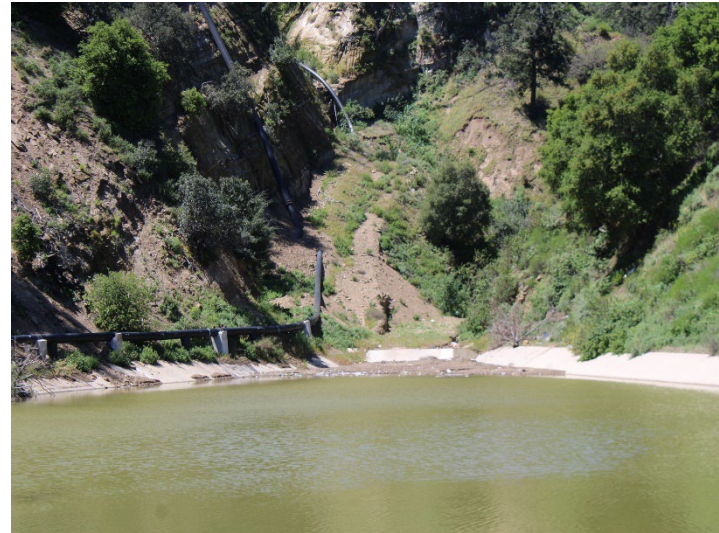
Photo 6: Basin A: April 16, 2024
