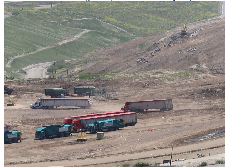
Photo 36: Working Area, CC4 Part 3: May 21, 2024
