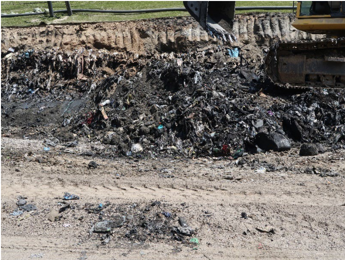
Photo 77: Closure Turf: June 11, 2024
