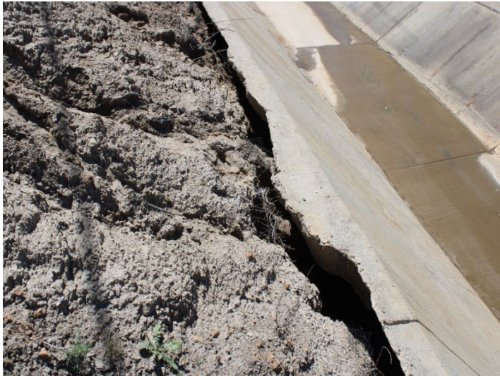
Photo 137: Eastside Drainage Channel: April 16, 2024
