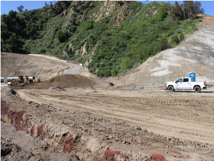
Photo 383: Road Realignment: April 16, 2024
