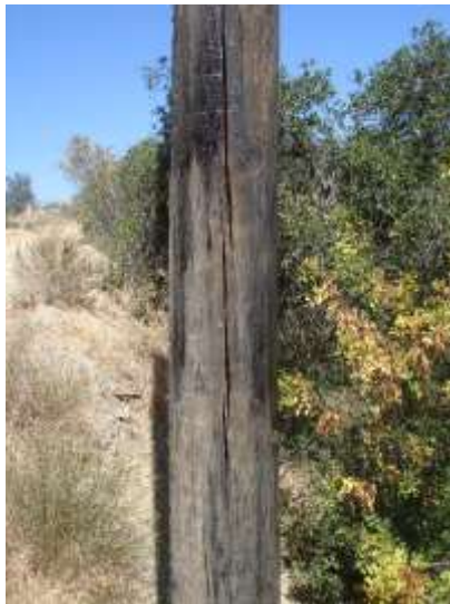
Photo 479: Edison Splitting Pole: June 24, 2015
