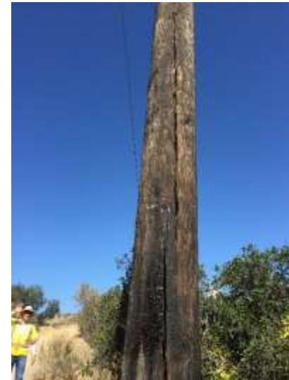
Photo 478: Edison Splitting Pole: June 24, 2015
