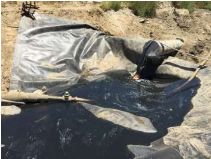
Photo 461: Condensate Collection Pipe Temporary Basin: June 24, 2015
