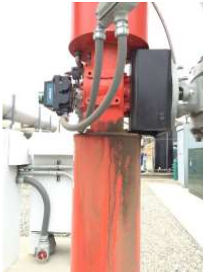
Photo 143: Gas to Energy Gas Shutoff Valve: April 23, 2015
