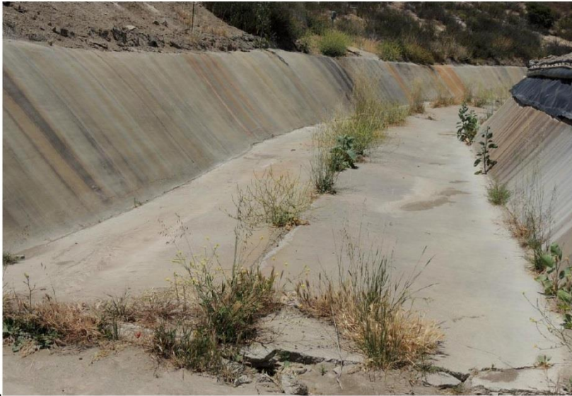
Photo 5: Uplifted bottom slab of drainage channel
