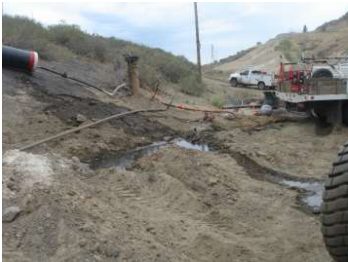
Photo 451: Gas Condensate Sump Replacement & Piping: June 9, 2015
