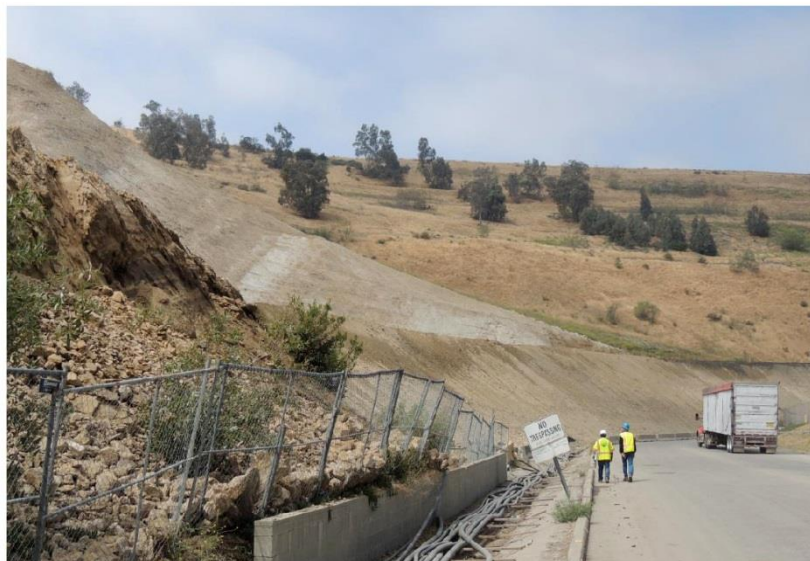
Photo 8: Soil loading block wall
