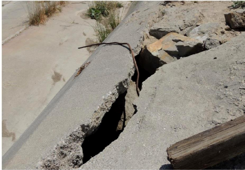
Photo 7: Broken Connection between downchute and drainage channel
