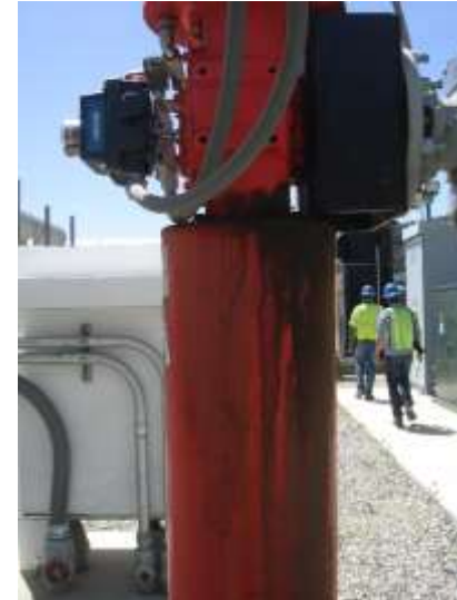
Photo 142: Gas to Energy Gas Shutoff Valve: April 9, 2015
