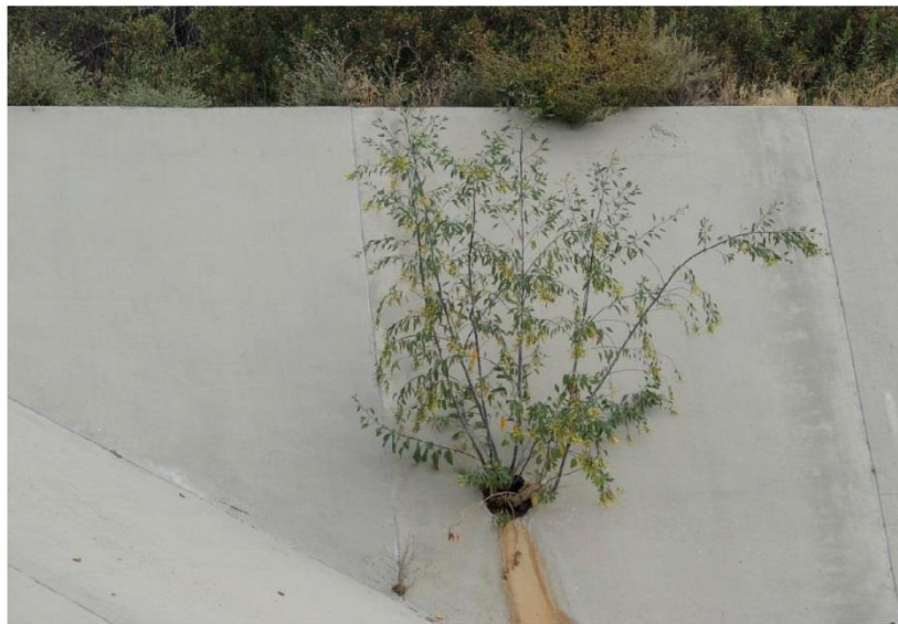
Photo 4: Bush growing in drain pier at terminal basin
