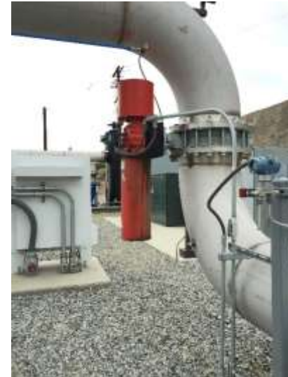
Photo 144: Gas to Energy Gas Shutoff Valve: June 9, 2015
