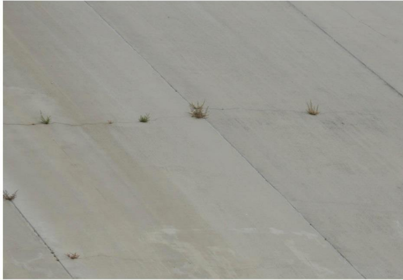
Photo 3: Vegetation growing through cracks of shotcrete face
