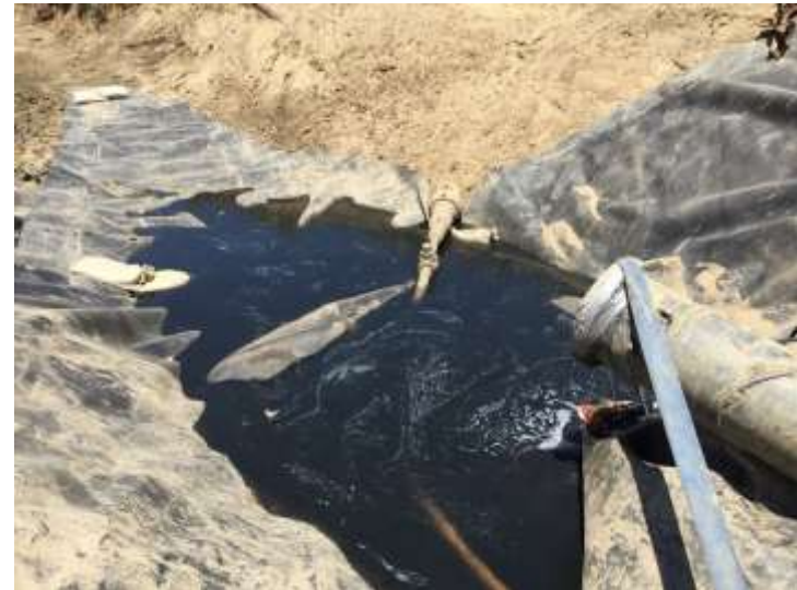
Photo 460: Condensate Collection Pipe Temporary Basin: June 24, 2015
