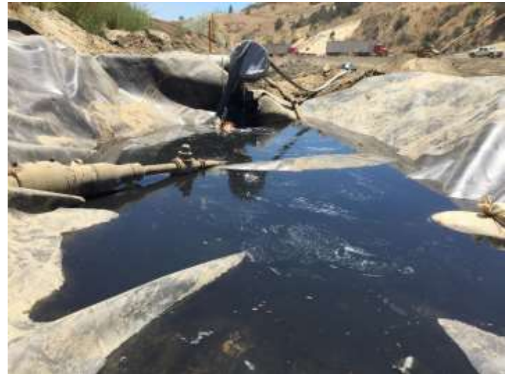
Photo 462: Condensate Collection Pipe Temporary Basin: June 24, 2015
