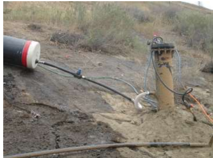
Photo 452: Gas Condensate Sump Replacement & Piping: June 9, 2015
