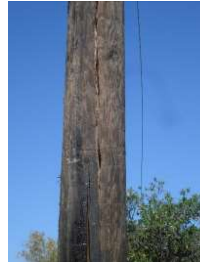
Photo 480: Edison Splitting Pole: June 24, 2015
