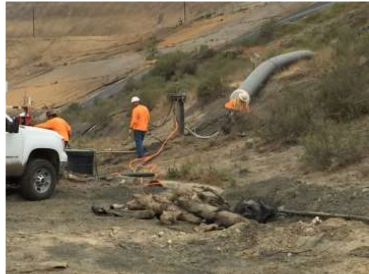
Photo 450: Gas Condensate Sump Replacement & Piping: June 9, 2015
